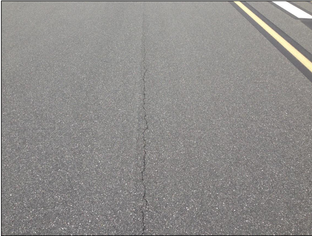
Runway 03-21, Section 6205, Sample Unit 301 – Low Severity (48) Longitudinal and Transverse Cracking
