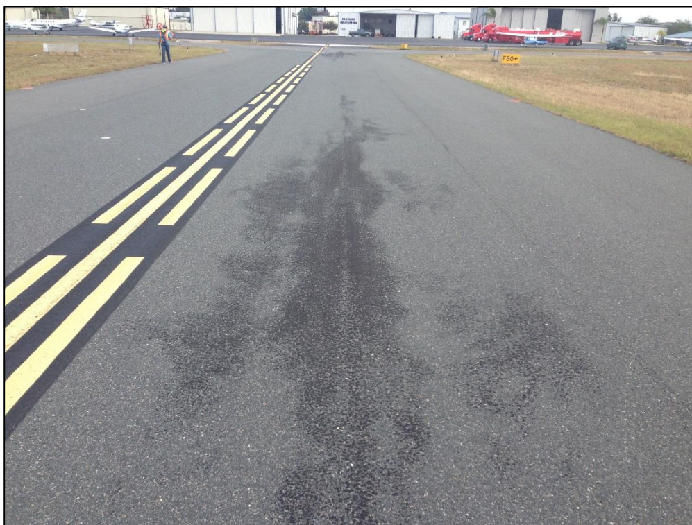
Taxiway Delta, Section 400, Sample Unit 252 – (42) Bleeding, Low Severity (57) Weathering
