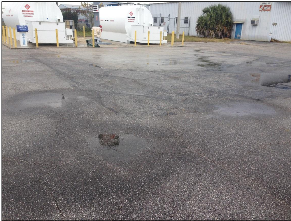
Re-Fueling Apron, Section 4210, Sample Unit 301 – Low Severity (43) Block Cracking, Low Severity (45) Depression, Low Severity (50) Patching, Low Severity (52) Raveling
