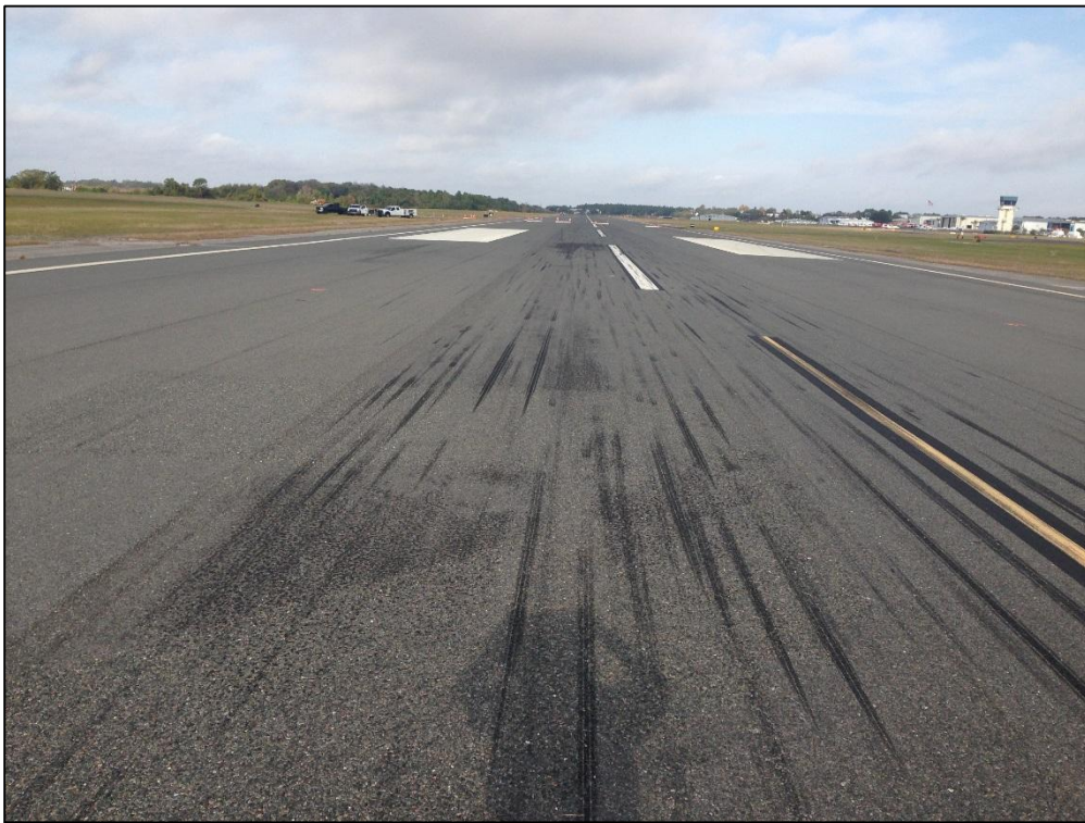
Runway 13-31, Section 6105, Sample Unit 312 – (42) Bleeding, Low Severity (52) Raveling, Medium Severity (52) Raveling
