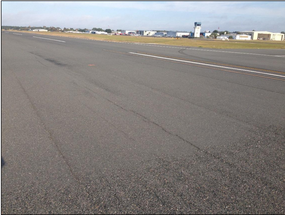
Runway 13-31, Section 6110, Sample Unit 120 – (42) Bleeding, Low Severity (48) Longitudinal and Transverse Cracking, Medium Severity (52) Raveling
