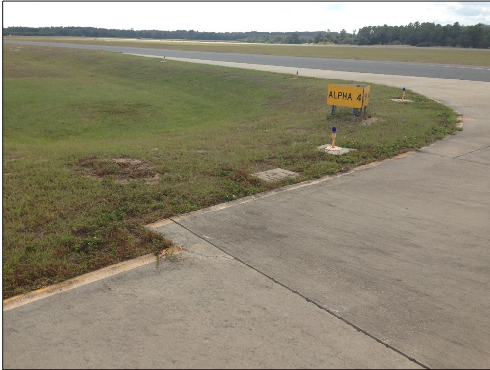
Apron North, Section 4130, Sample Unit 101 – Low Severity (62) Corner Break
