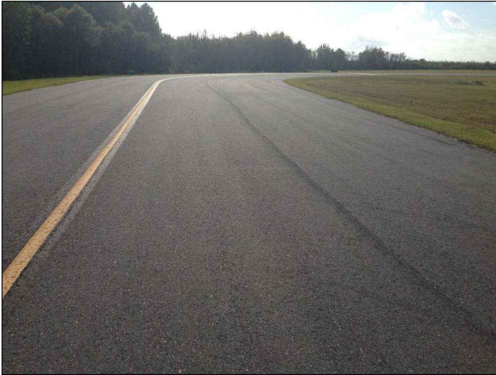
Taxiway Alpha, Section 100, Sample Unit 255 – Low Severity (57) Weathering
