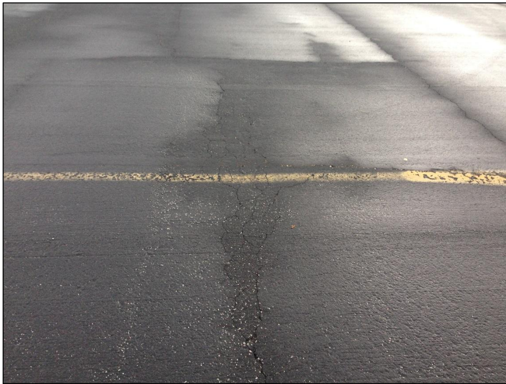
Apron North, Section 4105, Sample Unit 158 – Low Severity (41) Alligator Cracking, Medium Severity (41) Alligator Cracking
