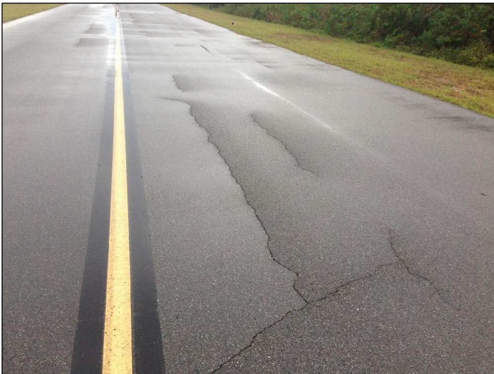
Taxiway Kilo, Section 700, Sample Unit 111 – Low Severity (48) Longitudinal and Transverse Cracking, Low Severity (57) Weathering
