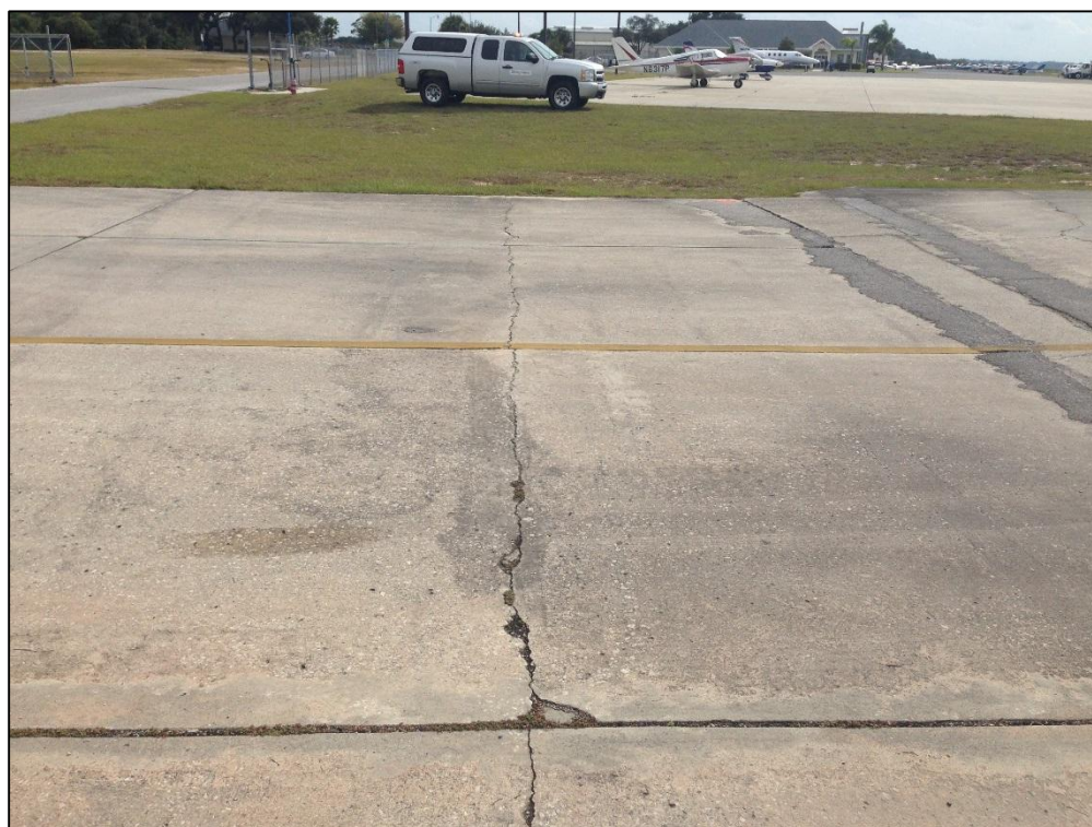
Apron North, Section 4135, Sample Unit 604 – Low Severity (63) Longitudinal, Transverse, and Diagonal Cracking, Low Severity (65) Joint Seal Damage, Low Severity (74) Joint Spalling,
