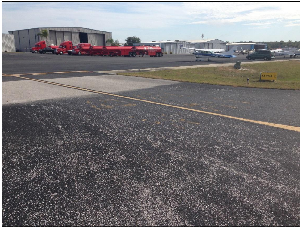
Taxiway A2, Section 130, Sample Unit 501 – Low Severity (48) Longitudinal and Transverse Cracking, Low Severity (52) Raveling
