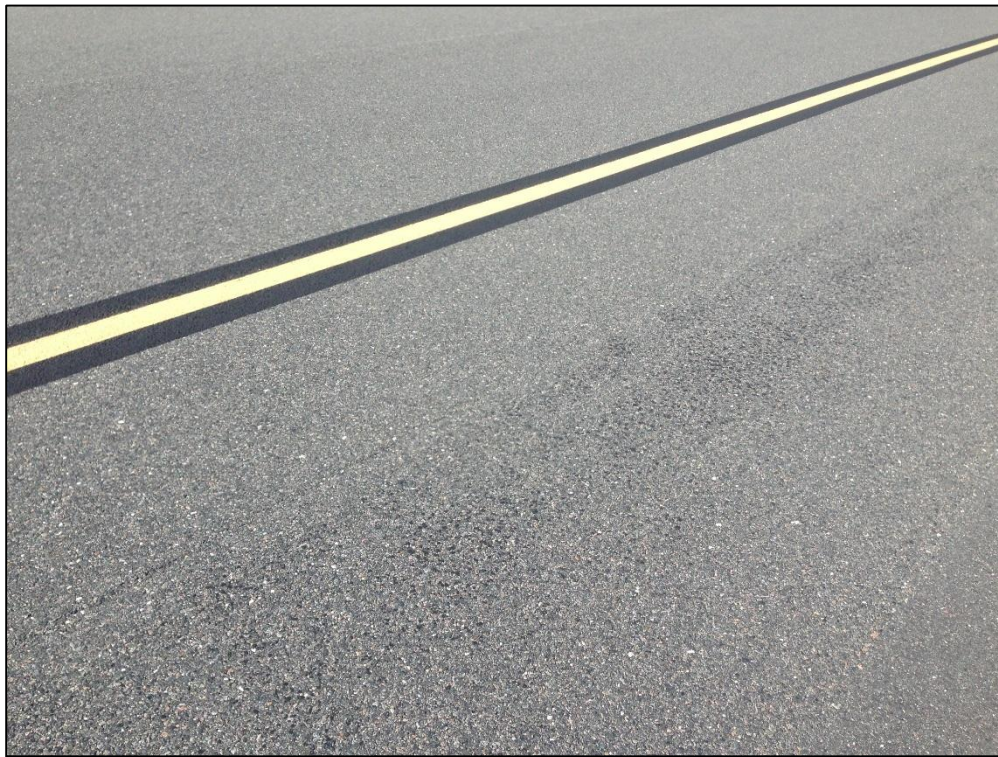
Taxiway Alpha, Section 110, Sample Unit 228 – (42) Bleeding, Low Severity (48) Longitudinal and Transverse Cracking, Low Severity (57) Weathering
