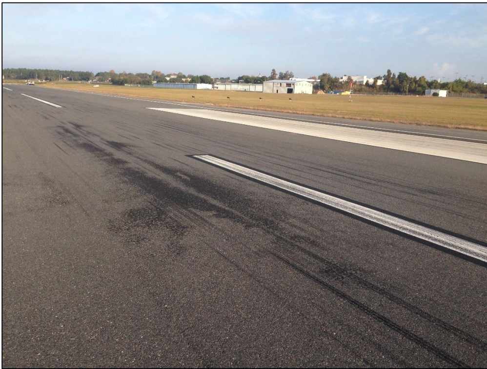
Runway 13-31, Section 6105, Sample Unit 348 – (42) Bleeding, Low Severity (48) Longitudinal and Transverse Cracking, Low Severity (57) Weathering
