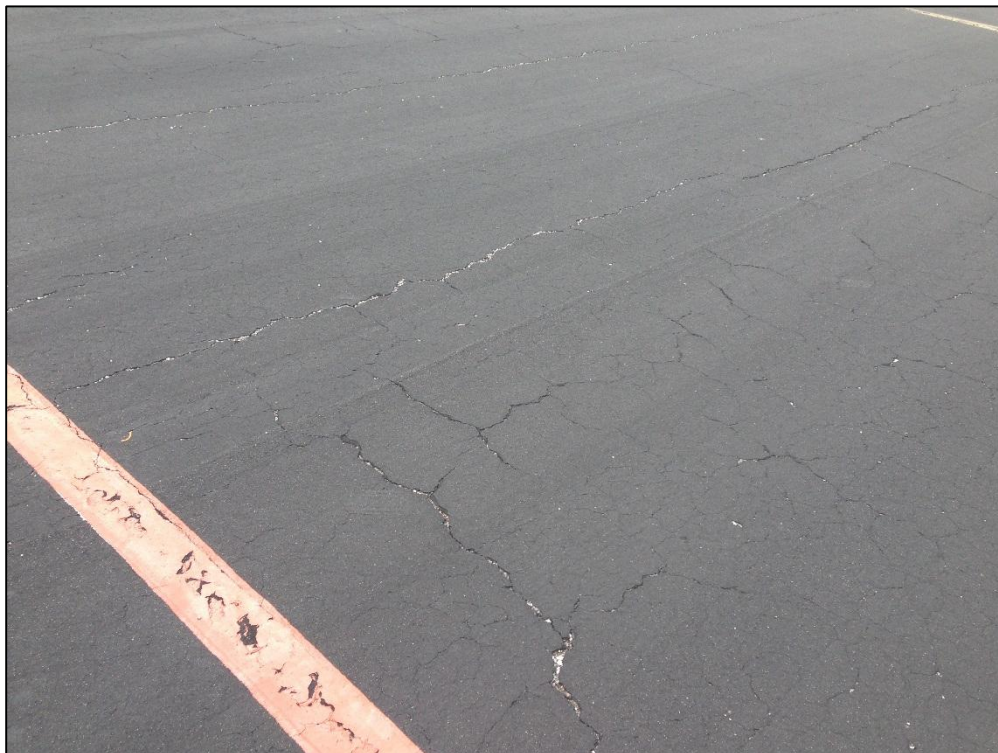
Apron North, Section 4105, Sample Unit 112 – Low Severity (48) Longitudinal and Transverse Cracking, Medium Severity (57) Weathering
