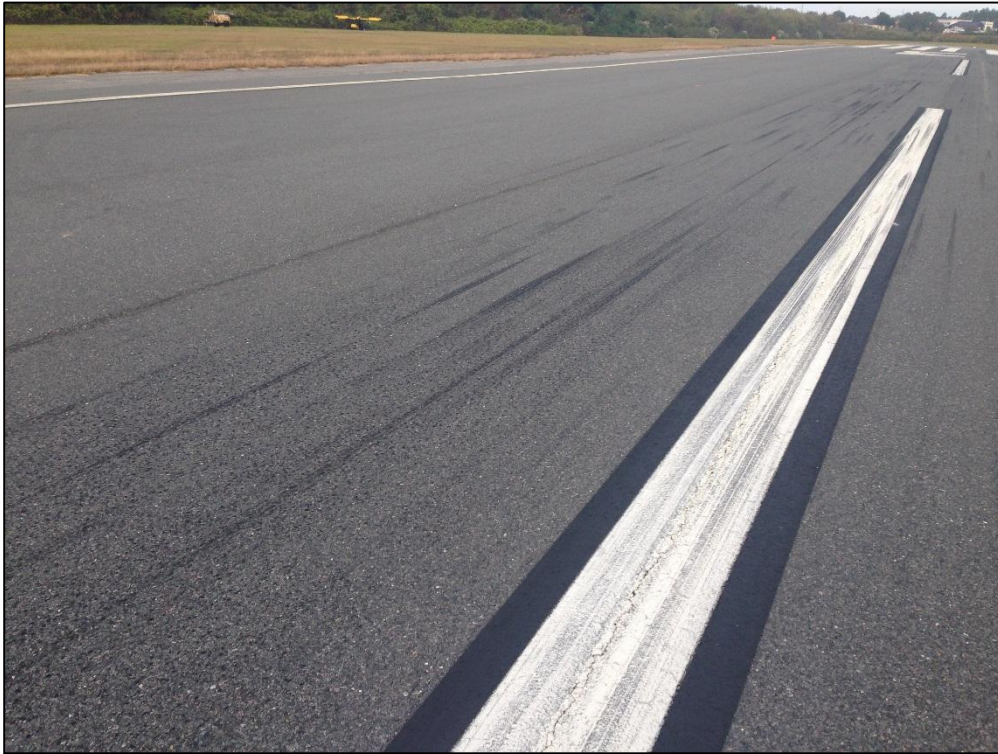
Runway 13-31, Section 6105, Sample Unit 354 – (42) Bleeding, Low Severity (48) Longitudinal and Transverse Cracking, Low Severity (57) Weathering
