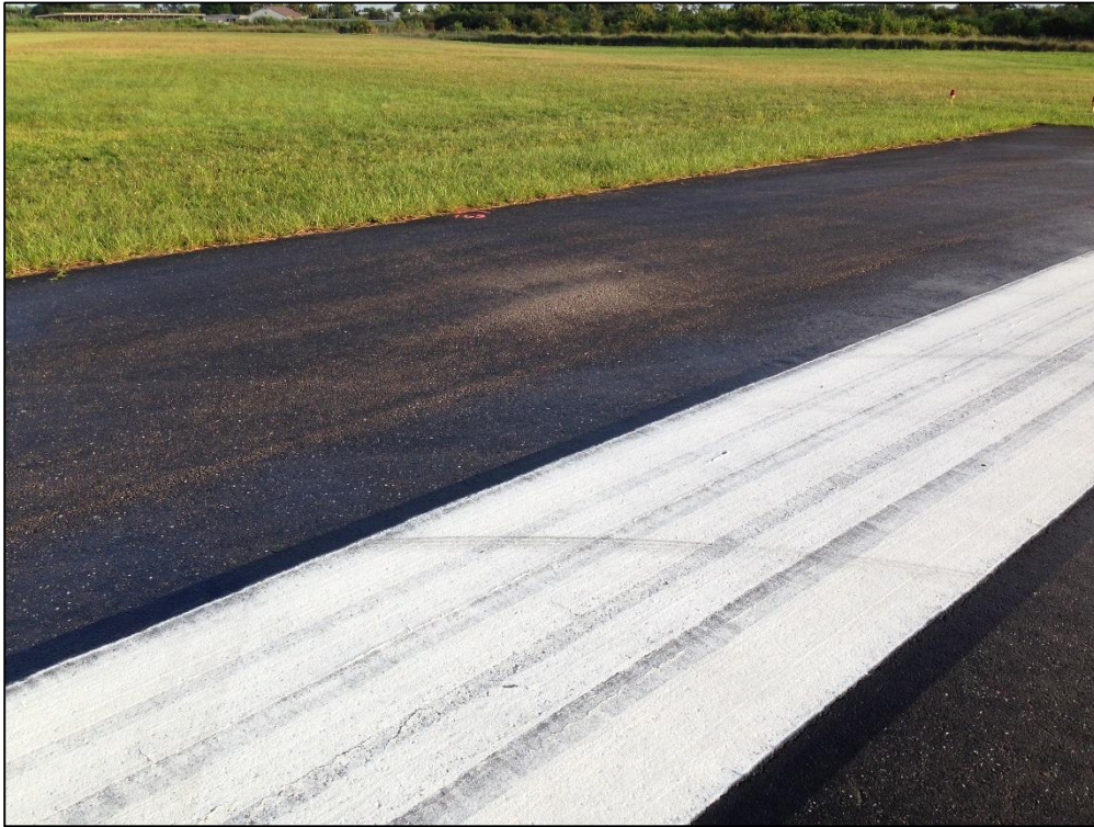
Runway 3-21, Section 6305, Sample Unit 163 – Low Severity (48) Longitudinal and Transverse Cracking, Low Severity (52) Raveling
