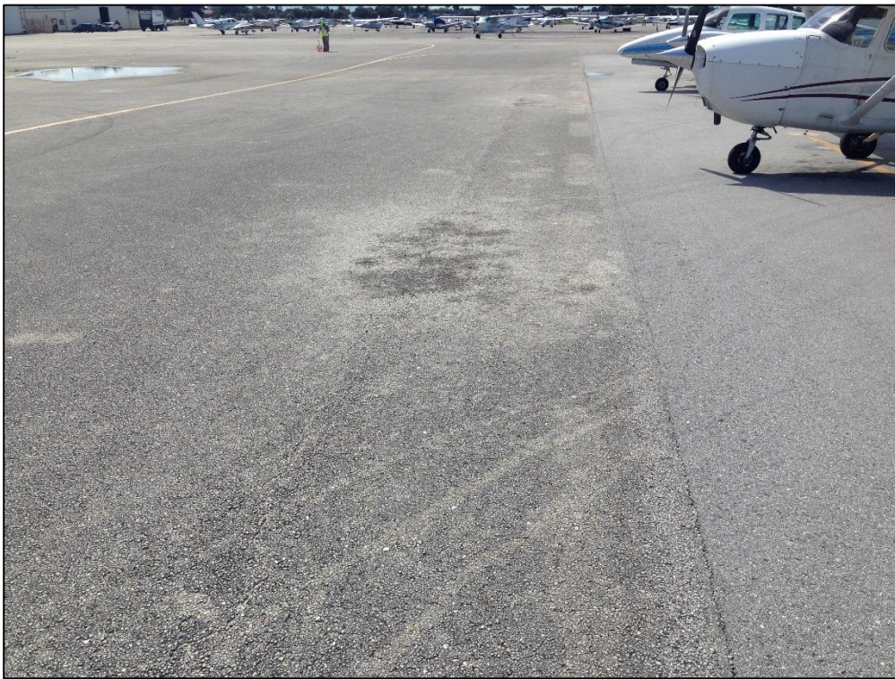
Apron GA, Section 4115, Sample Unit 512 – Low Severity (48) Longitudinal and Transverse Cracking, (49) Oil Spillage, Low Severity (52) Raveling
