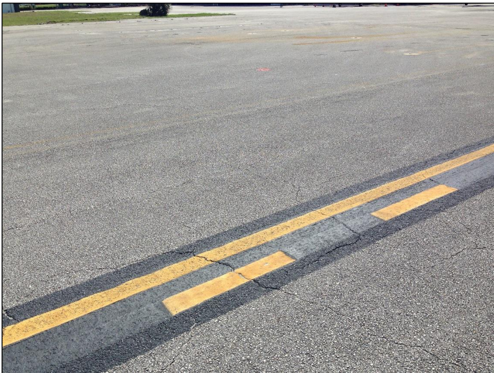
Apron GA, Section 4115, Sample Unit 720 – Low Severity (43) Block Cracking, Low Severity (48) Longitudinal and Transverse Cracking, Low Severity (52) Raveling
