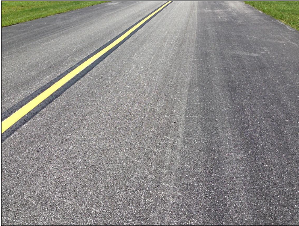
Taxiway A, Section 310, Sample Unit 302 – Low Severity (52) Raveling, Low Severity (57) Weathering
