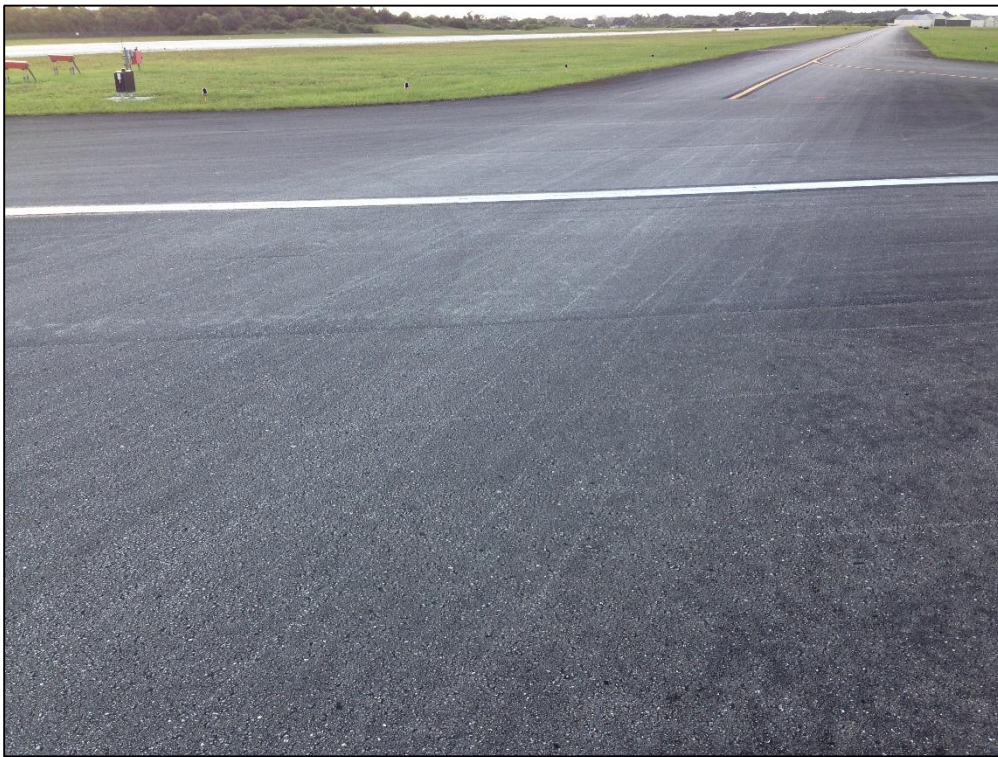
Runway 3-21, Section 6305, Sample Unit 152 – Low Severity (48) Longitudinal and Transverse Cracking, Low Severity (52) Raveling, Low Severity (57) Weathering
