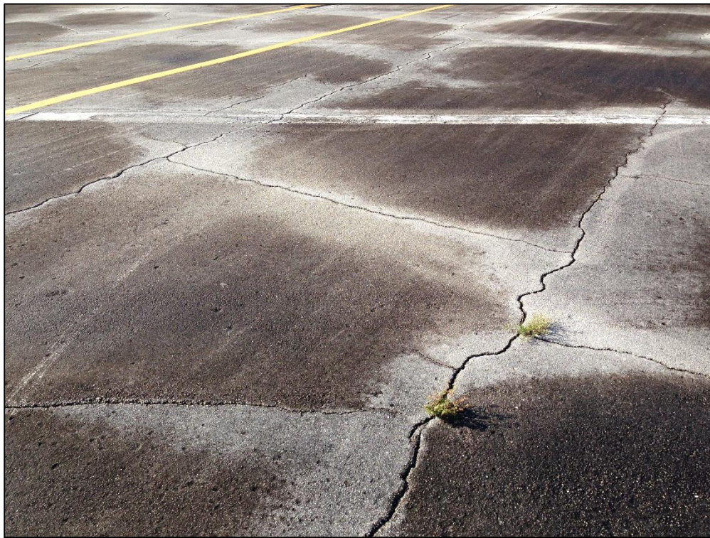
Runway 3-21, Section 6310, Sample Unit 109 – Low Severity (43) Block Cracking, Medium Severity (43) Block Cracking, Low Severity (52) Raveling
