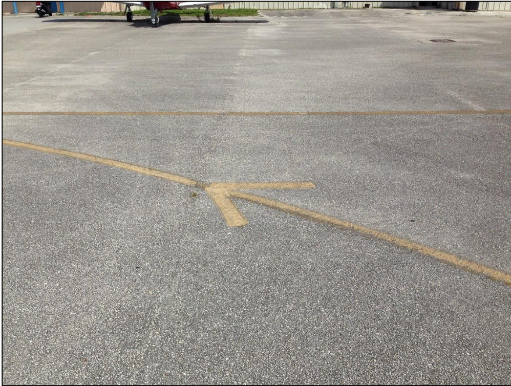
Apron GA, Section 4105, Sample Unit 516 – Low Severity (48) Longitudinal and Transverse Cracking, Low Severity (52) Raveling, Low Severity (57) Weathering
