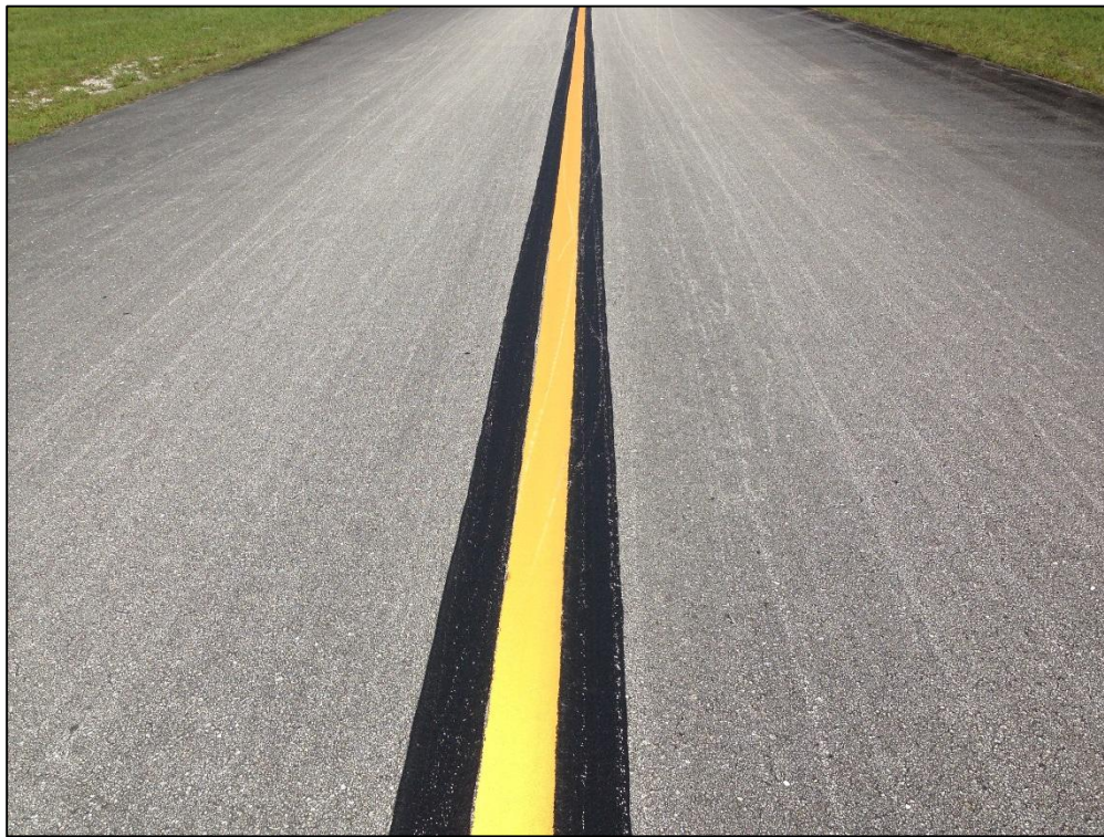
Taxiway B, Section 205, Sample Unit 109 – Low Severity (48) Longitudinal and Transverse Cracking, Low Severity (52) Raveling, Low Severity (57) Weathering
