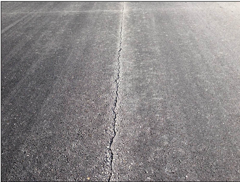
Runway 5-23, Section 6310, Sample Unit 108 – Low Severity (48) Longitudinal and Transverse Cracking, Low Severity (52) Raveling, Low Severity (57) Weathering
