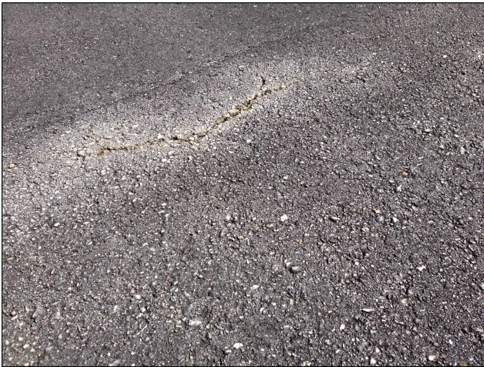
Taxiway Charlie, Section 305, Sample Unit 310 – Low Severity (48) Longitudinal and Transverse Cracking, Low Severity (52) Raveling, Low Severity (56) Swelling, Low Severity (57) Weathering
