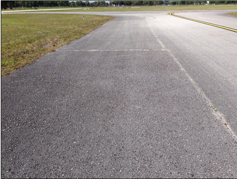
Taxiway Delta, Section 410, Sample Unit 102 – Low Severity (48) Longitudinal and Transverse Cracking, Low Severity (52) Raveling, Medium Severity (52) Raveling
