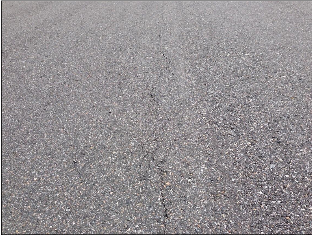
Taxiway Alpha, Section 120, Sample Unit 209 – Low Severity (48) Longitudinal and Transverse Cracking, Low Severity (52) Raveling, Low Severity (56) Swelling, Low Severity (57) Weathering
