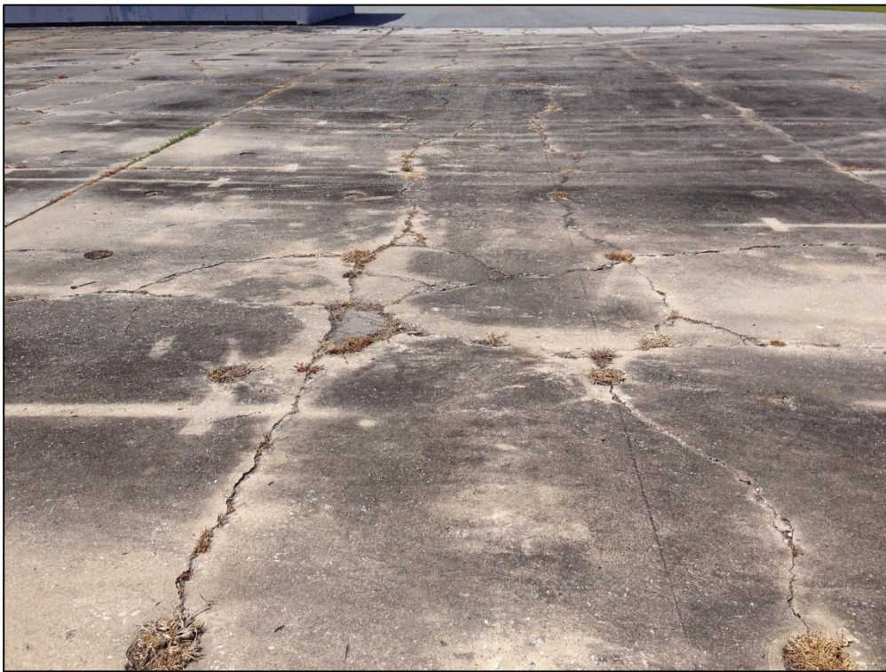
West Apron, Section 4325, Sample Unit 301 – Medium Severity (65) Joint Seal Damage, Medium Severity (72) Shattered Slab
