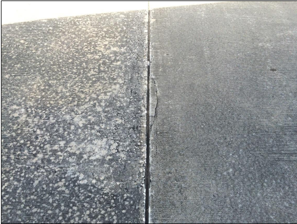
Center Apron, Section 4998, Sample Unit 103 – Low Severity (70) Scaling, Map Cracking, Crazing, Low Severity (74) Joint Spalling
