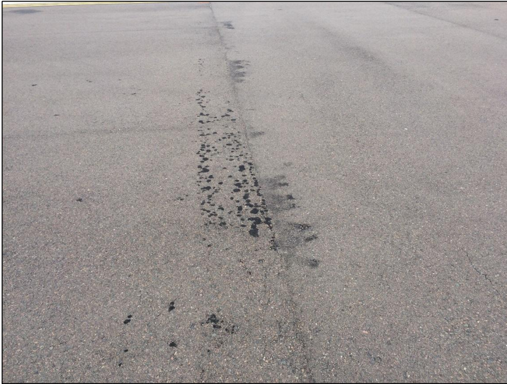
Terminal Apron, Section 4210, Sample Unit 250 – (42) Bleeding, Low Severity (57) Weathering
