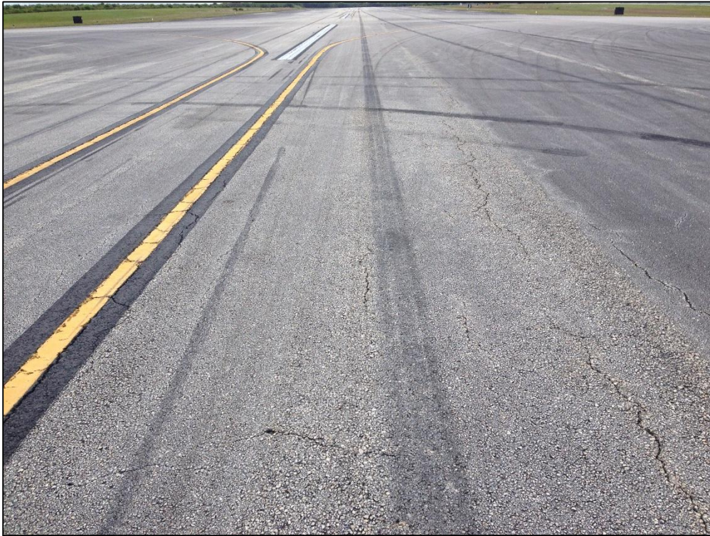
Runway 9L-27R, Section 6210, Sample Unit 377 – Low and Medium Severity (48) Longitudinal and Transverse Cracking, Low Severity (56) Swelling, Low Severity (52) Raveling, Low Severity (57) Weathering
