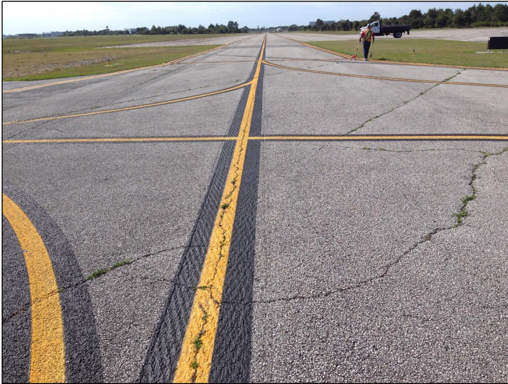
Taxiway Sierra, Section 510, Sample Unit 120 – Low and Medium Severity (48) Longitudinal and Transverse Cracking, Low Severity (52) Raveling, Low Severity (57) Weathering
