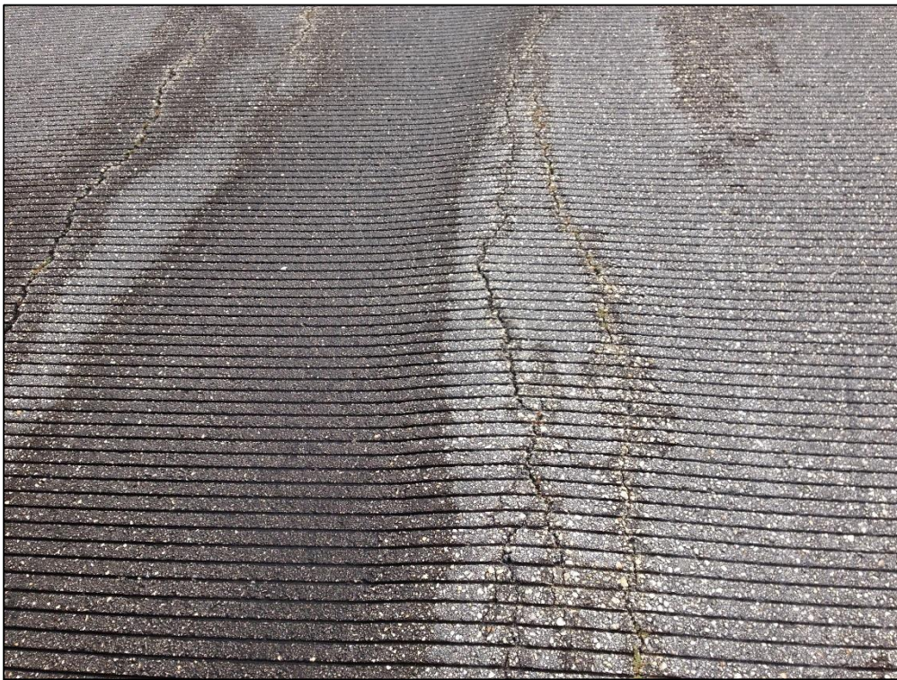
Runway 9R-27L, Section 6105, Sample Unit 382 – Low and Medium Severity (48) Longitudinal and Transverse Cracking, Low Severity (56) Swelling, Low Severity (57) Weathering
