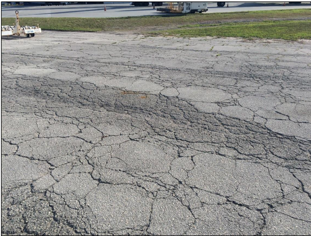
East Apron, Section 4410, Sample Unit 801 – Medium Severity (43) Block Cracking, High Severity (43) Block Cracking, Low Severity (52) Raveling, Medium Severity (52) Raveling
