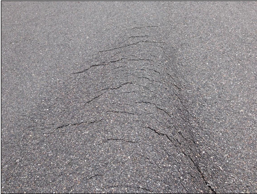
Taxiway Alpha, Section 120- (55) Slippage Cracking (*Not an inspected sample.)
