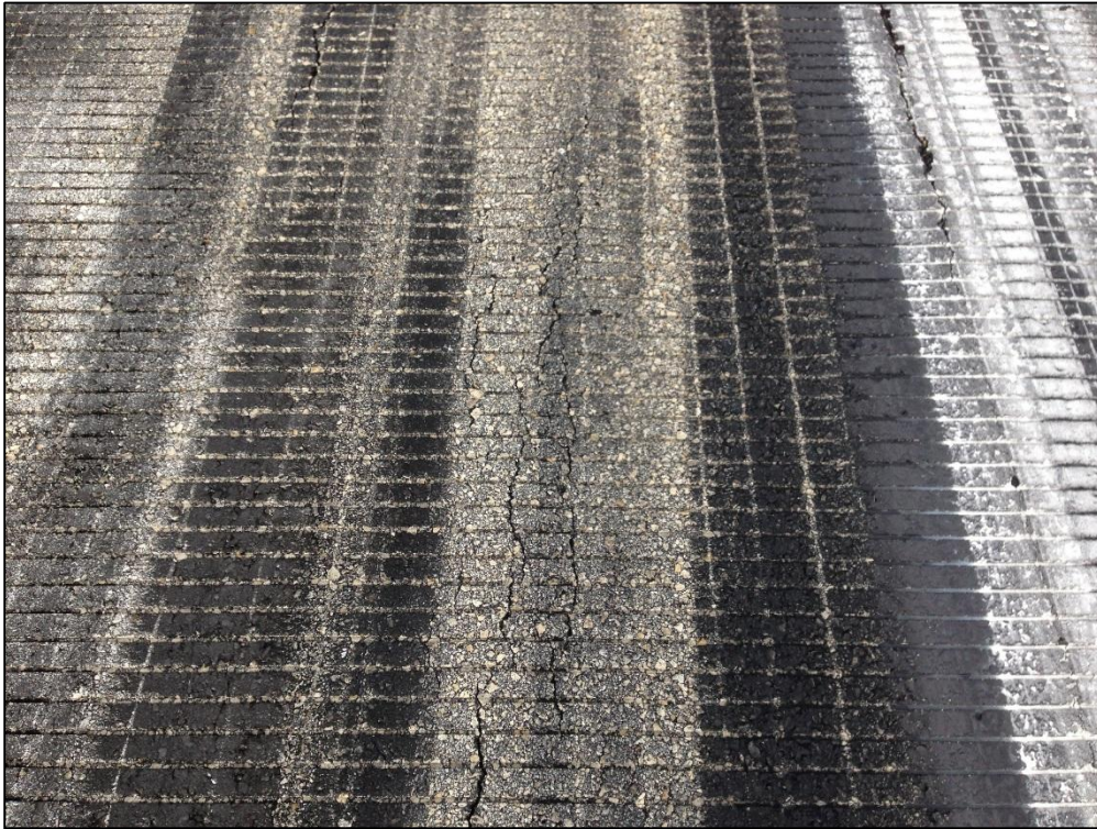
Runway 9R-27L, Section 6105, Sample Unit 326 – Low Severity (41) Alligator Cracking, Low Severity (48) Longitudinal and Transverse Cracking, Low Severity (52) Raveling, Low Severity (56) Swelling, Low Severity (57) Weathering
