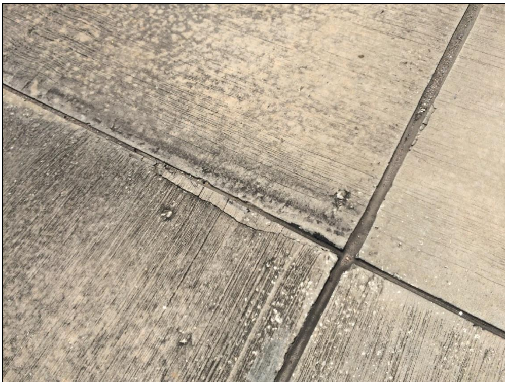
Terminal Apron, Section 4205, Sample Unit 202 – Low Severity (74) Joint Spalling
