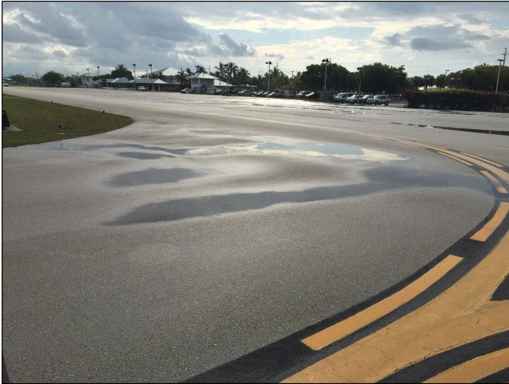
Taxiway Charlie, Section 205, Sample Unit 201 – Low Severity (45) Depression, Low Severity (57) Weathering
