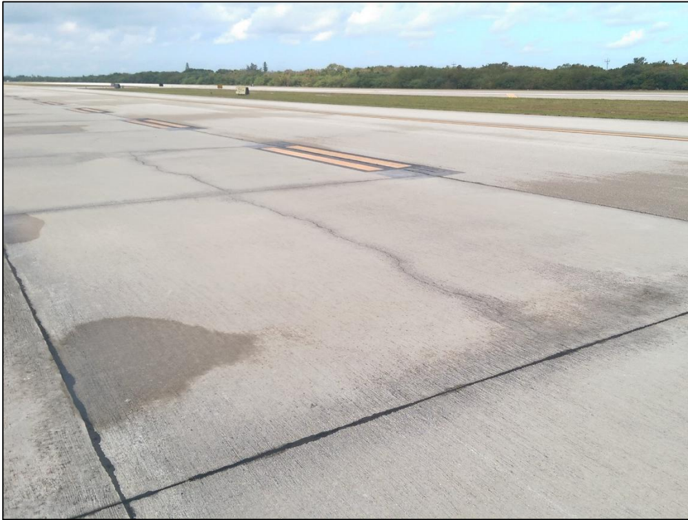
Apron Terminal, Section 4220, Sample Unit 305 – Low Severity (63) Longitudinal, Transverse, and Diagonal Cracking, Low Severity (65) Joint Seal Damage
