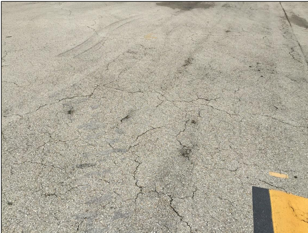
Apron East, Section 4510, Sample Unit 102 – Low Severity (43) Block Cracking, Low Severity (48) Longitudinal and Transverse Cracking, Low Severity (52) Raveling
