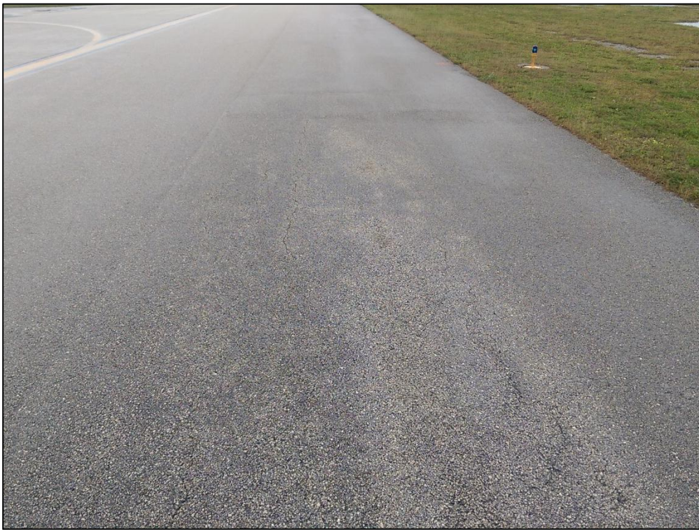
Taxiway Alpha, Section 105, Sample Unit 111 – Low Severity (48) Longitudinal and Transverse Cracking, Low Severity (52) Raveling, Medium Severity (52) Raveling
