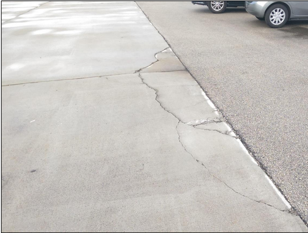
Apron Jet Center, Section 4310, Sample Unit 120 – Medium Severity (65) Joint Seal Damage, Medium Severity (74) Joint Spalling, Low Severity (62) Corner Break, Low Severity (75) Corner Spalling
