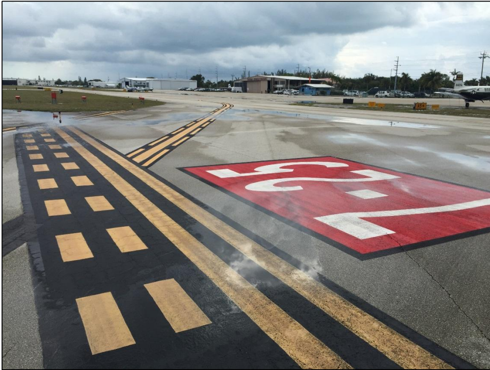
Taxiway Delta, Section 305, Sample Unit 301 – Low Severity (48) Longitudinal and Transverse Cracking, Low Severity (45) Depression, Low Severity (57) Weathering
