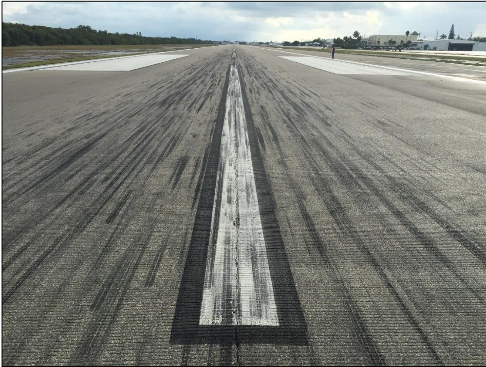
Runway 7-25, Section 6105, Sample Unit 118 – Low and Medium Severity (48) Longitudinal and Transverse Cracking, Medium Severity (52) Raveling
