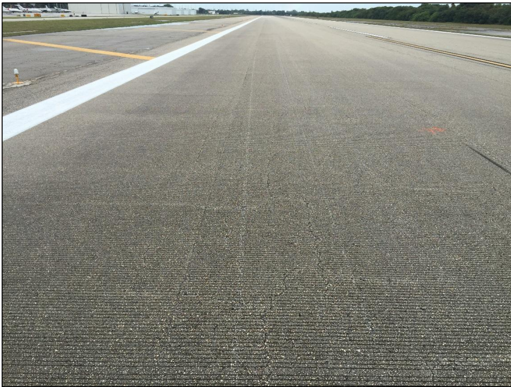
Runway 7-25, Section 6110, Sample Unit 310 – Low Severity (48) Longitudinal and Transverse Cracking, Low Severity (52) Raveling, Low Severity (57) Weathering
