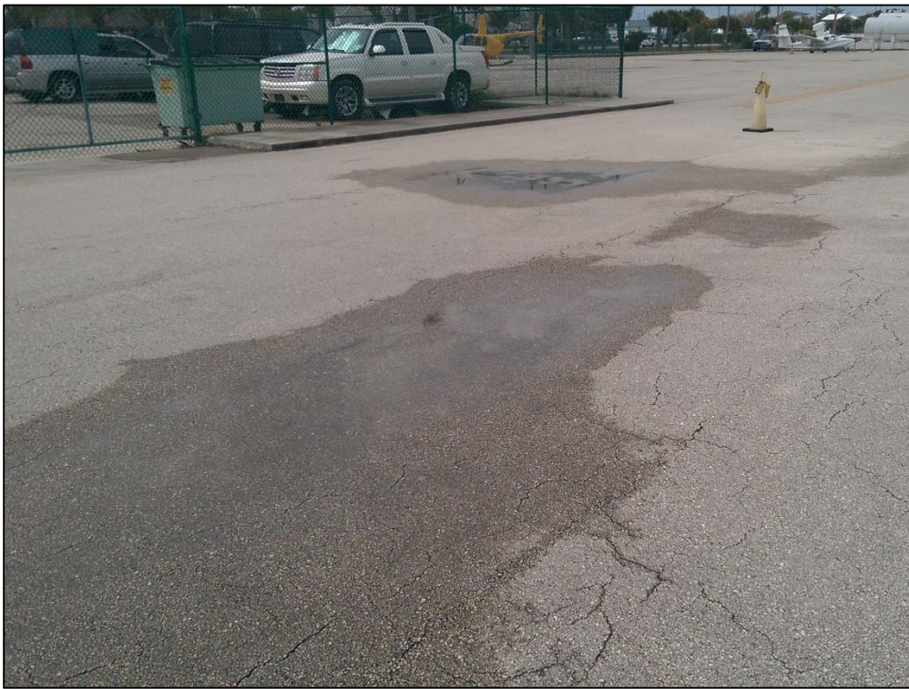
Apron Flight Center, Section 4105, Sample Unit 409 – Low Severity (43) Block Cracking, Low Severity (45) Depression, Low Severity (56) Swelling, Low Severity (57) Weathering
