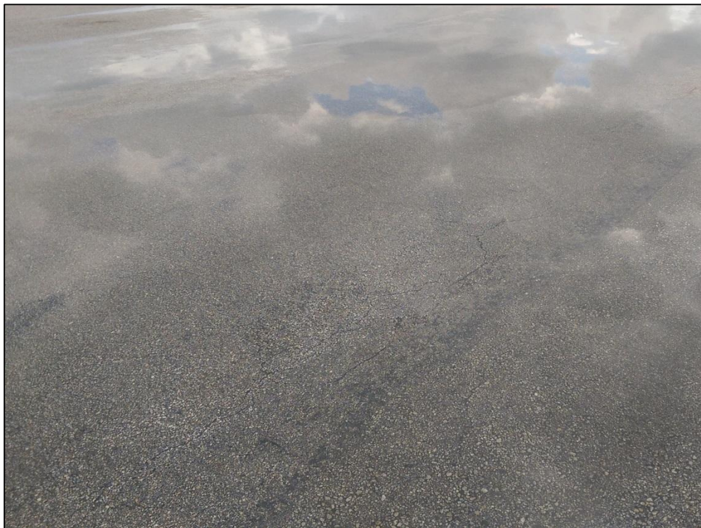
Apron Jet Center, Section 4315, Sample Unit 151 – Low Severity (45) Depression, Low Severity (48) Longitudinal and Transverse Cracking, Low Severity (57) Weathering
