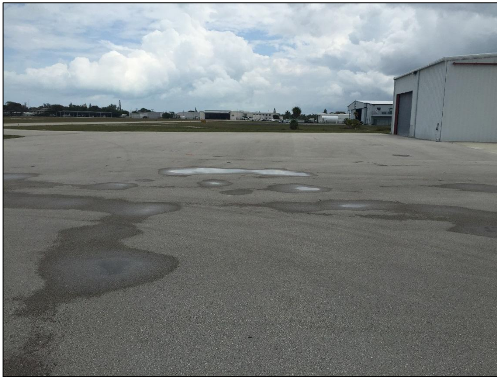
Apron Flight Center, Section 4115, Sample Unit 414 – Low Severity (45) Depression, Low Severity (52) Raveling
