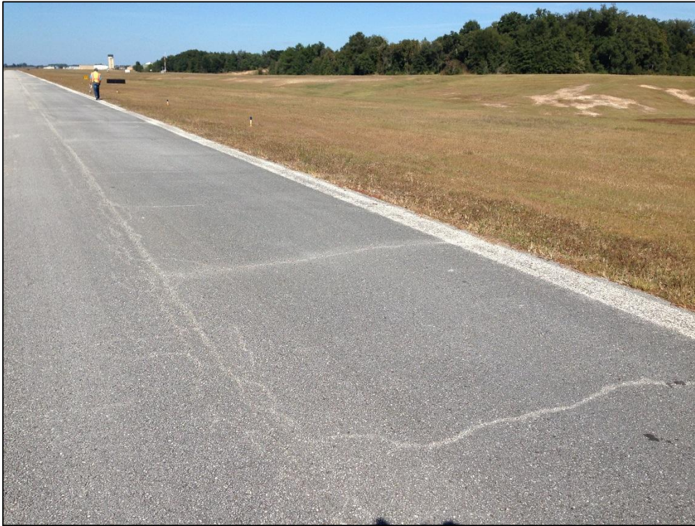
Taxiway Alpha, Section 540, Sample Unit 104 – Low Severity (43) Block Cracking, Low Severity (48) Longitudinal and Transverse Cracking, Low Severity (52) Raveling, High Severity (52) Raveling
