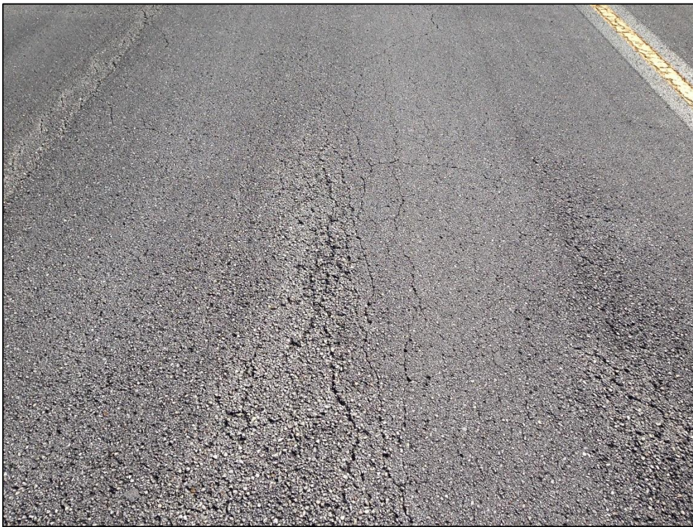
Taxiway Alpha, Section 540, Sample Unit 112 – Low Severity (41) Alligator Cracking, Low Severity (48) Longitudinal and Transverse Cracking, Low Severity (52) Raveling
