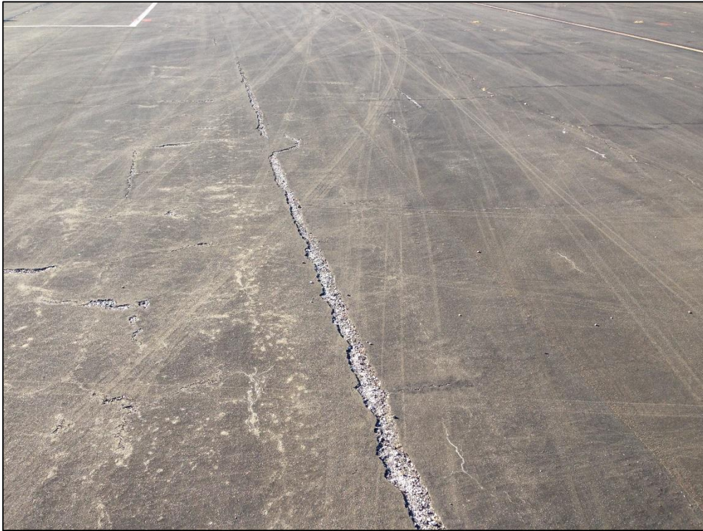
Center Apron, Section 4115, Sample Unit 310 – Low Severity (43) Block Cracking, Low Severity (48) Longitudinal and Transverse Cracking, High Severity (52) Raveling
