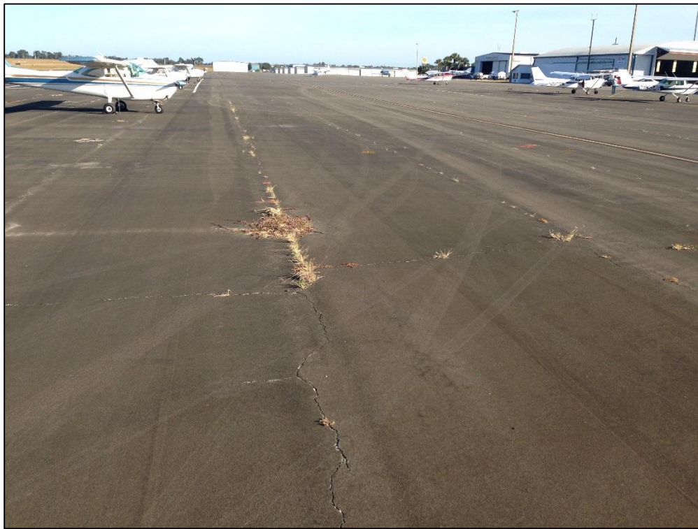
Center Apron, Section 4110, Sample Unit 206 – Low Severity (48) Longitudinal and Transverse Cracking
