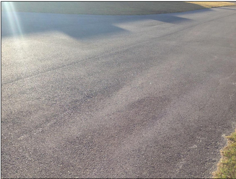
Taxiway A6, Section 575, Sample Unit 601 – Low Severity (52) Raveling, Low Severity (57) Weathering
