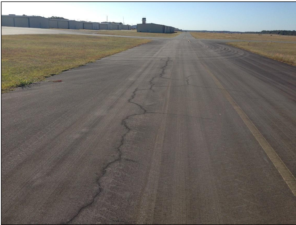
Taxiway North Apron, Section 595, Sample Unit 301 – Low Severity (48) Longitudinal and Transverse Cracking
