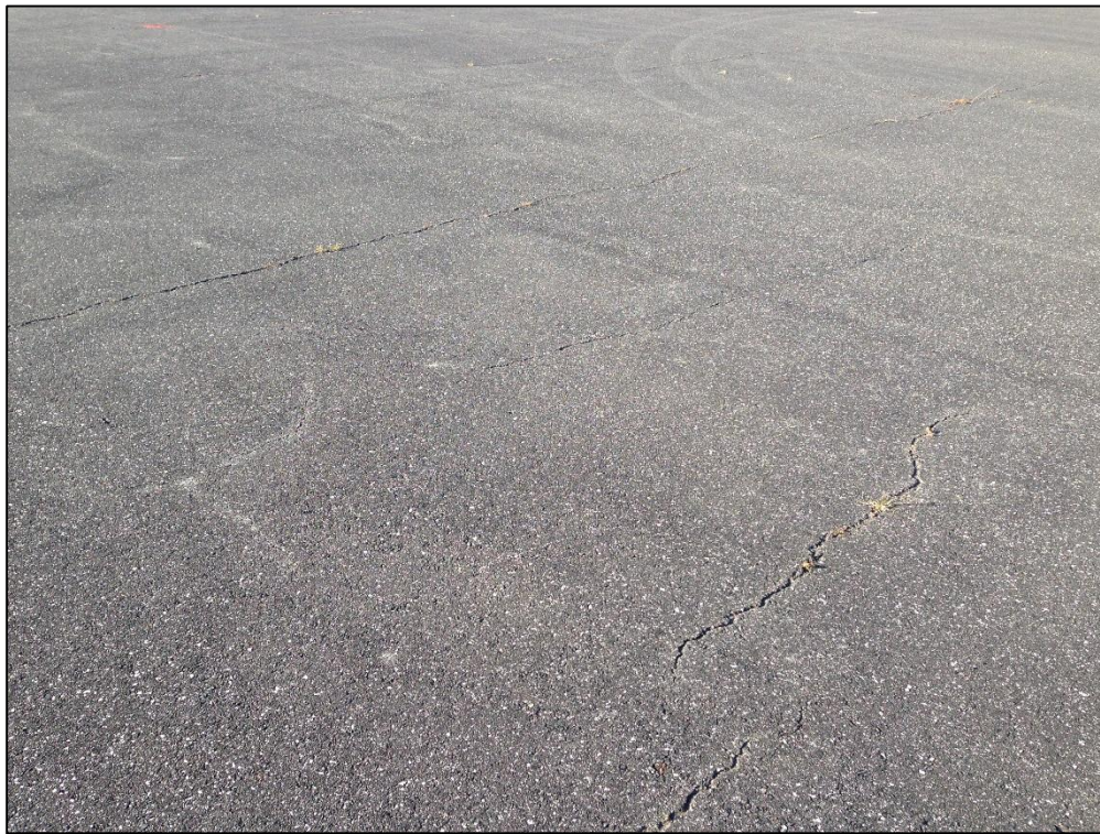
Center Apron, Section 4105, Sample Unit 303 – Low Severity (48) Longitudinal and Transverse Cracking, Medium Severity (48) Longitudinal and Transverse Cracking, Medium Severity (57) Weathering
