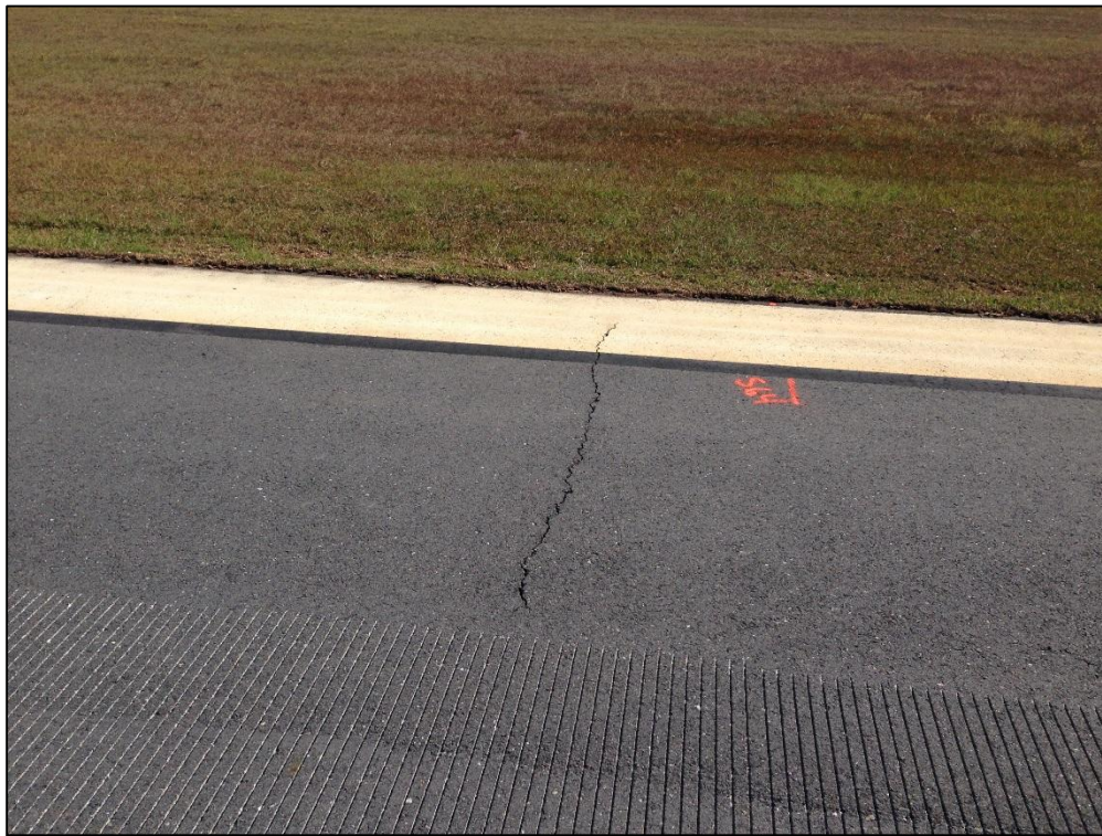
Runway 18-36, Section 6110, Sample Unit 564 – Low Severity (48) Longitudinal and Transverse Cracking, Low Severity (57) Weathering
