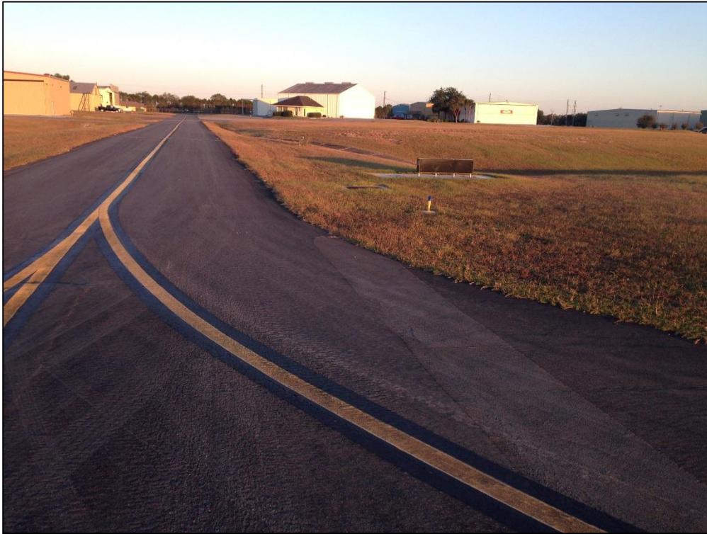
Taxiway A6, Section 560, Sample Unit 500 – Low Severity (48) Longitudinal and Transverse Cracking, Low Severity (50) Patching, Low Severity (57) Weathering
