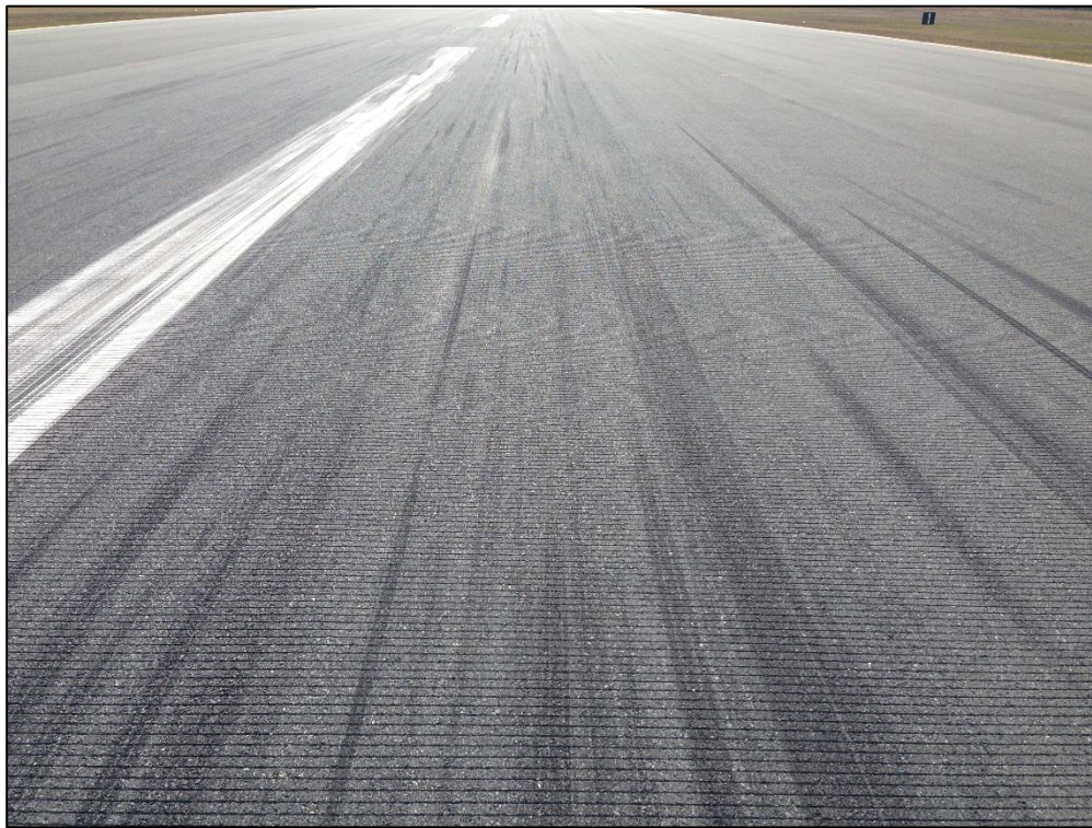
Runway 18-36, Section 6125, Sample Unit 315 – Low Severity (57) Weathering
