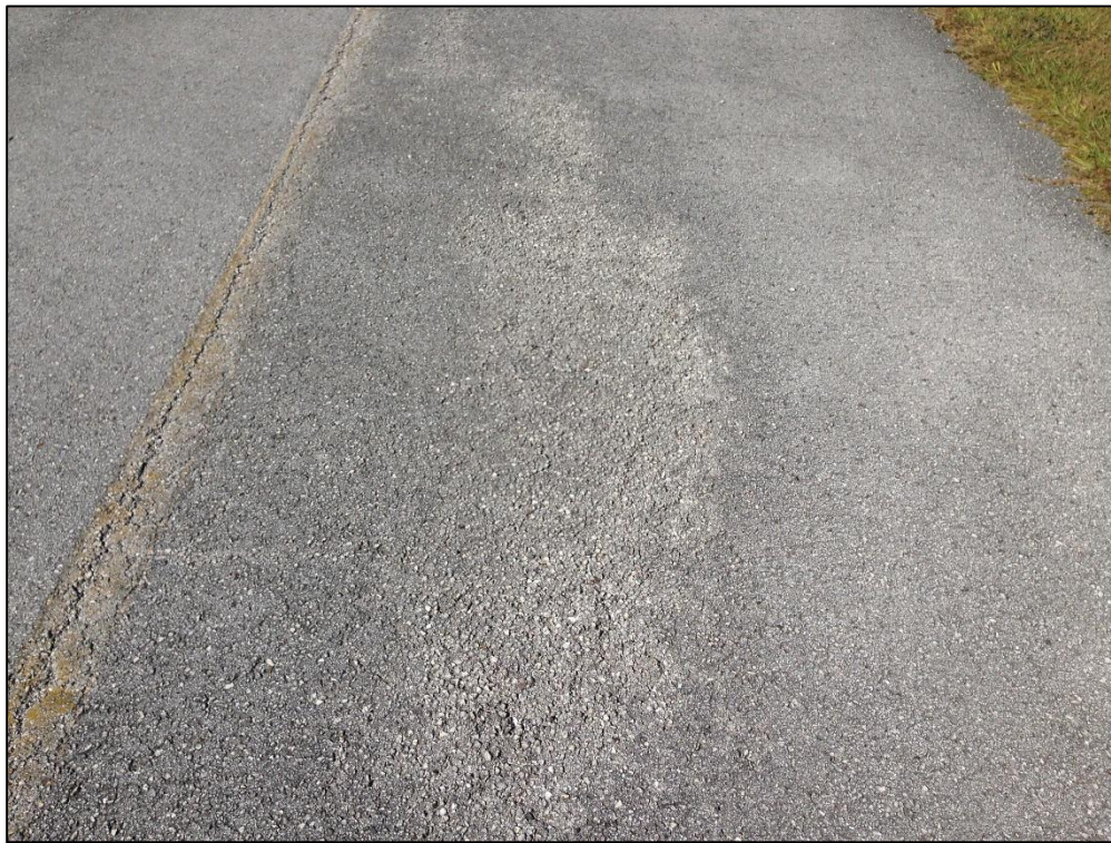
Taxiway T-Hangar, Section 585, Sample Unit 201 – Low Severity (48) Longitudinal and Transverse Cracking, Low Severity (52) Raveling, High Severity (52) Raveling
