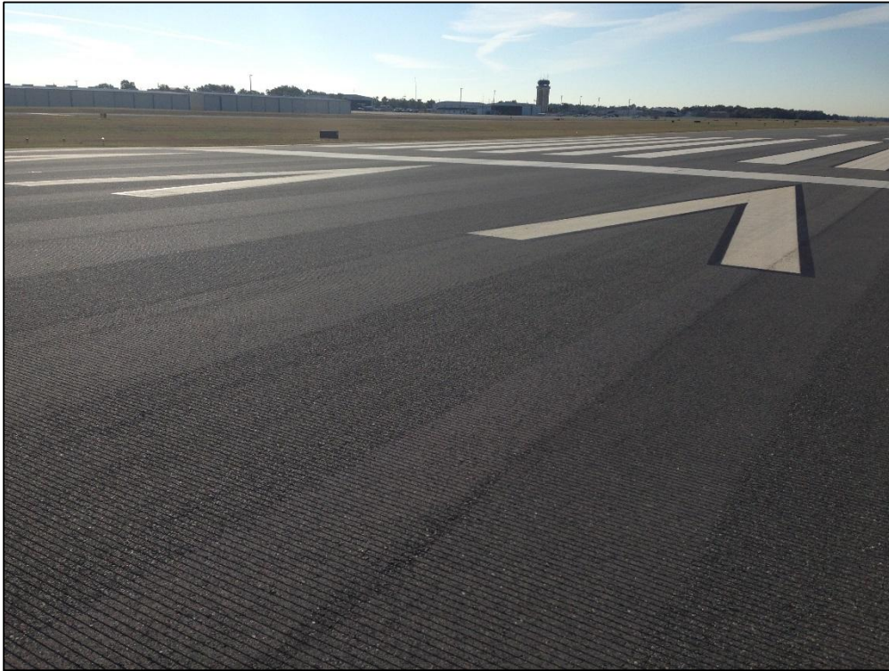
Runway 18-36, Section 6105, Sample Unit 422 – Low Severity (57) Weathering
