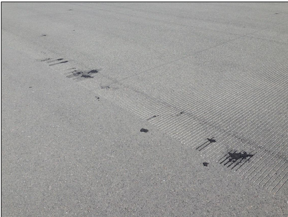
Runway 18-36, Section 6110, Sample Unit 176 – (42) Bleeding, Low Severity (57) Weathering
