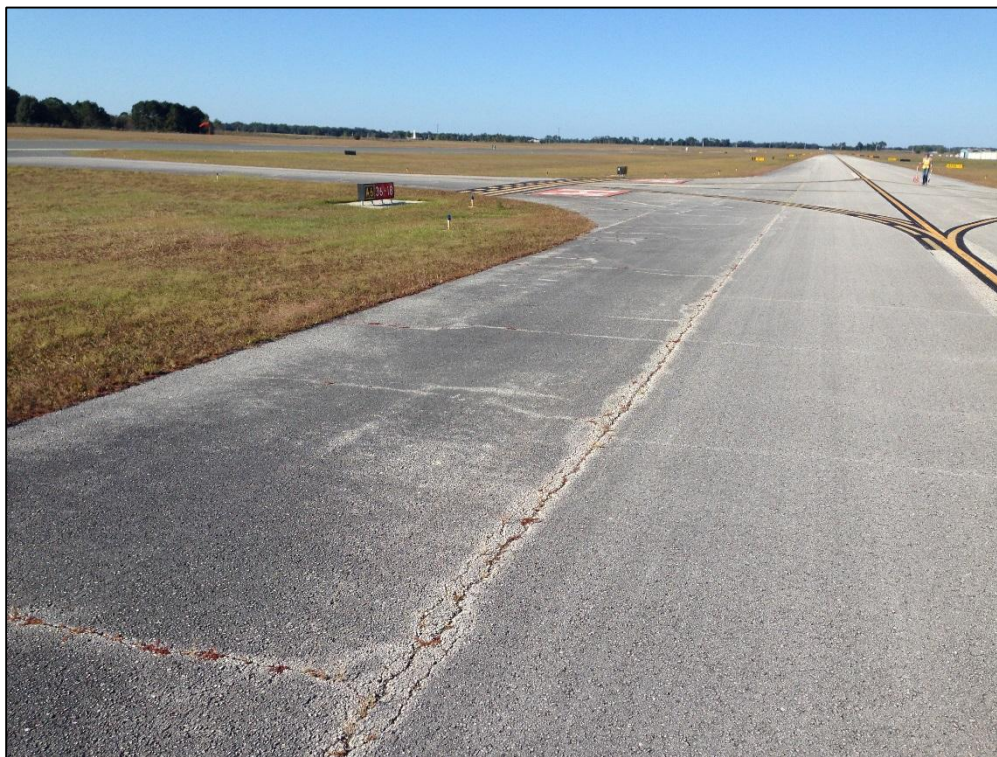
Taxiway Alpha, Section 505, Sample Unit 137 – Low Severity (43) Block Cracking, Low Severity (48) Longitudinal and Transverse Cracking, Low Severity (52) Raveling, Medium Severity (52) Raveling
