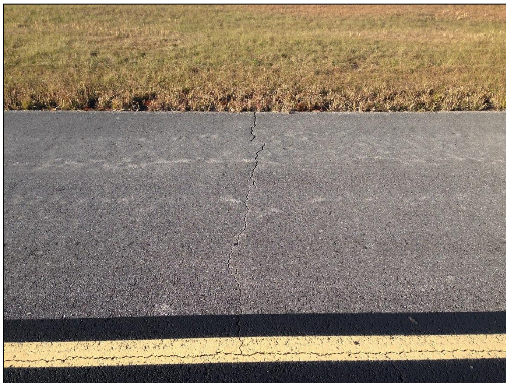
Taxiway Bravo, Section 105, Sample Unit 102 – Low Severity (48) Longitudinal and Transverse Cracking, Low Severity (52) Raveling, Low Severity (56) Swelling
