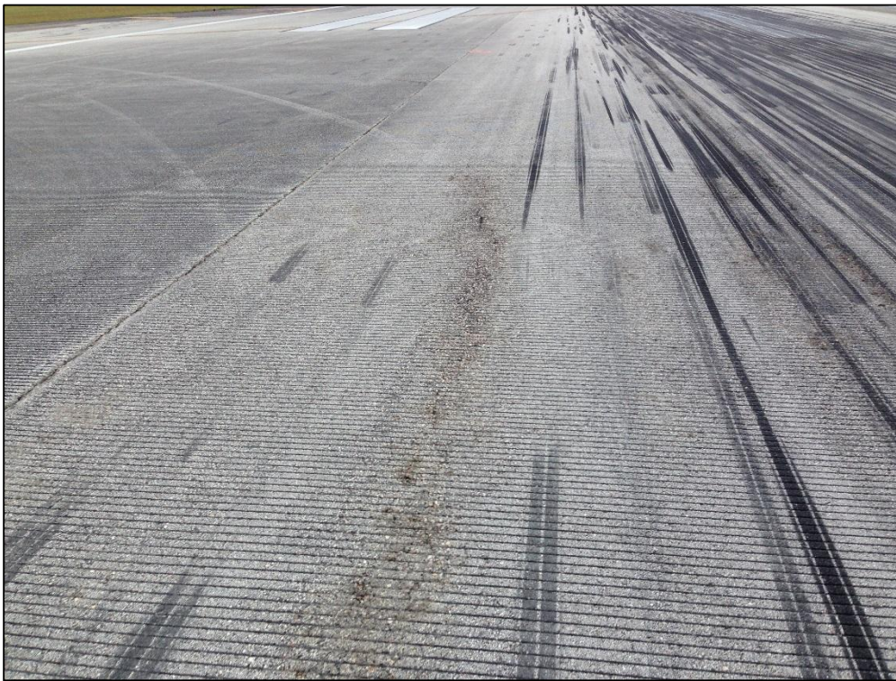
Runway 9L-27R, Section 6115, Sample Unit 360 – Low and Medium Severity (48) Longitudinal and Transverse Cracking, Low Severity (52) Raveling, Medium Severity (52) Raveling
