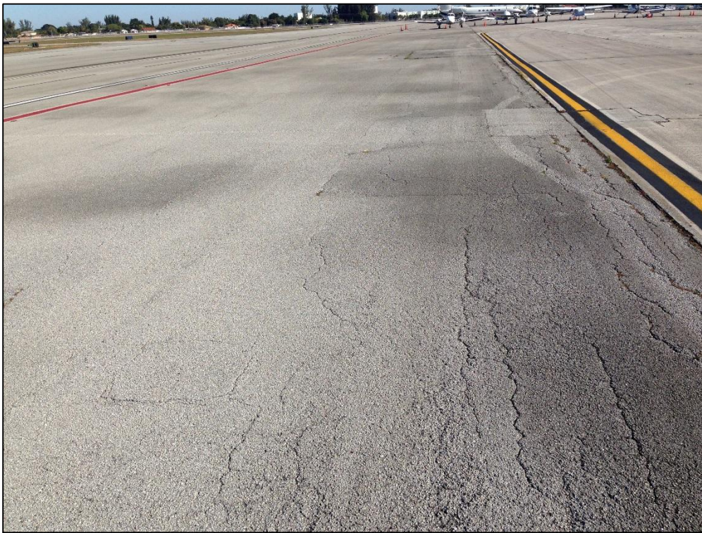
Apron Center, Section 4105, Sample Unit 164 – Low Severity (43) Block Cracking, Low Severity (45) Depression, Medium Severity (50) Patching, Low Severity (52) Raveling
