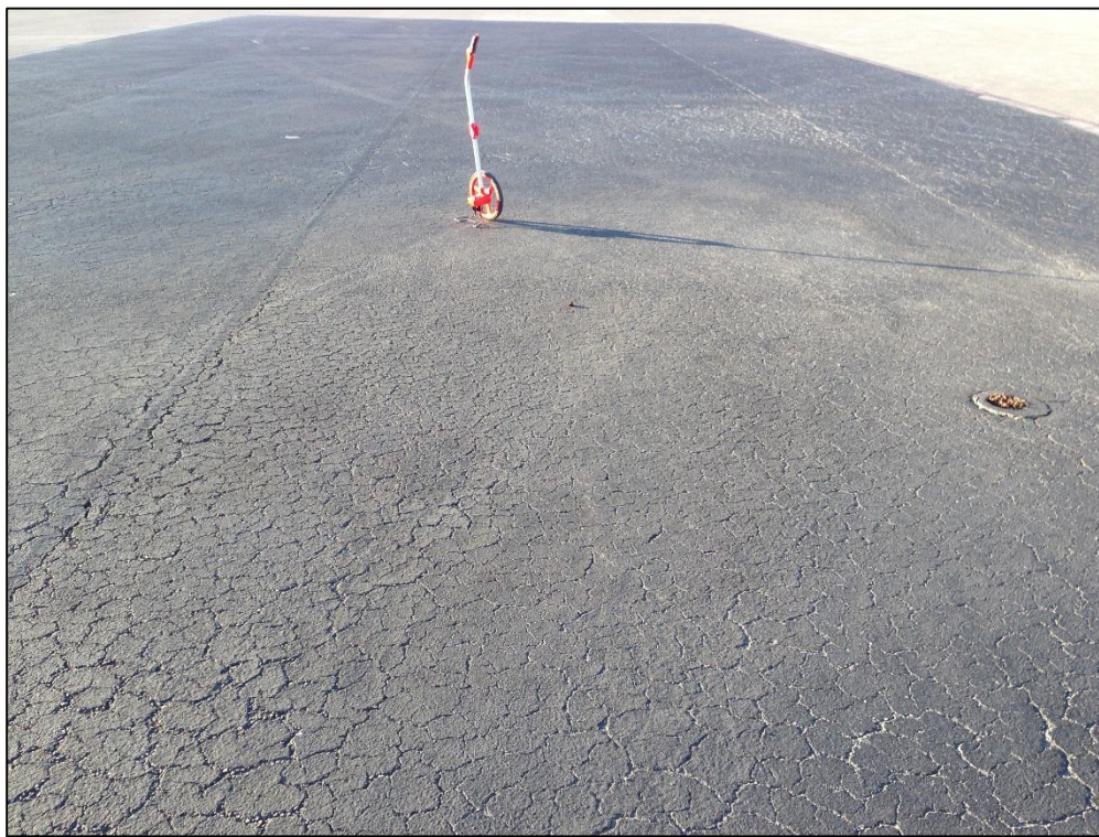
Apron Northeast, Section 4305, Sample Unit 426 – Low Severity (43) Block Cracking, Low Severity (45) Depression, Low Severity (48) Longitudinal and Transverse Cracking, Low Severity (52) Raveling, Medium Severity (57) Weathering
