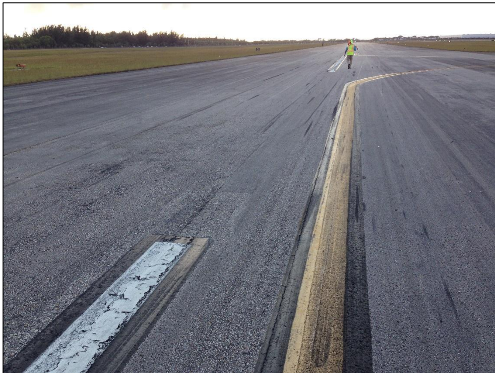
Runway 9R-27L, Section 6410, Sample Unit 171 – Low Severity (48) Longitudinal and Transverse Cracking, Low Severity (52) Raveling, Medium Severity (52) Raveling, Low Severity (56) Swelling
