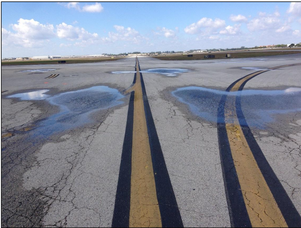
Apron Center, Section 4105, Sample Unit 151 – Low Severity (41) Alligator Cracking, Medium Severity (41) Alligator Cracking, Low Severity (43) Block Cracking, Low Severity (45) Depression, Medium Severity (45) Depression, High Severity (50) Patching, Low Severity (52) Raveling, Medium Severity (53) Rutting, Low Severity (57) Weathering
