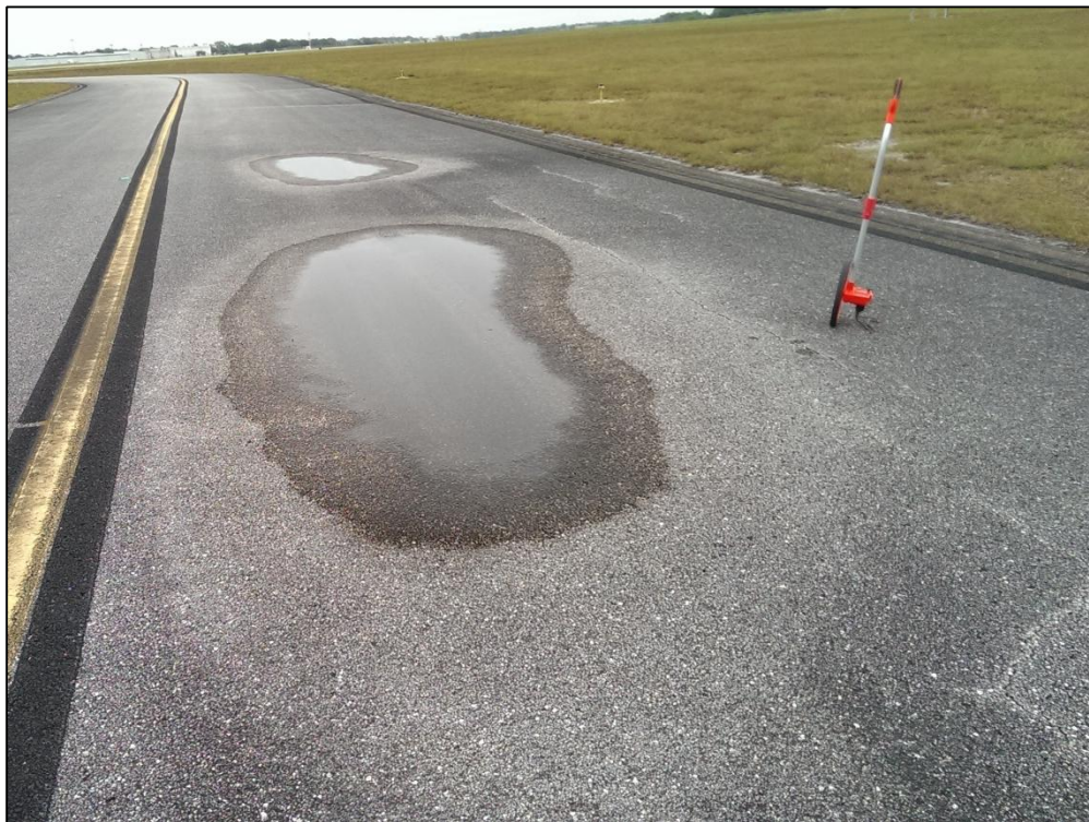
Taxiway E3, Section 420, Sample Unit 405 – Medium Severity (45) Depression, Low Severity (48) Longitudinal and Transverse Cracking, Low Severity (52) Raveling, Low Severity (57) Weathering
