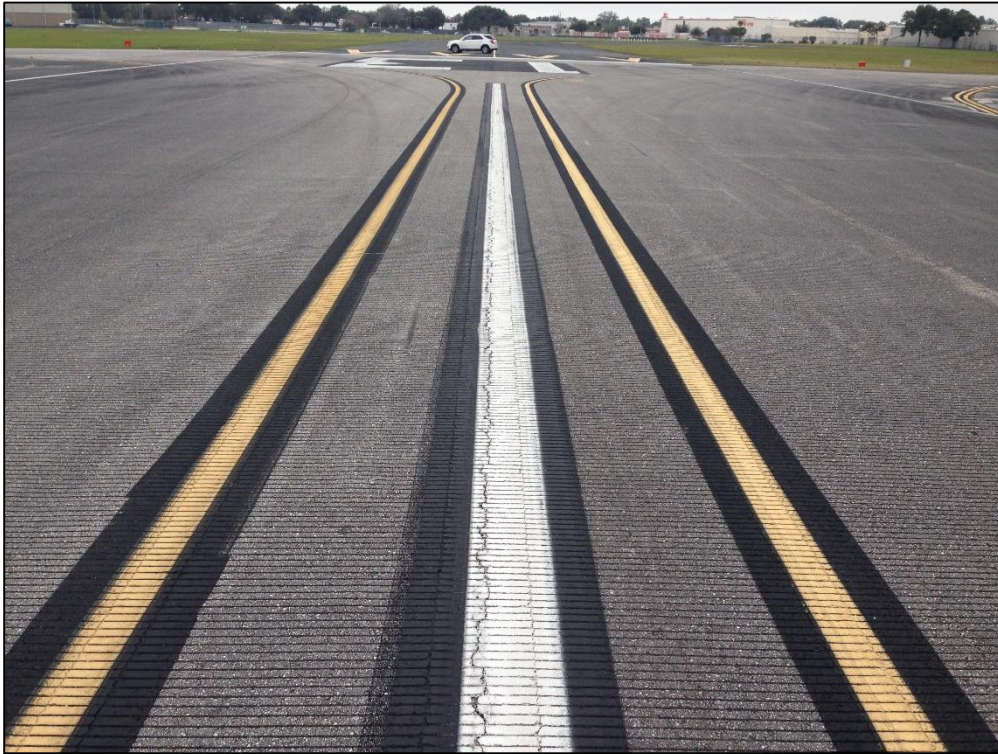
Runway 13-31, Section 6205, Sample Unit 195 – Low Severity (48) Longitudinal and Transverse Cracking, Low Severity (57) Weathering
