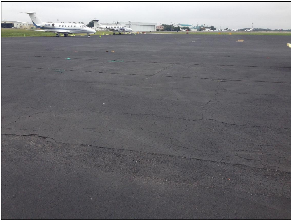
Apron West, Section 4660, Sample Unit 507 – Medium Severity (43) Block Cracking, Low Severity (52) Raveling
