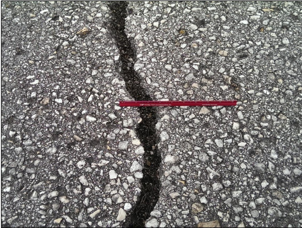
Taxiway E6, Section 805, Sample Unit 801 – High Severity (48) Longitudinal and Transverse Cracking, Low Severity (52) Raveling
