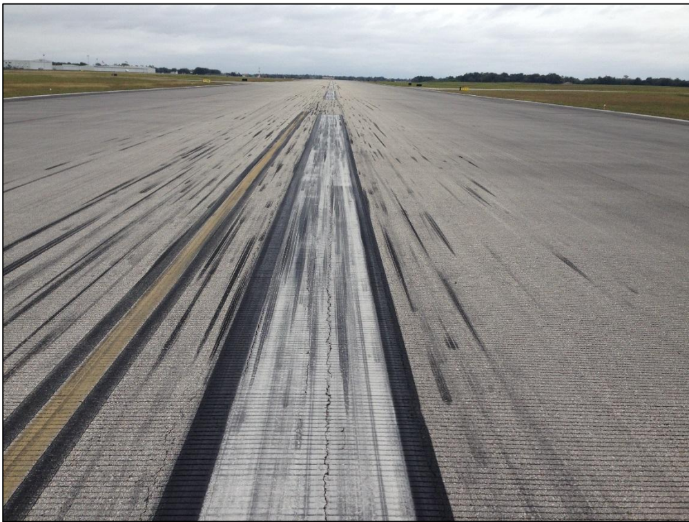
Runway 7-25, Section 6105, Sample Unit 342 – Low Severity (48) Longitudinal and Transverse Cracking, Low Severity (57) Weathering
