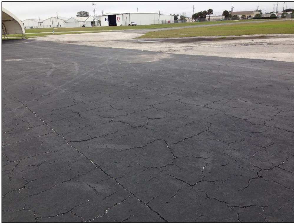
Apron North, Section 4158, Sample Unit 651 – High Severity (43) Block Cracking, Medium Severity (52) Raveling
