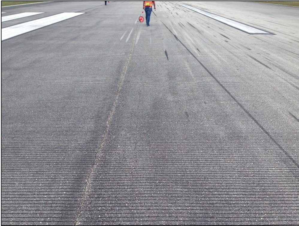
Runway 7-25, Section 6105, Sample Unit 409 – Low Severity (48) Longitudinal and Transverse Cracking, Low Severity (56) Swelling, Low Severity (57) Weathering
