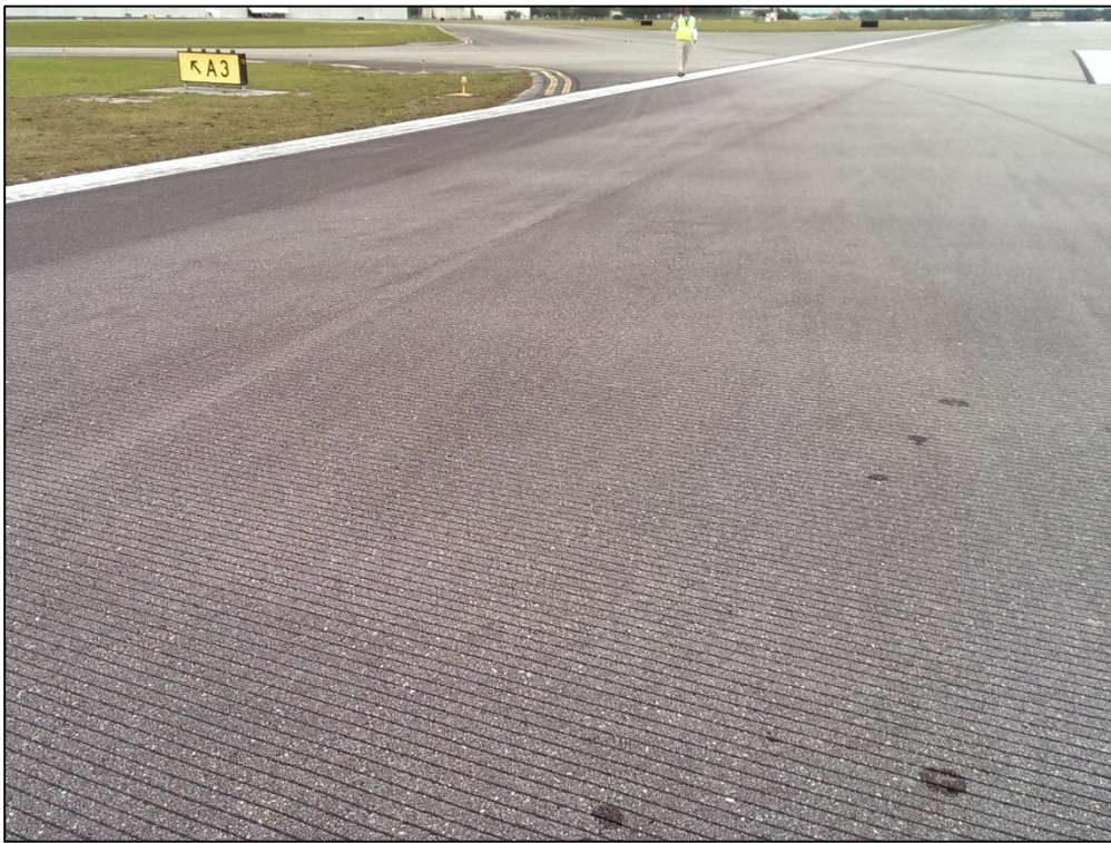
Runway 7-25, Section 6110, Sample Unit 176 – Low Severity (48) Longitudinal and Transverse Cracking, Low Severity (57) Weathering
