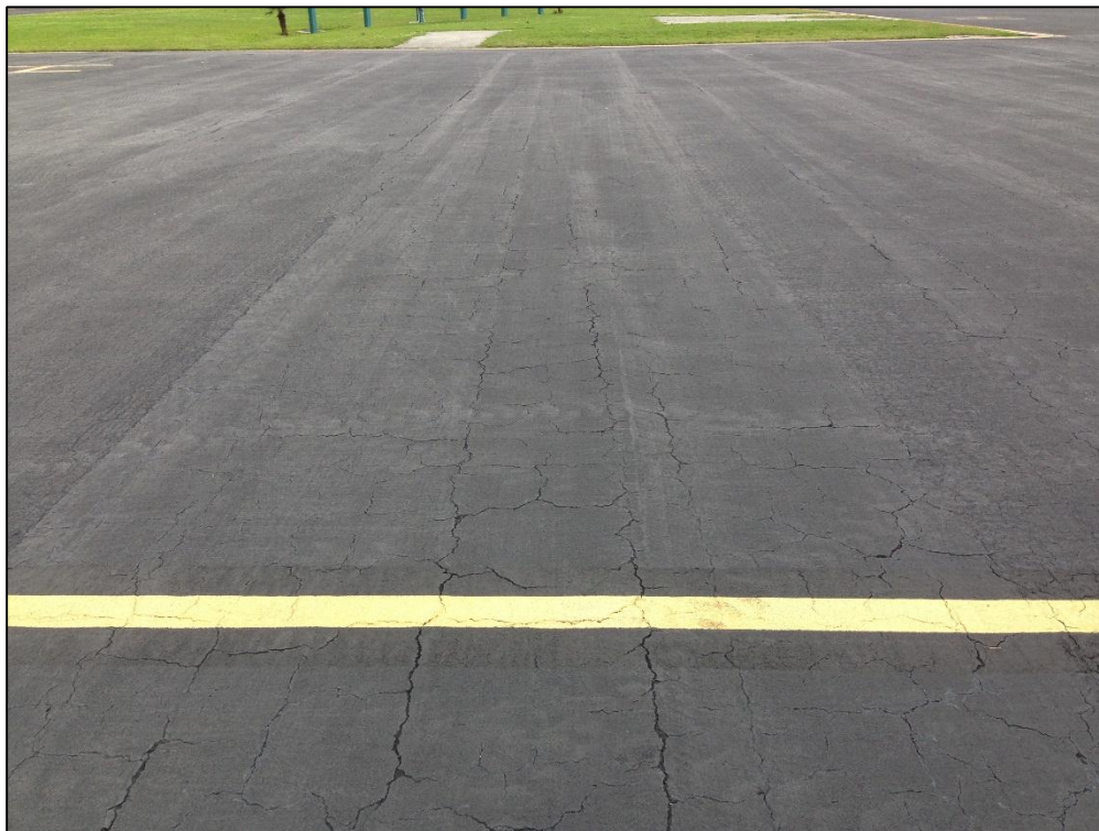
Apron North, Section 4145, Sample Unit 416 – Medium Severity (43) Block Cracking, Low Severity (57) Weathering, Medium Severity (57) Weathering
