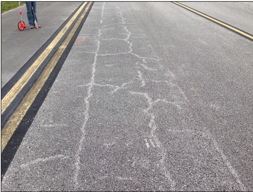
Taxiway Golf, Section 705, Sample Unit 701 – Low Severity (43) Block Cracking, Low Severity (52) Raveling, Low Severity (56) Swelling
