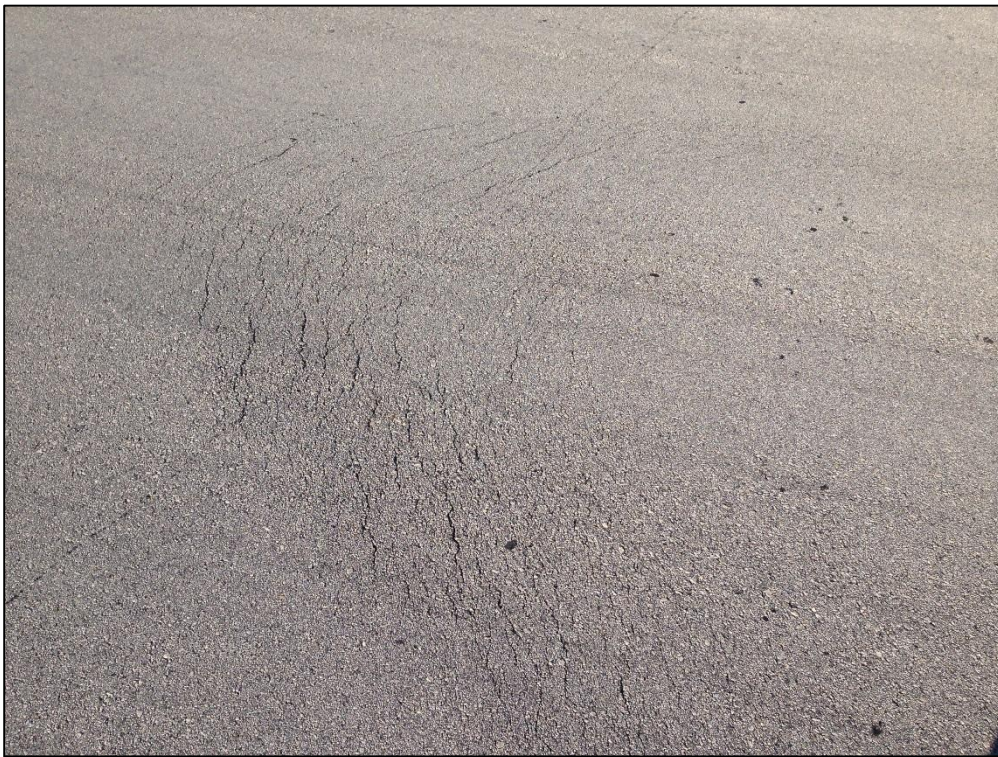
Taxiway C, Section 350, Sample Unit 252 – (55) Slippage Cracking, Low Severity (57) Weathering
