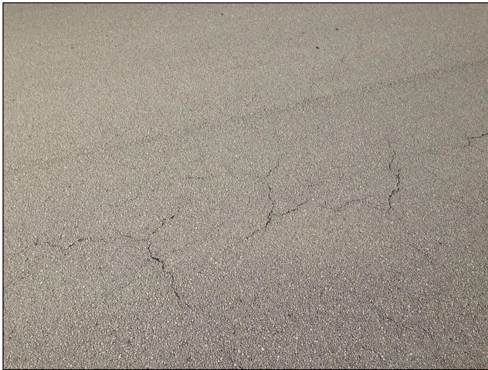
Taxiway C, Section 310, Sample Unit 119 – Low Severity (48) Longitudinal and Transverse Cracking, Low Severity (52) Raveling
