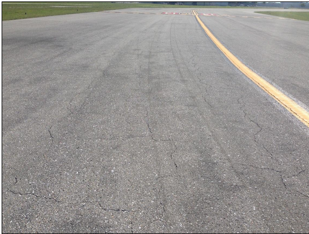
Taxiway B, Section 205, Sample Unit 107 – Low Severity (43) Block Cracking, Low Severity (52) Raveling, Low Severity (56) Swelling
