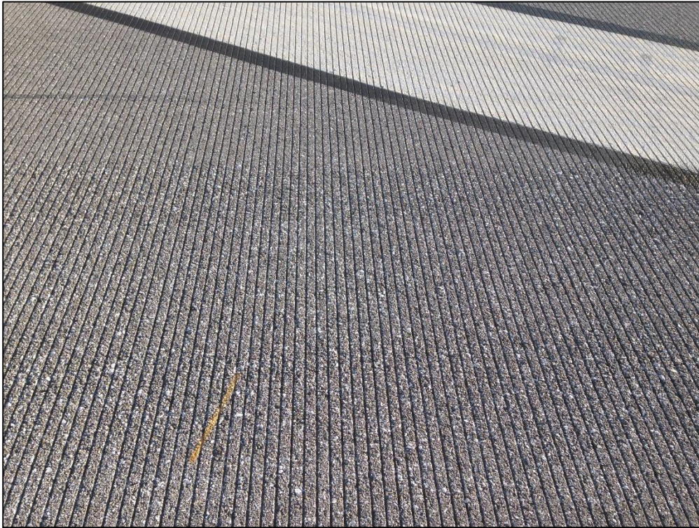
Runway 14-32, Section 6315, Sample Unit 225 – Low Severity (57) Weathering
