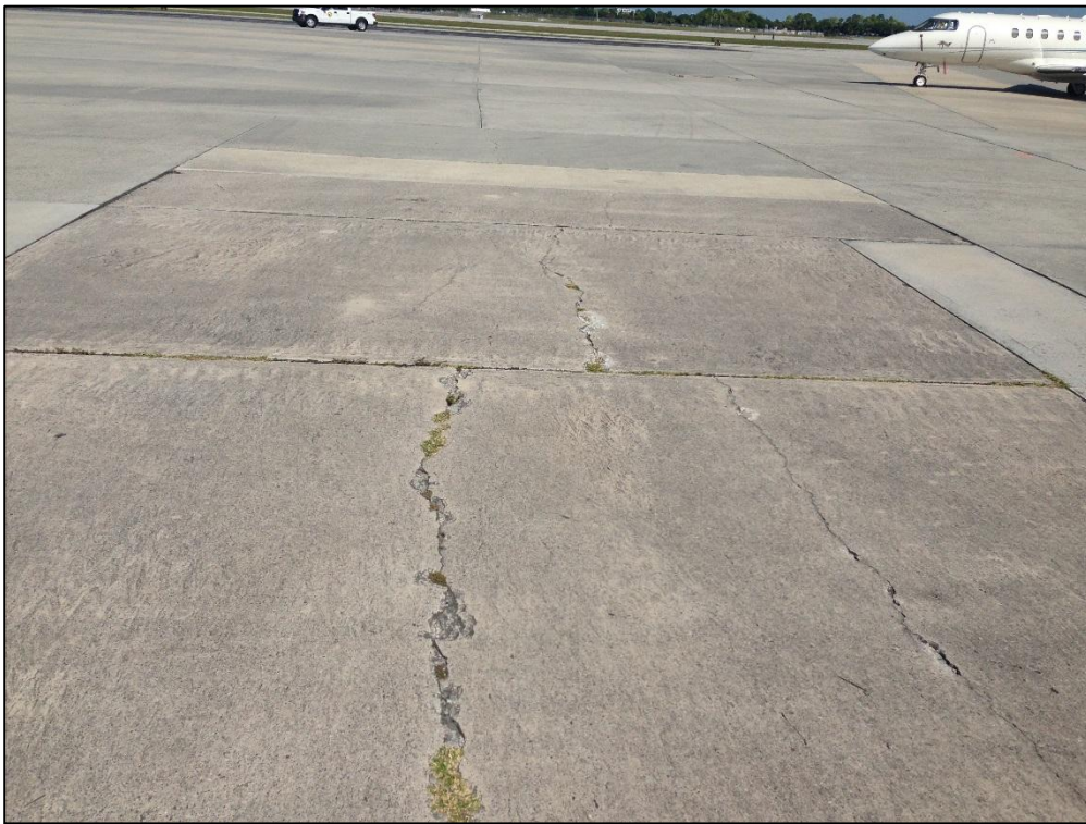
Apron SE GA, Section 4510, Sample Unit 414 – Low Severity (63) Longitudinal, Transverse, and Diagonal Cracking, Medium Severity (63) Longitudinal, Transverse, and Diagonal Cracking, Low Severity (65) Joint Seal Damage, Low Severity (67) Large Patching
