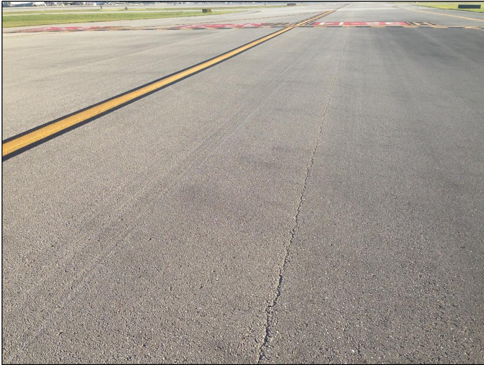
Taxiway H, Section 810, Sample Unit 411 – Low Severity (48) Longitudinal and Transverse Cracking, Medium Severity (48) Longitudinal and Transverse Cracking, Low Severity (52) Raveling, Low Severity (57) Weathering
