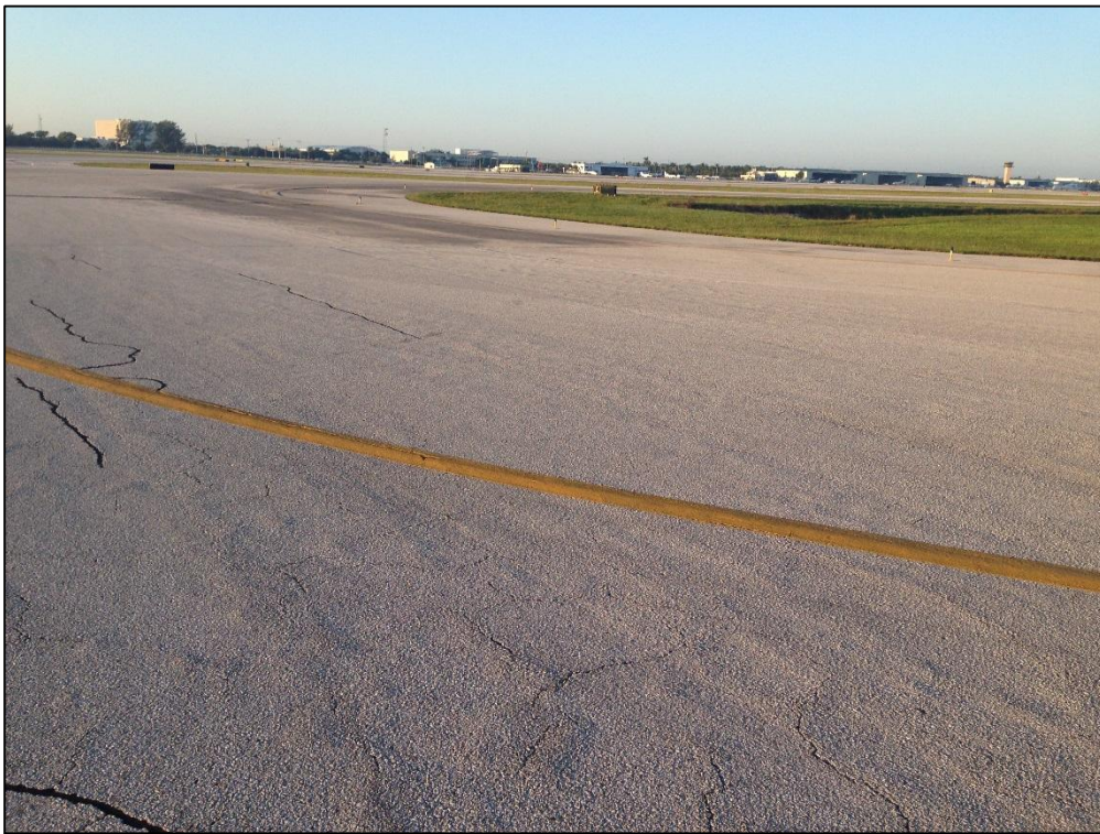
Taxiway H, Section 835, Sample Unit 444 – Low Severity (43) Block Cracking, Low Severity (48) Longitudinal and Transverse Cracking, Low Severity (52) Raveling Low Severity (56) Swelling
