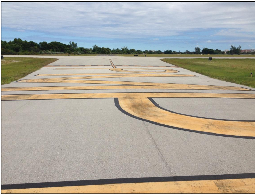
Taxiway R, Section 1850, Sample Unit 600 – Low Severity (48) Longitudinal and Transverse Cracking, Low Severity (52) Raveling, Low Severity (57) Weathering
