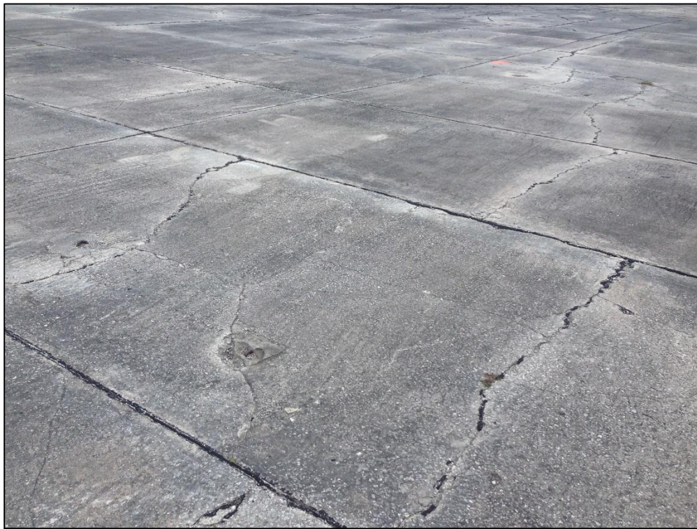
Apron SW GA, Section 4307, Sample Unit 548 – Medium Severity (63) Longitudinal, Transverse, and Diagonal Cracking, Low Severity (65) Joint Seal Damage, High Severity (72) Shattered Slab
