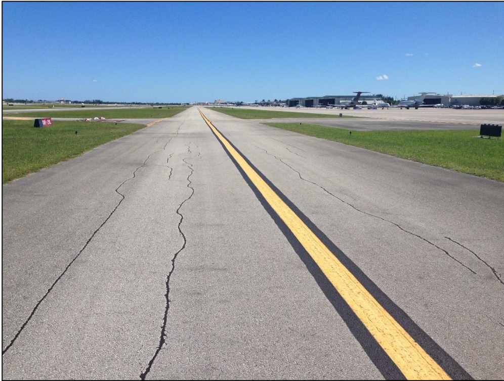
Taxiway R, Section 1805, Sample Unit 215 – Low Severity (48) Longitudinal and Transverse Cracking, Low Severity (52) Raveling
