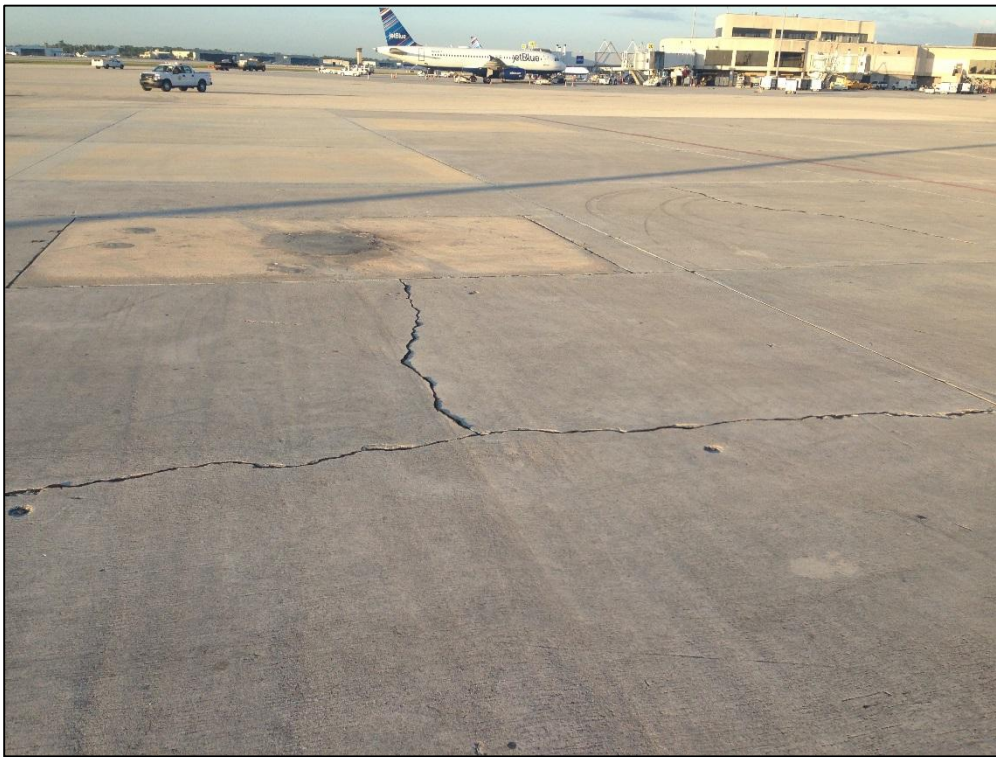
North Terminal Apron, Section 4150, Sample Unit 108 – Low Severity (63) Longitudinal, Transverse, and Diagonal Cracking, Medium Severity (63) Longitudinal, Transverse, and Diagonal Cracking, Low Severity (65) Joint Seal Damage
