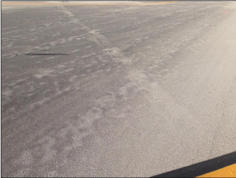
Run-Up Apron, Section 5105, Sample Unit 249 – Low Severity (48) Longitudinal and Transverse Cracking, Low Severity (56) Swelling, Medium Severity (57) Weathering
