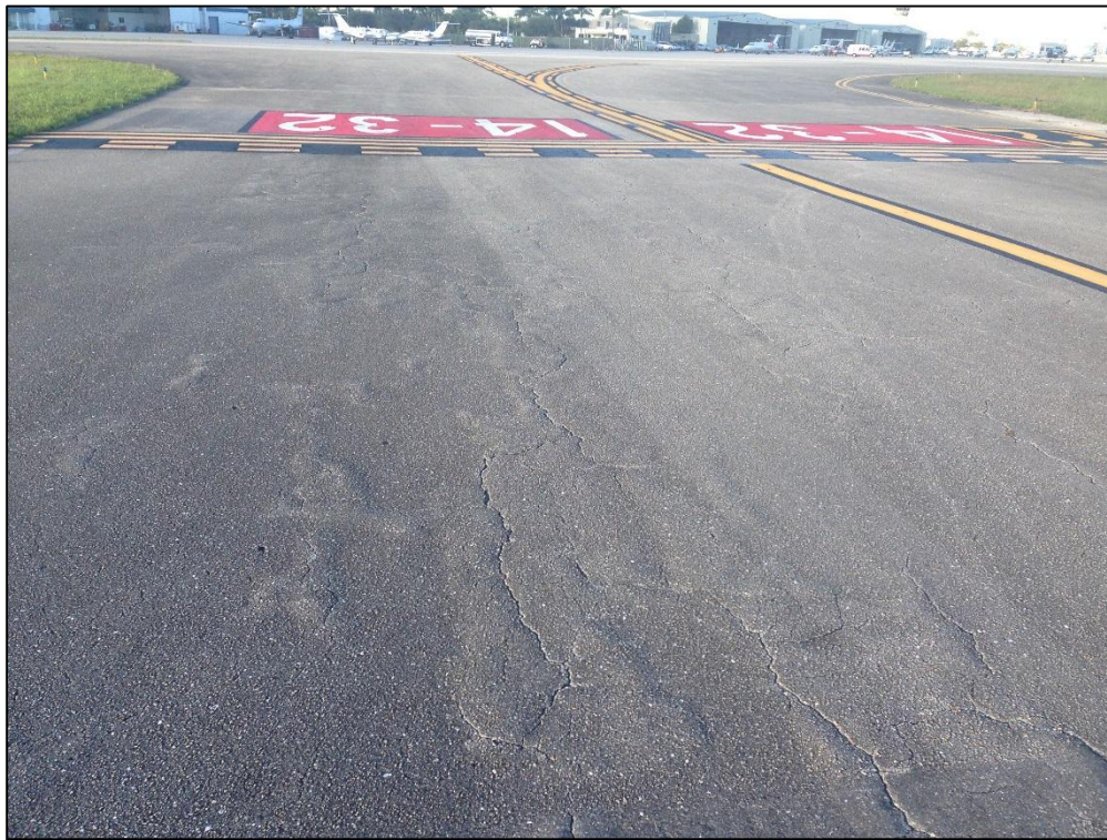
Taxiway F, Section 630, Sample Unit 103 – Medium Severity (43) Block Cracking, Low Severity (48) Longitudinal and Transverse Cracking, Low Severity (52) Raveling, Low Severity (56) Swelling
