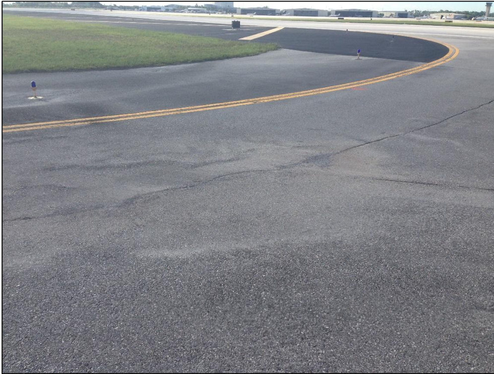
Taxiway A, Section 110, Sample Unit 802 – Low Severity (45) Depression, Low Severity (48) Longitudinal and Transverse Cracking, Medium Severity (48) Longitudinal and Transverse Cracking, Low Severity (52) Raveling, Low Severity (56) Swelling
