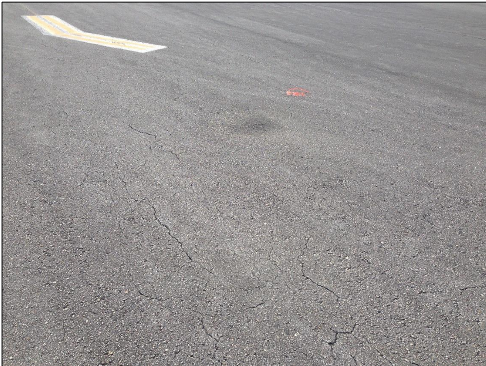
Taxiway F, Section 605, Sample Unit 124 – Low Severity (45) Depression, Low Severity (48) Longitudinal and Transverse Cracking, Low Severity (52) Raveling, Low Severity (56) Swelling
