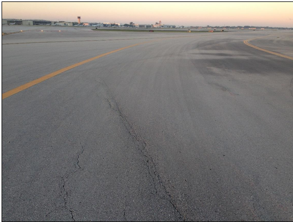
Taxiway G, Section 720, Sample Unit 100 – Low Severity (41) Alligator Cracking, Low Severity (48) Longitudinal and Transverse Cracking, Low Severity (52) Raveling, Low Severity (56) Swelling, Low Severity (57) Weathering
