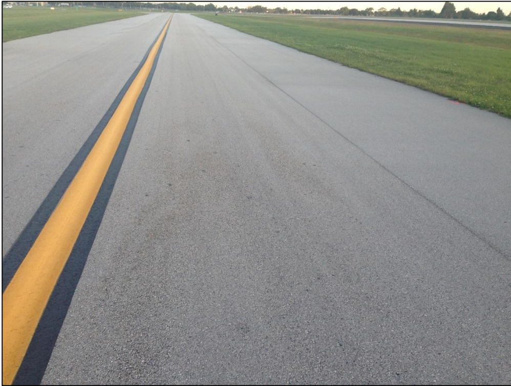
Taxiway F, Section 640, Sample Unit 115 – Low Severity (57) Weathering, Medium Severity (57) Weathering
