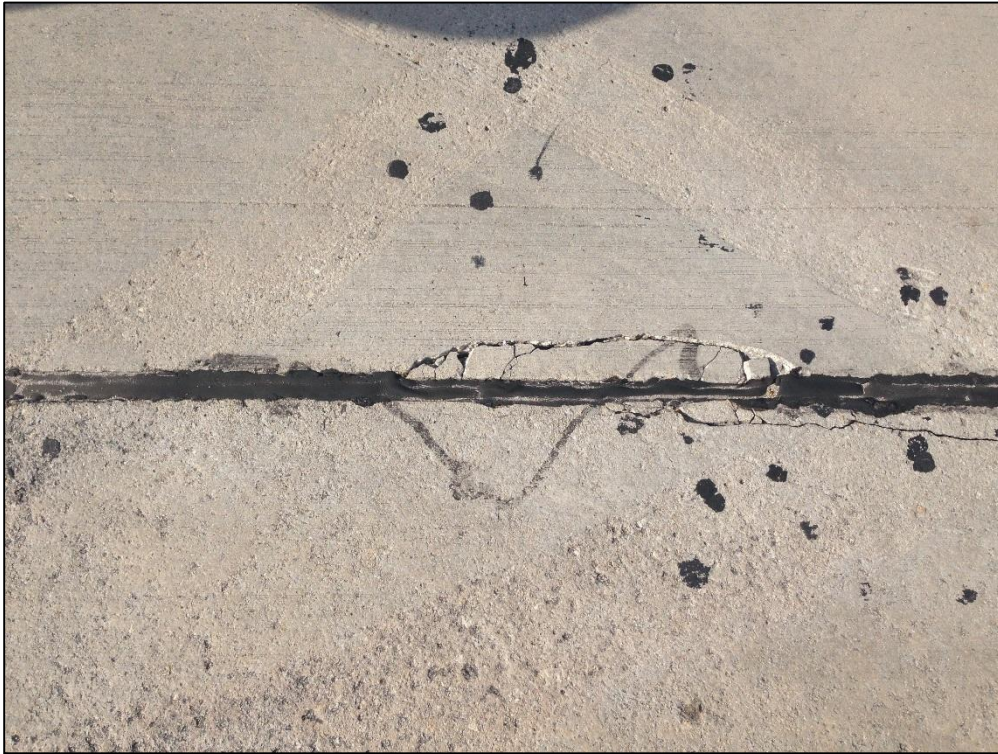
North Terminal Apron, Section 4115, Sample Unit 353 – Low Severity (74) Joint Spalling, Low Severity (65) Joint Seal Damage
