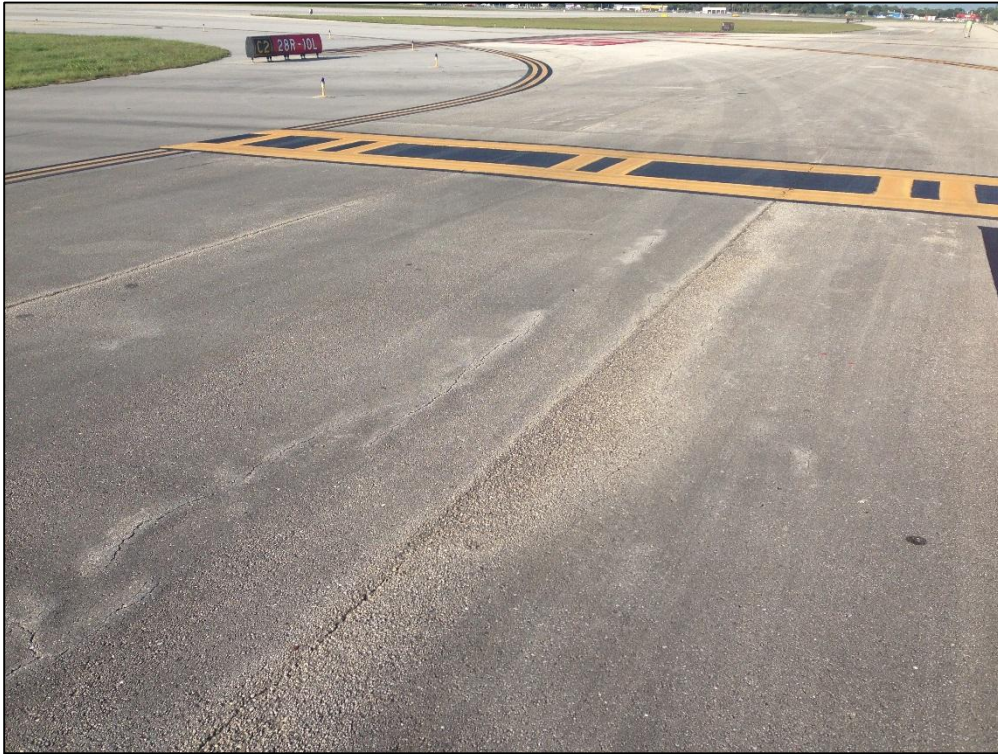
Taxiway C, Section 305, Sample Unit 108 – Low Severity (48) Longitudinal and Transverse Cracking, Low Severity (52) Raveling, Low Severity (56) Swelling, Medium Severity (57) Weathering
