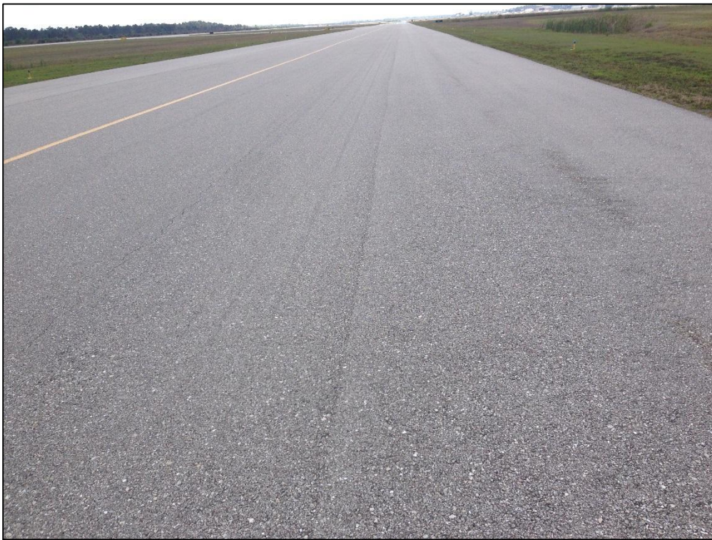
Taxiway Alpha, Section 330, Sample Unit 218 – Low Severity (48) Longitudinal and Transverse Cracking, Low Severity (52) Raveling, Low Severity (57) Weathering
