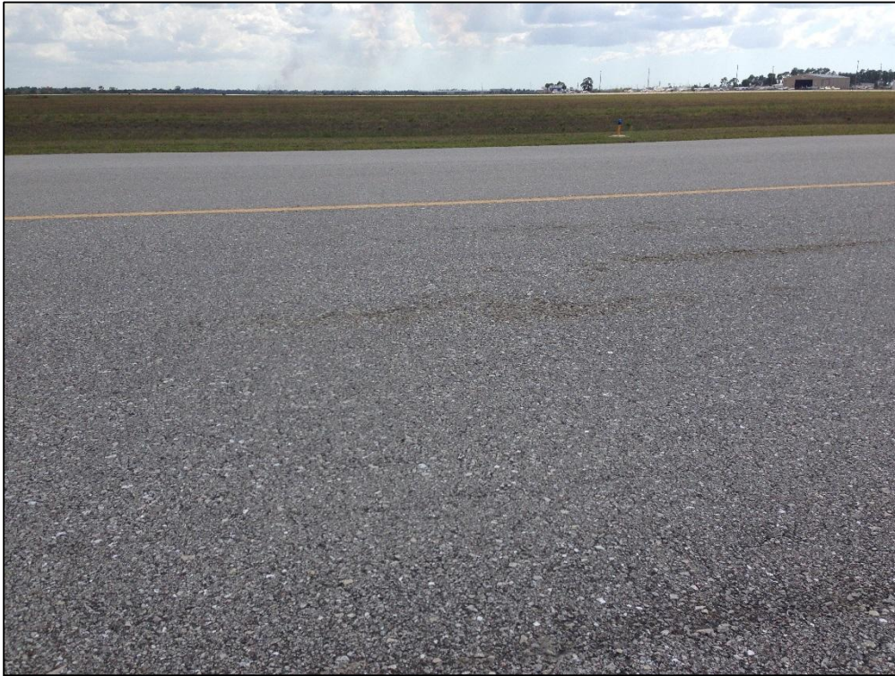
Taxiway Charlie, Section 310, Sample Unit 308 – Low Severity (48) Longitudinal and Transverse Cracking, Low Severity (52) Raveling, Low Severity (57) Weathering
