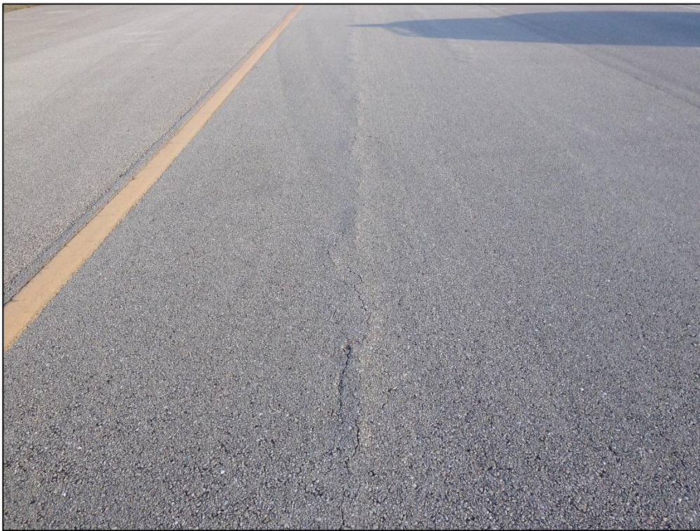
Taxiway Delta, Section 115, Sample Unit 134 – Low Severity (48) Longitudinal and Transverse Cracking, Low Severity (56) Swelling, Low Severity (57) Weathering
