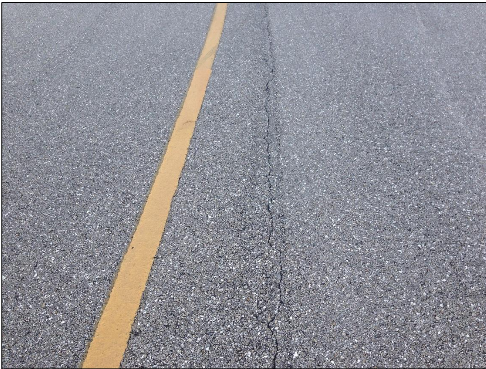
Taxiway Foxtrot, Section 1105, Sample Unit 107 – Low Severity (48) Longitudinal and Transverse Cracking, Low Severity (57) Weathering
