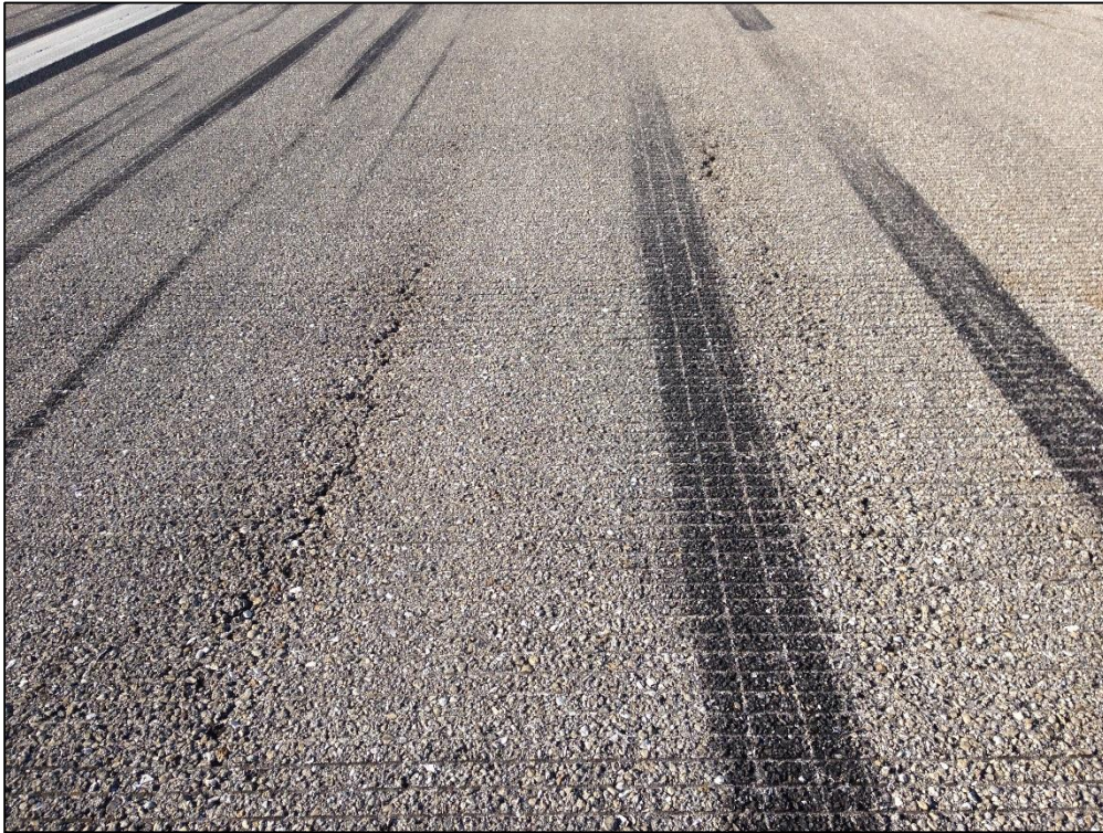
Runway 4-22, Section 6105, Sample Unit 377 – Low Severity (48) Longitudinal and Transverse Cracking, Low Severity (52) Raveling, Low Severity (57) Weathering
