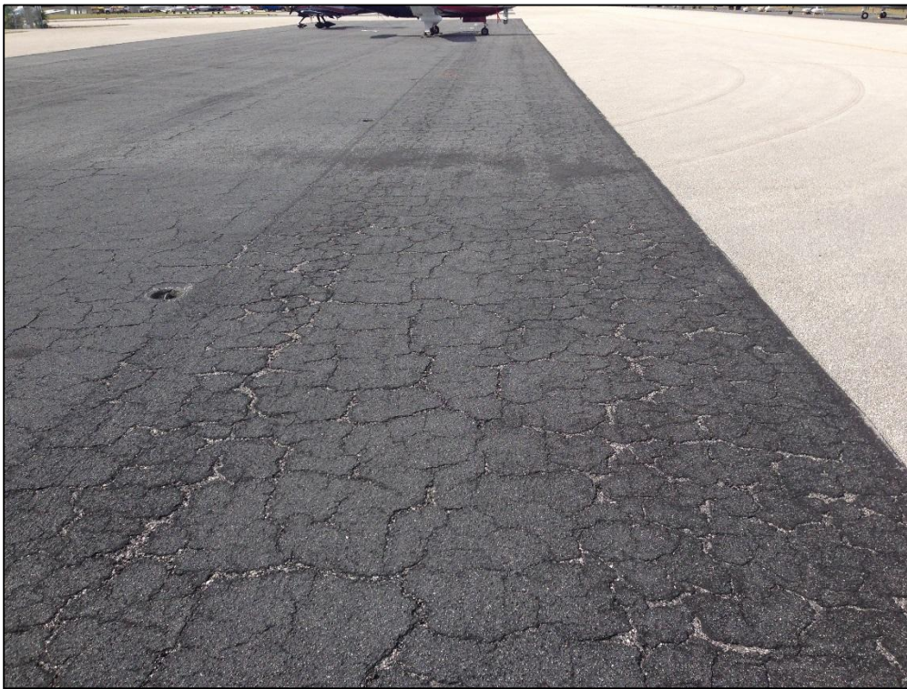
Apron South, Section 4105, Sample Unit 152 – Low Severity (43) Block Cracking, Low Severity (57) Weathering, Medium Severity (57) Weathering
