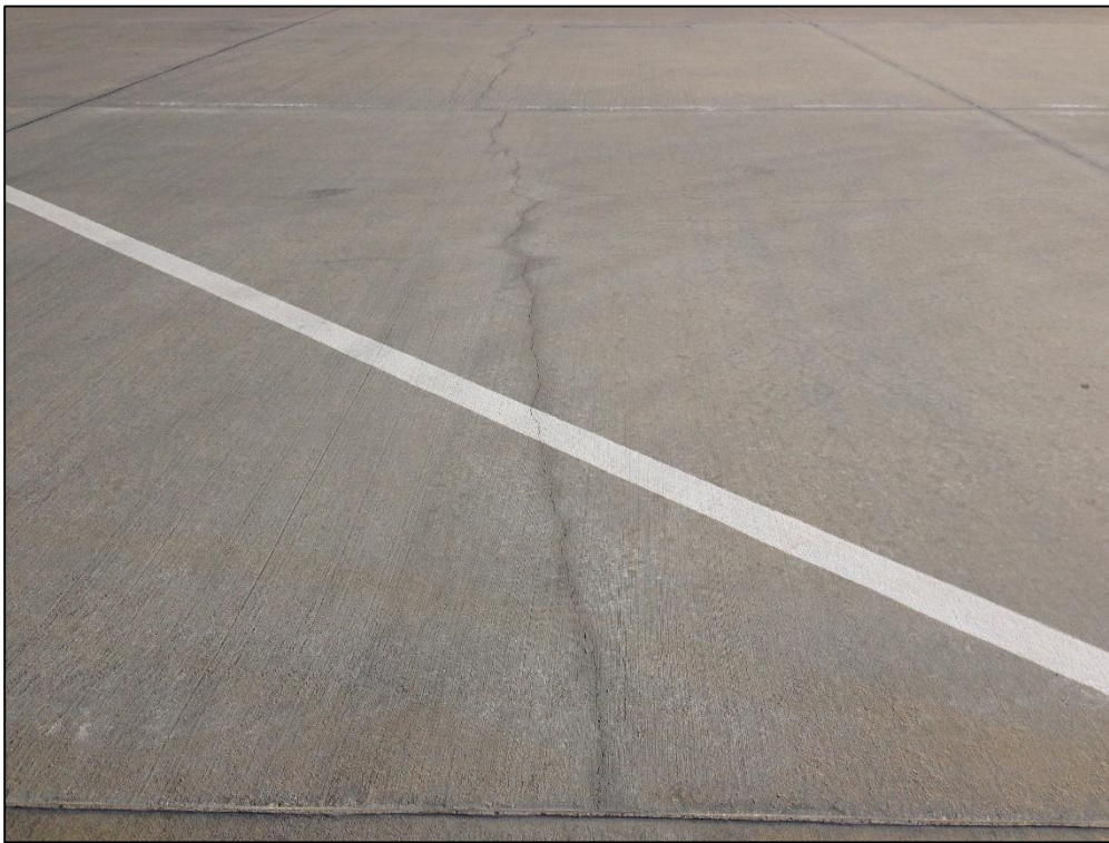
Apron Main, Section 4205, Sample Unit 200 – Low Severity (63) Longitudinal, Transverse, and Diagonal Cracking, (73) Shrinkage Cracks
