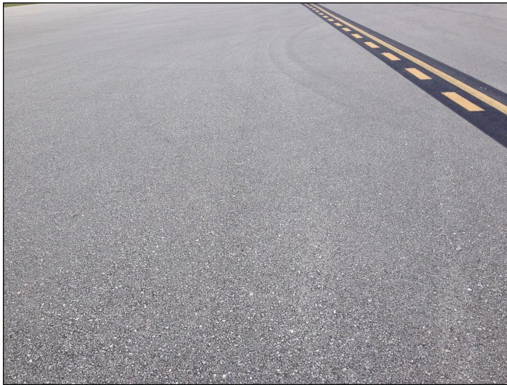
Apron Main, Section 4206, Sample Unit 93 – Low Severity (52) Raveling, Low Severity (57) Weathering
