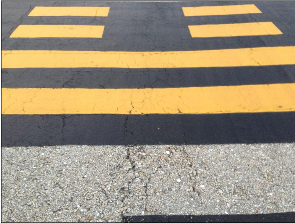
Taxiway Delta, Section 102, Sample Unit 96 – Low Severity (41) Alligator Cracking, Low Severity (52) Raveling, Low Severity (53) Rutting, Low Severity (57) Weathering
