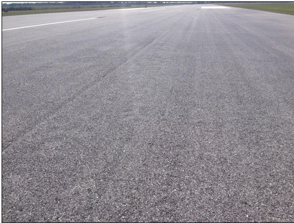
Runway 15-33, Section 6210, Sample Unit 372 – Low Severity (48) Longitudinal and Transverse Cracking, Low Severity (52) Raveling, Low Severity (56) Swelling, Low Severity (57) Weathering
