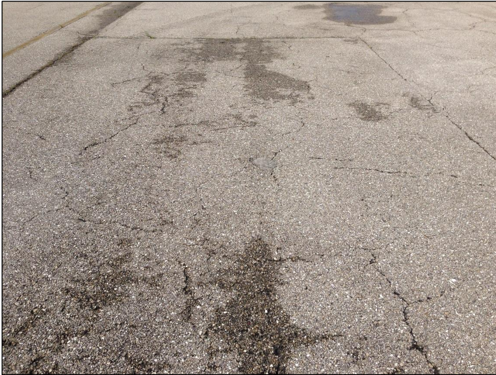
Apron North, Section 4305, Sample Unit 151 – Low Severity (43) Block Cracking, Low Severity (48) Longitudinal and Transverse Cracking, Low Severity (52) Raveling, Medium Severity (57) Weathering
