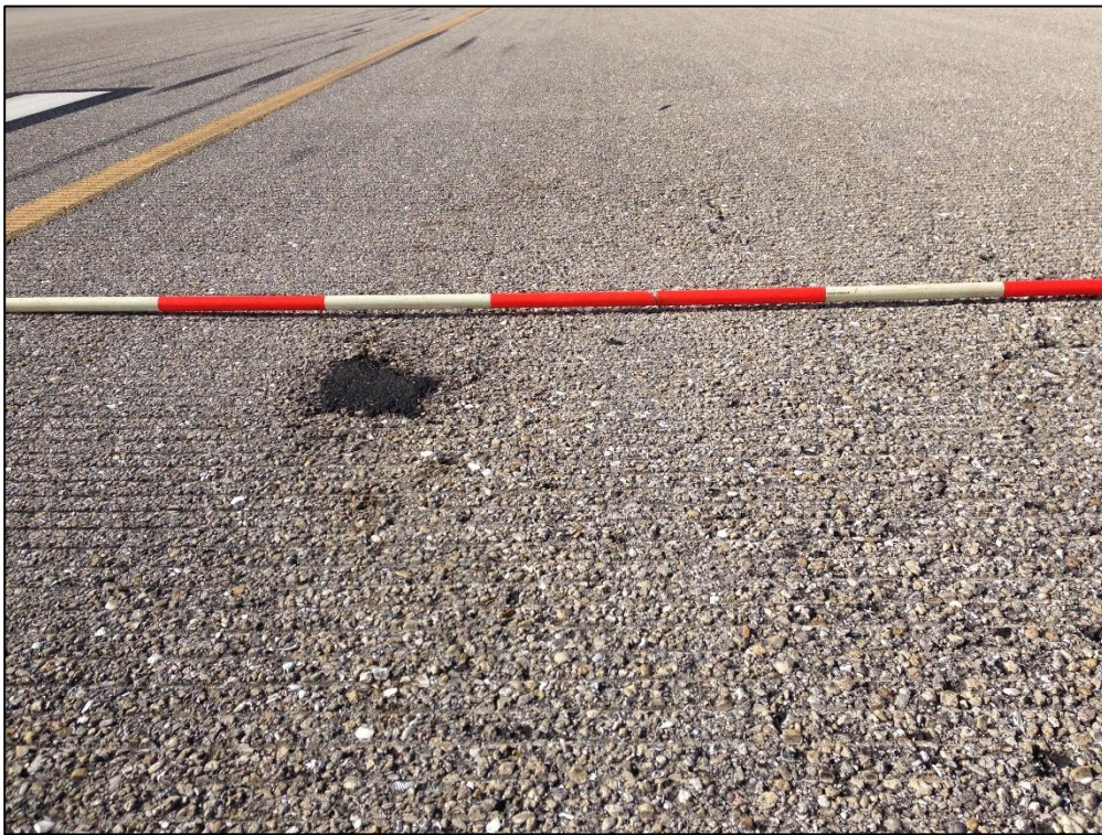
Runway 4-22, Section 6105, Sample Unit 355 – Low Severity (48) Longitudinal and Transverse Cracking, Medium Severity (50) Patching, Low Severity (52) Raveling, Medium Severity (52) Raveling, Low Severity (53) Rutting
