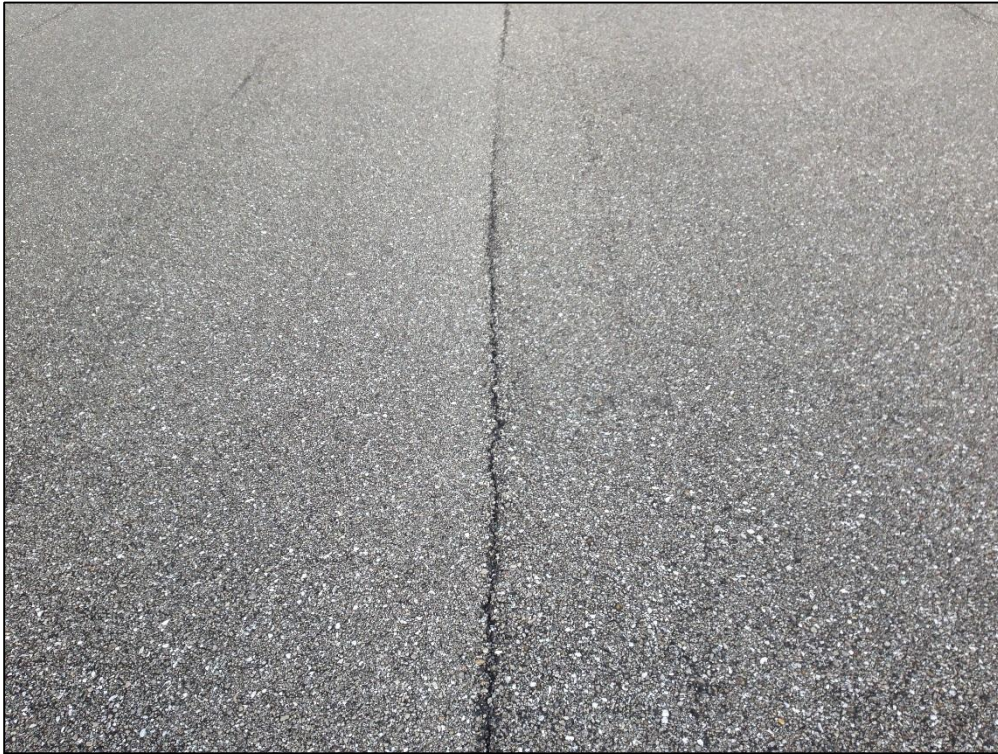
Runway 9-27, Section 6305, Sample Unit 312 – Low Severity (48) Longitudinal and Transverse Cracking, Low Severity (52) Raveling, Medium Severity (57) Weathering
