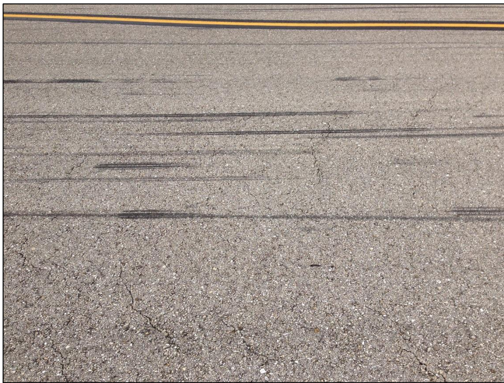
Runway 15-33, Section 6210, Sample Unit 306 – Low Severity (48) Longitudinal and Transverse Cracking, Low Severity (52) Raveling, Low Severity (57) Weathering
