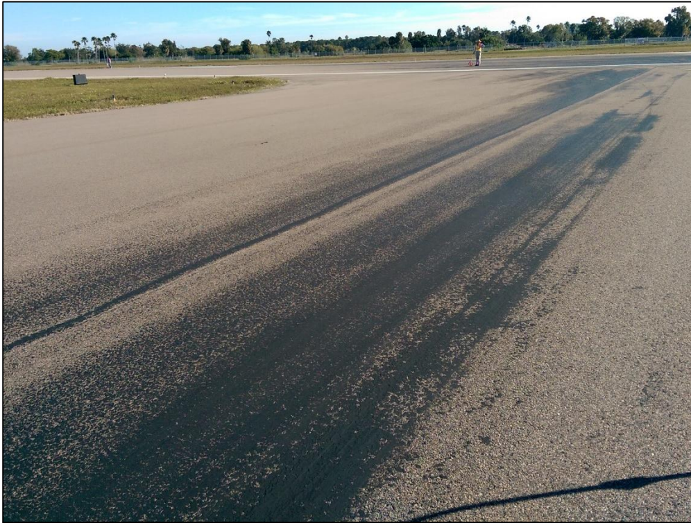
Taxiway Alpha, Section 160, Sample Unit 102 – (42) Bleeding, Low Severity (53) Rutting, Low Severity (57) Weathering
