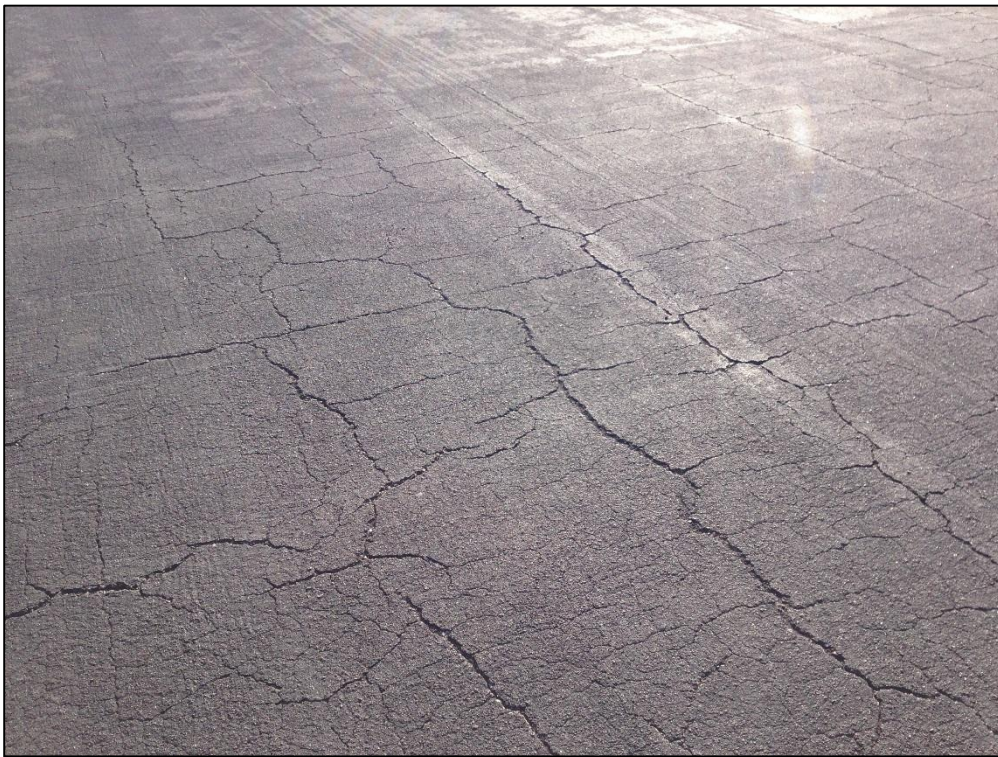
Apron Main, Section 4105, Sample Unit 322 – Low Severity (43) Block Cracking, Medium Severity (57) Weathering
