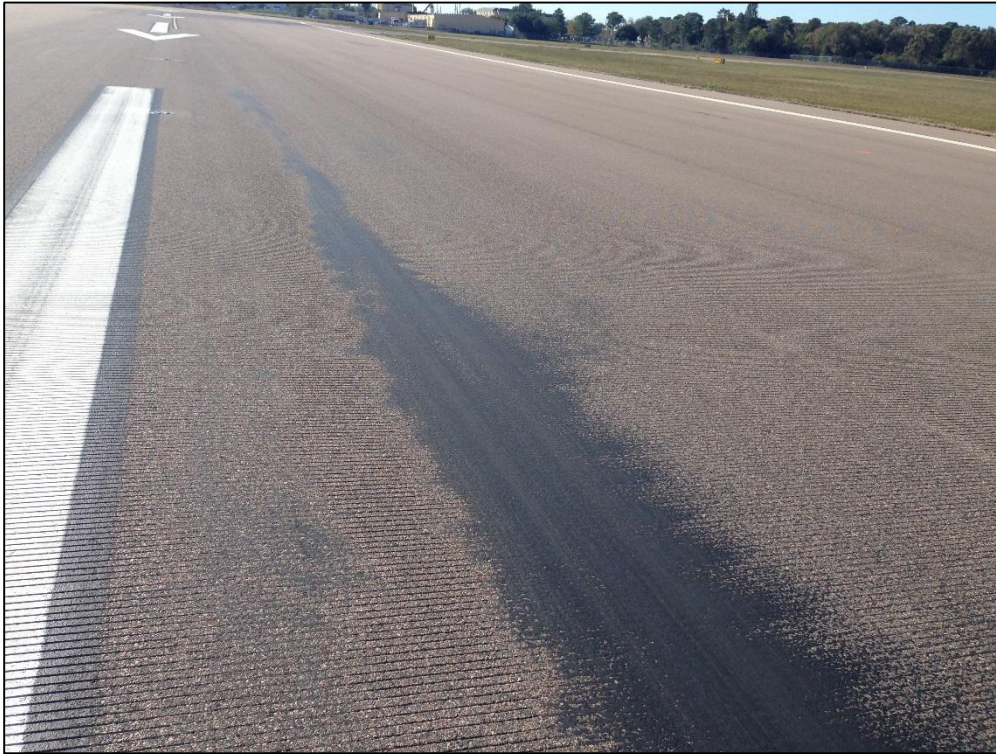
Runway 18L-36R, Section 6197, Sample Unit 286 – (42) Bleeding, Low Severity (57) Weathering
