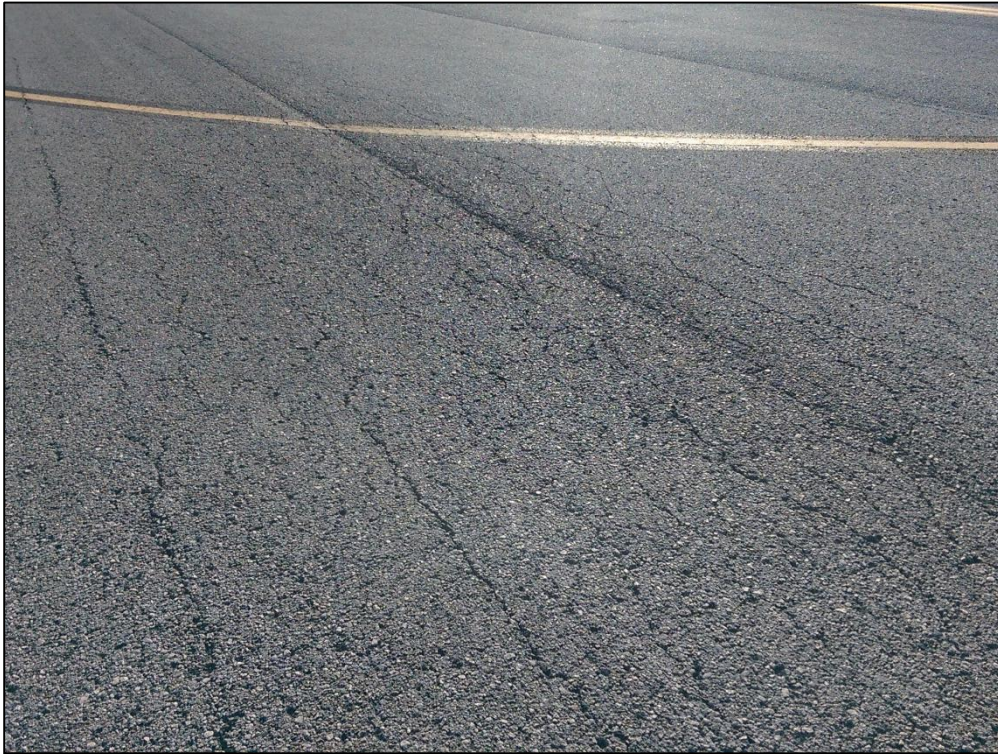
Taxiway Tango, Section 2050, Sample Unit 111 – Low Severity (41) Alligator Cracking, Low Severity (48) Longitudinal and Transverse Cracking, Low Severity (52) Raveling, Medium Severity (52) Raveling, Low Severity (53) Rutting
