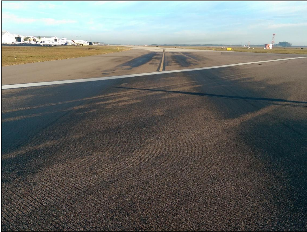
Runway 4-22, Section 6230, Sample Unit 210 – (42) Bleeding, Low Severity (53) Rutting, Low Severity (57) Weathering
