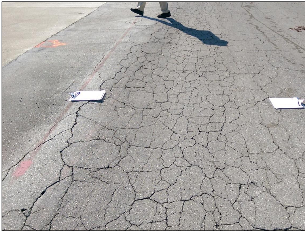
Apron Main, Section 4176, Sample Unit 805 – High Severity (41) Alligator Cracking, Low Severity (52) Raveling, High Severity (53) Rutting
