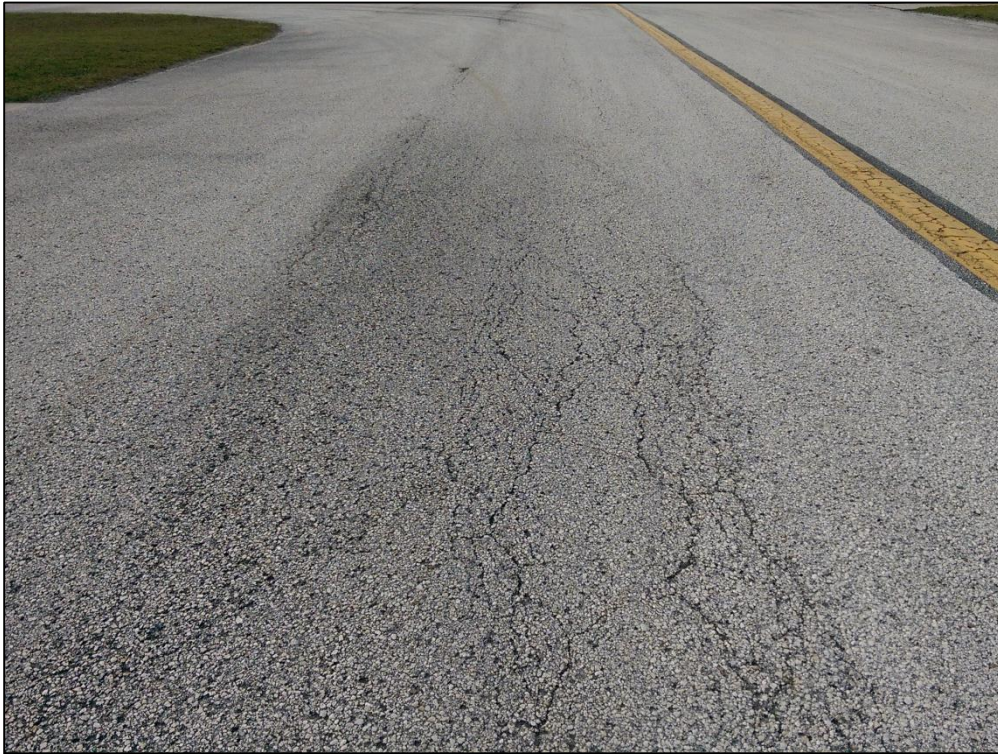
Taxiway Bravo, Section 220, Sample Unit 223 – Low Severity (41) Alligator Cracking, Medium Severity (41) Alligator Cracking, Low Severity (52) Raveling, Medium Severity (52) Raveling, Low Severity (53) Rutting
