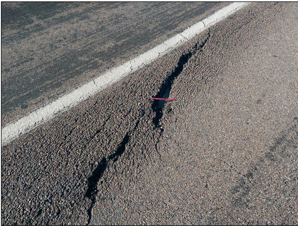
Apron Main, Section 4105, Sample Unit 109 – (55) Slippage Cracking, Low Severity (57) Weathering
