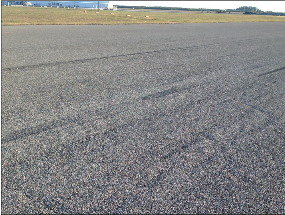
Runway 9-27, Section 6365, Sample Unit 390 – Low Severity (48) Longitudinal and Transverse Cracking, Low Severity (52) Raveling, Low Severity (56) Swelling
