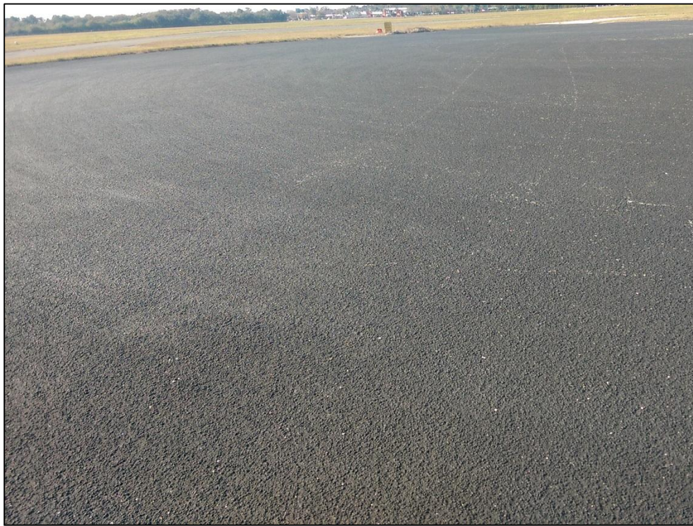
Apron Main, Section 4180, Sample Unit 100 – Medium Severity (52) Raveling
