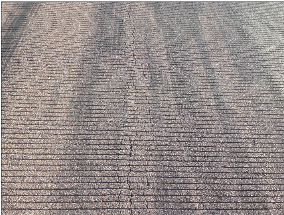
Runway 18L-36R, Section 6185, Sample Unit 449 – Low Severity (41) Alligator Cracking, Low Severity (48) Longitudinal and Transverse Cracking, Low Severity (57) Weathering
