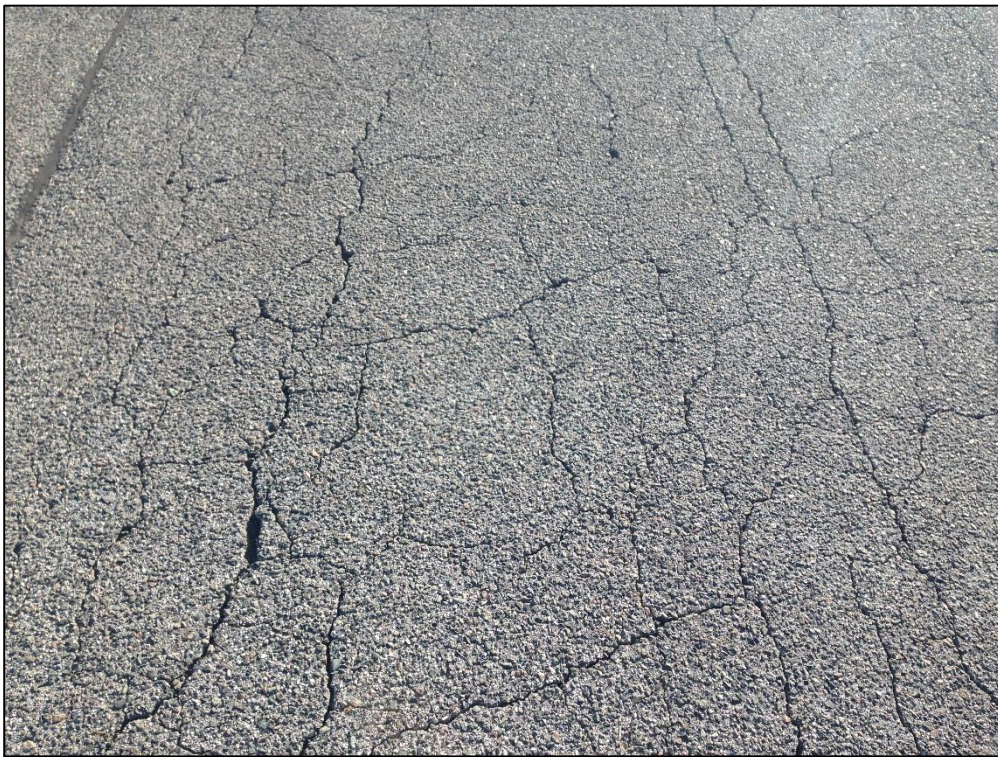
Runway 9-27, Section 6345, Sample Unit 369 – Medium Severity (41) Alligator Cracking, Low Severity (52) Raveling
