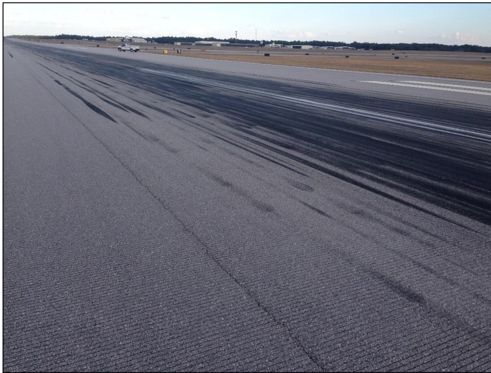
Runway 8-26, Section 6215, Sample Unit 330 – Low Severity (48) Longitudinal and Transverse Cracking, Low Severity (57) Weathering
