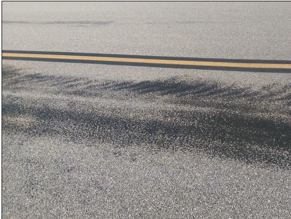
Taxiway A7, Section 215, Sample Unit 400 – (42) Bleeding, Low Severity (57) Weathering
