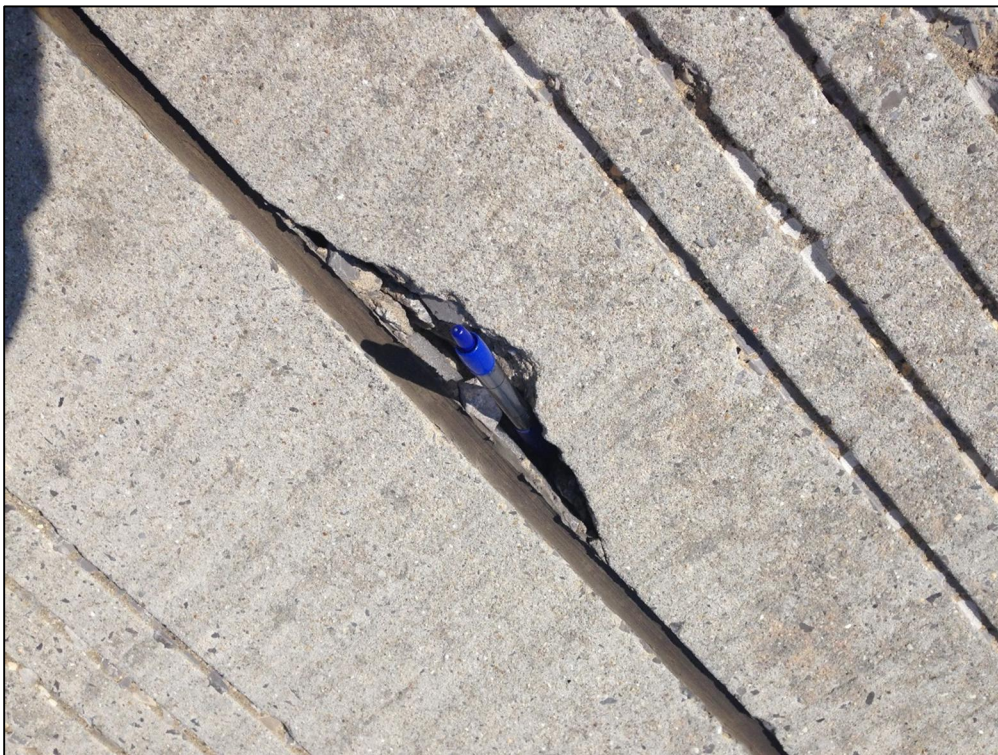
Runway 17-35, Section 6105, Sample Unit 346 – Medium Severity (74) Joint Spalling
