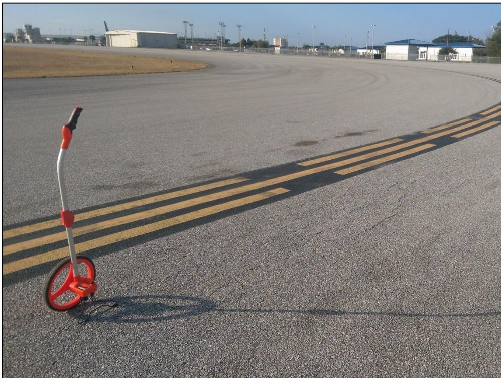
Taxiway A1, Section 120, Sample Unit 102 – Low Severity (41) Alligator Cracking, Low Severity (53) Rutting, Low Severity (57) Weathering
