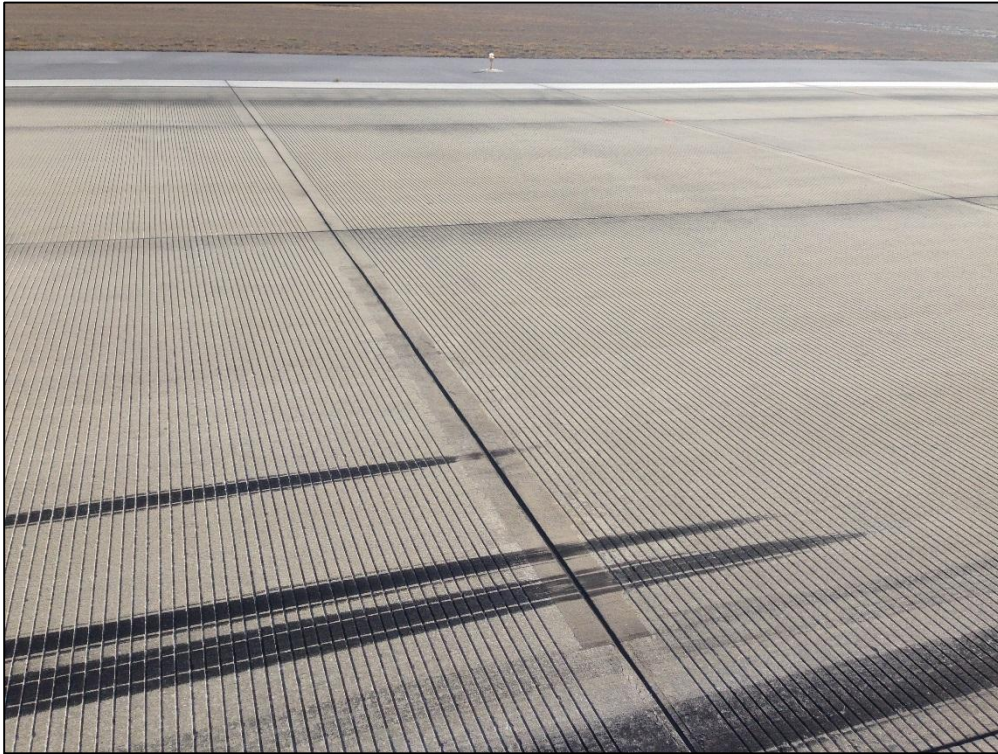
Runway 17-35, Section 6125, Sample Unit 402 – Low Severity (66) Small Patching
