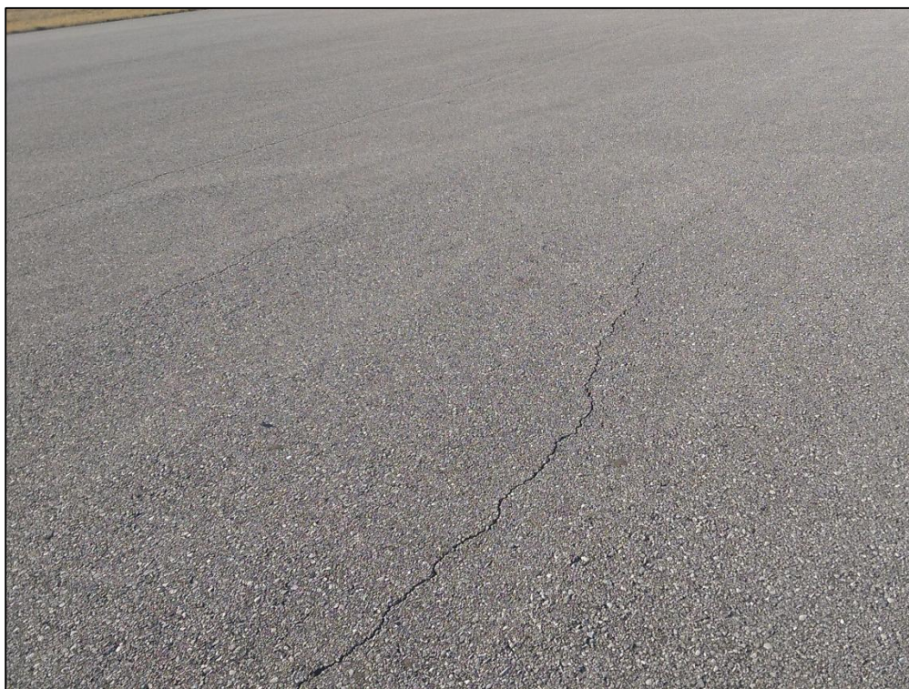
Taxiway Delta, Section 410, Sample Unit 601 – Low Severity (48) Longitudinal and Transverse Cracking, Low Severity (57) Weathering
