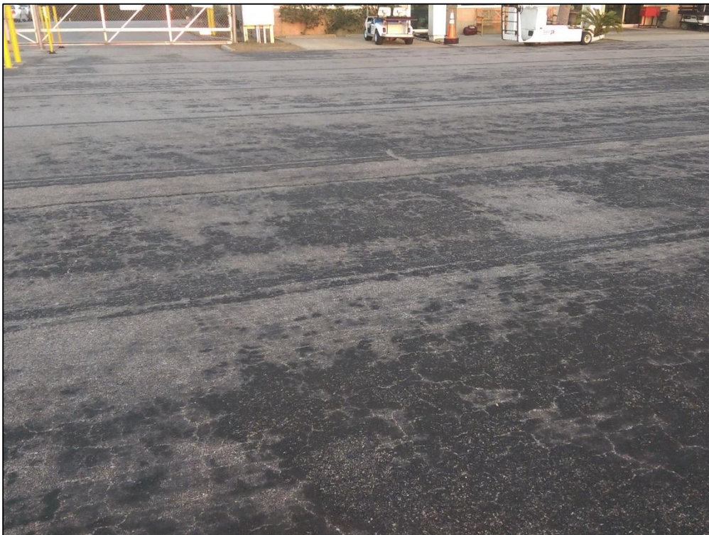
Apron South, Section 4510, Sample Unit 502 – Low Severity (43) Block Cracking, Low Severity (52) Raveling, Medium Severity (52) Raveling
