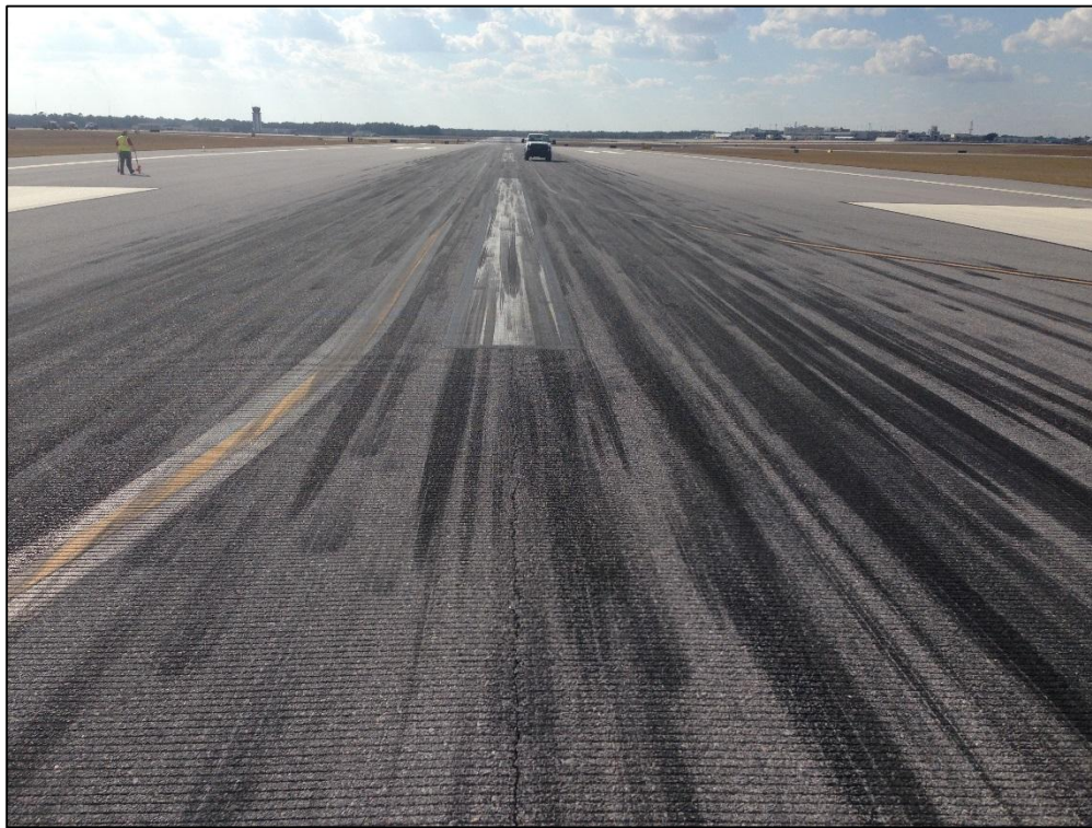
Runway 8-26, Section 6255, Sample Unit 418 – Low Severity (48) Longitudinal and Transverse Cracking, Low Severity (52) Raveling, Low Severity (57) Weathering
