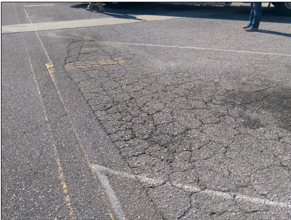
Terminal Apron, Section 4230, Sample Unit 101 – High Severity (41) Alligator Cracking, Low Severity (52) Raveling, Medium Severity (52) Raveling
