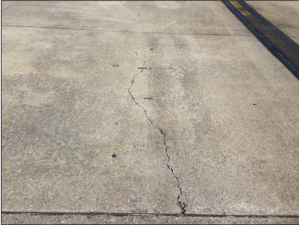
Terminal Apron, Section 4210, Sample Unit 803 – Low Severity (63) Longitudinal, Transverse, and Diagonal Cracking
