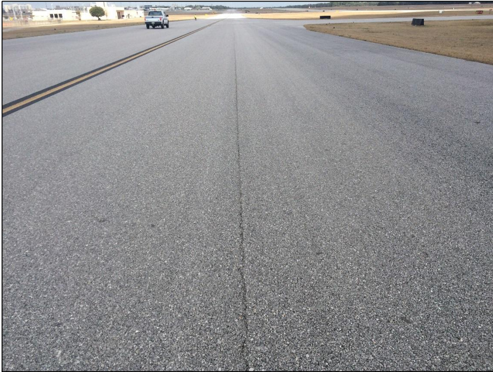
Taxiway Alpha, Section 105, Sample Unit 115 – Low Severity (48) Longitudinal and Transverse Cracking, Low Severity (52) Raveling, Low Severity (57) Weathering
