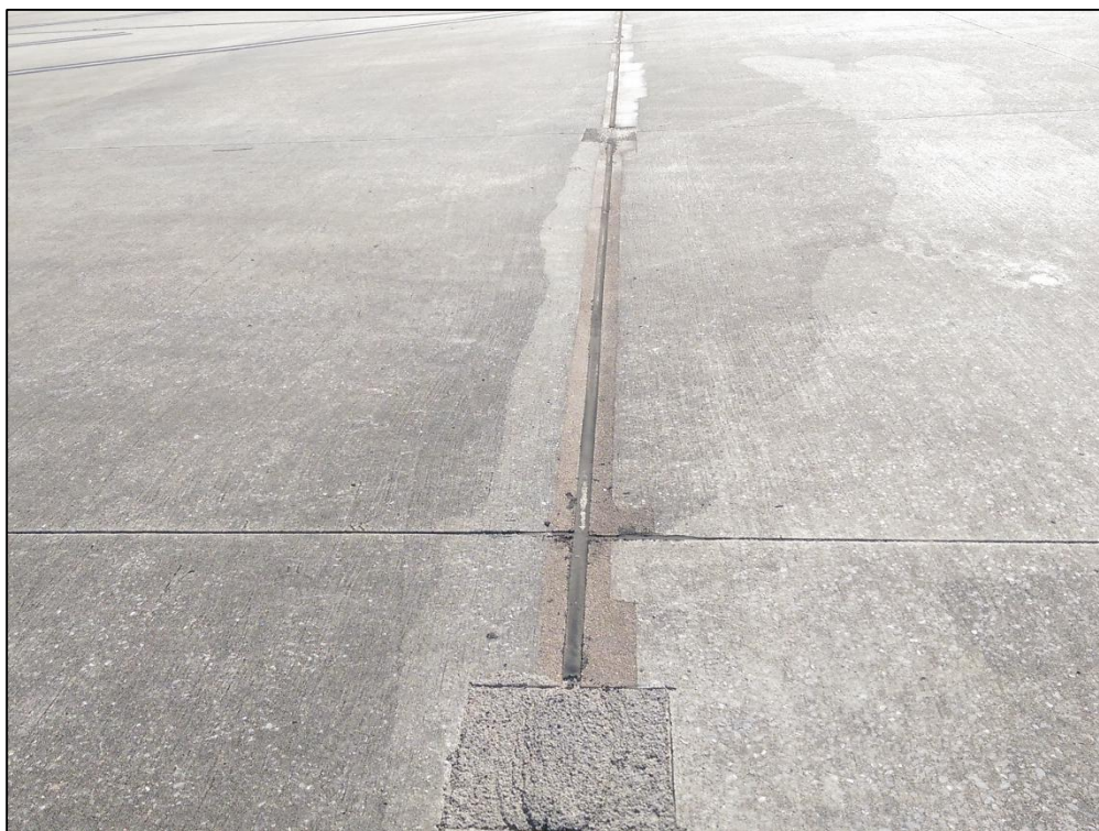
Terminal Apron, Section 4235, Sample Unit 936 – Low Severity (66) Small Patching, Low Severity (67) Large Patching
