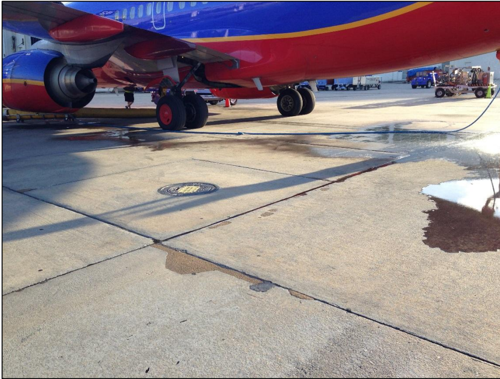
Apron South, Section 4430, Sample Unit 102 – Low Severity (66) Small Patching
