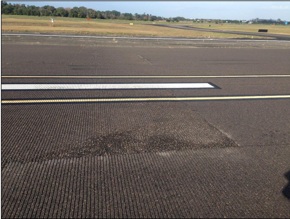
Runway 18-36, Section 6205, Sample Unit 312 – Low Severity (48) Longitudinal and Transverse Cracking, Low Severity (52) Raveling, High Severity (52) Raveling
