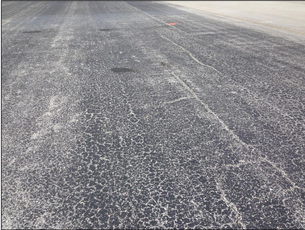
FBO Apron, Section 4305, Sample Unit 305 – Low Severity (43) Block Cracking, Low Severity (52) Raveling
