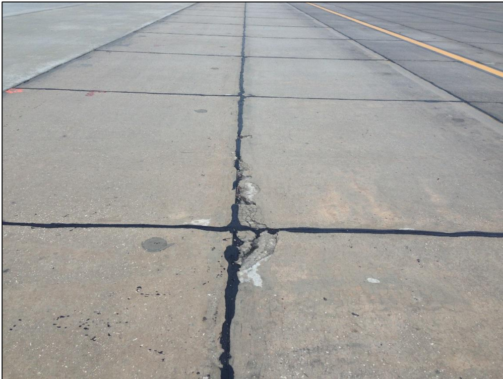
Apron SW, Section 4227, Sample Unit 510 – Low Severity (65) Joint Seal Damage, Low Severity (70) Scaling, Map Cracking, Cracking, Medium Severity (74) Joint Spalling, High Severity (74) Joint Spalling, High Severity (75) Corner Spalling
