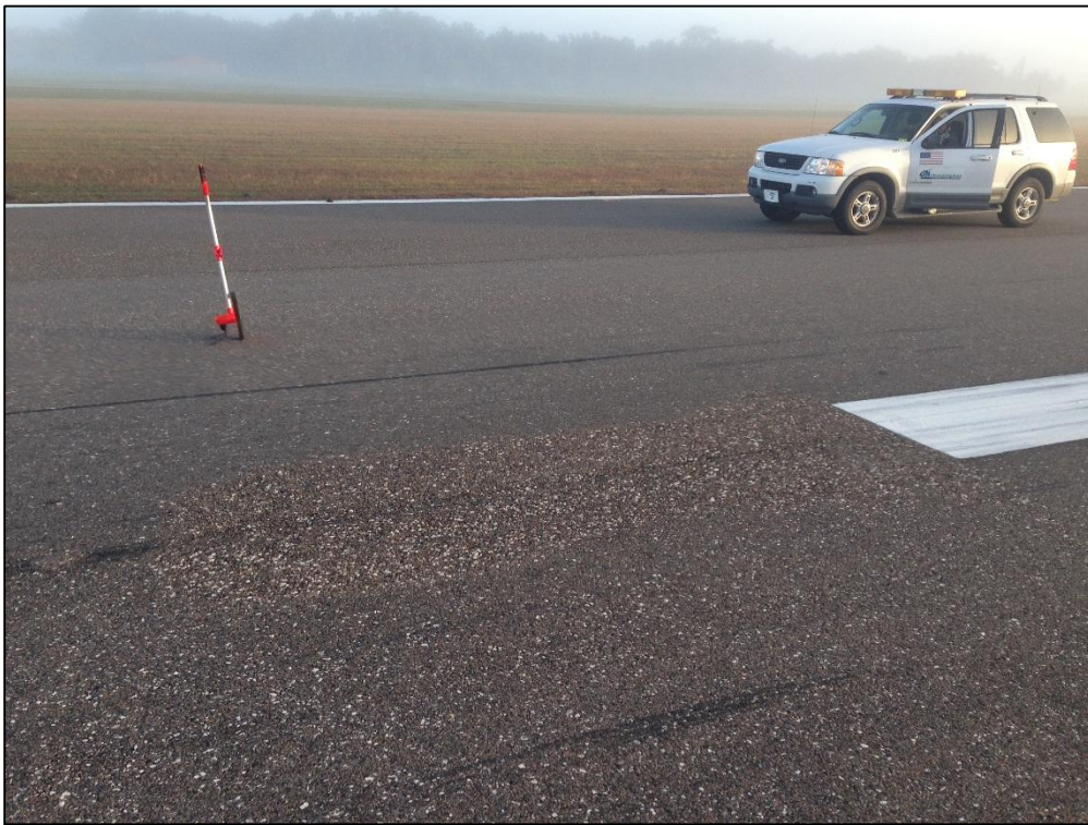
Runway 9R-27L, Section 6410, Sample Unit 221 – Low Severity (52) Raveling, Low Severity (57) Weathering
