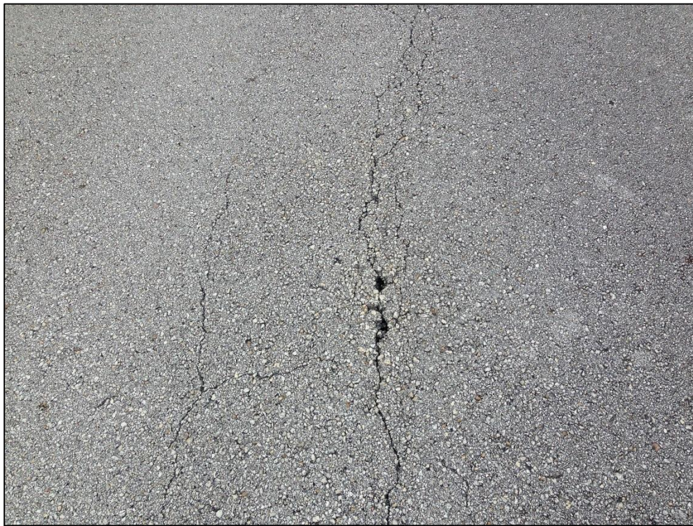
Taxiway Charlie, Section 315, Sample Unit 308 – Low Severity (41) Alligator Cracking, Low Severity (48) Longitudinal and Transverse Cracking, Low Severity (57) Weathering
