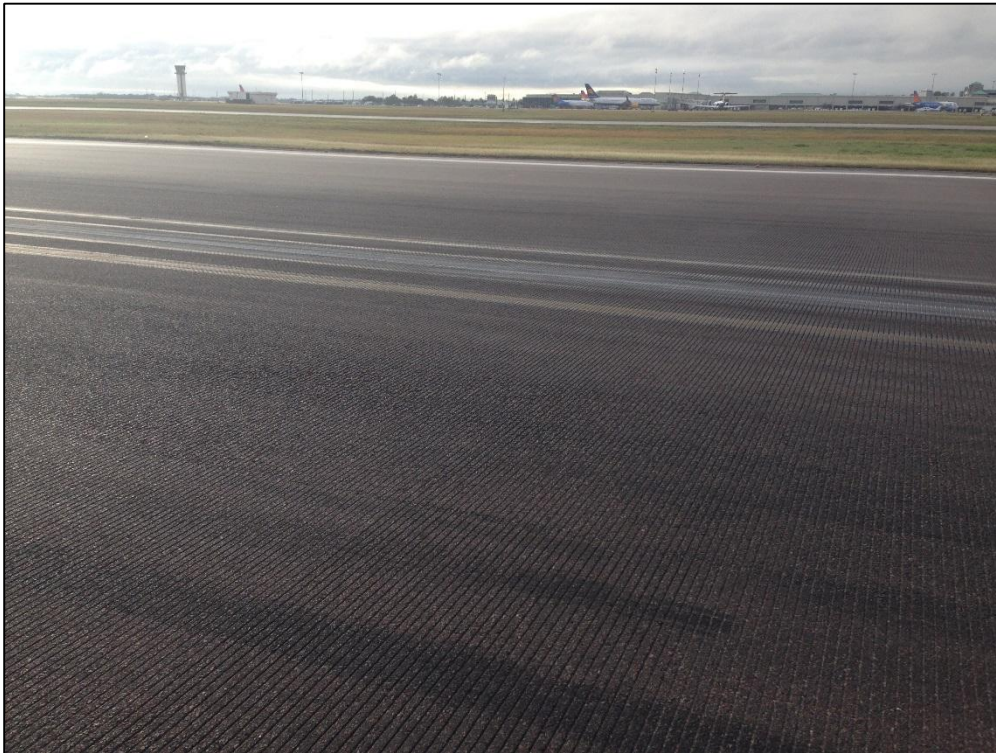
Runway 9L-27R, Section 6105, Sample Unit 352 – Low Severity (57) Weathering, High Severity (57) Weathering
