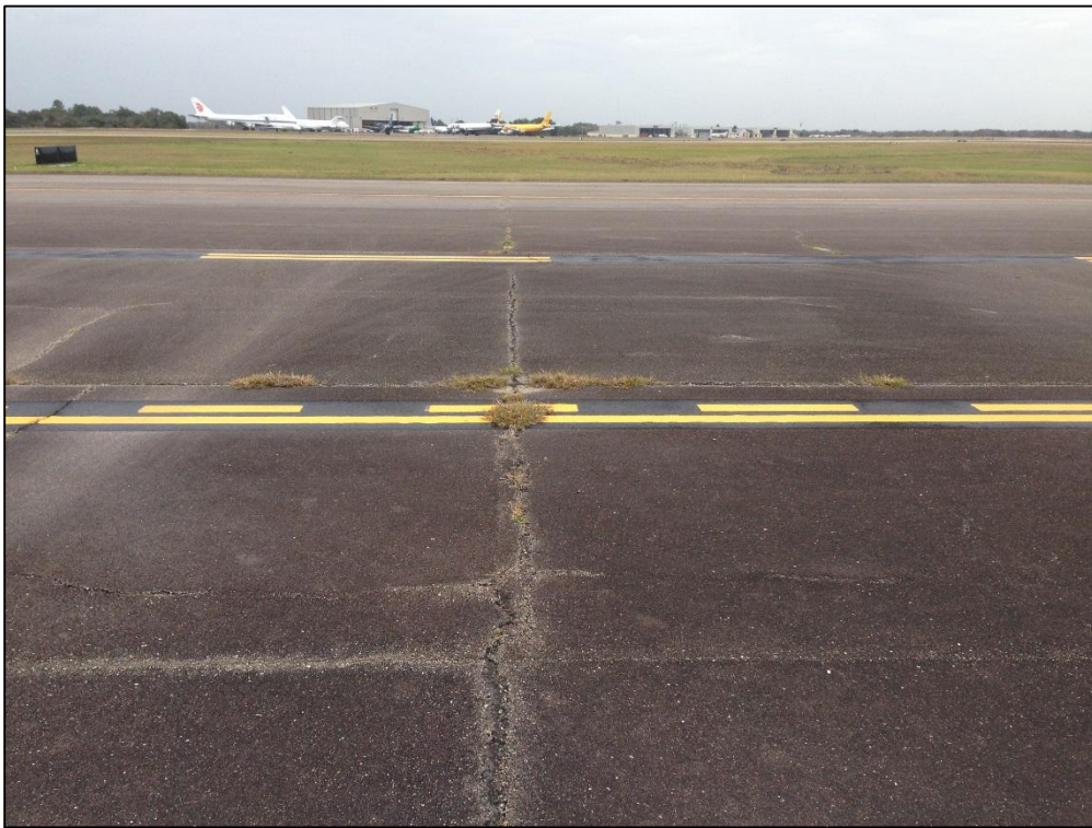
Apron Southwest, Section 4270, Sample Unit 100 – Low and Medium Severity (48) Longitudinal and Transverse Cracking, Low Severity (52) Raveling, Low Severity (57) Weathering
