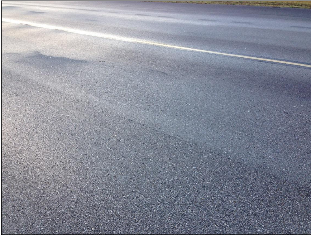
Taxiway Bravo, Section 204, Sample Unit 317 – Low Severity (48) Longitudinal and Transverse Cracking, Low Severity (57) Weathering
