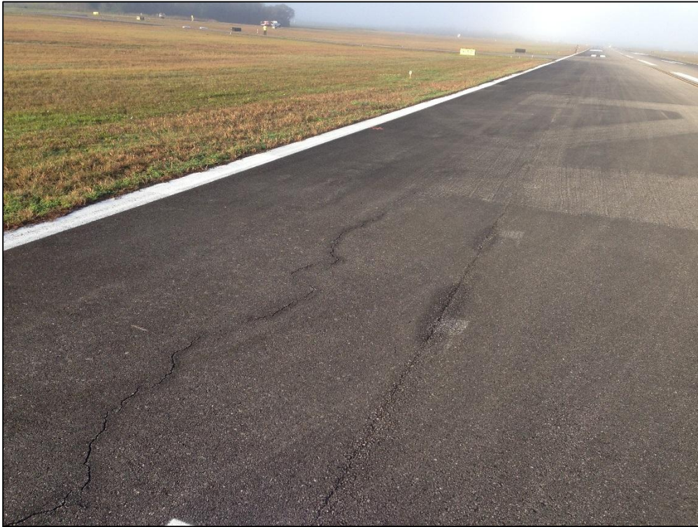
Runway 9R-27L, Section 6405, Sample Unit 172 – Low Severity (48) Longitudinal and Transverse Cracking, Low Severity (52) Raveling, Medium Severity (52) Raveling, Low Severity (57) Weathering
