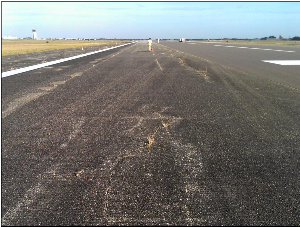
Runway 18-36, Section 6210, Sample Unit 104 – Low Severity (48) Longitudinal and Transverse Cracking, Low Severity (52) Raveling, Low Severity (56) Swelling, Low Severity (57) Weathering
