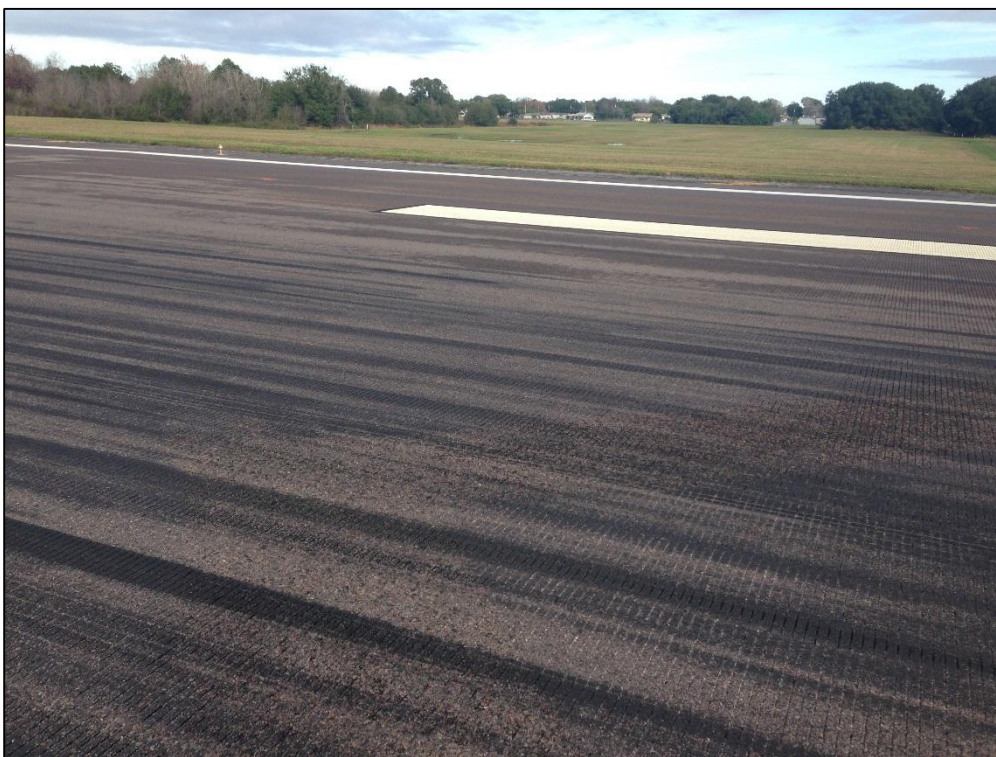
Runway 9L-27R, Section 6105, Sample Unit 448 – Low Severity (52) Raveling, Low Severity (57) Weathering
