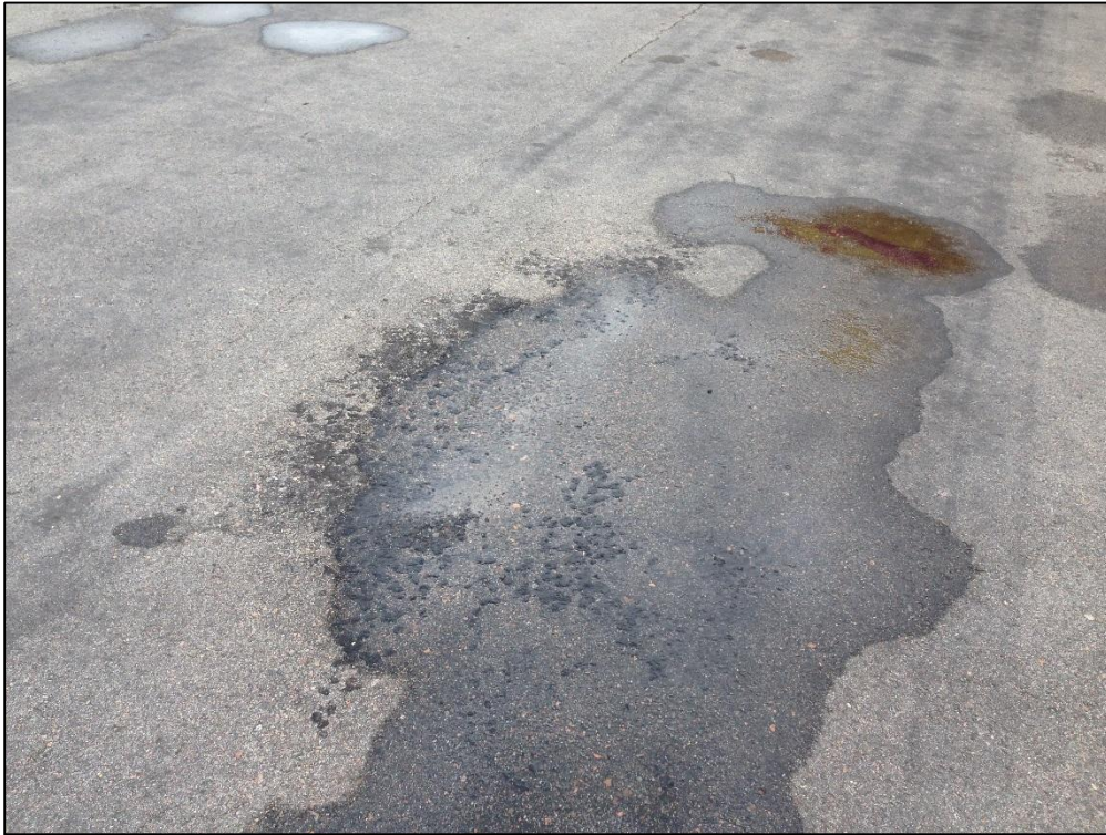
Apron North, Section 4310, Sample Unit 355 – (42) Bleeding, Low Severity (48) Longitudinal and Transverse Cracking, (49) Oil Spillage, Low Severity (57) Weathering
