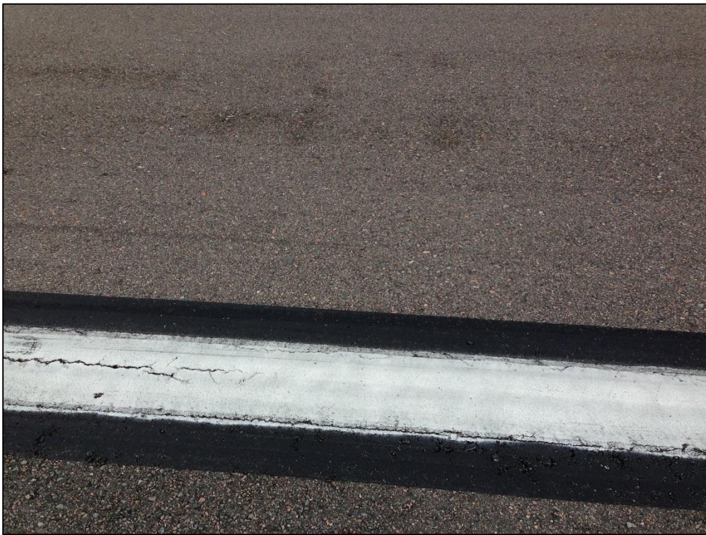
Runway 9C-27C, Section 6305, Sample Unit 104 – Low Severity (48) Longitudinal and Transverse Cracking, Low Severity (57) Weathering, Medium Severity (57) Weathering
