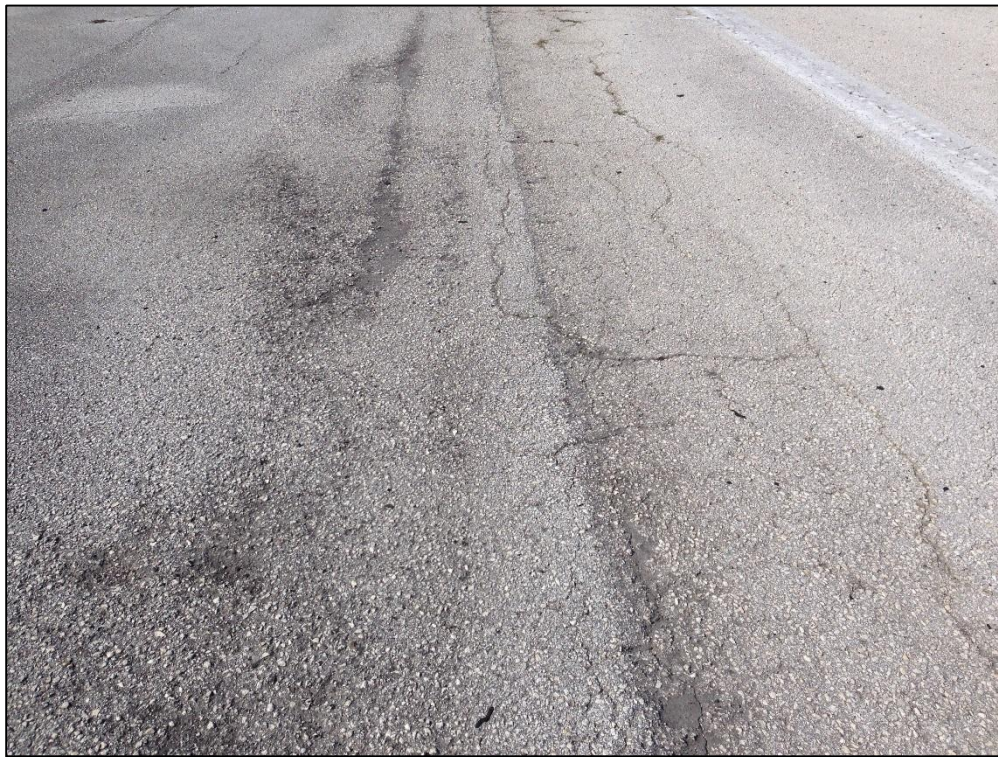
Taxiway Charlie, Section 310, Sample Unit 101 – Low Severity (43) Block Cracking, Low Severity (48) Longitudinal and Transverse Cracking, Low Severity (52) Raveling, Medium Severity (52) Raveling
