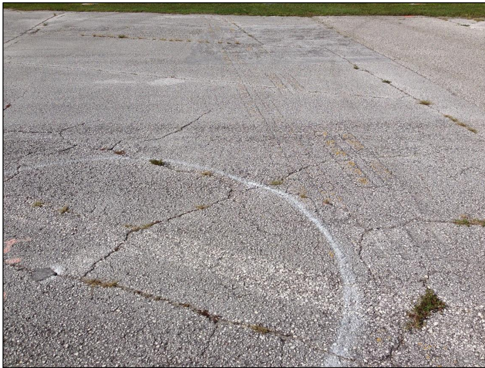
Taxiway A1, Section 610, Sample Unit 101 – Low Severity (43) Block Cracking, Low Severity (50) Patching, Low Severity (52) Raveling, Medium Severity (52) Raveling
