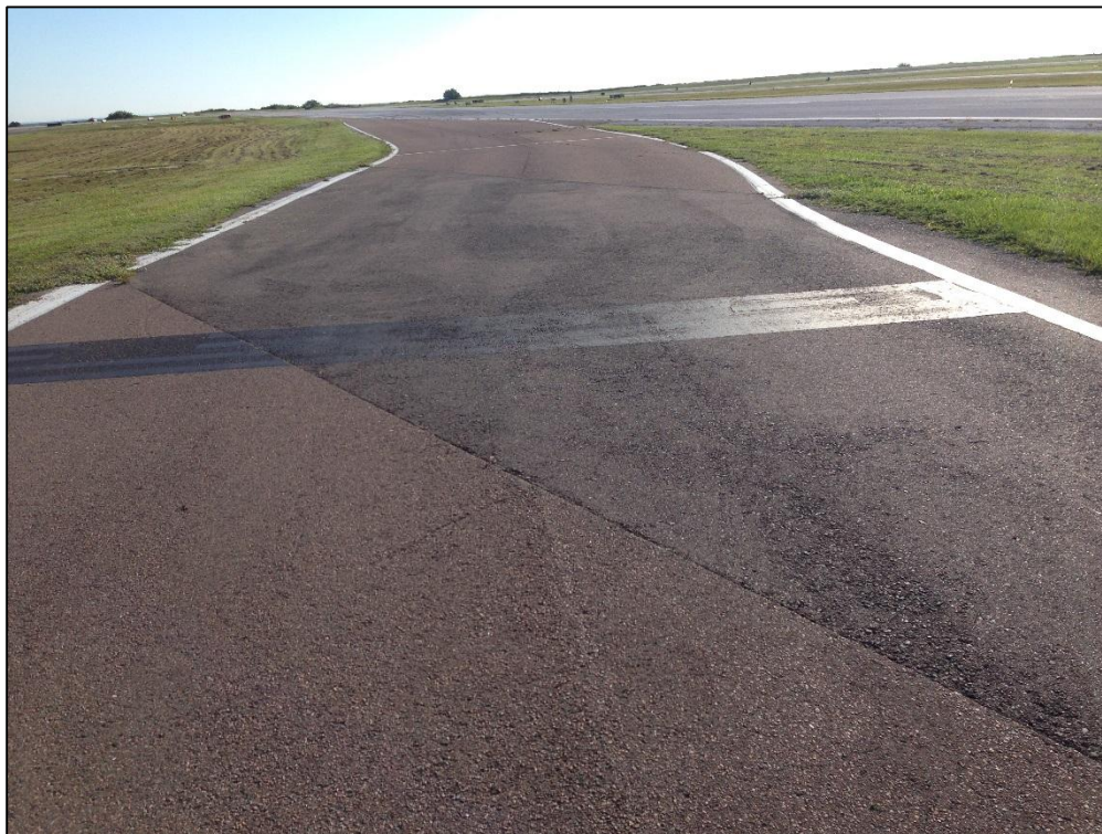
Taxiway November, Section 720, Sample Unit 103 – Low Severity (48) Longitudinal and Transverse Cracking, Low Severity (50) Patching, Low Severity (52) Raveling
