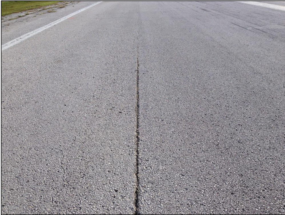
Runway 7-25, Section 6210, Sample Unit 151 – Low Severity (48) Longitudinal and Transverse Cracking, Medium Severity (48) Longitudinal and Transverse Cracking, Low Severity (52) Raveling
