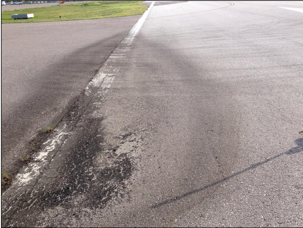
Runway 7-25, Section 6205, Sample Unit 173 – Low Severity (45) Depression, Low Severity (52) Raveling
