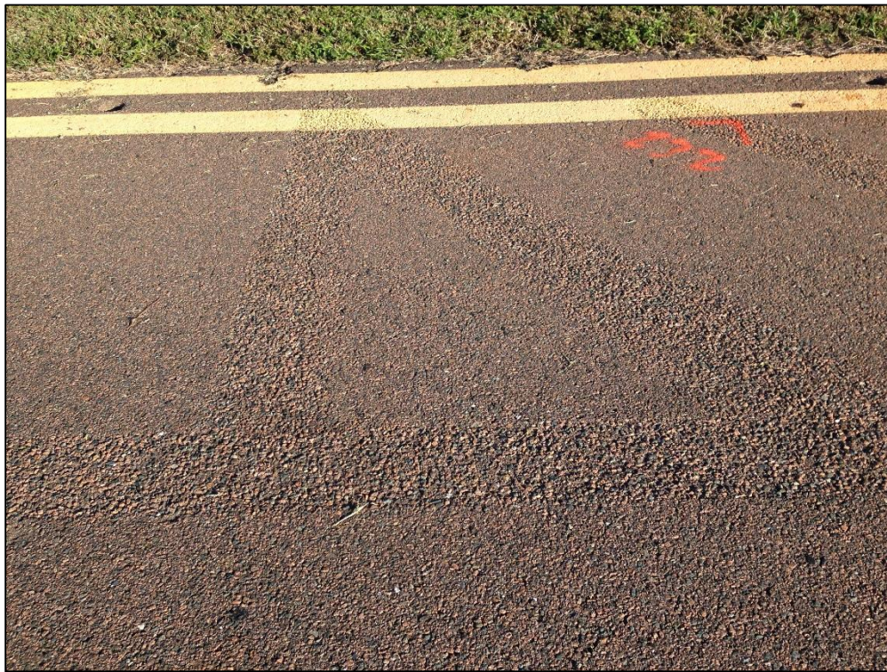
Taxiway Delta, Section 510, Sample Unit 232 – Low Severity (52) Raveling
