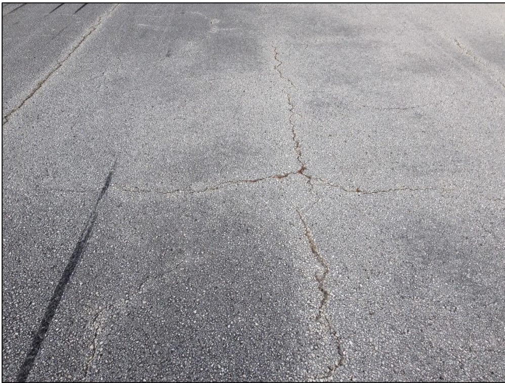
Runway 7-25, Section 6210, Sample Unit 114 – Low Severity (43) Block Cracking, Low Severity (48) Longitudinal and Transverse Cracking, Low Severity (52) Raveling
