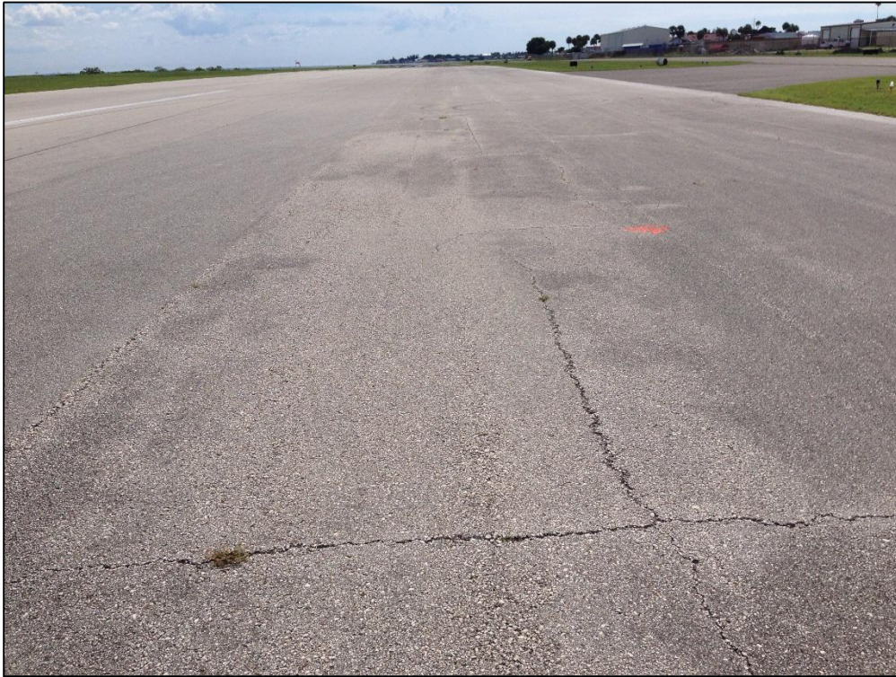
Runway 18-36, Section 6105, Sample Unit 330 – Low Severity (43) Block Cracking, Low Severity (48) Longitudinal and Transverse Cracking, Low Severity (52) Raveling
