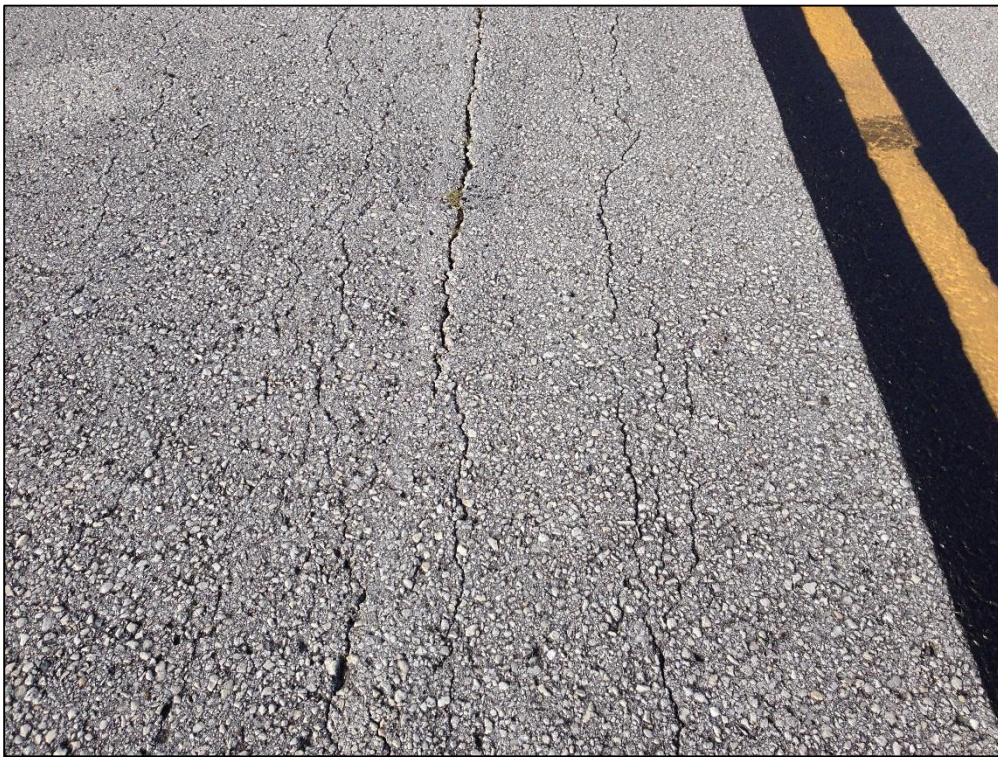
Runway 7-25, Section 6207, Sample Unit 166 – Low Severity (41) Alligator Cracking, Low Severity (48) Longitudinal and Transverse Cracking, Low Severity (52) Raveling
