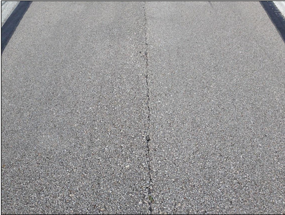
Runway 7-25, Section 6215, Sample Unit 101 – Low Severity (48) Longitudinal and Transverse Cracking, Low Severity (52) Raveling
