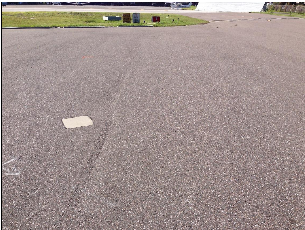
Apron NW, Section 4310, Sample Unit 603 – Low Severity (56) Swelling, Low Severity (57) Weathering
