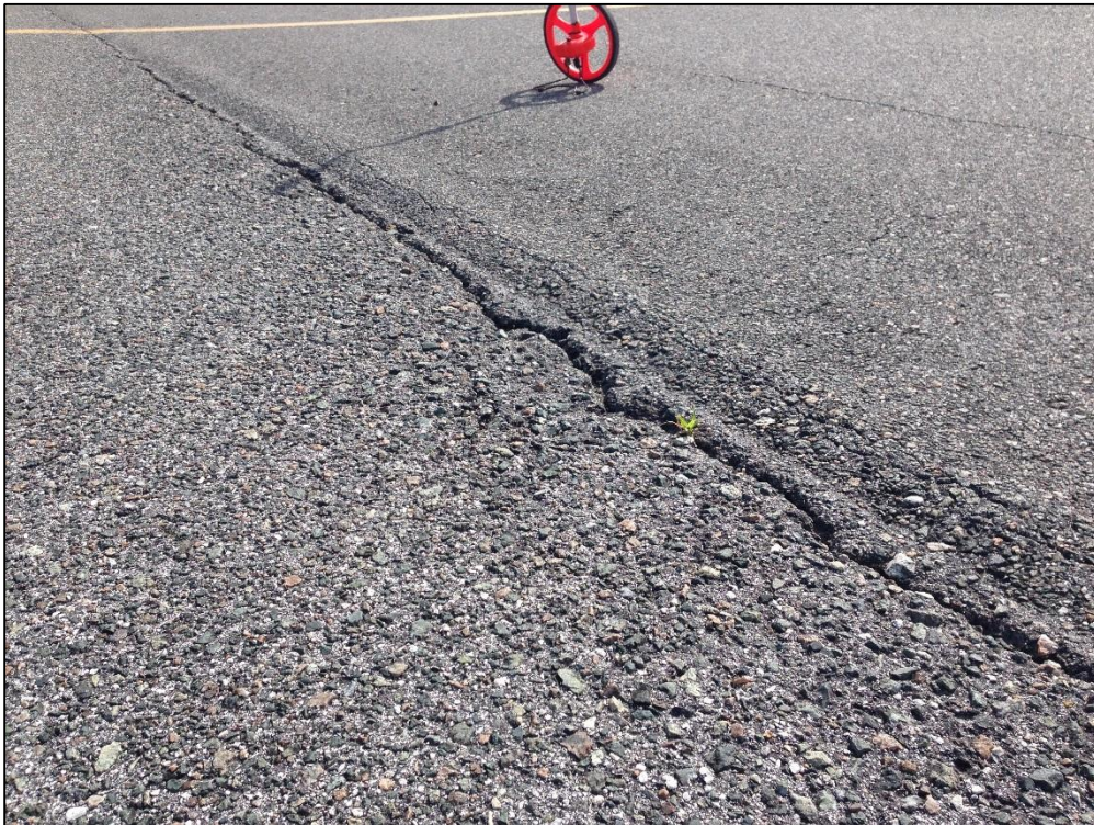
Taxiway Alpha, Section 105, Sample Unit 103 – Medium Severity (48) Longitudinal and Transverse Cracking, High Severity (48) Longitudinal and Transverse Cracking, Low Severity (52) Raveling, Low Severity (56) Swelling
