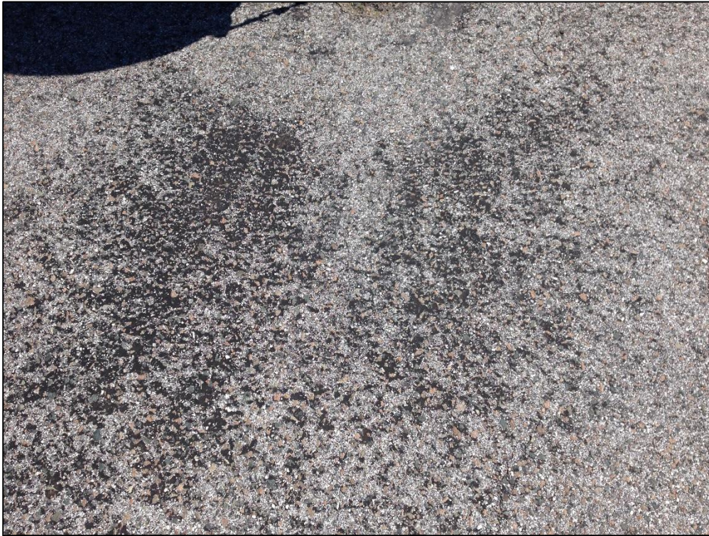
Apron, Section 4110, Sample Unit 204 – (42) Bleeding, Low Severity (52) Raveling
