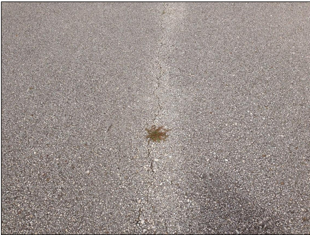
Runway 18-36, Section 6110, Sample Unit 504 – Low Severity (48) Longitudinal and Transverse Cracking, Low Severity (52) Raveling
