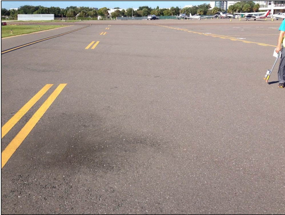
Apron NW, Section 4315, Sample Unit 249 – Low Severity (45) Depression, Low Severity (57) Weathering
