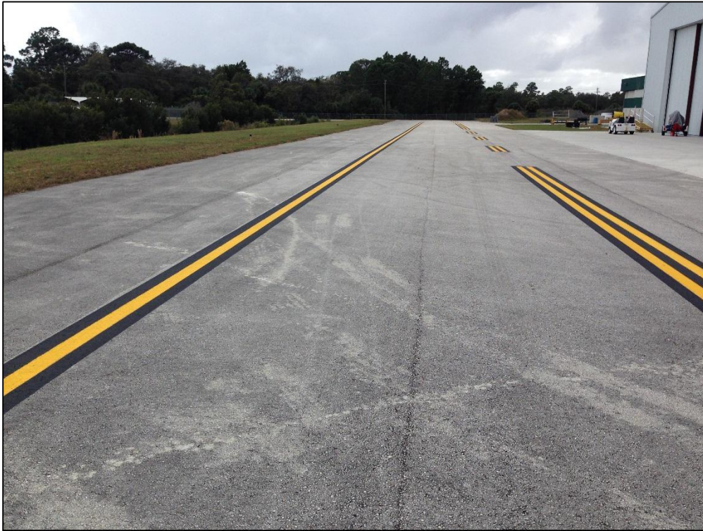
Taxiway Echo, Section 515, Sample Unit 628 – Medium Severity (57) Weathering
