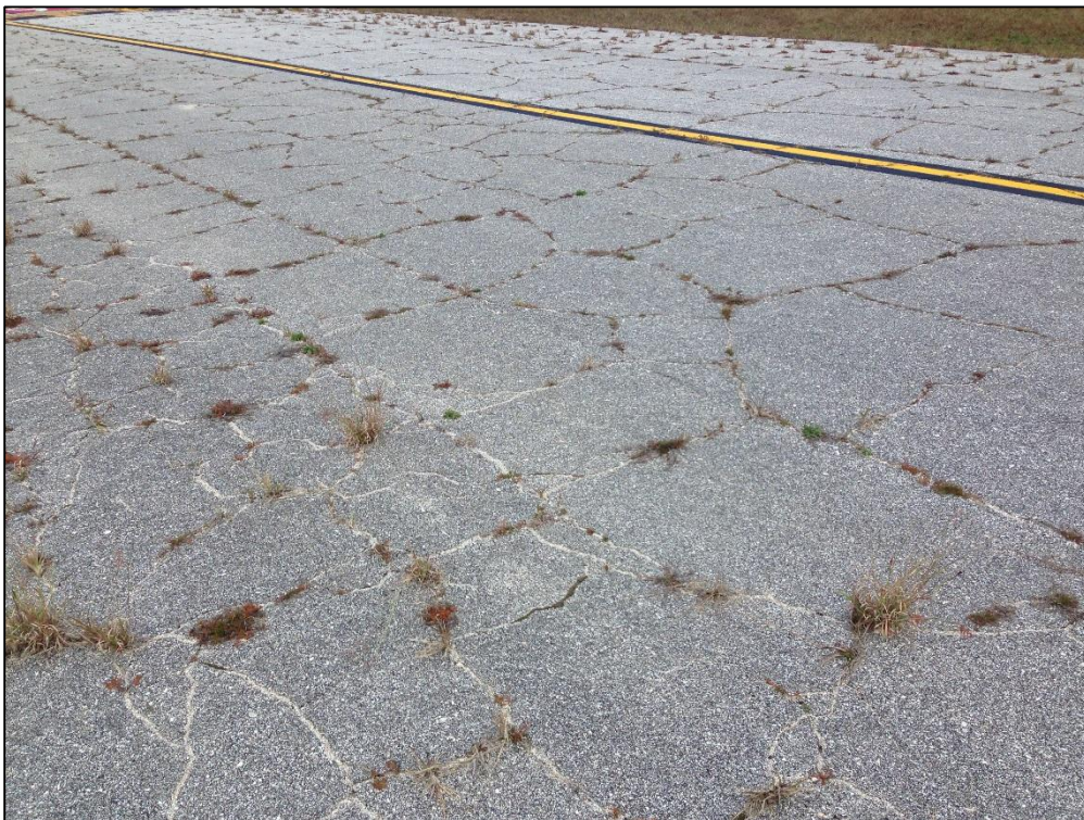
Taxiway Foxtrot, Section 605, Sample Unit 301 – Medium Severity (43) Block Cracking, Medium Severity (52) Raveling
