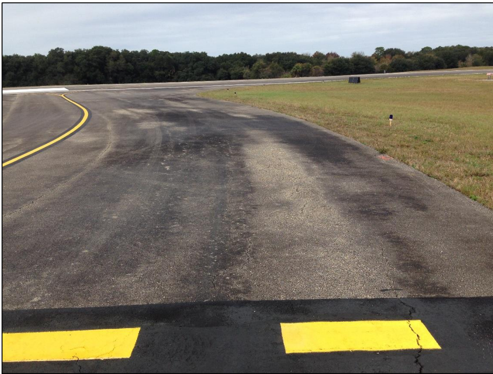
Taxiway Alpha, Section 120, Sample Unit 162 – Low Severity (48) Longitudinal and Transverse Cracking, Low Severity (52) Raveling, Low Severity (56) Swelling, Medium Severity (57) Weathering
