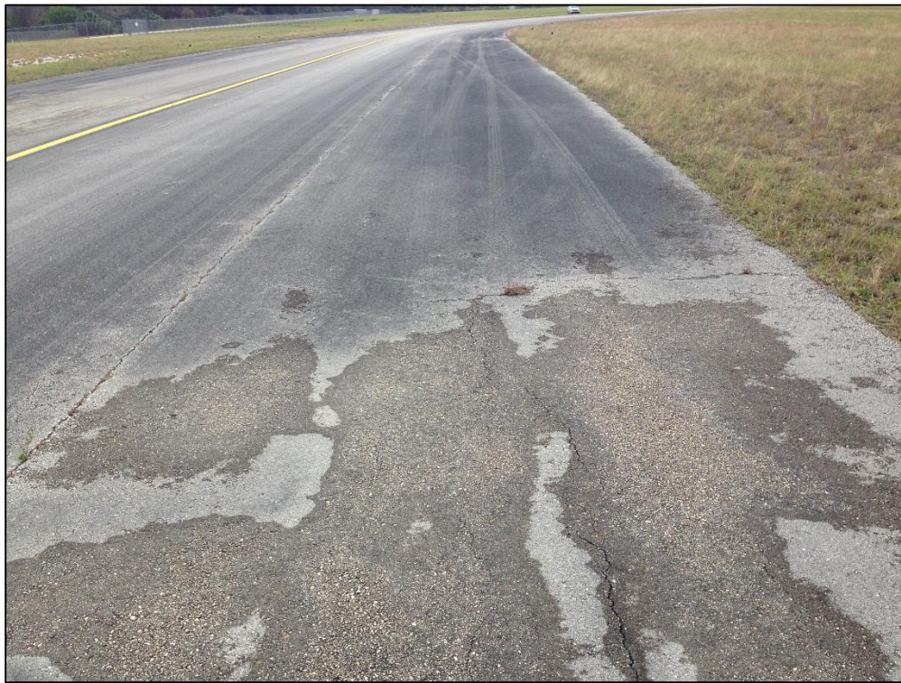
Taxiway Alpha, Section 105, Sample Unit 108 – Low Severity (48) Longitudinal and Transverse Cracking, Low Severity (56) Swelling, Medium Severity (57) Weathering
