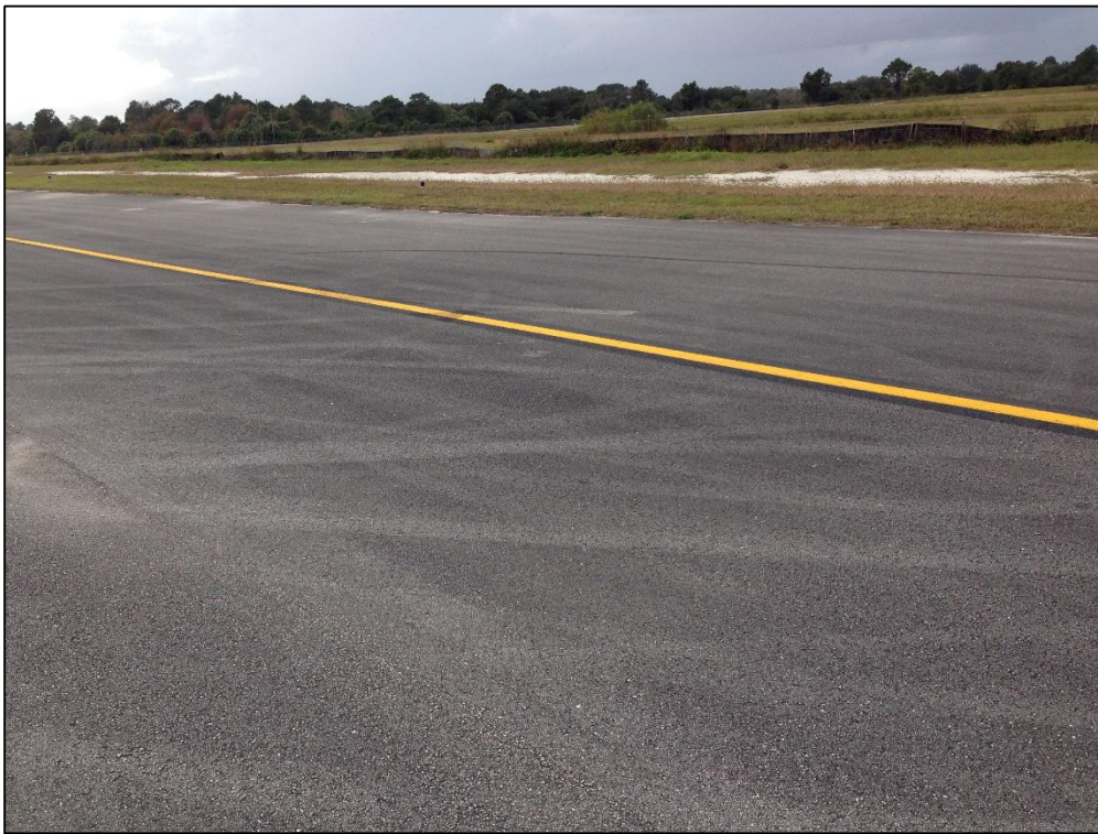
Taxiway Delta, Section 410, Sample Unit 414 – Medium Severity (57) Weathering
