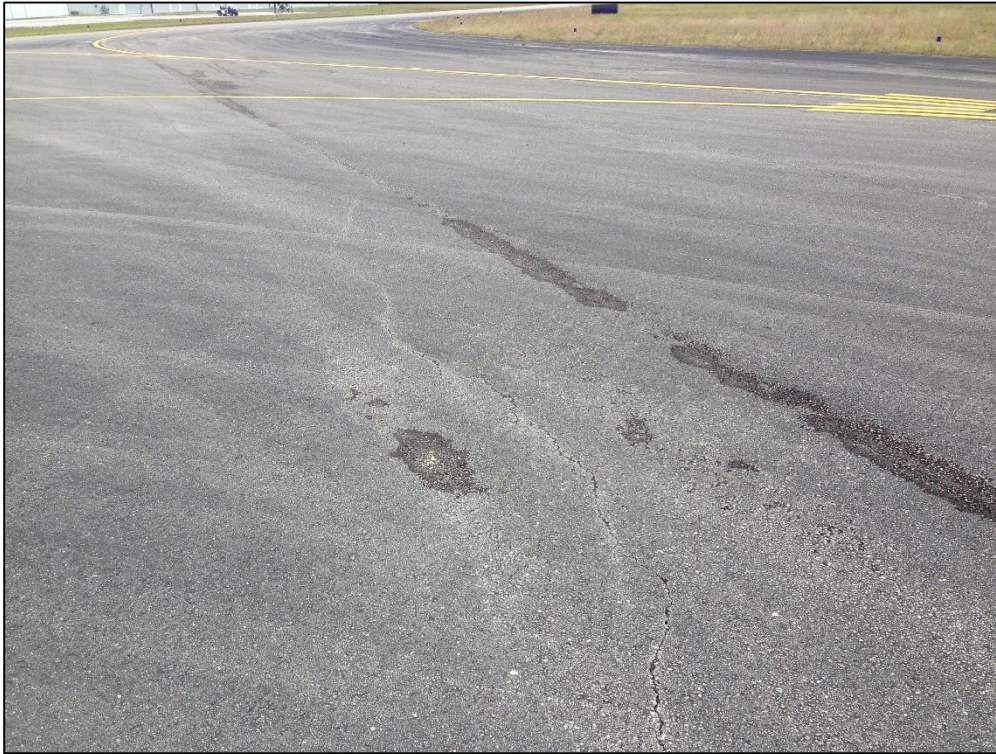
Taxiway Charlie, Section 305, Sample Unit 704 – Low Severity (48) Longitudinal and Transverse Cracking, Low Severity (50) Patching, Low Severity (52) Raveling, Medium Severity (57) Weathering
