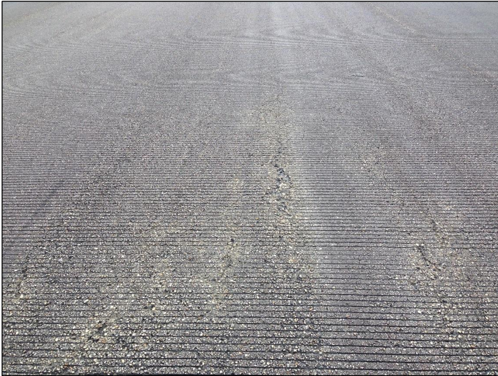
Runway 18-36, Section 6105, Sample Unit 360 – Low Severity (48) Longitudinal and Transverse Cracking, Medium Severity (52) Raveling
