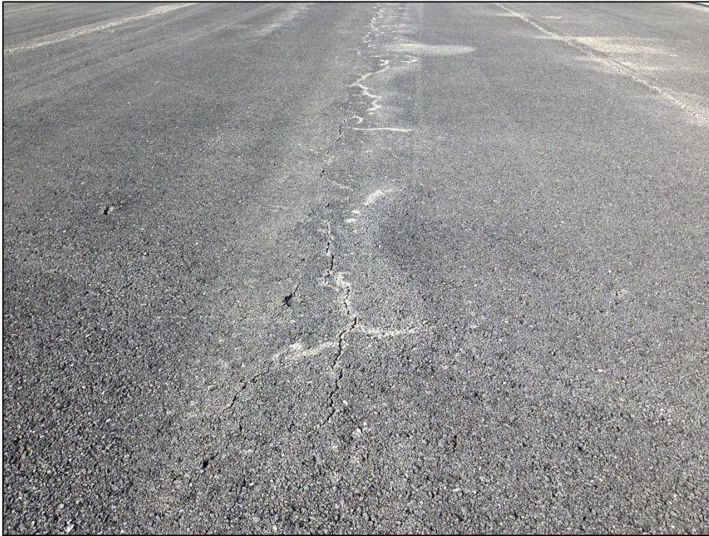
Runway 9-27, Section 6210, Sample Unit 155 – Low Severity (48) Longitudinal and Transverse Cracking, Low Severity (52) Raveling, Low Severity (56) Swelling, Medium Severity (57) Weathering
