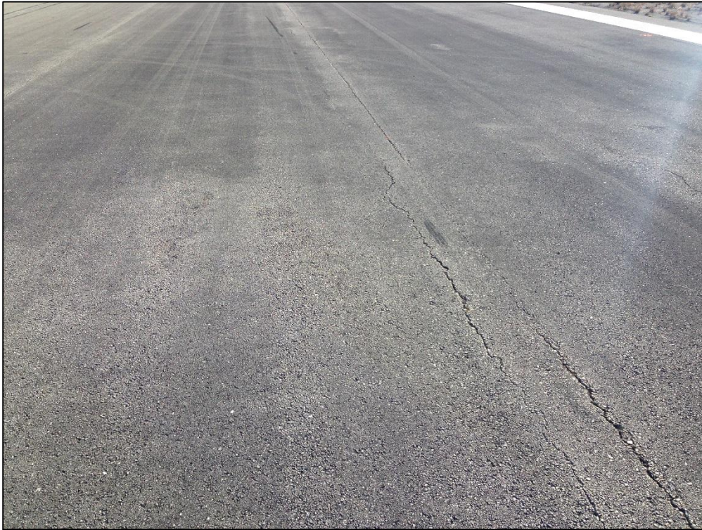
Runway 9-27, Section 6210, Sample Unit 130 – Low Severity (48) Longitudinal and Transverse Cracking, Low Severity (52) Raveling, Low Severity (56) Swelling, Low Severity (57) Weathering, Medium Severity (57) Weathering
