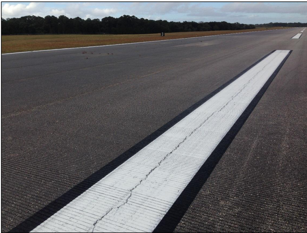
Runway 18-36, Section 6105, Sample Unit 380 – Low Severity (48) Longitudinal and Transverse Cracking, Low Severity (52) Raveling, Low Severity (57) Weathering, Medium Severity (57) Weathering
