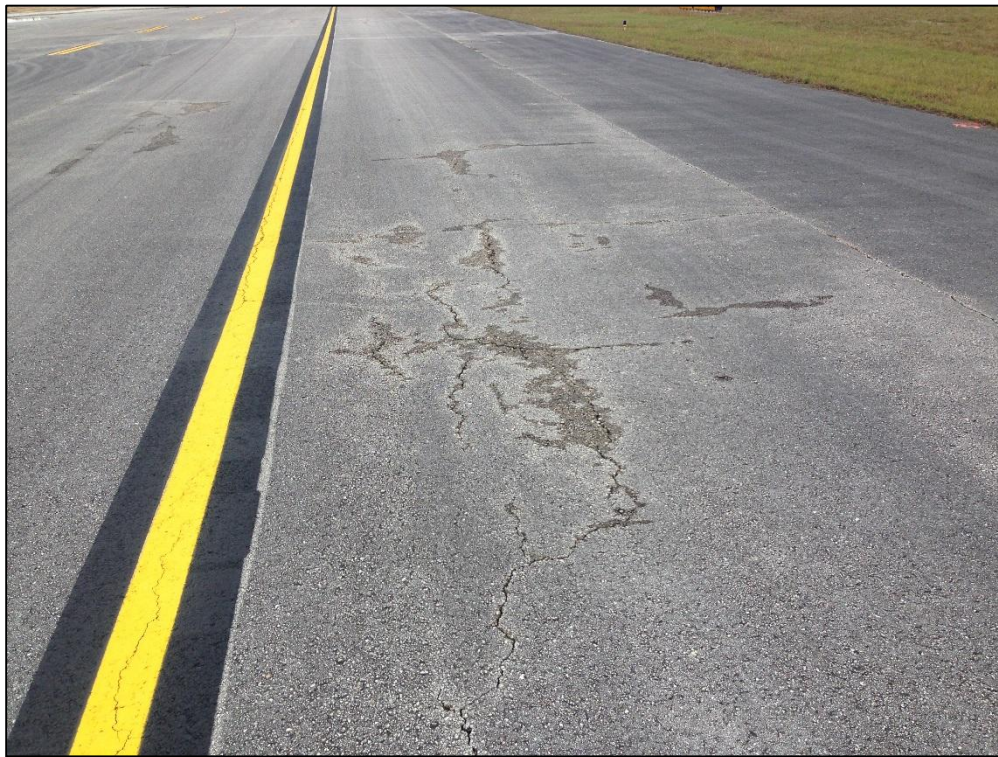
Taxiway Alpha, Section 110, Sample Unit 127 – Low Severity (43) Block Cracking, Low Severity (48) Longitudinal and Transverse Cracking, Medium Severity (57) Weathering
