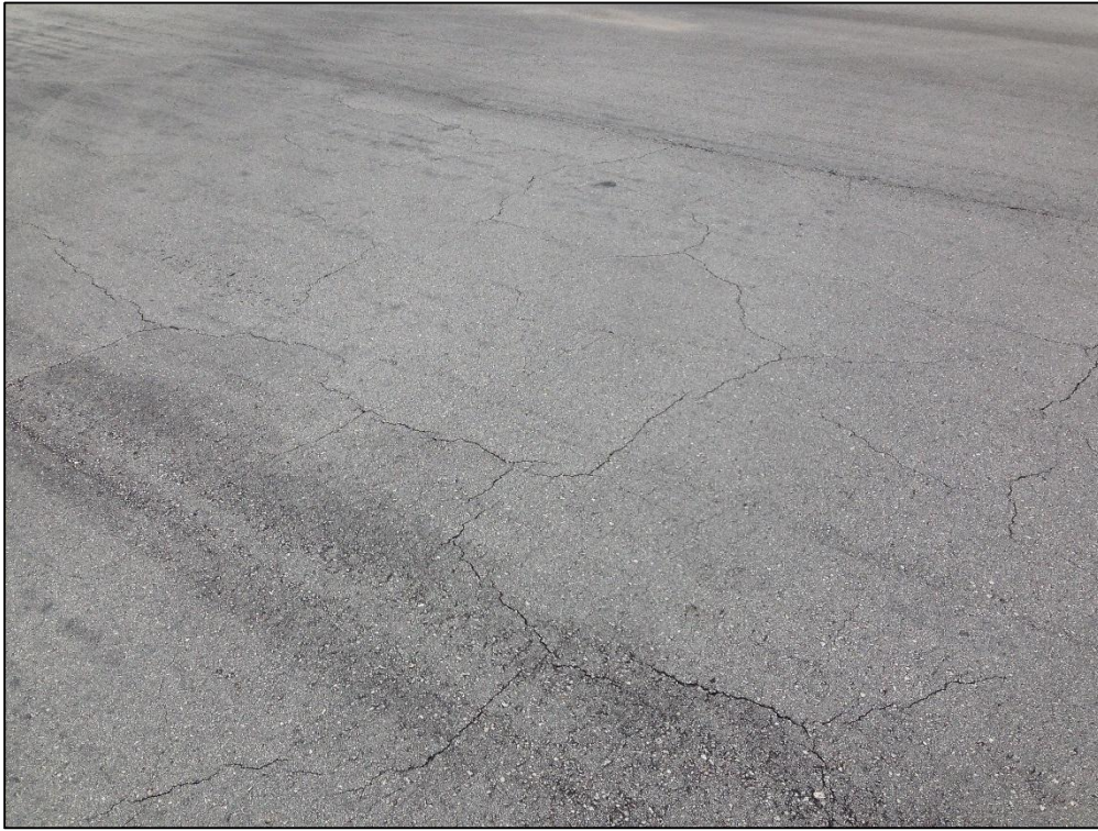
Apron South, Section 4205, Sample Unit 150 – Low Severity (43) Block Cracking, Low Severity (57) Weathering
