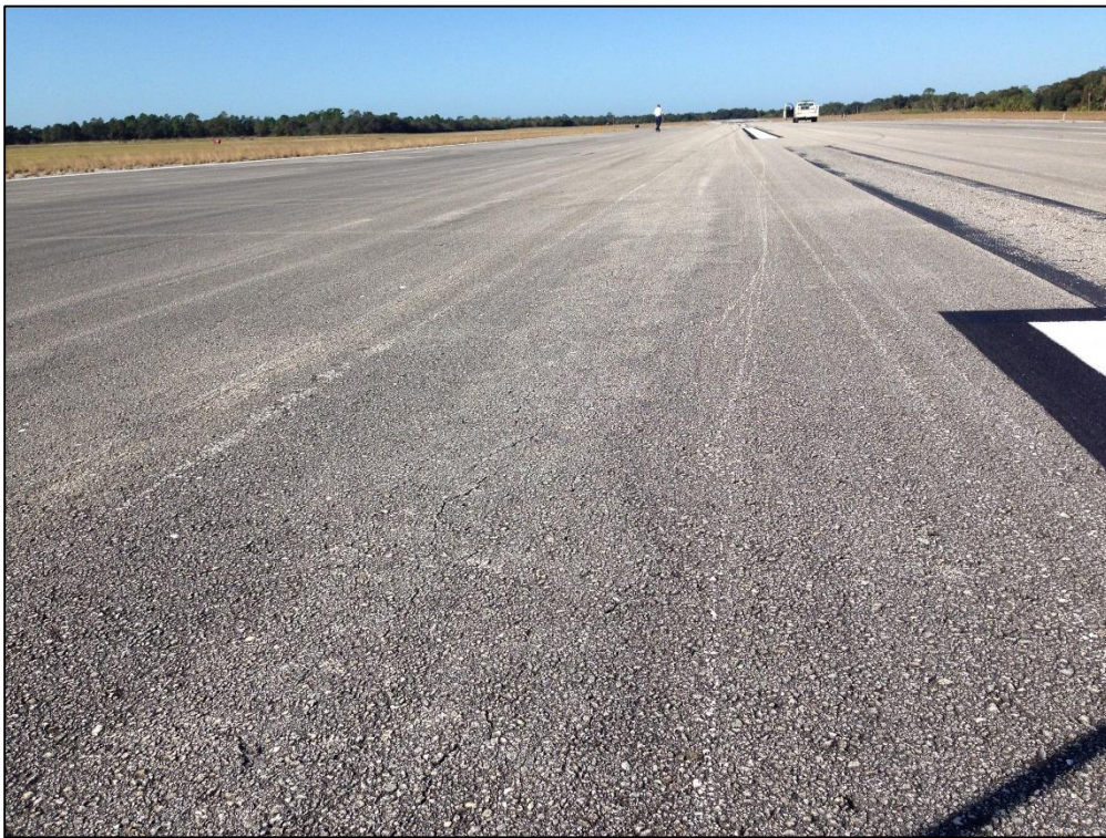
Runway 9-27, Section 6210, Sample Unit 136 – Low Severity (48) Longitudinal and Transverse Cracking, Low Severity (52) Raveling, Low Severity (56) Swelling, Medium Severity (57) Weathering
