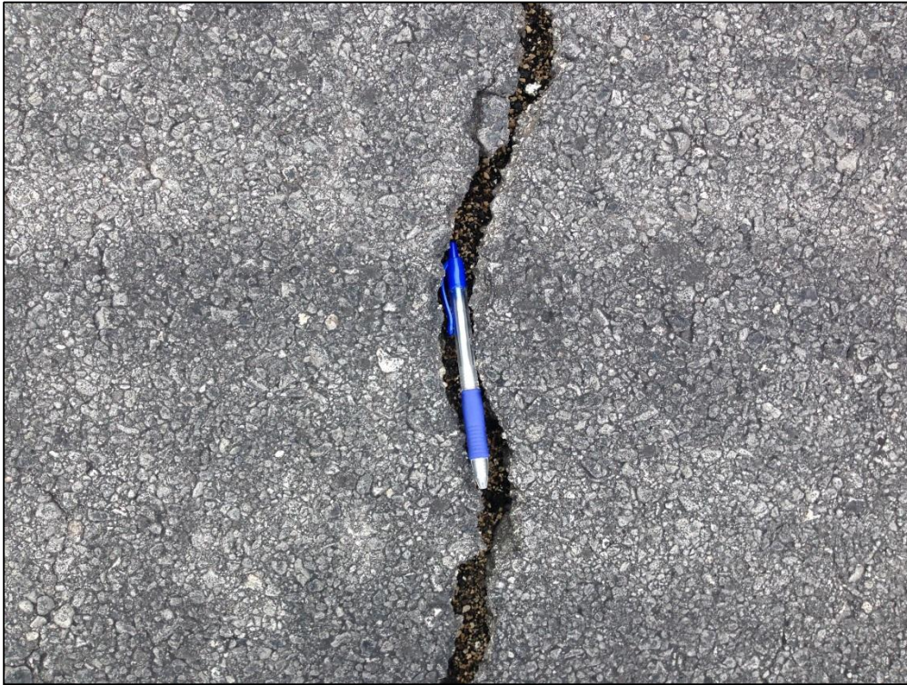
Runway18-36, Section 6110, Sample Unit 524 –Medium Severity (48) Longitudinal and Transverse Cracking, Low Severity (57) Weathering
