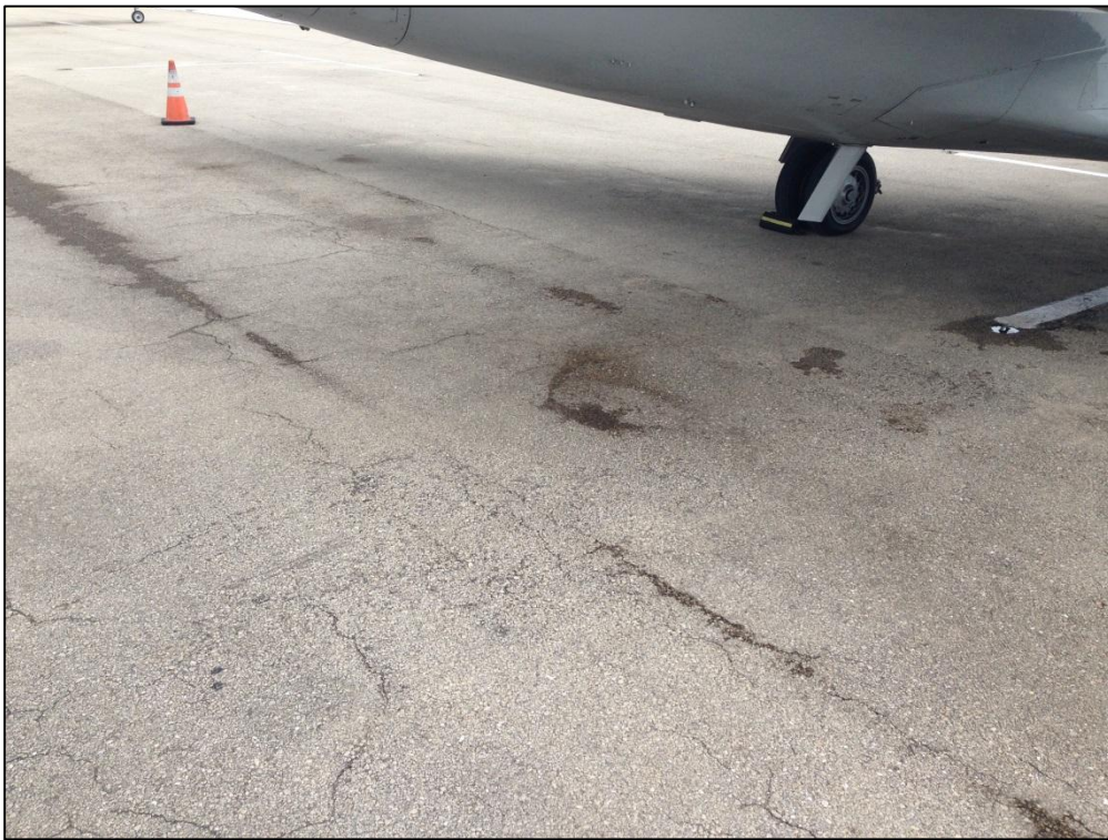
Apron GA, Section 4305, Sample Unit 303 – Low Severity (48) Longitudinal and Transverse Cracking, (49) Oil Spillage, Low Severity (52) Raveling, Low Severity (57) Weathering
