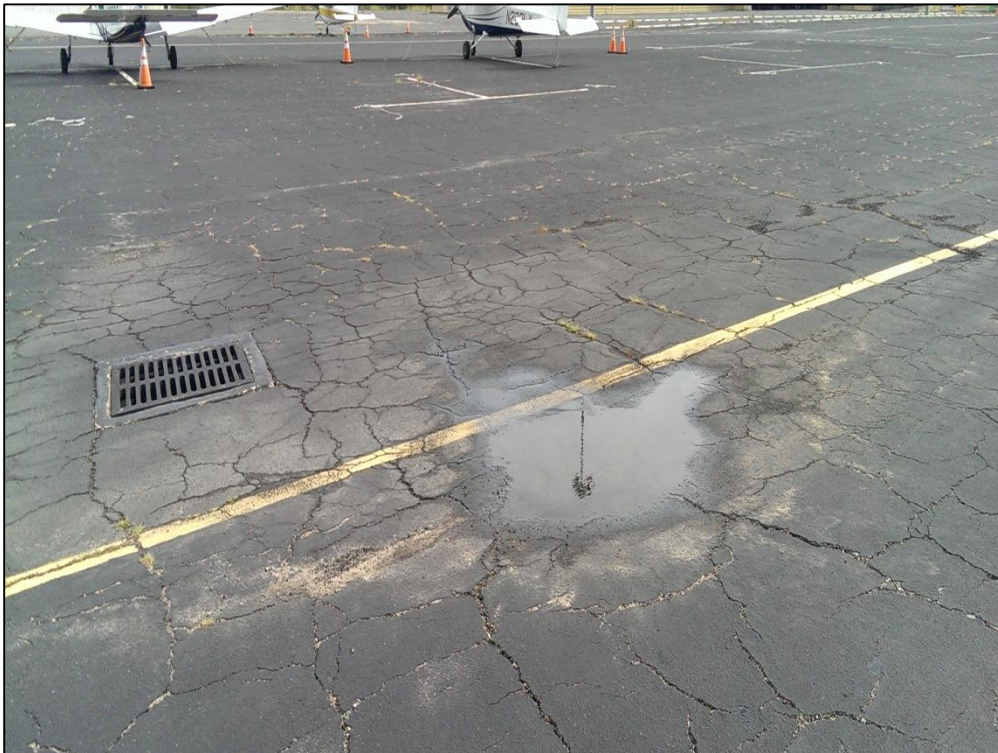
Apron GA, Section 4332, Sample Unit 359 –Low Severity (45) Depression, Low Severity (43) Block Cracking, Medium Severity (43) Block Cracking, Medium Severity (57) Weathering, and Low Severity (52) Raveling
