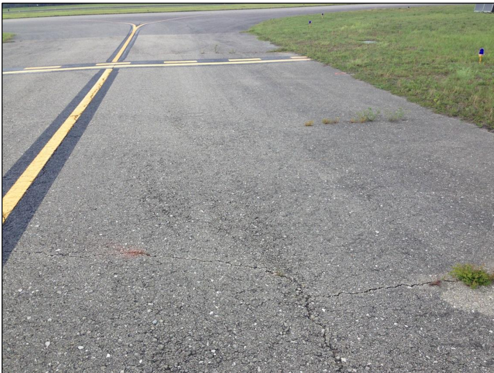
Taxiway R, Section 1810, Sample Unit 101 –Low Severity (48) Longitudinal and Transverse Cracking, Low Severity (52) Raveling
