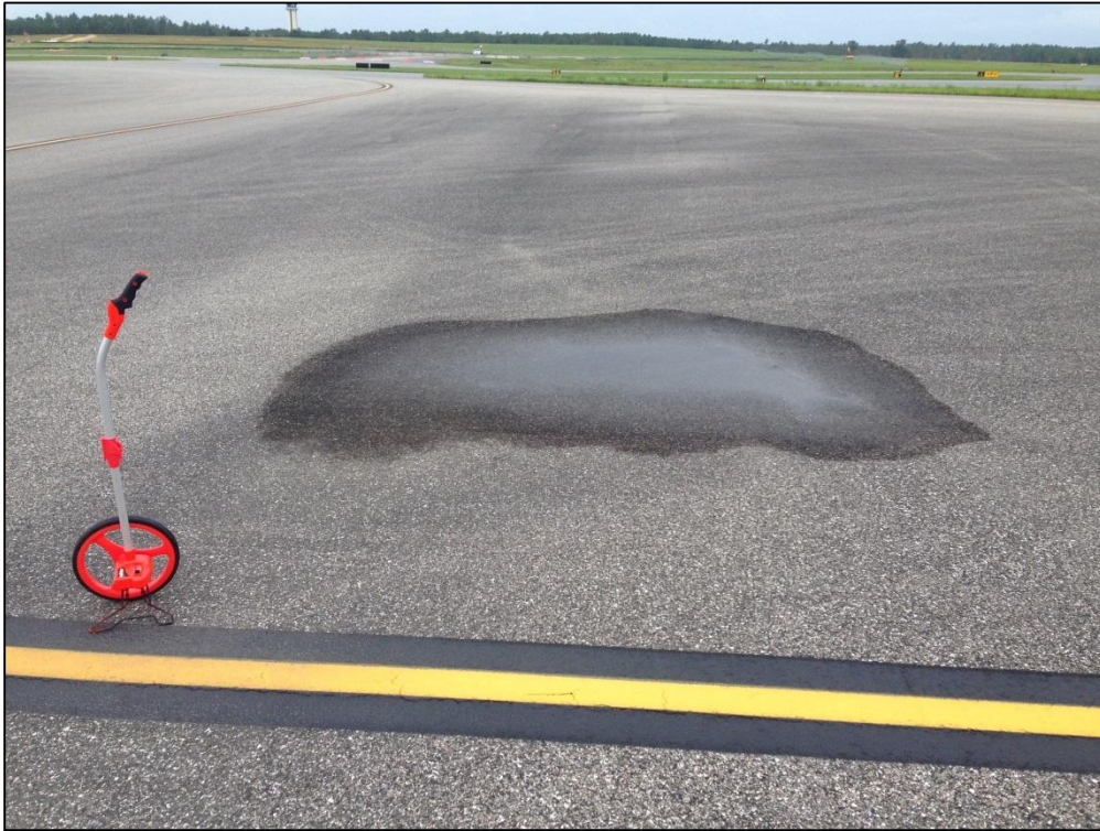
Taxiway M, Section 1325, Sample Unit 101 – Low Severity (45) Depression, Low Severity (48) Longitudinal and Transverse Cracking, Medium Severity (57) Weathering, Low Severity (57) Weathering
