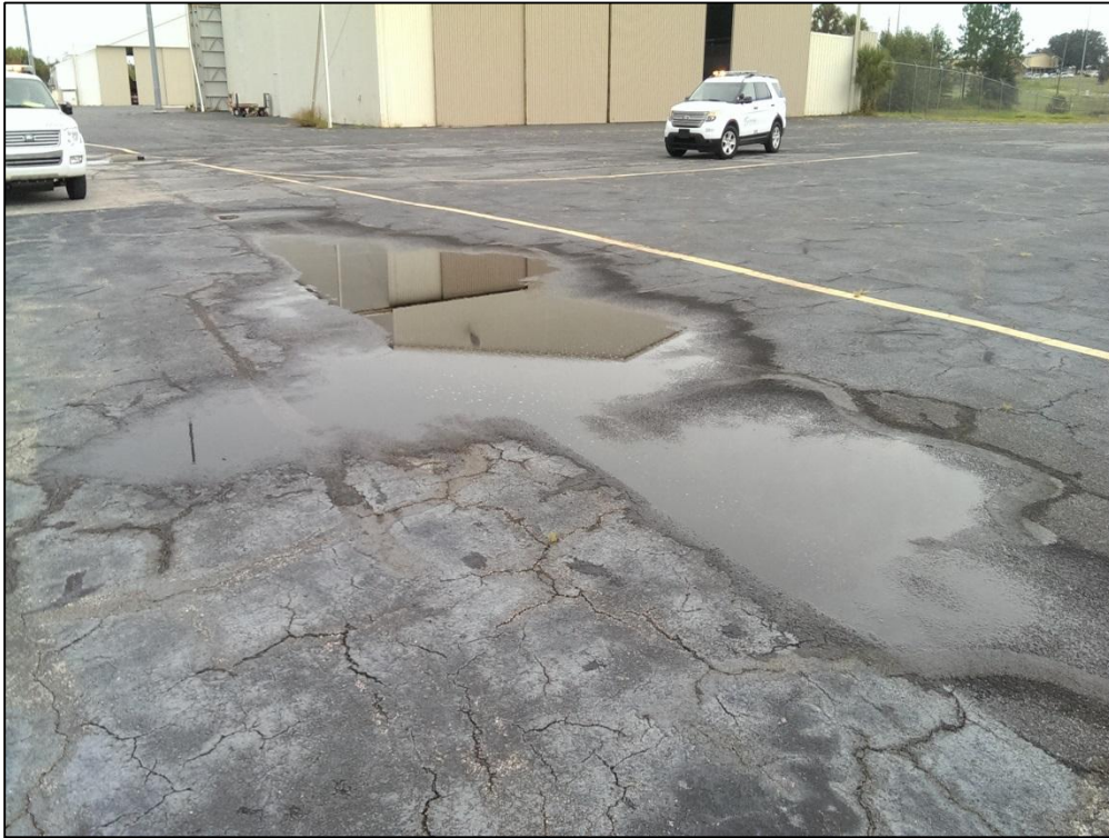
Apron GA, Section 4330, Sample Unit 661 –Medium Severity (45) Depression, Low Severity (43) Block Cracking, Medium Severity (43) Block Cracking, Medium Severity (43) Block Cracking, Medium Severity (57) Weathering, and Low Severity (52) Raveling
