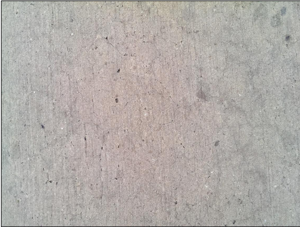
Terminal Apron, Section 4105, Sample Unit 265 –Low Severity (70) Scaling, Map Cracking, Crazing
