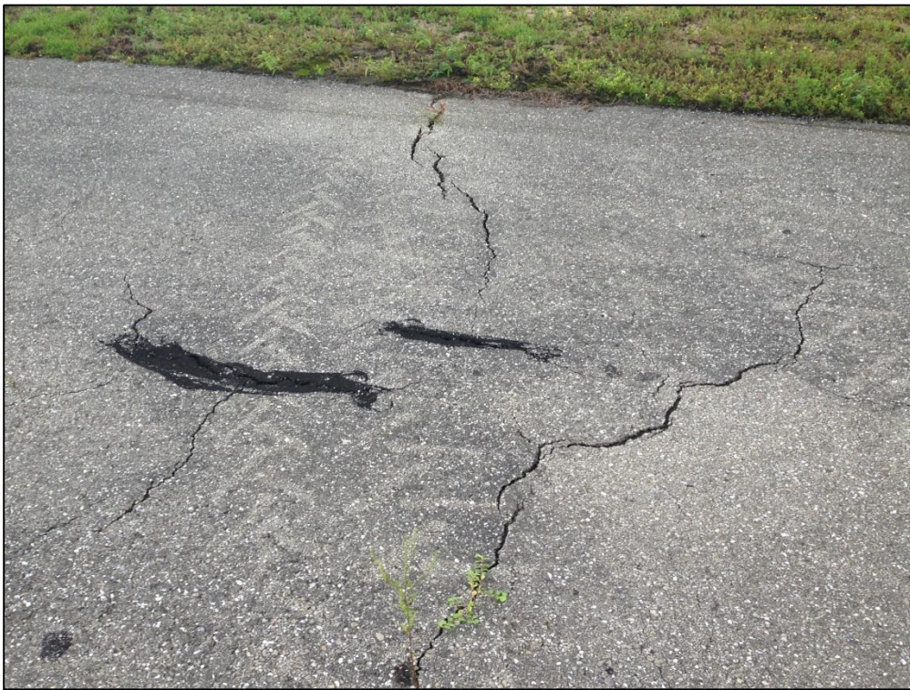
Taxiway K, Section 1120, Sample Unit 101 – Medium Severity (48) Longitudinal and Transverse Cracking, Low Severity (48) Longitudinal and Transverse Cracking, Low Severity (57) Weathering
