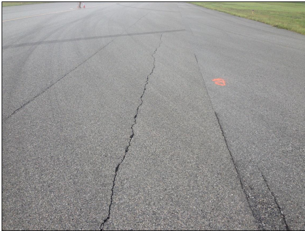
Taxiway P, Section 1605, Sample Unit 200 – Medium Severity (48) Longitudinal and Transverse Cracking, Low Severity (52) Raveling, Low Severity (57) Weathering
