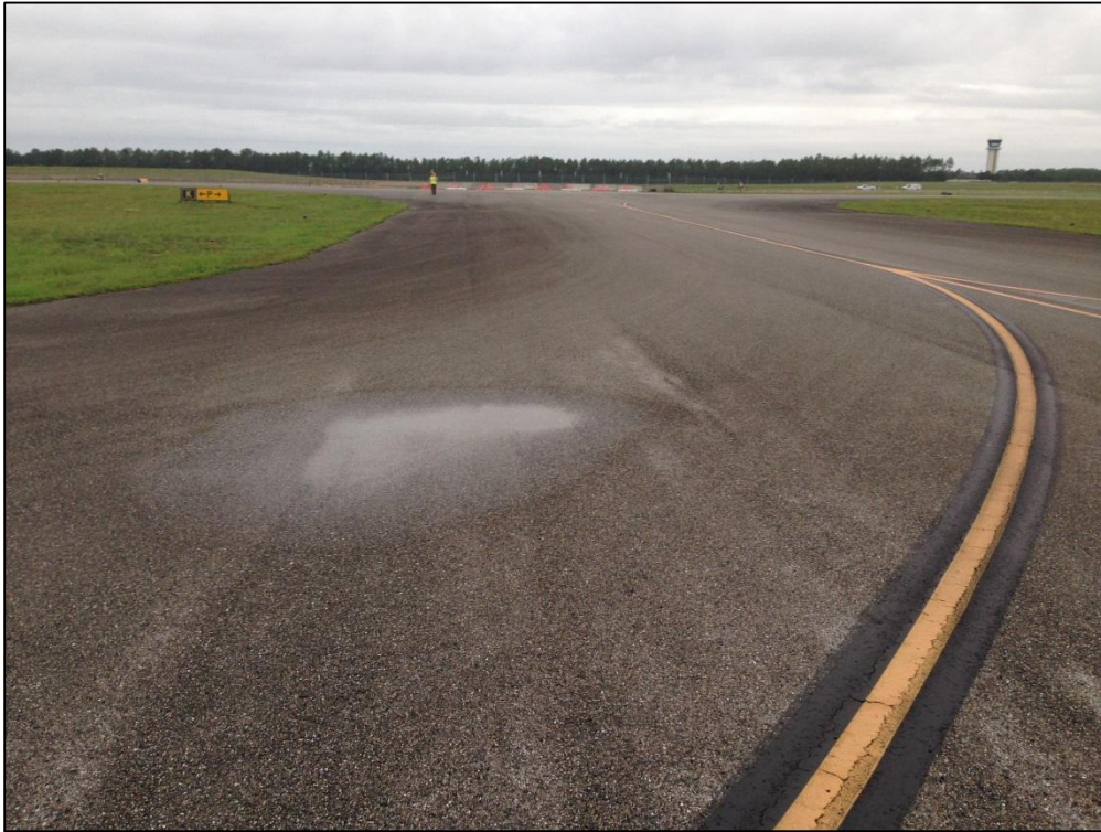
Taxiway K, Section 1110, Sample Unit 106 – Low Severity (45) Depression, Low Severity (52) Raveling, Low Severity (57) Weathering
