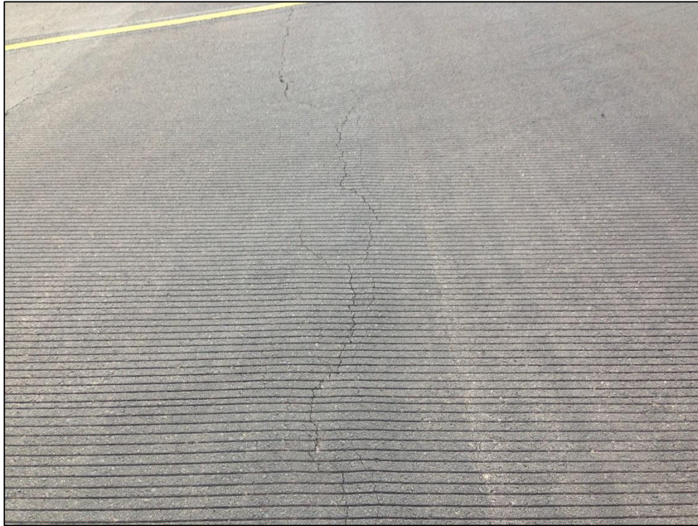
Runway 18-36, Section 6110, Sample Unit 588 – Medium Severity (48) Longitudinal and Transverse Cracking, Low Severity (48) Longitudinal and Transverse Cracking, Low Severity (57) Weathering
