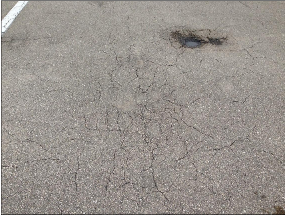
Apron GA, Section 4310, Sample Unit 306 – Low Severity (41) Alligator Cracking, High Severity (45) Depression, Low Severity (48) Longitudinal and Transverse Cracking Low Severity (52) Raveling, Low Severity (57) Weathering
