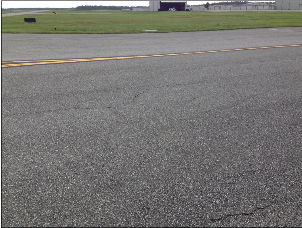
Taxiway E, Section 510, Sample Unit 101 –Low Severity (48) Longitudinal and Transverse Cracking, Low Severity (56) Swelling, Medium Severity (57) Weathering
