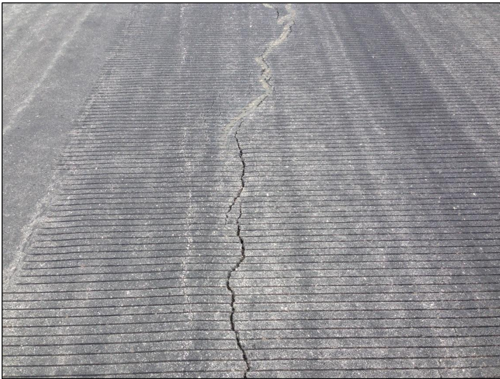
Runway 18-36, Section 6110, Sample Unit 548 –, Medium Severity (48) Longitudinal and Transverse Cracking, Low Severity (57) Weathering
