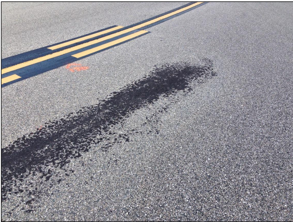
Taxiway M, Section 1315, Sample Unit 130 – (42) Bleeding, Medium Severity (57) Weathering
