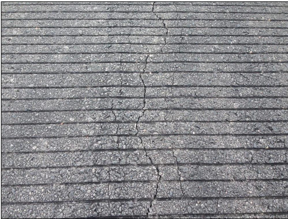
Runway 18-36, Section 6105, Sample Unit 351 – Low Severity (41) Alligator Cracking, Low Severity (57) Weathering
