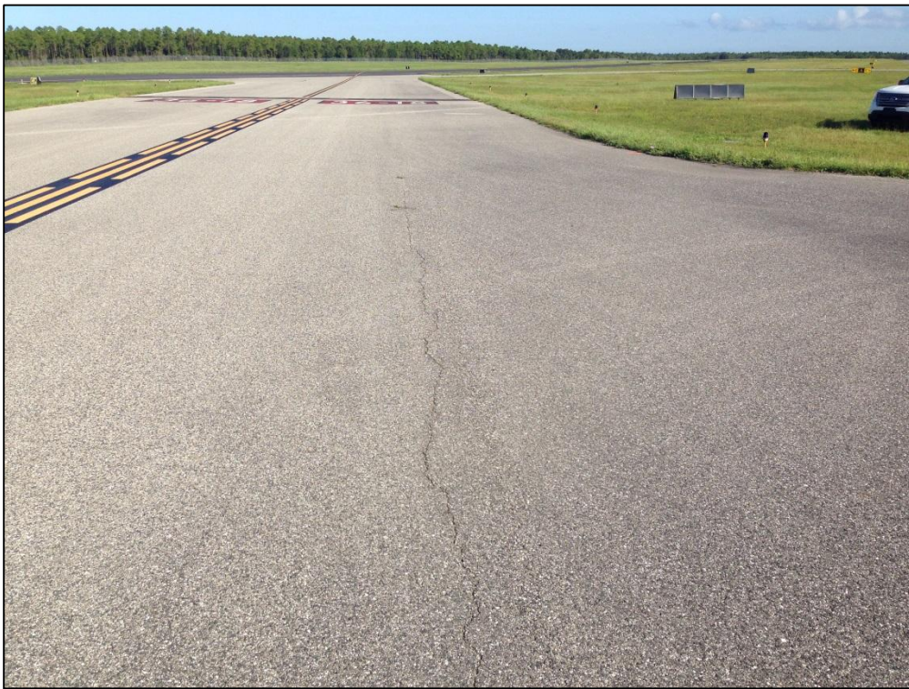
Taxiway D, Section 405, Sample Unit 109 – Low Severity (48) Longitudinal and Transverse Cracking, Low Severity (57) Weathering
