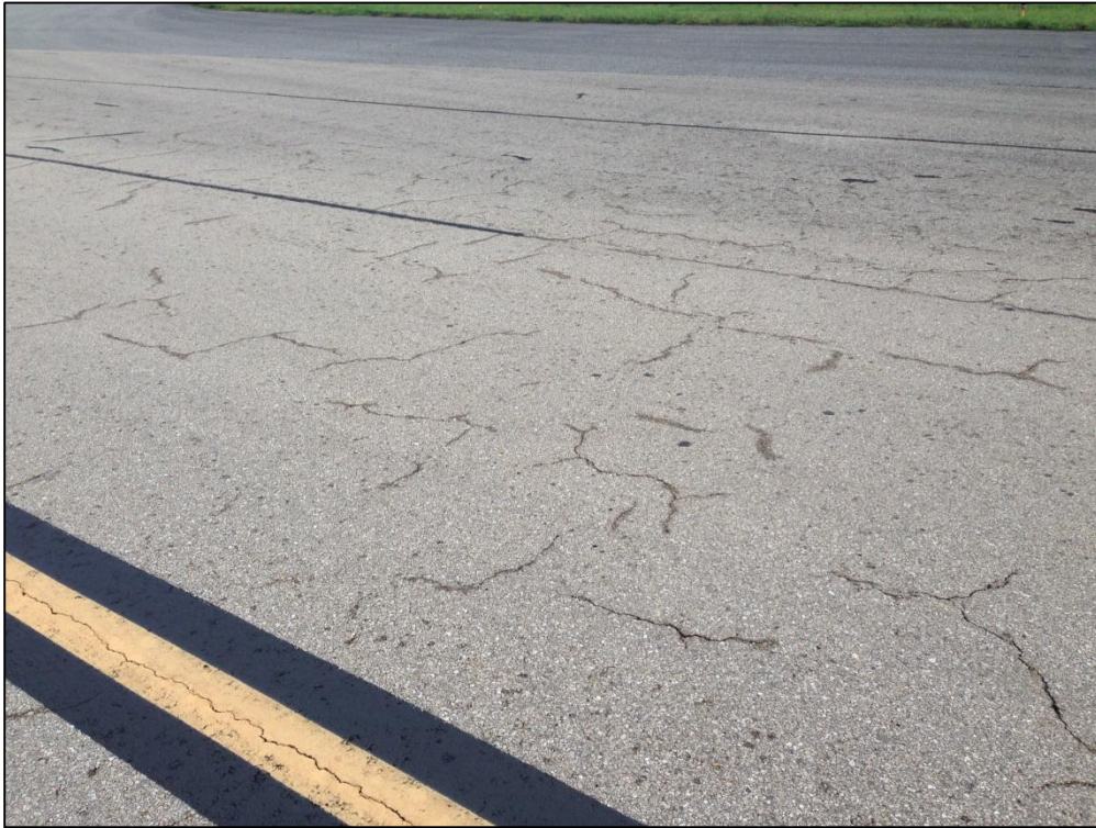
Taxiway S, Section 1905, Sample Unit 119 – Low Severity (48) Longitudinal and Transverse Cracking, Low Severity (52) Raveling, Low Severity (57) Weathering
