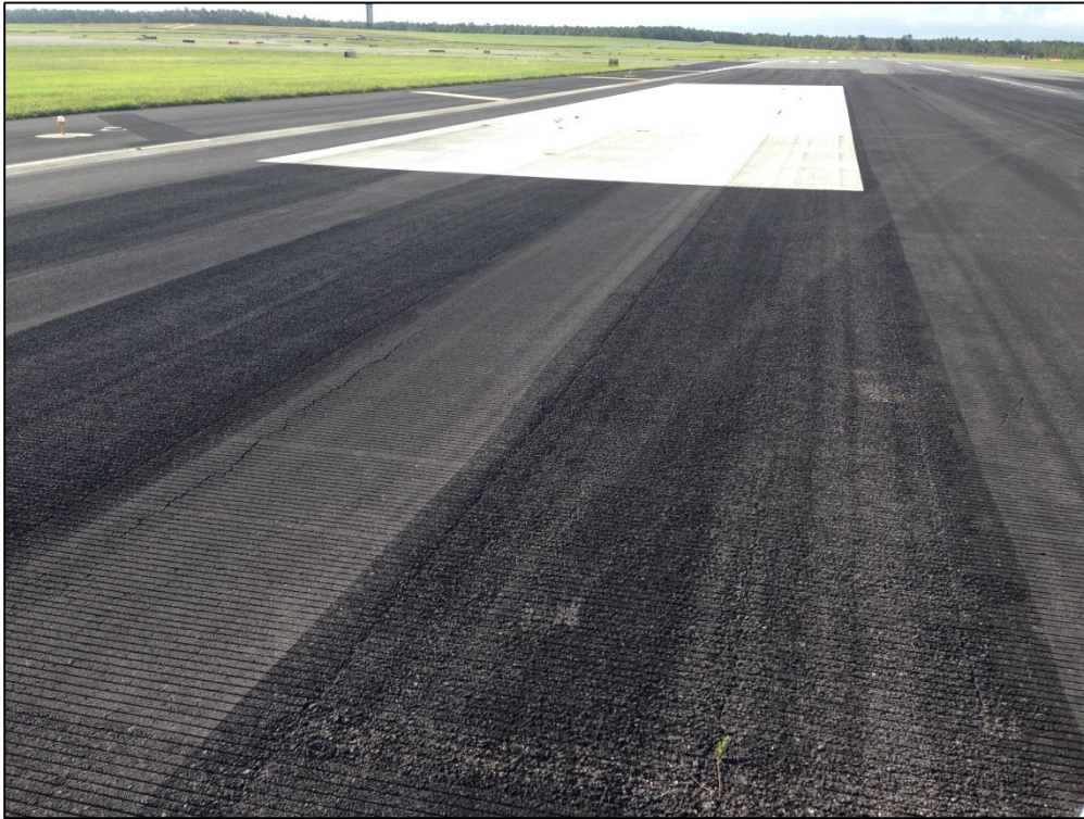
Runway 18-36, Section 6105, Sample Unit 311 – Medium Severity (52) Raveling, Low Severity (52) Raveling, Low Severity (57) Weathering, Low Severity (48) Longitudinal and Transverse Cracking
