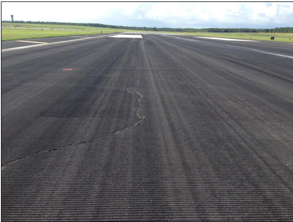
Runway 18-36, Section 6105, Sample Unit 315 – Medium Severity (48) Longitudinal and Transverse Cracking, Low Severity (52) Raveling, Low Severity (57) Weathering
