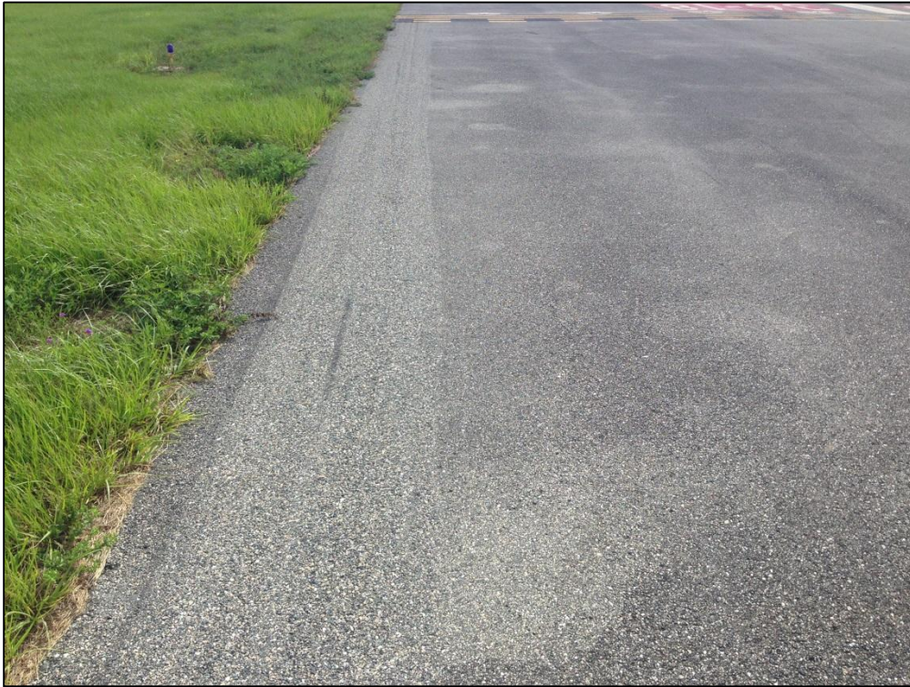
Taxiway A2, Section 125, Sample Unit 101 –Low Severity (52) Raveling, Medium Severity (57) Weathering
