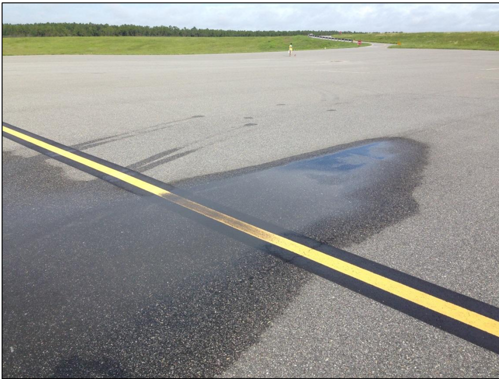
Apron at T-Hangers, Section 4505, Sample Unit 303 –Low Severity (45) Depression, Medium Severity (57) Weathering, Low Severity (57) Weathering
