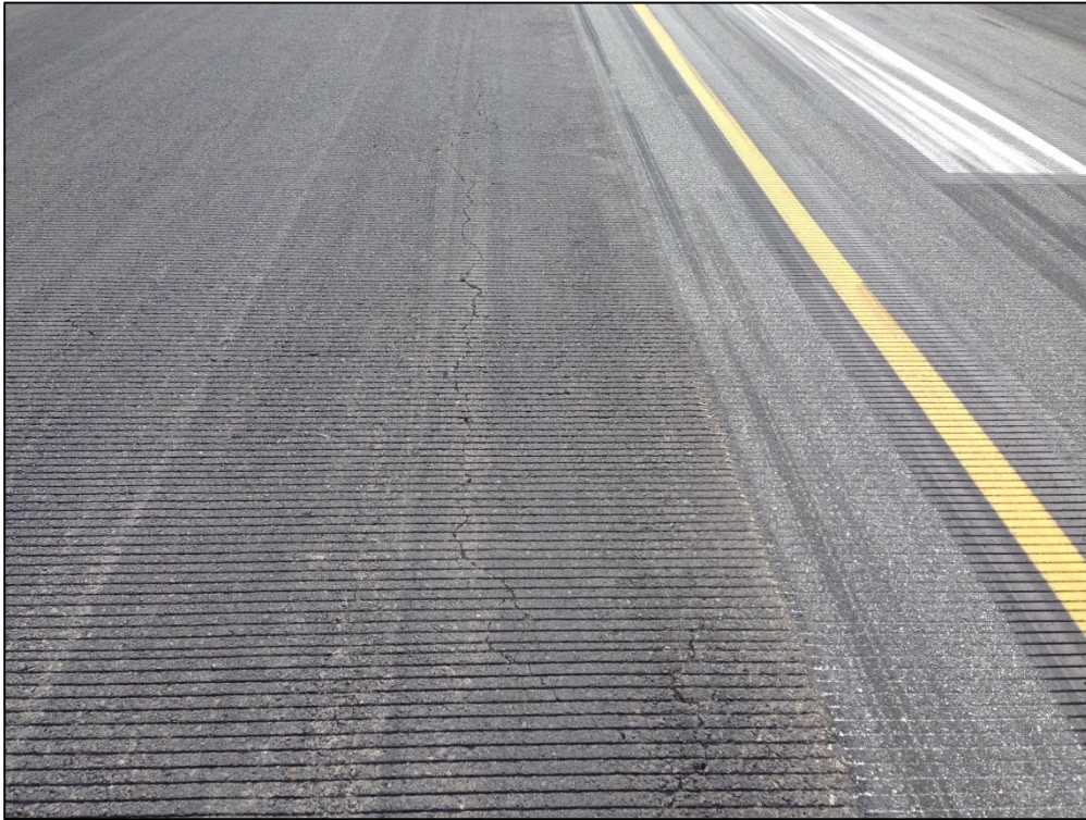
Runway 18-36, Section 6105, Sample Unit 344 – Low Severity (41) Alligator Cracking, Low Severity (48) Longitudinal and Transverse Cracking, Low Severity (50) Patching, Low Severity (57) Weathering
