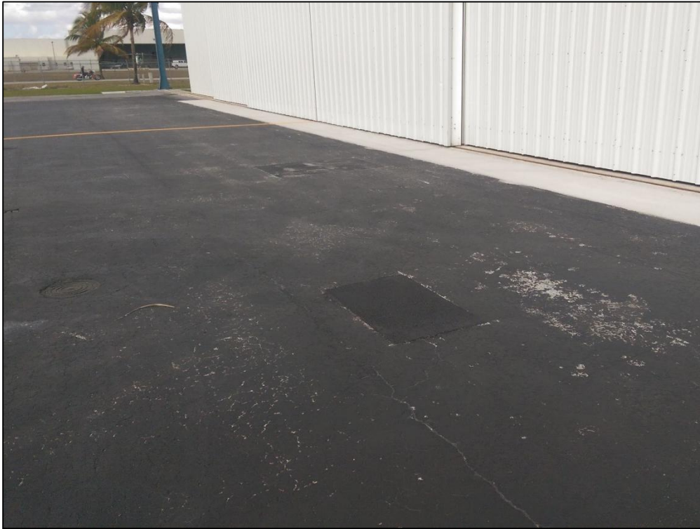
Apron Southeast, Section 4410, Sample Unit 501 – Low Severity (48) Longitudinal and Transverse Cracking, Low Severity (50) Patching, Medium Severity (57) Weathering
