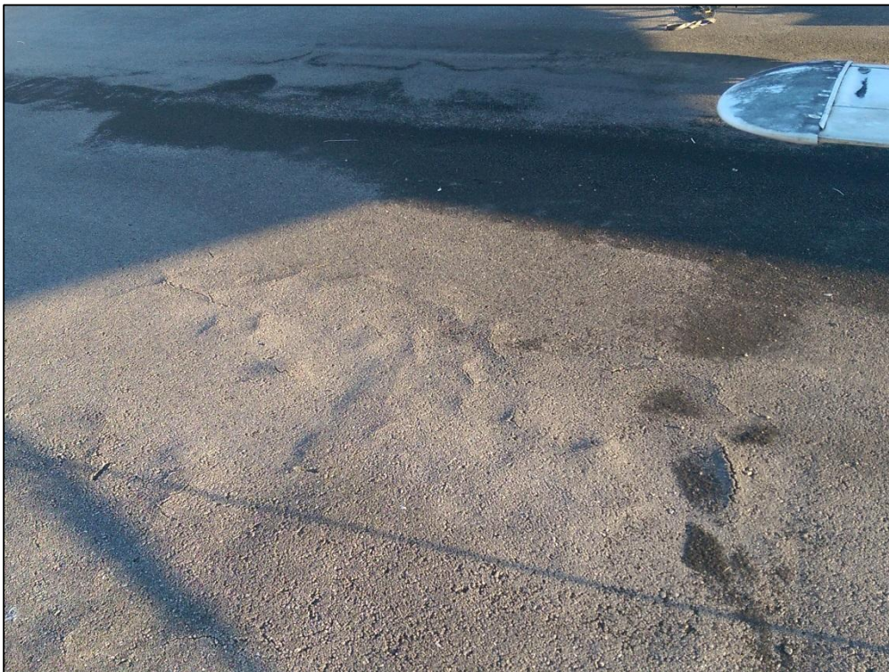
Apron North, Section 4205, Sample Unit 312 – Low Severity (48) Longitudinal and Transverse Cracking, Low Severity (56) Swelling, Low Severity (57) Weathering
