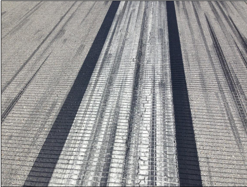
Runway 9R-27L, Section 6305, Sample Unit 342 – Low Severity (48) Longitudinal and Transverse Cracking, Low Severity (52) Raveling, Low Severity (57) Weathering, Medium Severity (57) Weathering
