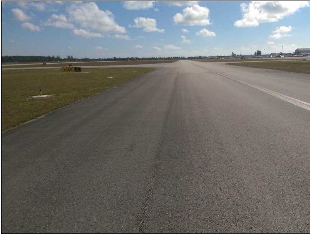
Taxiway Alpha, Section 105, Sample Unit 129 – Low Severity (48) Longitudinal and Transverse Cracking, Low Severity (57) Weathering
