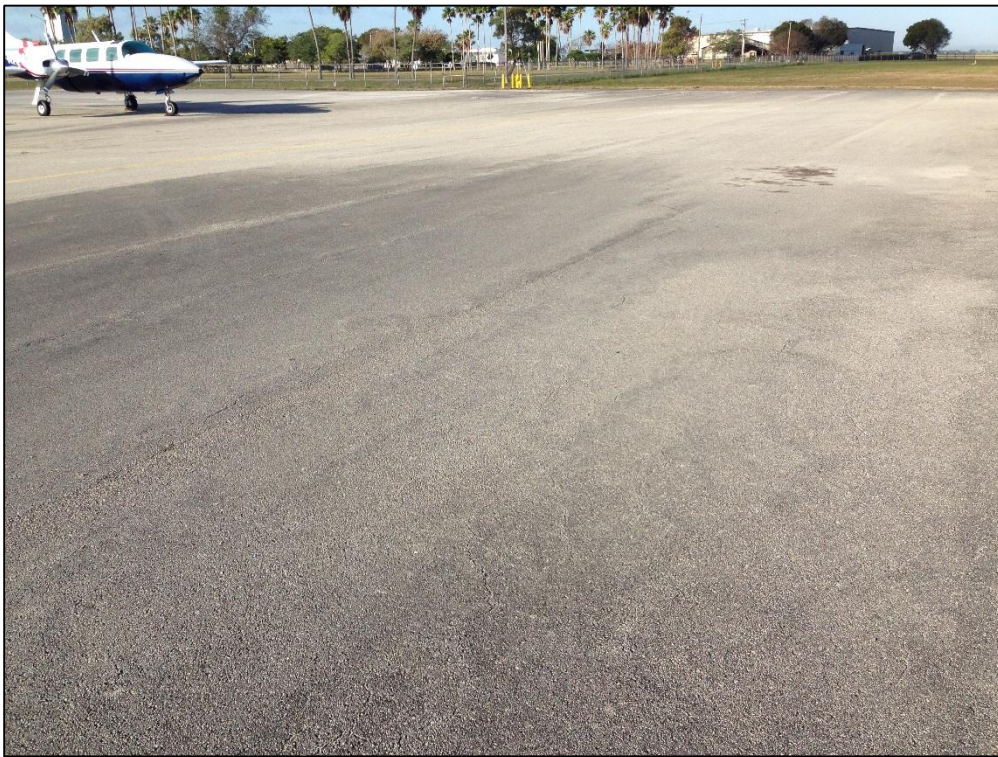
Apron North, Section 4220, Sample Unit 532 – Low Severity (48) Longitudinal and Transverse Cracking, (49) Oil Spillage, Low Severity (52) Raveling, Low Severity (56) Swelling, Medium Severity (57) Weathering
