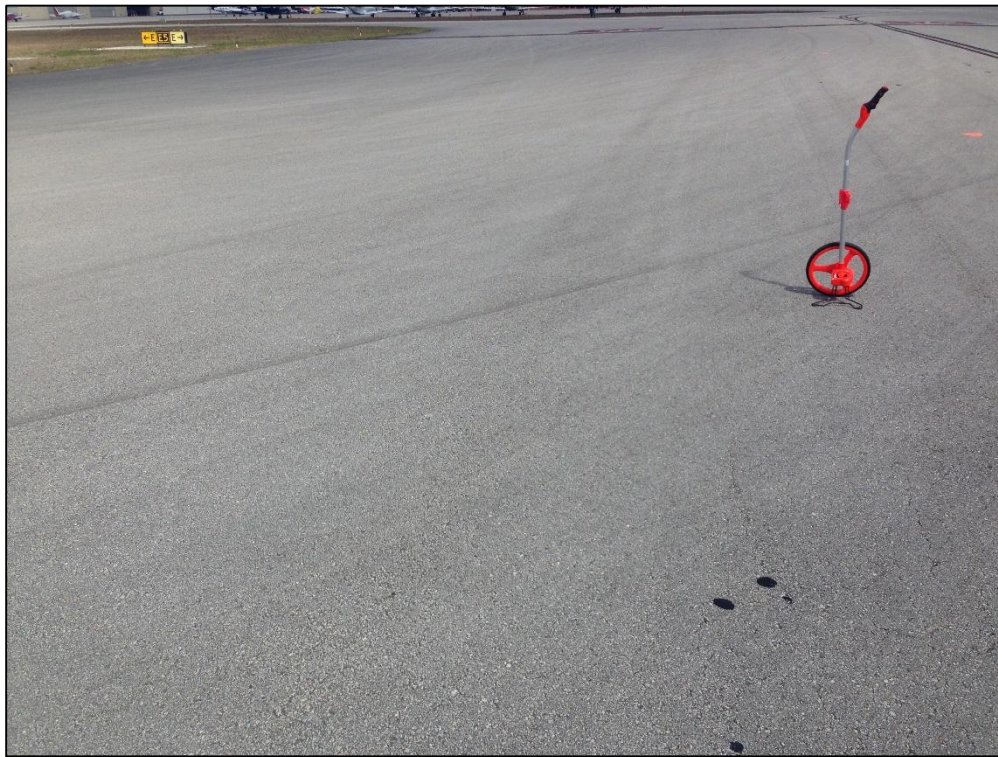
Taxiway E5, Section 529, Sample Unit 100 – Low Severity (48) Longitudinal and Transverse Cracking, Medium Severity (57) Weathering
