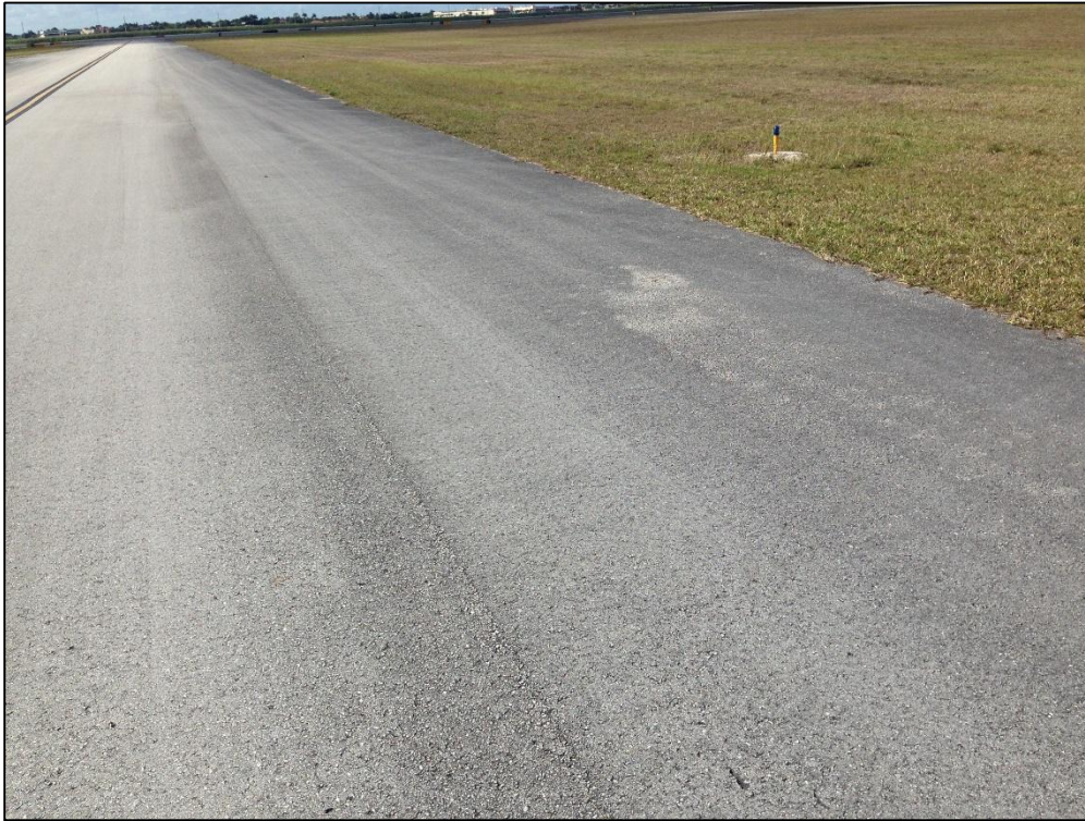
Taxiway Golf, Section 705, Sample Unit 209 – Low Severity (48) Longitudinal and Transverse Cracking, Low Severity (52) Raveling, Low Severity (57) Weathering, Medium Severity (57) Weathering
