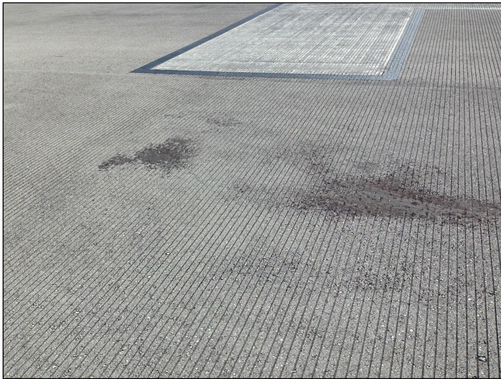
Runway 13-31, Section 6205, Sample Unit 378 – (42) Bleeding, Low Severity (48) Longitudinal and Transverse Cracking, Low Severity (57) Weathering, Medium Severity (57) Weathering
