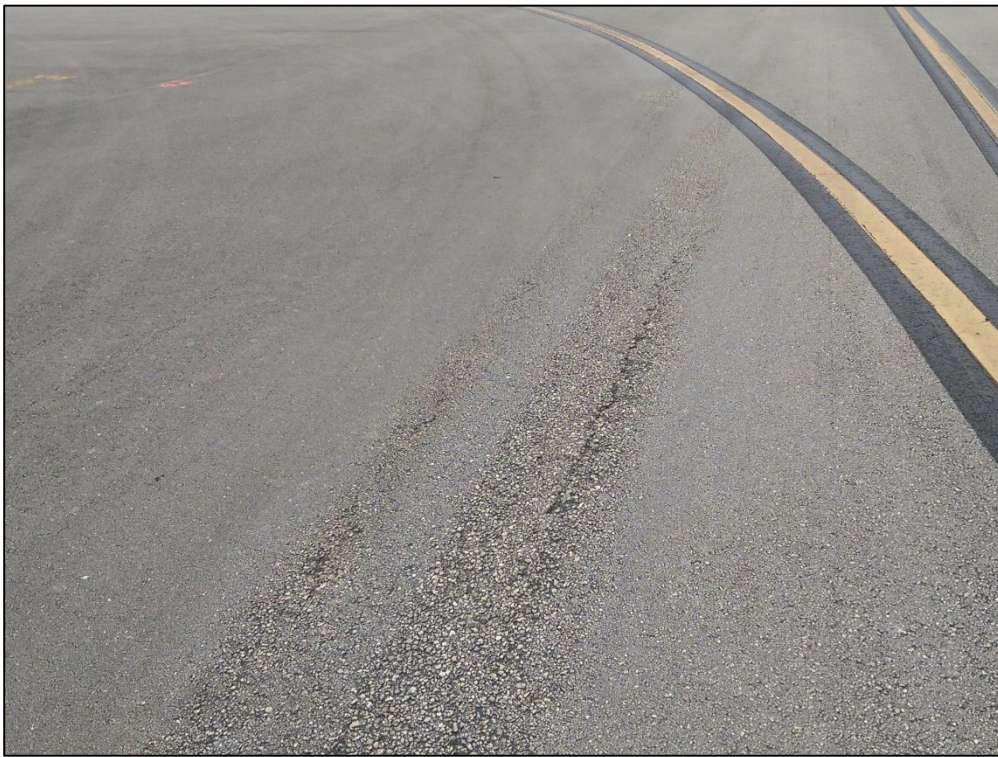
Taxiway Echo, Section 505, Sample Unit 159 – Low Severity (48) Longitudinal and Transverse Cracking, Low Severity (52) Raveling, Medium Severity (52) Raveling
