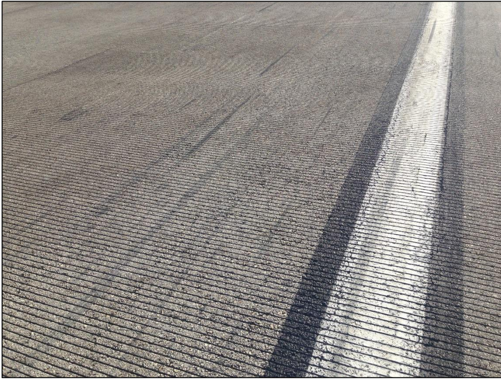
Runway 9L-27R, Section 6105, Sample Unit 383 – Low Severity (48) Longitudinal and Transverse Cracking, Low Severity (57) Weathering, Medium Severity (57) Weathering
