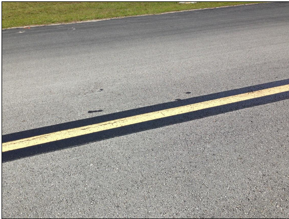
Taxiway Charlie, Section 910, Sample Unit 118 – (42) Bleeding, Low Severity (48) Longitudinal and Transverse Cracking, Low Severity (57) Weathering
