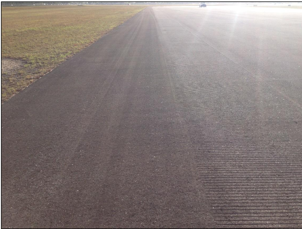
Runway 9L-27R, Section 6110, Sample Unit 184 – Low Severity (57) Weathering, Medium Severity (57) Weathering
