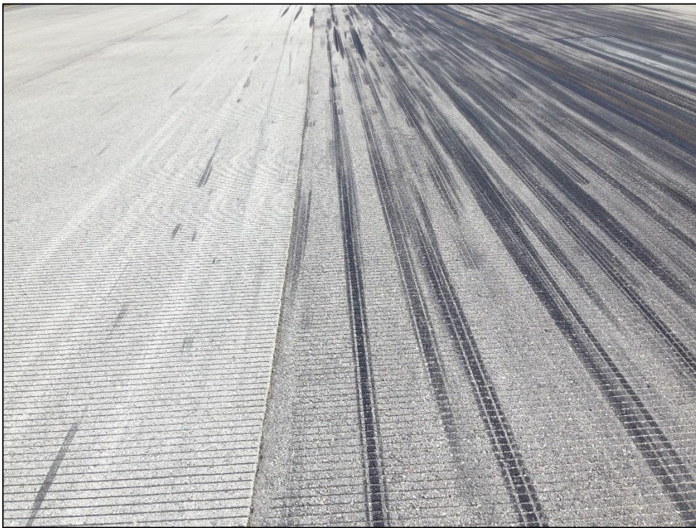
Runway 9R-27L, Section 6305, Sample Unit 325 – Low Severity (48) Longitudinal and Transverse Cracking, Low Severity (57) Weathering, Medium Severity (57) Weathering
