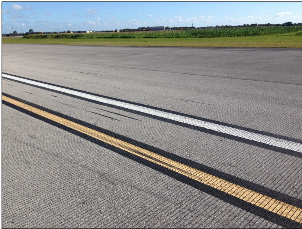
Runway 13-31, Section 6205, Sample Unit 353 – Low Severity (48) Longitudinal and Transverse Cracking, Low Severity (57) Weathering, Medium Severity (57) Weathering
