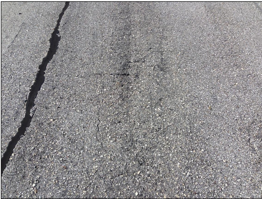
Runway 4-22, Section 6105, Sample Unit 109 – Low Severity (48) Longitudinal and Transverse Cracking, Low Severity (52) Raveling, Medium Severity (52) Raveling, Low Severity (56) Swelling
