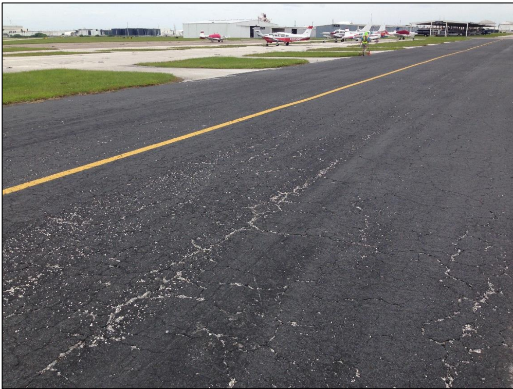
Taxiway Charlie, Section 310, Sample Unit 101 – Low Severity (43) Block Cracking, Low Severity (52) Raveling
