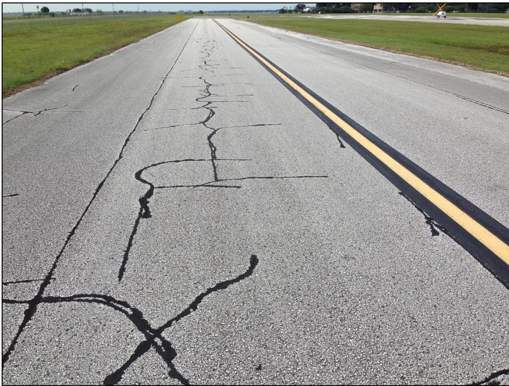
Taxiway Alpha, Section 105, Sample Unit 105 – Low Severity (48) Longitudinal and Transverse Cracking, Low Severity (52) Raveling
