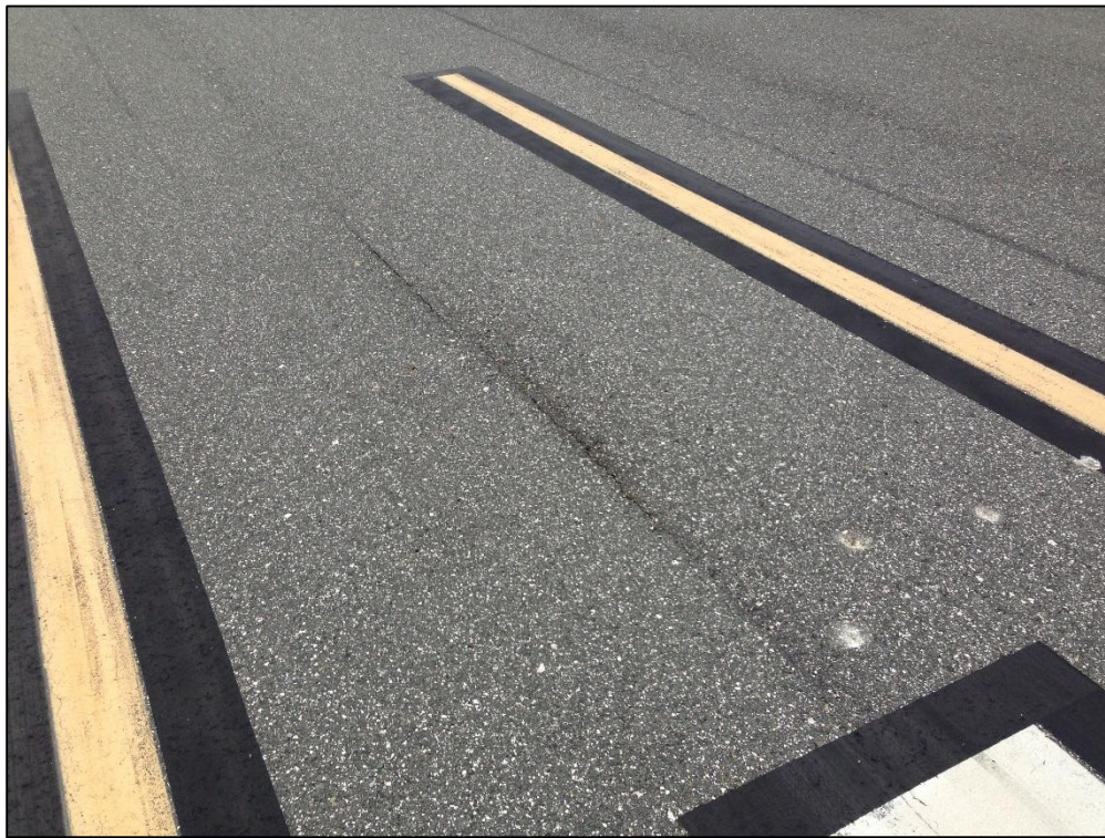
Runway 18-36, Section 6205, Sample Unit 114 – Low Severity (48) Longitudinal and Transverse Cracking, Low Severity (57) Weathering
