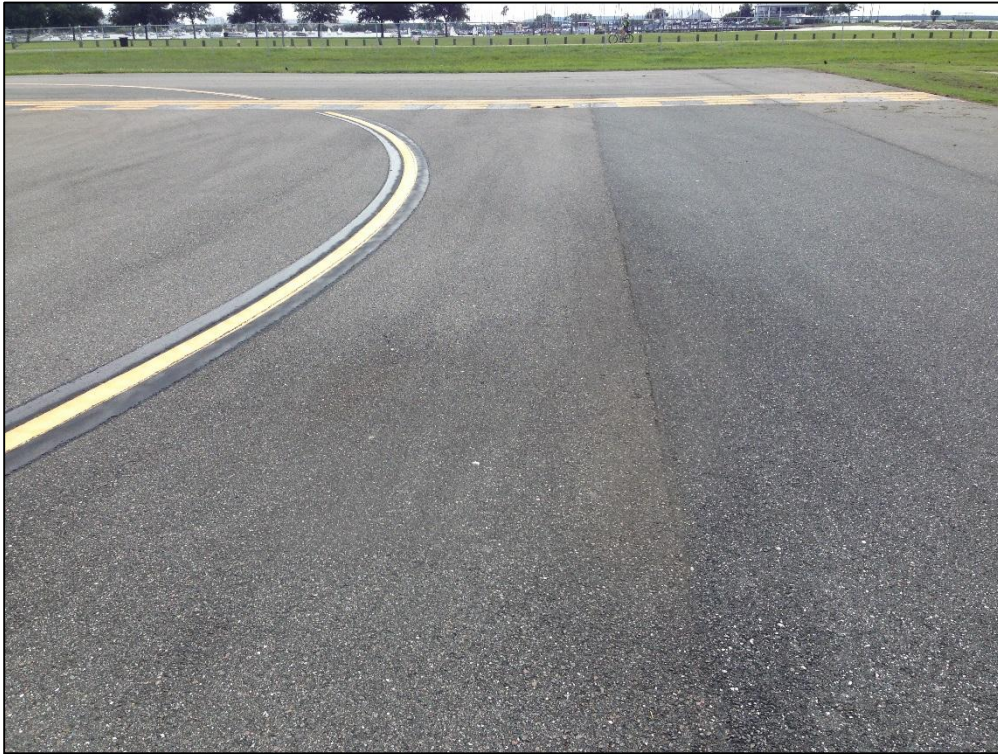
Taxiway Alpha, Section 103, Sample Unit 97 – Low Severity (45) Depression, Low Severity (48) Longitudinal and Transverse Cracking, Low Severity (57) Weathering
