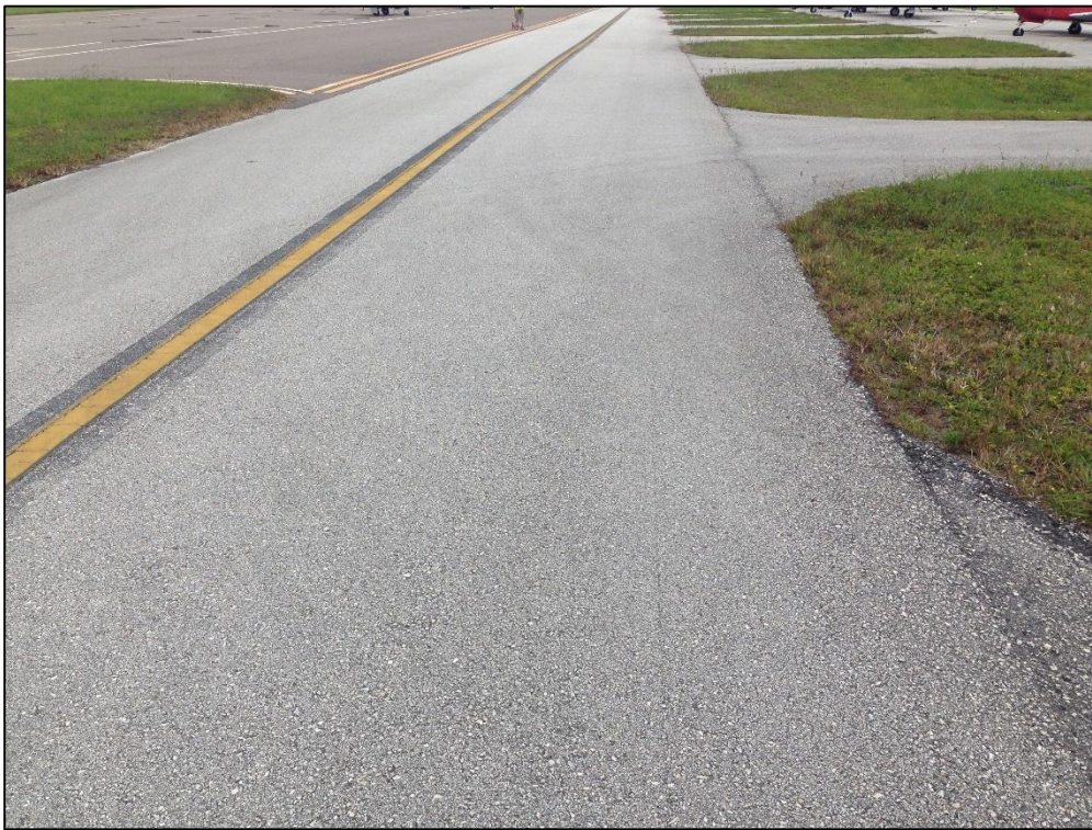
Taxiway Center, Section 315, Sample Unit 202 – Low Severity (48) Longitudinal and Transverse Cracking, Low Severity (52) Raveling, Low Severity (57) Weathering
