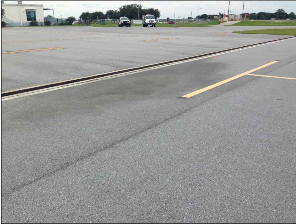
Apron, Section 4110, Sample Unit 302 – Low Severity (45) Depression, Low Severity (52) Raveling, Low Severity (57) Weathering
