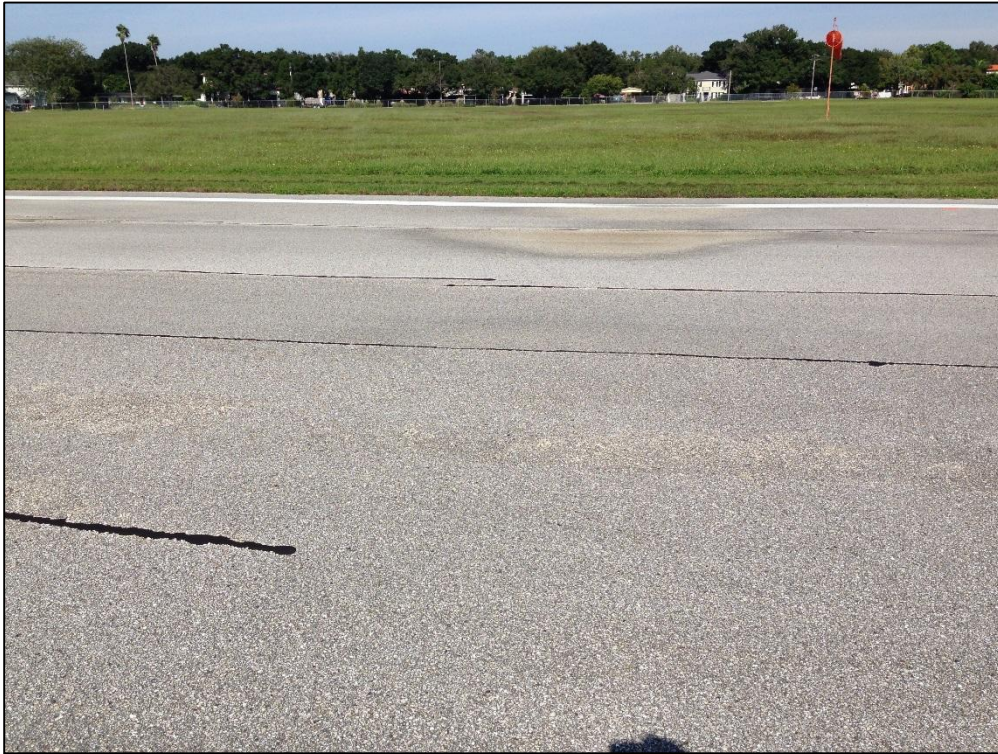
Runway 4-22, Section 6105, Sample Unit 125 – Low Severity (45) Depression, Low Severity (48) Longitudinal and Transverse Cracking, Low Severity (52) Raveling, Medium Severity (52) Raveling, Low Severity (56) Swelling
