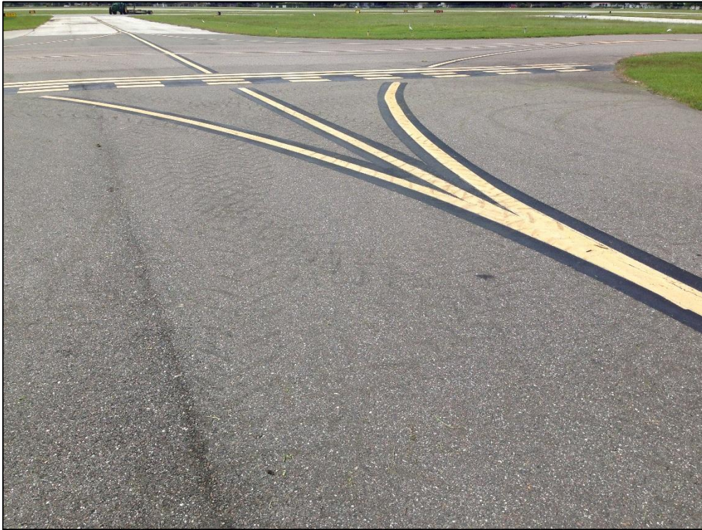
Taxiway Echo, Section 650, Sample Unit 300 – Low Severity (48) Longitudinal and Transverse Cracking, Low Severity (57) Weathering
