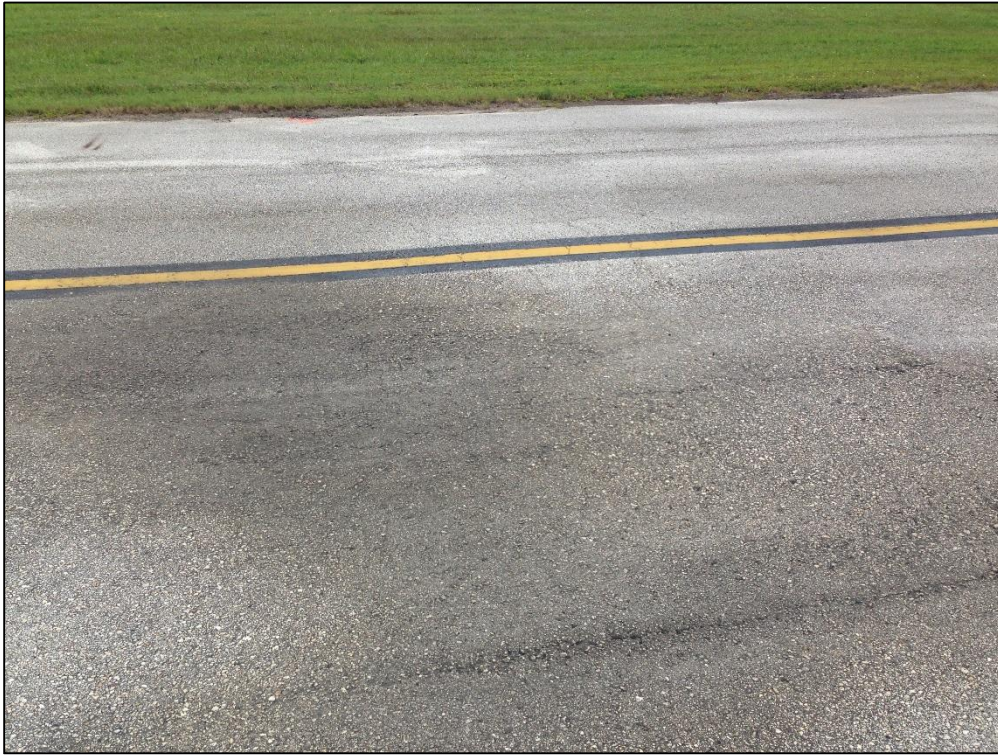
Taxiway Echo, Section 510, Sample Unit 100 – Low Severity (45) Depression , Low Severity (48) Longitudinal and Transverse Cracking, Low Severity (52) Raveling
