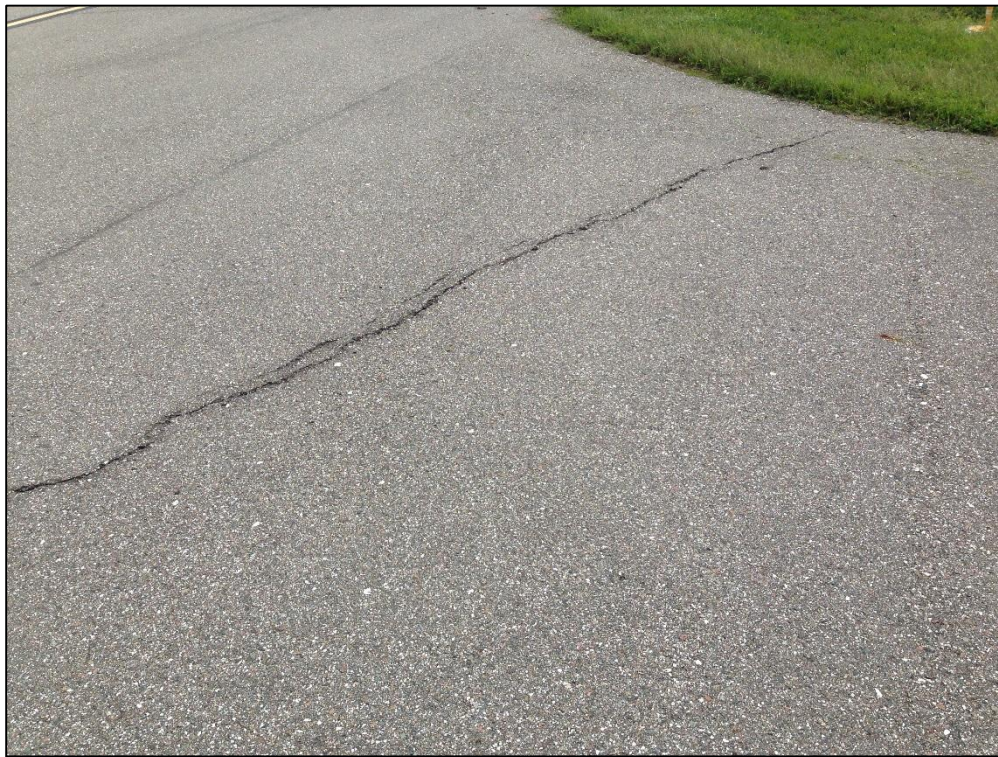
Apron Run-Up, Section 5110, Sample Unit 100 – Low Severity (48) Longitudinal and Transverse Cracking, Low Severity (57) Weathering
