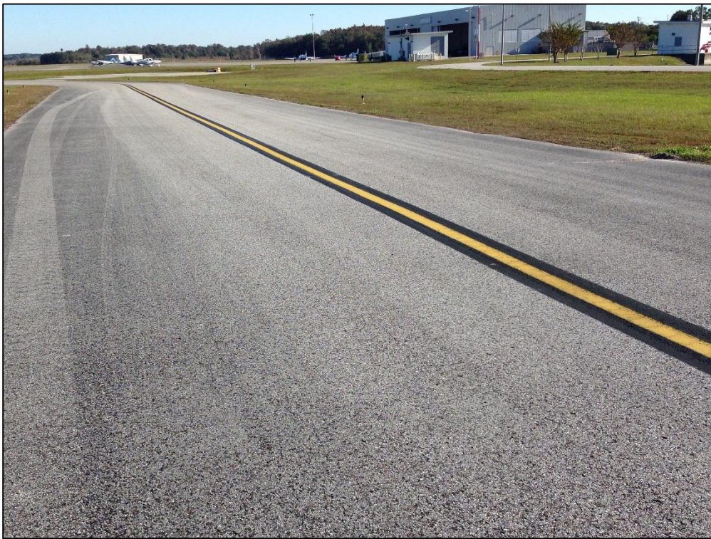
Taxiway Charlie, Section 405, Sample Unit 103 – Low Severity (52) Raveling, Medium Severity (57) Weathering
