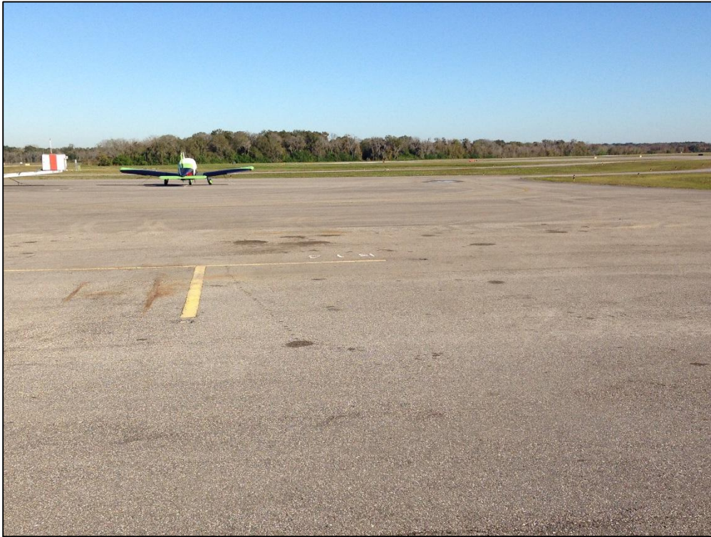
North Apron B, Section 4205, Sample Unit 352 – Low Severity (52) Raveling, Medium Severity (57) Weathering
