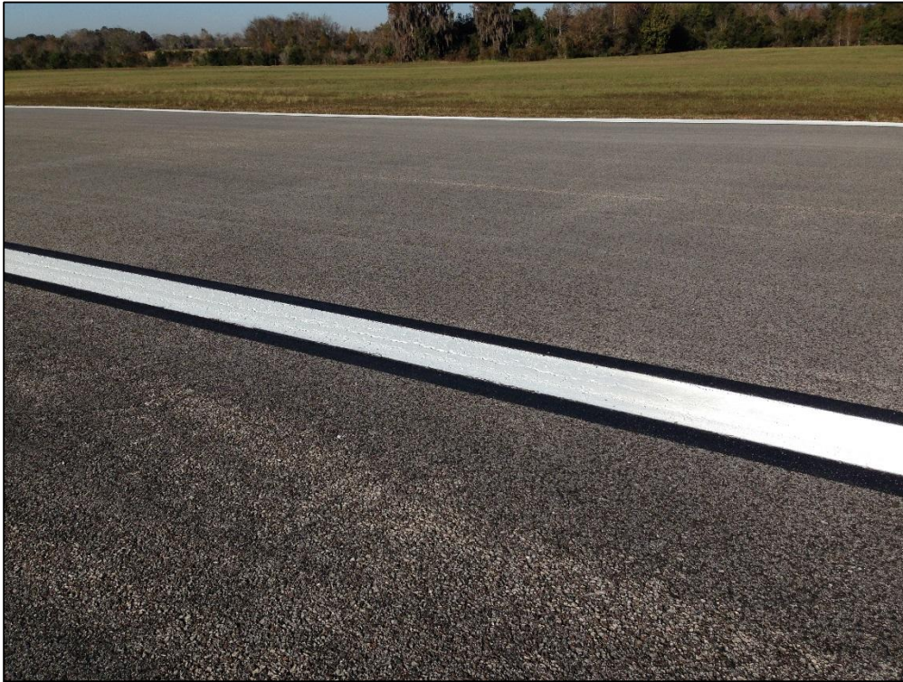
Runway 5-23, Section 6205, Sample Unit 191 – Low Severity (48) Longitudinal and Transverse Cracking, Low Severity (52) Raveling, Low Severity (57) Weathering
