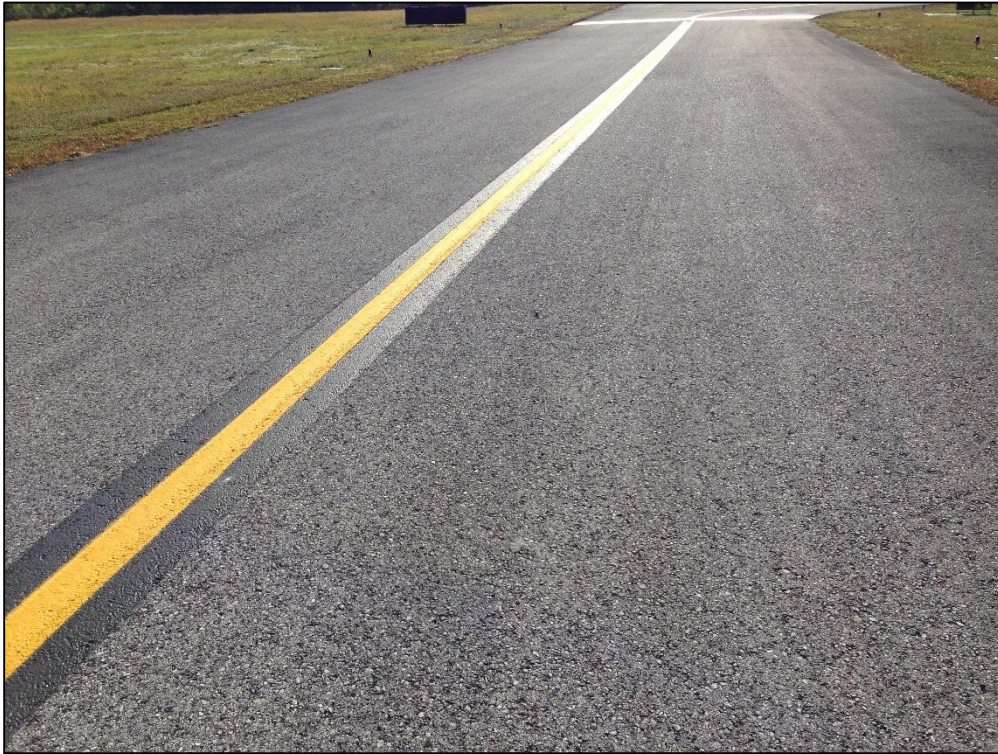
Taxiway E4, Section 525, Sample Unit 101 – Medium Severity (57) Weathering
