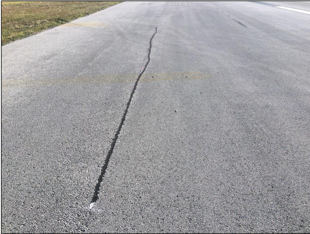
Runway 18-36, Section 6105, Sample Unit 156 – Low Severity (48) Longitudinal and Transverse Cracking, Medium Severity (57) Weathering
