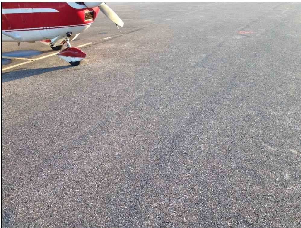
South Apron A, Section 4105, Sample Unit 400 – Low Severity (56) Swelling, Medium Severity (57) Weathering
