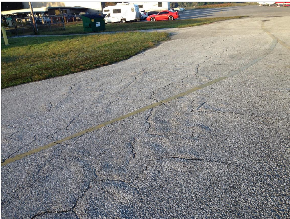
Taxiway Bravo, Section 210, Sample Unit 203 – Low Severity (43) Block Cracking, Medium Severity (52) Raveling, Low Severity (56) Swelling
