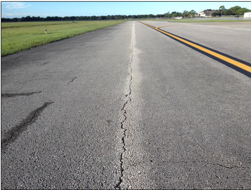
Taxiway B, Section 205, Sample Unit 207 – Low Severity (48) Longitudinal and Transverse Cracking, Low Severity (52) Raveling, Low Severity (57) Weathering
