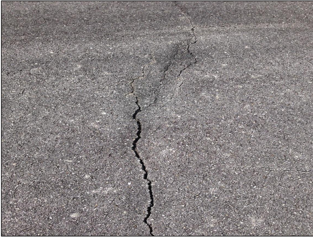
Taxiway C1, Section 345, Sample Unit 308 – Medium Severity (48) Longitudinal and Transverse Cracking, Low Severity (57) Weathering
