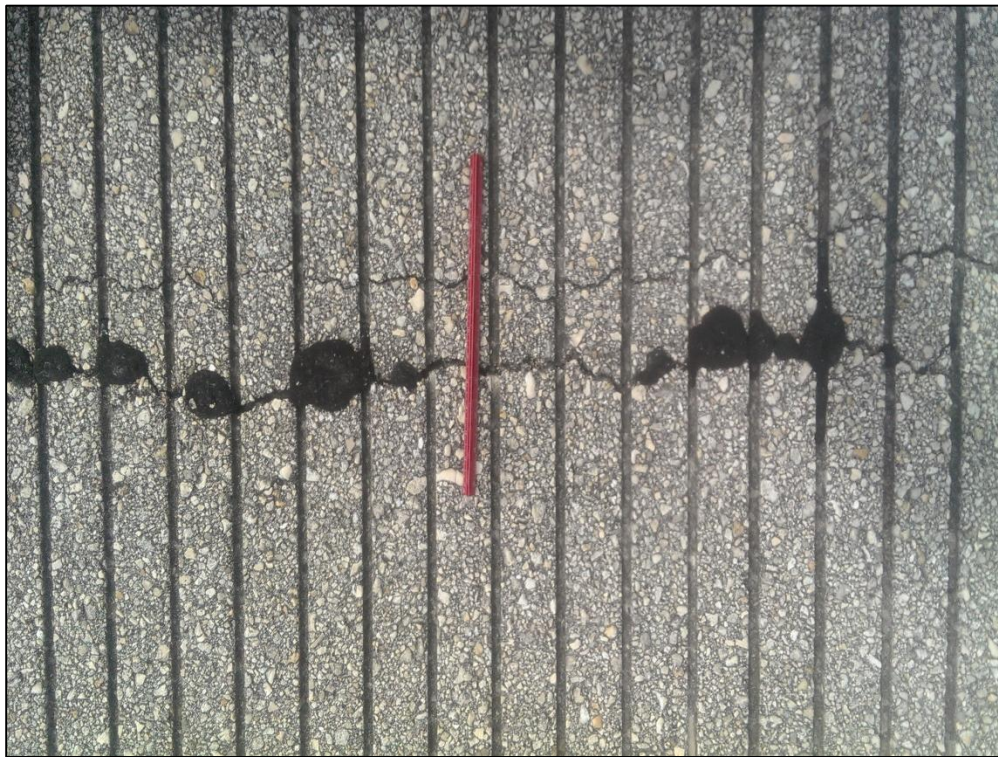
Runway 12R-30L, Section 6110, Sample Unit 181 – (42) Bleeding, Low Severity (41) Alligator Cracking
