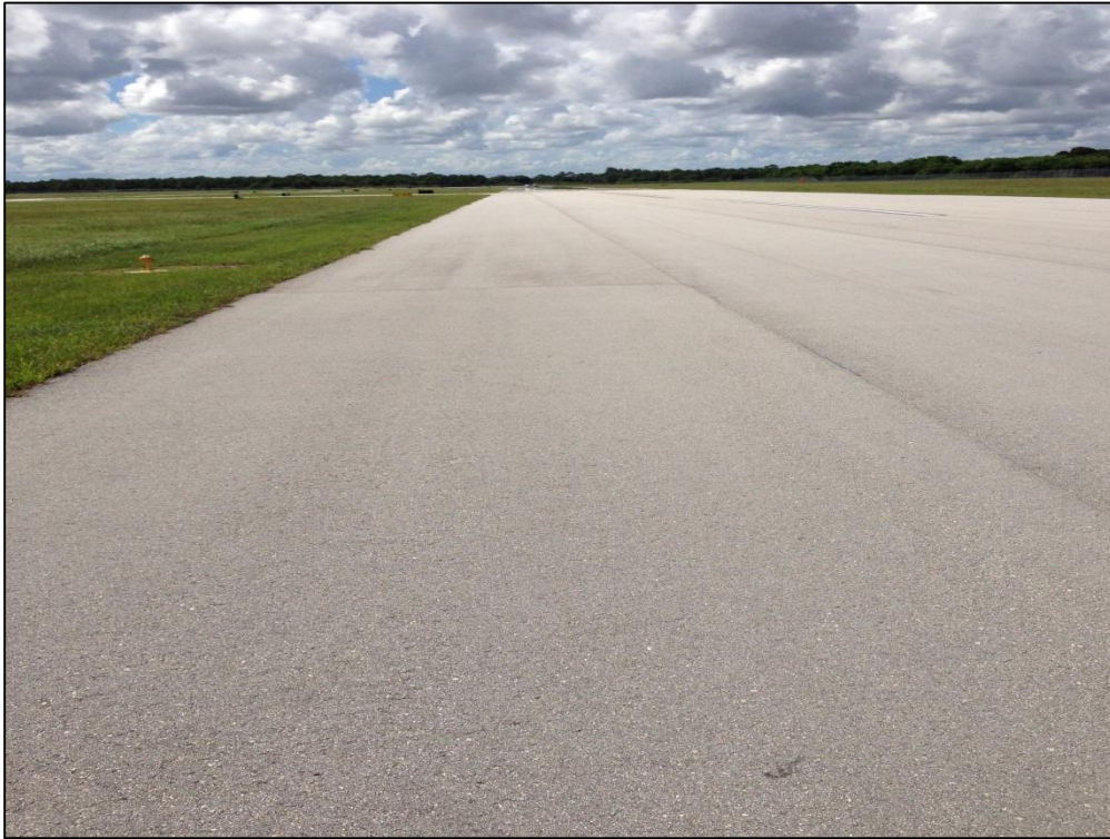
Runway 12L-30R, Section 6210, Sample Unit 516 – Low Severity (57) Weathering
