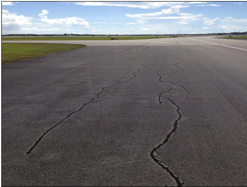
Taxiway C, Section 305, Sample Unit 316 – Low Severity (48) Longitudinal and Transverse Cracking
