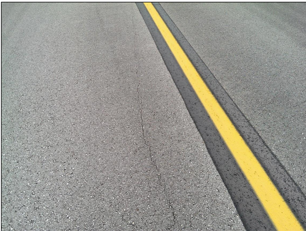
Taxiway D, Section 418, Sample Unit 408 – Low Severity (48) Longitudinal and Transverse Cracking, Low Severity (57) Weathering
