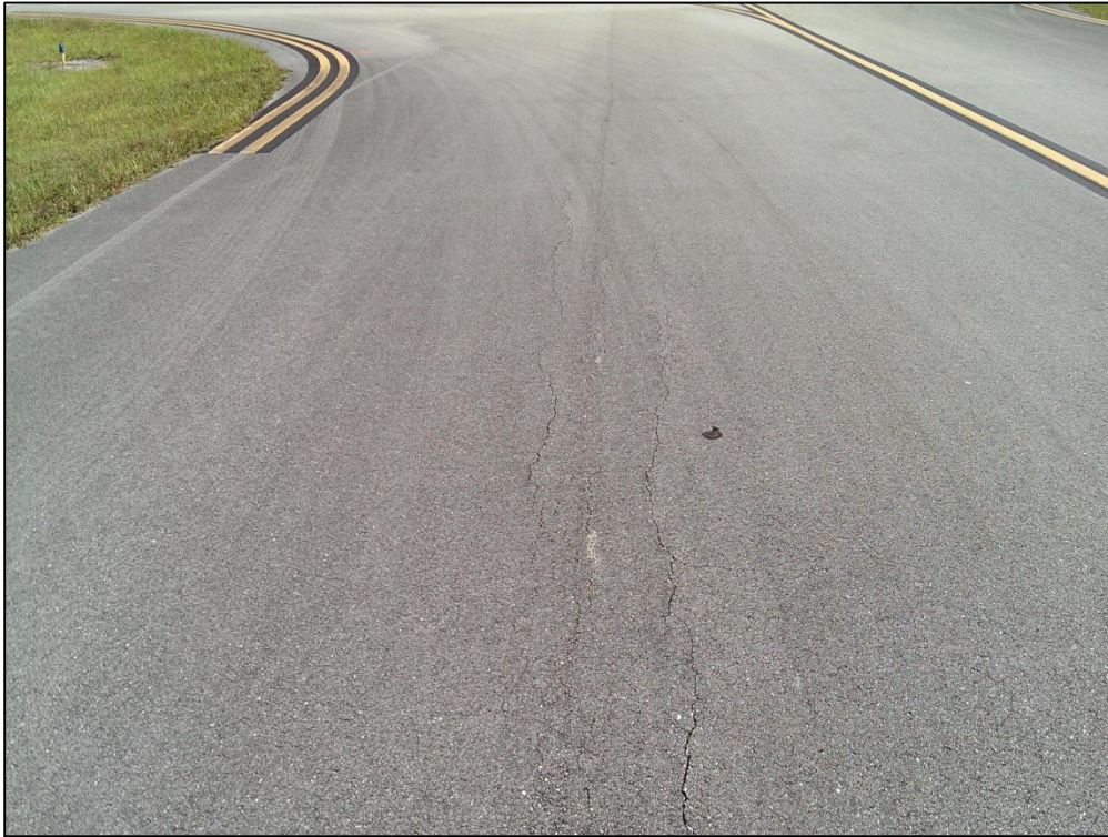
Taxiway A, Section 125, Sample Unit 126 – Low Severity (41) Alligator Cracking, Low Severity (57) Weathering,
