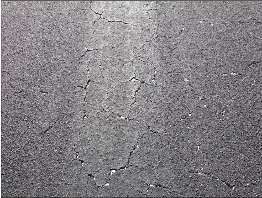
Apron W, Section 4405, Sample Unit 202 – Medium Severity (57) Weathering
