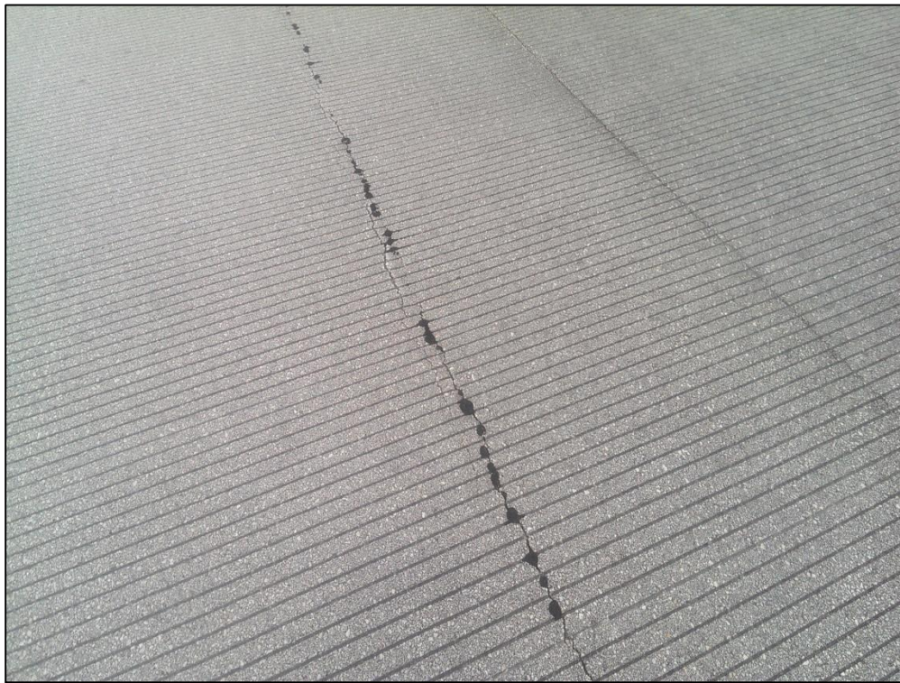
Runway 12R-30L, Section 6110, Sample Unit 181 – Low Severity (48) Longitudinal and Transverse Cracking, (42) Bleeding, Low Severity (41) Alligator Cracking
