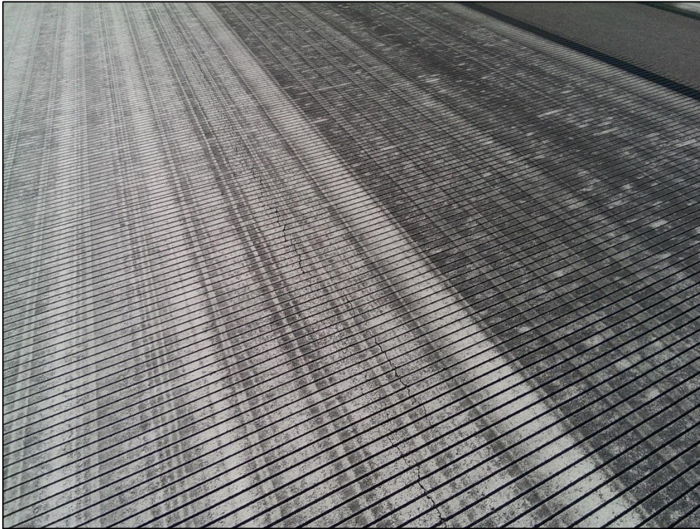
Runway 12R-30L, Section 6105, Sample Unit 122 – Low Severity (48) Longitudinal and Transverse Cracking, Low Severity (57) Weathering
