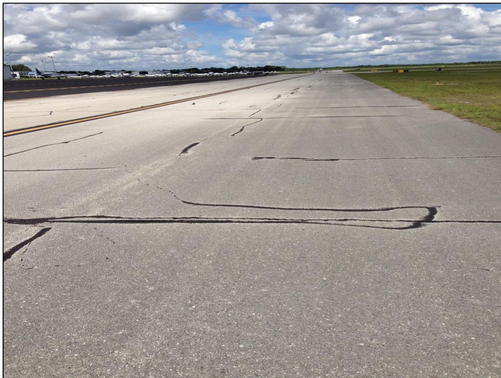
Taxiway C, Section 315, Sample Unit 318 – Low Severity (48) Longitudinal and Transverse Cracking, Low Severity (57) Weathering
