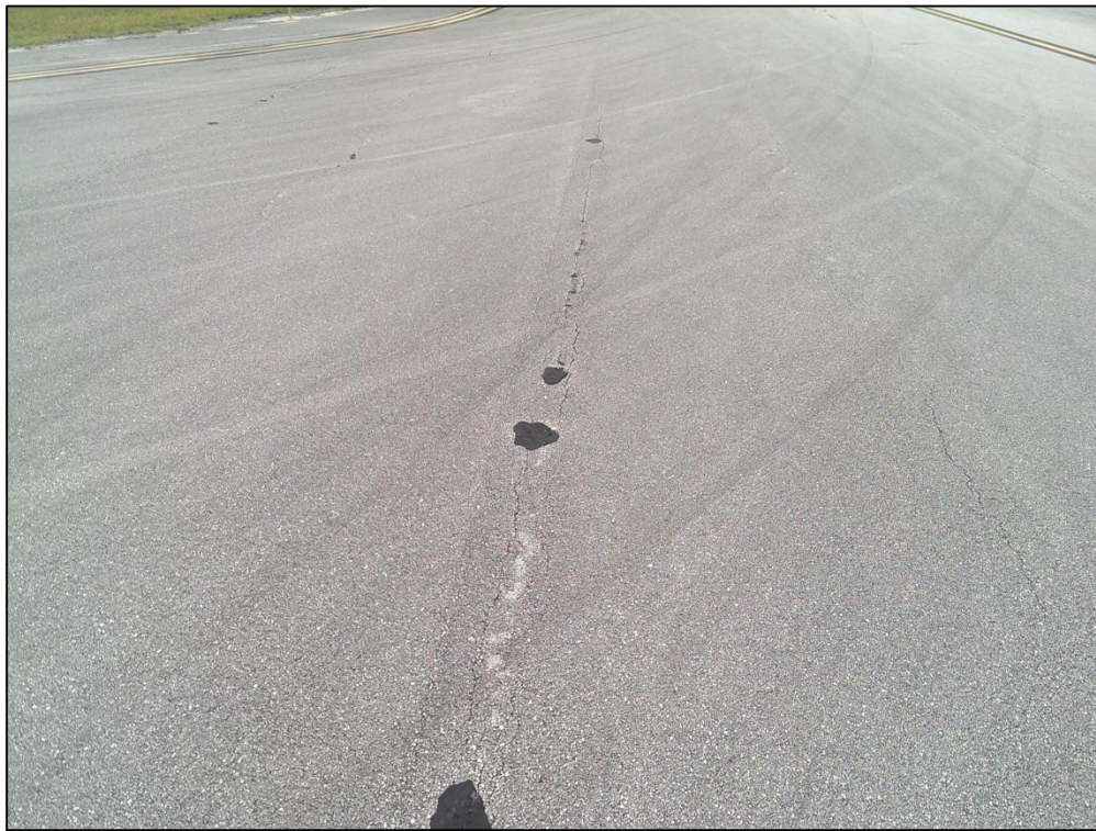
Taxiway C2, Section 350, Sample Unit 201 – Low Severity (41) Alligator Cracking, (42) Bleeding, Low Severity (48) Longitudinal and Transverse Cracking
