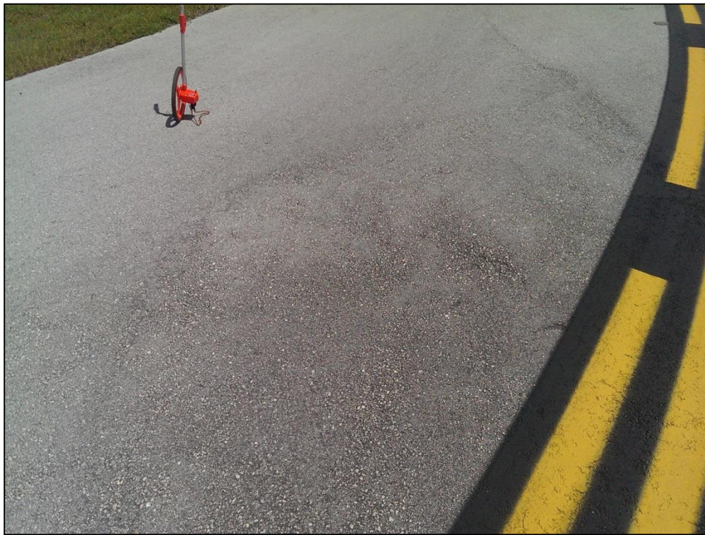
Taxiway F, Section 615, Sample Unit 615 – Low Severity (52) Raveling
