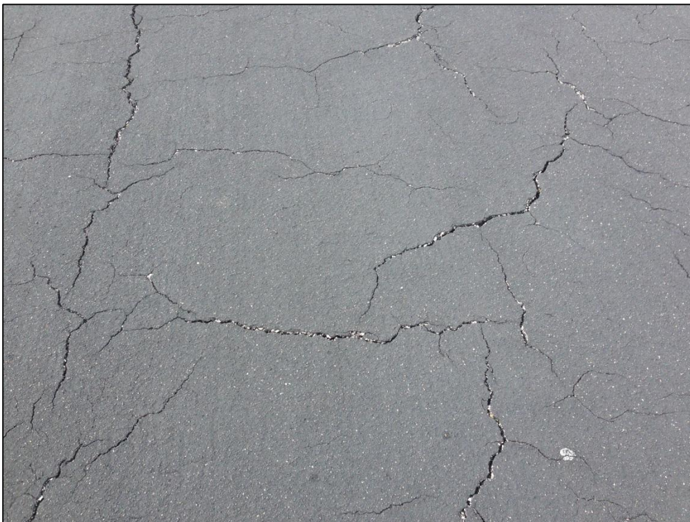
Apron CENTER, Section 4205, Sample Unit 503 – Low Severity (43) Block Cracking, Medium Severity (57) Weathering
