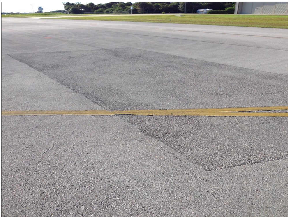
Apron RU 12R, Section 5205, Sample Unit 204 – Medium Severity (50) Patching, Low Severity (57) Weathering
