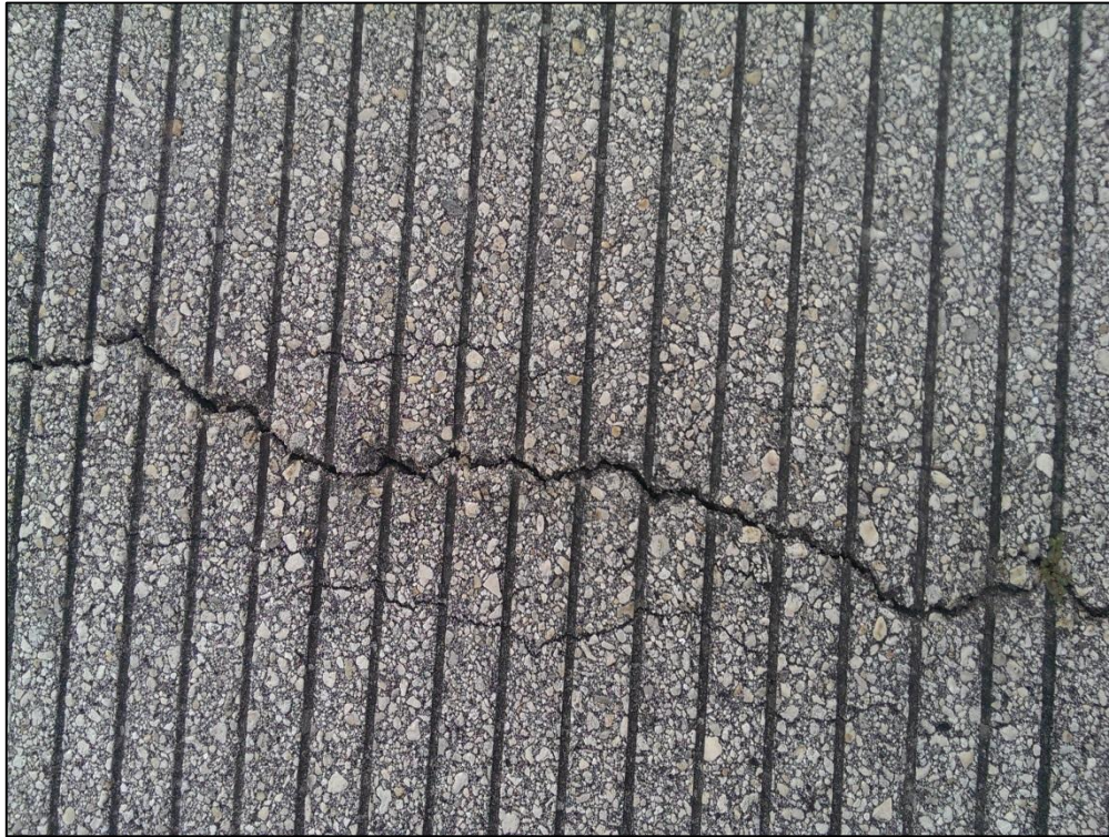
Runway 12R-30L, Section 6110, Sample Unit 195 – Low Severity (41) Alligator Cracking
