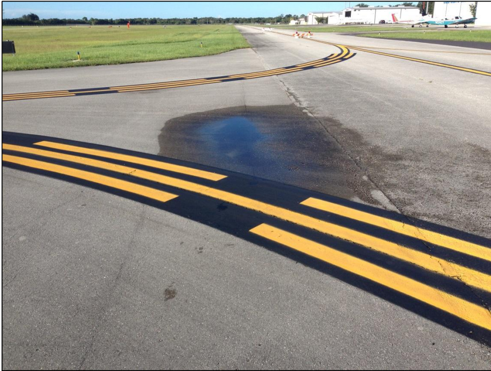
Taxiway B1, Section 151, Sample Unit 100 – Low Severity (45) Depression, Low Severity (57) Weathering
