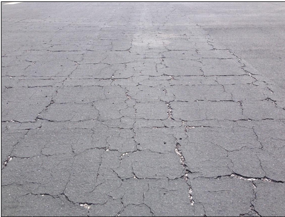
Apron CENTER, Section 4240, Sample Unit 663 – Low Severity (43) Block Cracking, Medium Severity (57) Weathering
