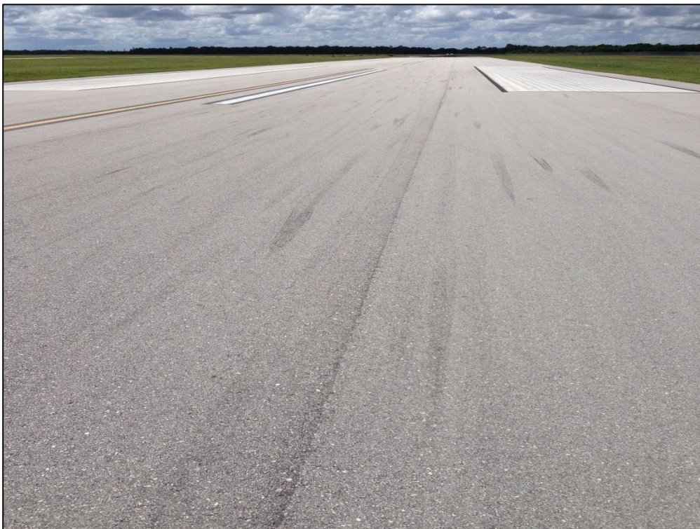
Runway 12L-30R, Section 6215, Sample Unit 128 – Low Severity (57) Weathering
