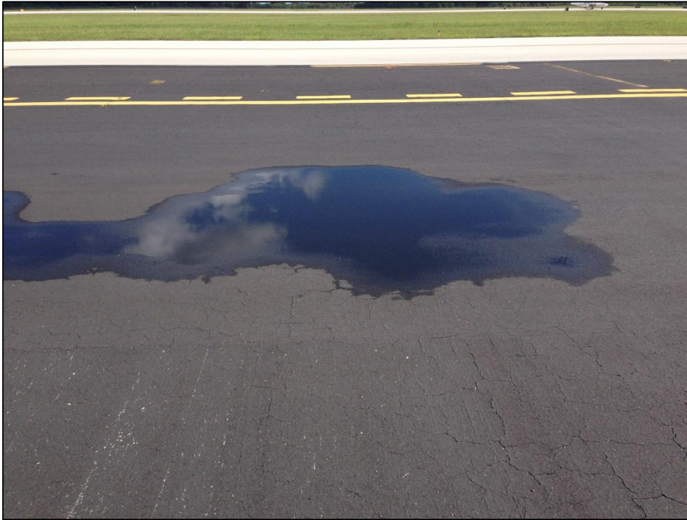
Apron CENTER, Section 4215, Sample Unit 706 – Low Severity (43) Block Cracking, Low Severity (45) Depression, Medium Severity (57) Weathering
