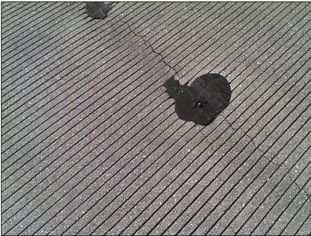
Runway 12R-30L, Section 6110, Sample Unit 134 – Low Severity (48) Longitudinal and Transverse Cracking, (42) Bleeding
