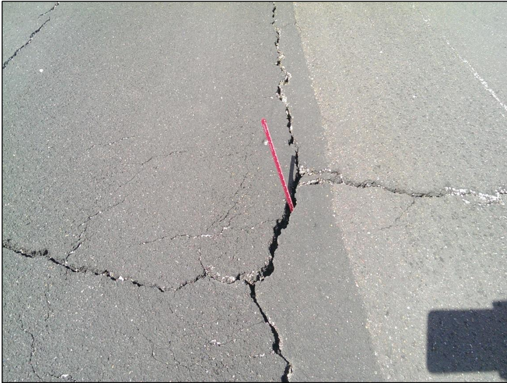
Apron NE, Section 5405, Sample Unit 102 – Medium Severity (43) Block Cracking, Low Severity (52) Raveling
