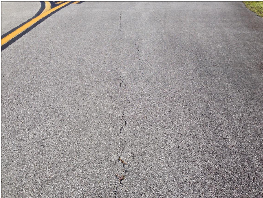
Taxiway B, Section 206, Sample Unit 223 – Low Severity (48) Longitudinal and Transverse Cracking, Low Severity (57) Weathering
