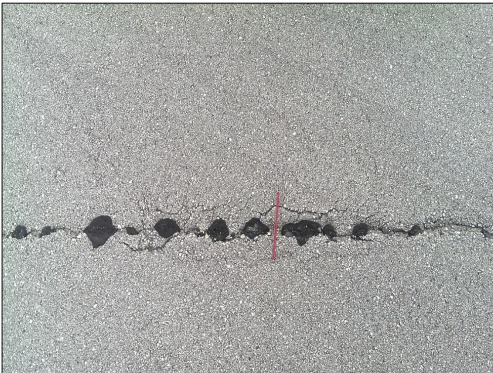
Taxiway D, Section 405, Sample Unit 400 – Low Severity (41) Alligator Cracking, (42) Bleeding
