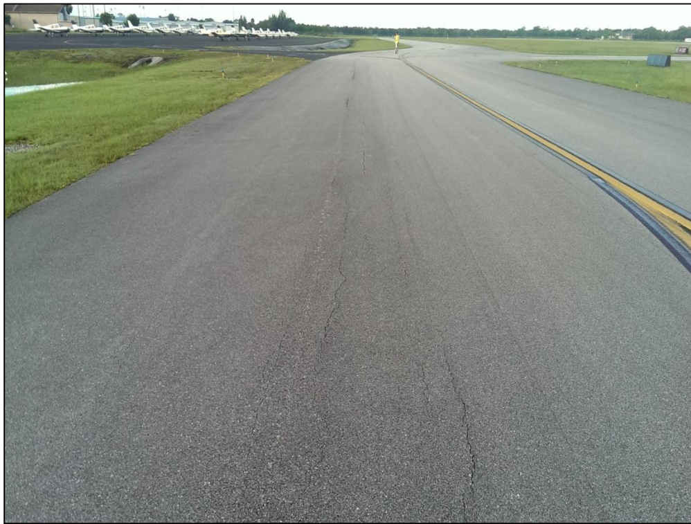
Taxiway A, Section 110, Sample Unit 116 –Medium and Low Severity (48) Longitudinal and Transverse Cracking, Low Severity (57) Weathering, and Low Severity (52) Raveling
