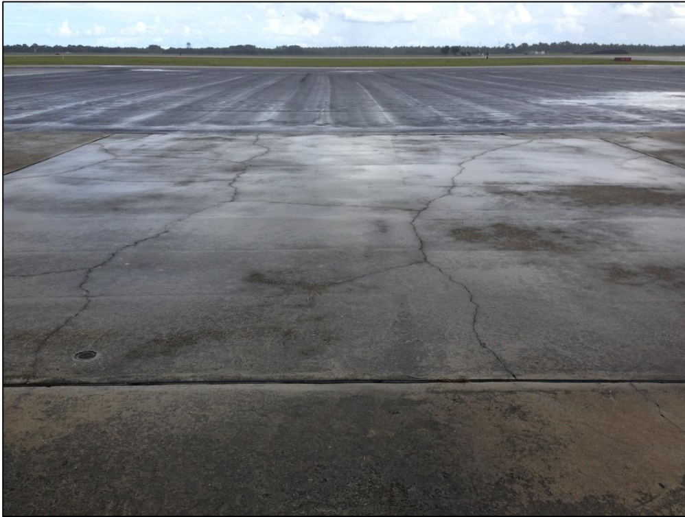
Apron CENTER, Section 4235, Sample Unit 100 – Medium Severity (72) Shattered Slab
