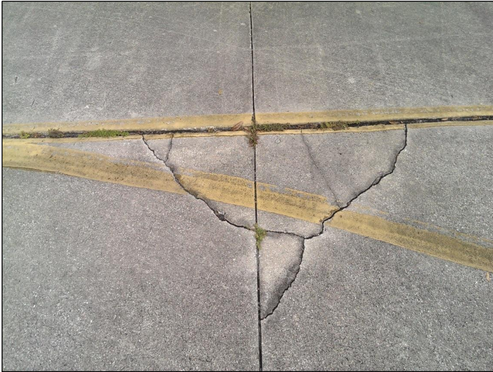
Apron SW, Section 4115, Sample Unit 203 – Medium Severity (62) Corner Break
