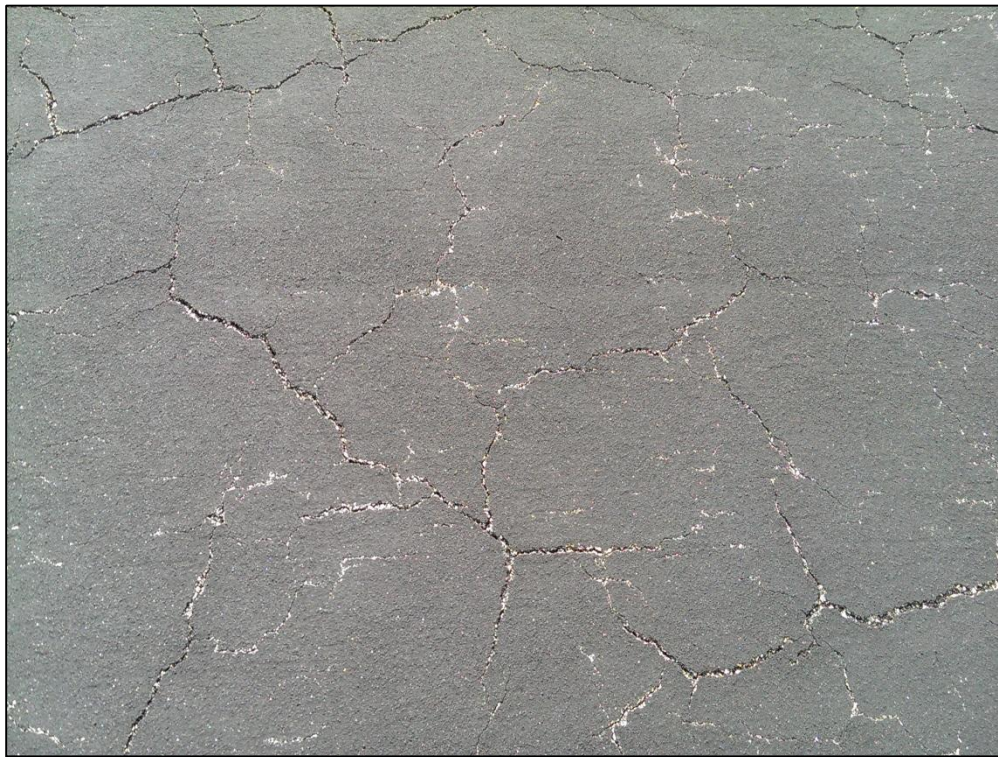
Apron SW, Section 4105, Sample Unit 156 – Low Severity (43) Block Cracking, Medium Severity (52) Raveling
