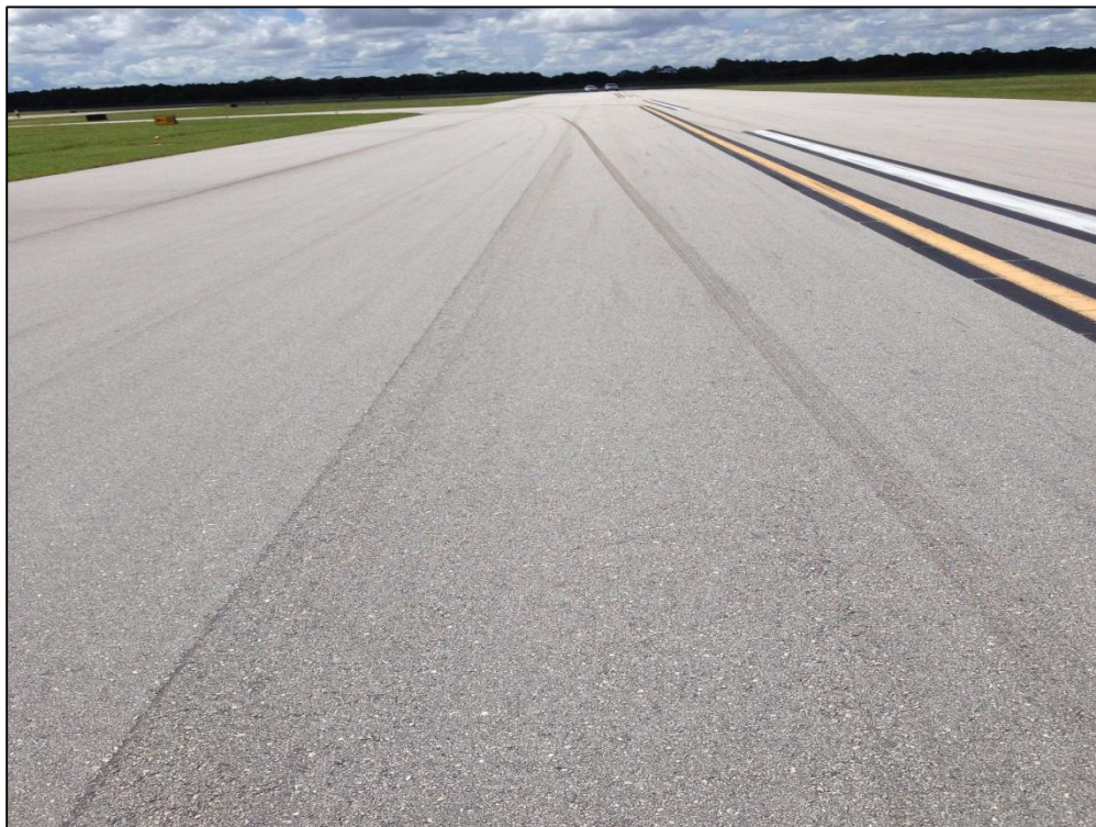
Runway 12L-30R, Section 6205, Sample Unit 308 – Low Severity (57) Weathering
