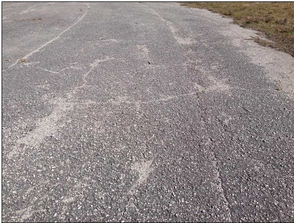
Taxiway Foxtrot, Section 550, Sample Unit 145 – Medium Severity (43) Block Cracking, High Severity (52) Raveling
