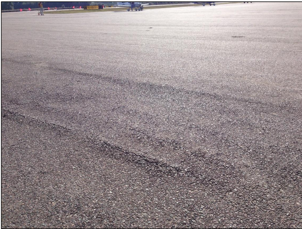
Apron, Section 4105, Sample Unit 300 – Low Severity (48) Longitudinal and Transverse Cracking, Low Severity (56) Swelling, Low Severity (57) Weathering
