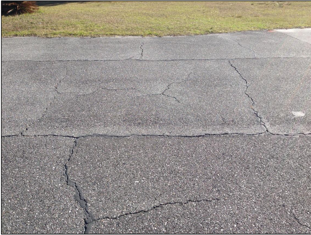
Apron T-Hangars, Section 4315, Sample Unit 100 – Low Severity (48) Longitudinal and Transverse Cracking, Low Severity (52) Raveling
