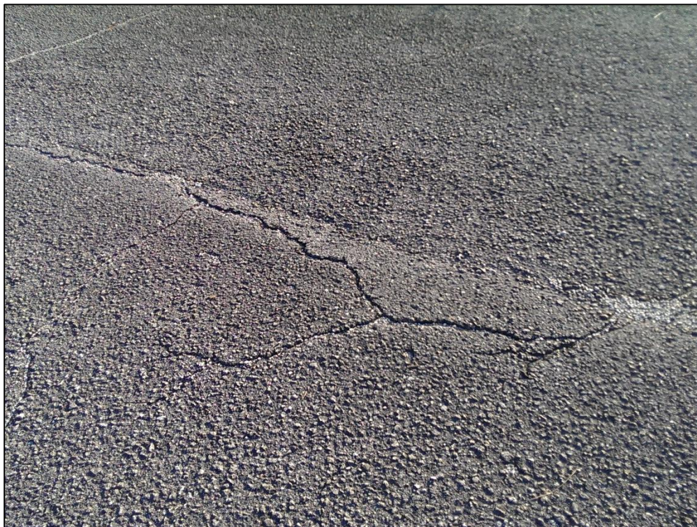
Taxiway Golf, Section 450, Sample Unit 105 – Medium Severity (43) Block Cracking, High Severity (52) Raveling
