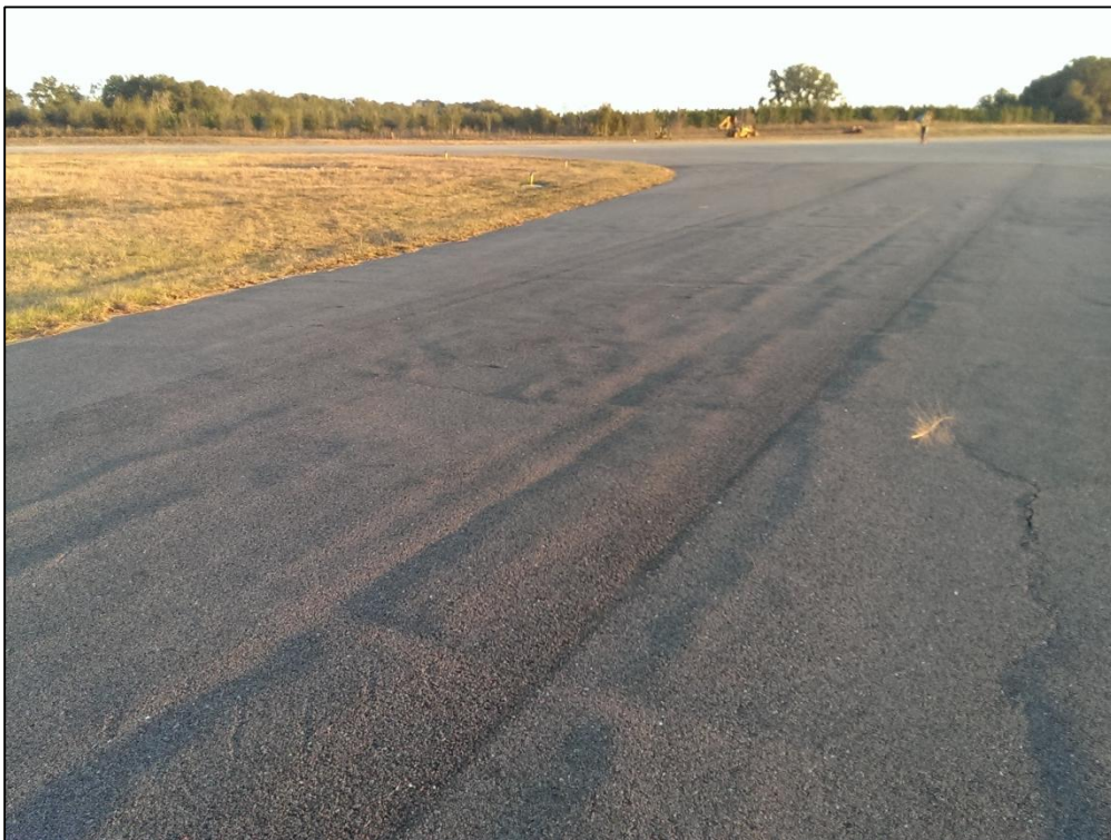
Taxiway Charlie, Section 105, Sample Unit 101 – Low Severity (48) Longitudinal and Transverse Cracking, Low Severity (56) Swelling, Low Severity (57) Weathering
