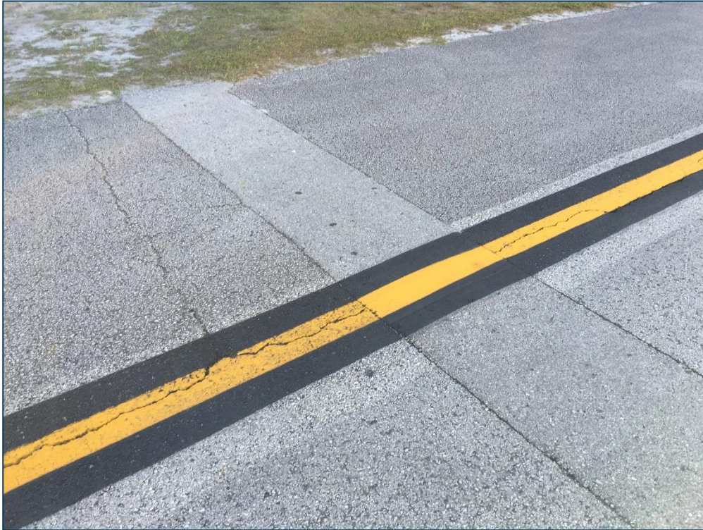
T-Hangars Taxiway, Section 710, Sample Unit 200 – Low Severity (48) Longitudinal and Transverse Cracking, Low Severity (50) Patching, Low Severity (52) Raveling, Medium Severity (52) Raveling
