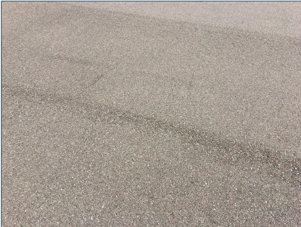
Apron, Section 4105, Sample Unit 502 – Low Severity (52) Raveling, Low Severity (57) Weathering
