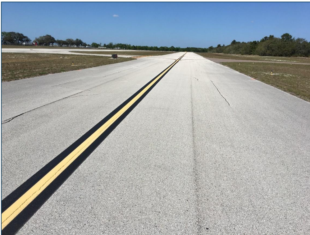
Taxiway A, Section 110, Sample Unit 115 – Low Severity (48) Longitudinal and Transverse Cracking, Low Severity (52) Raveling
