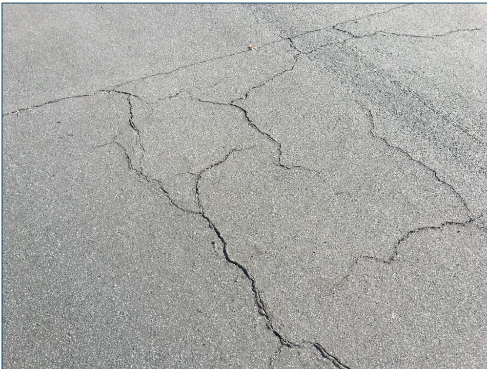
Apron, Section 4130, Sample Unit 610 – Low Severity (43) Block Cracking, Low Severity (48) Longitudinal and Transverse Cracking, Low Severity (57) Weathering
