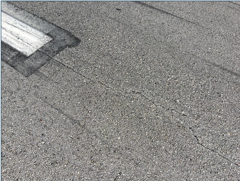
Runway 10-28, Section 6120, Sample Unit 366 – Low Severity (48) Longitudinal and Transverse Cracking, Low Severity (52) Raveling, Medium Severity (52) Raveling
