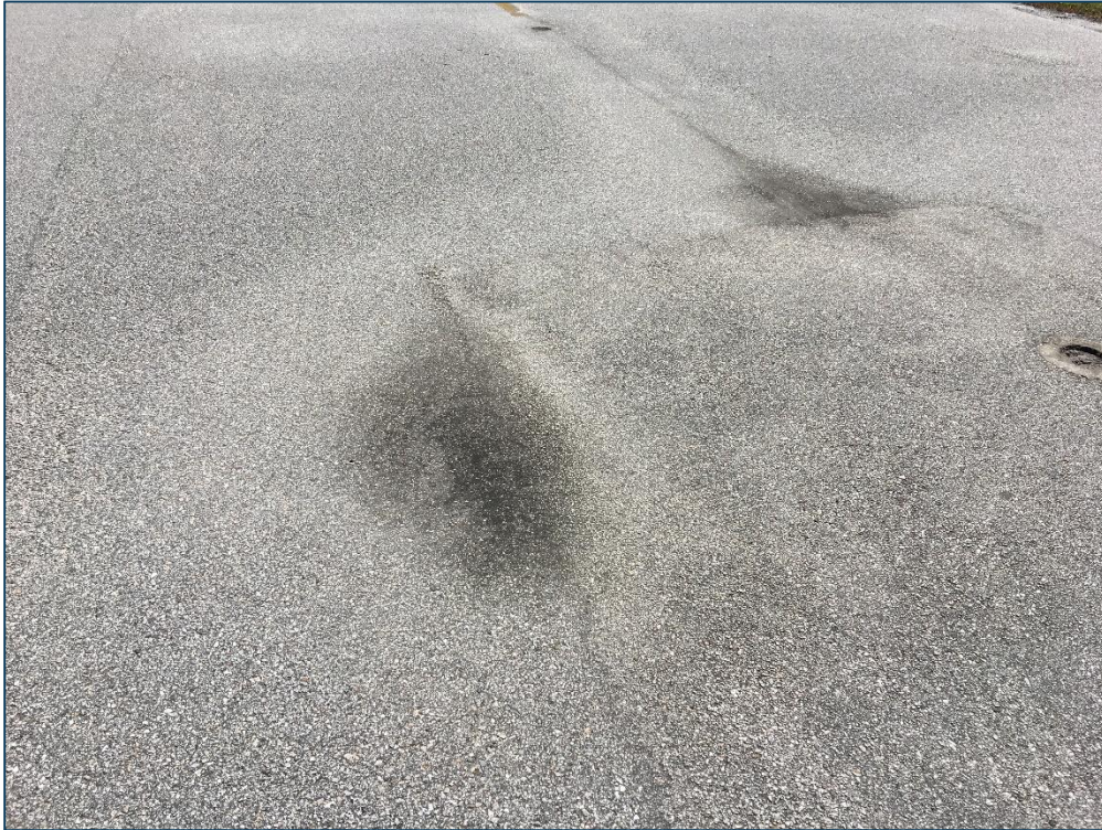
Apron, Section 4135, Sample Unit 111 – Low Severity (45) Depression, Low Severity (52) Raveling
