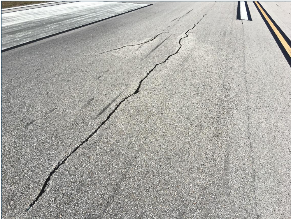
Runway 10-28, Section 6115, Sample Unit 321 – Low Severity (48) Longitudinal and Transverse Cracking, Low Severity (52) Raveling, Medium Severity (52) Raveling
