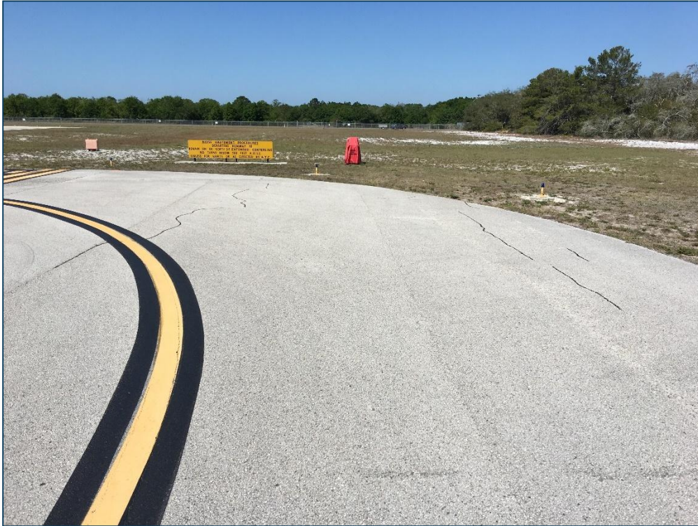
Taxiway A, Section 110, Sample Unit 101 – Low Severity (48) Longitudinal and Transverse Cracking, Low Severity (52) Raveling
