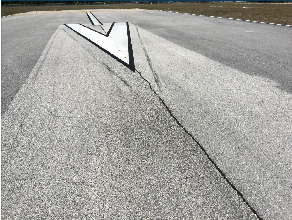
Runway 10-28, Section 6103, Sample Unit 296 – Low Severity (48) Longitudinal and Transverse Cracking, Low Severity (52) Raveling, Medium Severity (52) Raveling, Low Severity (56) Swelling
