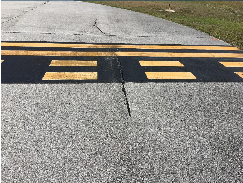
Taxiway A, Section 115, Sample Unit 600 – Medium Severity (48) Longitudinal and Transverse Cracking, Low Severity (52) Raveling, Medium Severity (52) Raveling
