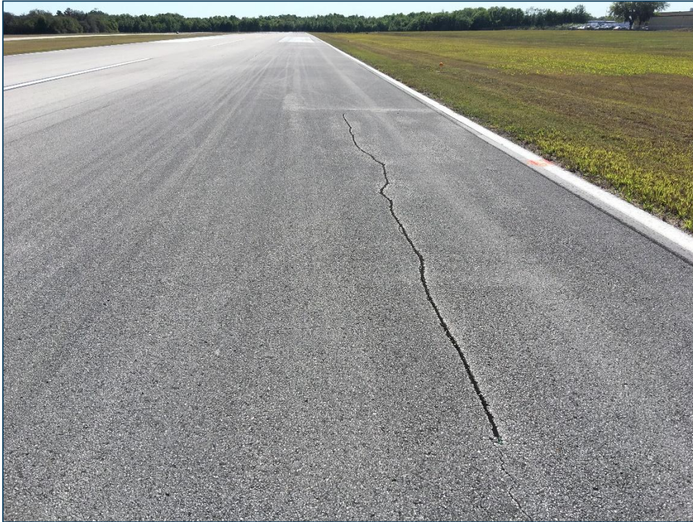
Runway 10-28, Section 6115, Sample Unit 346 – Low Severity (48) Longitudinal and Transverse Cracking, Low Severity (52) Raveling, Medium Severity (52) Raveling
