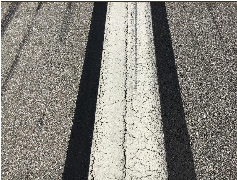
Runway 13-31, Section 6110, Sample Unit 176 – Low Severity (48) Longitudinal and Transverse Cracking, Low Severity (57) Weathering
