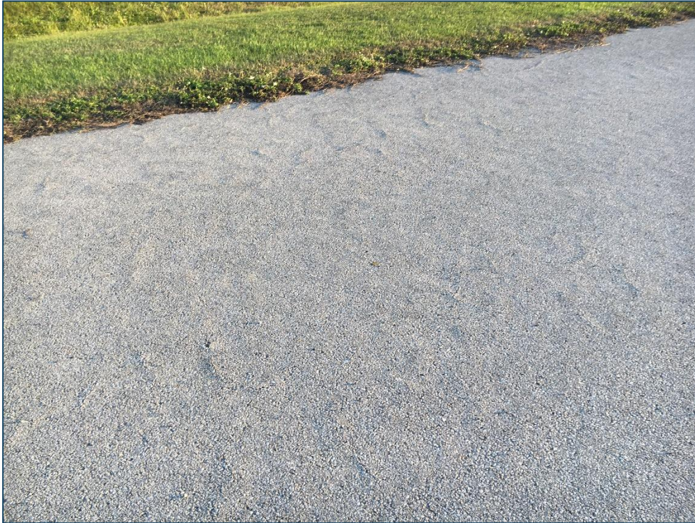
Taxiway to East Apron, Section 710, Sample Unit 101 – Low Severity (48) Longitudinal and Transverse Cracking, Low Severity (52) Raveling
