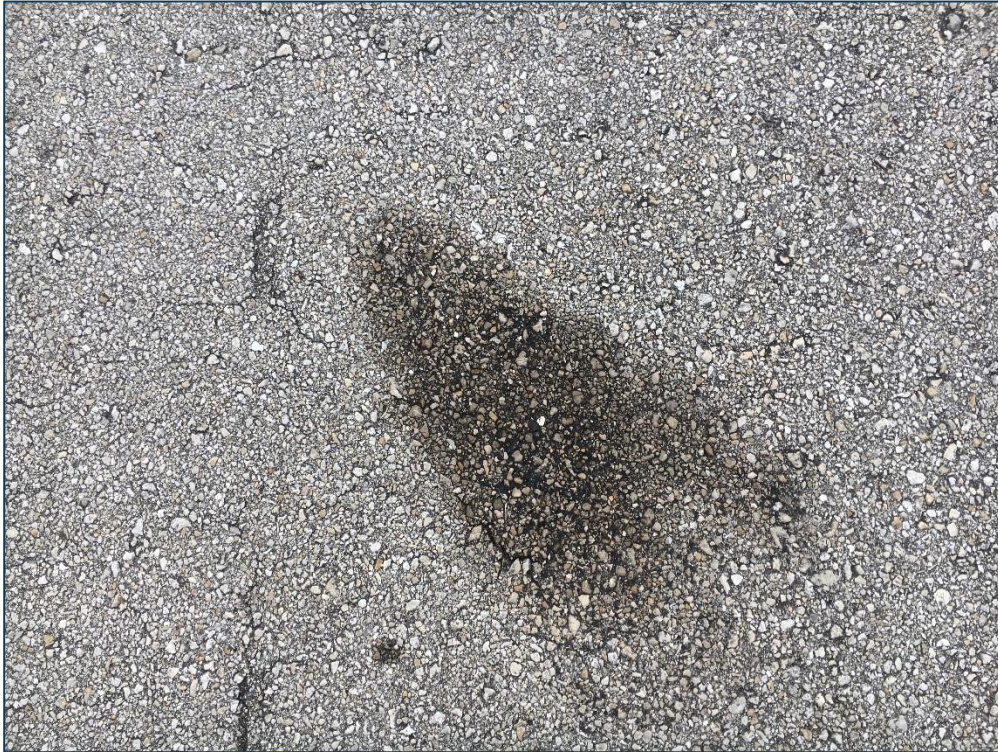
Apron Hangar, Section 4210, Sample Unit 201 – (49) Oil Spillage, Low Severity (57) Weathering
