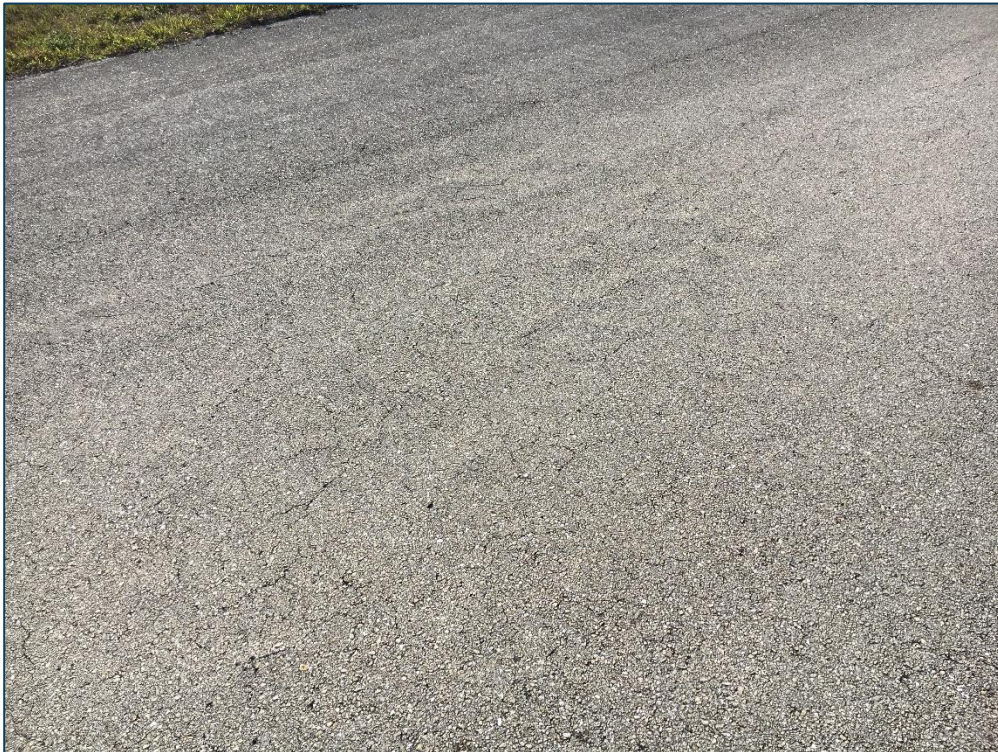
Taxiway A, Section 105, Sample Unit 108 – Low Severity (48) Longitudinal and Transverse Cracking, Low Severity (56) Swelling, Low Severity (57) Weathering
