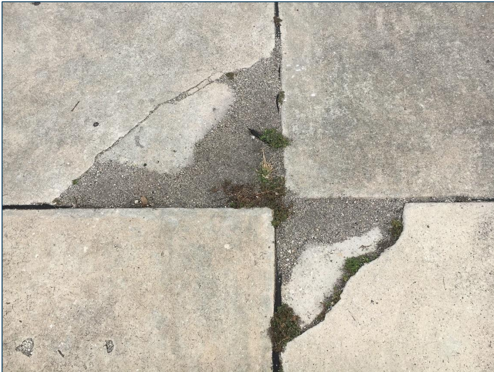
Apron Hangar, Section 4205, Sample Unit 100 – High Severity (62) Corner Break, Medium Severity (65) Joint Seal Damage
