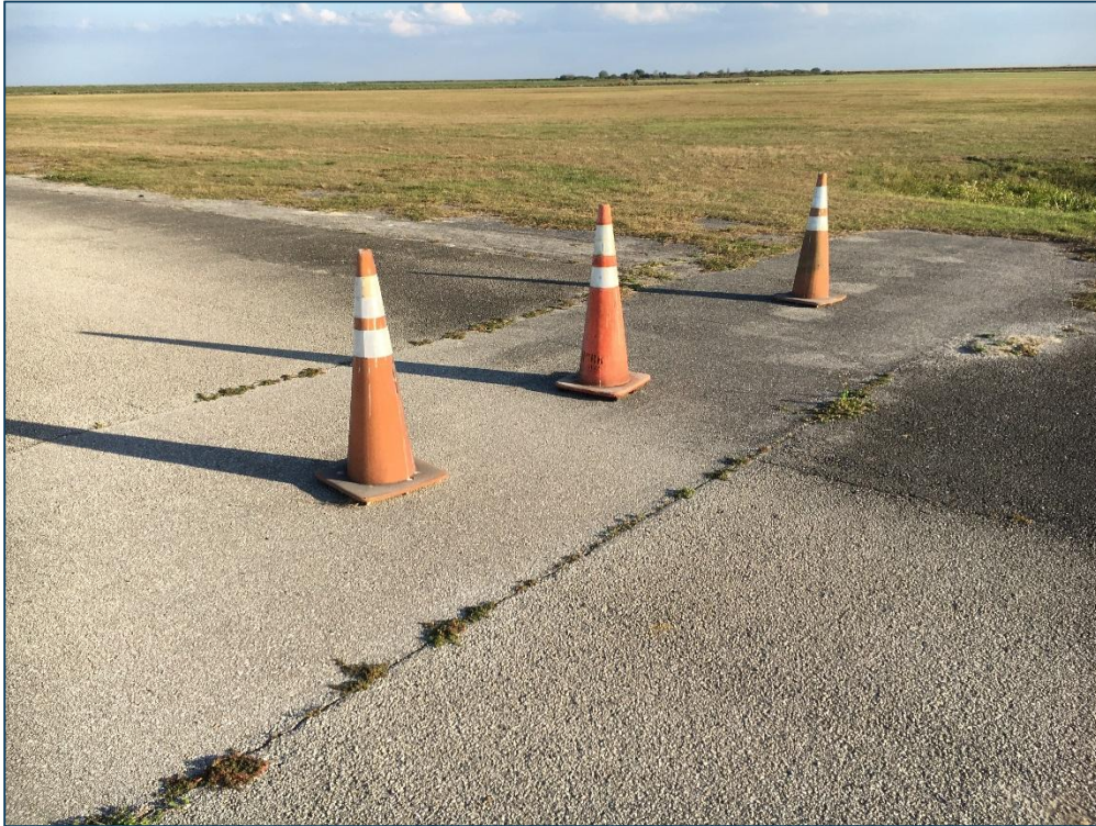
Taxiway A2, Section 215, Sample Unit 112 – Low Severity (48) Longitudinal and Transverse Cracking, Low Severity (50) Patching, Medium Severity (52) Raveling
