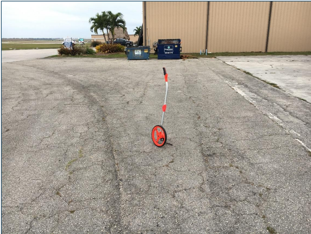
Taxiway to Hangar, Section 405, Sample Unit 104 – Low Severity (41) Alligator Cracking, Low Severity (43) Block Cracking, Low Severity (45) Depression, Low Severity (52) Raveling, Medium Severity (52) Raveling
