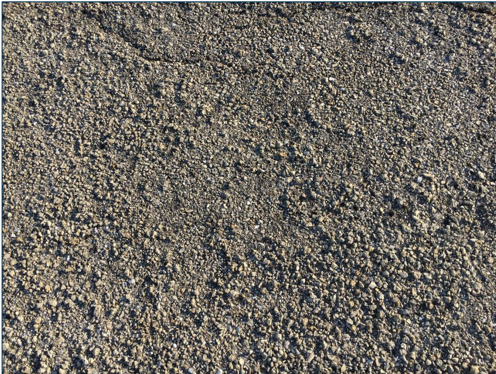
Taxiway A2, Section 210, Sample Unit 109 – Low Severity (48) Longitudinal and Transverse Cracking, Low Severity (52) Raveling, Medium Severity (52) Raveling
