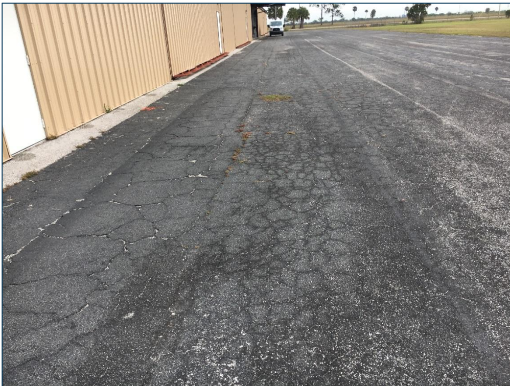
West Apron, Section 4105, Sample Unit 150 – Low Severity (41) Alligator Cracking, Low and Medium Severity (52) Raveling
