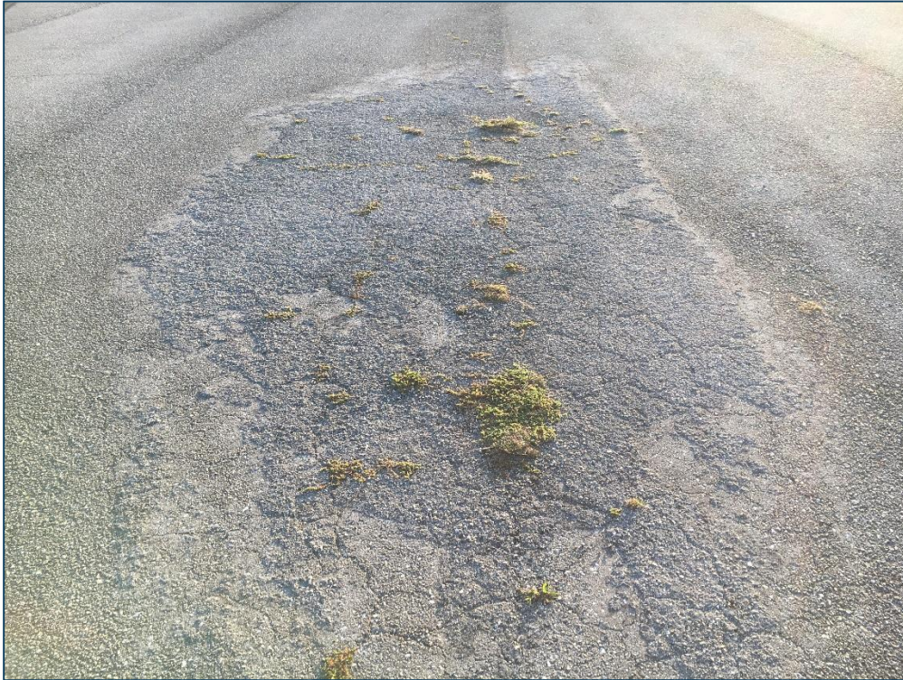
South Apron, Section 4305, Sample Unit 201 – High Severity (52) Raveling
