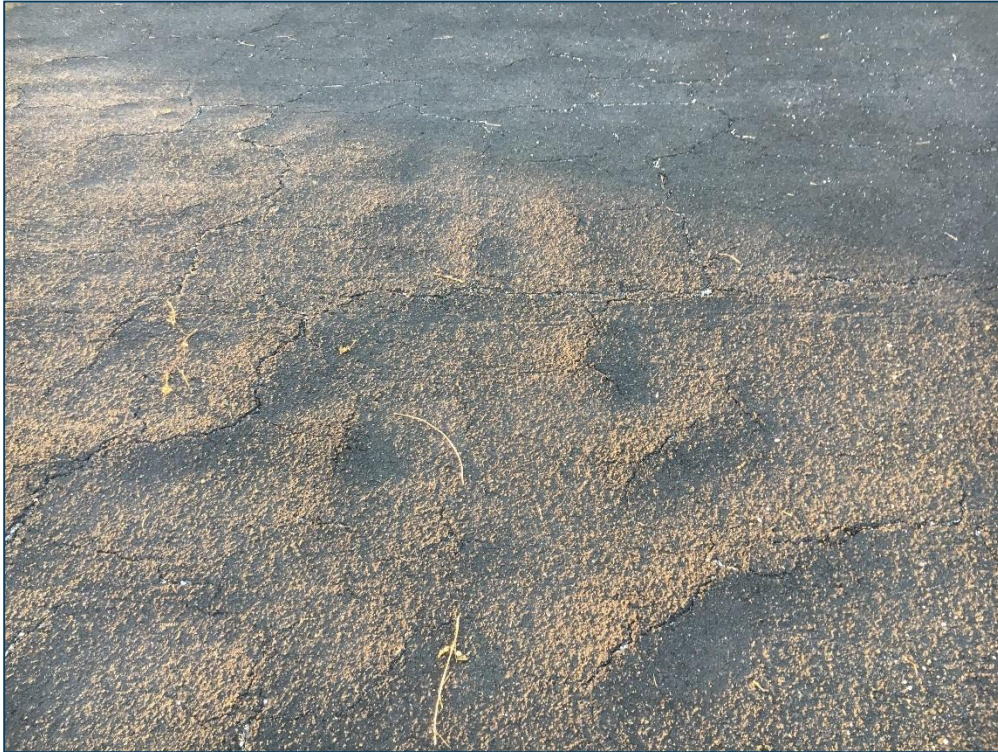
East Apron, Section 4505, Sample Unit 200 – Low Severity (43) Block Cracking, Low Severity (52) Raveling, Low Severity (56) Swelling
