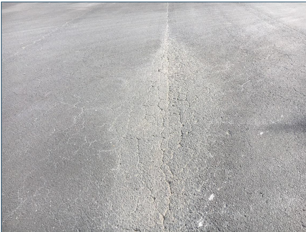
Apron NW, Section 4405, Sample Unit 304 – Medium Severity (41) Alligator Cracking, Low Severity (52) Raveling, Low Severity (53) Rutting
