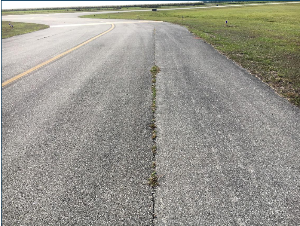
Taxiway A1, Section 104, Sample Unit 102 – Medium Severity (48) Longitudinal and Transverse Cracking, Low Severity (52) Raveling, Low Severity (57) Weathering
