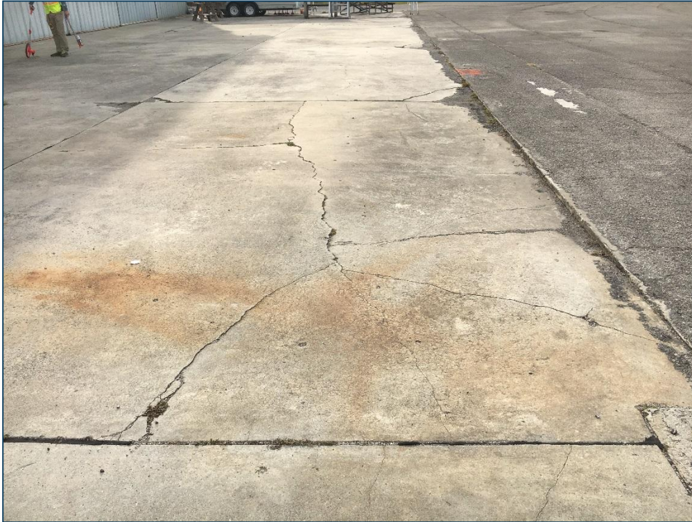
Apron Hangar, Section 4205, Sample Unit 100 – Medium Severity (72) Shattered Slab, High Severity (71) Faulting, Medium Severity (65) Joint Seal Damage
