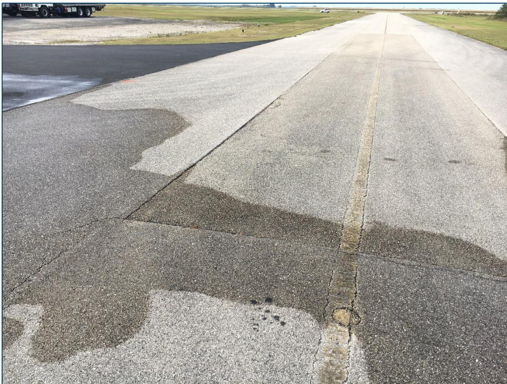
Taxiway S, Section 605, Sample Unit 109 – Low Severity (48) Longitudinal and Transverse Cracking, Low Severity (50) Patching, Low Severity (52) Raveling
