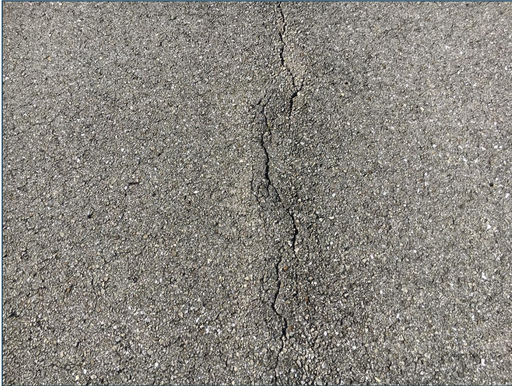
Taxiway A, Section 103, Sample Unit 112 – Low Severity (48) Longitudinal and Transverse Cracking, Low Severity (56) Swelling, Low Severity (57) Weathering
