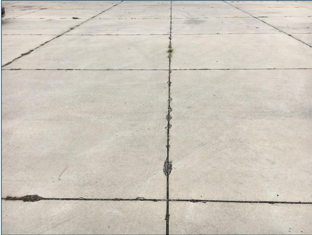
West Apron, Section 4110, Sample Unit 98 – Low Severity (74) Joint Spalling, High Severity (65) Joint Seal Damage
