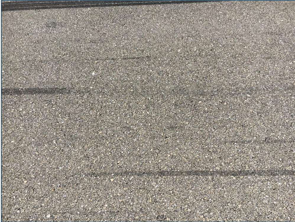
Runway 13-31, Section 6103, Sample Unit 80 – Low Severity (57) Weathering
