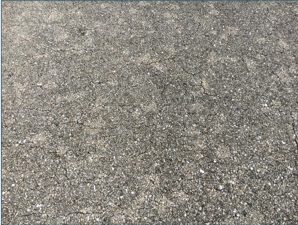
Taxiway S, Section 605, Sample Unit 101 – Low Severity (48) Longitudinal and Transverse Cracking, Low Severity (52) Raveling
