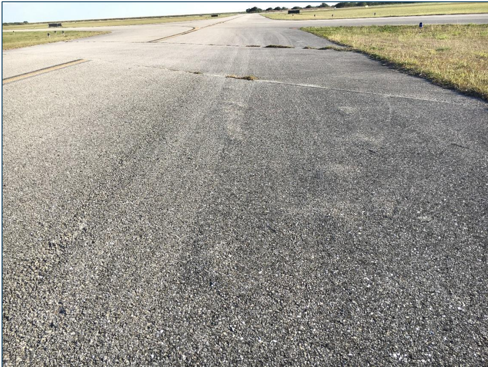
Taxiway A3, Section 410, Sample Unit 108 – Low Severity (50) Patching, Low Severity (52) Raveling, Medium Severity (52) Raveling, Low Severity (56) Swelling
