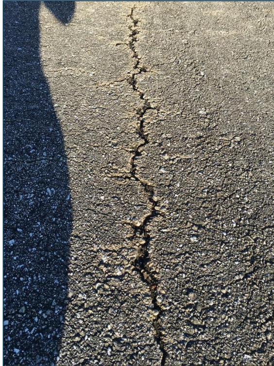
Runway 14-32, Section 6110, Sample Unit 105 – Medium Severity (48) Longitudinal and Transverse Cracking, Low Severity (52) Raveling, Low Severity (57) Weathering
