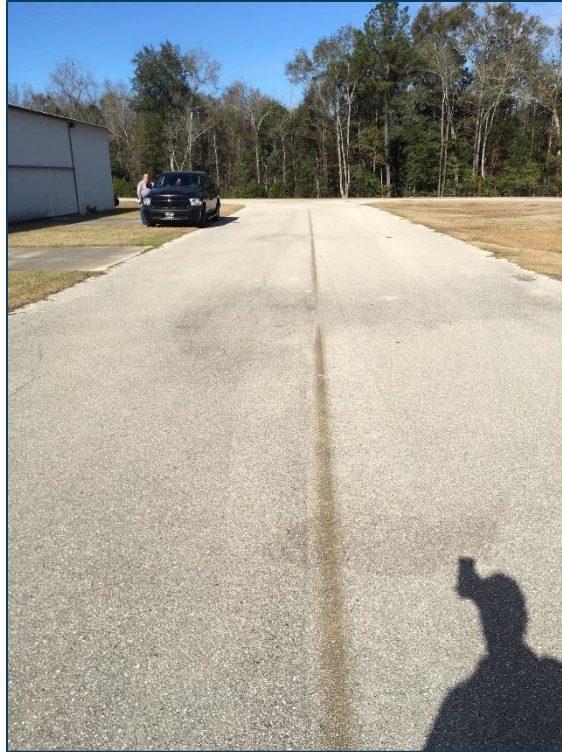
Taxiway Hangar, Section 125, Sample Unit 202 – Low Severity (45) Depression, Medium Severity (45) Depression, Low Severity (48) Longitudinal and Transverse Cracking, Low Severity (52) Raveling, Low Severity (57) Weathering
