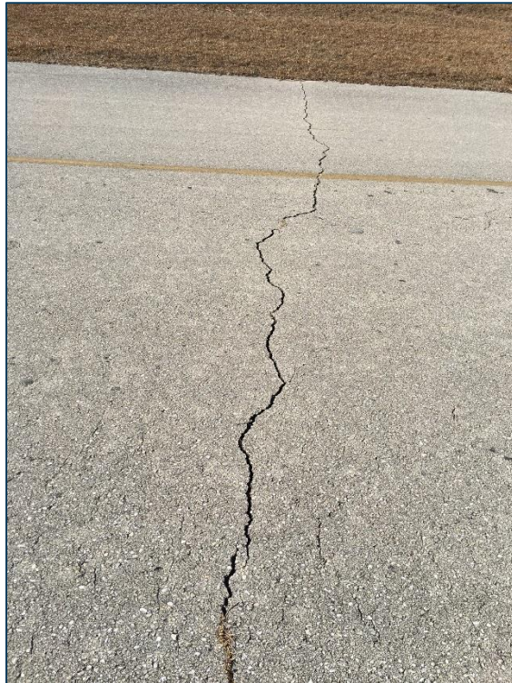
Taxiway Hangar, Section 115, Sample Unit 100 – Low and Medium Severity (48) Longitudinal and Transverse Cracking, Low Severity (52) Raveling, Low Severity (57) Weathering
