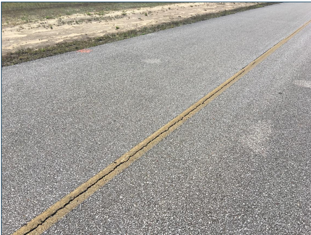
Taxiway B, Section 205, Sample Unit 103 – Low and Medium Severity (48) Longitudinal and Transverse Cracking, Low Severity (52) Raveling
