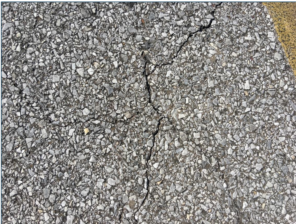
Taxiway A, Section 105, Sample Unit 101 – Low Severity (48) Longitudinal and Transverse Cracking, Low Severity (52) Raveling, Medium Severity (52) Raveling
