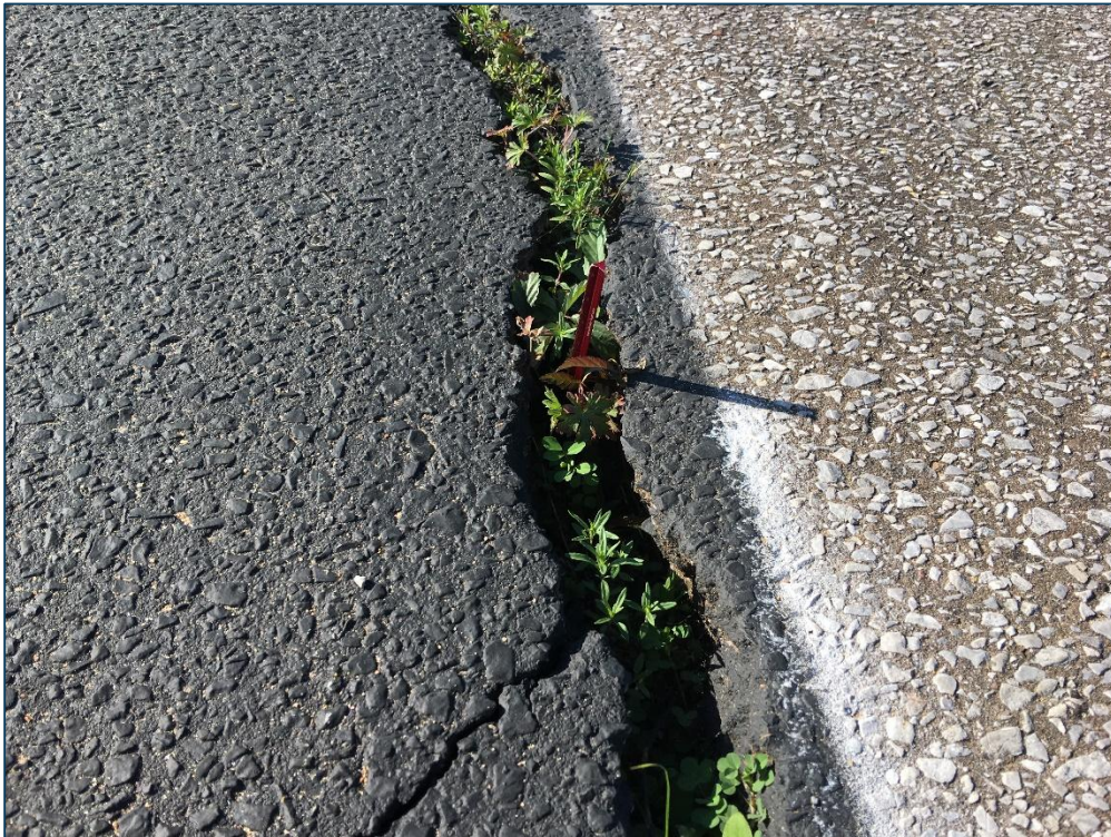
Taxiway B, Section 205, Sample Unit 120 – Low Severity (48) Longitudinal and Transverse Cracking, High Severity (48) Longitudinal and Transverse Cracking, Low Severity (52) Raveling
