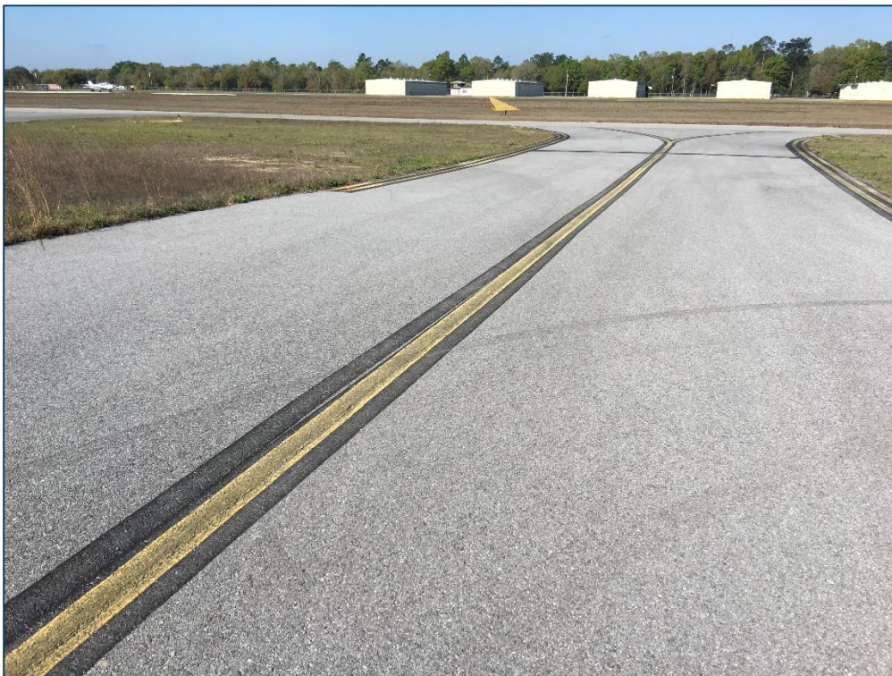
Taxiway To Hangar, Section 605, Sample Unit 301 – Low Severity (57) Weathering
