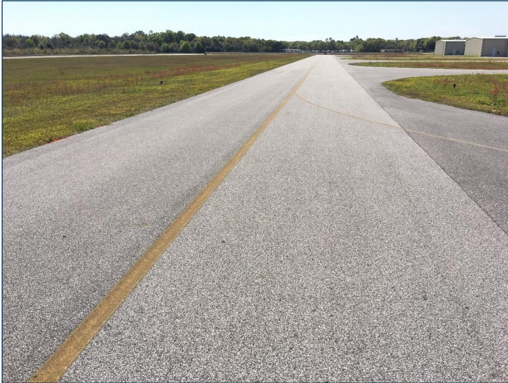
Taxiway A, Section 510, Sample Unit 103 – Low Severity (52) Raveling
