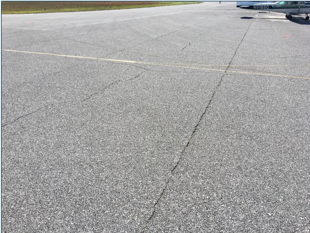
Apron West, Section 4110, Sample Unit 106 – Low and Medium Severity (48) Longitudinal and Transverse Cracking, Low Severity (52) Raveling, Medium Severity (52) Raveling
