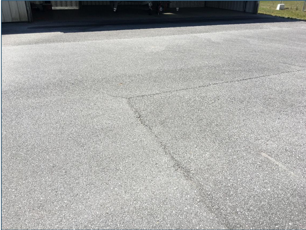
Apron West, Section 4130, Sample Unit 108 – Low Severity (48) Longitudinal and Transverse Cracking, Low Severity (50) Patching, Low Severity (52) Raveling, Low Severity (57) Weathering
