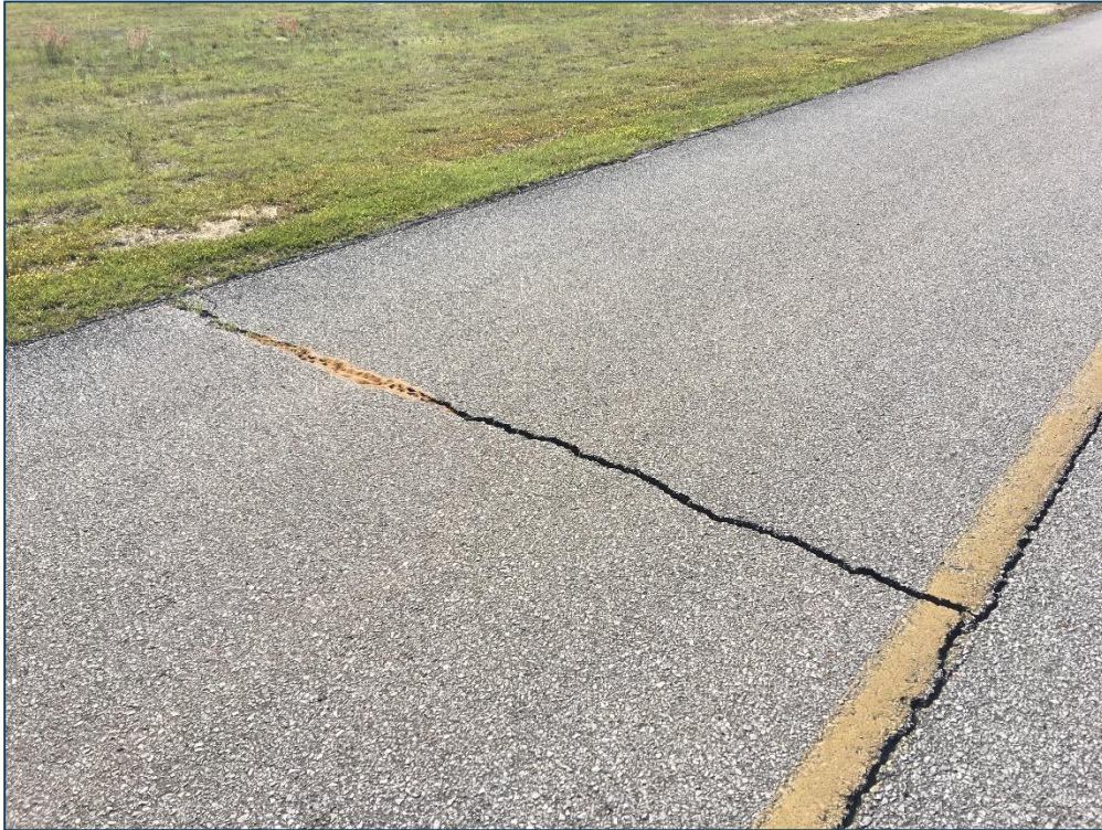
Taxiway B, Section 205, Sample Unit 111 – Low and Medium Severity (48) Longitudinal and Transverse Cracking, Low Severity (52) Raveling
