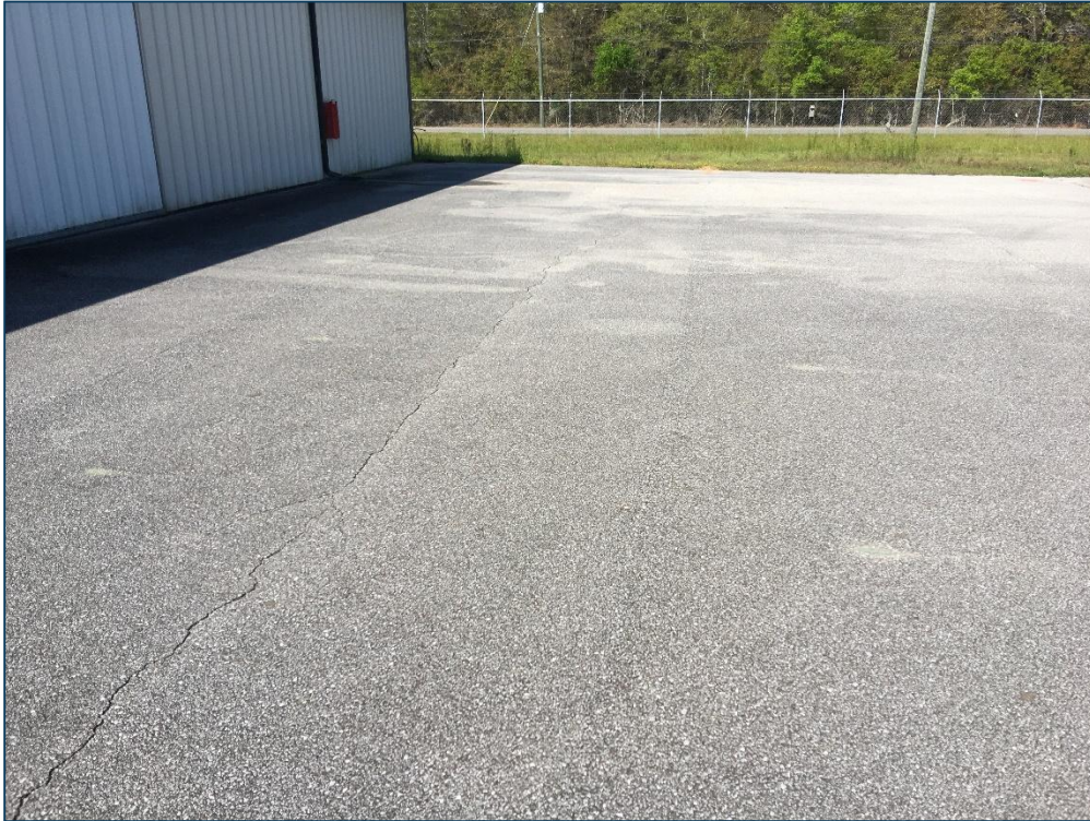
Apron West, Section 4125, Sample Unit 300 – Low Severity (48) Longitudinal and Transverse Cracking, Low Severity (52) Raveling
