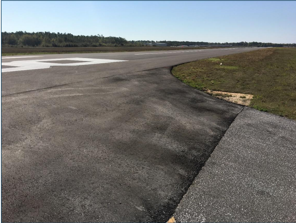
Taxiway A, Section 115, Sample Unit 110 – Low Severity (50) Patching, Low Severity (52) Raveling
