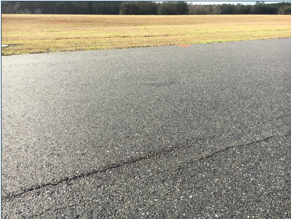
Runway 7-25, Section 6110, Sample Unit 146 – Low Severity (48) Longitudinal and Transverse Cracking, Low Severity (56) Swelling, Low Severity (57) Weathering
