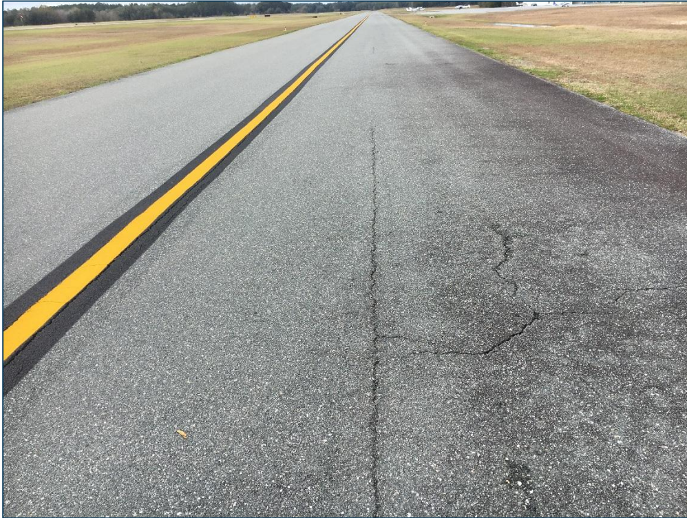
Taxiway A, Section 105, Sample Unit 104 – Low and Medium Severity (48) Longitudinal and Transverse Cracking, Low Severity (57) Weathering
