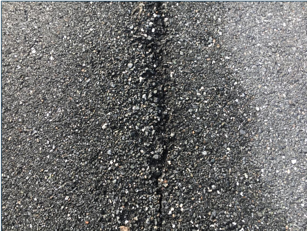
Taxiway C, Section 205, Sample Unit 101 – Low Severity (48) Longitudinal and Transverse Cracking, Low Severity (52) Raveling, Low Severity (57) Weathering
