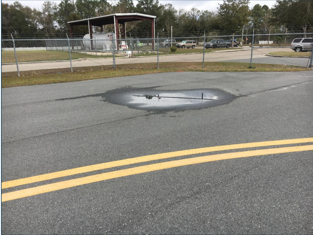
Apron, Section 4105, Sample Unit 454 – Low Severity (45) Depression, Low Severity (57) Weathering
