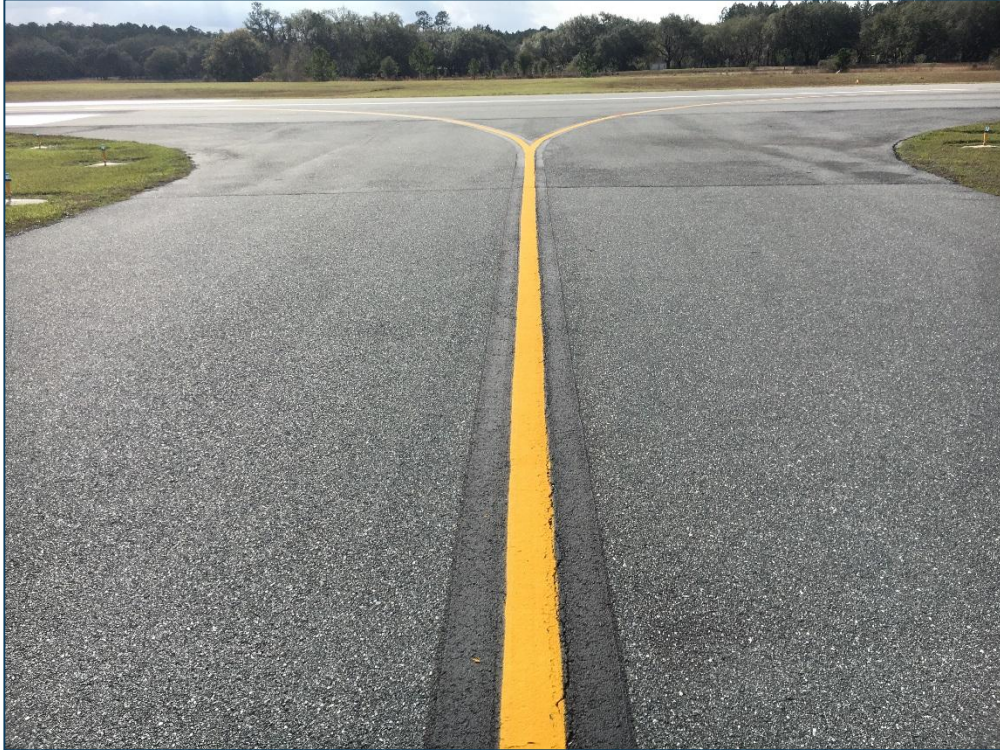
Taxiway A3, Section 135, Sample Unit 100 – Low Severity (48) Longitudinal and Transverse Cracking, Low Severity (57) Weathering
