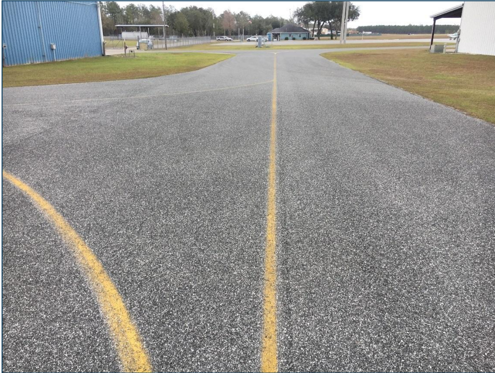
Taxilane to T-Hangar, Section 4115, Sample Unit 100 – Low Severity (52) Raveling
