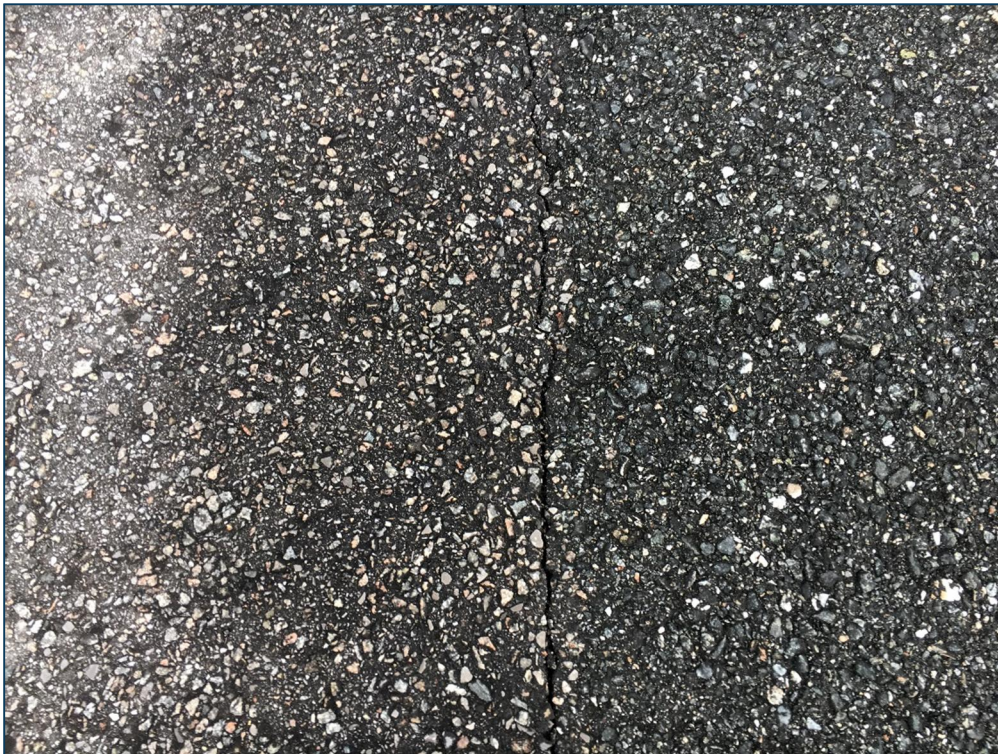
Apron Run-Up, Section 4205, Sample Unit 302 – Low Severity (48) Longitudinal and Transverse Cracking, Low Severity (52) Raveling, Medium Severity (52) Raveling
