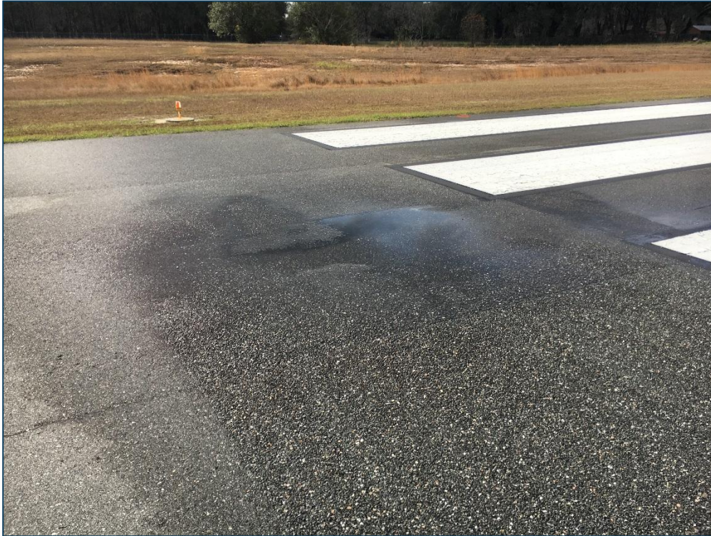
Runway 7-25, Section 6105, Sample Unit 103 – Low Severity (45) Depression, Low Severity (48) Longitudinal and Transverse Cracking, Low Severity (57) Weathering
