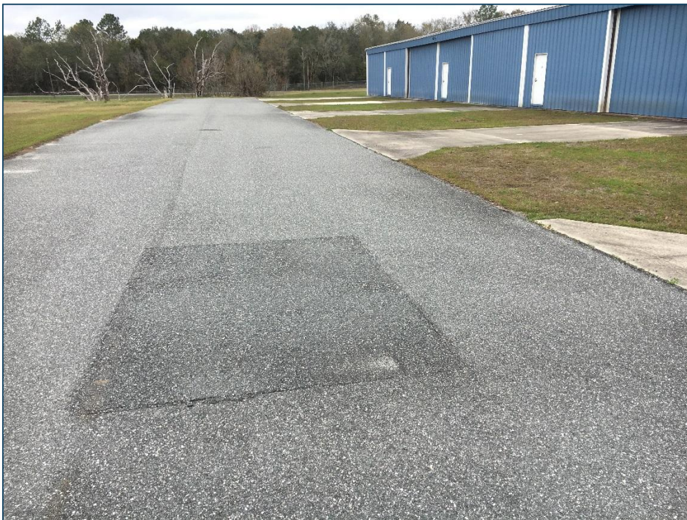
Taxilane to T-Hangar, Section 4125, Sample Unit 401 – Low Severity (50) Patching, Low Severity (52) Raveling, Low Severity (57) Weathering
