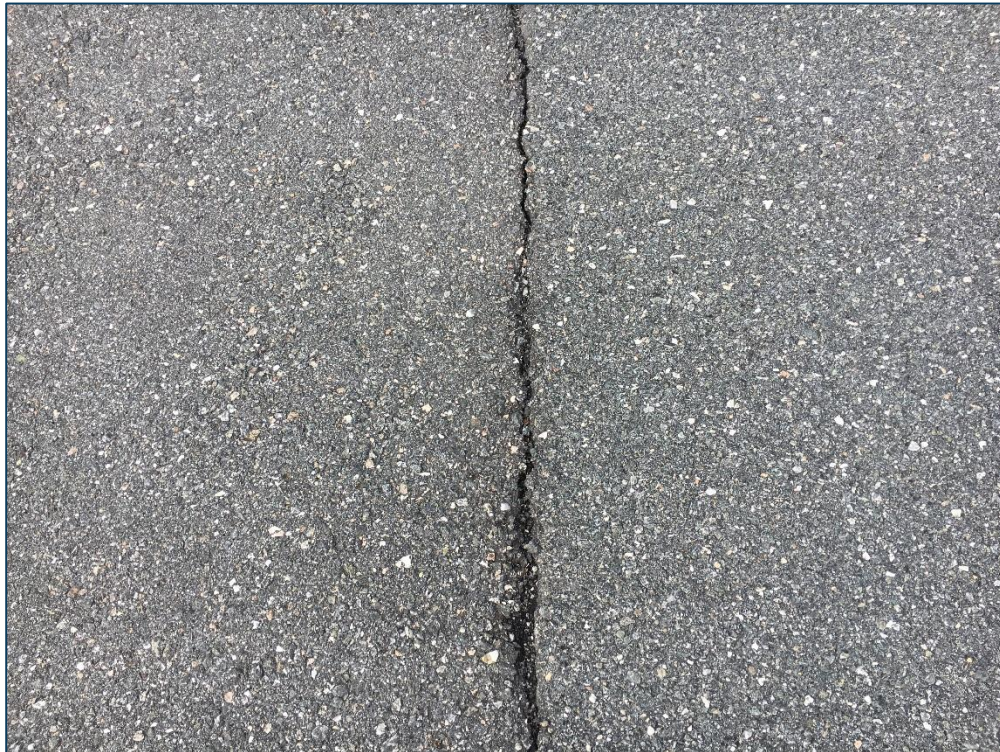
Taxiway A2, Section 125, Sample Unit 100 – Low Severity (48) Longitudinal and Transverse Cracking, Low Severity (52) Raveling, Low Severity (57) Weathering
