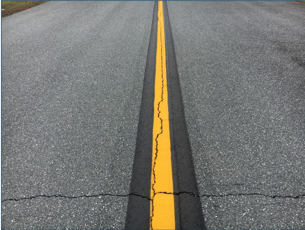
Taxiway A1, Section 115, Sample Unit 101 – Low and Medium Severity (48) Longitudinal and Transverse Cracking, Low Severity (57) Weathering
