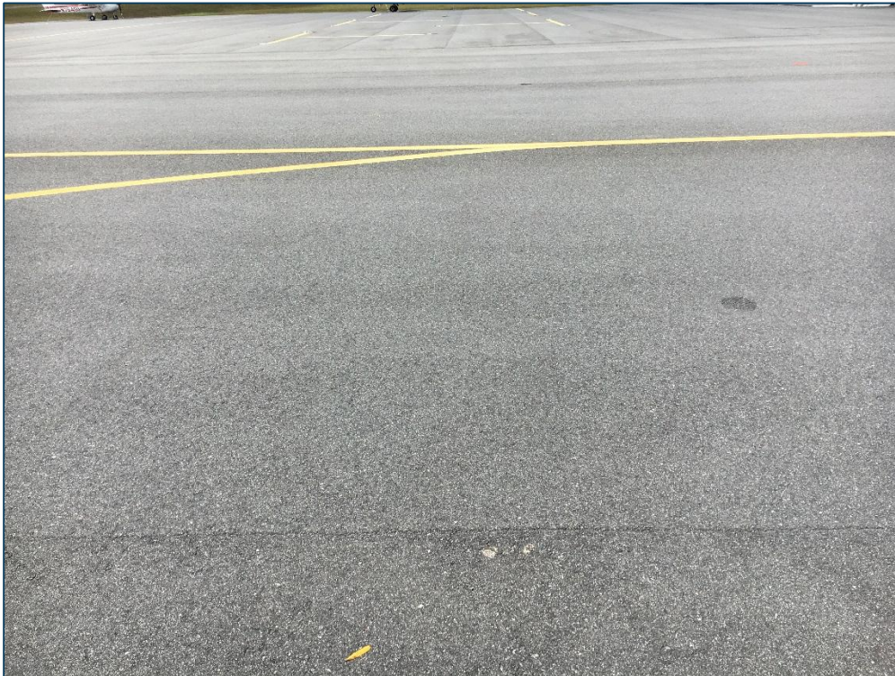
Apron, Section 4105, Sample Unit 202 – Low Severity (48) Longitudinal and Transverse Cracking, Low Severity (57) Weathering
