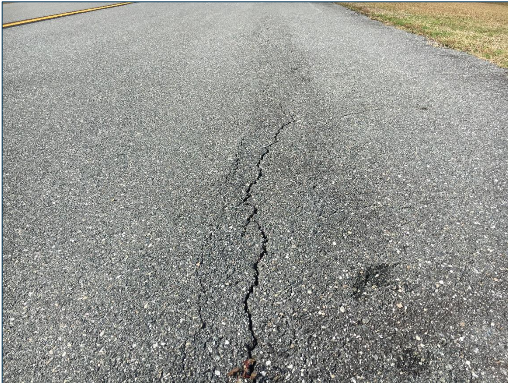
Taxiway A, Section 105, Sample Unit 112 – Low and Medium Severity (48) Longitudinal and Transverse Cracking, Low Severity (56) Swelling, Low Severity (57) Weathering
