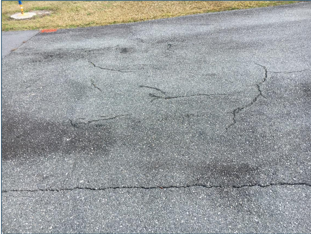
Taxiway to AP, Section 305, Sample Unit 100 – Low and Medium Severity (48) Longitudinal and Transverse Cracking, Low Severity (52) Raveling, Medium Severity (52) Raveling
