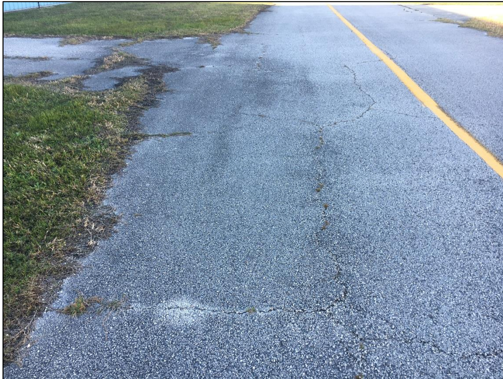
North T-Hangar Taxilane, Section 4205, Sample Unit 403 – Low Severity (43) Block Cracking, Low Severity (52) Raveling, Medium Severity (52) Raveling
