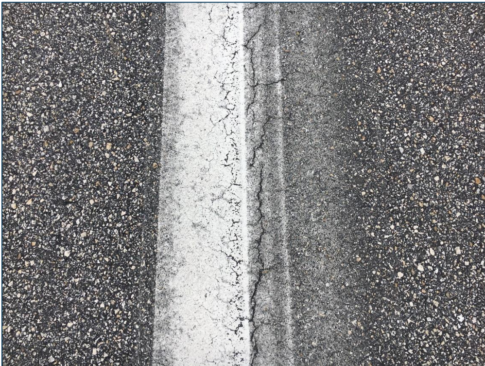
Runway 17-35, Section 6205, Sample Unit 154 – Low Severity (48) Longitudinal and Transverse Cracking, Low Severity (57) Weathering
