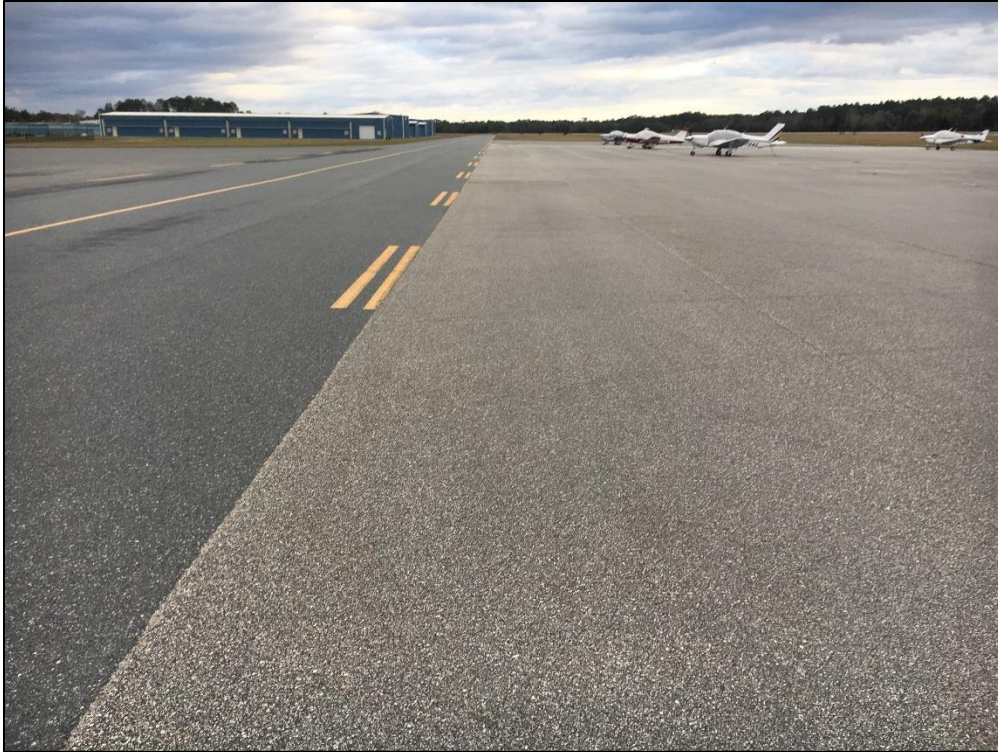
Apron, Section 4115, Sample Unit 403 – Low Severity (48) Longitudinal and Transverse Cracking, Low Severity (57) Weathering
