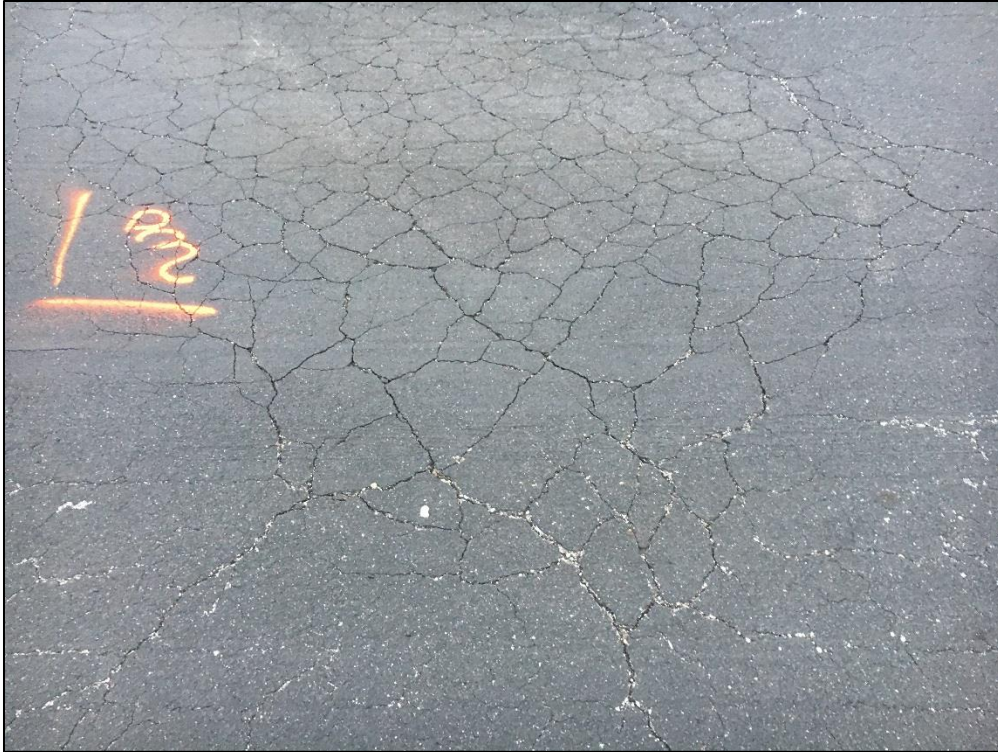
Apron, Section 4215, Sample Unit 200 – Medium Severity (41) Alligator Cracking, Low Severity (45) Depression, Low Severity (52) Raveling
