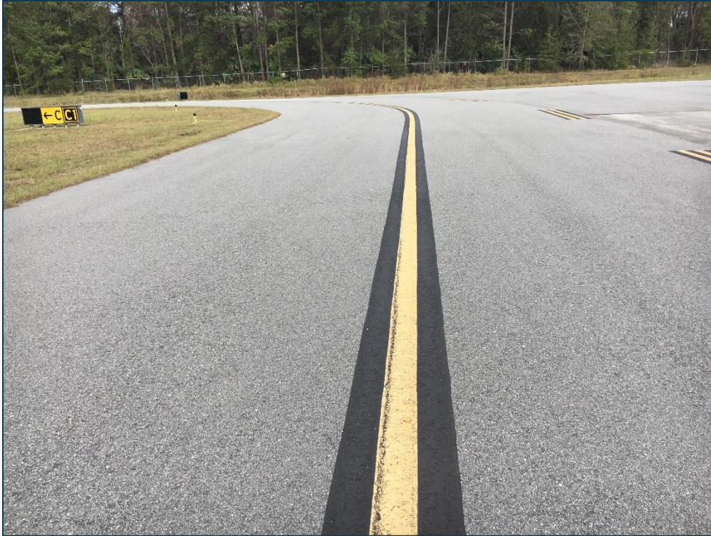
Taxiway C1, Section 330, Sample Unit 102 – Low Severity (48) Longitudinal and Transverse Cracking, Low Severity (57) Weathering
