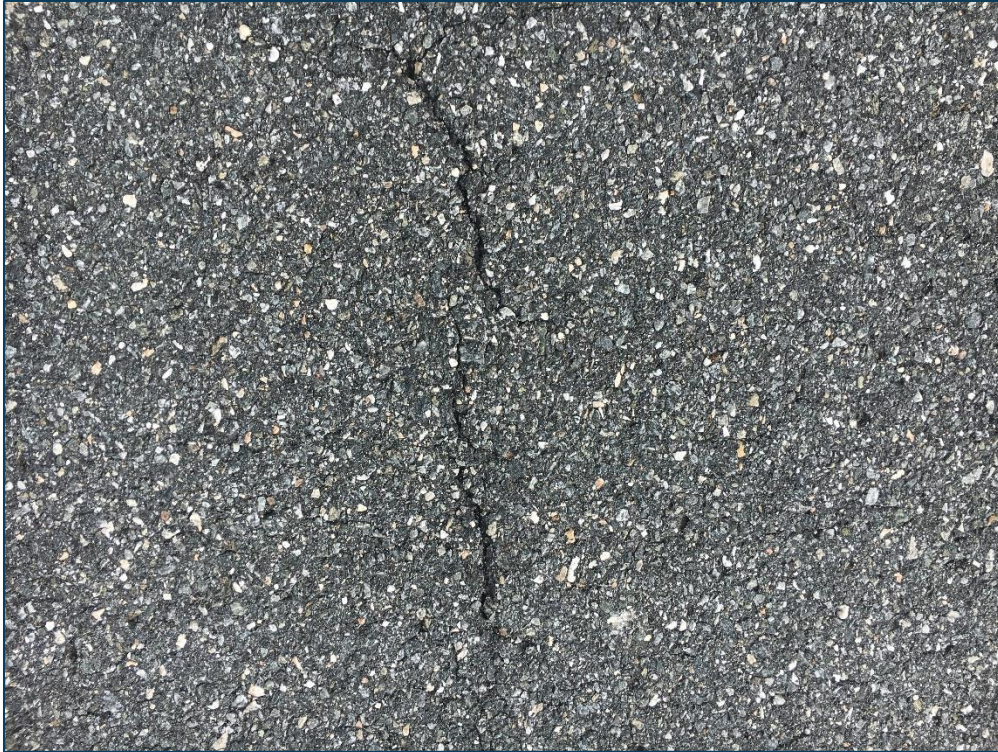
Taxiway A1, Section 117, Sample Unit 102 – Low Severity (48) Longitudinal and Transverse Cracking, Low Severity (52) Raveling, Low Severity (57) Weathering
