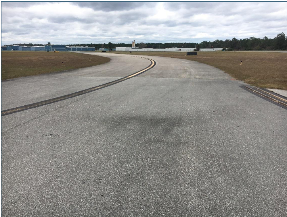
Taxiway B, Section 220, Sample Unit 100 – Low Severity (45) Depression, Low Severity (57) Weathering
