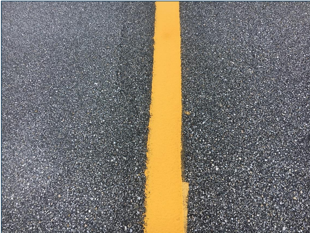
Taxiway C2, Section 320, Sample Unit 103 – Low Severity (57) Weathering
