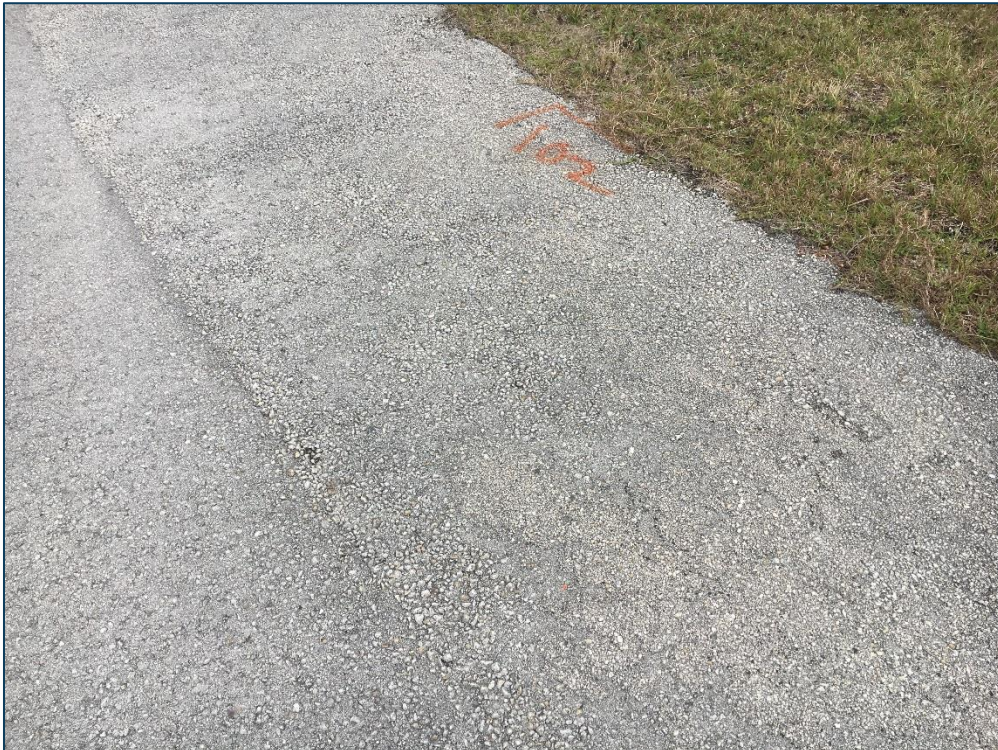
Taxiway A, Section 100, Sample Unit 102 – Low Severity (52) Raveling, Medium Severity (52) Raveling
