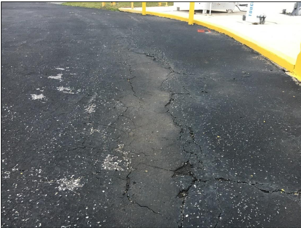
Apron, Section 4215, Sample Unit 100 – Low Severity (41) Alligator Cracking, Low Severity (52) Raveling
