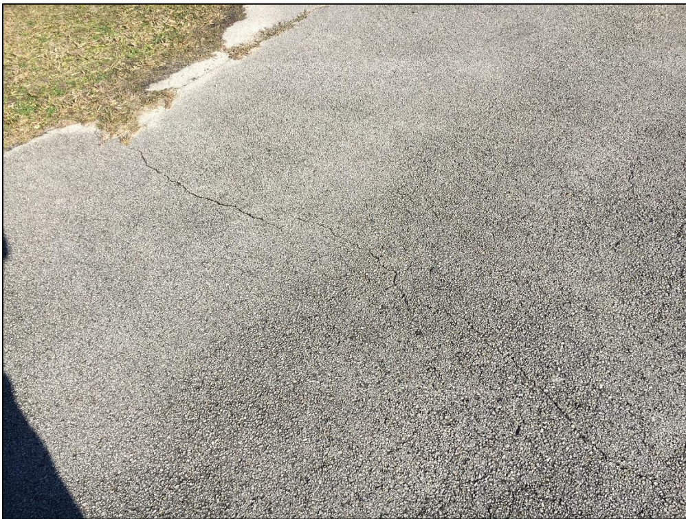
East T-Hangar Taxiways, Section 4305, Sample Unit 100 – Low Severity (48) Longitudinal and Transverse Cracking, Low Severity (57) Weathering
