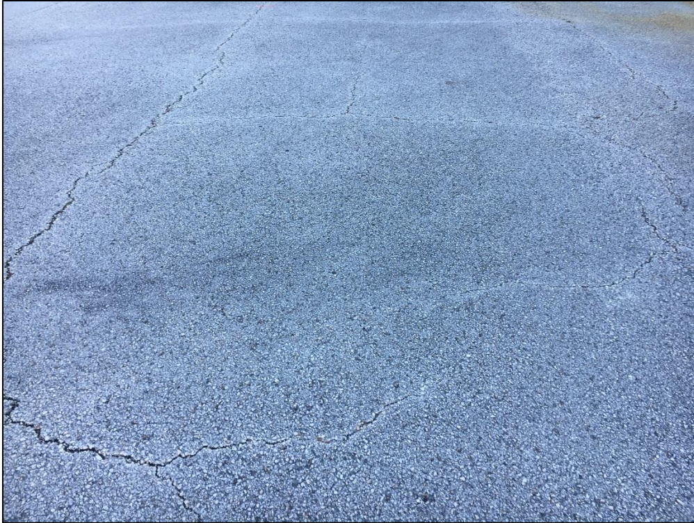
North T-Hangar Taxilane, Section 4210, Sample Unit 204 – Low Severity (43) Block Cracking, Low Severity (52) Raveling
