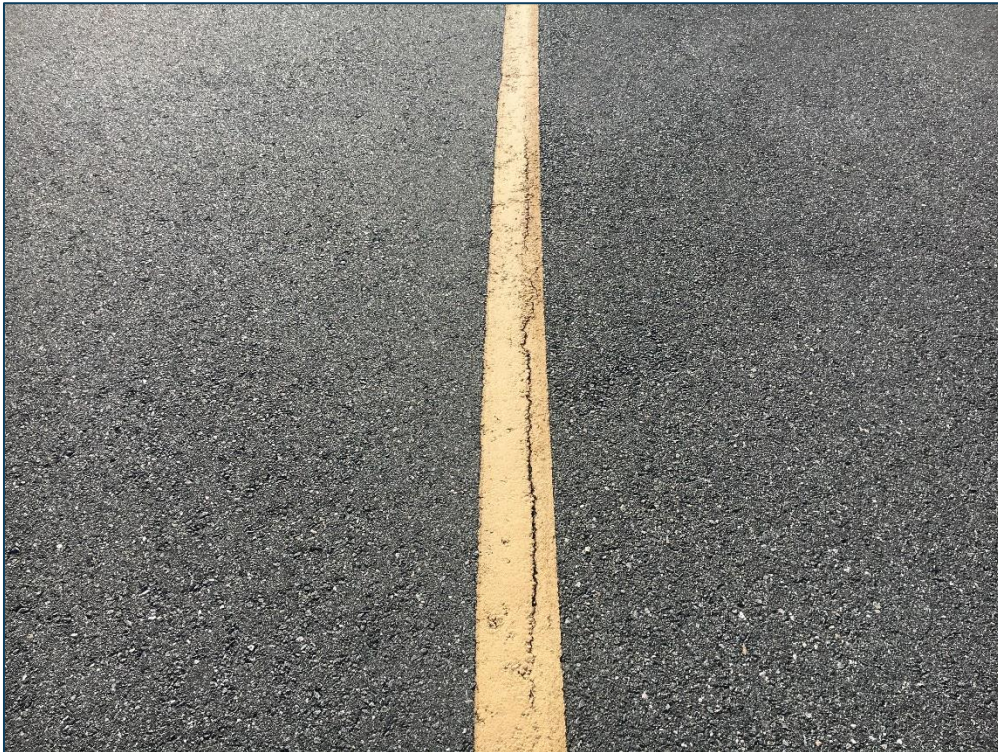
Taxiway B, Section 205, Sample Unit 124 – (42) Bleeding, Low Severity (48) Longitudinal and Transverse Cracking, Medium Severity (52) Raveling, Low Severity (57) Weathering
