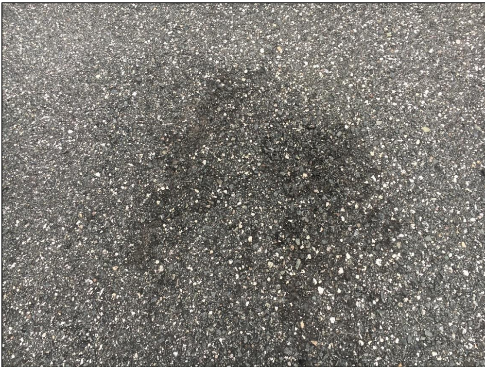
Apron, Section 4105, Sample Unit 201 – (49) Oil Spillage, Low Severity (57) Weathering
