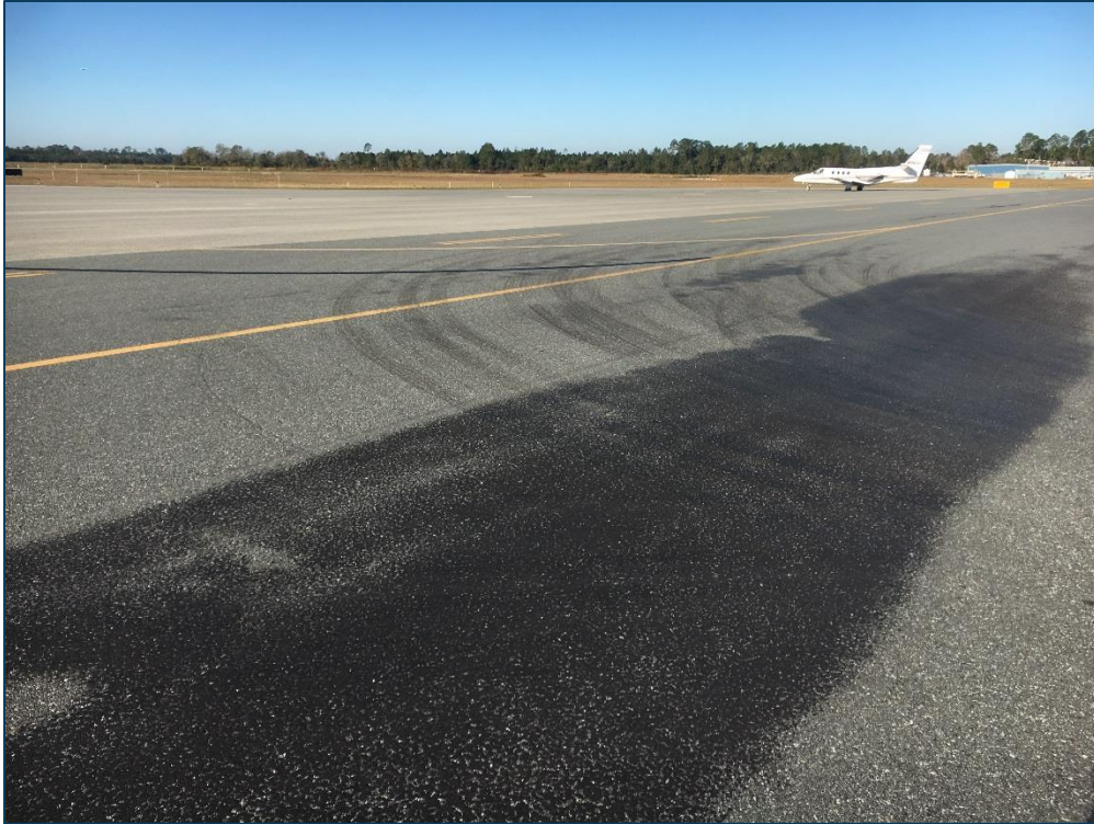
Taxiway B, Section 215, Sample Unit 108 – (42) Bleeding, Low Severity (52) Raveling, Low Severity (57) Weathering
