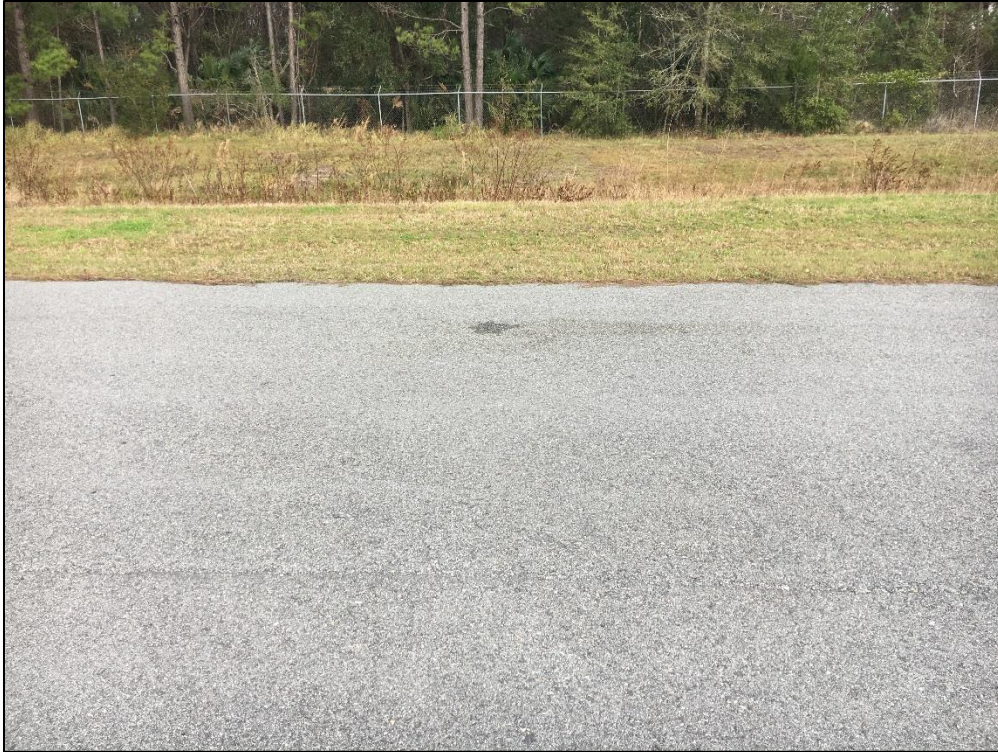
Run-Up Apron RW 35, Section 5210, Sample Unit 101 – Low Severity (57) Weathering, Low Severity (48) Longitudinal and Transverse Cracking
