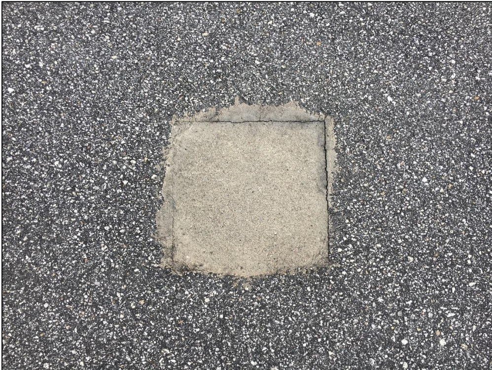
Run-Up Apron RW 35, Section 5205, Sample Unit 100 – Low Severity (50) Patching, Low Severity (57) Weathering
