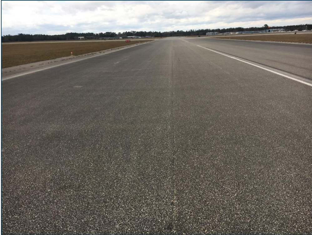
Runway 17-35, Section 6205, Sample Unit 130 – Low Severity (48) Longitudinal and Transverse Cracking, Low Severity (57) Weathering
