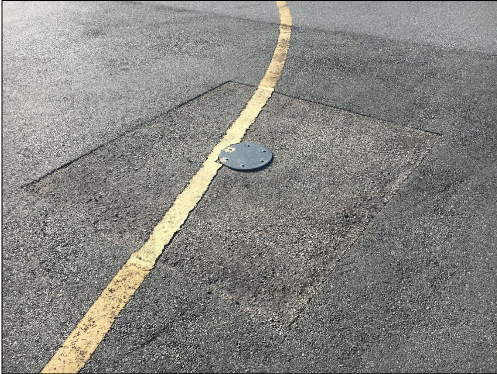
Apron E T-Hangar, Section 4310, Sample Unit 501 – Low Severity (50) Patching, Low Severity (57) Weathering
