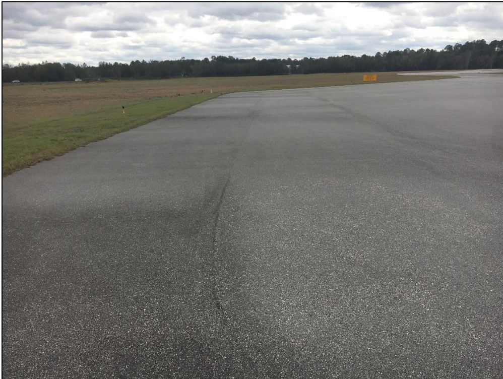
Run-Up Apron RW 27, Section 5105, Sample Unit 100 – Low Severity (57) Weathering
