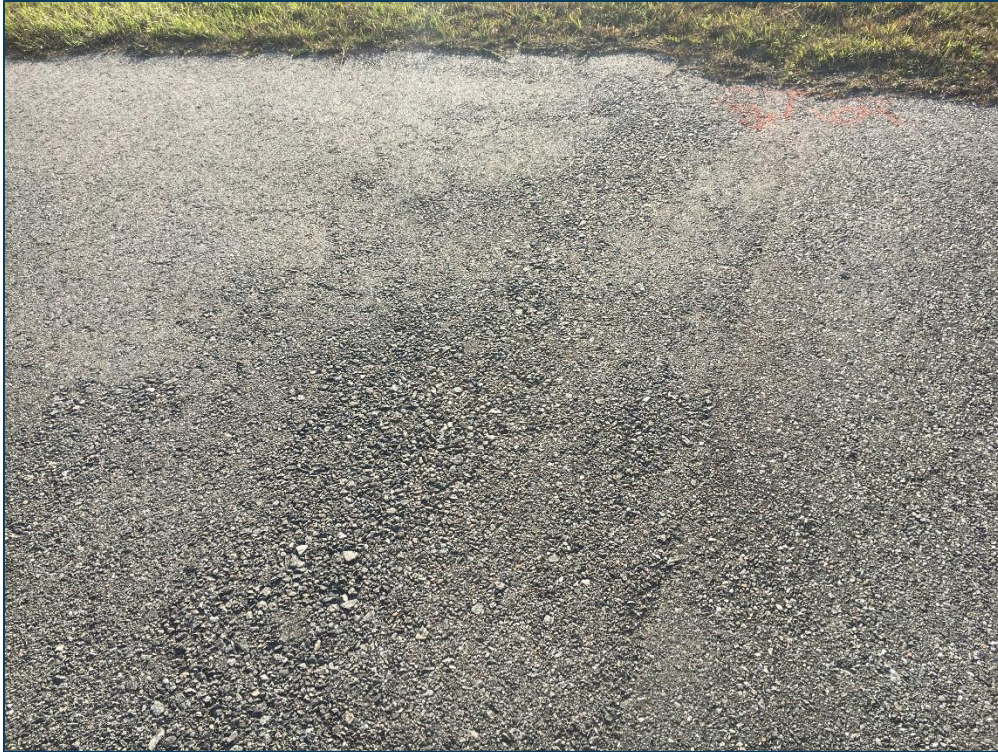
Taxiway C, Section 305, Sample Unit 103 – Low Severity (52) Raveling, Low Severity (57) Weathering
