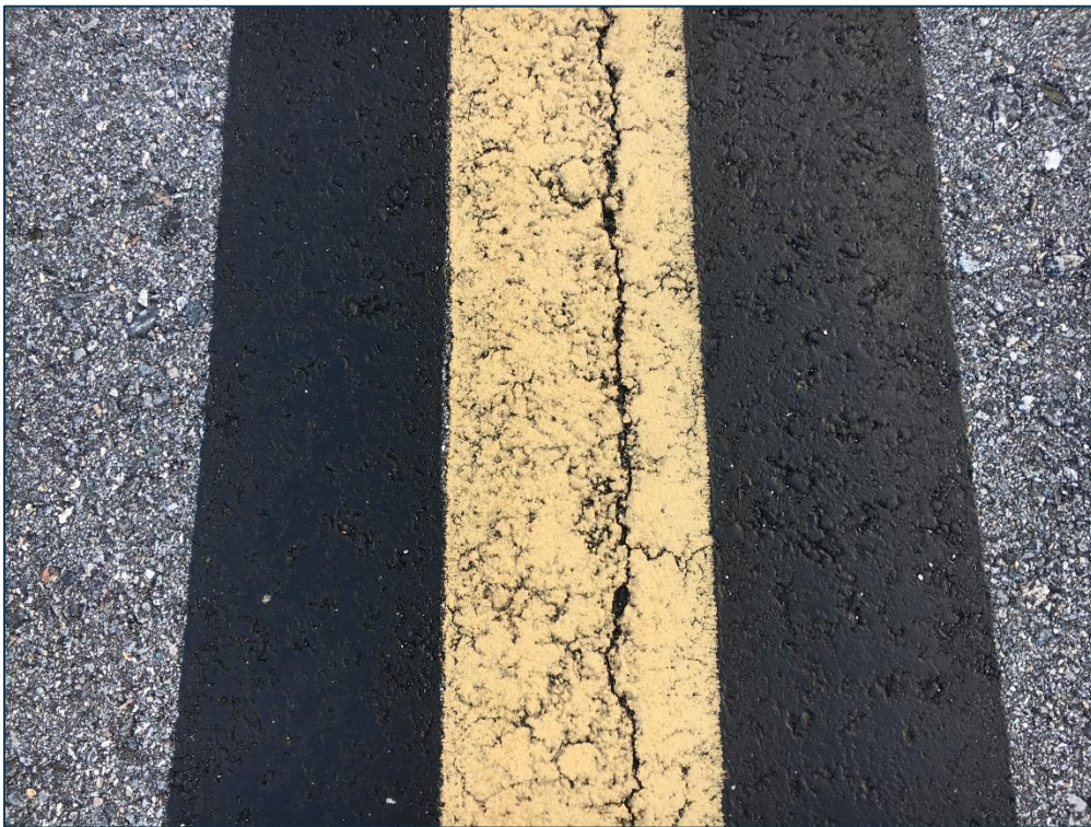
Taxiway C, Section 310, Sample Unit 120 – Low Severity (48) Longitudinal and Transverse Cracking, Low Severity (57) Weathering
