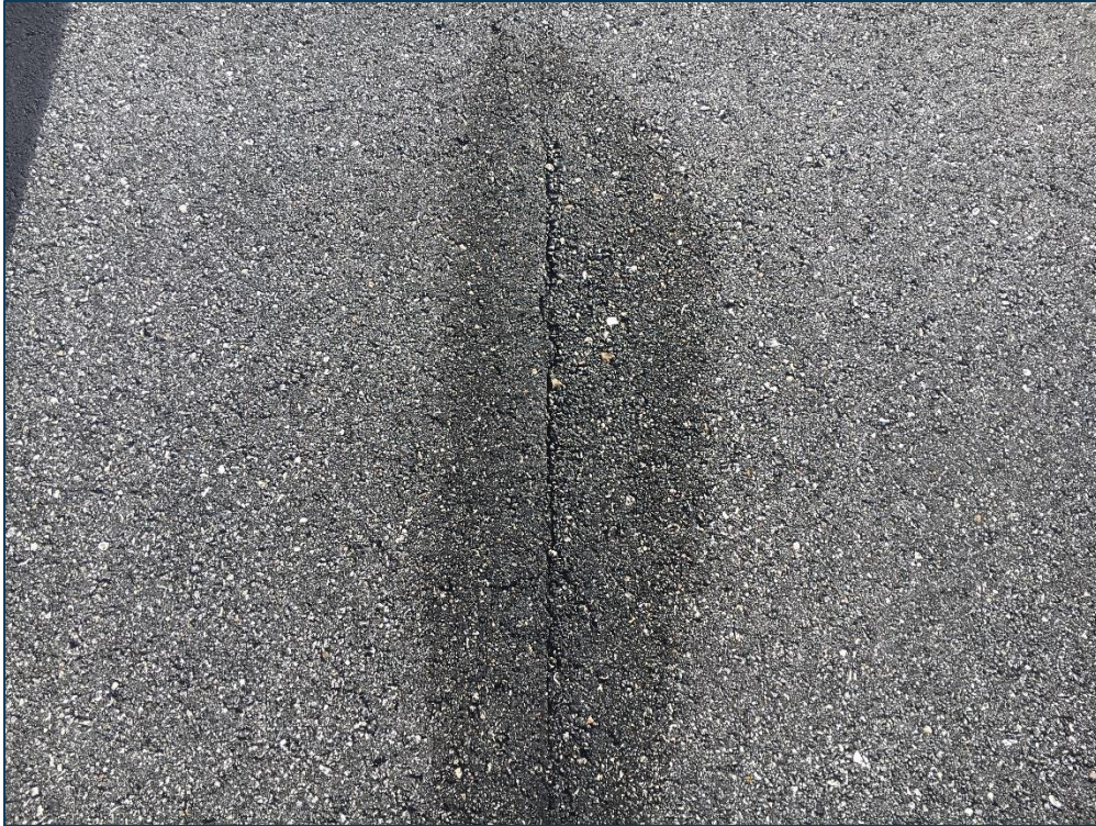
Runway 9-27, Section 6110, Sample Unit 190 – Low Severity (48) Longitudinal and Transverse Cracking, Low Severity (57) Weathering
