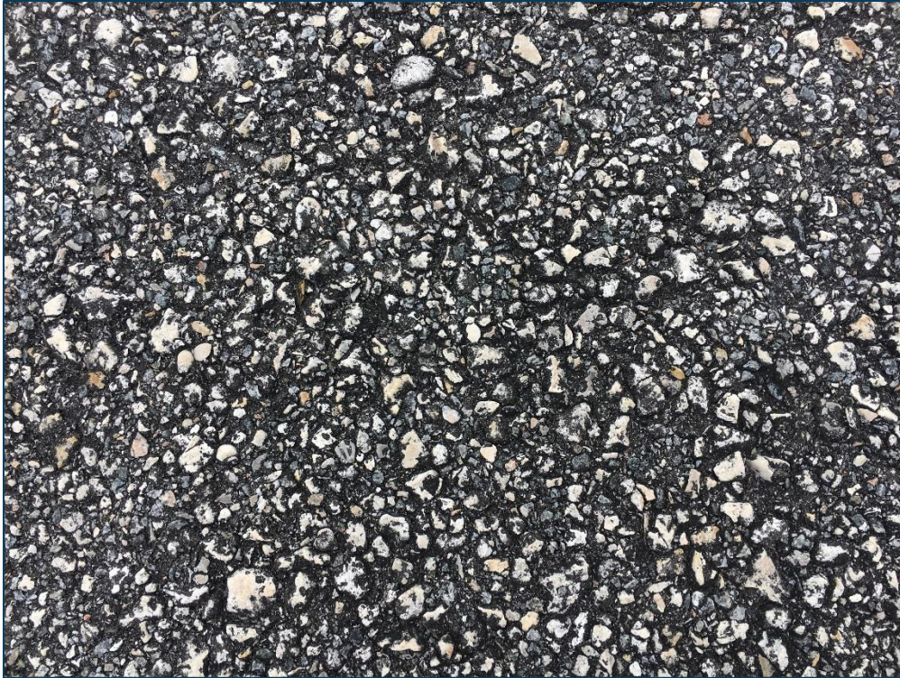
Taxiway C3, Section 410, Sample Unit 103 – Low Severity (52) Raveling
