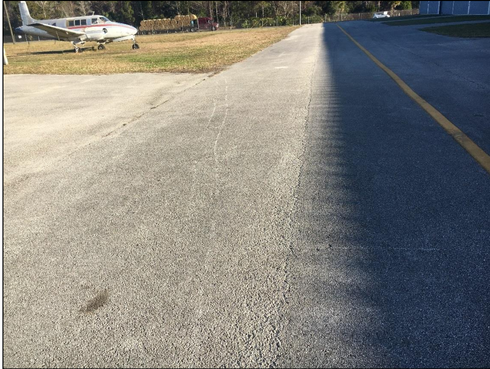
North T-Hangar Taxilane, Section 4220, Sample Unit 503 – Low and Medium Severity (48) Longitudinal and Transverse Cracking, Low Severity (52) Raveling, Medium Severity (52) Raveling
