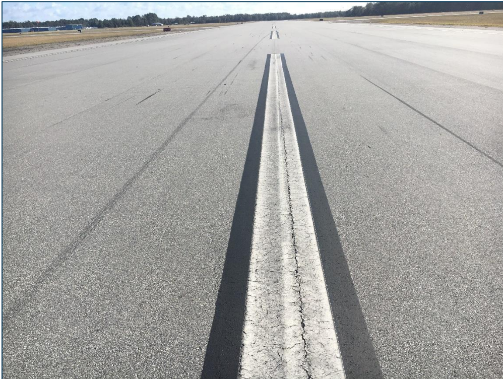
Runway 9-27, Section 6105, Sample Unit 134 – Low Severity (48) Longitudinal and Transverse Cracking, Low Severity (57) Weathering
