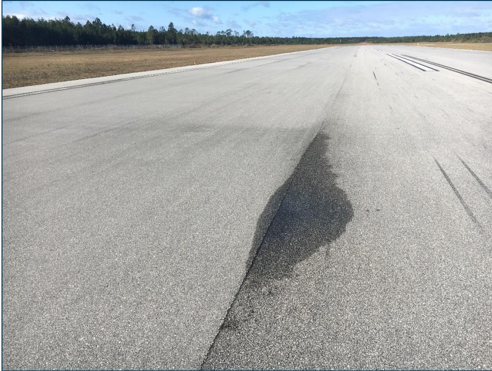
Runway 9-27, Section 6115, Sample Unit 98 – Low Severity (48) Longitudinal and Transverse Cracking, Low Severity (57) Weathering
