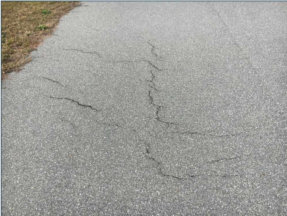
Taxiway A, Section 105, Sample Unit 103 – (55) Slippage Cracking, Low Severity (57) Weathering
