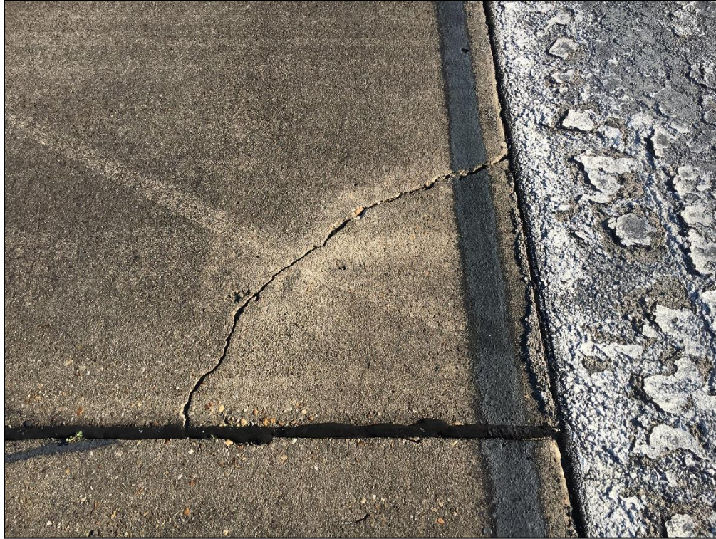
Runway 12-30, Section 6125, Sample Unit 396 – Low Severity (62) Corner Break, High Severity (65) Joint Seal Damage
