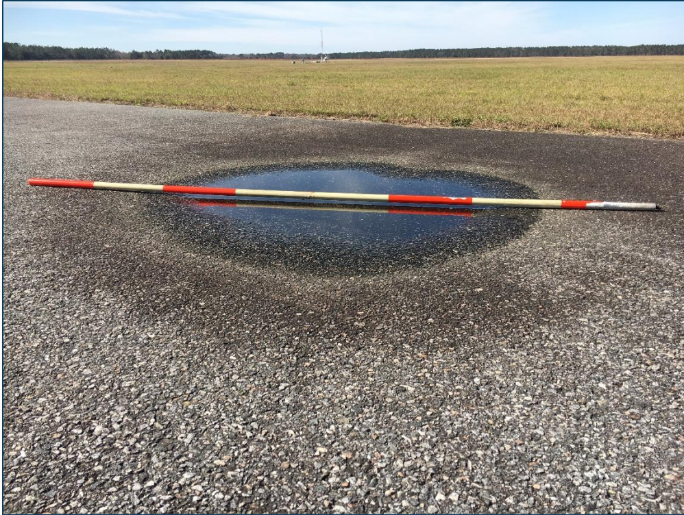
Taxiway A & B, Section 105, Sample Unit 112 – Low Severity (45) Depression, Low Severity (52) Raveling, Medium Severity (52) Raveling
