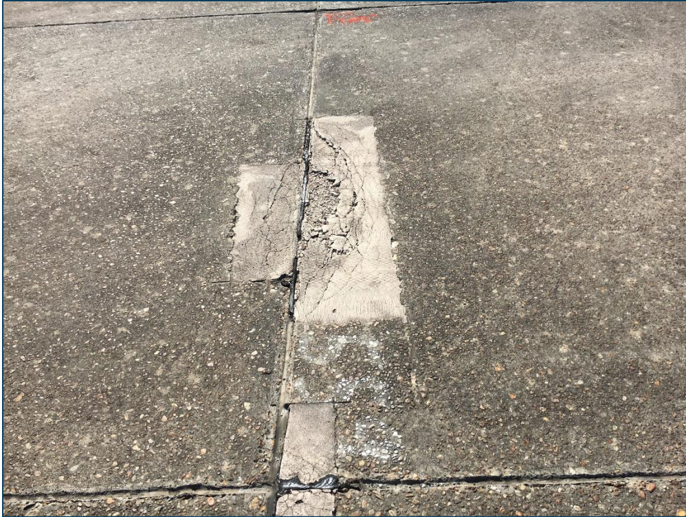
Apron, Section 4105, Sample Unit 205 – High Severity (66) Small Patching, Medium Severity (66) Small Patching
