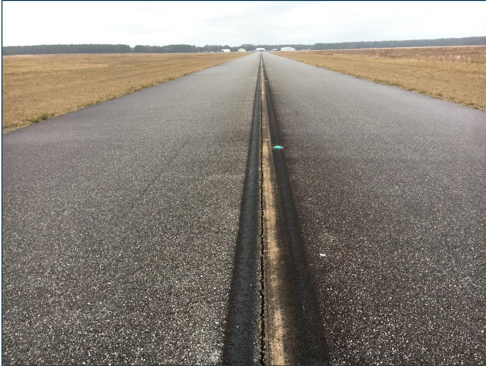
Taxiway C, Section 205, Sample Unit 111 – Medium Severity (48) Longitudinal and Transverse Cracking, Low Severity (52) Raveling
