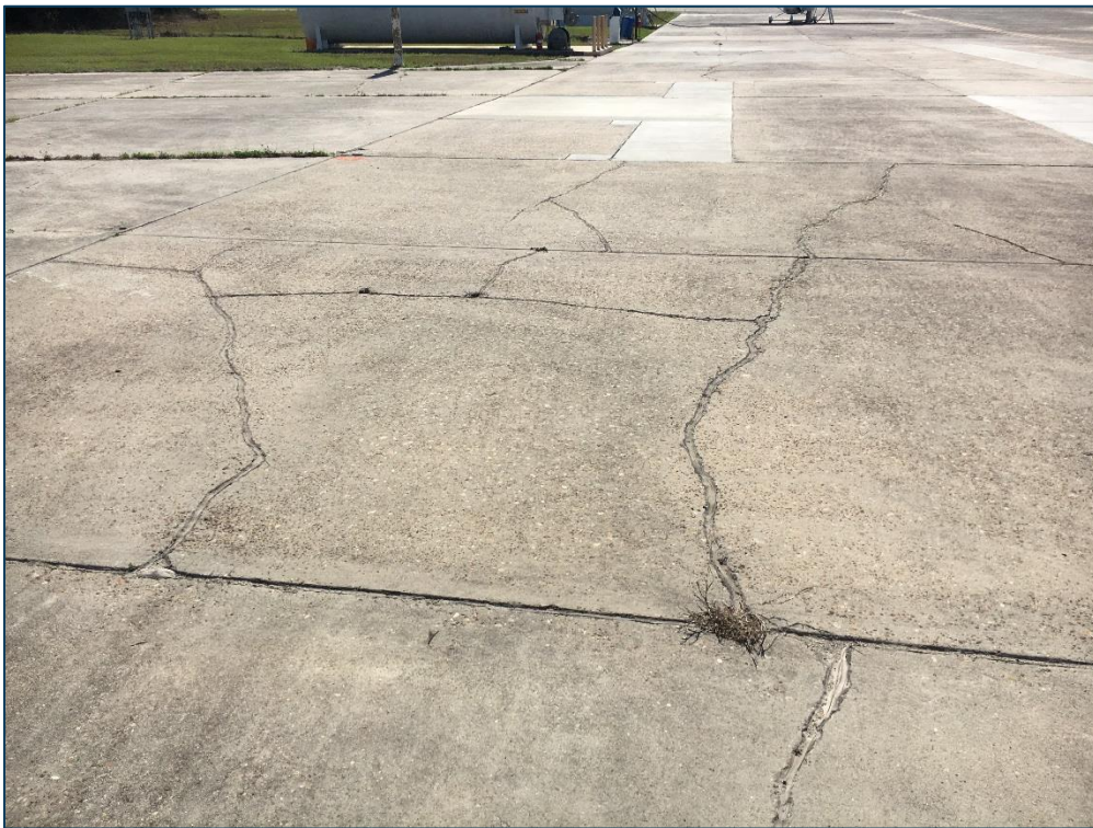
Apron, Section 4105, Sample Unit 611 – Medium Severity (72) Shattered Slab
