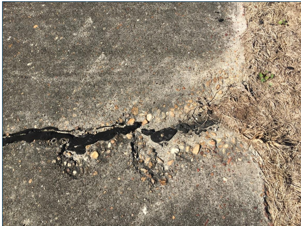
Apron, Section 4105, Sample Unit 503 – Medium Severity (63) Longitudinal, Transverse, and Diagonal Cracking, High Severity (65) Joint Seal Damage
