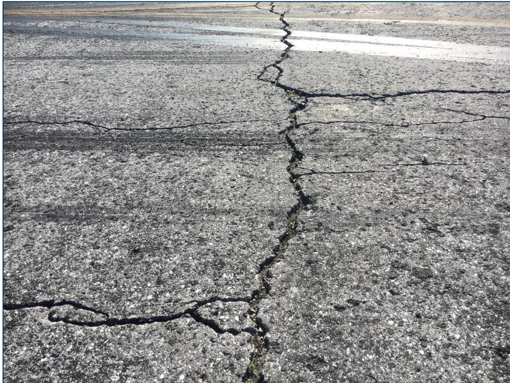
Taxiway C, Section 215, Sample Unit 141 – Medium Severity (43) Block Cracking, Low Severity (52) Raveling, Medium Severity (52) Raveling
