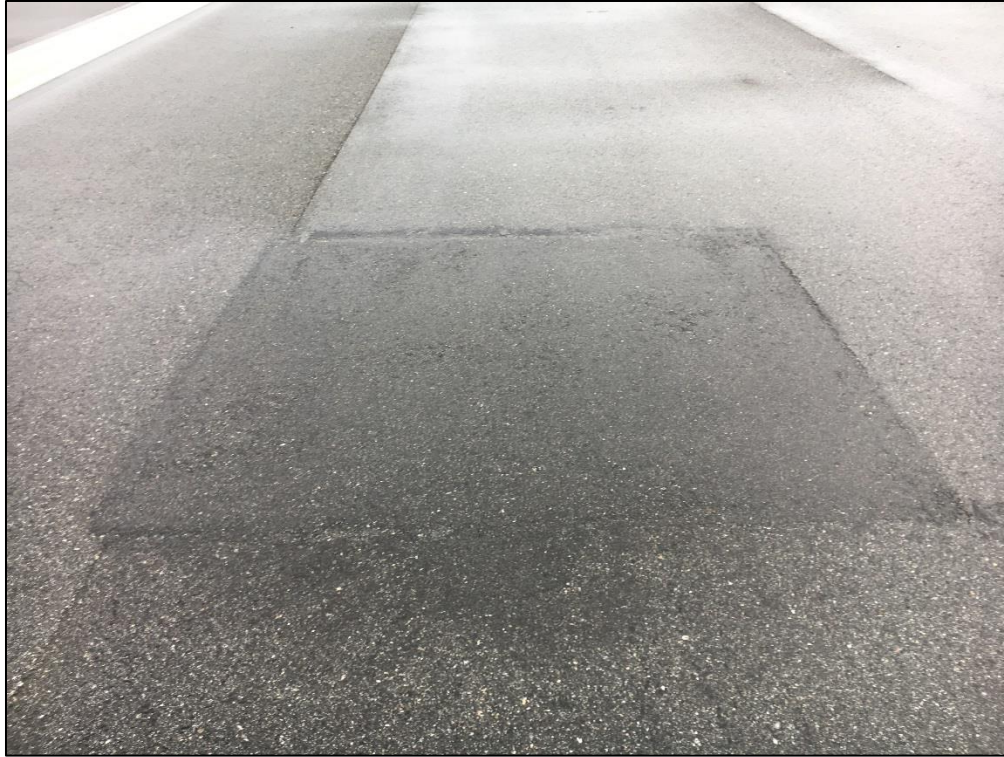
Runway 18-36, Section 6315, Sample Unit 326 – Low Severity (48) Longitudinal and Transverse Cracking, Low Severity (50) Patching, Low Severity (57) Weathering
