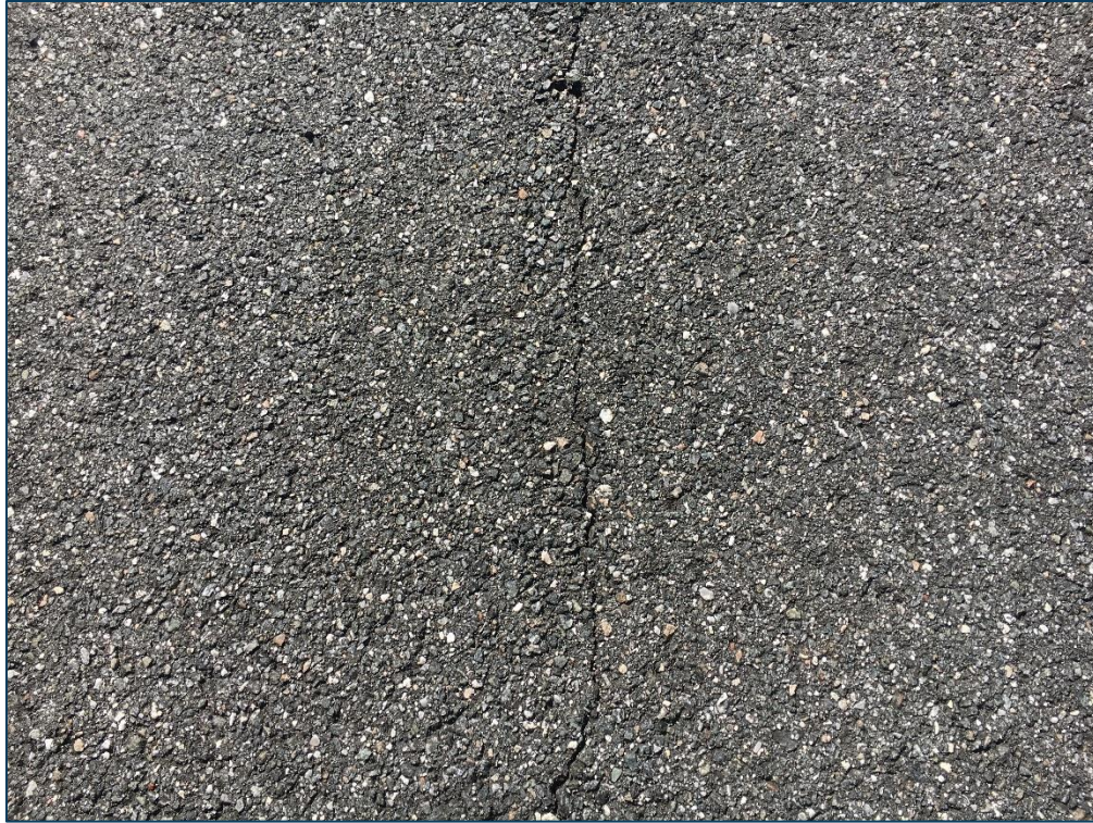
T-Hangar Taxilane, Section 4110, Sample Unit 601 – Low Severity (48) Longitudinal and Transverse Cracking, Low Severity (57) Weathering
