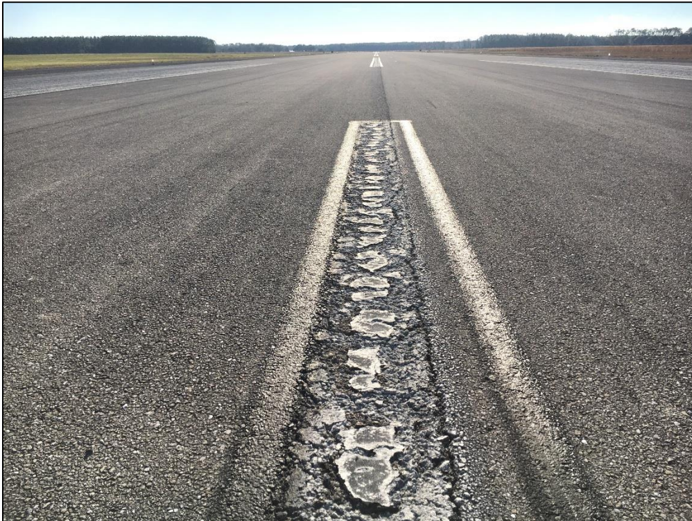
Runway 12-30, Section 6115, Sample Unit 374 – Low Severity (48) Longitudinal and Transverse Cracking, Low Severity (52) Raveling, Medium Severity (52) Raveling
