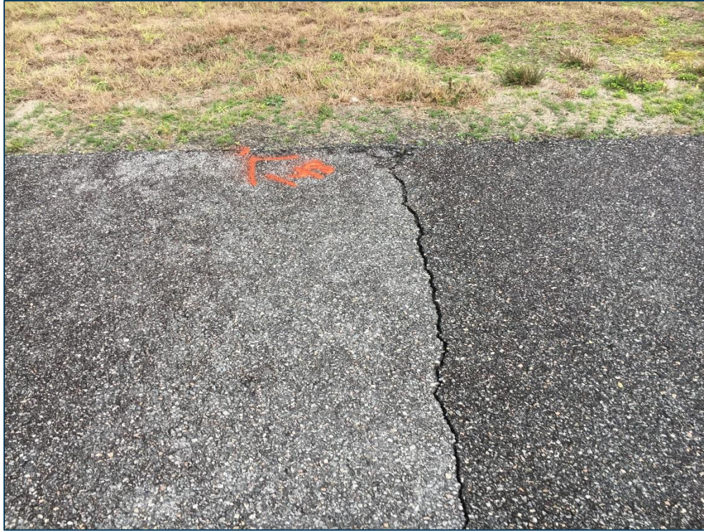
Taxiway C, Section 210, Sample Unit 148 – Medium Severity (48) Longitudinal and Transverse Cracking, Low Severity (52) Raveling
