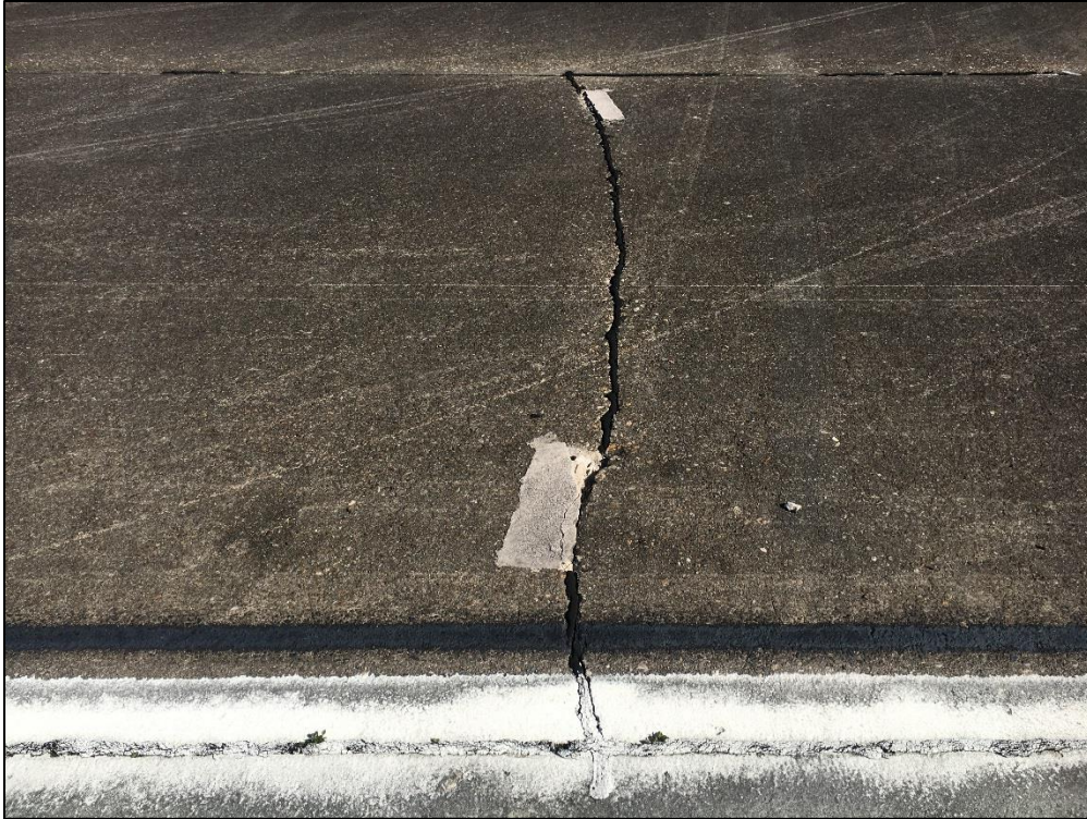
Runway 12-30, Section 6110, Sample Unit 302 – Medium Severity (63) Longitudinal, Transverse, and Diagonal Cracking, High Severity (65) Joint Seal Damage, Low Severity (66) Small Patching
