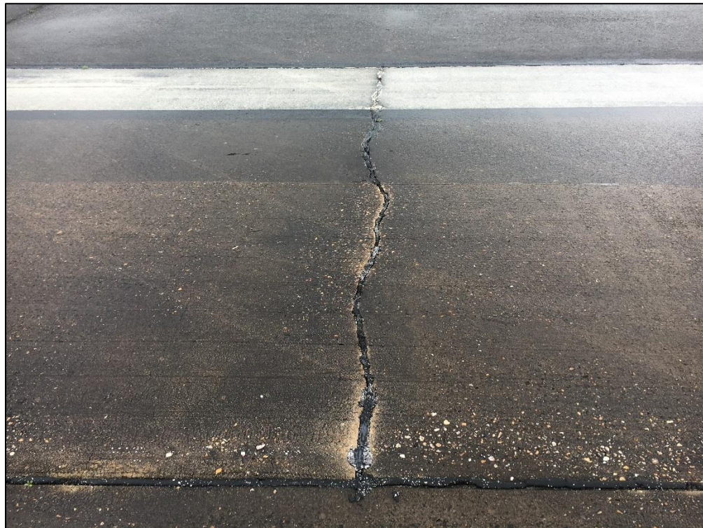
Runway 18-36, Section 6325, Sample Unit 393 – Medium Severity (63) Longitudinal, Transverse, and Diagonal Cracking, High Severity (65) Joint Seal Damage
