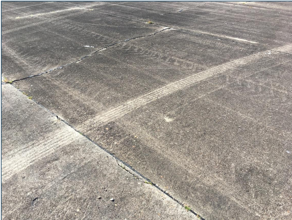
Runway 11-29, Section 6220, Sample Unit 103 – Low Severity (63) Longitudinal, Transverse, and Diagonal Cracking, Medium Severity (65) Joint Seal Damage, Low Severity (74) Joint Spalling
