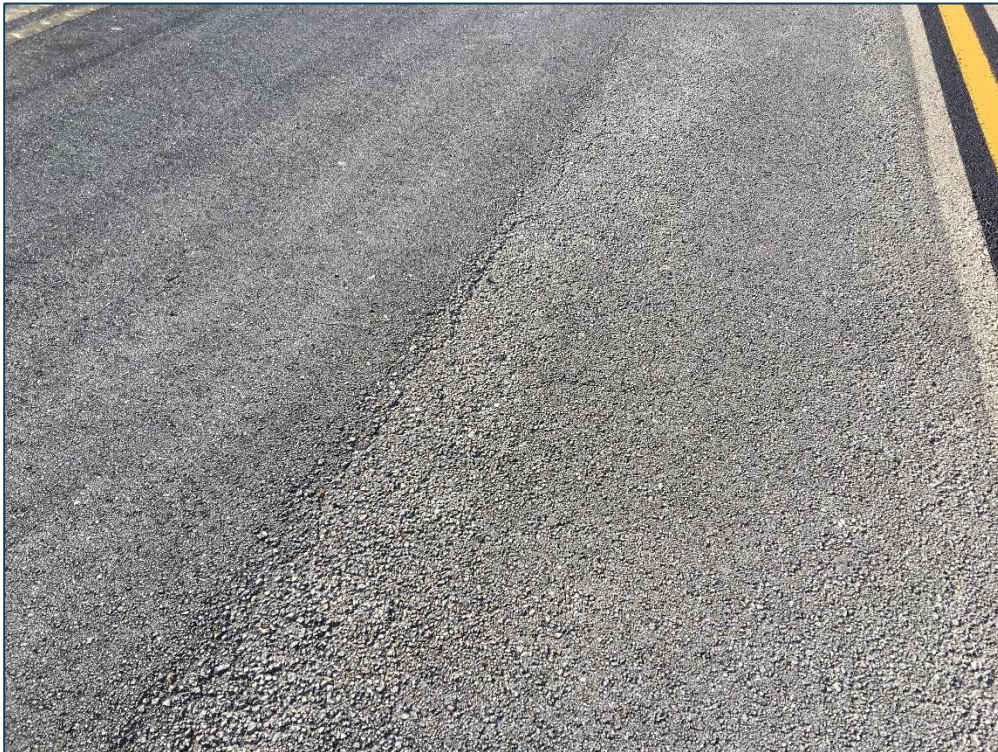
Taxiway B, Section 210, Sample Unit 111 – Low Severity (48) Longitudinal and Transverse Cracking, Low Severity (52) Raveling, Medium Severity (52) Raveling
