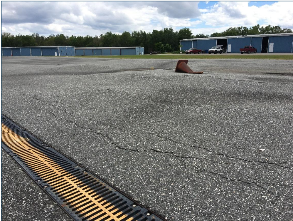
Apron T-Hangars, Section 4520, Sample Unit 402 – Low Severity (48) Longitudinal and Transverse Cracking, High Severity (56) Swelling
