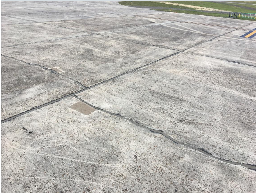
Apron, Section 4105, Sample Unit 205 – Low Severity (63) Longitudinal, Transverse, and Diagonal Cracking, Low Severity (66) Small Patching
