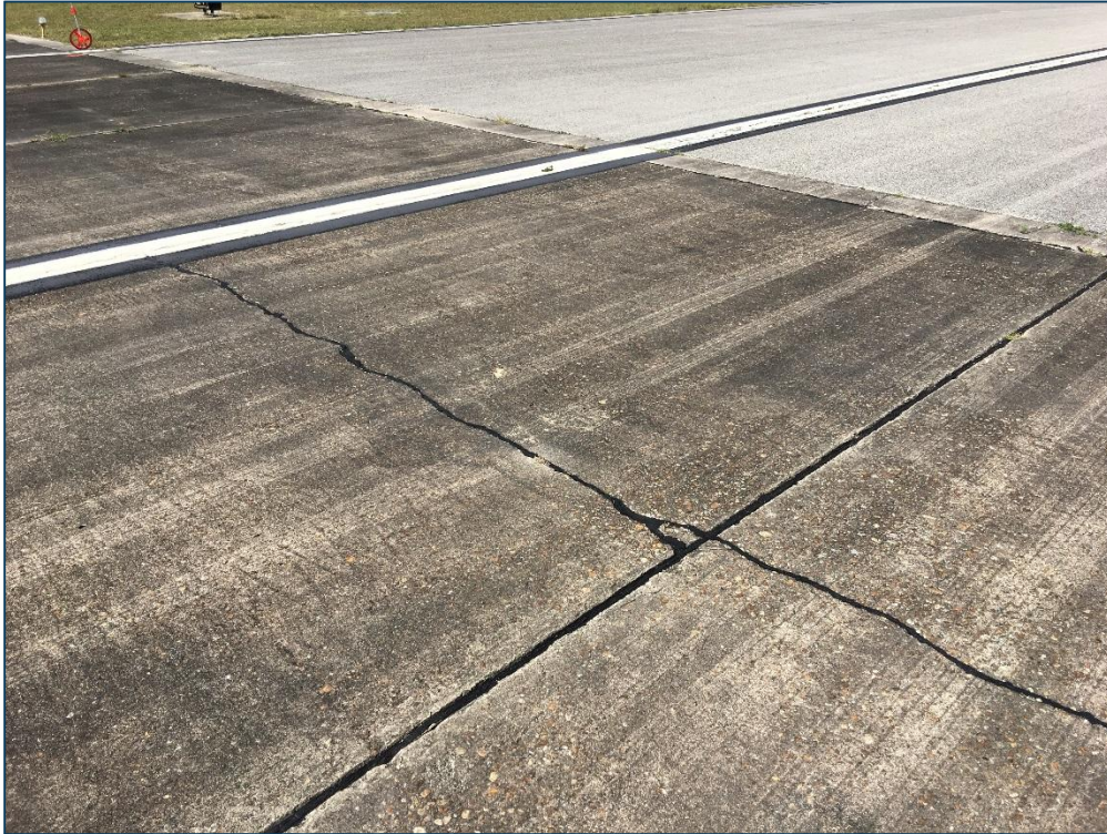
Runway 11-29, Section 6205, Sample Unit 195 – Low Severity (63) Longitudinal, Transverse, and Diagonal Cracking, Medium Severity (65) Joint Seal Damage
