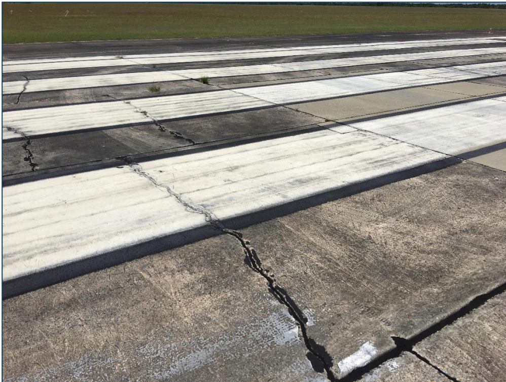
Runway 5-23, Section 6105, Sample Unit 297 – Low Severity (63) Longitudinal, Transverse, and Diagonal Cracking, Medium Severity (65) Joint Seal Damage, Low Severity (66) Small Patching
