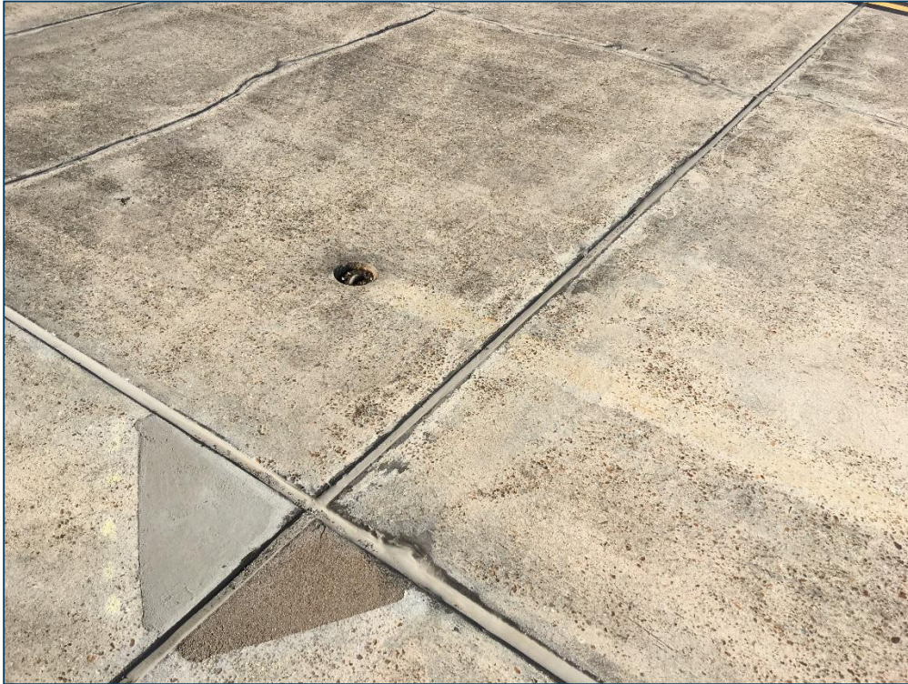
Apron, Section 4105, Sample Unit 500 – Low Severity (63) Longitudinal, Transverse, and Diagonal Cracking, Low Severity (66) Small Patching
