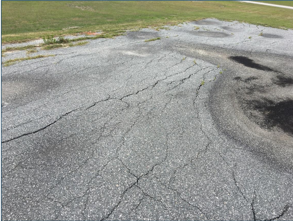
Apron T-Hangars, Section 4520, Sample Unit 402 – Low and Medium Severity (48) Longitudinal and Transverse Cracking, High Severity (56) Swelling
