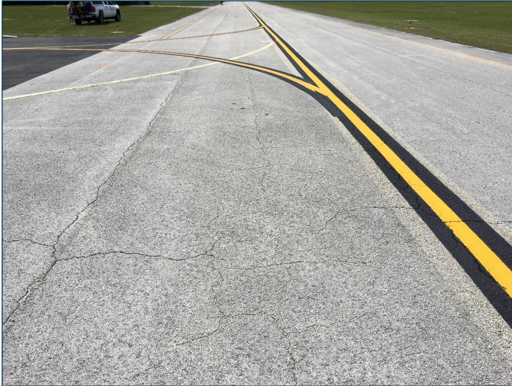
Taxiway A, Section 105, Sample Unit 122 – Low Severity (43) Block Cracking, Low Severity (48) Longitudinal and Transverse Cracking, Medium Severity (52) Raveling
