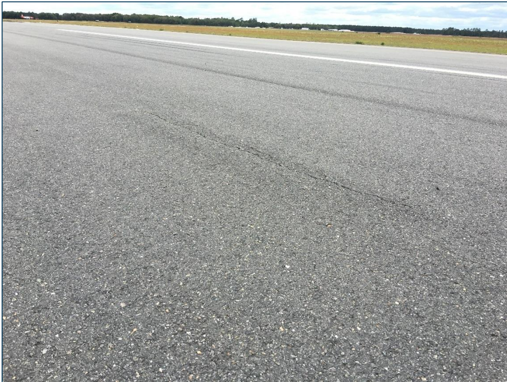
Runway 5-23, Section 6115, Sample Unit 332 – Low Severity (48) Longitudinal and Transverse Cracking, Low Severity (56) Swelling, Low Severity (57) Weathering
