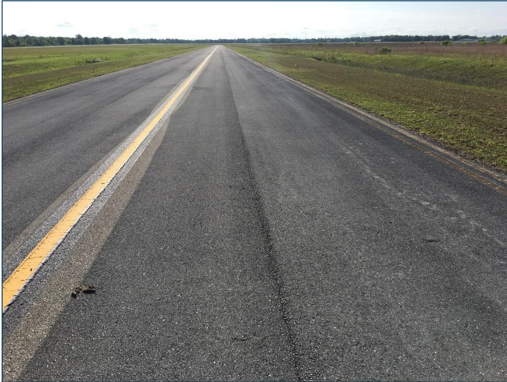
Taxiway C, Section 305, Sample Unit 139 – Low Severity (48) Longitudinal and Transverse Cracking, Low Severity (52) Raveling
