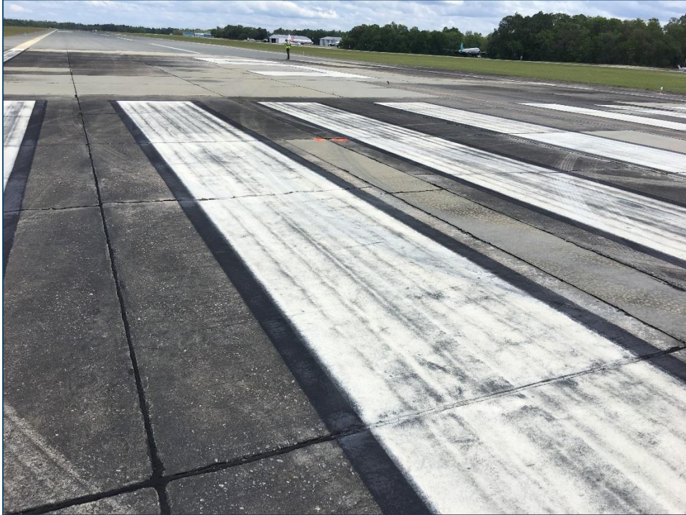
Runway 5-23, Section 6110, Sample Unit 96 – Medium Severity (65) Joint Seal Damage, Low Severity (67) Large Patching
