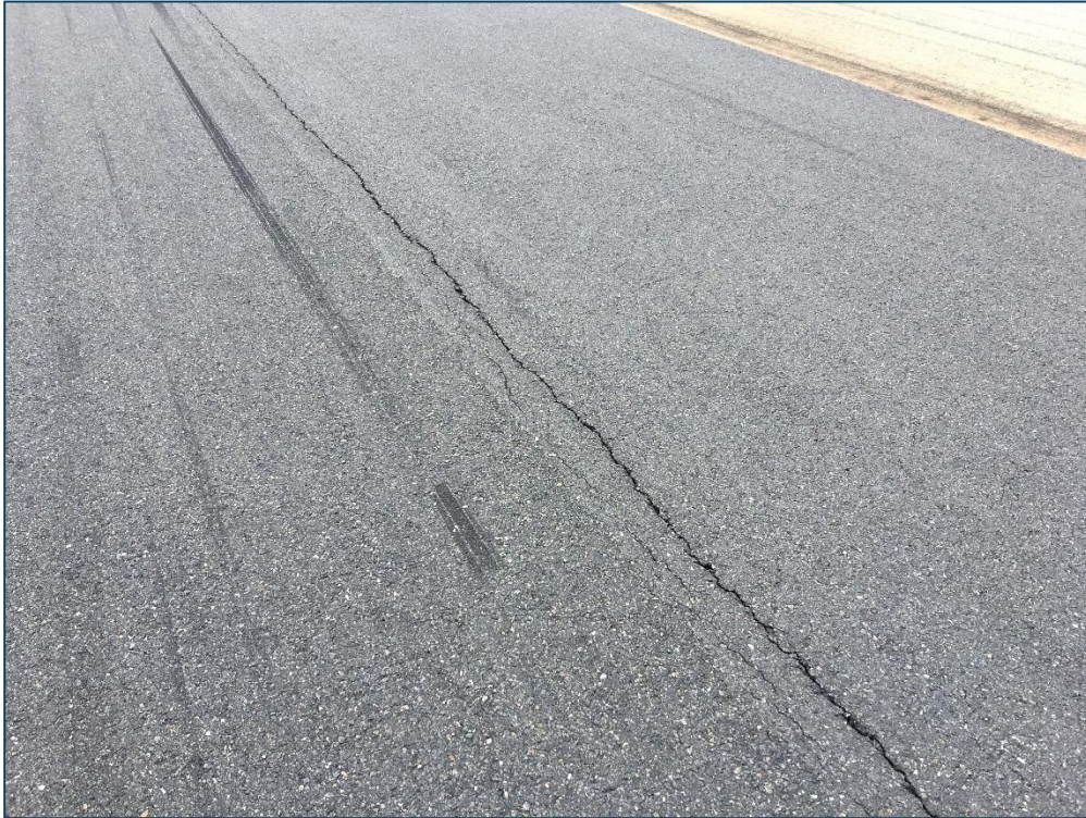
Runway 5-23, Section 6115, Sample Unit 307 – Low Severity (48) Longitudinal and Transverse Cracking, Low Severity (56) Swelling, Low Severity (57) Weathering
