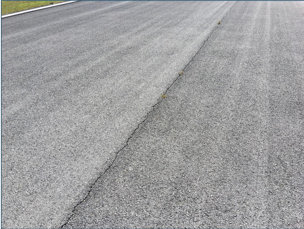
Runway 11-29, Section 6215, Sample Unit 156 – Low and Medium Severity (48) Longitudinal and Transverse Cracking, Low Severity (52) Raveling
