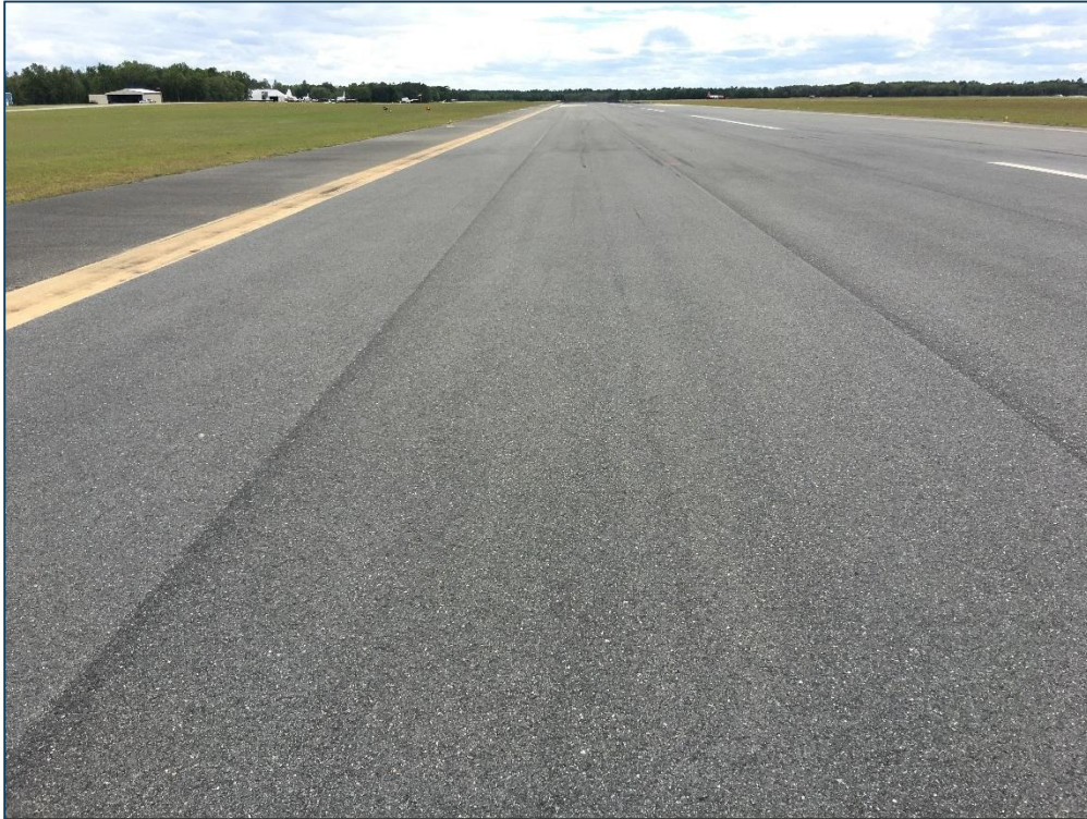
Runway 5-23, Section 6120, Sample Unit 542 – Low Severity (48) Longitudinal and Transverse Cracking, Low Severity (57) Weathering
