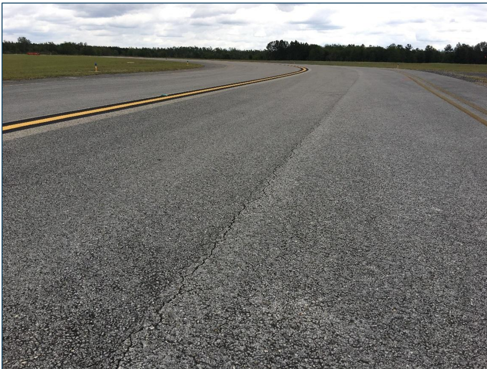
Taxiway A, Section 105, Sample Unit 147 – Low Severity (48) Longitudinal and Transverse Cracking, Medium Severity (52) Raveling
