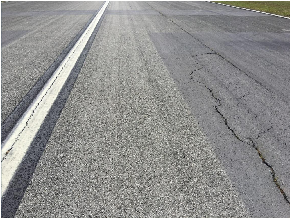
Runway 11-29, Section 6215, Sample Unit 170 – Low and Medium Severity (48) Longitudinal and Transverse Cracking, Low Severity (52) Raveling
