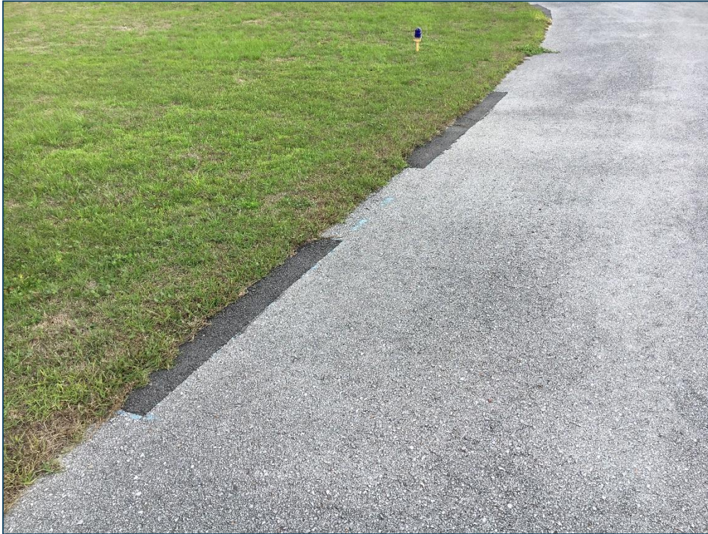
Taxiway A, Section 530, Sample Unit 100 – Low Severity (50) Patching, Low Severity (52) Raveling, Low Severity (57) Weathering
