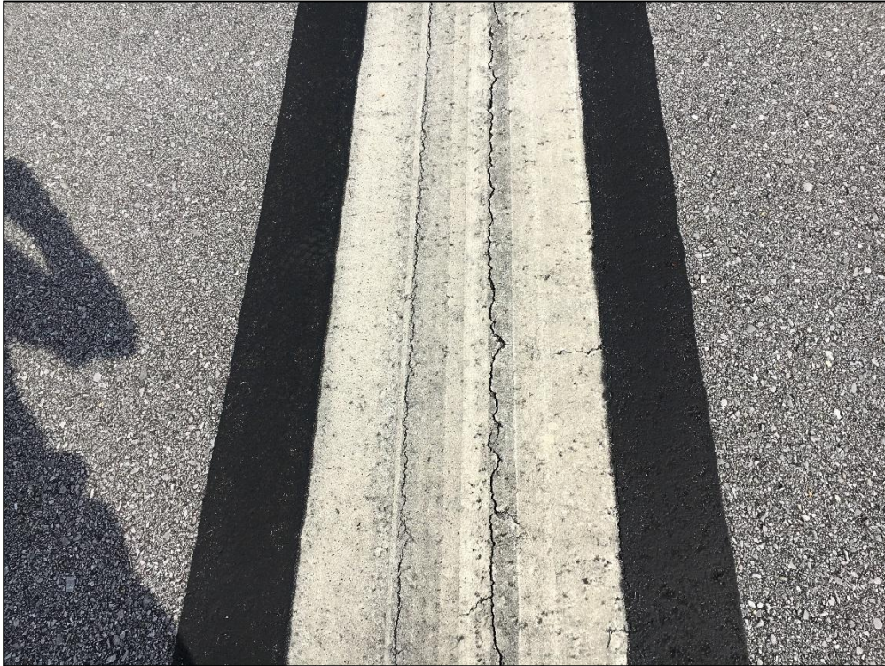
Runway 9-27, Section 6110, Sample Unit 130 – Low Severity (48) Longitudinal and Transverse Cracking, Low Severity (57) Weathering
