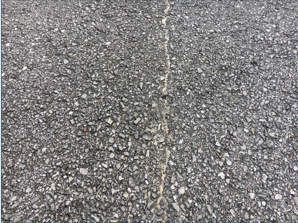
South Apron, Section 4305, Sample Unit 99 – Low Severity (48) Longitudinal and Transverse Cracking, Low Severity (52) Raveling, Low Severity (57) Weathering
