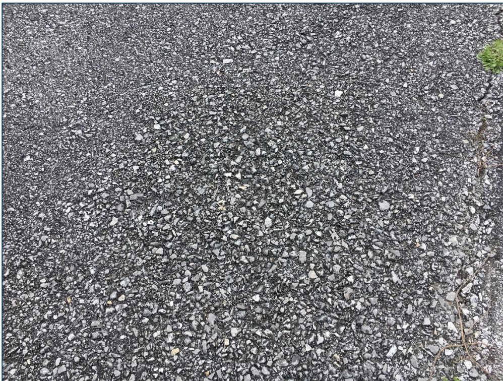
Taxiway A1, Section 305, Sample Unit 101 – Low Severity (48) Longitudinal and Transverse Cracking, Low Severity (52) Raveling, Low Severity (57) Weathering
