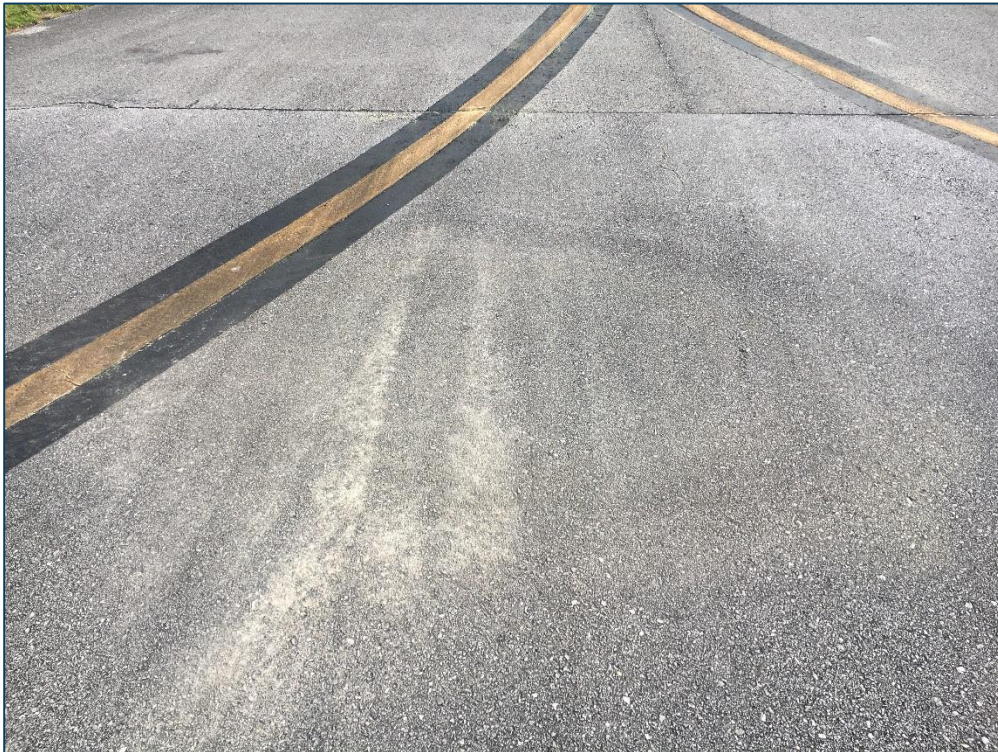
Taxiway B, Section 710, Sample Unit 116 – Low Severity (45) Depression, Low Severity (48) Longitudinal and Transverse Cracking, Low Severity (57) Weathering
