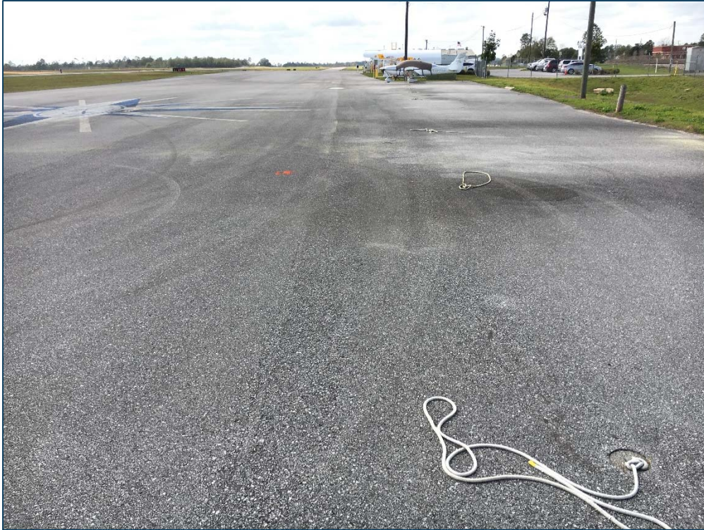
Northeast Apron, Section 4110, Sample Unit 205 – Low Severity (45) Depression, Low Severity (52) Raveling, Low Severity (57) Weathering
