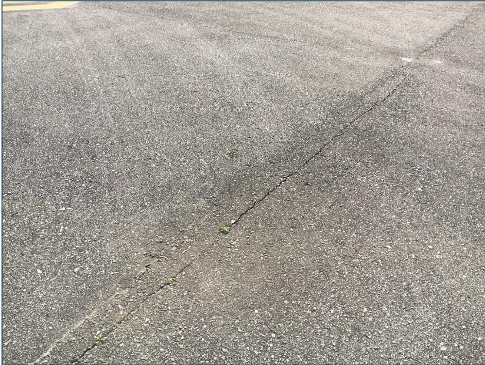
Taxiway A4, Section 525, Sample Unit 101 – Low Severity (48) Longitudinal and Transverse Cracking, Low Severity (45) Depression, Low Severity (52) Raveling, Low Severity (57) Weathering
