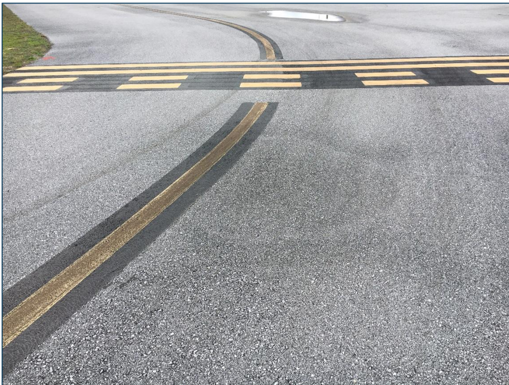
Taxiway A, Section 110, Sample Unit 101 – Low Severity (45) Depression, Low Severity (57) Weathering
