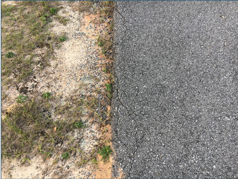
Taxiway B, Section 710, Sample Unit 104 – Low Severity (48) Longitudinal and Transverse Cracking, Low Severity (57) Weathering
