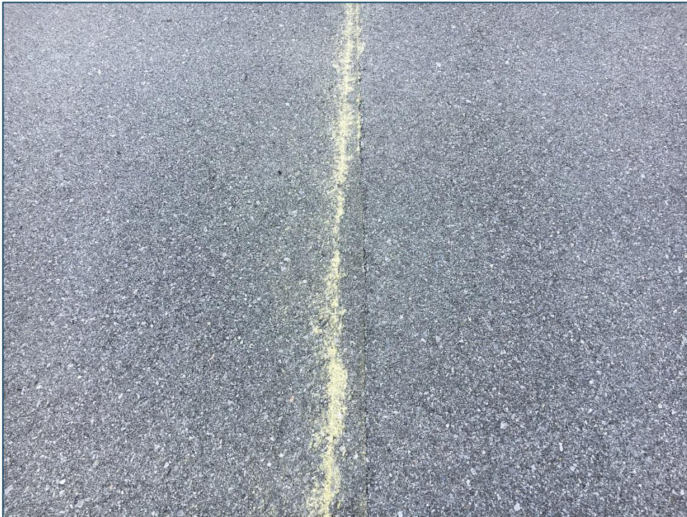
West Apron, Section 4405, Sample Unit 106 – Low Severity (48) Longitudinal and Transverse Cracking, Low Severity (57) Weathering
