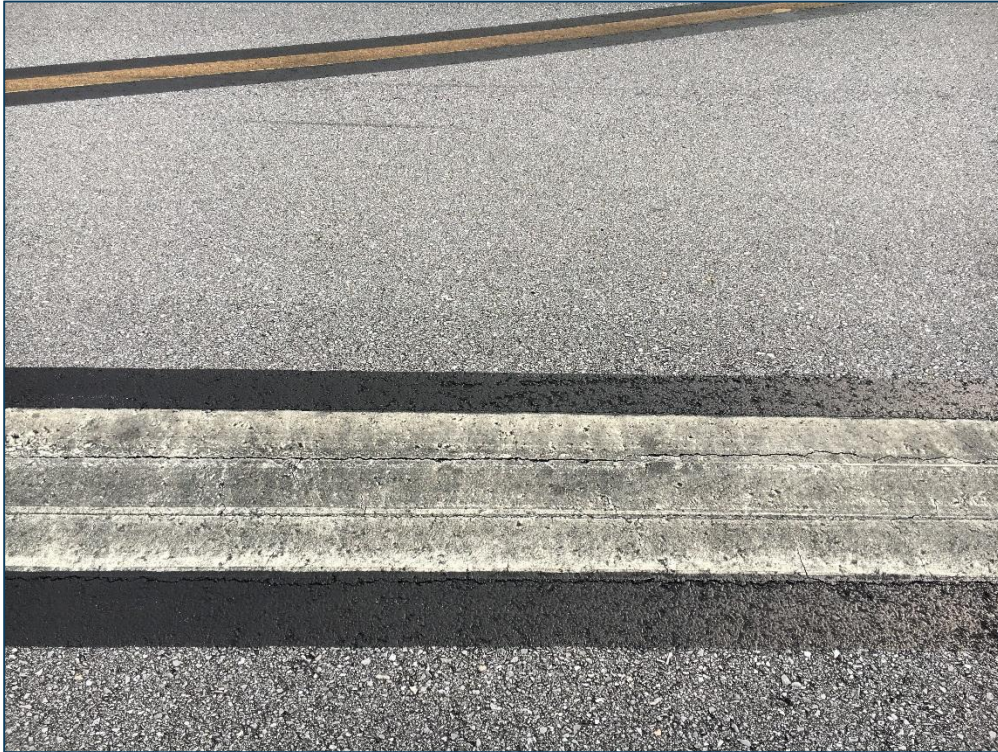
Taxiway A2, Section 405, Sample Unit 100 – Low Severity (48) Longitudinal and Transverse Cracking, Low Severity (52) Raveling, Low Severity (57) Weathering
