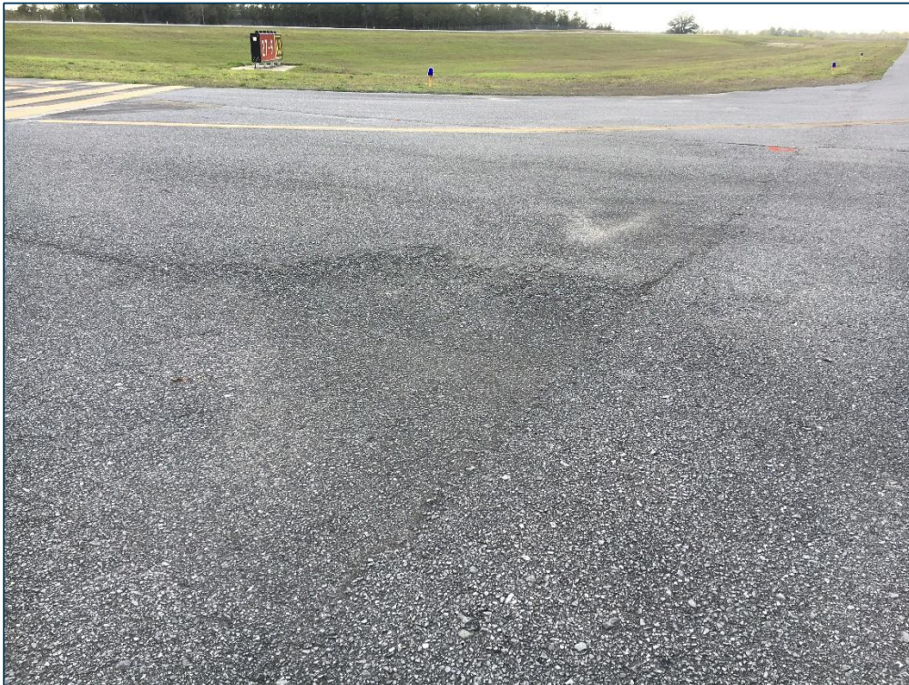
Taxiway A3, Section 603, Sample Unit 101 – Low Severity (45) Depression, Low Severity (52) Raveling, Low Severity (57) Weathering
