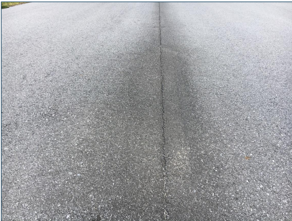
T-Hangar Taxilane, Section 4410, Sample Unit 501 – Low Severity (48) Longitudinal and Transverse Cracking, Low Severity (57) Weathering
