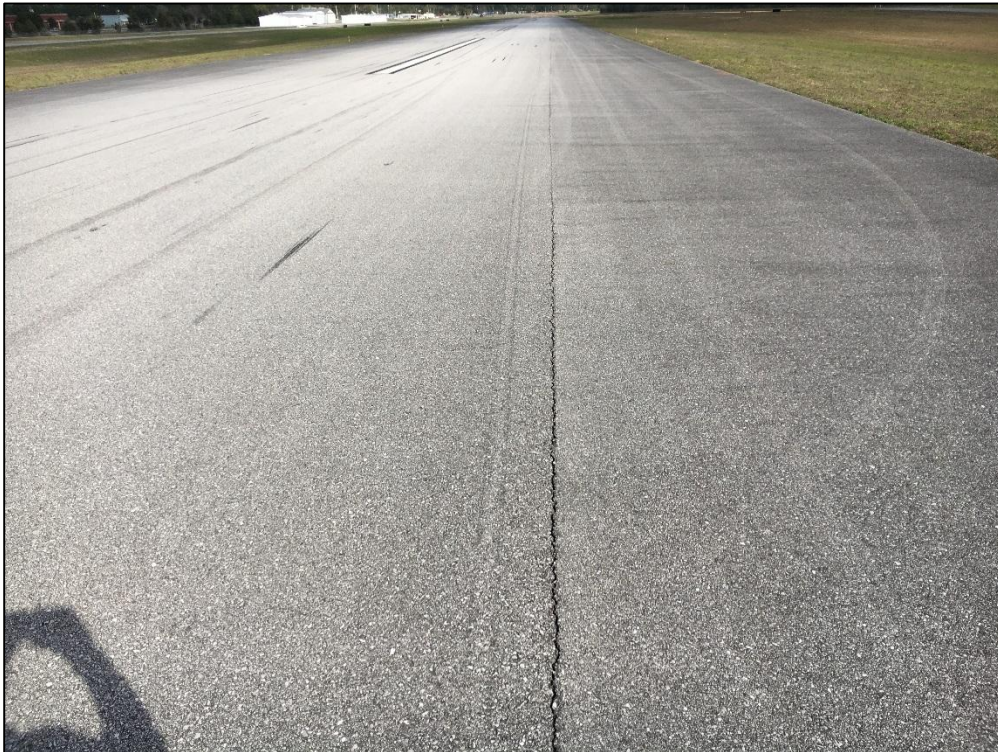
Runway 9-27, Section 6110, Sample Unit 103 - Low Severity (48) Longitudinal and Transverse Cracking, Low Severity (52) Raveling, Low Severity (57) Weathering
