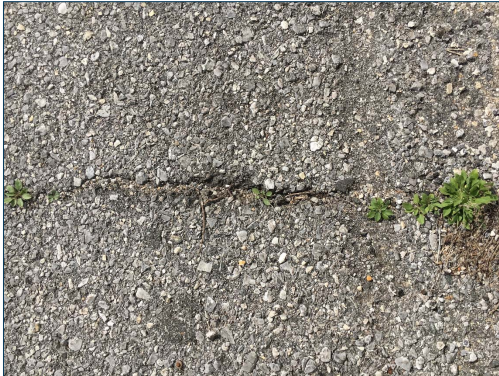
Apron, Section 4210, Sample Unit 301 – Low Severity (48) Longitudinal and Transverse Cracking, Low Severity (52) Raveling, Low Severity (57) Weathering
