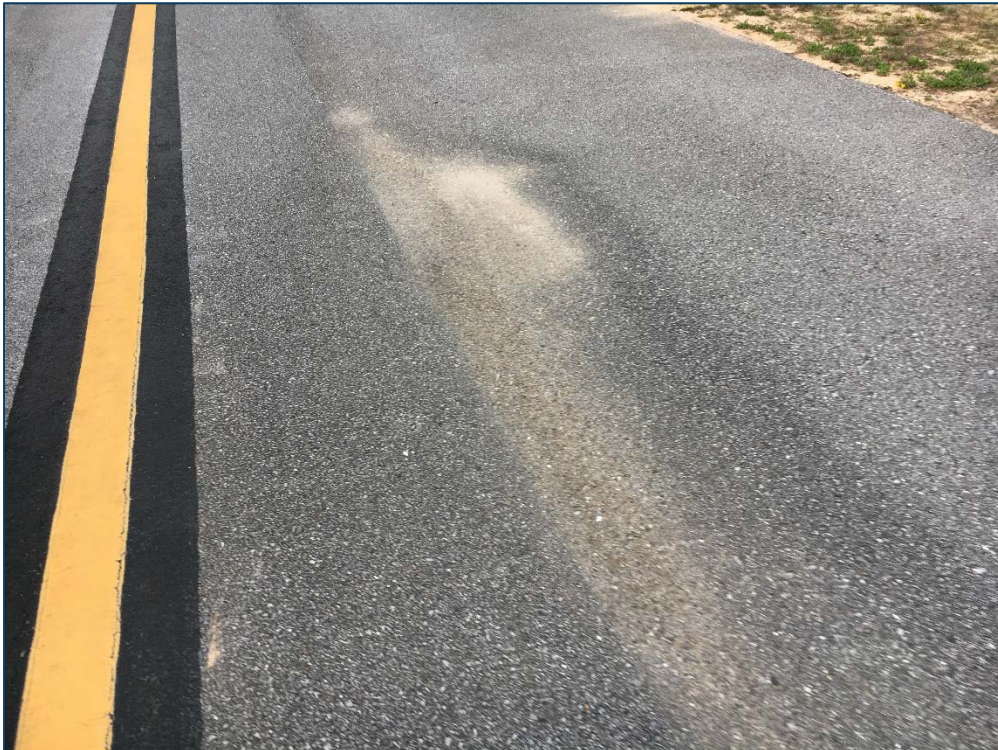
South Apron, Section 4305, Sample Unit 99 – Low Severity (45) Depression, Low Severity (48) Longitudinal and Transverse Cracking, Low Severity (52) Raveling, Low Severity (57) Weathering
