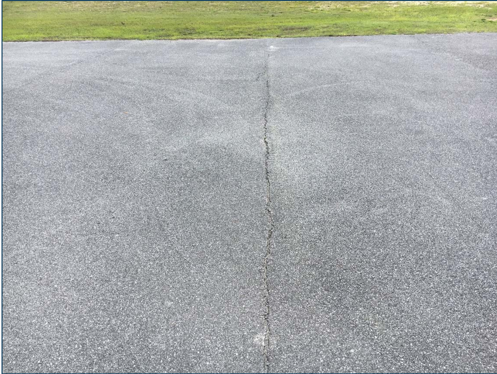
Apron North, Section 4205, Sample Unit 103 – Medium Severity (48) Longitudinal and Transverse Cracking, Low Severity (45) Depression, Low Severity (52) Raveling, Low Severity (57) Weathering
