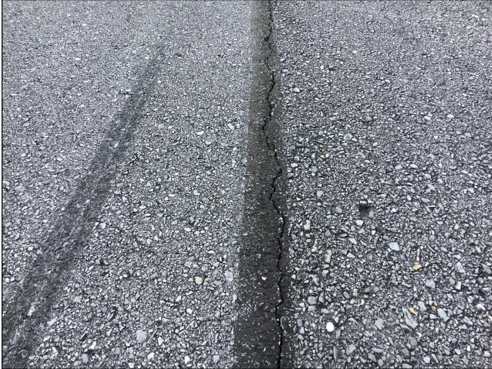
Runway 9-27, Section 6120, Sample Unit 95 – Low Severity (48) Longitudinal and Transverse Cracking, Low Severity (52) Raveling
