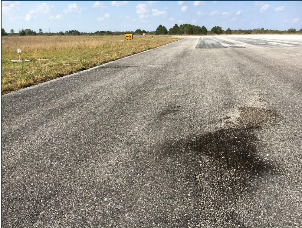
Runway 5-23, Section 6102, Sample Unit 074 – Low Severity (52) Raveling, Medium Severity (52) Raveling
