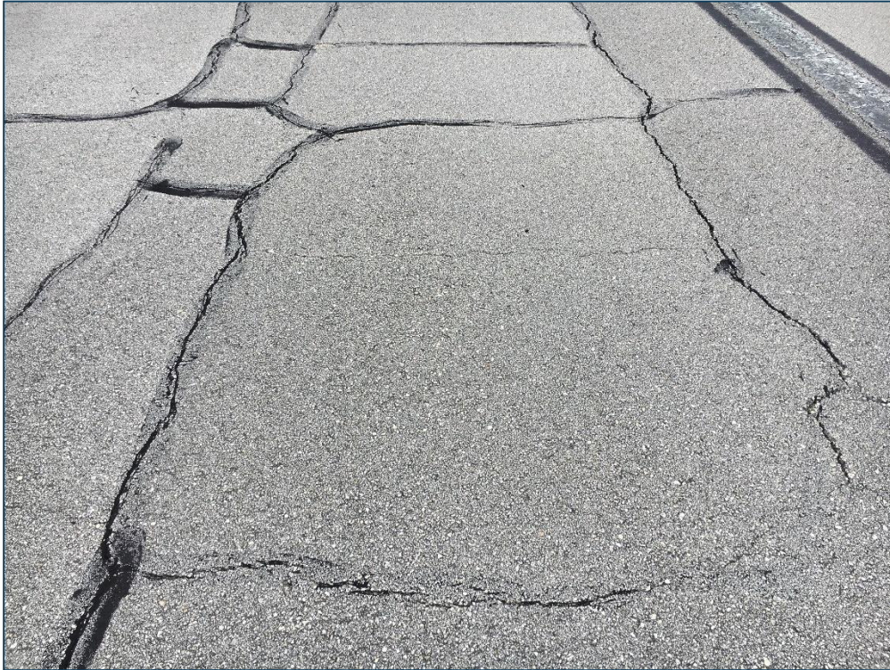
Runway 10-28, Section 6205, Sample Unit 130 – Low Severity (43) Block Cracking, Low Severity (48) Longitudinal and Transverse Cracking, Low Severity (57) Weathering
