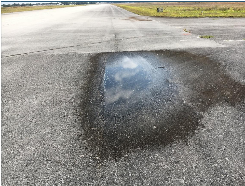
Runway 5-23, Section 6102, Sample Unit 099 – Medium Severity (48) Longitudinal and Transverse Cracking, Low Severity (45) Depression, Low Severity (52) Raveling
