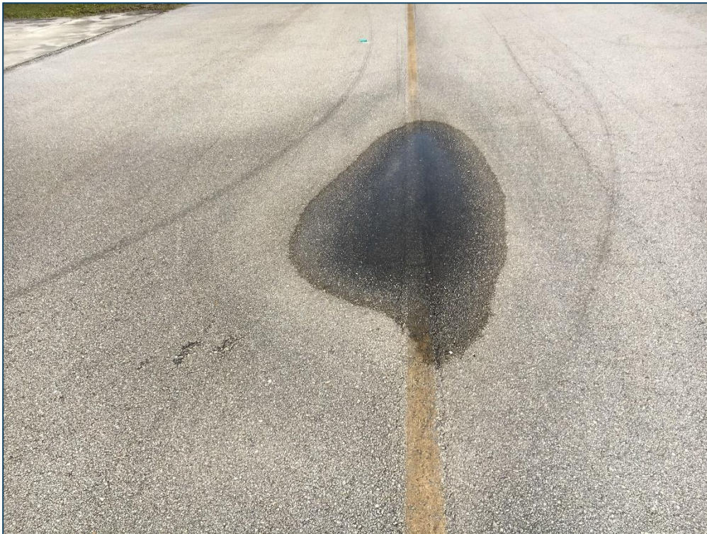
Apron T-Hangar, Section 4605, Sample Unit 402 – Low Severity (45) Depression, Low Severity (52) Raveling, Medium Severity (52) Raveling
