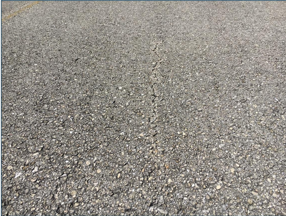
Taxiway E, Section 505, Sample Unit 129 – Low Severity (48) Longitudinal and Transverse Cracking, Low Severity (52) Raveling, Low Severity (57) Weathering
