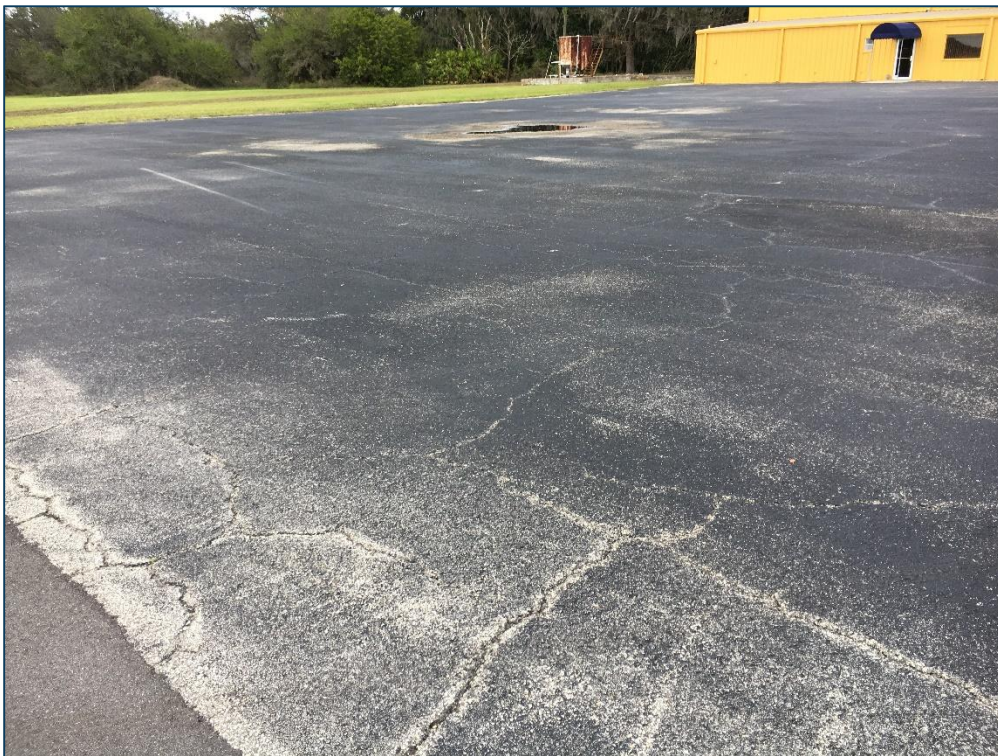
Apron SE, Section 4405, Sample Unit 300 – Low Severity (43) Block Cracking, Low Severity (45) Depression, Low Severity (52) Raveling
