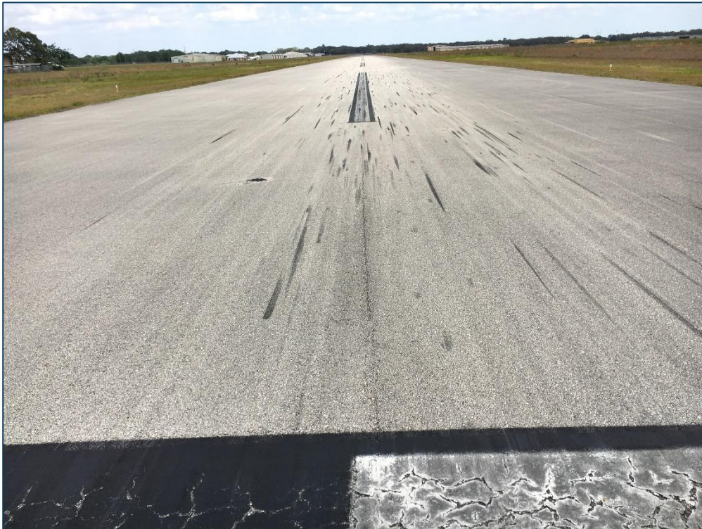
Runway 10-28, Section 6205, Sample Unit 105 – Low Severity (48) Longitudinal and Transverse Cracking, Low Severity (52) Raveling, Low Severity (57) Weathering
