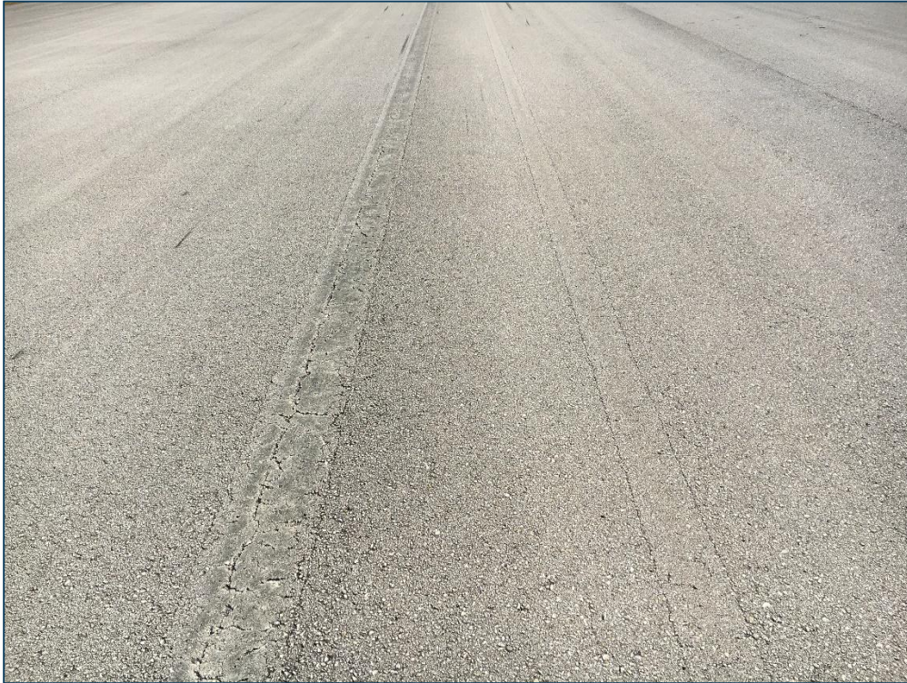
Runway 5-23, Section 6105, Sample Unit 121 – Low Severity (52) Raveling, Low Severity (57) Weathering
