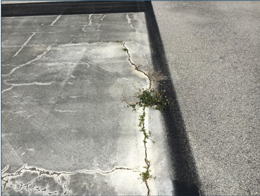
Runway 10-28, Section 6220, Sample Unit 176 – Medium Severity (48) Longitudinal and Transverse Cracking, Low Severity (52) Raveling, Low Severity (57) Weathering
