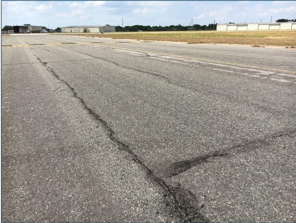
Taxiway A, Section 105, Sample Unit 103 – Medium Severity (43) Block Cracking, Low Severity (52) Raveling
