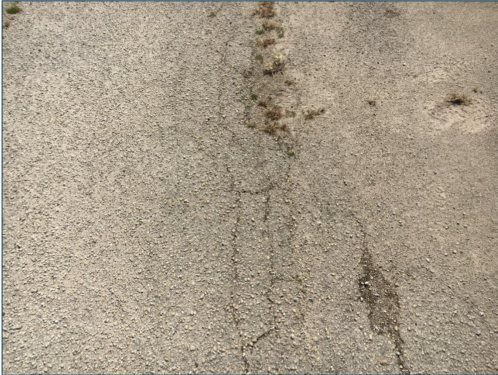
South Apron, Section 4305, Sample Unit 302 – Low Severity (41) Alligator Cracking, Medium Severity (52) Raveling
