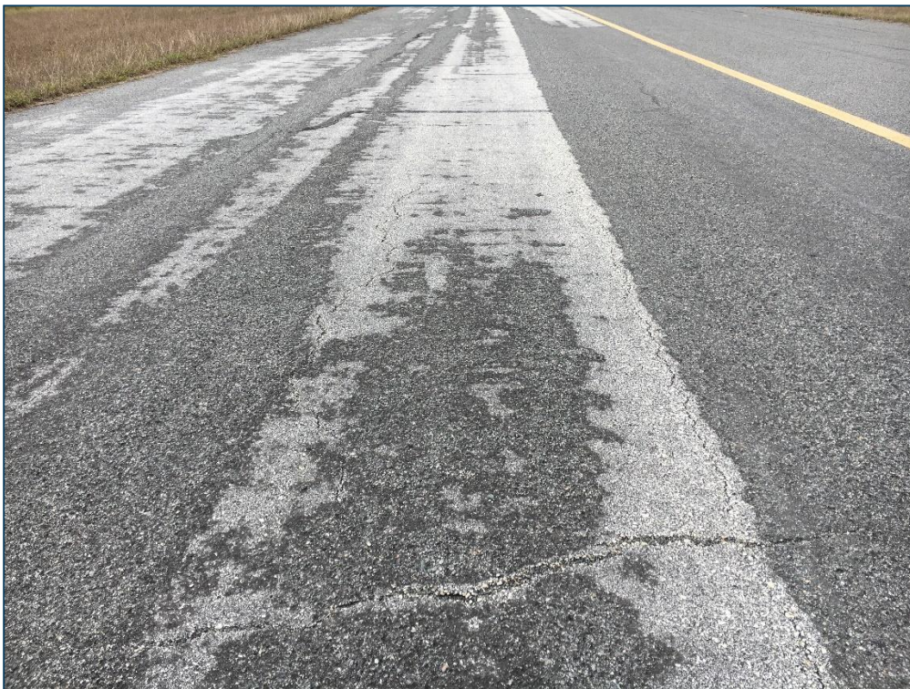
Taxiway A, Section 120, Sample Unit 108 – Low Severity (48) Longitudinal and Transverse Cracking, Low Severity (52) Raveling
