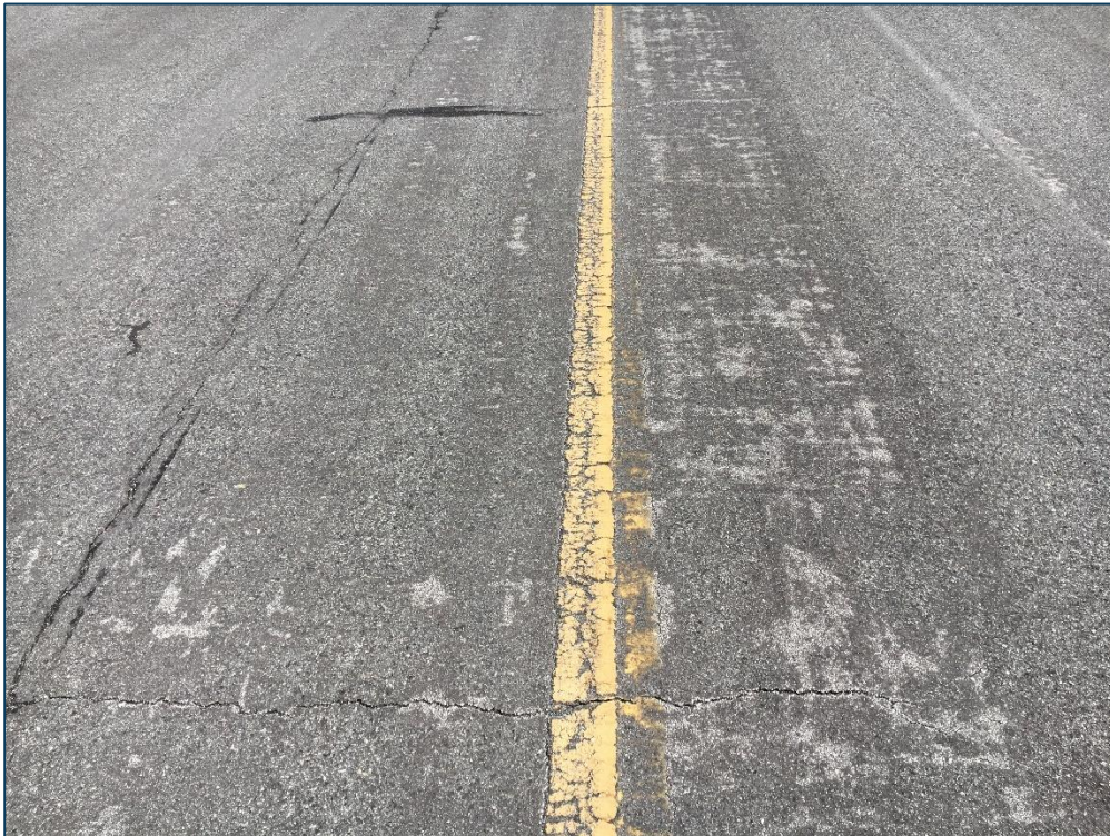
Taxiway A, Section 135, Sample Unit 110 – Low Severity (48) Longitudinal and Transverse Cracking, Low Severity (52) Raveling
