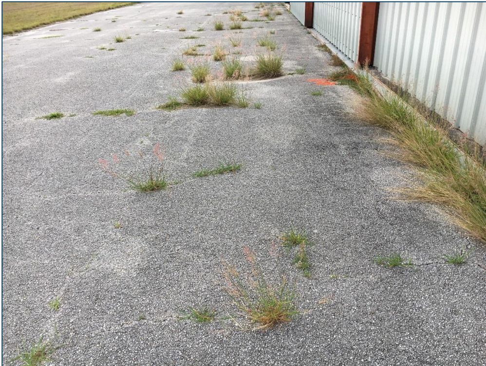
Apron NW, Section 4105, Sample Unit 101 – Low Severity (43) Block Cracking, Medium Severity (43) Block Cracking, Low Severity (52) Raveling
