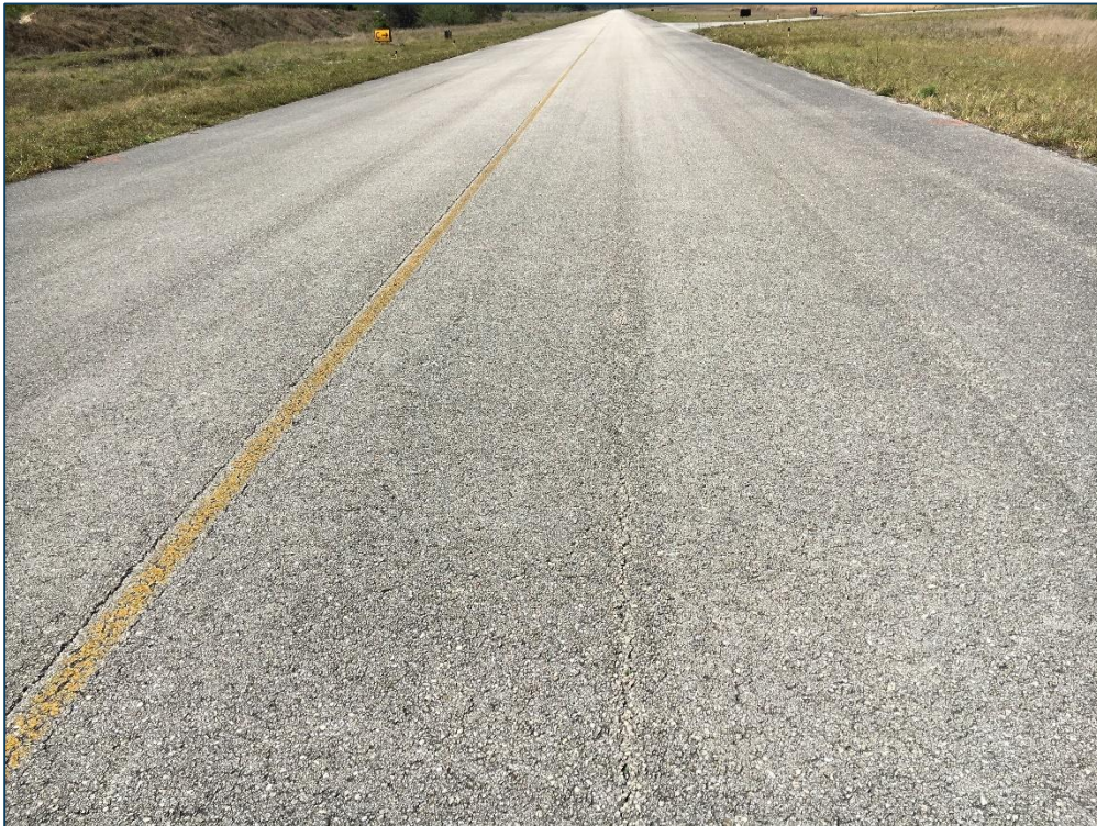
Taxiway E, Section 505, Sample Unit 113 – Low Severity (48) Longitudinal and Transverse Cracking, Low Severity (52) Raveling, Low Severity (57) Weathering
