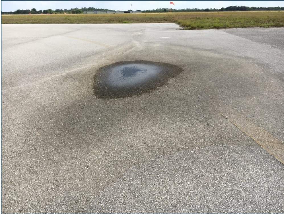
Apron NE, Section 4215, Sample Unit 200 – Low Severity (45) Depression, Low Severity (57) Weathering
