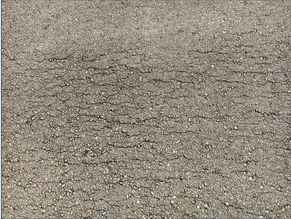
Runway 5-23, Section 6105, Sample Unit 177 – Low Severity (48) Longitudinal and Transverse Cracking, Low Severity (52) Raveling, Low Severity (57) Weathering
