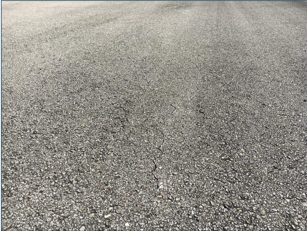
Taxiway E, Section 502, Sample Unit 104 – Low Severity (48) Longitudinal and Transverse Cracking, Low Severity (52) Raveling, Low Severity (57) Weathering
