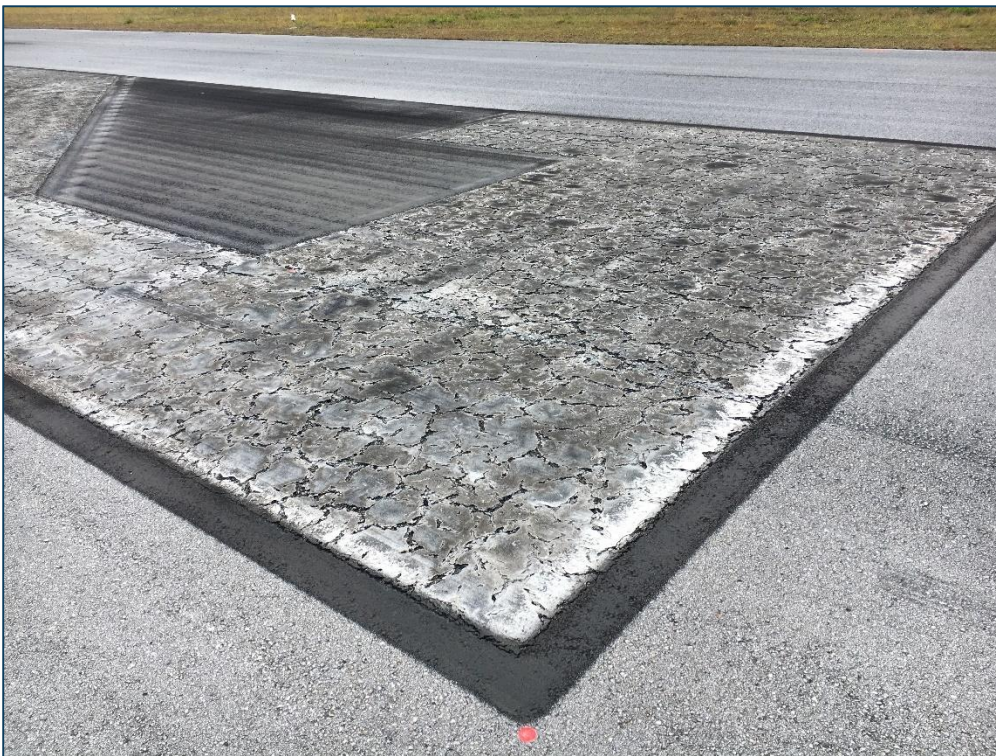
Runway 5-23, Section 6105, Sample Unit 151 – Low Severity (52) Raveling, Medium Severity (52) Raveling
