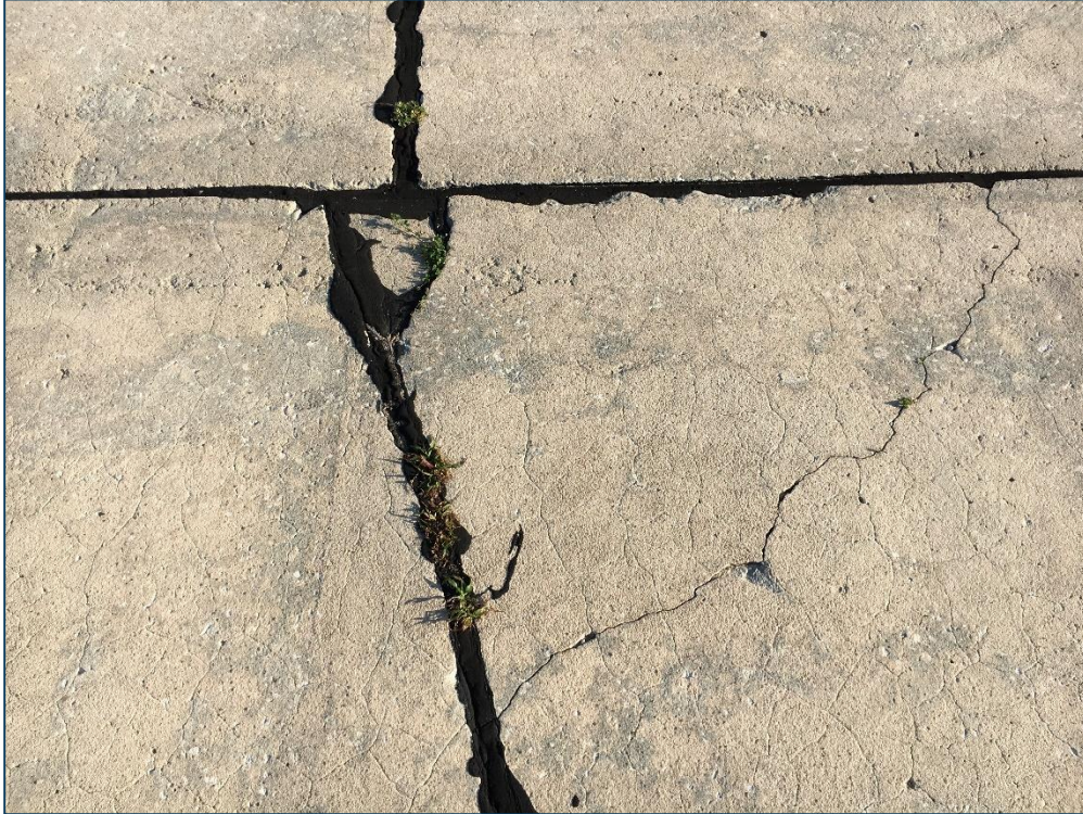
Runway 9-27, Section 6110, Sample Unit 300 – Medium Severity (63) Longitudinal, Transverse, and Diagonal Cracking, Low Severity (65) Joint Seal Damage, (73) Shrinkage Cracks
