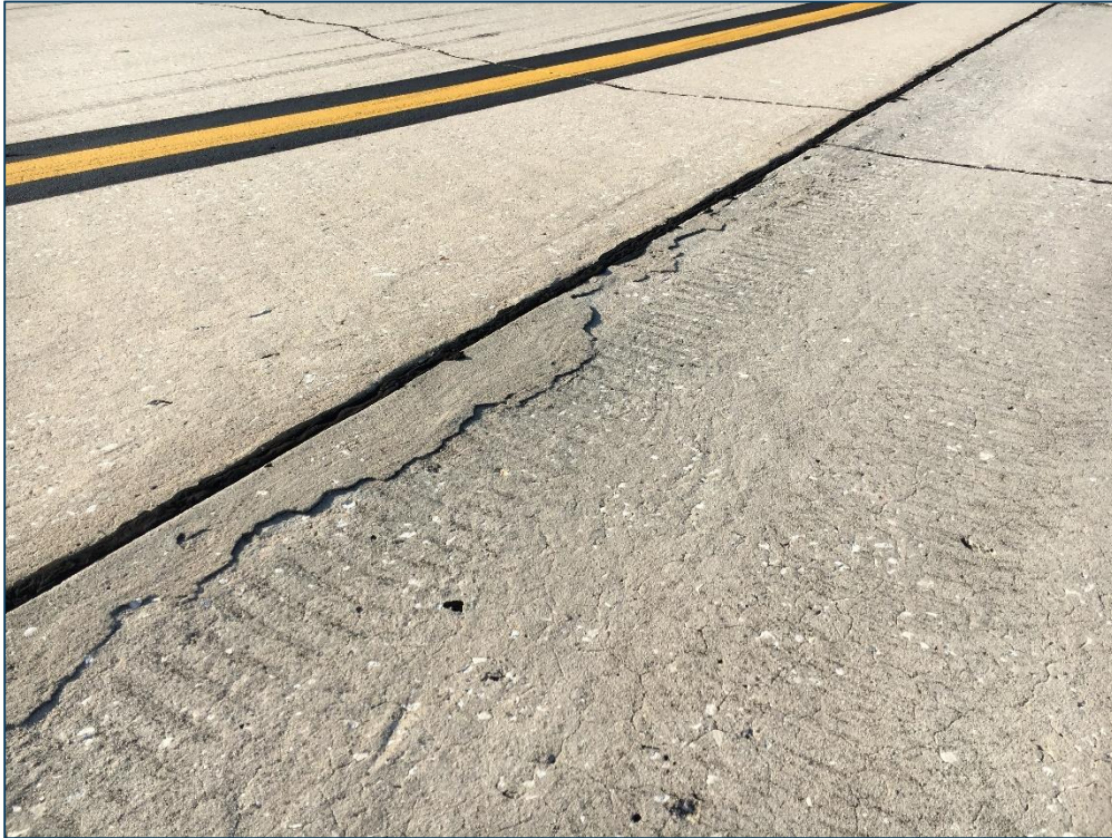
Runway 3-21, Section 6210, Sample Unit 367 – Low Severity (63) Longitudinal, Transverse, and Diagonal Cracking, Low Severity (65) Joint Seal Damage, Low Severity (70) Scaling, Map Cracking, Cracking, (73) Shrinkage Cracks
