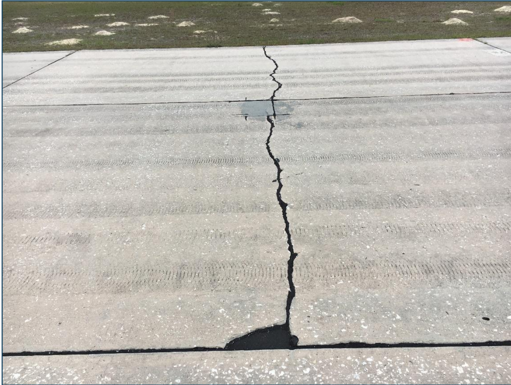
Taxiway A, Section 105, Sample Unit 107 – Low Severity (63) Longitudinal, Transverse, and Diagonal Cracking, Low Severity (65) Joint Seal Damage, Low Severity (66) Small Patching, (73) Shrinkage Cracks
