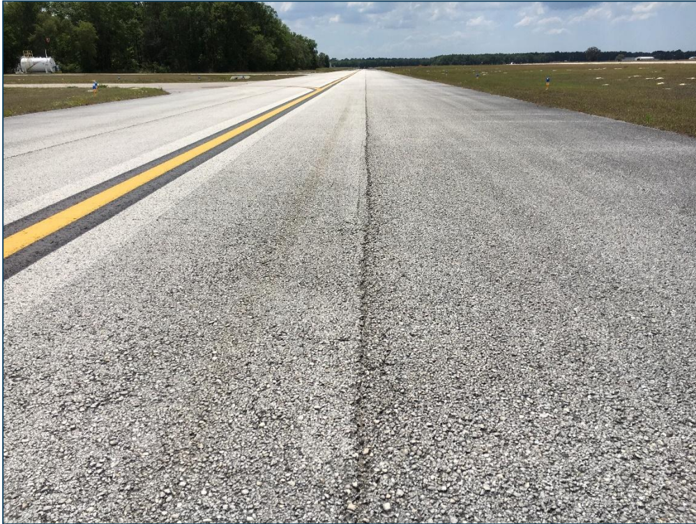
Taxiway B, Section 210, Sample Unit 128 – Low Severity (48) Longitudinal and Transverse Cracking, Low Severity (52) Raveling
