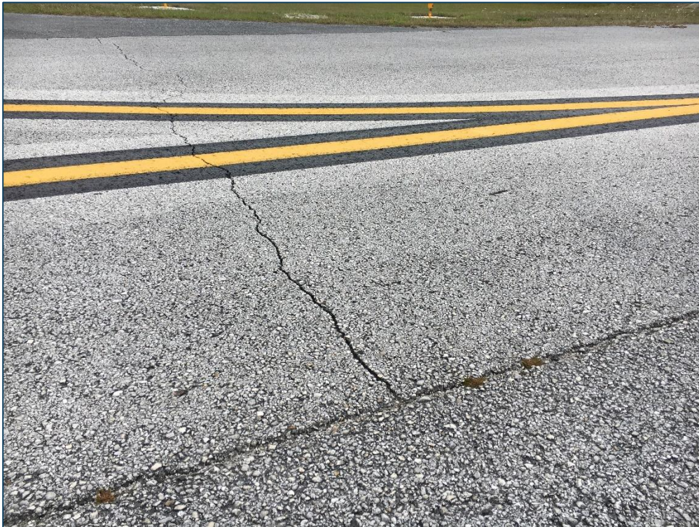
Taxiway B, Section 210, Sample Unit 104 – Low and Medium Severity (48) Longitudinal and Transverse Cracking, Low Severity (52) Raveling
