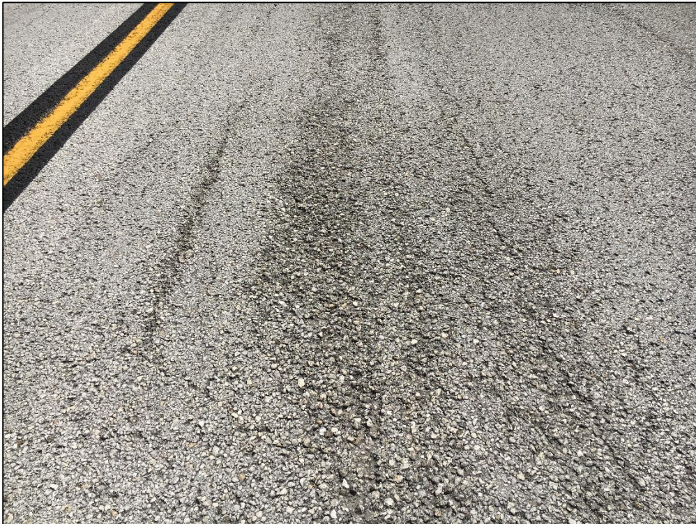
Taxiway A3, Section 125, Sample Unit 301 – Low Severity (48) Longitudinal and Transverse Cracking, Medium Severity (52) Raveling, High Severity (52) Raveling
