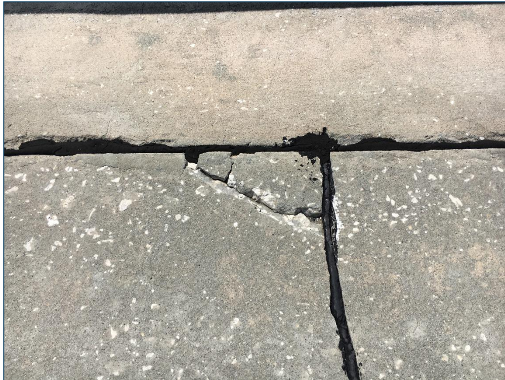
Runway 9-27, Section 6110, Sample Unit 439 – Low Severity (63) Longitudinal, Transverse, and Diagonal Cracking, Low Severity (65) Joint Seal Damage, Low Severity (74) Joint Spalling
