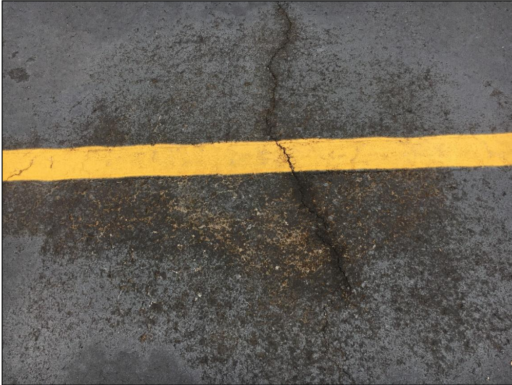
Apron NE, Section 4140, Sample Unit 207 – Low Severity (48) Longitudinal and Transverse Cracking, (49) Oil Spillage, Low Severity (57) Weathering
