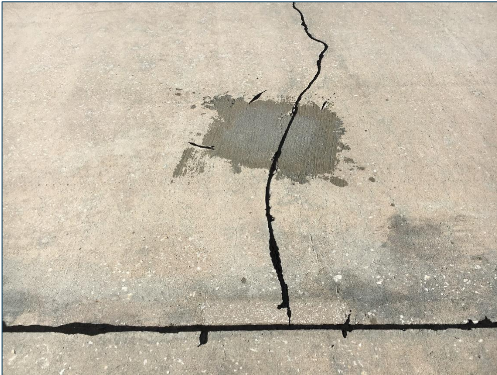
Runway 9-27, Section 6110, Sample Unit 349 – Medium Severity (63) Longitudinal, Transverse, and Diagonal Cracking, Low Severity (65) Joint Seal Damage, Low Severity (66) Small Patching, (73) Shrinkage Cracks
