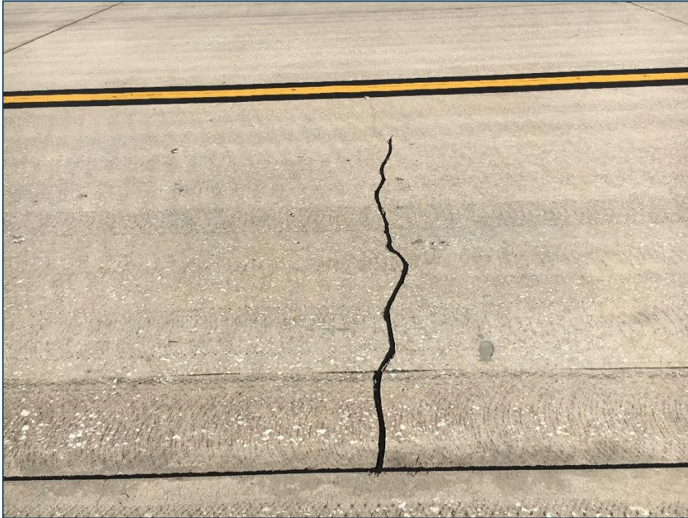
Taxiway A, Section 105, Sample Unit 268 – Low Severity (63) Longitudinal, Transverse, and Diagonal Cracking, Low Severity (65) Joint Seal Damage
