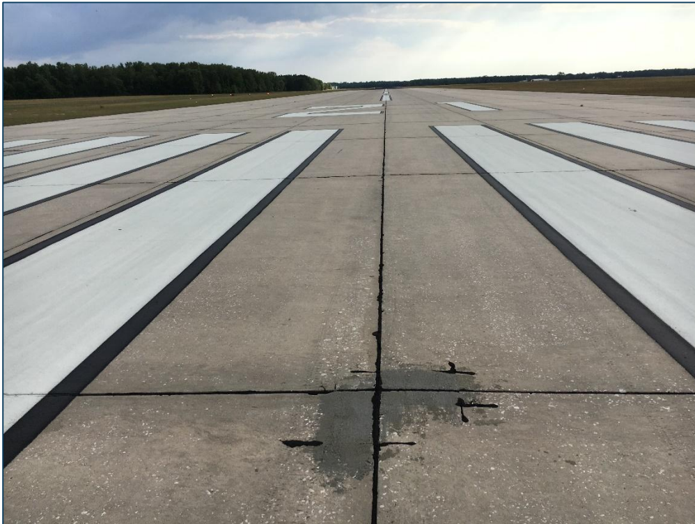
Runway 3-21, Section 6210, Sample Unit 398 – Low Severity (65) Joint Seal Damage, Low Severity (66) Small Patching
