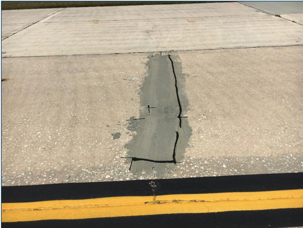
Taxiway A, Section 105, Sample Unit 191 – Low Severity (63) Longitudinal, Transverse, and Diagonal Cracking, Low Severity (65) Joint Seal Damage, Low Severity (67) Large Patching
