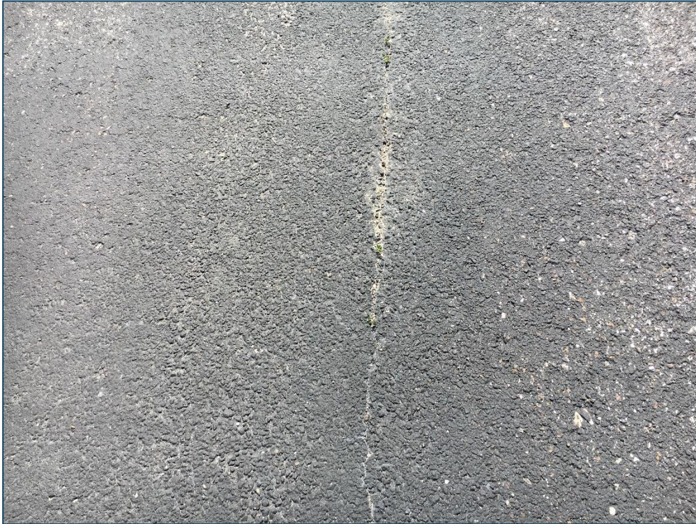
South Apron, Section 4210, Sample Unit 504 – Low Severity (48) Longitudinal and Transverse Cracking, Low Severity (52) Raveling
