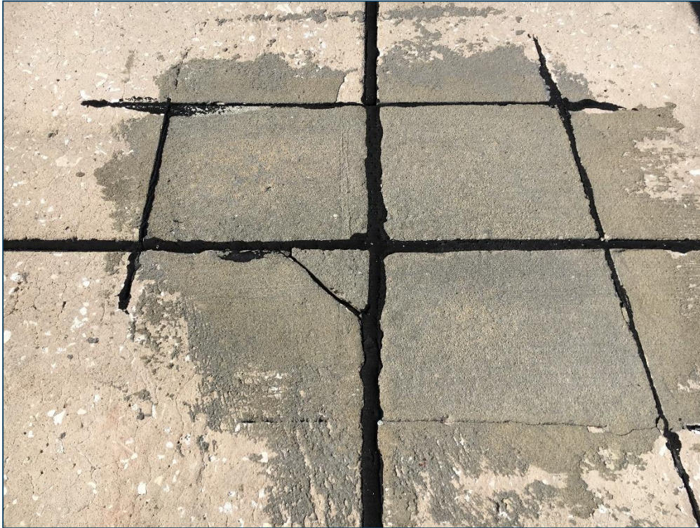
Runway 3-21, Section 6210, Sample Unit 301 – Low Severity (65) Joint Seal Damage, Medium Severity (66) Small Patching, Low Severity (74) Joint Spalling, Low Severity (75) Corner Spalling
