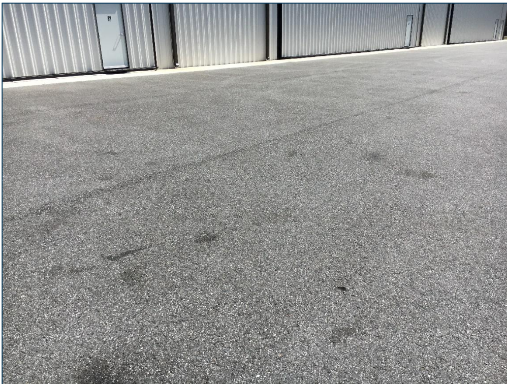
South Apron, Section 4225, Sample Unit 302 – Low Severity (57) Weathering
