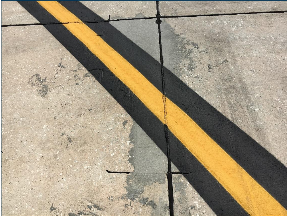
Runway 9-27, Section 6110, Sample Unit 398 – Low Severity (65) Joint Seal Damage, Low Severity (66) Small Patching, (73) Shrinkage Cracks
