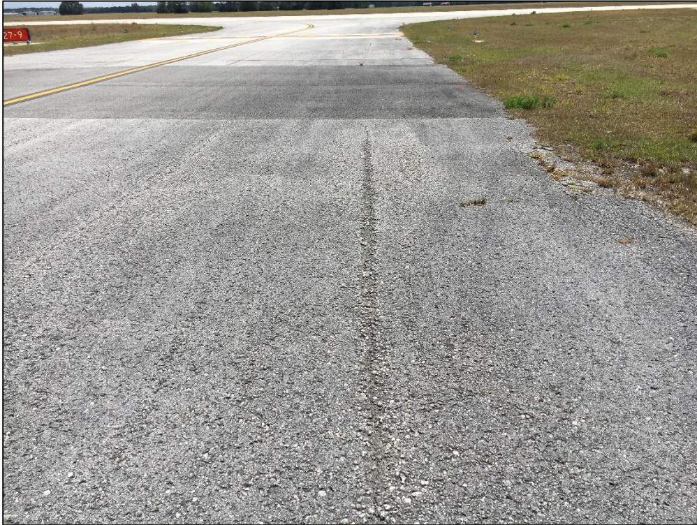
Taxiway A6, Section 135, Sample Unit 605 – Low Severity (48) Longitudinal and Transverse Cracking, Low Severity (50) Patching, Medium Severity (52) Raveling, High Severity (52) Raveling
