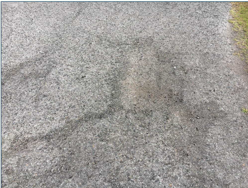
Taxiway B, Section 205, Sample Unit 148 – Medium Severity (52) Raveling, High Severity (52) Raveling
