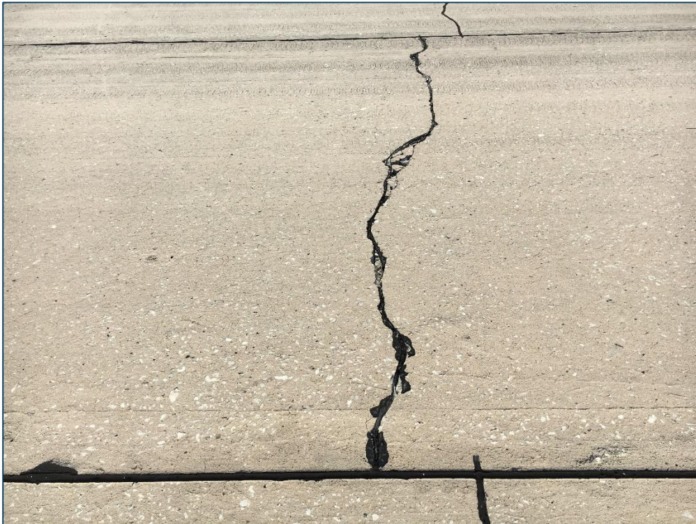
Runway 3-21, Section 6210, Sample Unit 337 – Medium Severity (63) Longitudinal, Transverse, and Diagonal Cracking, Low Severity (65) Joint Seal Damage
