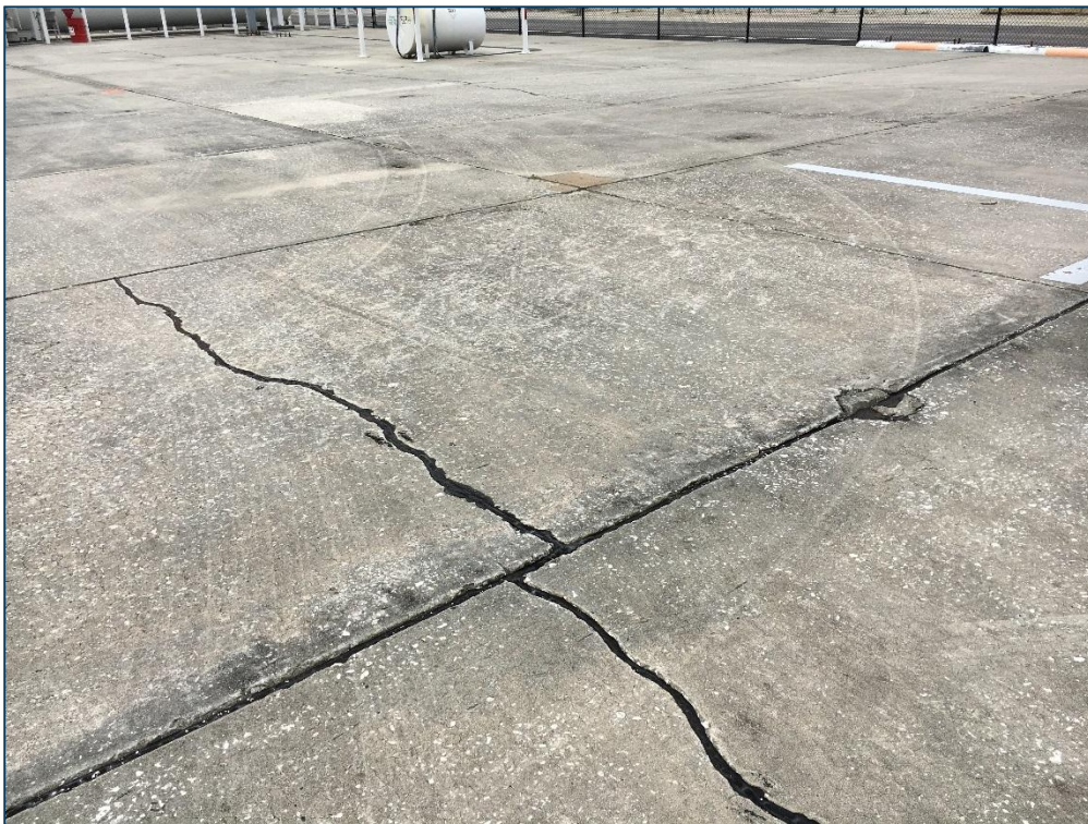
North Apron, Section 4110, Sample Unit 807 – Low Severity (63) Longitudinal, Transverse, and Diagonal Cracking, Low Severity (74) Joint Spalling, (73) Shrinkage Cracks
