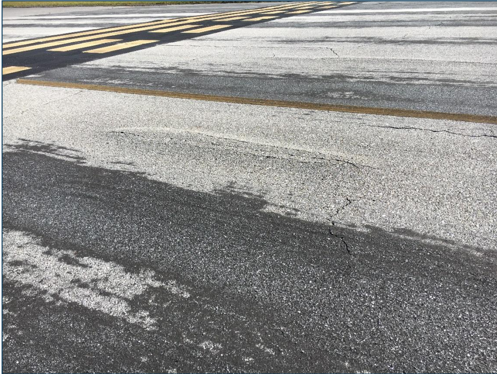
Taxiway F, Section 610, Sample Unit 103 – Low Severity (52) Raveling, Low Severity (56) Swelling
