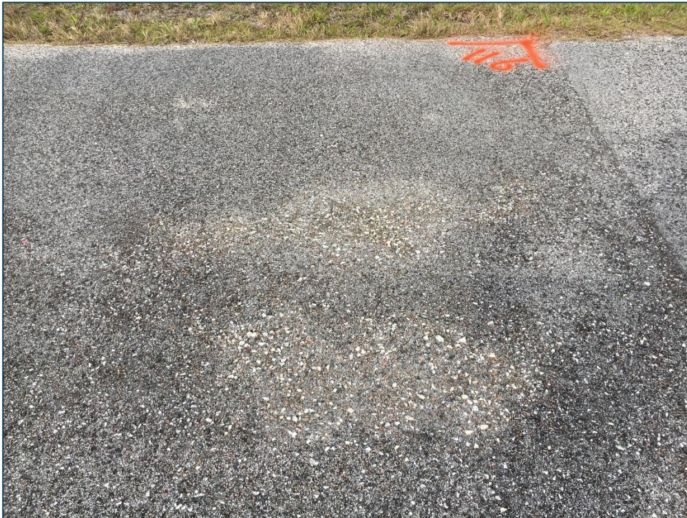
Taxiway A2, Section 114, Sample Unit 116 – Low Severity (45) Depression, Low Severity (57) Weathering
