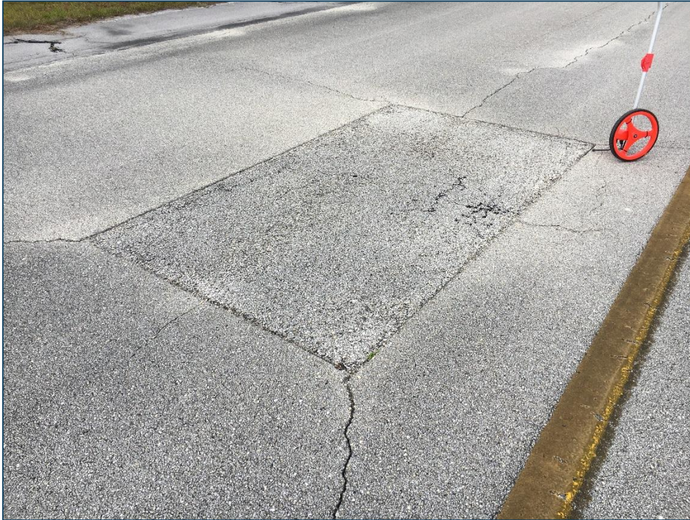
Taxiway A3, Section 115, Sample Unit 105 – Medium Severity (48) Longitudinal and Transverse Cracking, Medium Severity (50) Patching, Low Severity (52) Raveling
