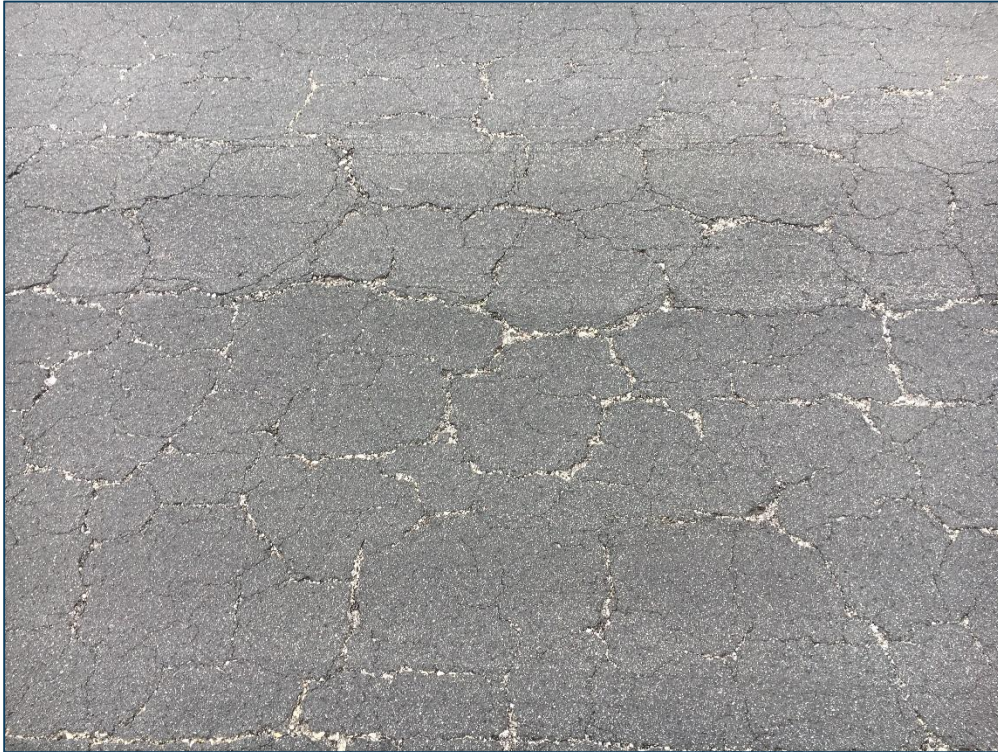
Apron FBO, Section 4405, Sample Unit 202 – Low Severity (43) Block Cracking, Low Severity (52) Raveling
