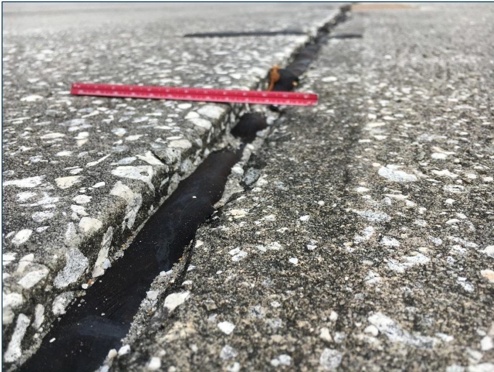
North Apron, Section 4130, Sample Unit 202 – High Severity (65) Joint Seal Damage, Medium Severity (71) Faulting
