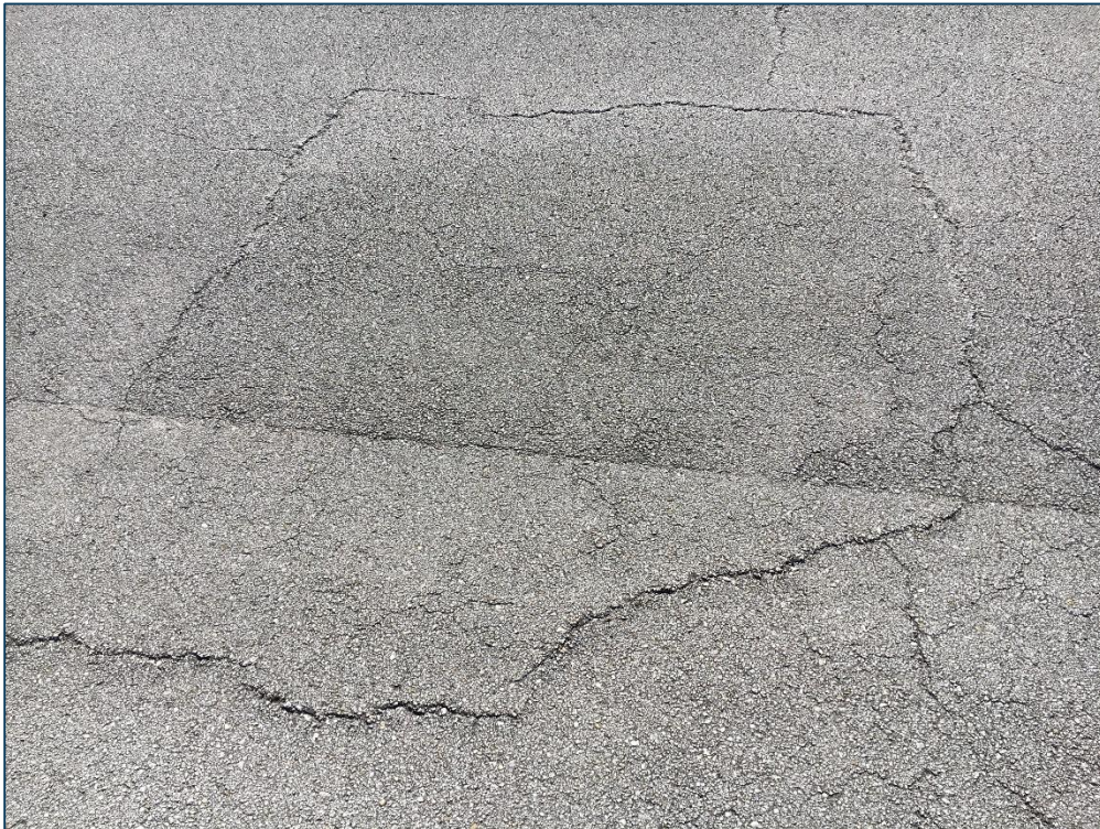
Runway 5-23, Section 6305, Sample Unit 153 – Low Severity (43) Block Cracking, Low Severity (52) Raveling
