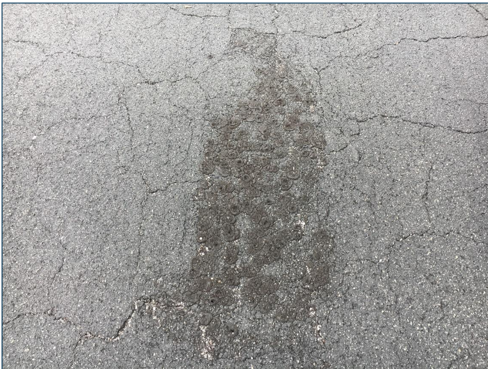
Apron FBO, Section 4405, Sample Unit 105 – (42) Bleeding, Low Severity (43) Block Cracking
