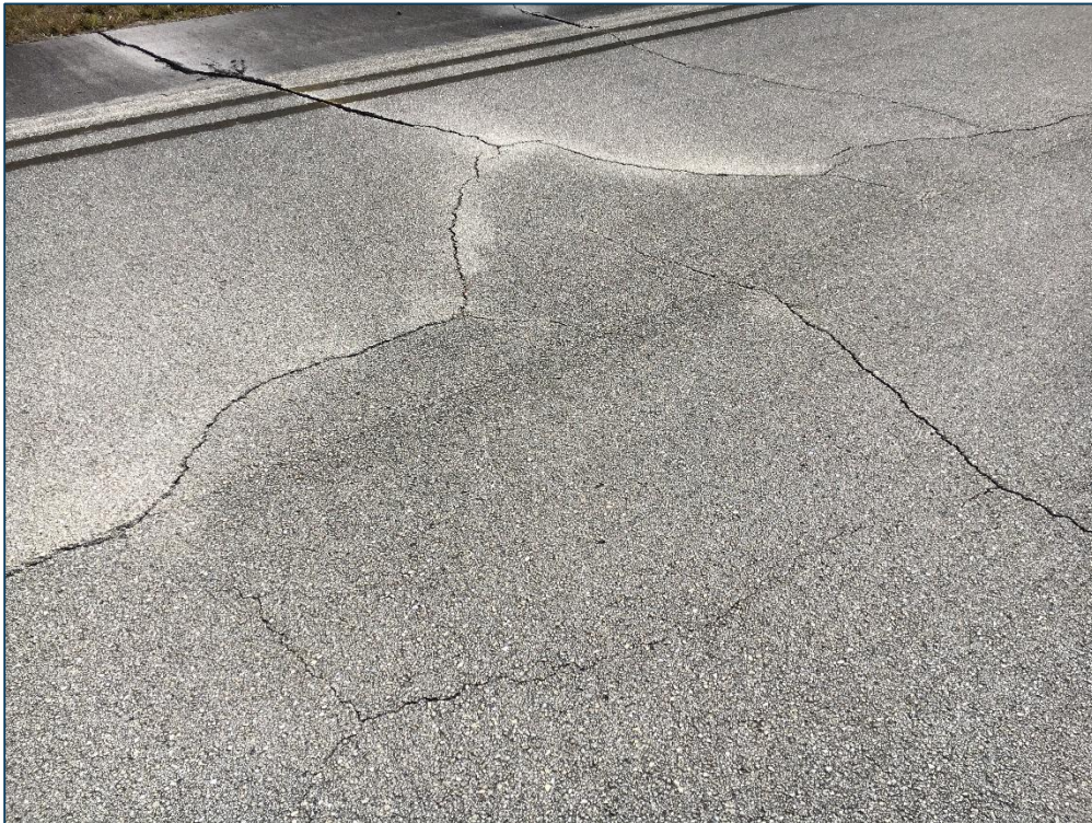
Taxiway C3, Section 315, Sample Unit 105 – Low Severity (43) Block Cracking, Low Severity (52) Raveling
