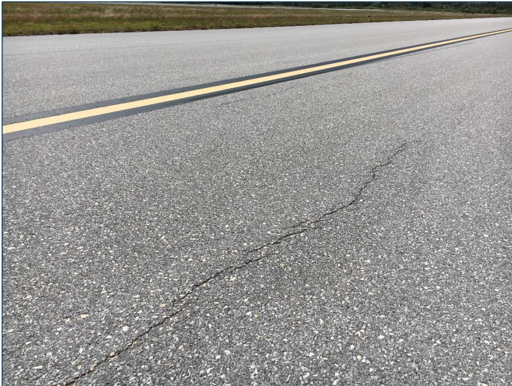
Taxiway D, Section 405, Sample Unit 108 – Low Severity (48) Longitudinal and Transverse Cracking, Low Severity (56) Swelling, Low Severity (57) Weathering
