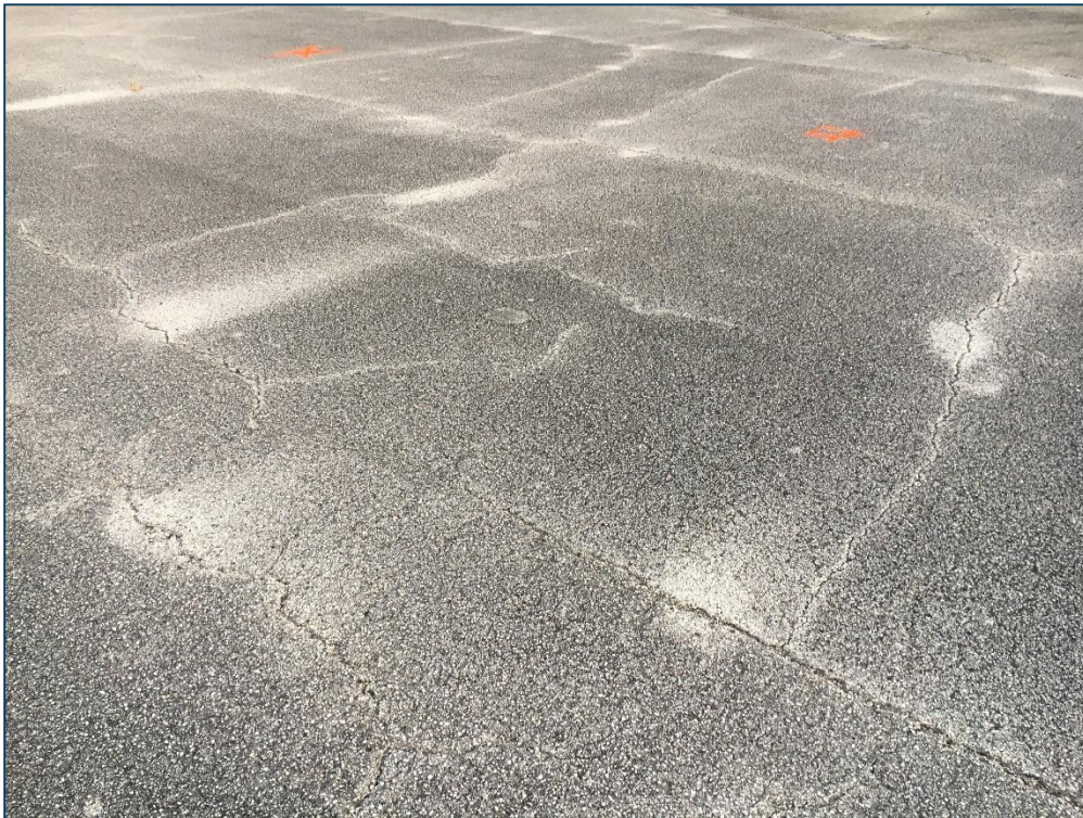
Runway RW 9R-27L, Section 6205, Sample Unit 300 – Medium Severity (43) Block Cracking, Medium Severity (52) Raveling
