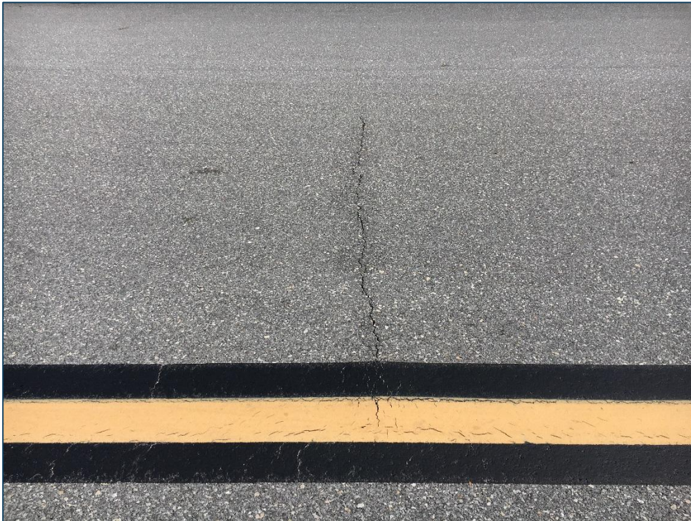
Taxiway C1, Section 305, Sample Unit 102 – Low Severity (48) Longitudinal and Transverse Cracking, Low Severity (52) Raveling, Low Severity (57) Weathering
