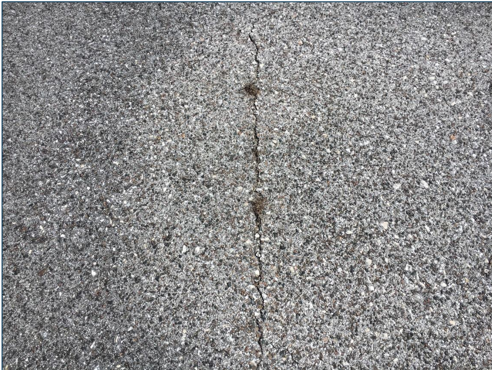
Runway 9L-27R, Section 6110, Sample Unit 504 – Low Severity (48) Longitudinal and Transverse Cracking, Low Severity (57) Weathering
