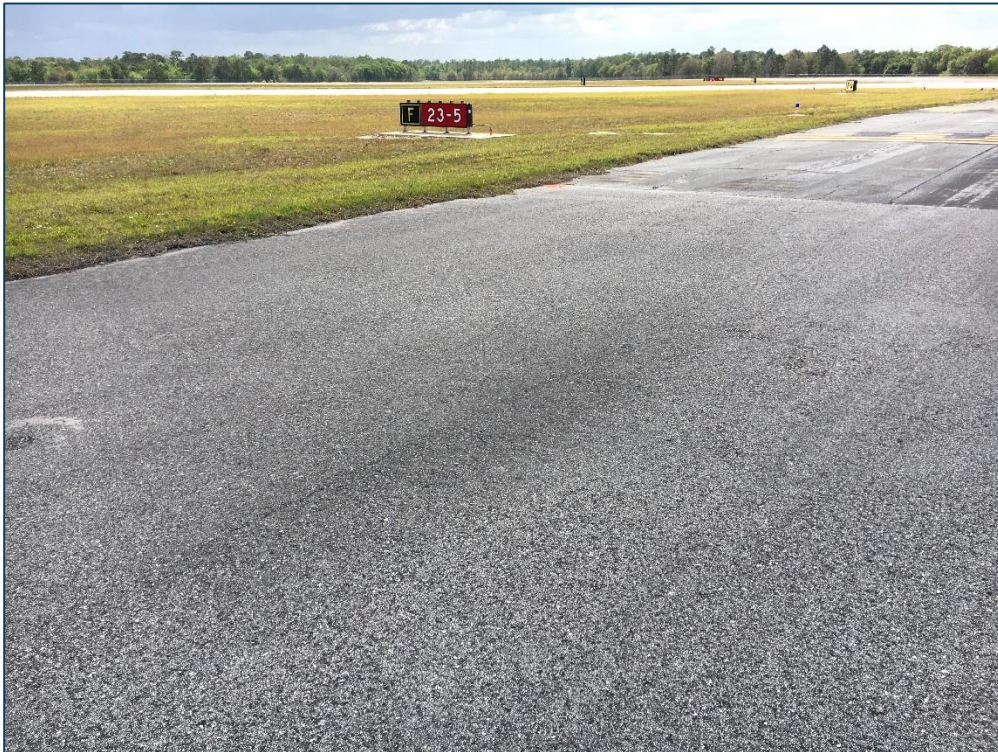
Taxiway F, Section 605, Sample Unit 101 – Low Severity (48) Longitudinal and Transverse Cracking, Low Severity (45) Depression, Medium Severity (52) Raveling, Low Severity (57) Weathering
