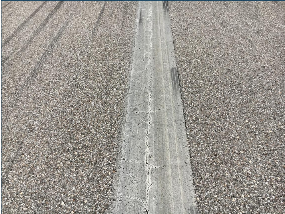
Runway RW 9L-27R, Section 6115, Sample Unit 378 – Low Severity (48) Longitudinal and Transverse Cracking, Low Severity (57) Weathering
