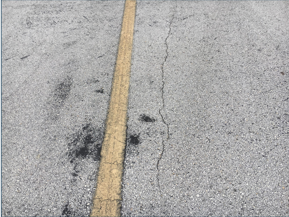
T-Hangar Taxilane, Section 4205, Sample Unit 207 – Low Severity (48) Longitudinal and Transverse Cracking, Medium Severity (52) Raveling
