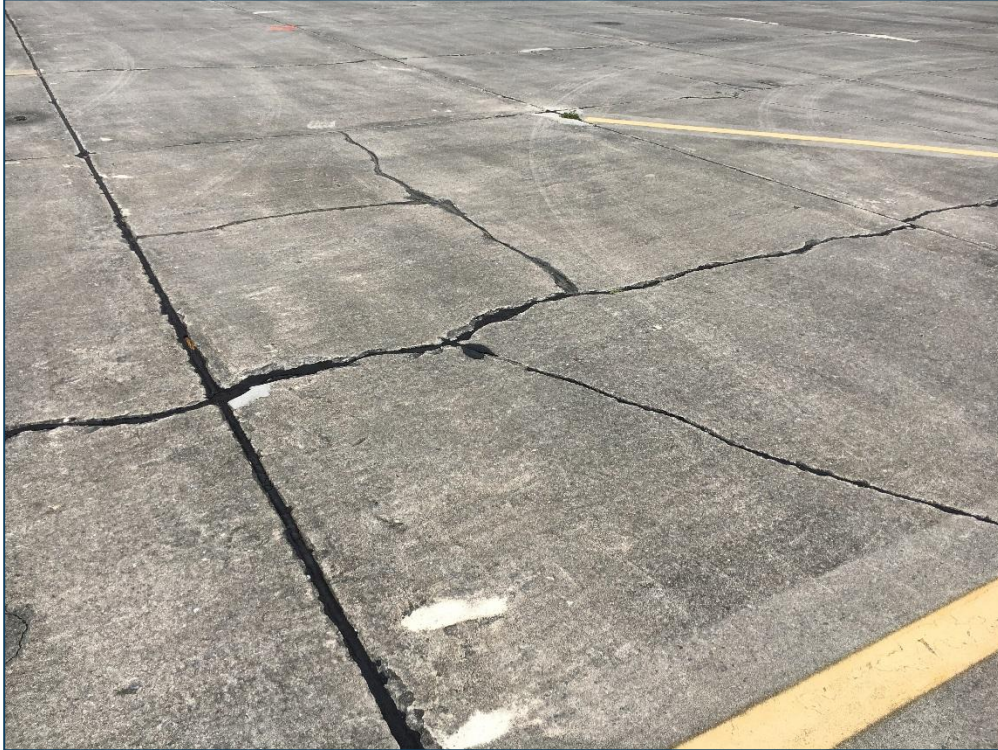
North Apron, Section 4110, Sample Unit 405 – Low Severity (63) Longitudinal, Transverse, and Diagonal Cracking, Low Severity (65) Joint Seal Damage, Low Severity (72) Shattered Slab
