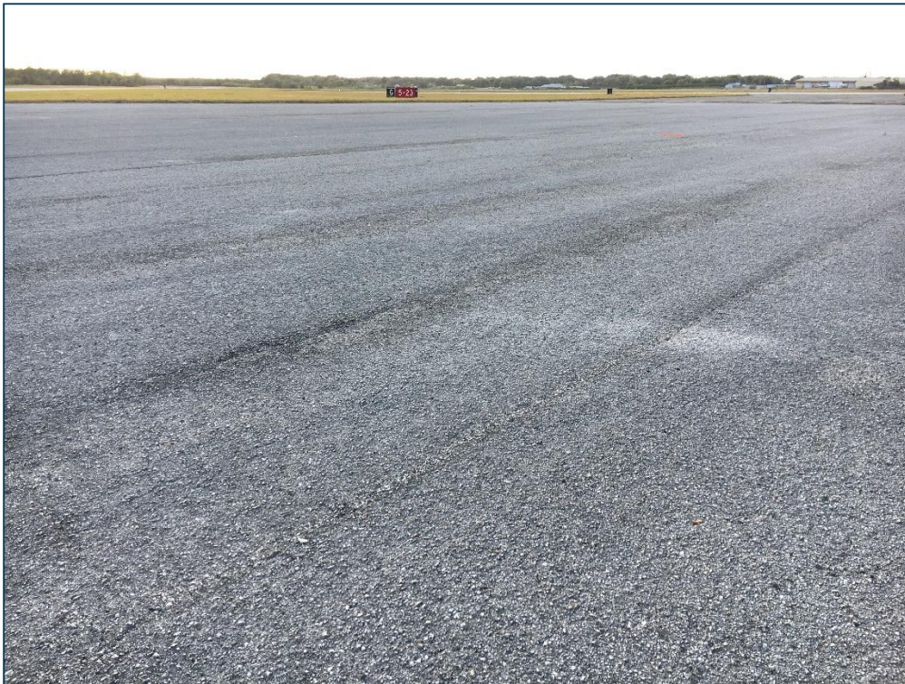
Taxiway G, Section 710, Sample Unit 106 – Low Severity (45) Depression, Low Severity (48) Longitudinal and Transverse Cracking, Medium Severity (52) Raveling, High Severity (52) Raveling
