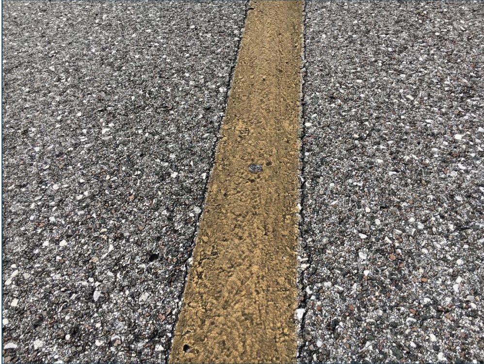
Taxiway D, Section 420, Sample Unit 204 – Low Severity (48) Longitudinal and Transverse Cracking, Low Severity (52) Raveling, Medium Severity (52) Raveling
