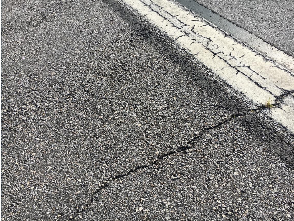
Taxiway H, Section 802, Sample Unit 100 – Low Severity (48) Longitudinal and Transverse Cracking, Low Severity (52) Raveling, Low Severity (57) Weathering
