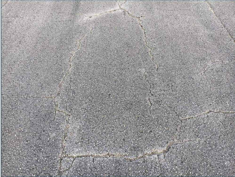
Runway RW 9R-27L, Section 6205, Sample Unit 361 – Medium Severity (43) Block Cracking, Medium Severity (52) Raveling
