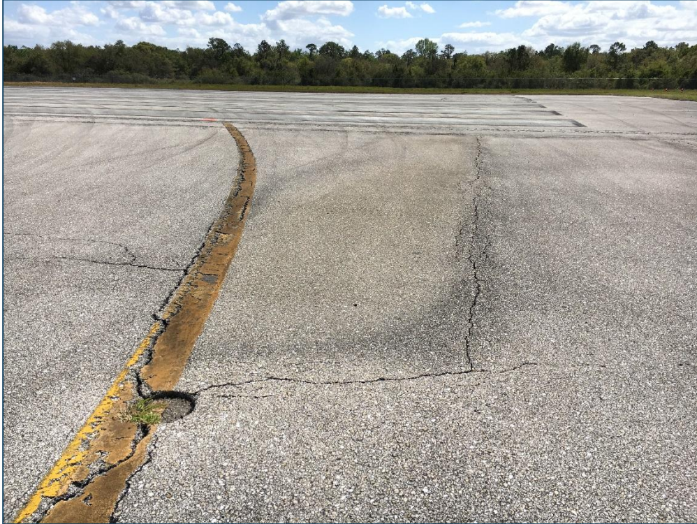
Taxiway C3, Section 320, Sample Unit 112 – Low Severity (45) Depression, Low Severity (48) Longitudinal and Transverse Cracking, Low Severity (52) Raveling, Low Severity (56) Swelling
