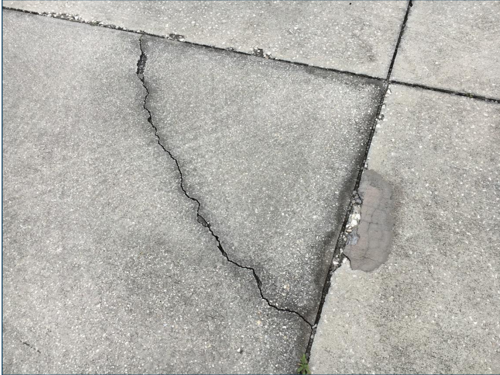
T-Hangar Apron, Section 4210, Sample Unit 306 – Low Severity (62) Corner Break, Medium Severity (74) Joint Spalling, High Severity (65) Joint Seal Damage
