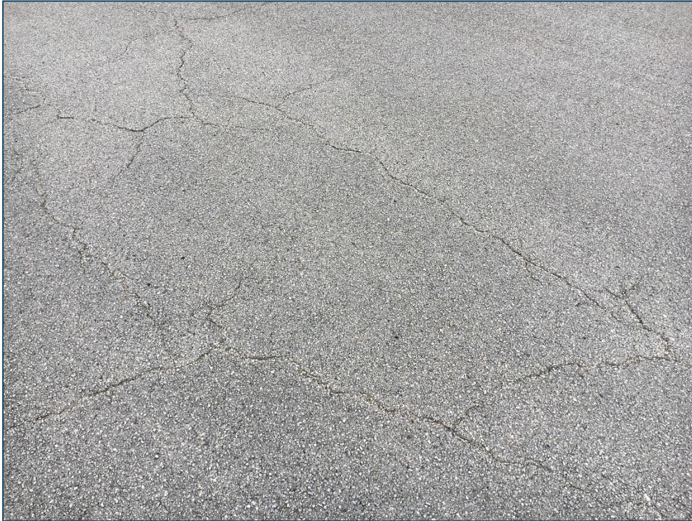
Hold Apron on Taxiway A, Section 5105, Sample Unit 102 – Medium Severity (43) Block Cracking, Medium Severity (52) Raveling
