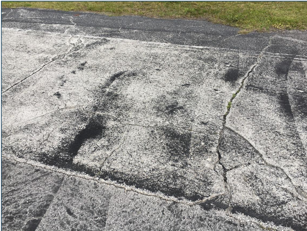
T-Hangar Taxilane, Section 4205, Sample Unit 102 – Medium Severity (43) Block Cracking, Low Severity (52) Raveling, Low Severity (52) Raveling
