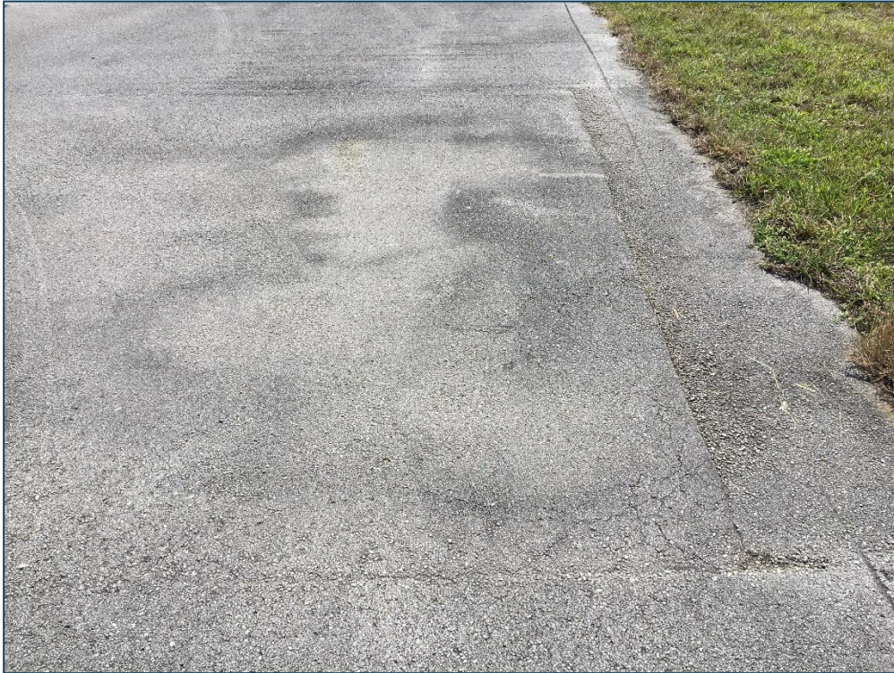
Runway 5-23, Section 6305, Sample Unit 100 – Low Severity (45) Depression, Low Severity (48) Longitudinal and Transverse Cracking, Low Severity (52) Raveling, Medium Severity (52) Raveling
