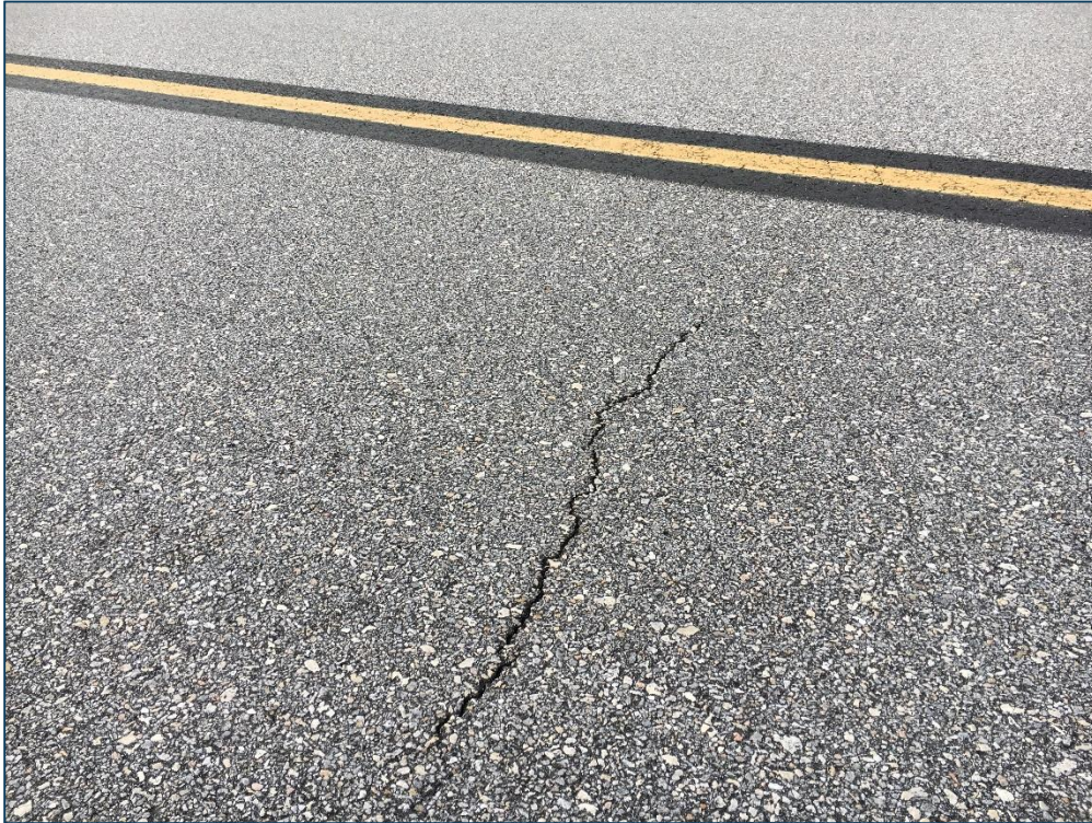
Taxiway A1, Section 105, Sample Unit 102 – Low Severity (48) Longitudinal and Transverse Cracking, Low Severity (57) Weathering
