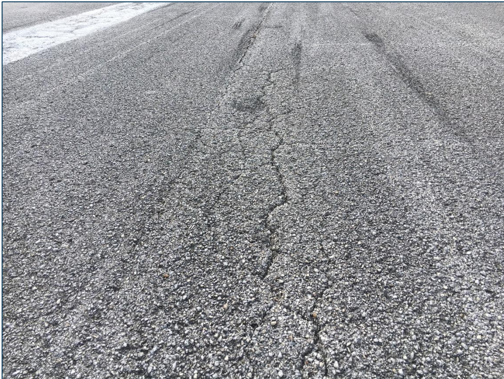
Runway RW 9R-27L, Section 6205, Sample Unit 375 – Low Severity (41) Alligator Cracking, Medium Severity (52) Raveling
