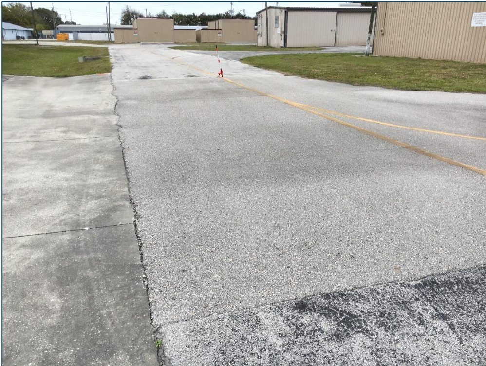
T-Hangar Taxilane, Section 4205, Sample Unit 207 – Medium Severity (50) Patching, Low Severity (52) Raveling
