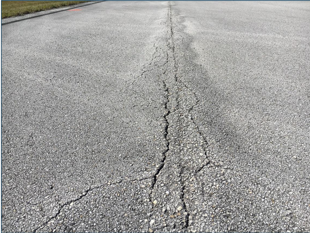
Runway 5-23, Section 6315, Sample Unit 125 – Medium Severity (48) Longitudinal and Transverse Cracking, Low Severity (56) Swelling, Low Severity (52) Raveling, Medium Severity (52) Raveling
