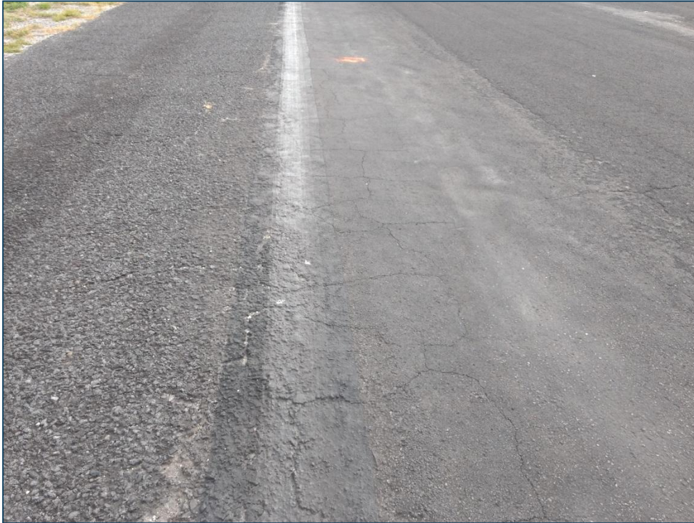
Taxiway A, Section 105, Sample Unit 100 - Medium Severity (43) Block Cracking, Medium Severity (52) Raveling
