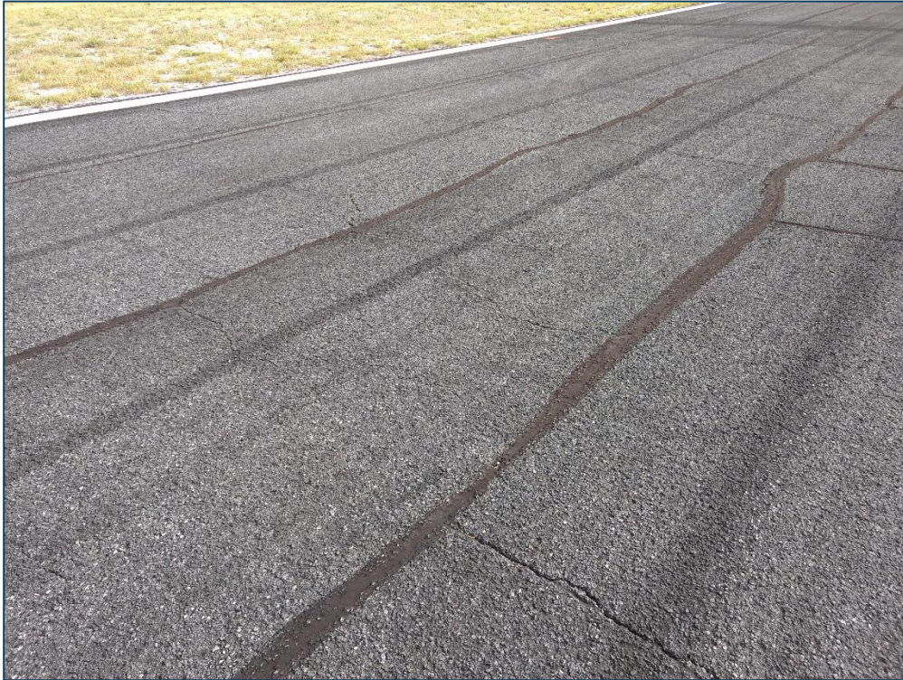
Runway 5-23, Section 6105, Sample Unit 115 - Low Severity (43) Block Cracking, Medium Severity (52) Raveling
