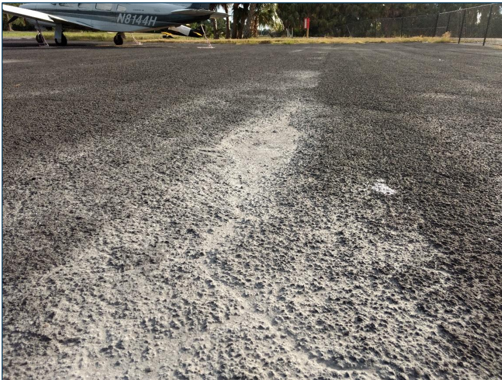
Apron, Section 4105, Sample Unit 100 - Low Severity (43) Block Cracking, Low Severity (45) Depression, Medium Severity (52) Raveling
