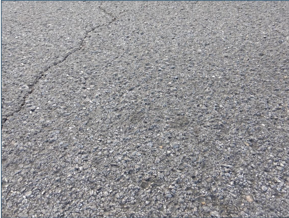
Runway 5-23, Section 6105, Sample Unit 143 - Low Severity (43) Block Cracking, Medium Severity (52) Raveling
