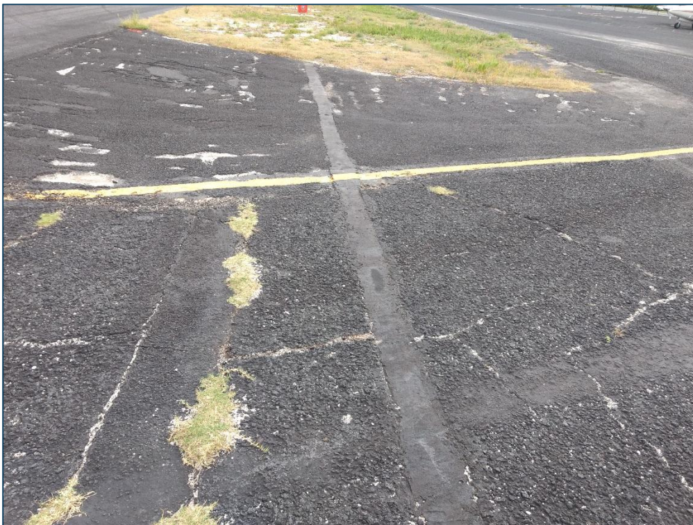
Taxiway A, Section 105, Sample Unit 100 - Medium Severity (43) Block Cracking, Low Severity (50) Patching, Medium Severity (50) Patching, Medium Severity (52) Raveling, High Severity (52) Raveling
