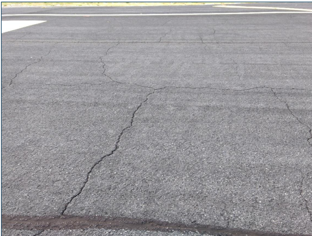
Runway 5-23, Section 6105, Sample Unit 135 - Low Severity (43) Block Cracking, Medium Severity (43) Block Cracking, Medium Severity (52) Raveling
