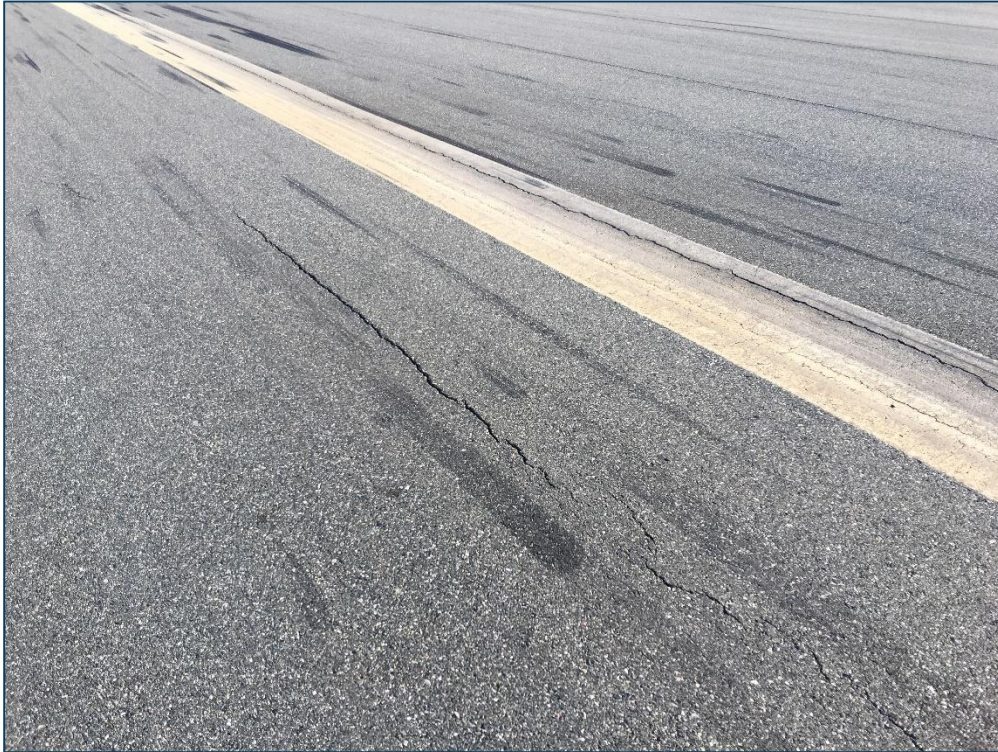
Runway 17-35, Section 6105, Sample Unit 306 – Low and Medium Severity (48) Longitudinal and Transverse Cracking, Low Severity (57) Weathering
