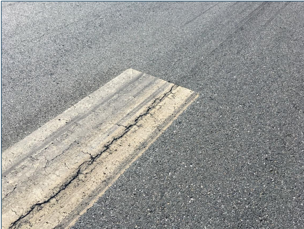
Runway 17-35, Section 6115, Sample Unit 346 – Low Severity (48) Longitudinal and Transverse Cracking, Low Severity (57) Weathering, Medium Severity (57) Weathering
