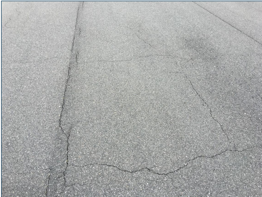
Runway 17-35, Section 6125, Sample Unit 452 – Low Severity (43) Block Cracking, Low Severity (48) Longitudinal and Transverse Cracking, Low Severity (57) Weathering
