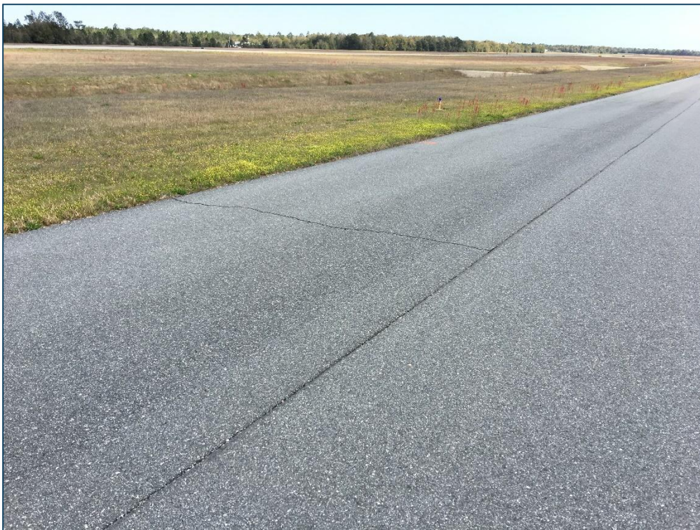
Taxiway A, Section 110, Sample Unit 193 – Low Severity (48) Longitudinal and Transverse Cracking, Low Severity (57) Weathering
