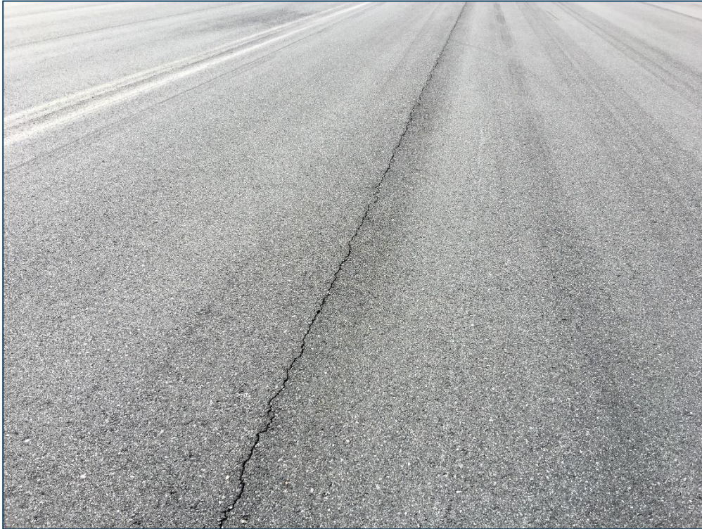
Runway 17-35, Section 6115, Sample Unit 394 – Low Severity (48) Longitudinal and Transverse Cracking, Low Severity (57) Weathering
