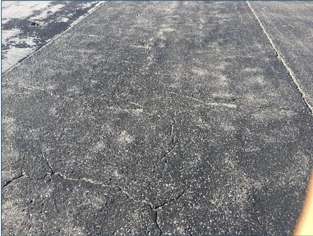
Apron, Section 4115, Sample Unit 210 – Low Severity (43) Block Cracking, Low and Medium Severity (48) Longitudinal and Transverse Cracking, Low Severity (52) Raveling Medium Severity (52) Raveling
