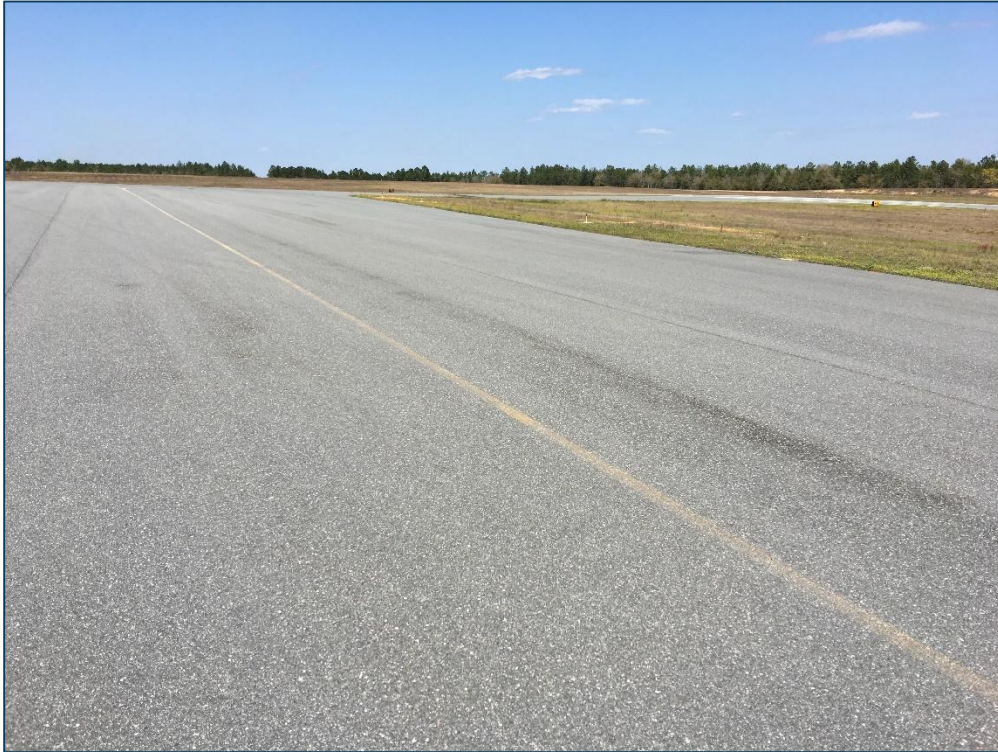
Taxiway A, Section 125, Sample Unit 255 – Low Severity (48) Longitudinal and Transverse Cracking, Low Severity (52) Raveling Low Severity (57) Weathering
