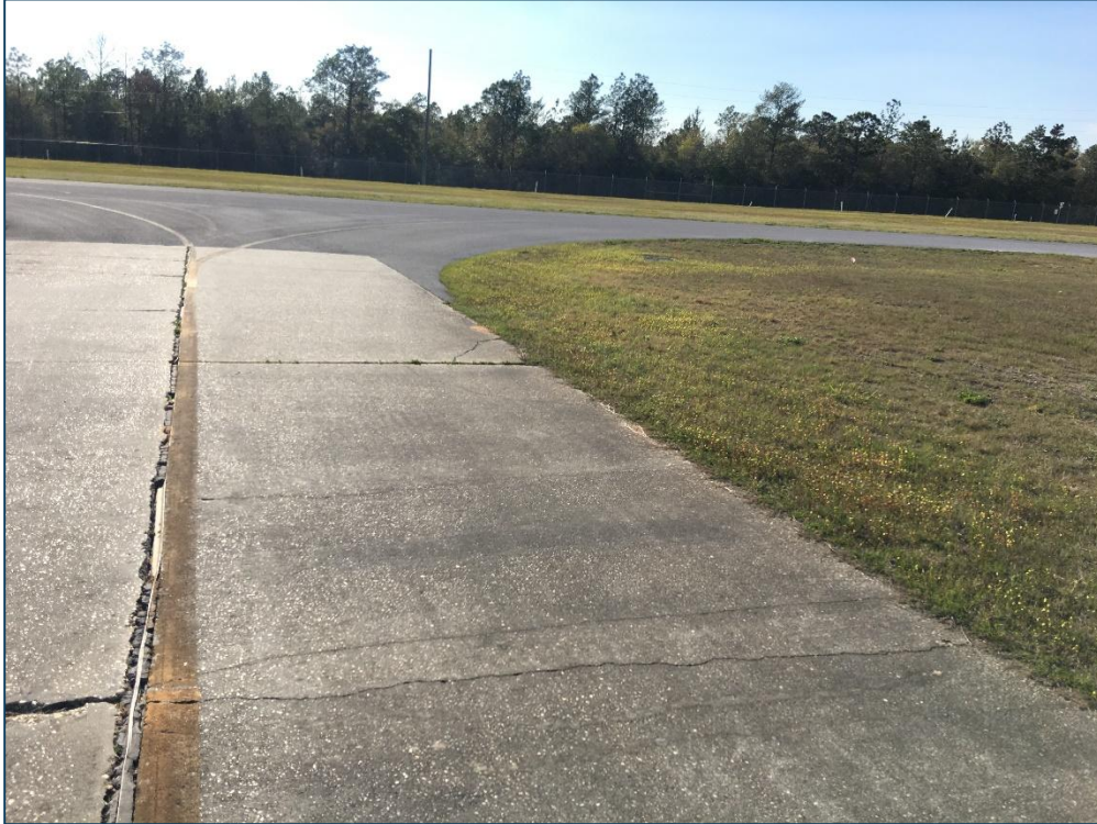
Hangar Apron, Section 4215, Sample Unit 302 – Medium Severity (62) Corner Break, Low Severity (63) Longitudinal, Transverse, and Diagonal Cracking, High Severity (65) Joint Seal Damage,
