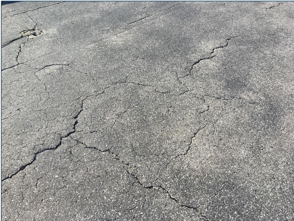
Apron, Section 4110, Sample Unit 306 – Low Severity (43) Block Cracking, Medium Severity (43) Block Cracking, Low Severity (52) Raveling
