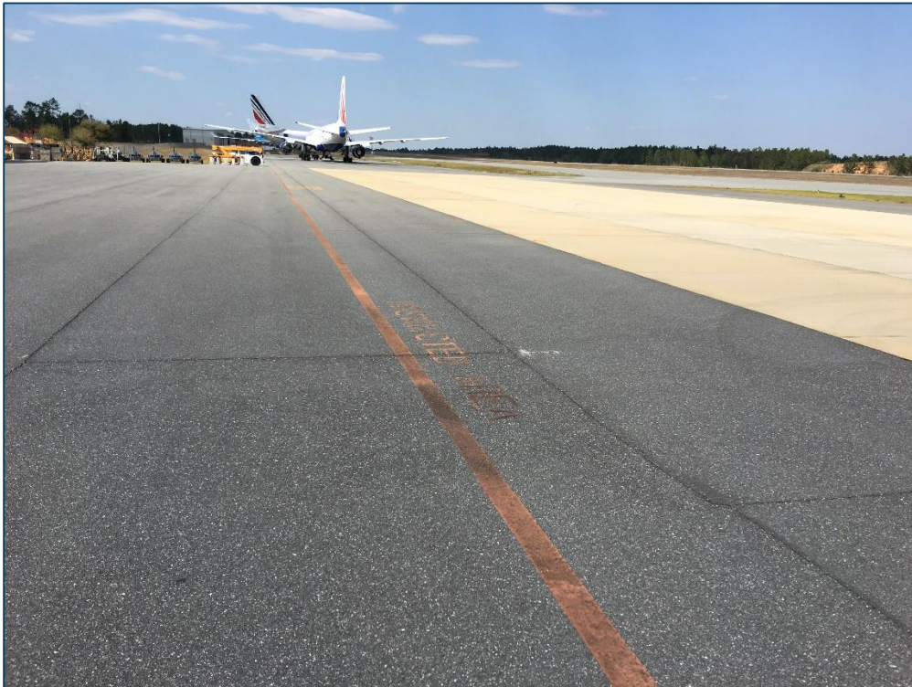
Apron, Section 4120, Sample Unit 317 – Low Severity (48) Longitudinal and Transverse Cracking, Low Severity (57) Weathering
