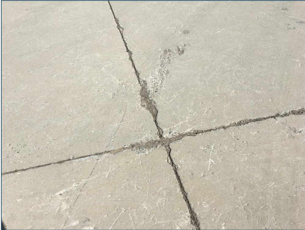
North Apron, Section 4350, Sample Unit 260 – High Severity (65) Joint Seal Damage, Low Severity (74) Joint Spalling
