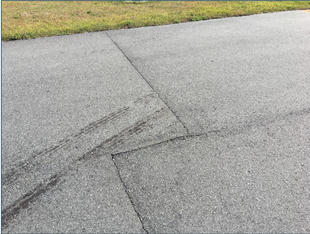
Taxiway A, Section 105, Sample Unit 103 – Low Severity (48) Longitudinal and Transverse Cracking, Low Severity (57) Weathering
