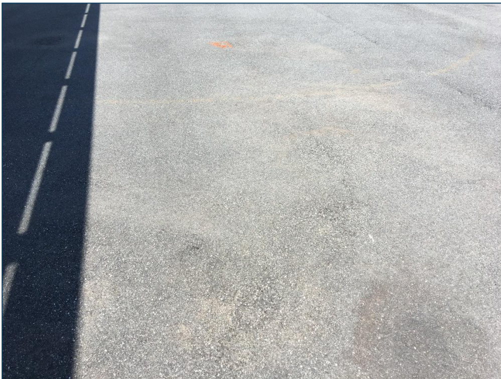
North Apron, Section 4355, Sample Unit 263 – Low Severity (48) Longitudinal and Transverse Cracking, Low Severity (52) Raveling Low Severity (57) Weathering
