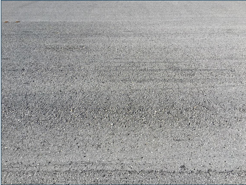
Runway 9-27, Section 6110, Sample Unit 171 – Low Severity (48) Longitudinal and Transverse Cracking, Low Severity (52) Raveling, Medium Severity (52) Raveling
