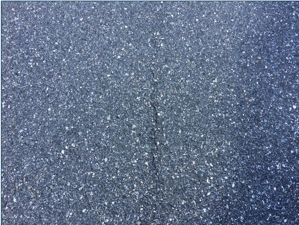
Taxiway A, Section 105, Sample Unit 107 – Low Severity (48) Longitudinal and Transverse Cracking, Low Severity (57) Weathering
