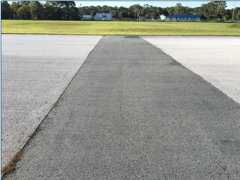
Runway 9-27, Section 6105, Sample Unit 146 – Low Severity (50) Patching, Low Severity (52) Raveling, Low Severity (57) Weathering
