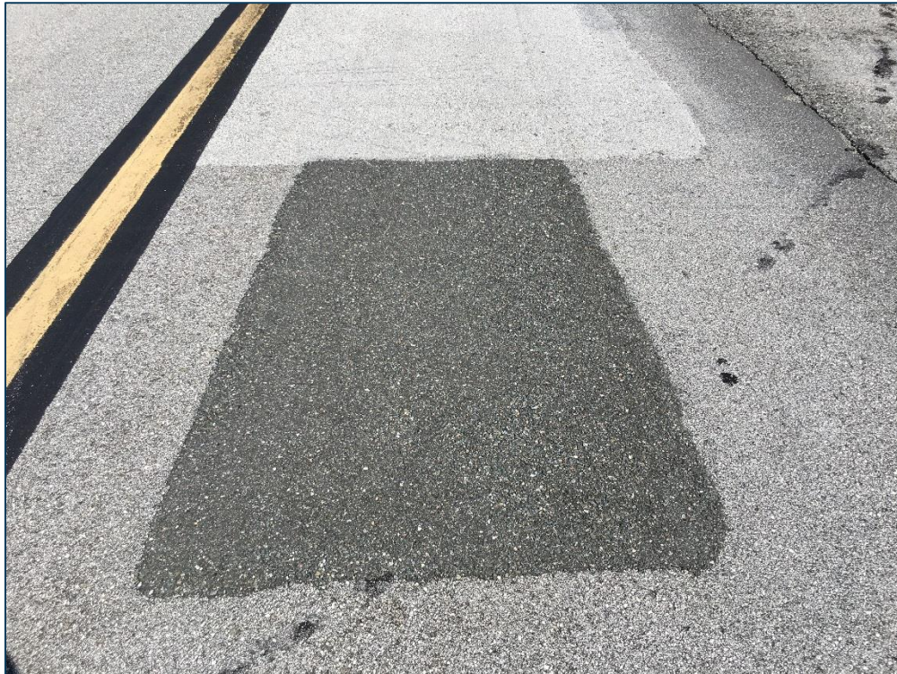
Connector Taxiway, Section 205, Sample Unit 101 – Low Severity (48) Longitudinal and Transverse Cracking, Low Severity (50) Patching, Low Severity (57) Weathering
