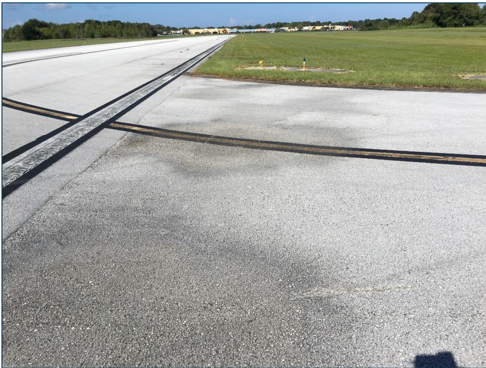
Taxiway A1, Section 115, Sample Unit 100 – Low Severity (45) Depression , Medium Severity (45) Depression, Low Severity (48) Longitudinal and Transverse Cracking, Low Severity (52) Raveling, Medium Severity (52) Raveling
