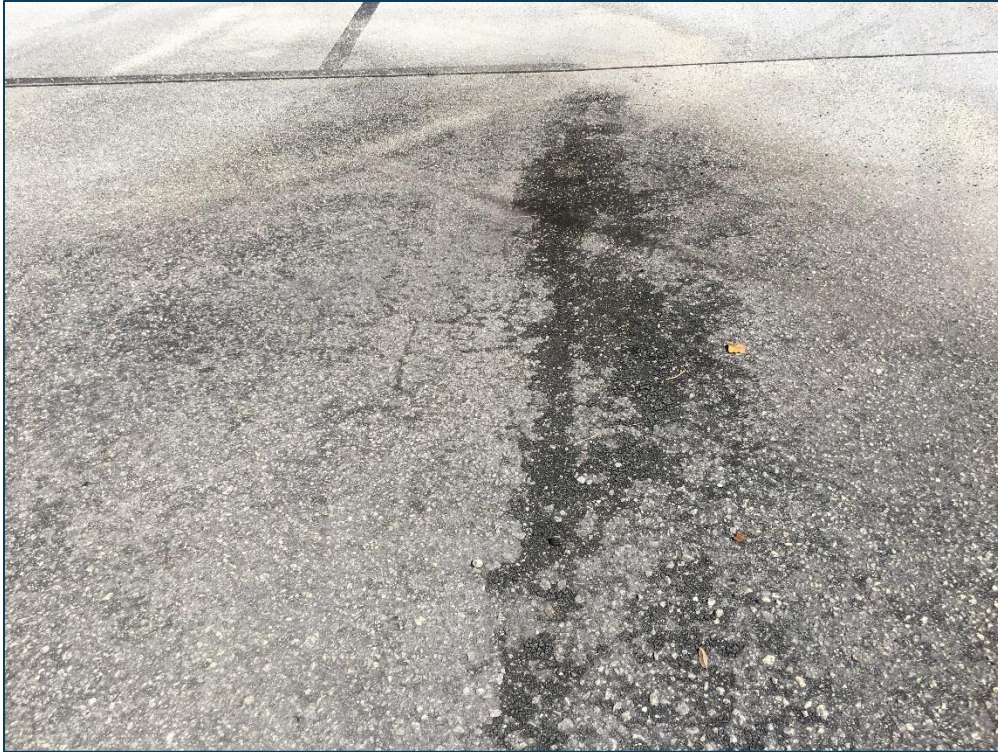
Main Apron, Section 4105, Sample Unit 198 – Low Severity (45) Depression, (49) Oil Spillage, Low Severity (52) Raveling, Medium Severity (52) Raveling
