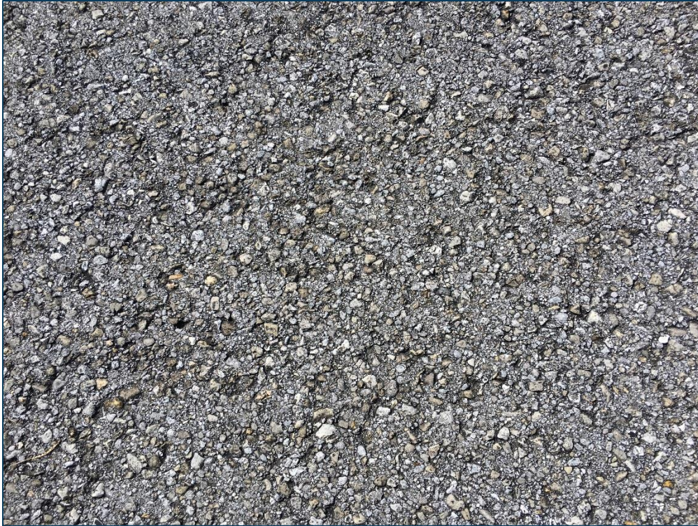
Connector Taxiway, Section 210, Sample Unit 101 – Low Severity (52) Raveling, Medium Severity (52) Raveling
