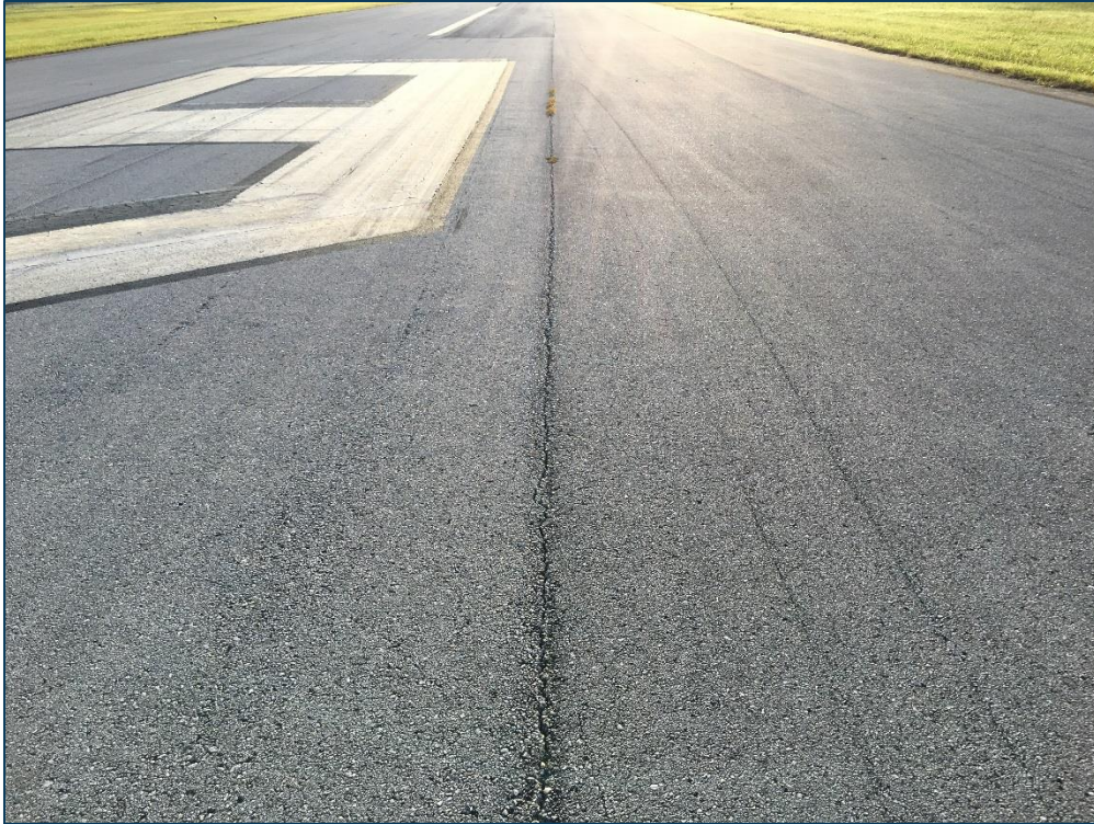
Runway 9-27, Section 6105, Sample Unit 101 – Low Severity (48) Longitudinal and Transverse Cracking, Low Severity (52) Raveling, Low Severity (57) Weathering
