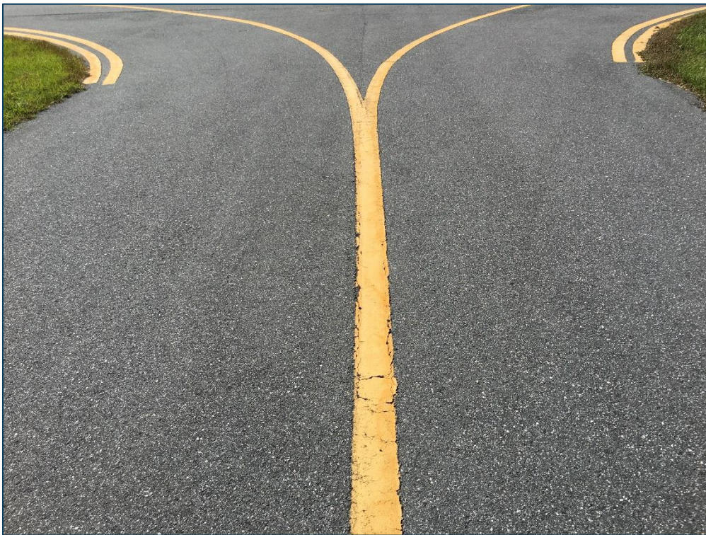
Taxiway to Hangar, Section 215, Sample Unit 100 – Low Severity (48) Longitudinal and Transverse Cracking, Low Severity (57) Weathering
