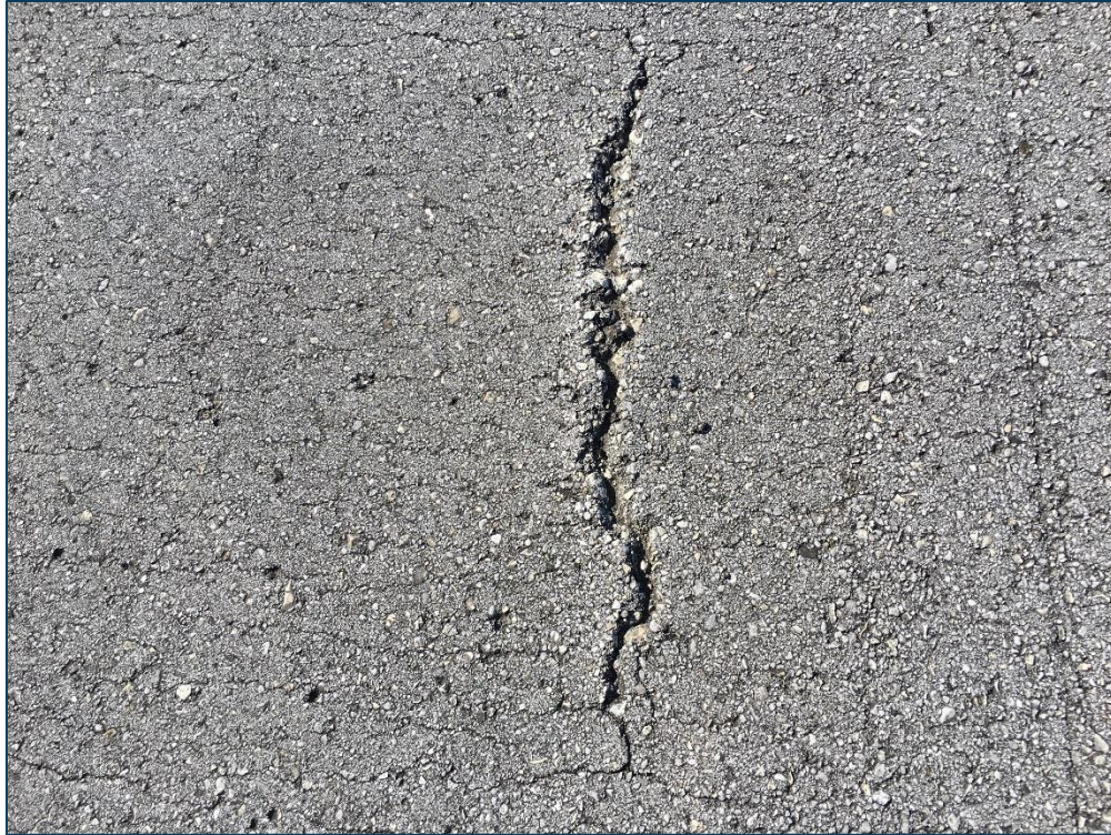
Taxiway A2, Section 118, Sample Unit 100 – Medium Severity (48) Longitudinal and Transverse Cracking, Low Severity (52) Raveling, Medium Severity (52) Raveling
