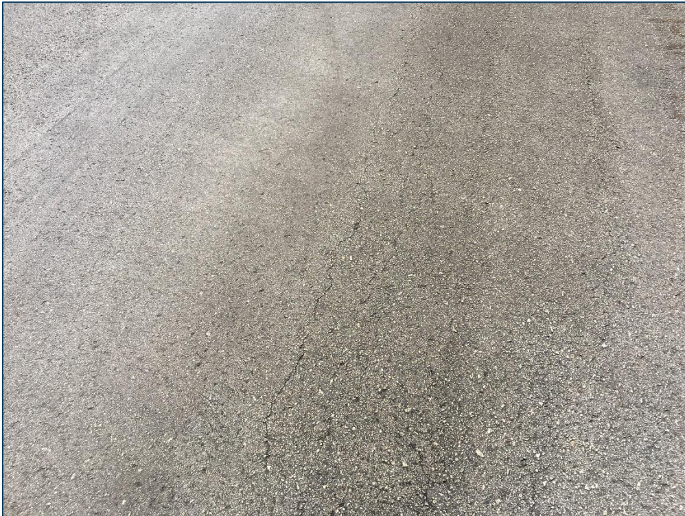
Main Apron, Section 4120, Sample Unit 221 – Low Severity (48) Longitudinal and Transverse Cracking, Low Severity (52) Raveling, Low Severity (57) Weathering
