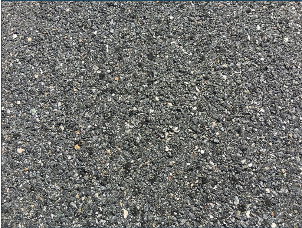
Taxiway A, Section 105, Sample Unit 127 – (42) Bleeding, Low Severity (57) Weathering
