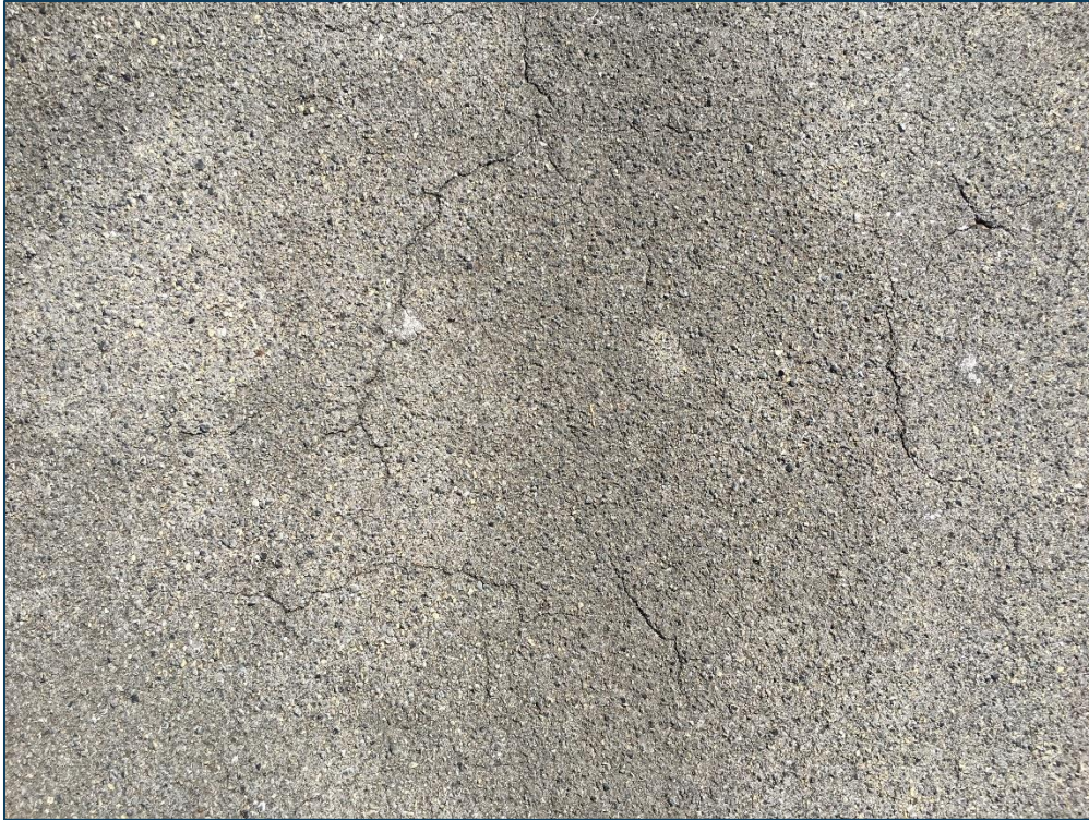
Main Apron, Section 4120, Sample Unit 202 – Low Severity (48) Longitudinal and Transverse Cracking, Low Severity (52) Raveling
