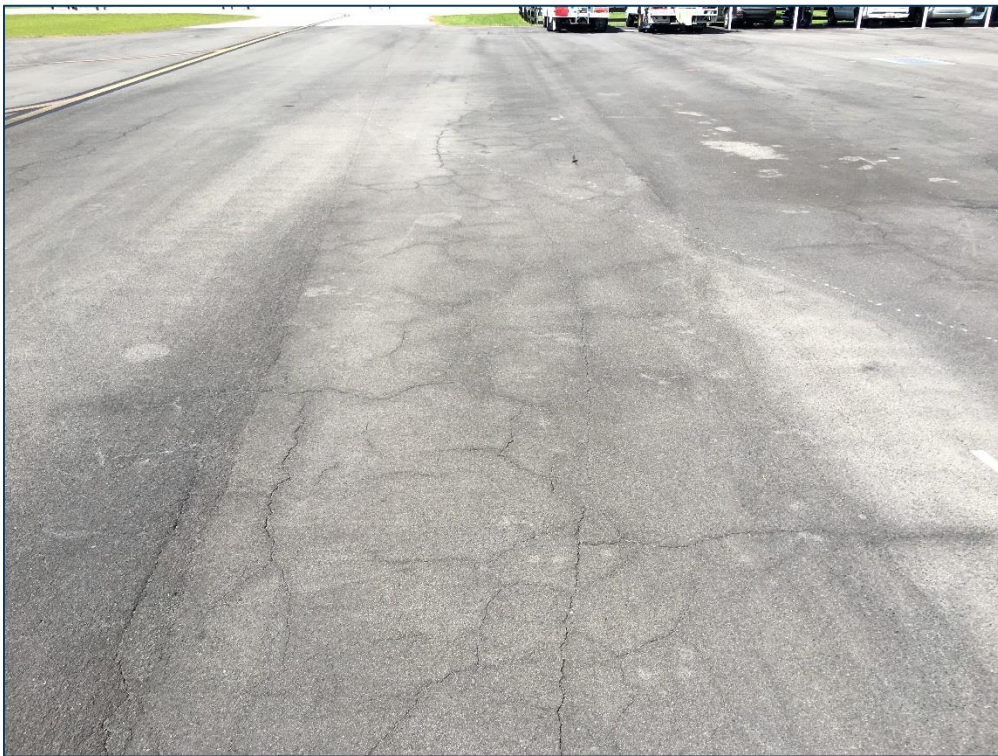
T-Hangar Apron, Section 4205, Sample Unit 412 – Low Severity (43) Block Cracking, Low Severity (52) Raveling
