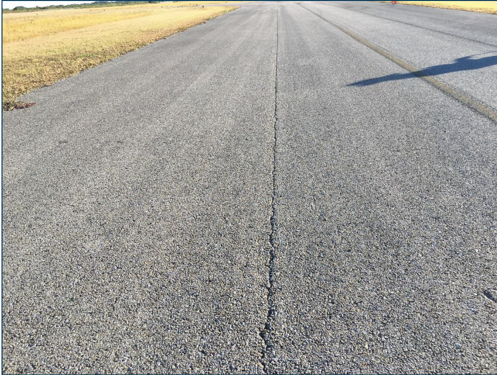
Parallel Taxiway, Section 125, Sample Unit 101 - Low Severity (48) Longitudinal and Transverse Cracking, Medium Severity (48) Longitudinal and Transverse Cracking, Low Severity (52) Raveling, Medium Severity (52) Raveling
