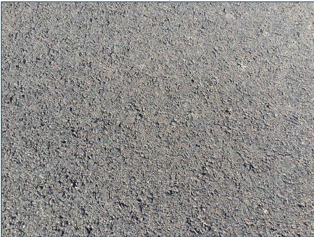
Taxilane to North Hangars, Section 245, Sample Unit 601 - Low Severity (57) Weathering
