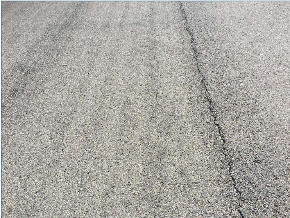
Parallel Taxiway, Section 115, Sample Unit 111 – Low and Medium Severity (48) Longitudinal and Transverse Cracking, Low Severity (52) Raveling, Low Severity (56) Swelling
