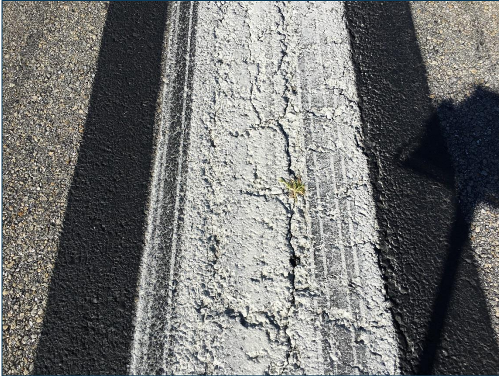
Runway 18-36, Section 6105, Sample Unit 111 – Low Severity (48) Longitudinal and Transverse Cracking, Low Severity (52) Raveling, Low Severity (57) Weathering
