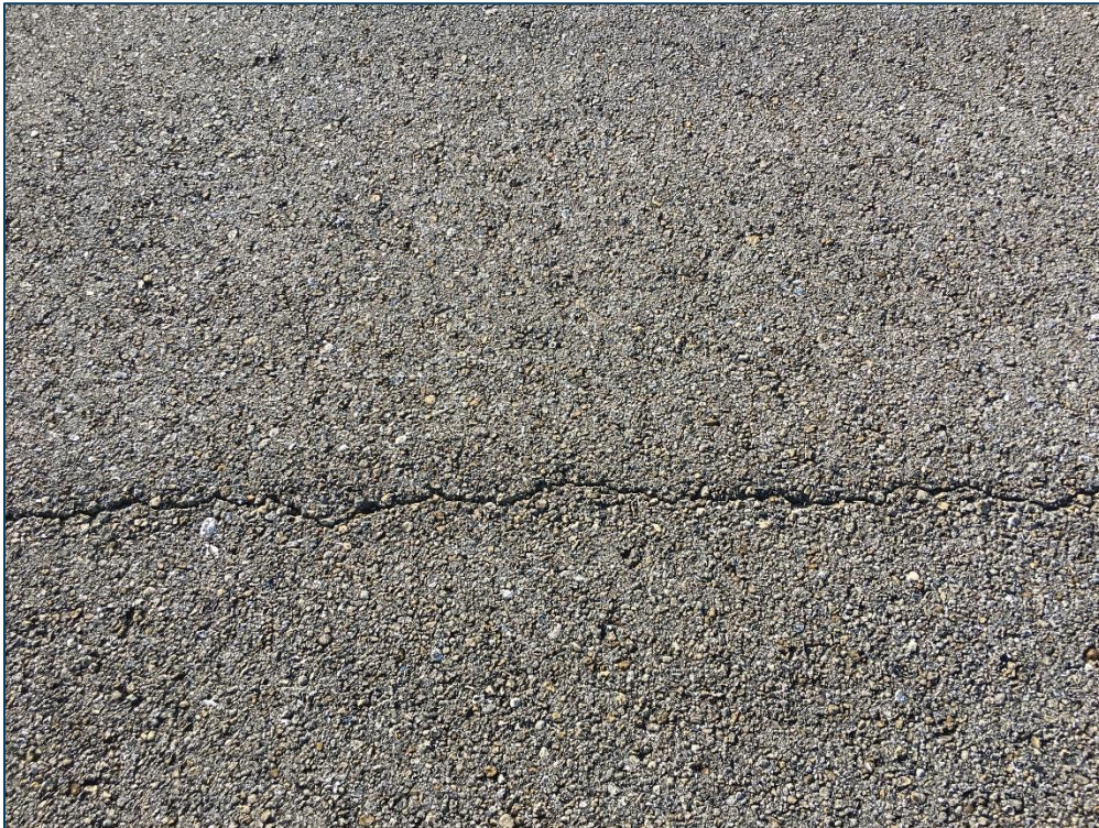
Runway 18-36, Section 6105, Sample Unit 171 – Low Severity (48) Longitudinal and Transverse Cracking, Low Severity (57) Weathering
