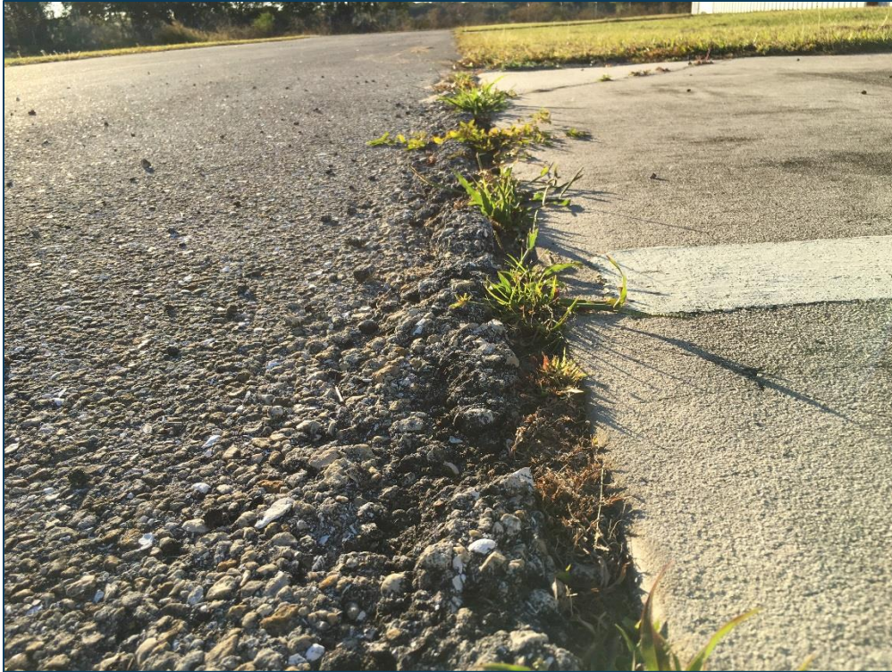
Taxilane To West Hangars, Section 210, Sample Unit 102 - Low Severity (52) Raveling, Low Severity (54) Shoving
