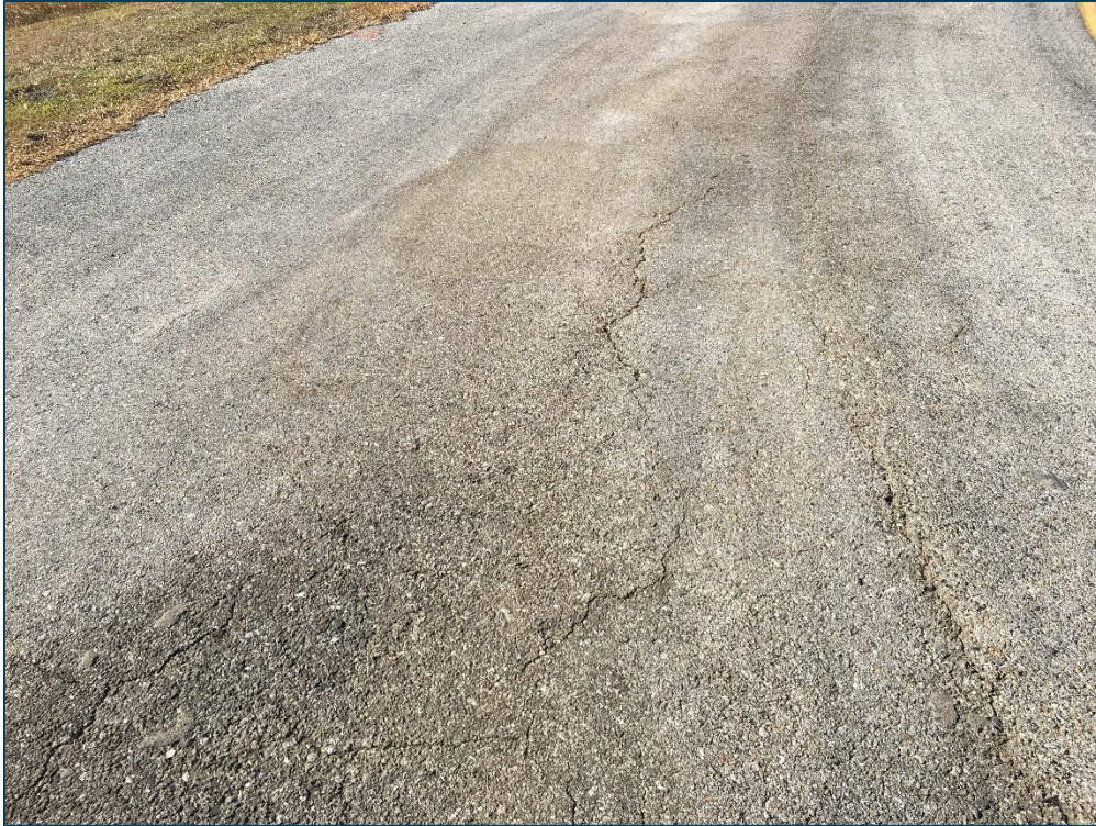
Parallel Taxiway, Section 105, Sample Unit 101 – Low Severity (45) Depression, Low and Medium Severity (48) Longitudinal and Transverse Cracking, Low Severity (52) Raveling, Medium Severity (52) Raveling
