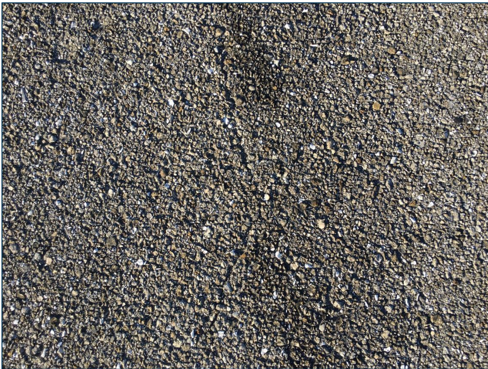
Apron AP, Section 4105, Sample Unit 102 – Low Severity (48) Longitudinal and Transverse Cracking, Low Severity (52) Raveling, Low Severity (56) Swelling
