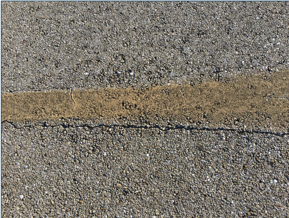
Taxilane To Hangars, Section 205, Sample Unit 105 – Low and Medium Severity (48) Longitudinal and Transverse Cracking, Low Severity (52) Raveling
