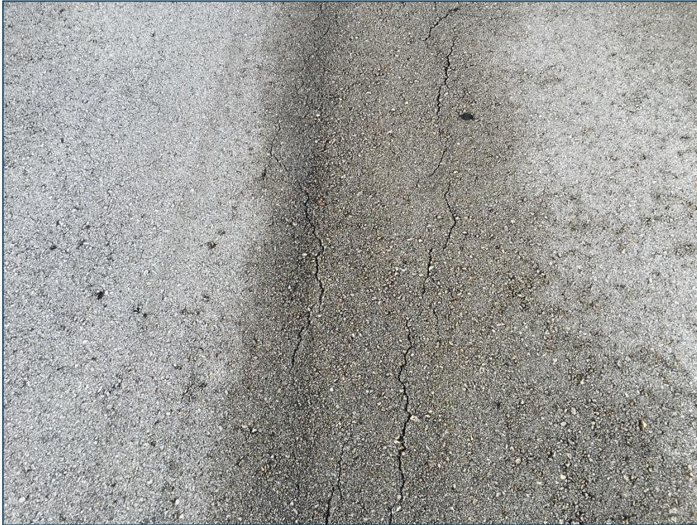
Taxiway B1, Section 315, Sample Unit 300 – Low Severity (48) Longitudinal and Transverse Cracking, Low Severity (52) Raveling
