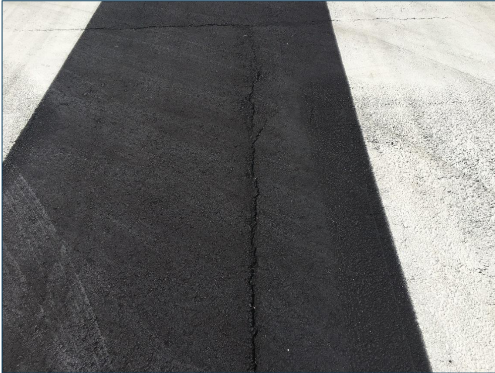
Runway 11-29, Section 6105, Sample Unit 100 – Low Severity (48) Longitudinal and Transverse Cracking, Low Severity (57) Weathering
