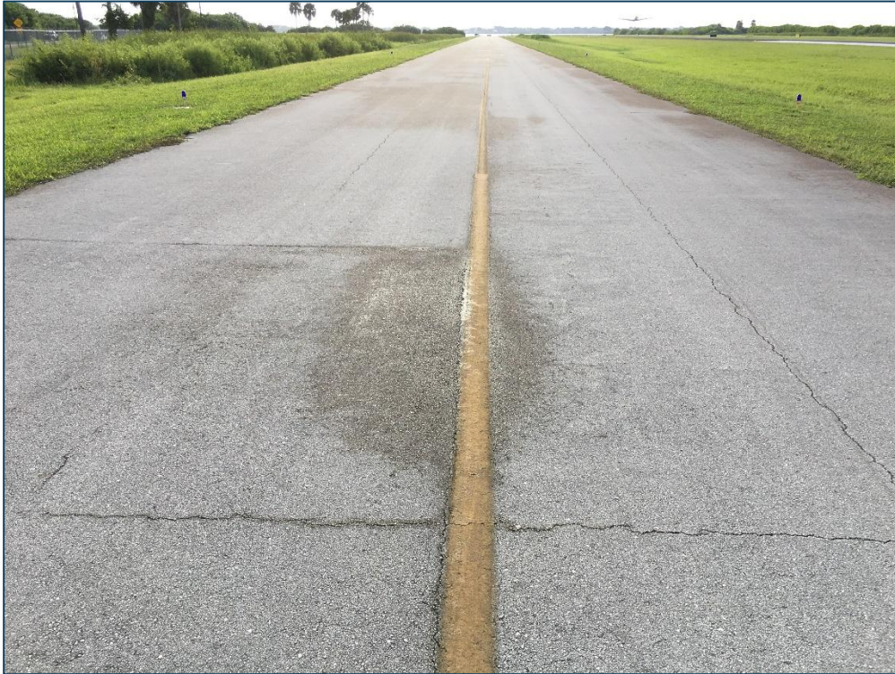
Taxiway B, Section 210, Sample Unit 109 – Low Severity (48) Longitudinal and Transverse Cracking, Low Severity (52) Raveling
