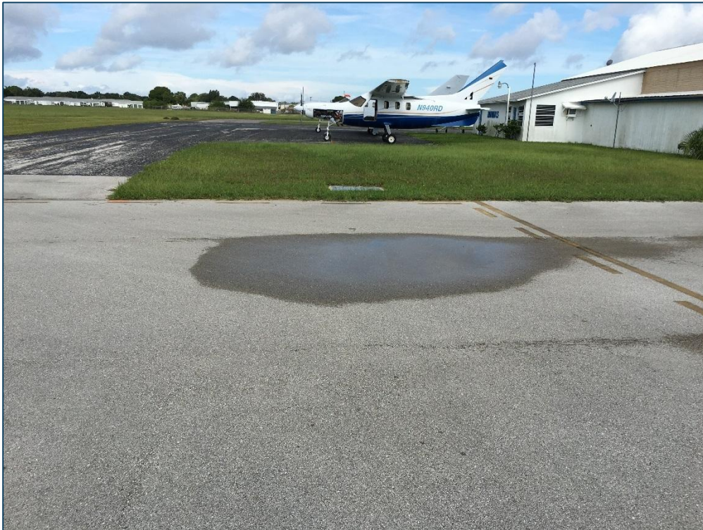
Apron N, Section 4215, Sample Unit 221 – Low Severity (45) Depression, Low Severity (48) Longitudinal and Transverse Cracking, Low Severity (52) Raveling
