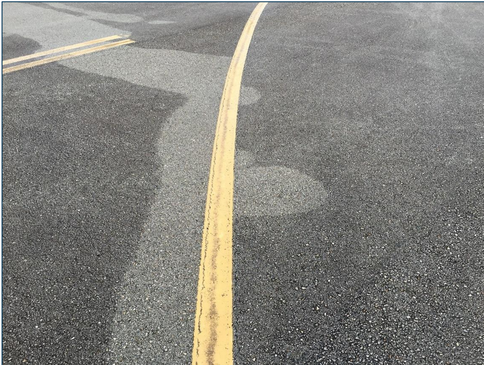
Apron RU RW29, Section 5105, Sample Unit 102 – Low Severity (48) Longitudinal and Transverse Cracking, Low Severity (57) Weathering
