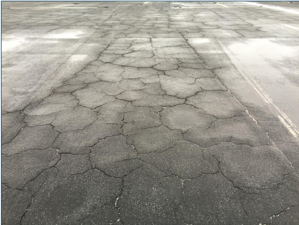
Apron S, Section 4111, Sample Unit 205 – Medium Severity (43) Block Cracking, Low Severity (45) Depression
