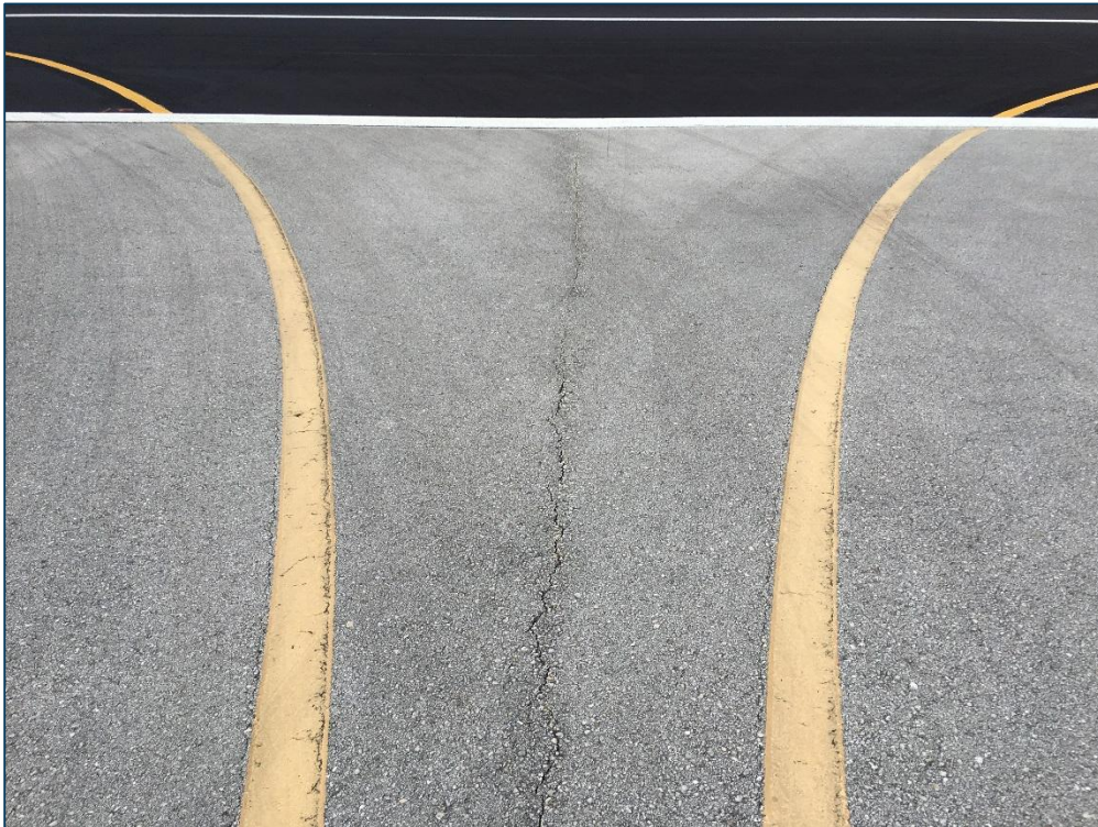
Taxiway A3, Section 505, Sample Unit 100 – Low Severity (48) Longitudinal and Transverse Cracking, Low Severity (57) Weathering, and Low Severity (52) Raveling
