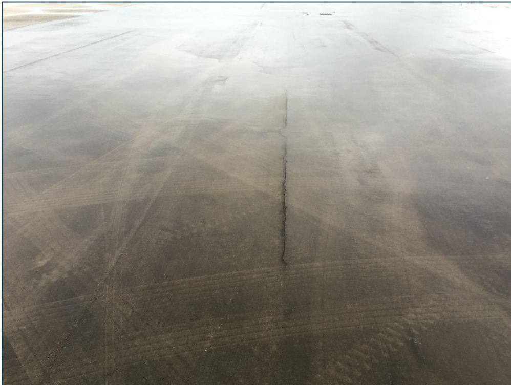
Apron SW, Section 4305, Sample Unit 200 – Low Severity (48) Longitudinal and Transverse Cracking, Low Severity (57) Weathering
