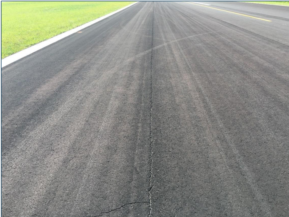
Runway 11-29, Section 6105, Sample Unit 137 – Low Severity (48) Longitudinal and Transverse Cracking, Low Severity (57) Weathering
