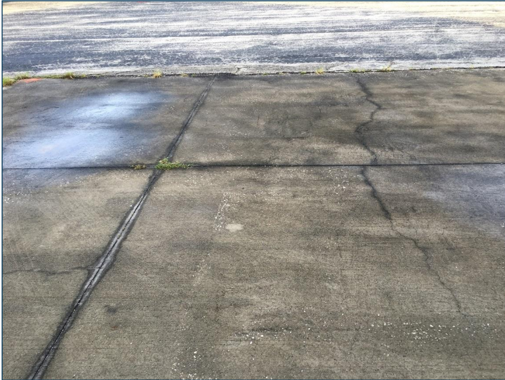
Apron N, Section 4203, Sample Unit 100 – Low Severity (63) Longitudinal, Transverse, and Diagonal Cracking, (73) Shrinkage Cracks, High Severity (65) Joint Seal Damage
