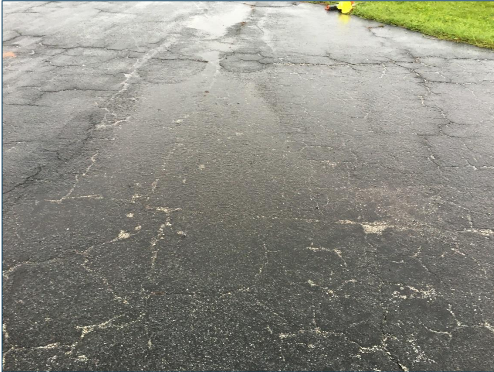
Apron S, Section 4105, Sample Unit 599 – Medium Severity (43) Block Cracking, Low Severity (45) Depression, Low Severity (52) Raveling
