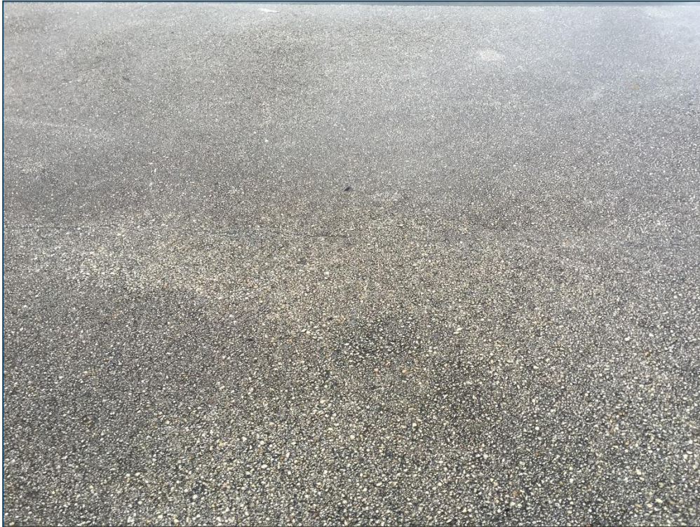
Apron SW, Section 4310, Sample Unit 101 – Low Severity (48) Longitudinal and Transverse Cracking, Low Severity (52) Raveling, Low Severity (57) Weathering
