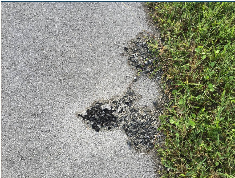
Taxiway B, Section 210, Sample Unit 116 – Low Severity (56) Swelling, Medium Severity (52) Raveling.
