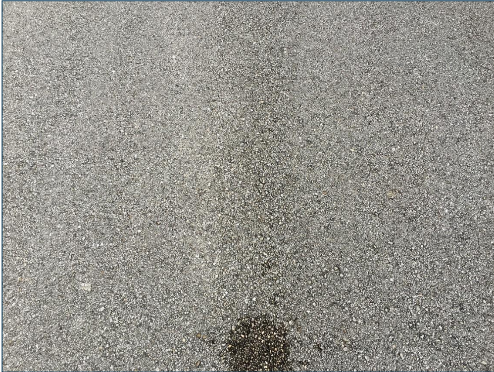
Apron N, Section 4220, Sample Unit 501 – (49) Oil Spillage, (73) Shrinkage Cracks, Low Severity (52) Raveling, Low Severity (57) Weathering
