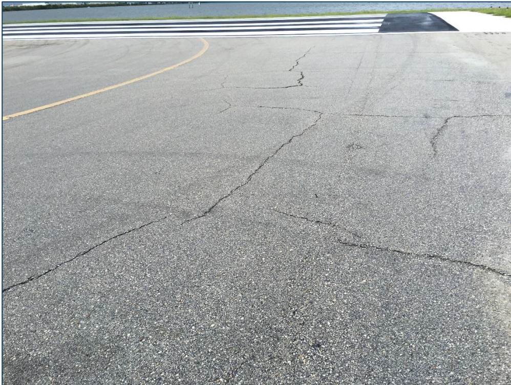
Taxiway A5, Section 110, Sample Unit 101 – Low Severity (48) Longitudinal and Transverse Cracking, Low Severity (57) Weathering, and Low Severity (52) Raveling
