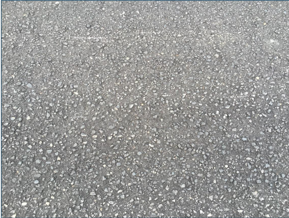
Runway 11-29, Section 6105, Sample Unit 149 – Low Severity (52) Raveling
