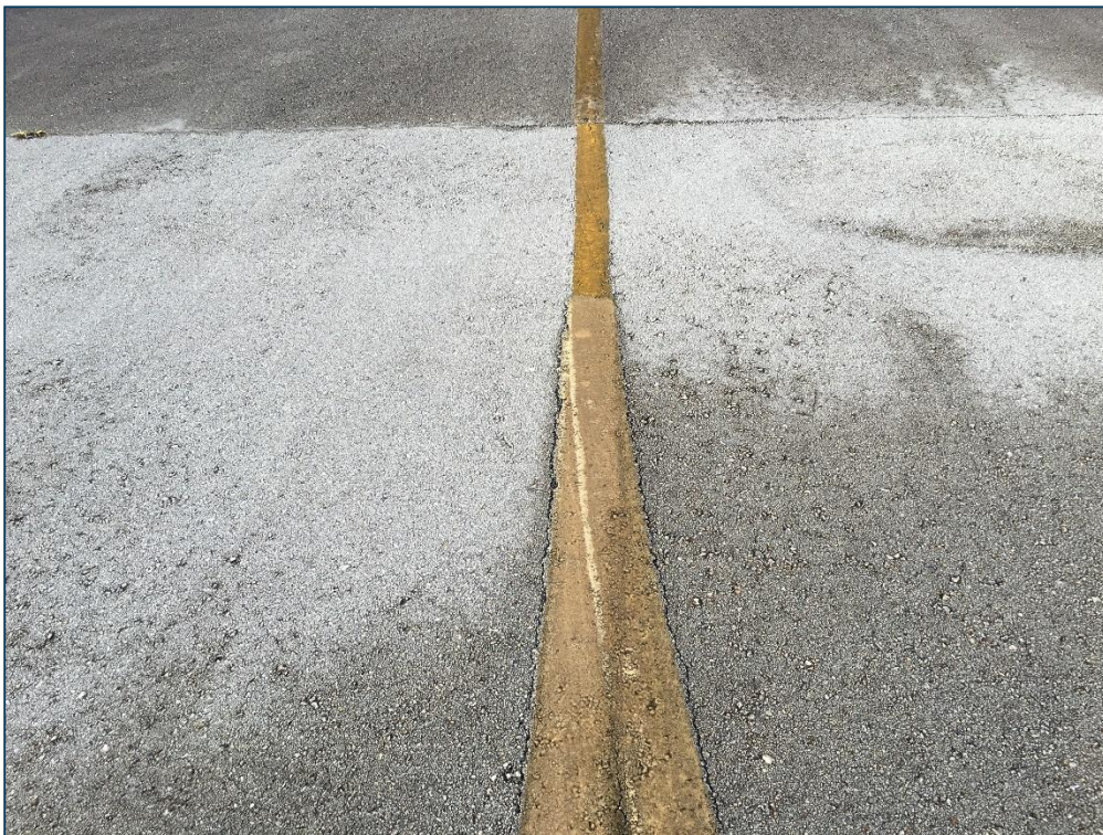
Taxiway B2, Section 410, Sample Unit 400 – Low Severity (48) Longitudinal and Transverse Cracking, Low Severity (52) Raveling
