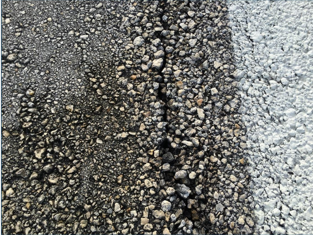
Taxiway B4, Section 216, Sample Unit 124 – Medium Severity (48) Longitudinal and Transverse Cracking, Low Severity (52) Raveling
