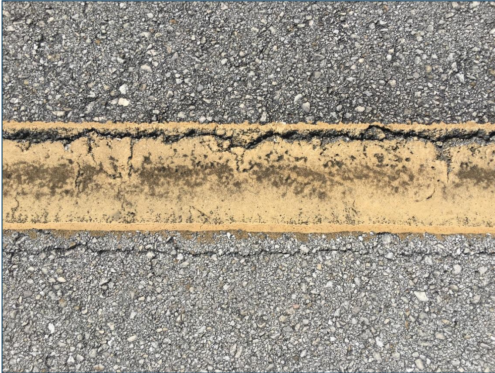
Taxiway A2, Section 405, Sample Unit 400 – Low Severity (48) Longitudinal and Transverse Cracking, Low Severity (57) Weathering
