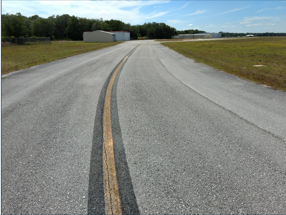
Taxiway A, Section 115, Sample Unit 151 – Low and Medium Severity (48) Longitudinal and Transverse Cracking, Low Severity (52) Raveling, Medium Severity (52) Raveling
