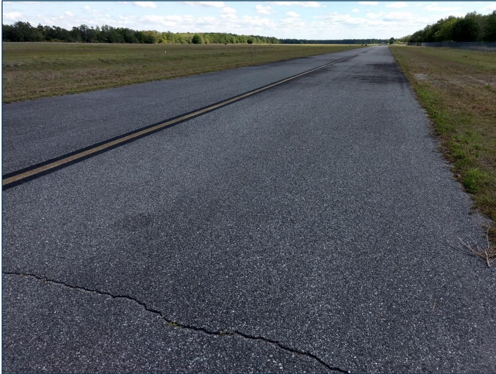
Taxiway B, Section 210, Sample Unit 107 – Low and Medium Severity (48) Longitudinal and Transverse Cracking, Low Severity (52) Raveling, Medium Severity (52) Raveling
