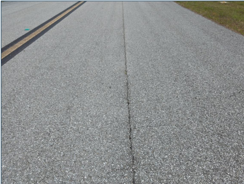
Taxiway A, Section 110, Sample Unit 130 – Low Severity (48) Longitudinal and Transverse Cracking, Low Severity (52) Raveling
