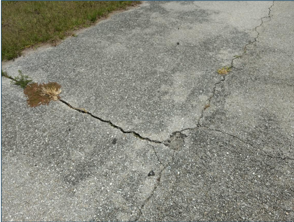
Taxiway A, Section 110, Sample Unit 114 – Low and Medium Severity (48) Longitudinal and Transverse Cracking, Low Severity (52) Raveling, Medium Severity (52) Raveling
