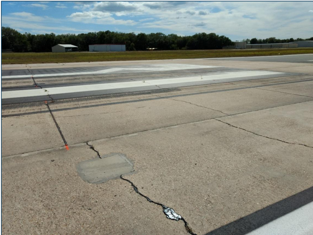
Runway 13-31, Section 6110, Sample Unit 194 – Low Severity (63) Longitudinal, Transverse, and Diagonal Cracking, Low Severity (66) Small Patching, Low Severity (65) Joint Seal Damage
