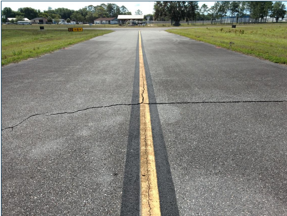
Taxiway B2, Section 220, Sample Unit 102 – Low and Medium Severity (48) Longitudinal and Transverse Cracking, Low Severity (52) Raveling
