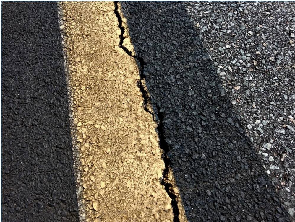
Taxiway B, Section 210, Sample Unit 123 – Medium Severity (48) Longitudinal and Transverse Cracking, Low Severity (52) Raveling
