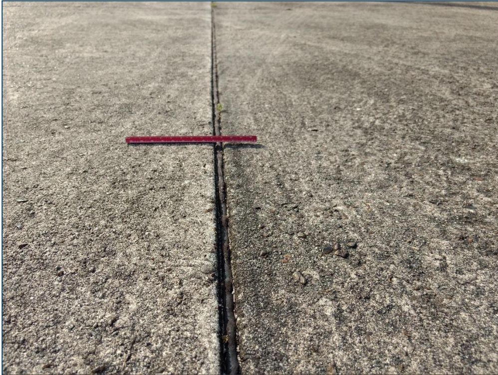
Apron, Section 4105, Sample Unit 101 – Low Severity (65) Joint Seal Damage, Low Severity (71) Faulting
