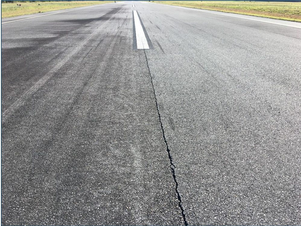
Runway 4-22, Section 6210, Sample Unit 115 – Low and Medium Severity (48) Longitudinal and Transverse Cracking, Low Severity (52) Raveling, Low Severity (57) Weathering
