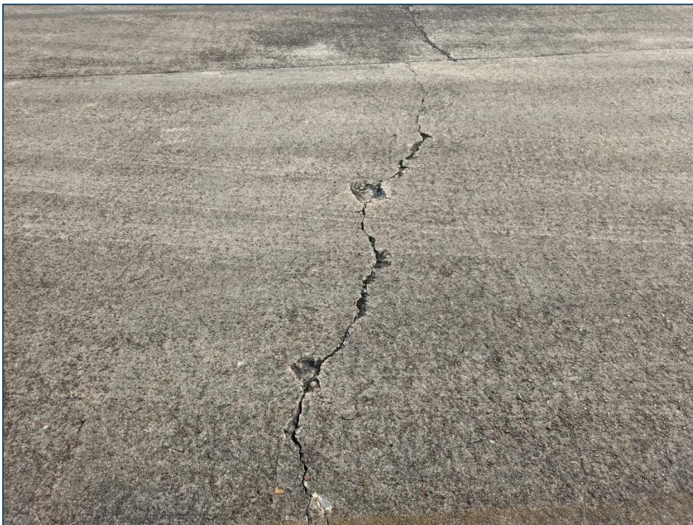
Apron, Section 4105, Sample Unit 401 –Medium Severity (63) Longitudinal, Transverse, and Diagonal Cracking
