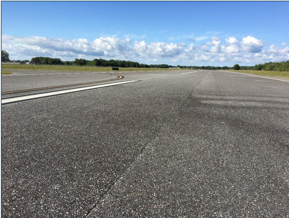
Runway 4-22, Section 6210, Sample Unit 174 – Low Severity (48) Longitudinal and Transverse Cracking, Low Severity (52) Raveling, Low Severity (57) Weathering
