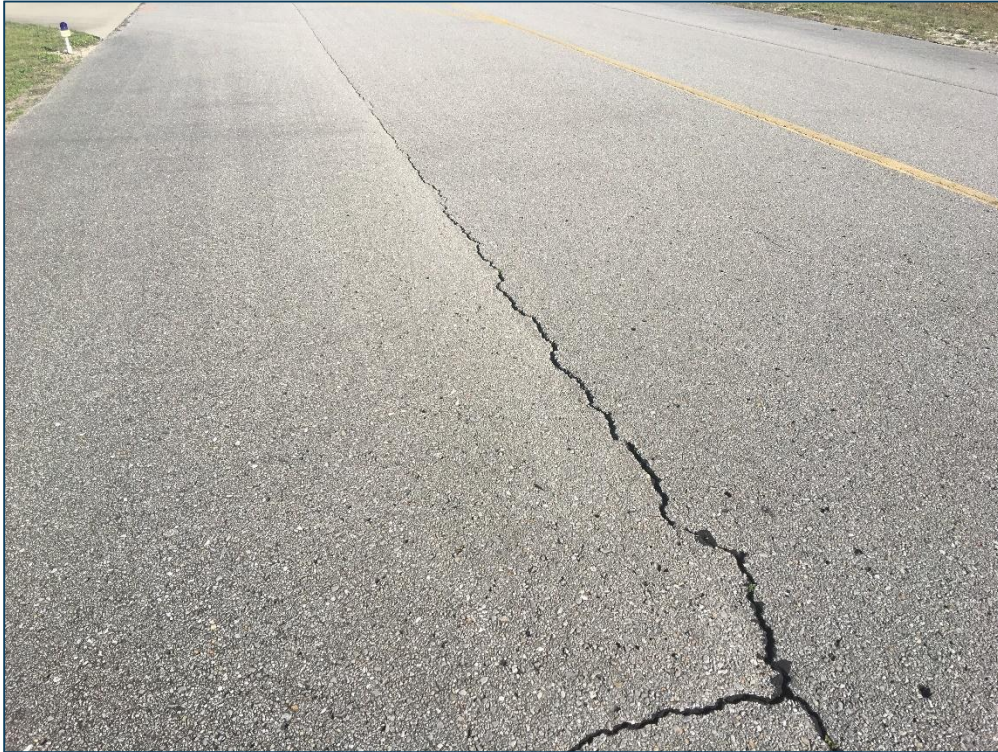
Taxiway A1, Section 105, Sample Unit 108 – Low and Medium Severity (48) Longitudinal and Transverse Cracking, Low Severity (52) Raveling, Medium Severity (52) Raveling
