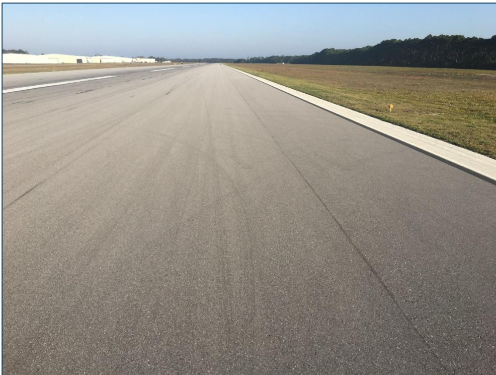
Runway 14-32, Section 6110, Sample Unit 168 – Low Severity (57) Weathering
