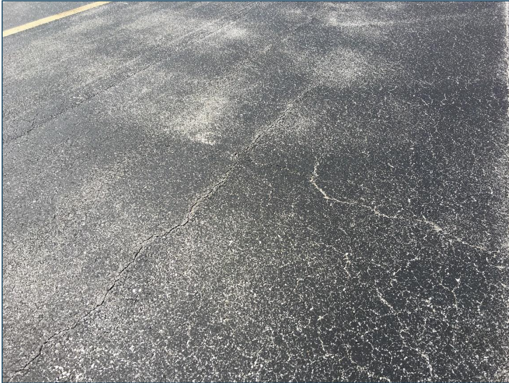
Apron, Section 4120, Sample Unit 84 – Low Severity (48) Longitudinal and Transverse Cracking, Low Severity (52) Raveling, Medium Severity (52) Raveling
