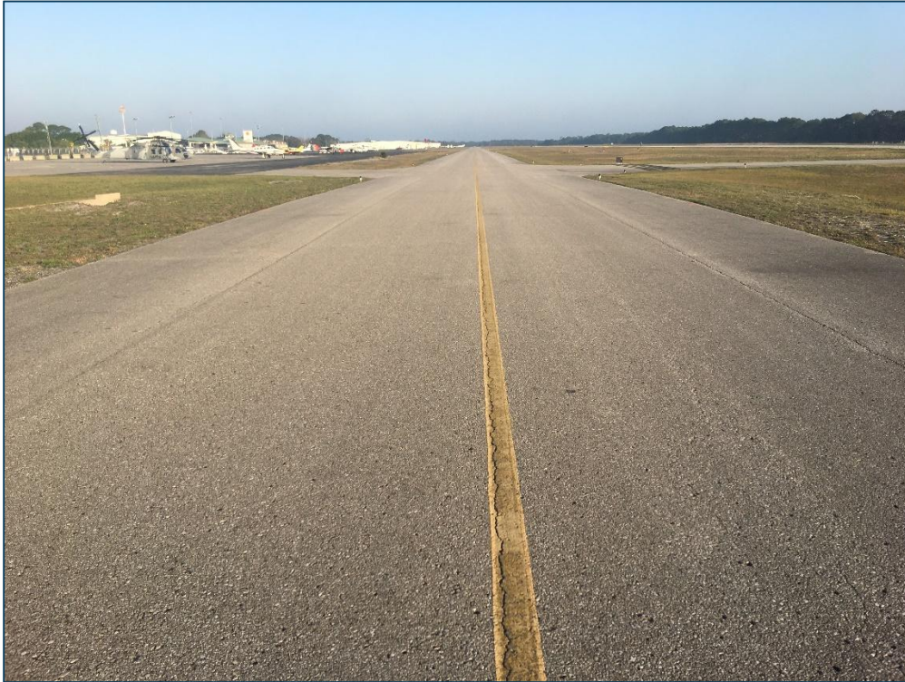
Taxiway A, Section 135, Sample Unit 146 – Low Severity (48) Longitudinal and Transverse Cracking, Low Severity (52) Raveling, Medium Severity (52) Raveling
