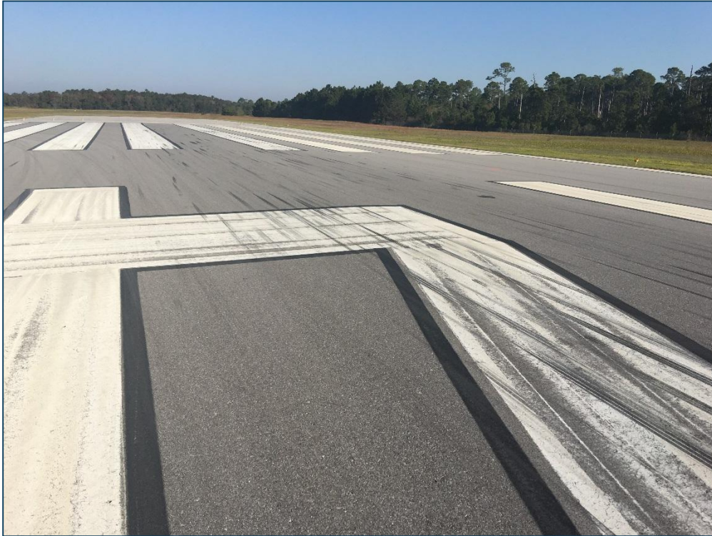
Runway 14-32, Section 6115, Sample Unit 302 – Low Severity (57) Weathering
