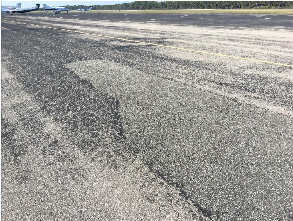
Apron, Section 4125, Sample Unit 709 – Low and Medium Severity (48) Longitudinal and Transverse Cracking, Medium Severity (50) Patching, Medium Severity (52) Raveling
