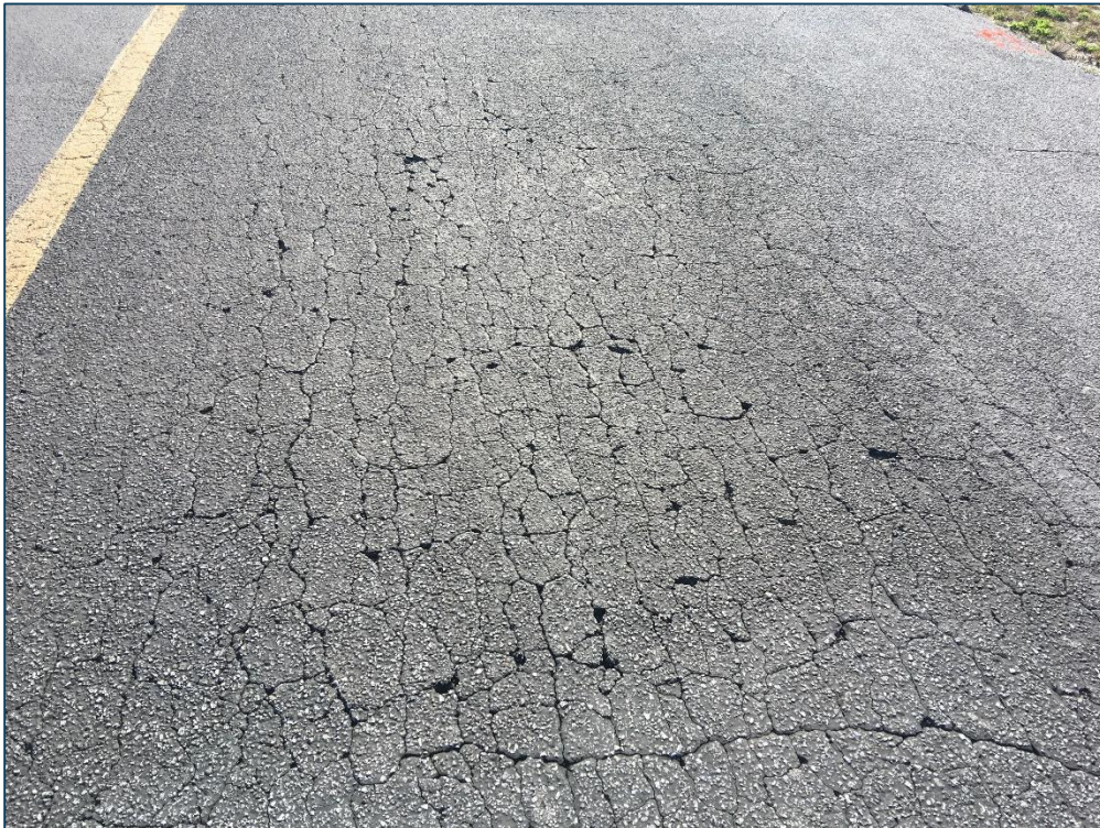
Taxiway Connector, Section 209, Sample Unit 201 – Medium Severity (41) Alligator Cracking, Low Severity (48) Longitudinal and Transverse Cracking, Low Severity (52) Raveling
