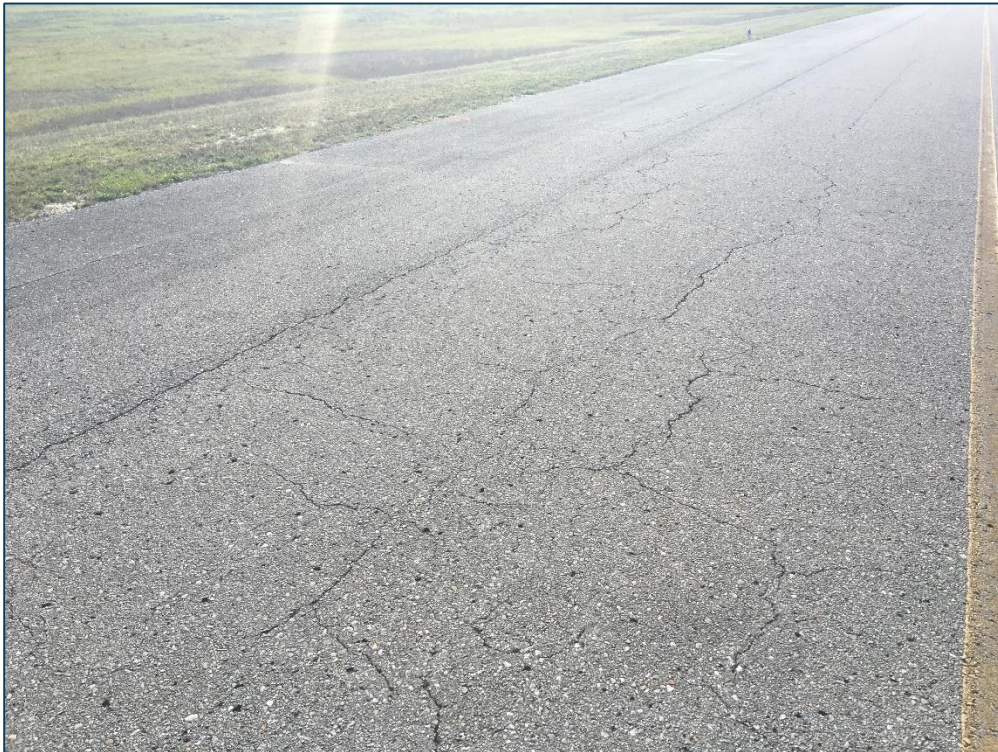
Taxiway A, Section 115, Sample Unit 127 – Low Severity (43) Block Cracking, Low Severity (48) Longitudinal and Transverse Cracking, Medium Severity (52) Raveling, Low Severity (56) Swelling
