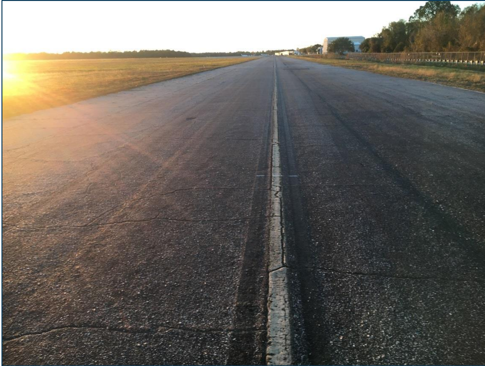
Taxiway A, Section 105, Sample Unit 141 - Low Severity (43) Block Cracking, Medium Severity (43) Block Cracking, Low Severity (52) Raveling, Low Severity (53) Rutting
