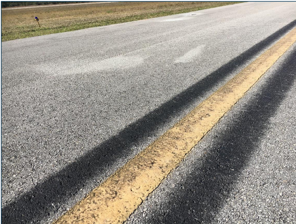
Taxiway B, Section 205, Sample Unit 113 - Low Severity (48) Longitudinal and Transverse Cracking, Low Severity (52) Raveling, Medium Severity (52) Raveling, Low Severity (56) Swelling
