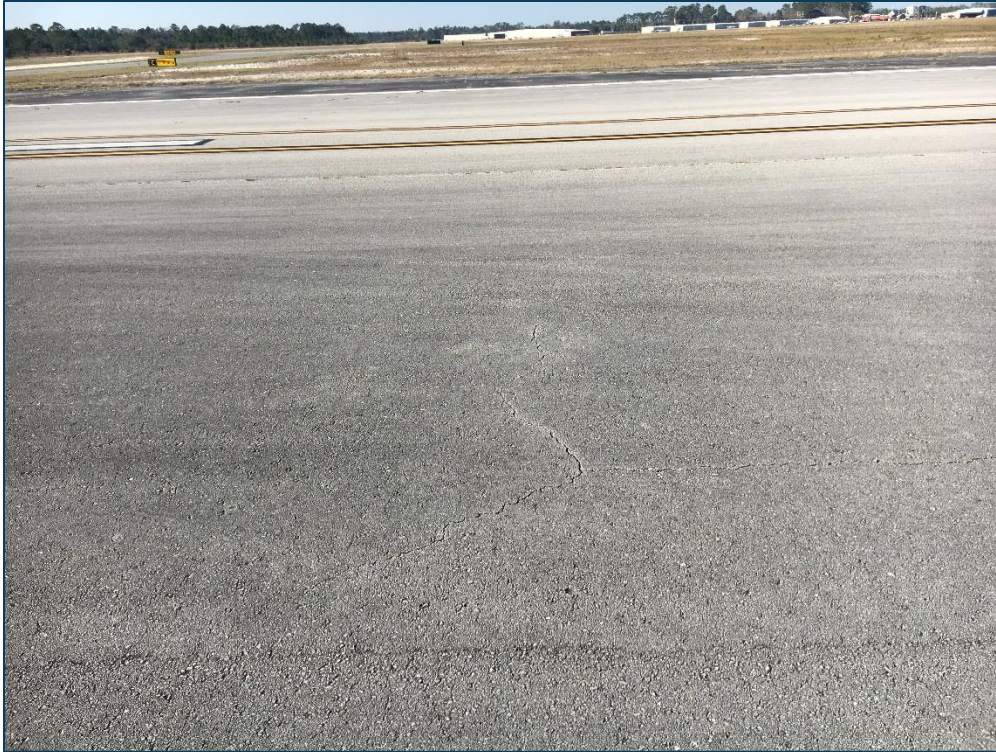
Runway 6-24, Section 6205, Sample Unit 149 - Low Severity (48) Longitudinal and Transverse Cracking, Medium Severity (48) Longitudinal and Transverse Cracking, Low Severity (52) Raveling, Medium Severity (52) Raveling
