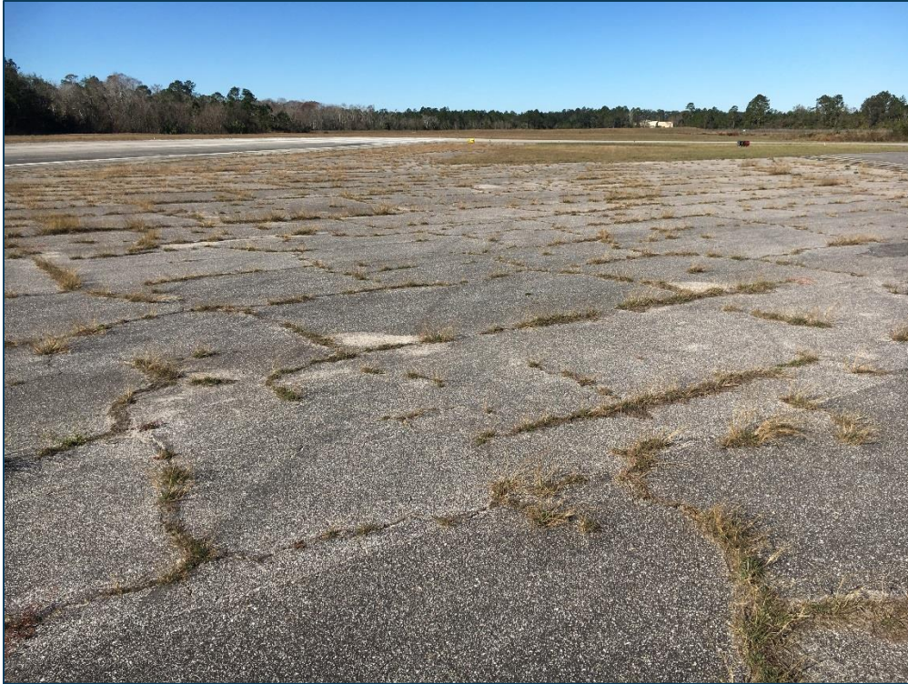
Run-Up Apron RW 11, Section 5103, Sample Unit 602 – Medium Severity (43) Block Cracking, Low Severity (52) Raveling
