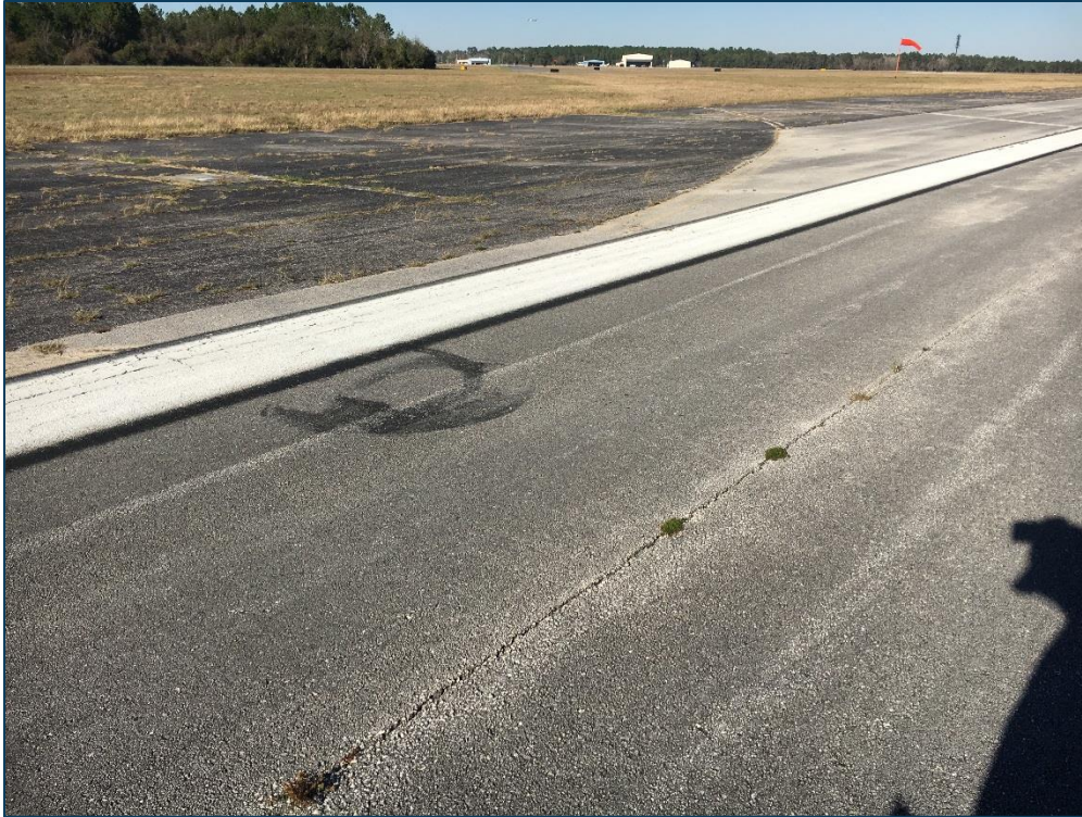
Runway 6-24, Section 6205, Sample Unit 117 – Low Severity (48) Longitudinal and Transverse Cracking, Low Severity (56) Swelling, Low Severity (52) Raveling
