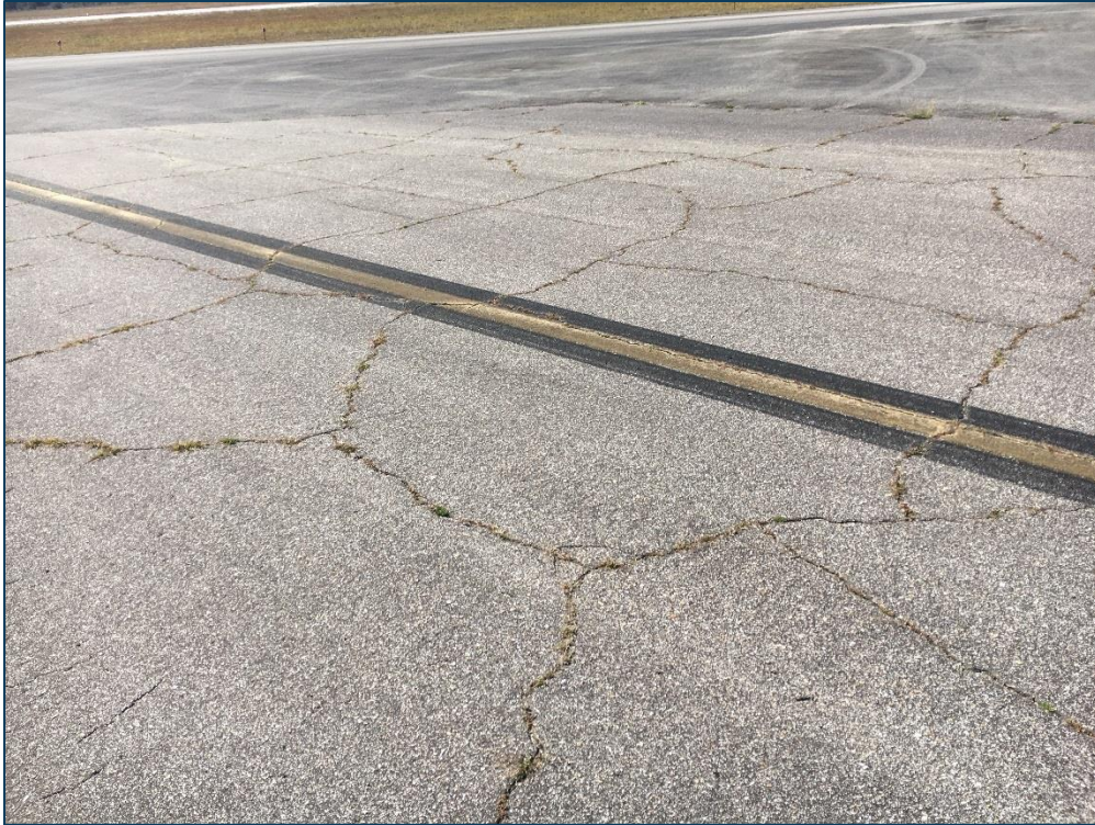
Taxiway C, Section 307, Sample Unit 104 - Medium Severity (43) Block Cracking, Low Severity (52) Raveling
