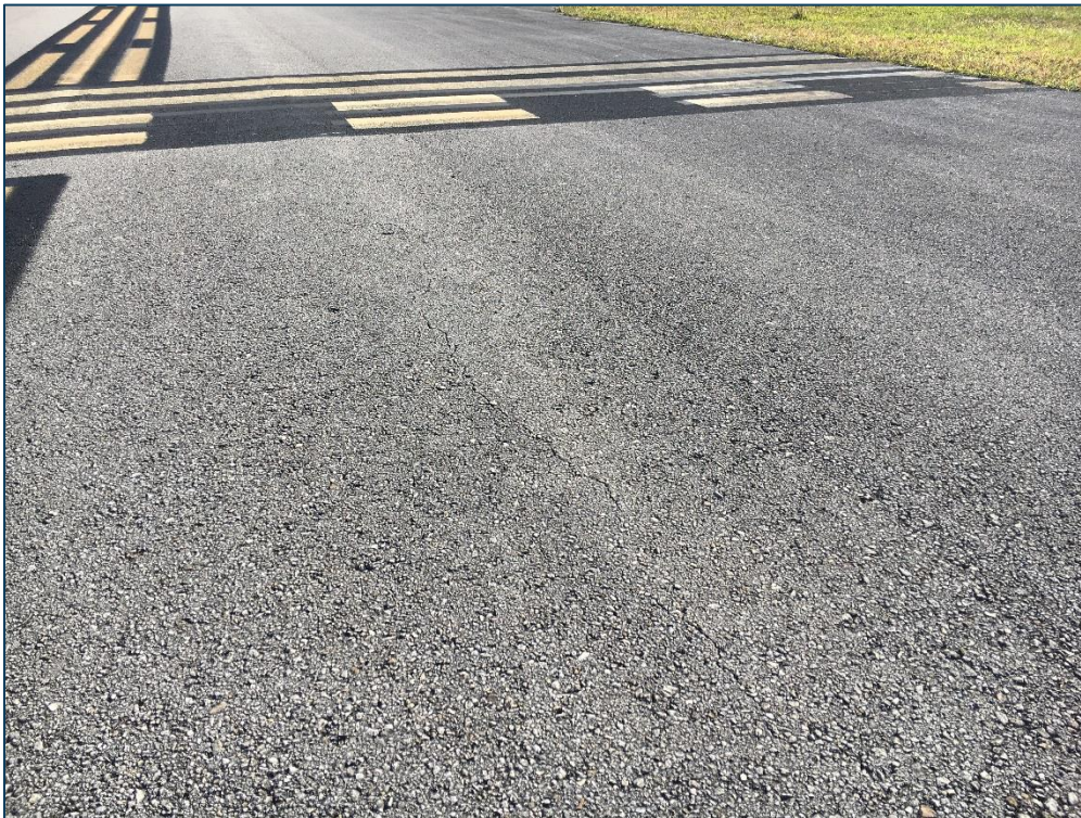
Taxiway A, Section 102, Sample Unit 101 - Low Severity (48) Longitudinal and Transverse Cracking, Low Severity (52) Raveling, Medium Severity (52) Raveling, Low Severity (56) Swelling
