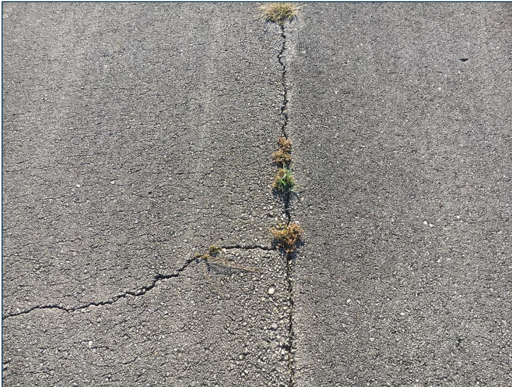
Runway 6-24, Section 6205, Sample Unit 107 - Low Severity (48) Longitudinal and Transverse Cracking, Medium Severity (48) Longitudinal and Transverse Cracking, Low Severity (52) Raveling, Medium Severity (52) Raveling
