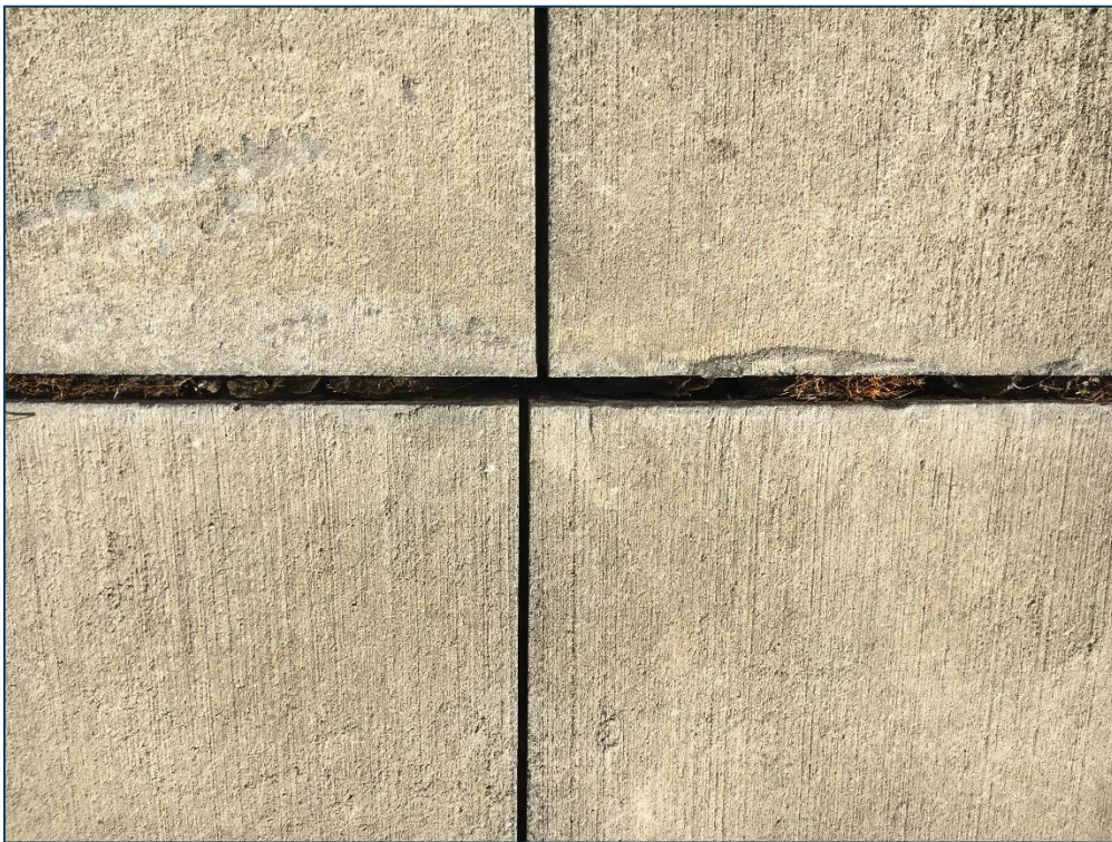
North Apron, Section 4405, Sample Unit 101 – High Severity (65) Joint Seal Damage
