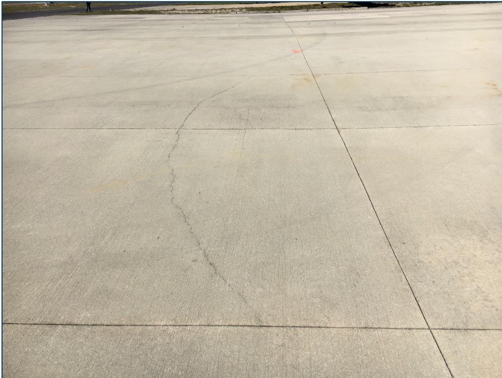
GA Apron, Section 4510, Sample Unit 100 – Low Severity (63) Longitudinal, Transverse, and Diagonal Cracking, High Severity (65) Joint Seal Damage
