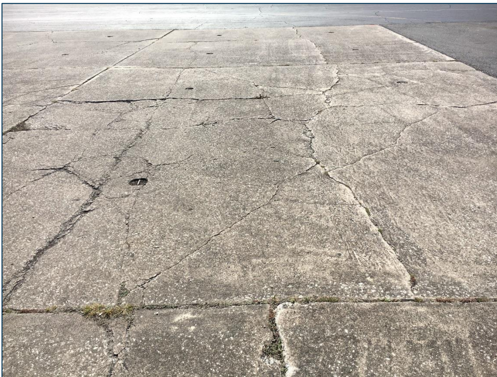
Apron, Section 4105, Sample Unit 101 – High Severity (72) Shattered Slab, High Severity (65) Joint Seal Damage
