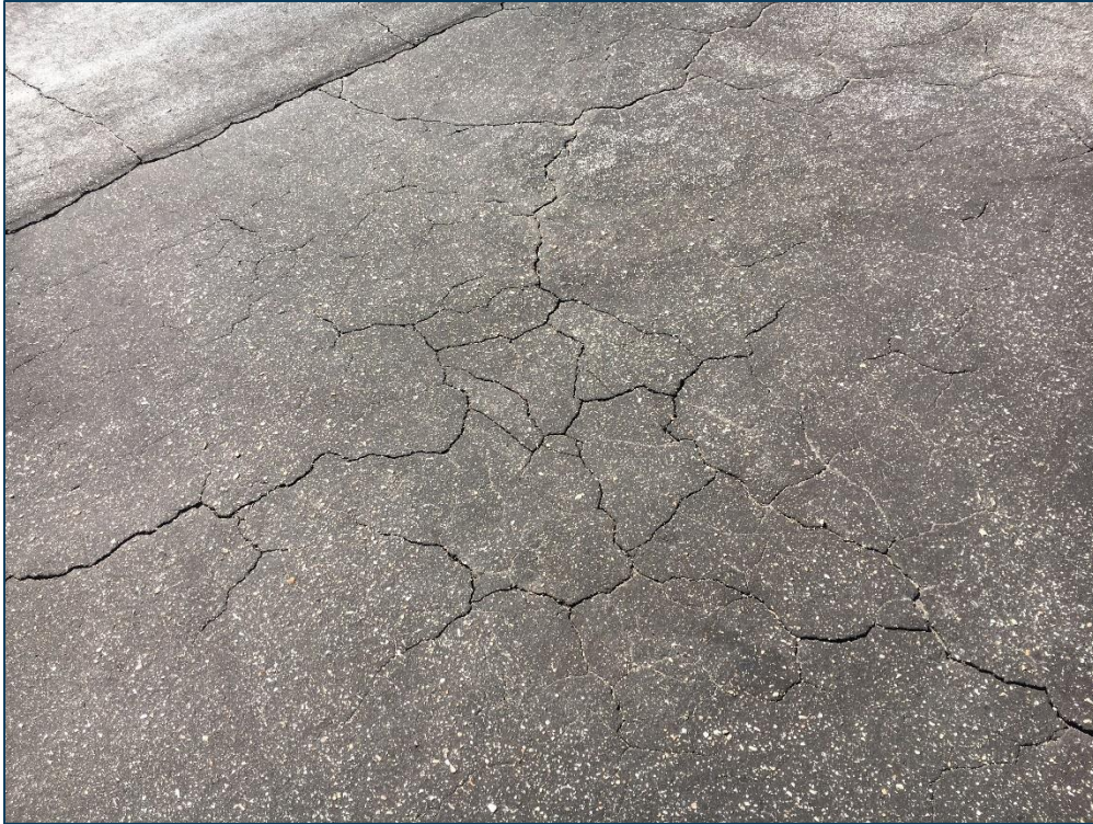
Apron, Section 4115, Sample Unit 401 – Medium Severity (41) Alligator Cracking, Medium Severity (48) Longitudinal and Transverse Cracking, Low Severity (52) Raveling
