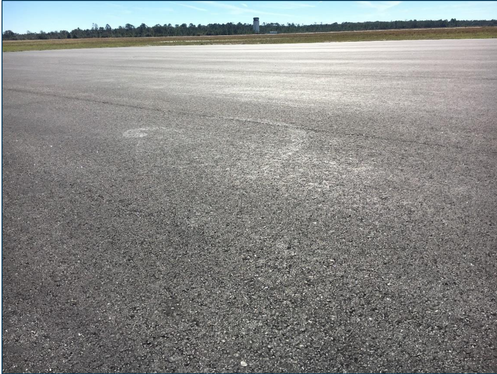
Apron Mid, Section 4610, Sample Unit 102 – Low Severity (57) Weathering
