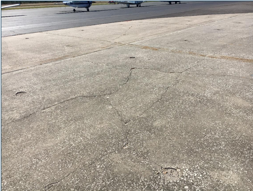
Apron, Section 4120, Sample Unit 402 – High Severity (65) Joint Seal Damage, Medium Severity (72) Shattered Slab
