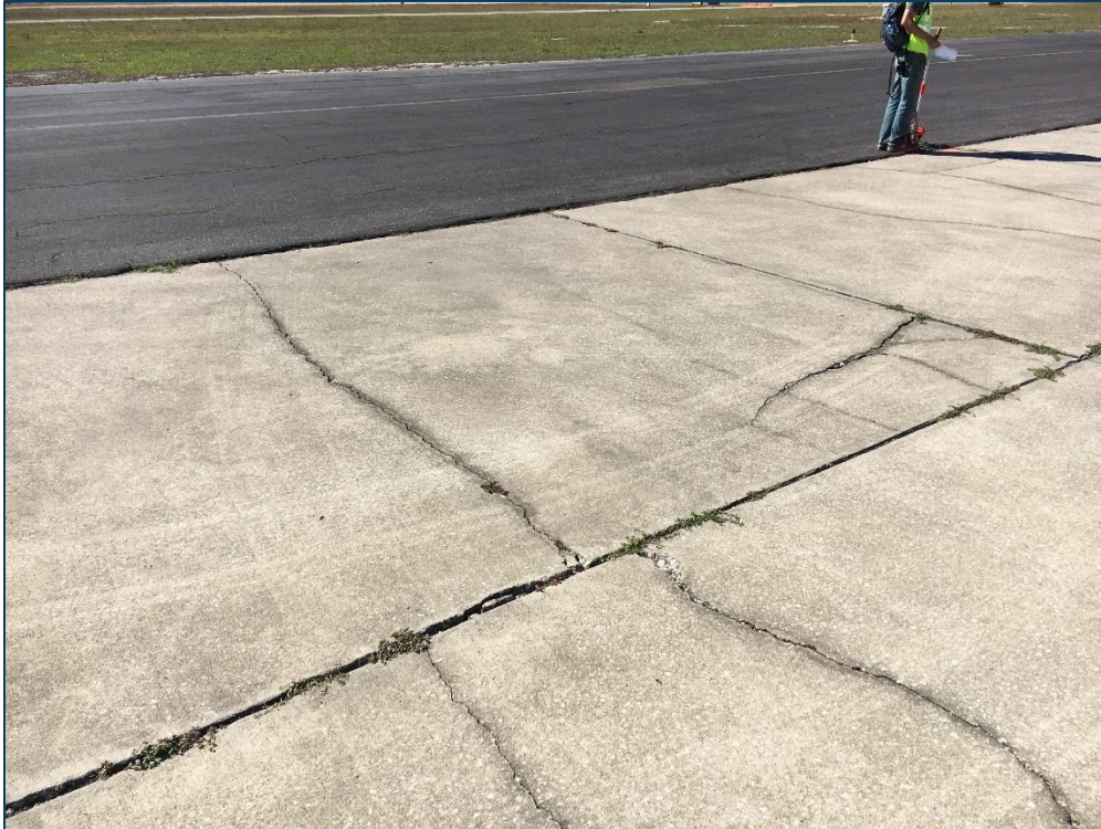
Apron, Section 4130, Sample Unit 101 – Medium Severity (63) Longitudinal, Transverse, and Diagonal Cracking, Medium Severity (62) Corner Break, High Severity (65) Joint Seal Damage
