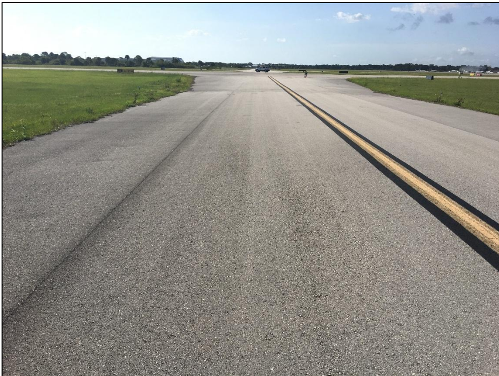
Taxiway B, Section 205, Sample Unit 127 - Low Severity (48) Longitudinal and Transverse Cracking, Low Severity (57) Weathering
