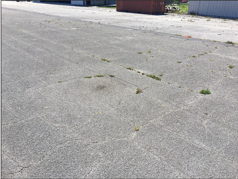
Center Apron, Section 4125, Sample Unit 199 - Low and Medium Severity (43) Block Cracking, Low and Medium Severity (52) Raveling
