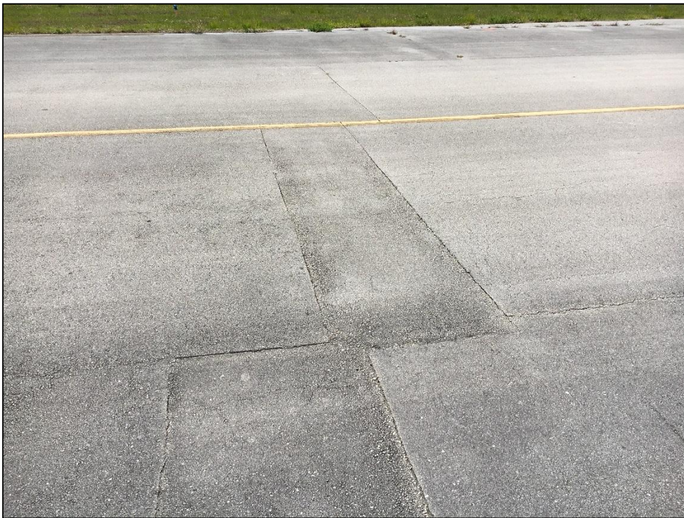
Taxiway E, Section 515, Sample Unit 611 - Low Severity (48) Longitudinal and Transverse Cracking, Low Severity (50) Patching, Low Severity (57) Weathering
