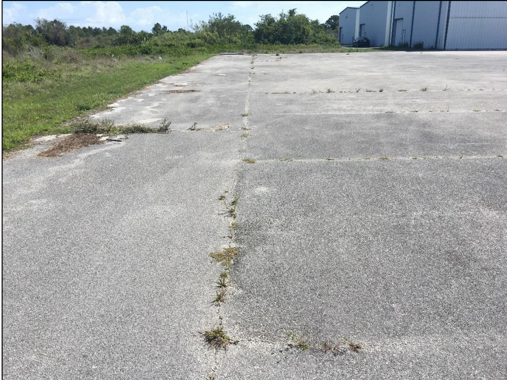
East Apron, Section 4405, Sample Unit 300 - Low Severity (48) Longitudinal and Transverse Cracking, Low Severity (52) Raveling, Low Severity (56) Swelling, Low Severity (57) Weathering
