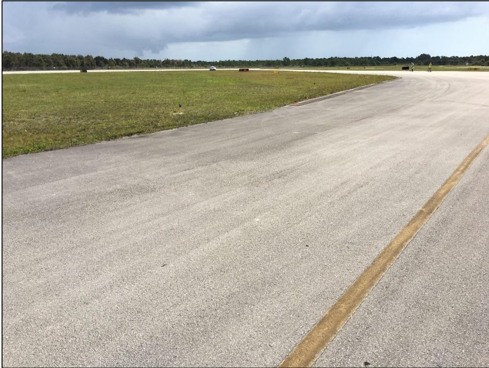
Taxiway A, Section 105, Sample Unit 108 - Low Severity (45) Depression, Low Severity (48) Longitudinal and Transverse Cracking, Low Severity (57) Weathering
