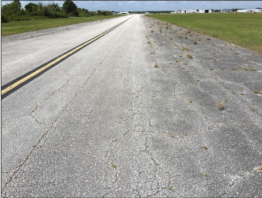
Taxiway D, Section 415, Sample Unit 314 - Medium Severity (43) Block Cracking, Low and Medium Severity (52) Raveling
