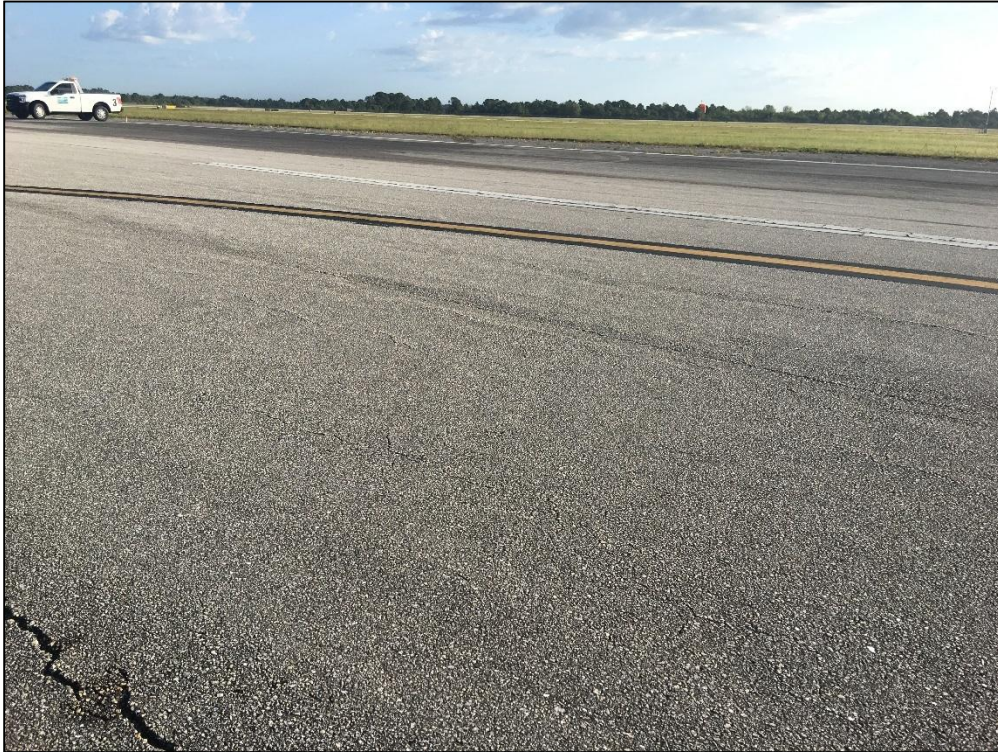
Runway 14-32, Section 6205, Sample Unit 156 - Low and Medium Severity (48) Longitudinal and Transverse Cracking, Low Severity (56) Swelling, Low Severity (57) Weathering
