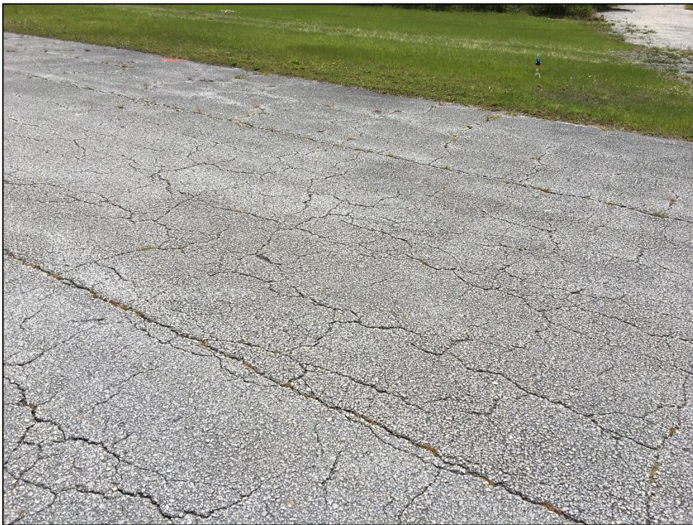
Taxiway D, Section 415, Sample Unit 310 - Medium Severity (43) Block Cracking, Medium Severity (52) Raveling
