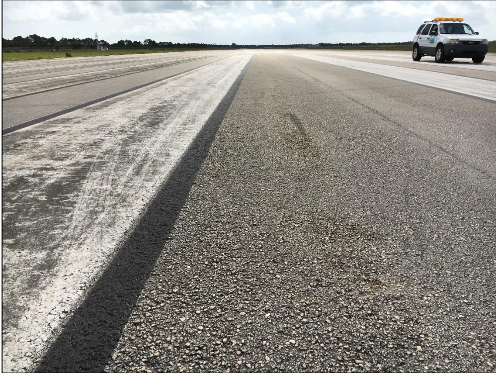
Runway 10R-28L, Section 6115, Sample Unit 300 - Low Severity (48) Longitudinal and Transverse Cracking, Low Severity (52) Raveling, Low Severity (57) Weathering
