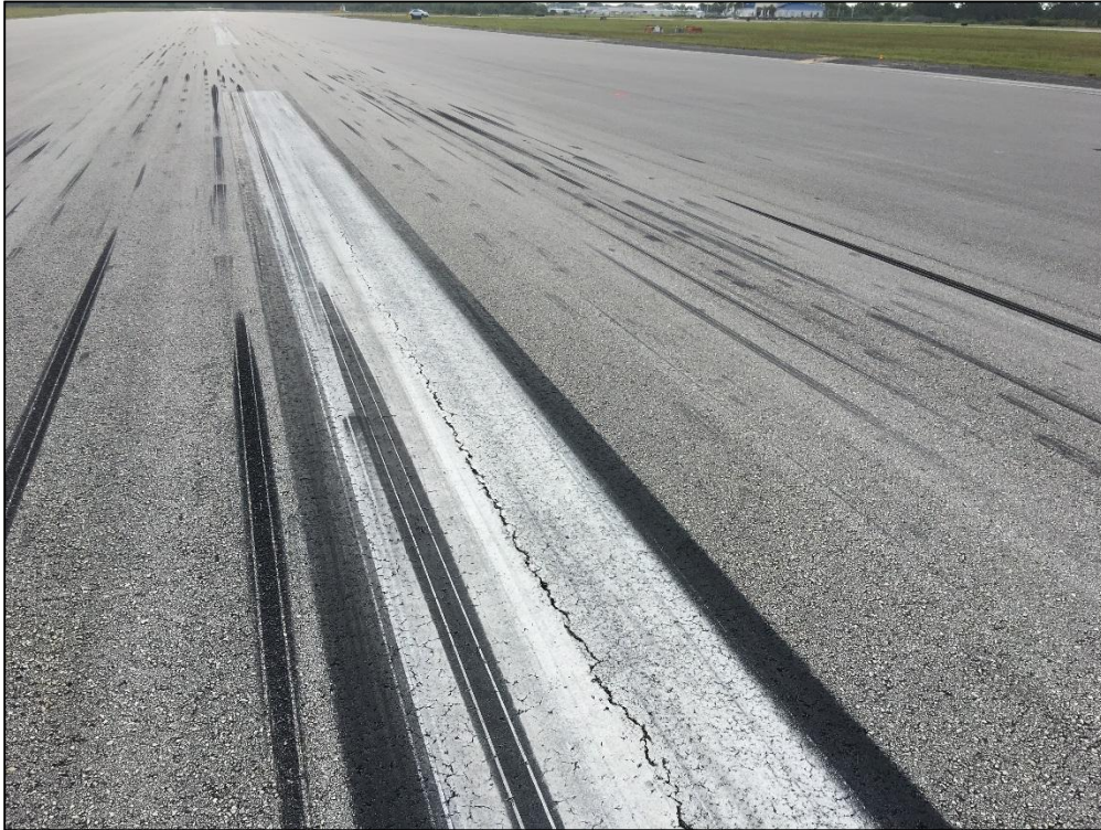
Runway 10R-28L, Section 6105, Sample Unit 354 - Low Severity (48) Longitudinal and Transverse Cracking, Low Severity (52) Raveling, Low Severity (57) Weathering
