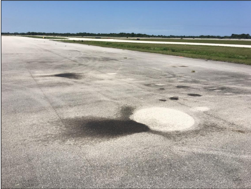
Center Apron, Section 4105, Sample Unit 109 - Low Severity (48) Longitudinal and Transverse Cracking, (49) Oil Spillage, Low Severity (52) Raveling, Low Severity (57) Weathering
