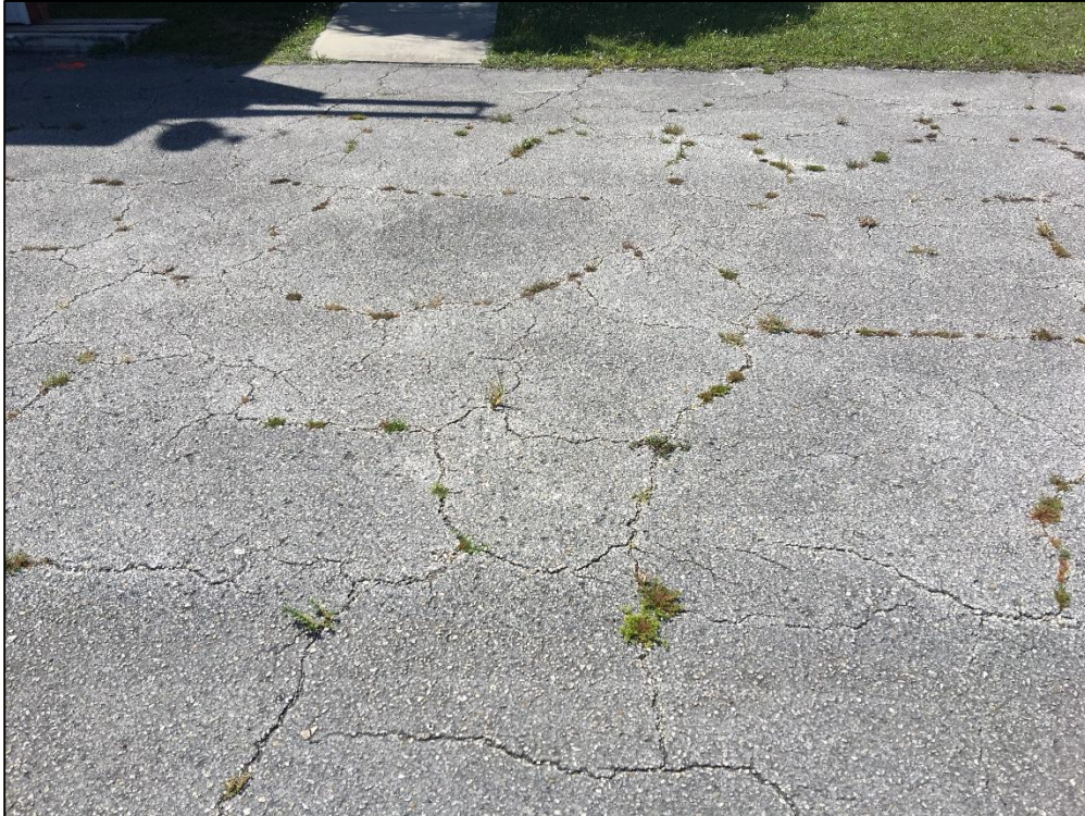
Center Apron, Section 4127, Sample Unit 98 - Medium Severity (43) Block Cracking, Low and Medium Severity (52) Raveling
