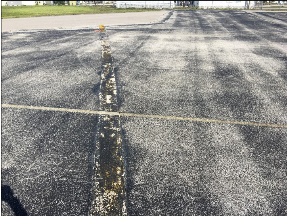
South Apron, Section 4205, Sample Unit 502 - Low Severity (43) Block Cracking, Low Severity (52) Raveling
