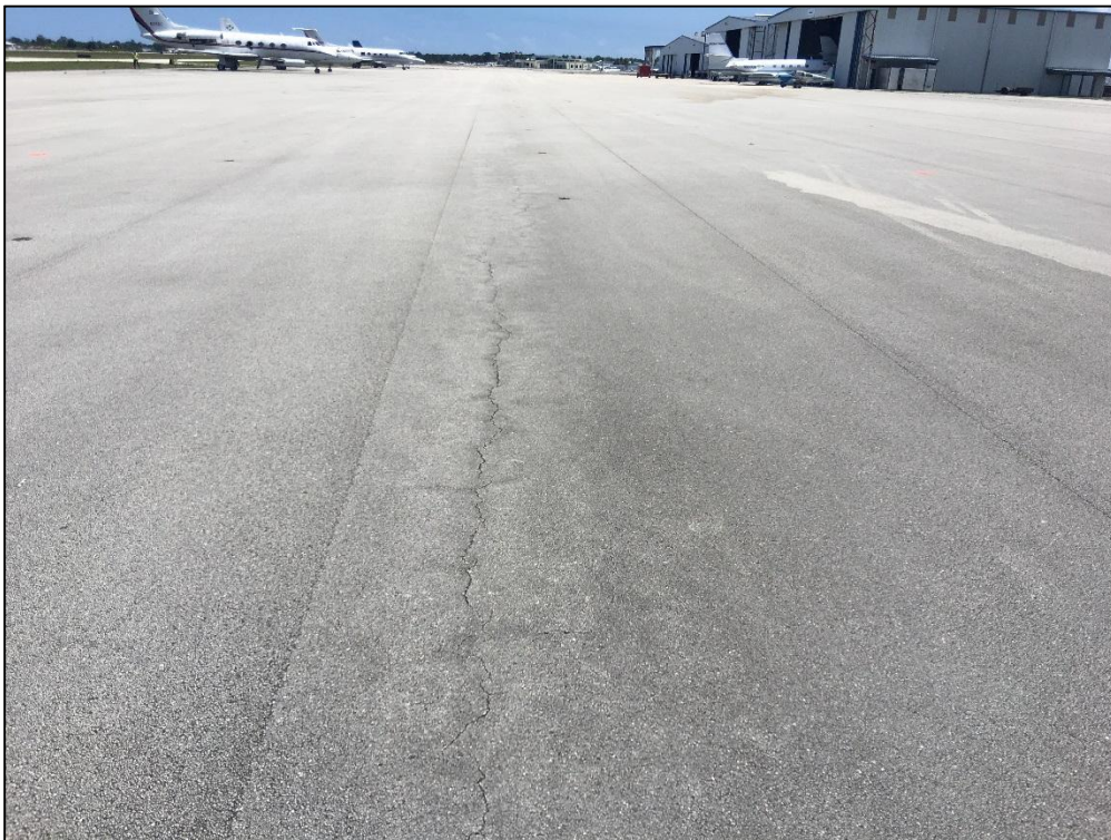
Center Apron, Section 4105, Sample Unit 306 - Low Severity (48) Longitudinal and Transverse Cracking, Low Severity (52) Raveling, Low Severity (56) Swelling, Low Severity (57) Weathering
