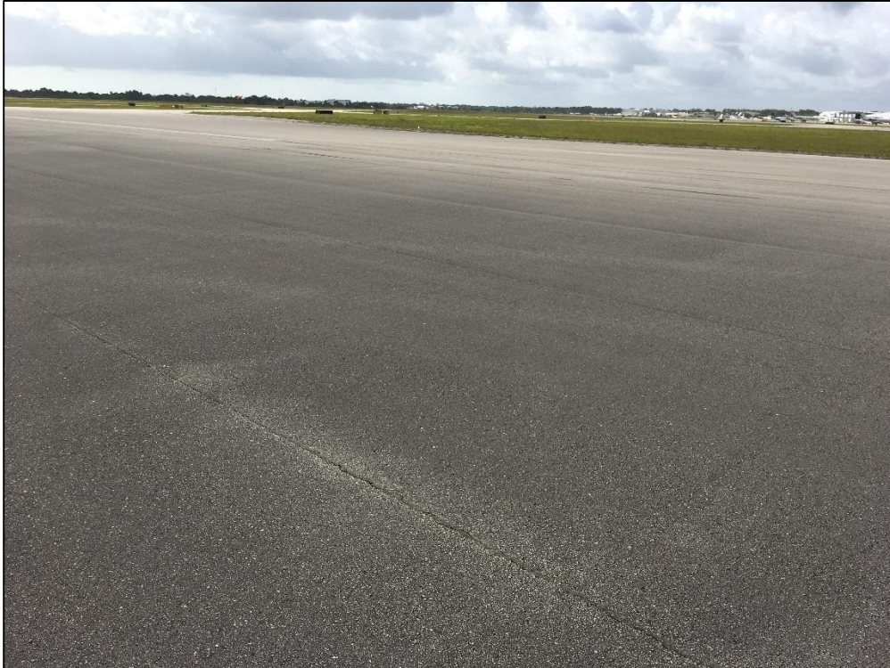
Runway 10R-28L, Section 6110, Sample Unit 127 - Low Severity (48) Longitudinal and Transverse Cracking, Low Severity (57) Weathering
