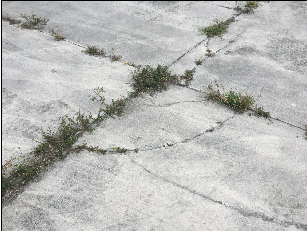
Southeast Apron, Section 4305, Sample Unit 602 - Medium Severity (62) Corner Break, High Severity (65) Joint Seal Damage, (73) Shrinkage Cracking, Low Severity (74) Joint Spall
