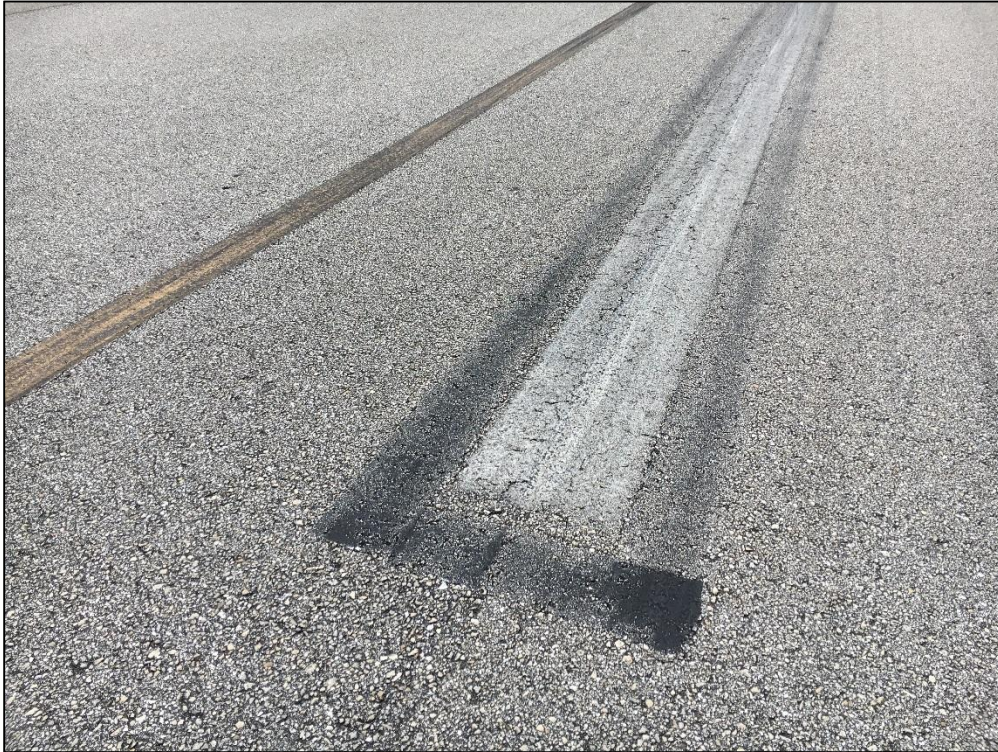
Runway 10L-28R, Section 6305, Sample Unit 126 - Low Severity (48) Longitudinal and Transverse Cracking, Low Severity (57) Weathering
