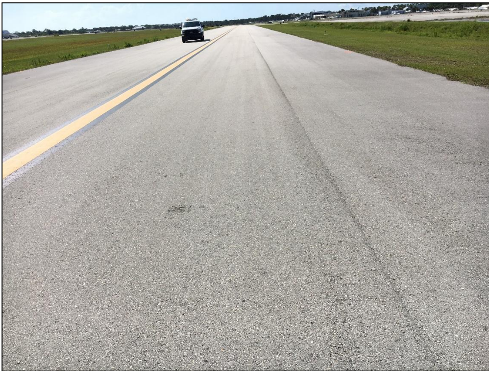
Taxiway C, Section 305, Sample Unit 430 - Low Severity (48) Longitudinal and Transverse Cracking, Low Severity (57) Weathering
