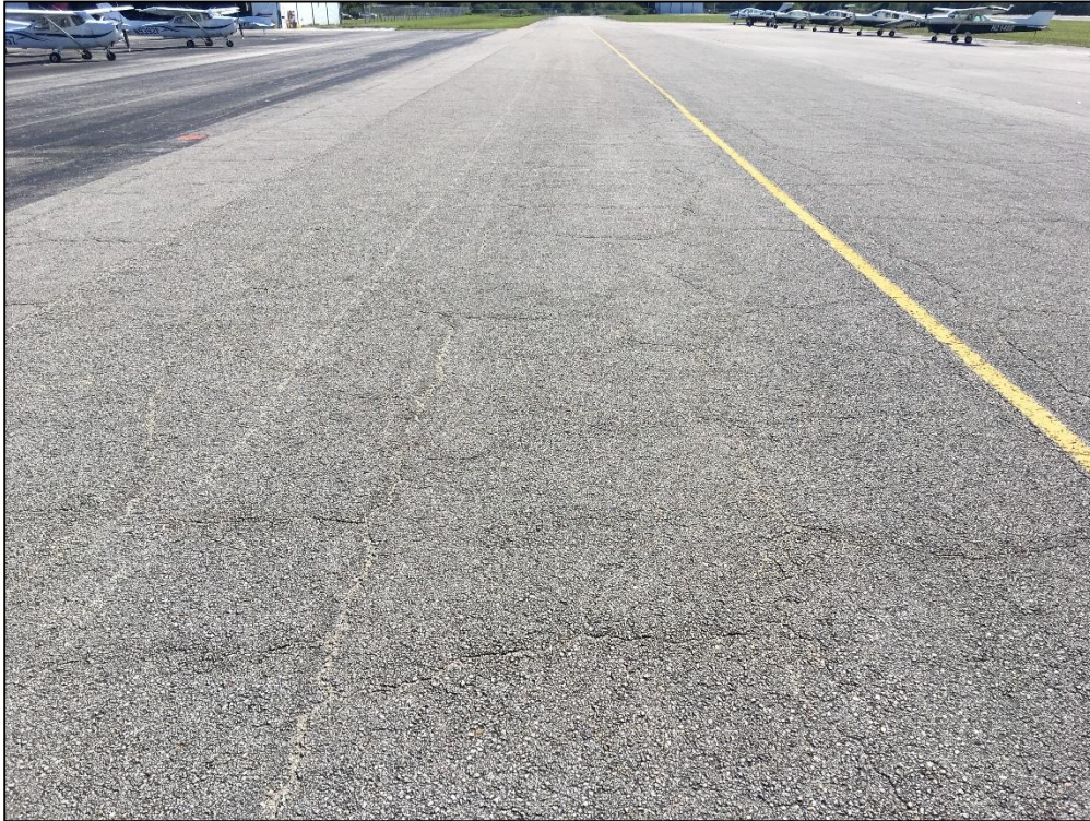
Taxiway D, Section 405, Sample Unit 309 – Low and Medium Severity (43) Block Cracking, Medium Severity (52) Raveling
