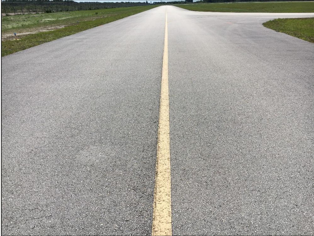
Taxiway F, Section 605, Sample Unit 628 - Low Severity (57) Weathering
