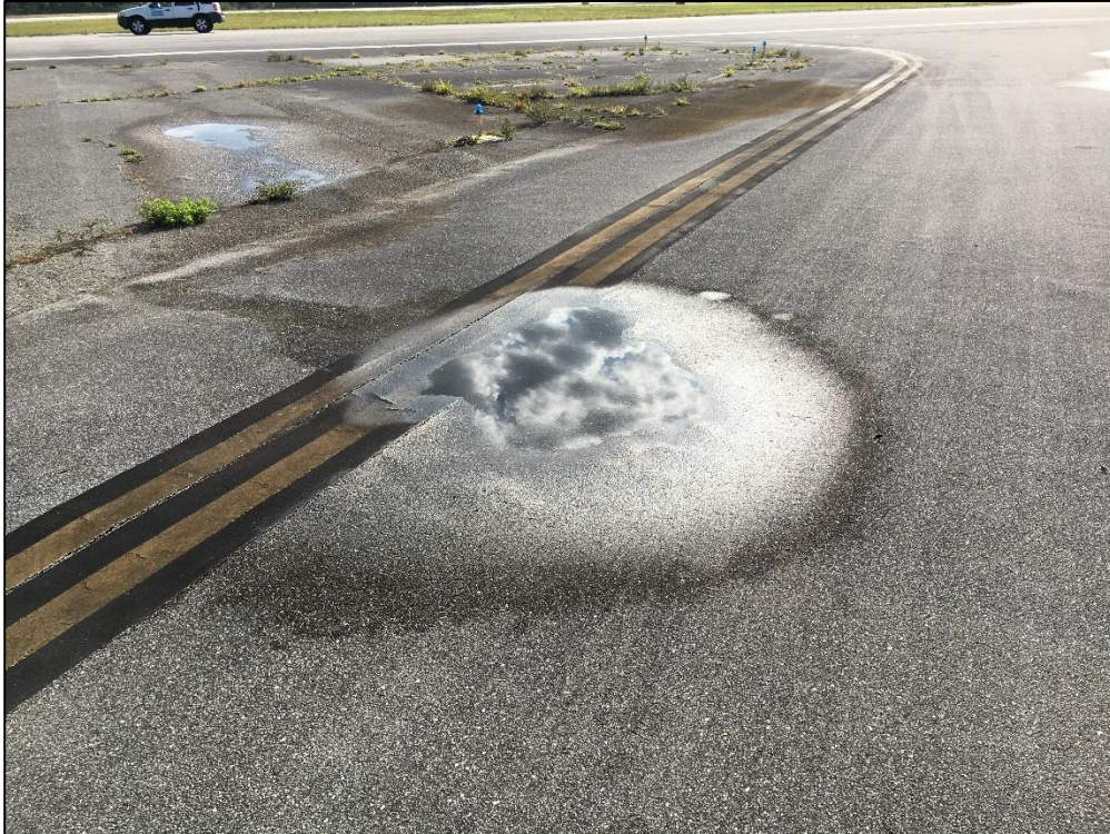
Taxiway A, Section 104, Sample Unit 139 - Low Severity (45) Depression, Low Severity (57) Weathering
