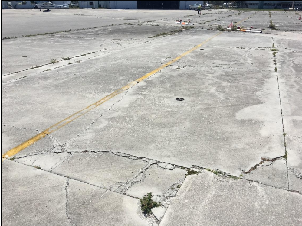
Center Apron, Section 4112, Sample Unit 303 - High Severity (72) Shattered Slab
