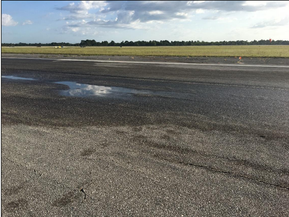
Runway 14-32, Section 6205, Sample Unit 163 - Low Severity (48) Longitudinal and Transverse Cracking, Low Severity (56) Swelling, Low Severity (57) Weathering
