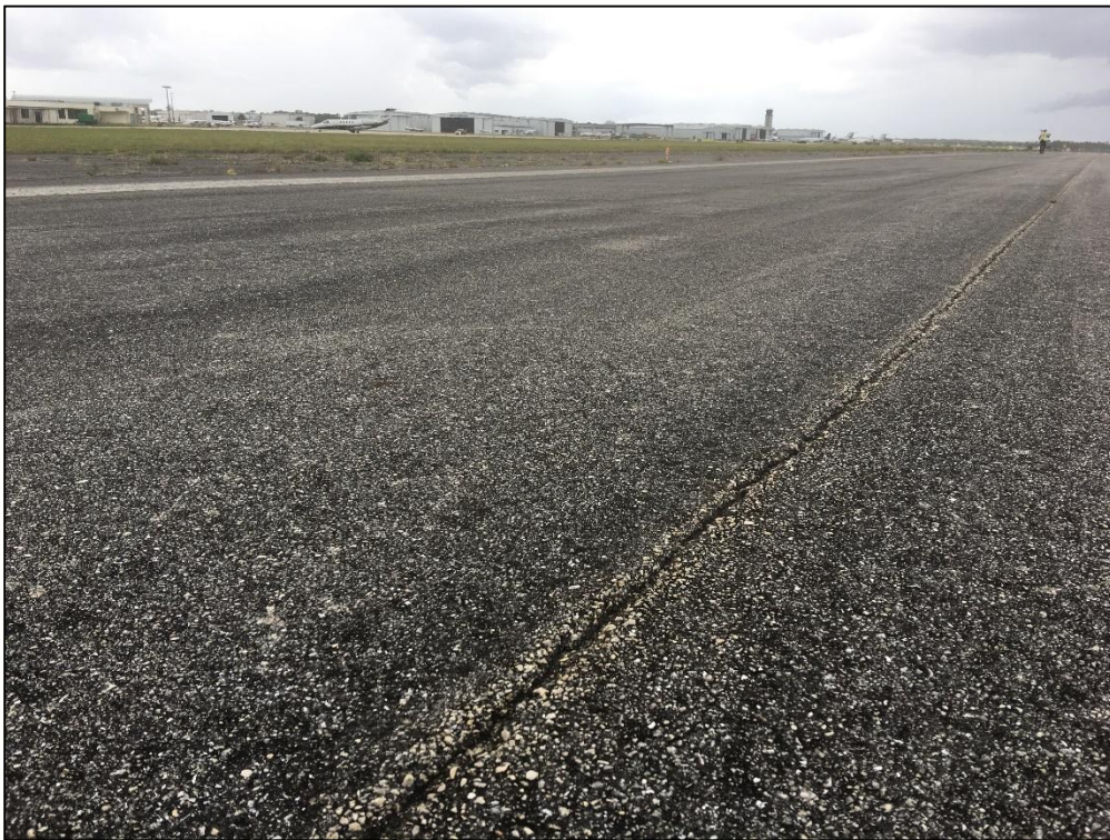
Runway 14-32, Section 6205, Sample Unit 114 - Medium Severity (48) Longitudinal and Transverse Cracking, Low Severity (52) Raveling, Low Severity (56) Swelling, Low Severity (57) Weathering
