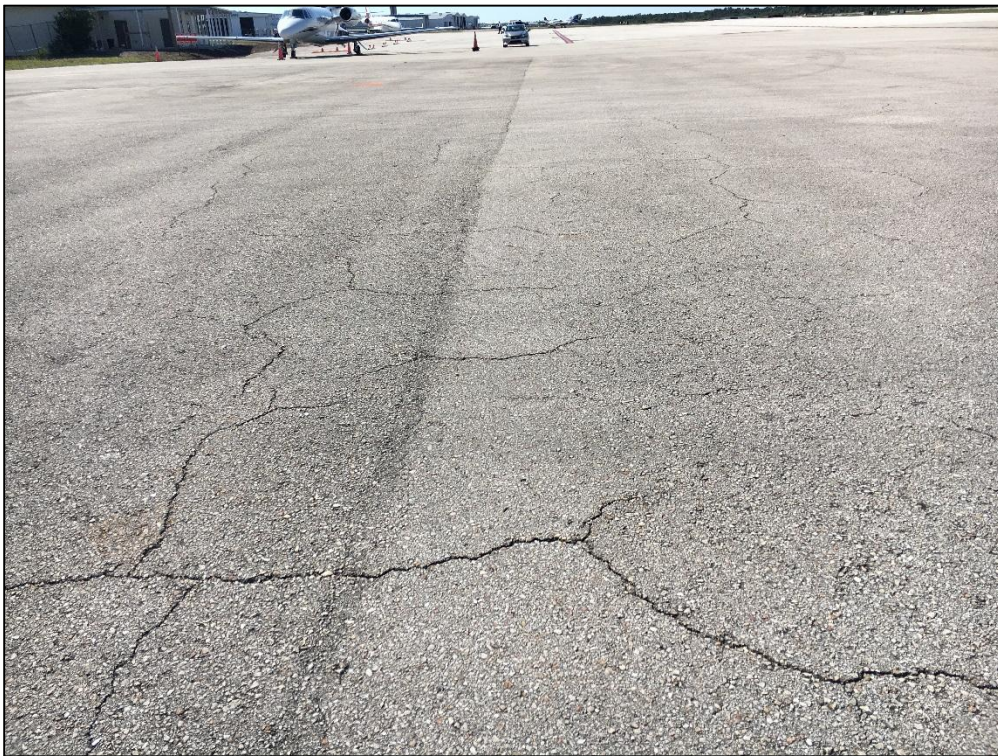
South Apron, Section 4220, Sample Unit 307 - Low Severity (43) Block Cracking, Low Severity (56) Swelling, Low Severity (57) Weathering
