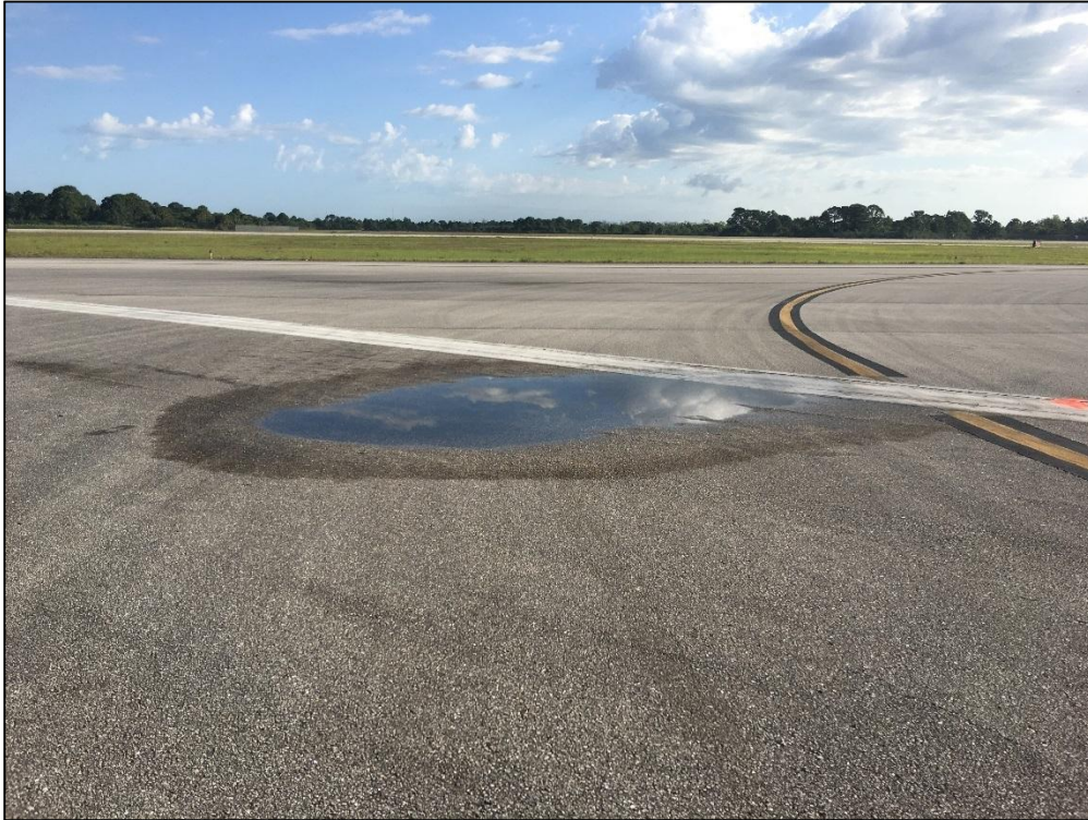
Runway 14-32, Section 6205, Sample Unit 182 - Medium Severity (45) Depression, Low Severity (48) Longitudinal and Transverse Cracking, Low Severity (56) Swelling
