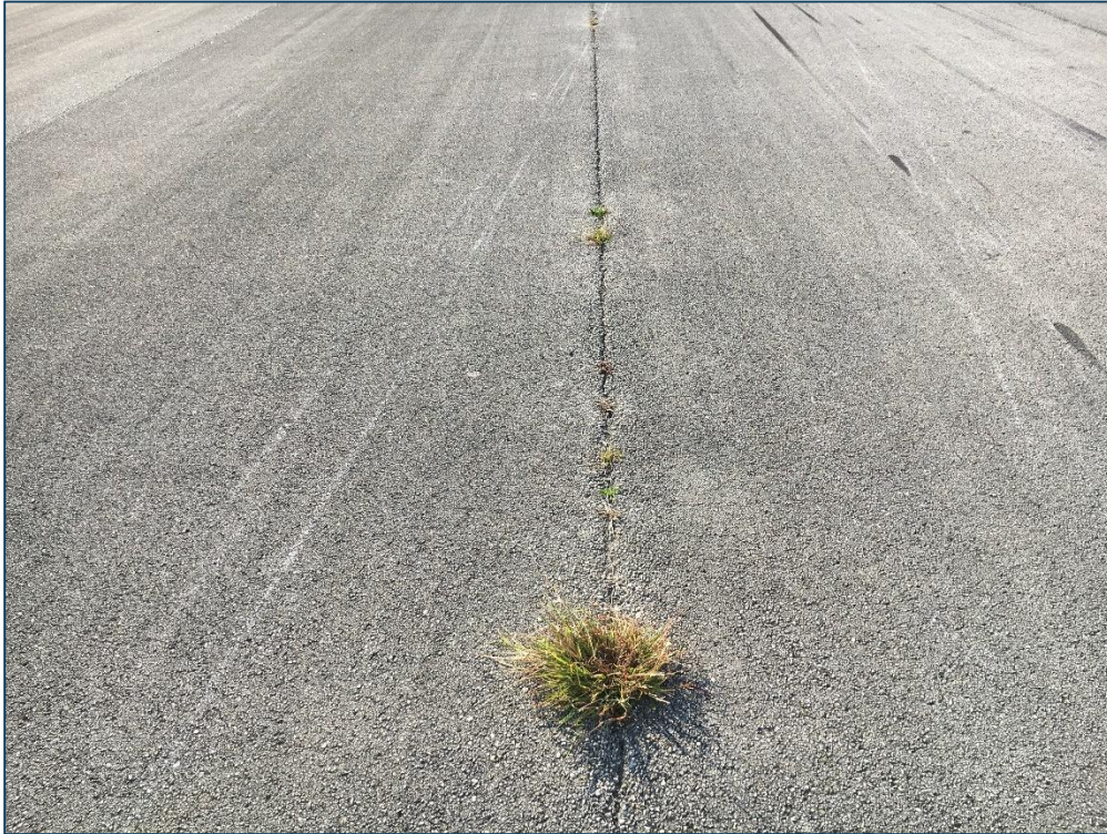
Runway 11-29, Section 6205, Sample Unit 163 – Medium Severity (48) Longitudinal and Transverse Cracking, Low Severity (52) Raveling, Low Severity (57) Weathering
