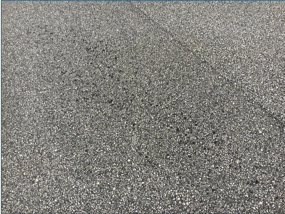
Taxiway B, Section 230, Sample Unit 105 – (42) Bleeding, Low Severity (48) Longitudinal and Transverse Cracking, Low Severity (52) Raveling, Low Severity (57) Weathering
