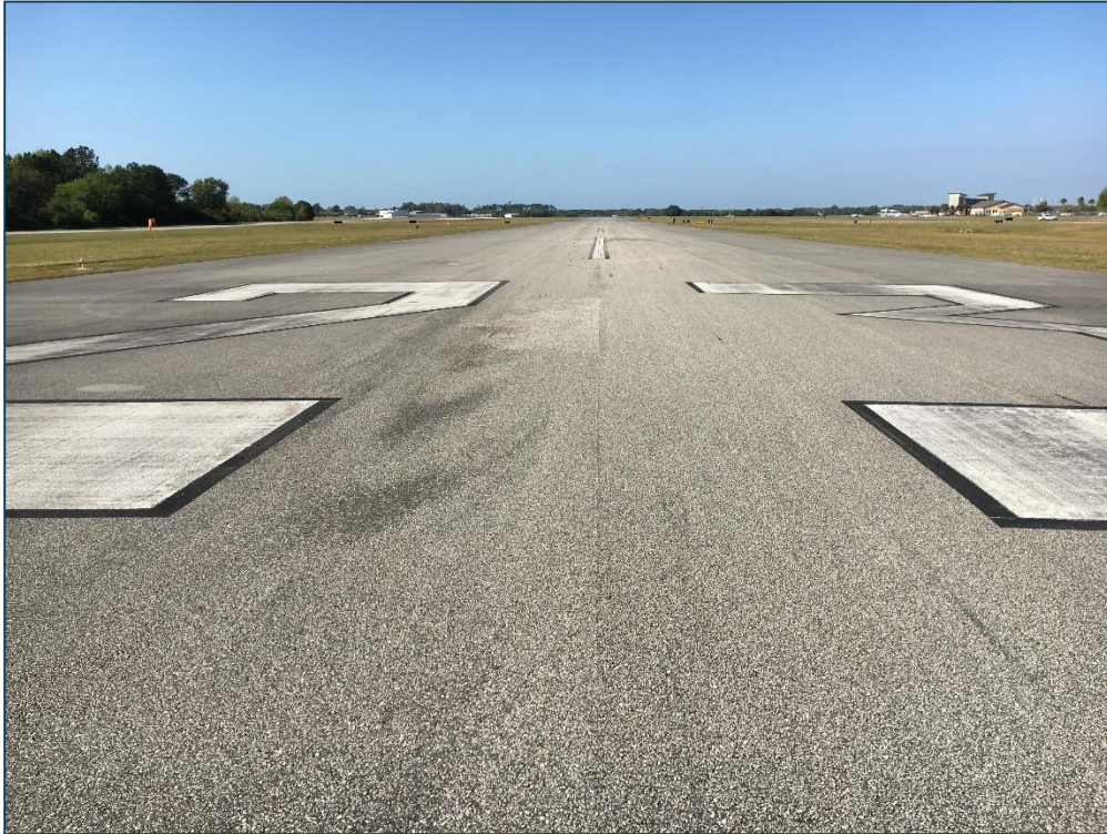
Runway 5-23, Section 6115, Sample Unit 147 – Low Severity (48) Longitudinal and Transverse Cracking, Low Severity (52) Raveling, Low Severity (57) Weathering
