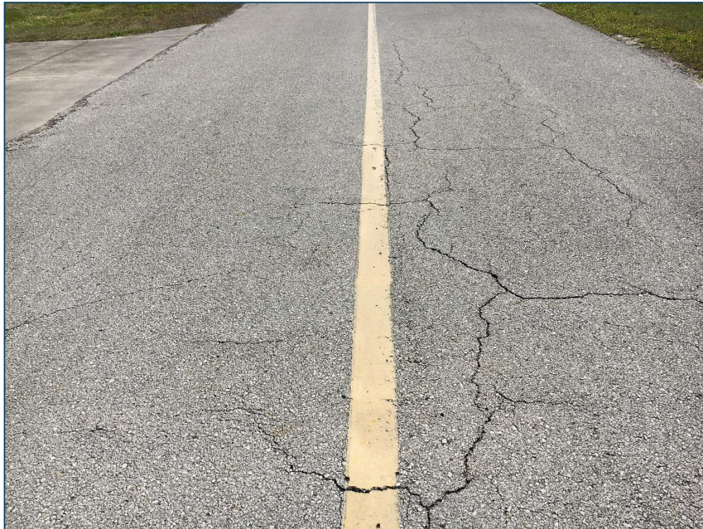
Apron T-Hangars, Section 4205, Sample Unit 454 – Low Severity (43) Block Cracking, Low Severity (48) Longitudinal and Transverse Cracking, Low Severity (52) Raveling, Medium Severity (52) Raveling, Low Severity (54) Shoving, Low Severity (56) Swelling
