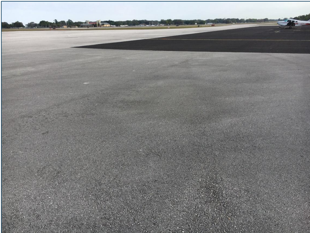
Apron, Section 4110, Sample Unit 255 – (42) Bleeding, Low Severity (45) Depression, Low Severity (48) Longitudinal and Transverse Cracking, Low Severity (52) Raveling, Low Severity (56) Swelling, Low Severity (57) Weathering
