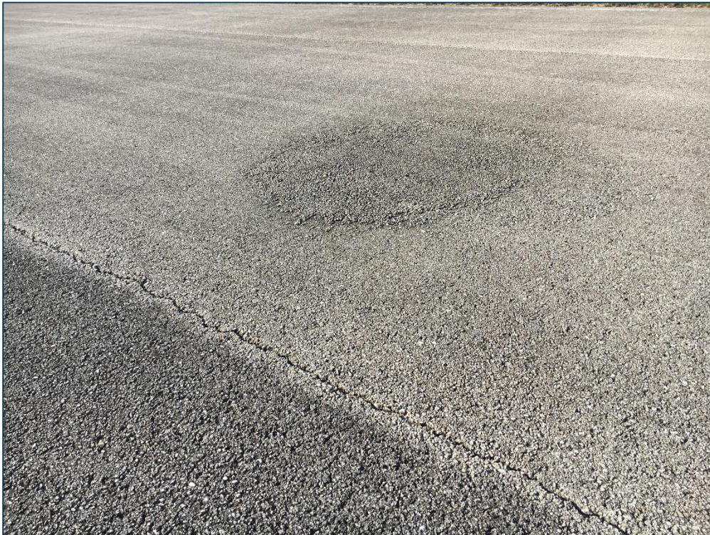
Runway 11-29, Section 6205, Sample Unit 151 – Low Severity (45) Depression, Low Severity (48) Longitudinal and Transverse Cracking, Low Severity (52) Raveling, Low Severity (57) Weathering
