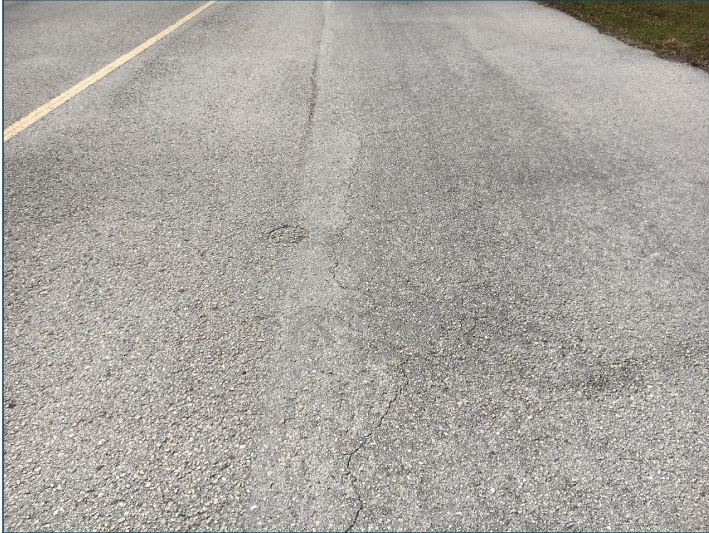
Taxiway B, Section 215, Sample Unit 111 – Low Severity (48) Longitudinal and Transverse Cracking, Medium Severity (52) Raveling, High Severity (52) Raveling
