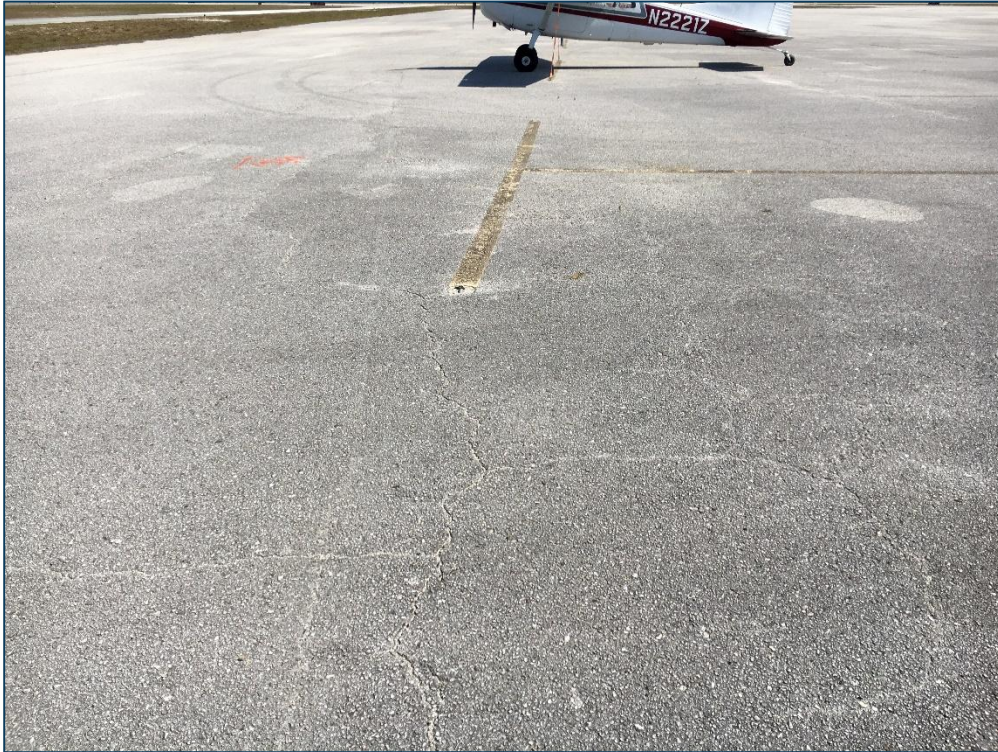
Apron, Section 4105, Sample Unit 154 – Low Severity (43) Block Cracking, Low Severity (48) Longitudinal and Transverse Cracking, Low Severity (52) Raveling, Medium Severity (52) Raveling
