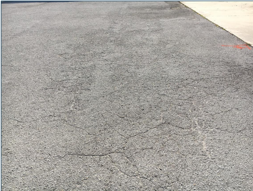
Apron, Section 4125, Sample Unit 101 – Low Severity (41) Alligator Cracking, Medium Severity (41) Alligator Cracking, Medium Severity (52) Raveling, High Severity (52) Raveling
