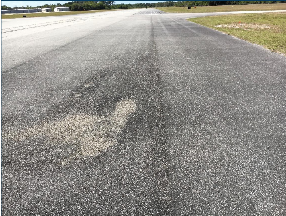
Runway 5-23, Section 6105, Sample Unit 114 – Low Severity (48) Longitudinal and Transverse Cracking, Low Severity (52) Raveling, Low Severity (57) Weathering
