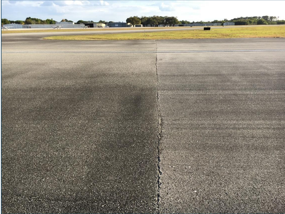
Runway 11-29, Section 6210, Sample Unit 136 – Low Severity (48) Longitudinal and Transverse Cracking, Low Severity (57) Weathering
