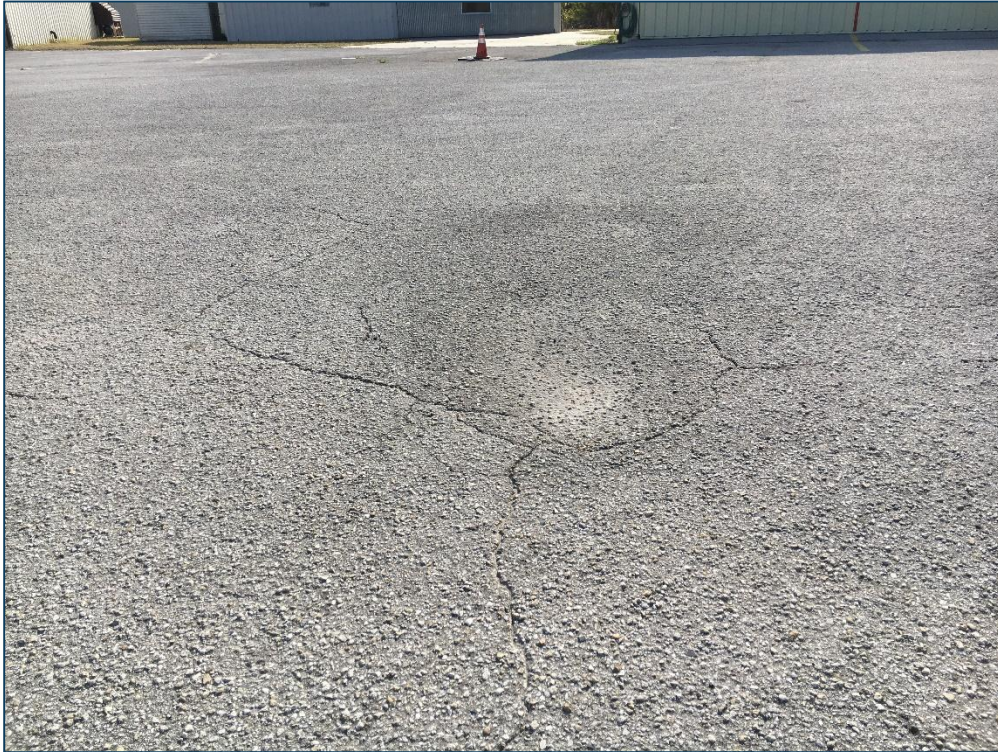
Apron, Section 4125, Sample Unit 101 – Low Severity (45) Depression, Medium Severity (45) Depression, Low Severity (48) Longitudinal and Transverse Cracking
