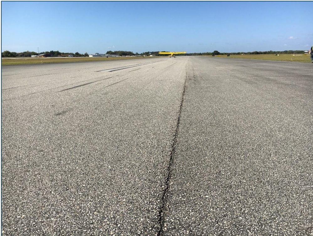
Runway 5-23, Section 6105, Sample Unit 135 – Low Severity (48) Longitudinal and Transverse Cracking, Low Severity (52) Raveling, Low Severity (57) Weathering
