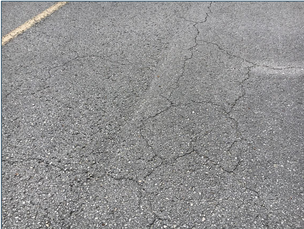
Taxiway B, Section 205, Sample Unit 204 – Low Severity (43) Block Cracking, Low Severity (48) Longitudinal and Transverse Cracking, Low Severity (52) Raveling, Medium Severity (52) Raveling
