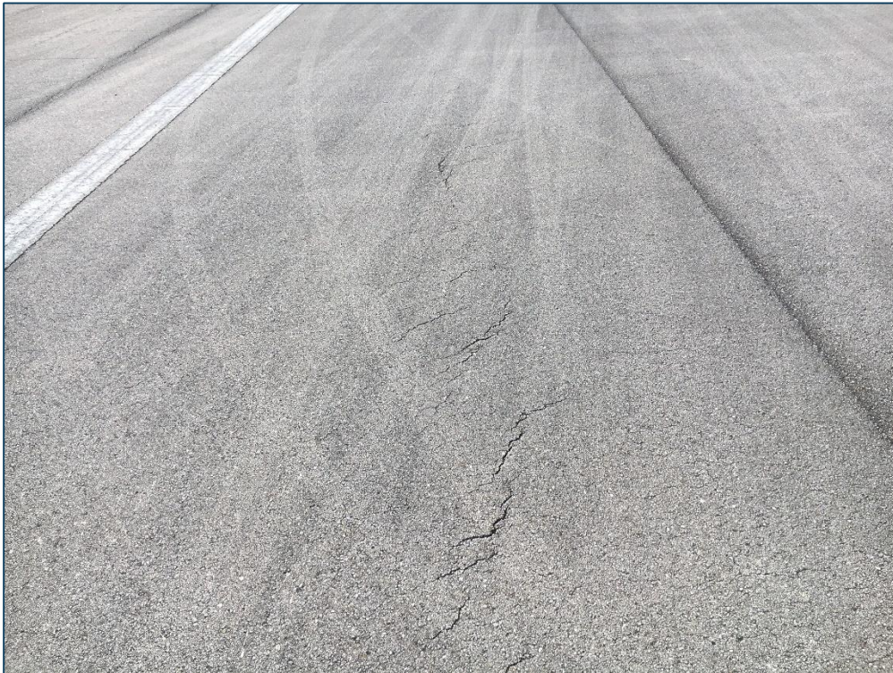
Runway 11-29, Section 6205, Sample Unit 103 – Low Severity (48) Longitudinal and Transverse Cracking, Low Severity (52) Raveling, Low Severity (57) Weathering
