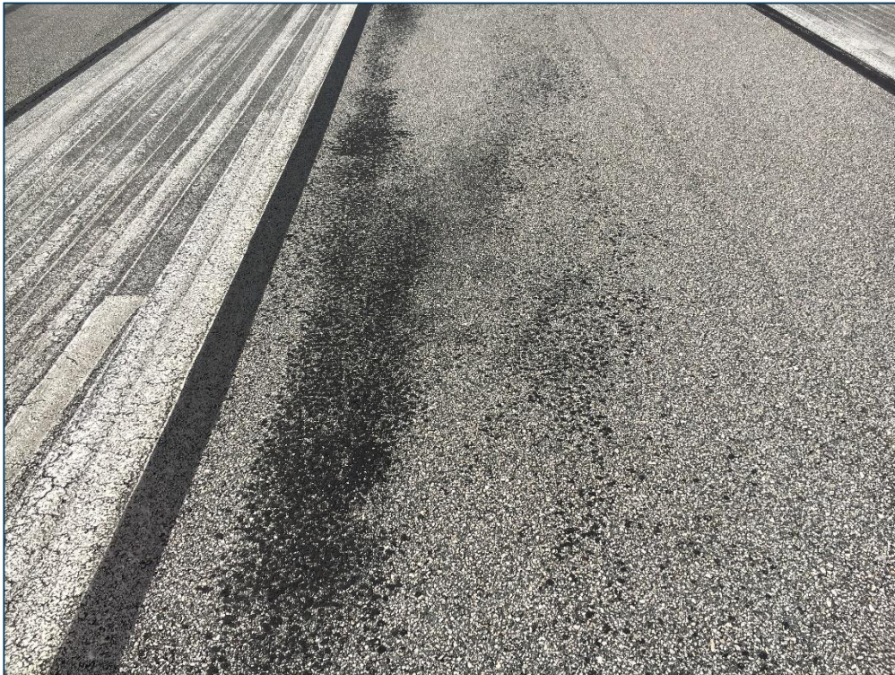
Runway 5-23, Section 6105, Sample Unit 101 – (42) Bleeding, Low Severity (48) Longitudinal and Transverse Cracking, Low Severity (52) Raveling, Low Severity (57) Weathering
