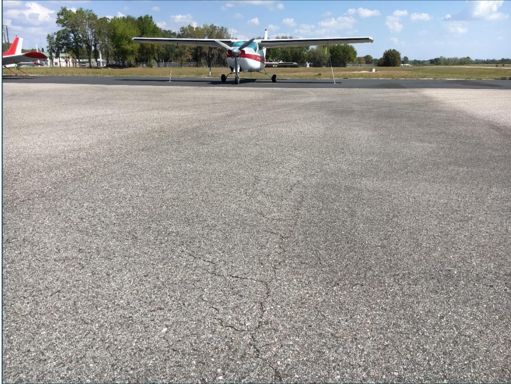
Apron North, Section 4505, Sample Unit 305 – Low Severity (48) Longitudinal and Transverse Cracking, Low Severity (52) Raveling, Low Severity (57) Weathering
