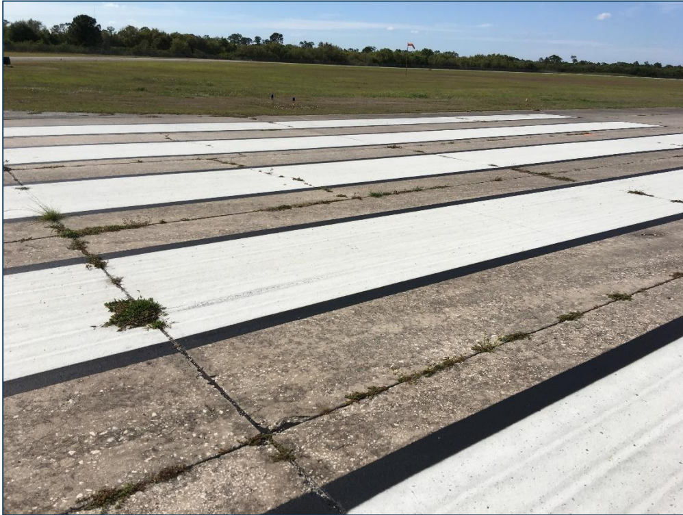
Runway 18-36, Section 6105, Sample Unit 301 – Medium Severity (63) Longitudinal, Transverse, and Diagonal Cracking, Medium Severity (65) Joint Seal Damage, Low Severity (74) Joint Spalling
