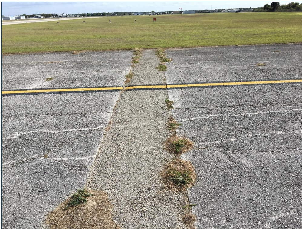
Taxiway A1, Section 210, Sample Unit 201– Low Severity (43) Block Cracking, High Severity (50) Patching, Medium Severity (52) Raveling
