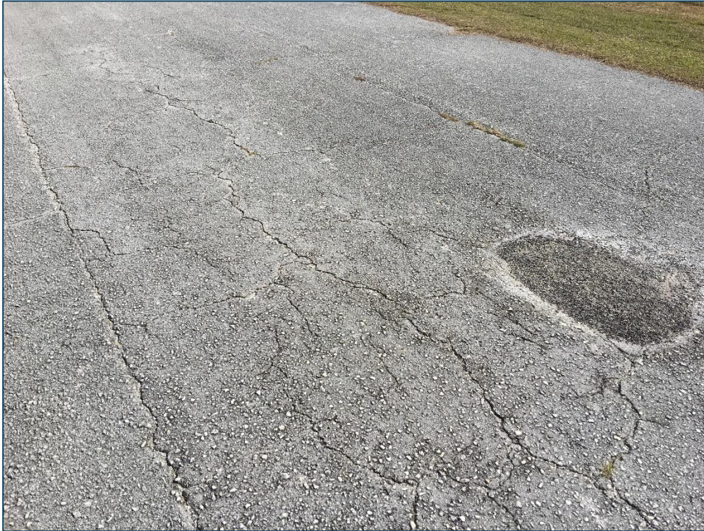
Taxiway A, Section 205, Sample Unit 103 – Low Severity (43) Block Cracking, Medium Severity (43) Block Cracking, High Severity (50) Patching, Medium Severity (52) Raveling
