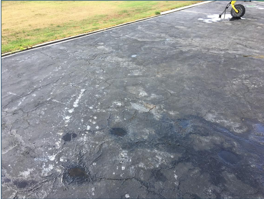
Crop Apron, Section 4105, Sample Unit 201 – Low Severity (43) Block Cracking, Low Severity (45) Depression, Low Severity (56) Swelling
