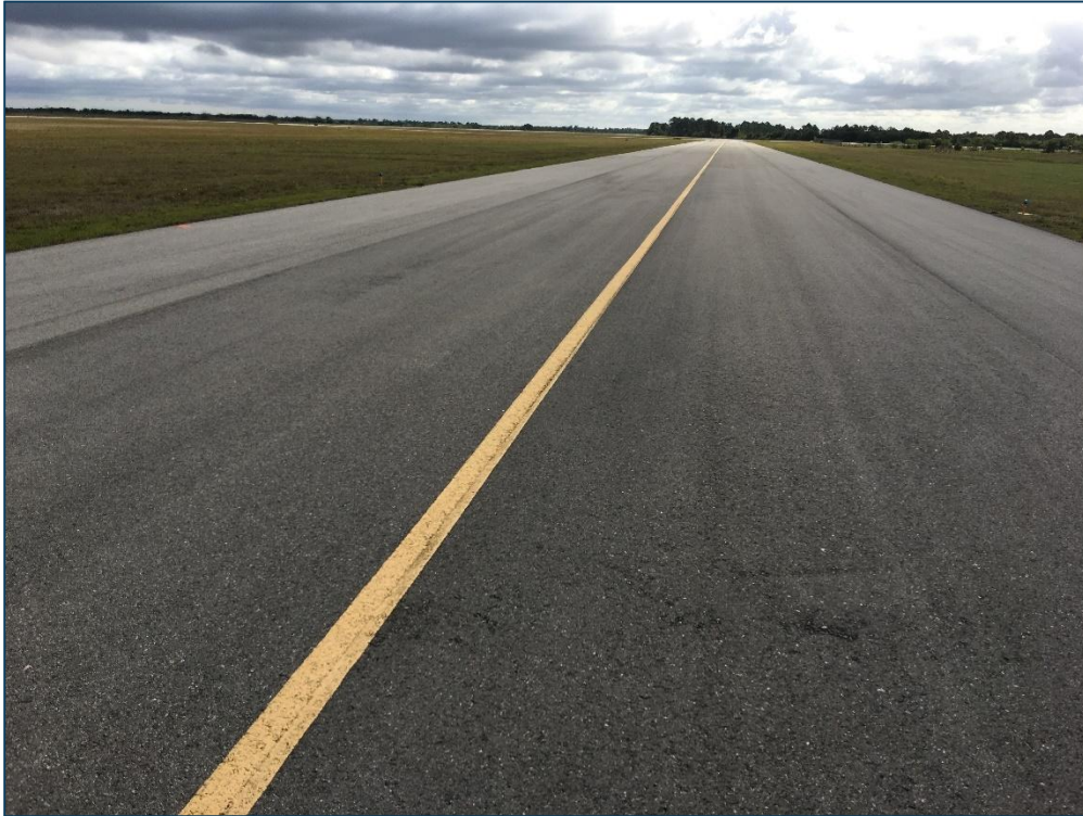
Taxiway B, Section 105, Sample Unit 105 – Low Severity (57) Weathering
