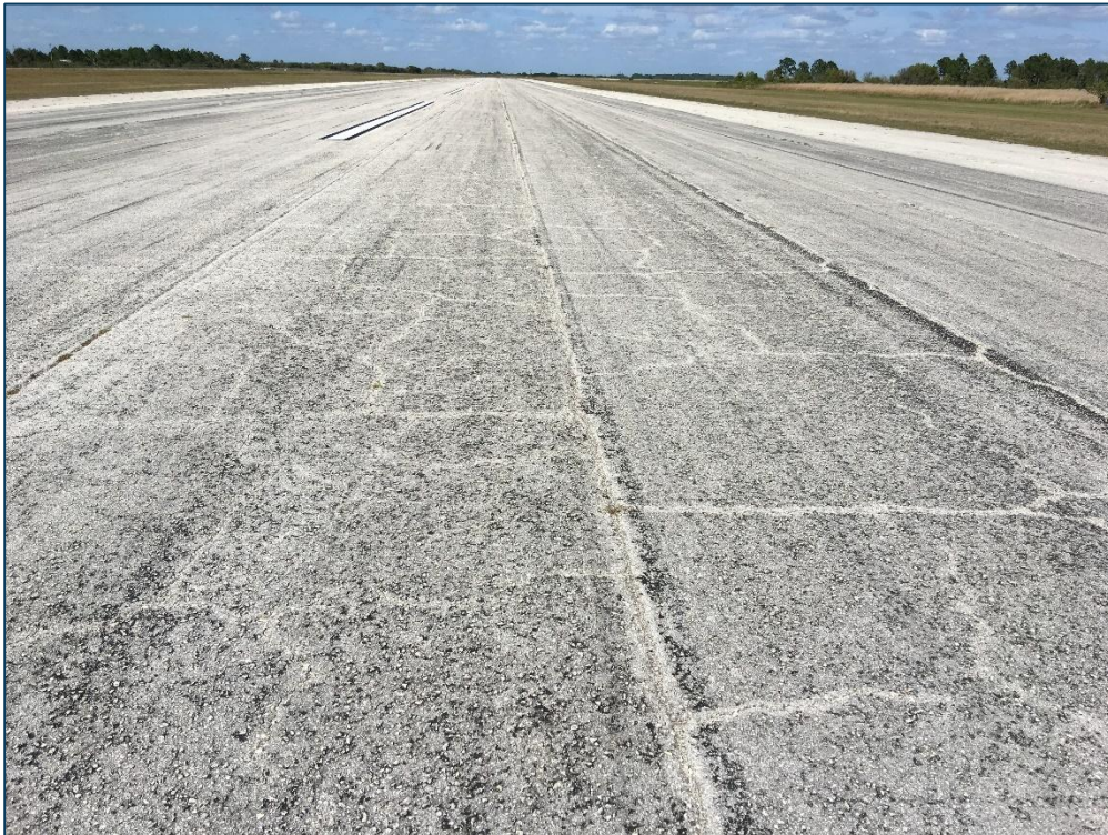
Runway 18-36, Section 6115, Sample Unit 324 – Medium Severity (43) Block Cracking, Low and Medium Severity (48) Longitudinal and Transverse Cracking, Medium Severity (52) Raveling
