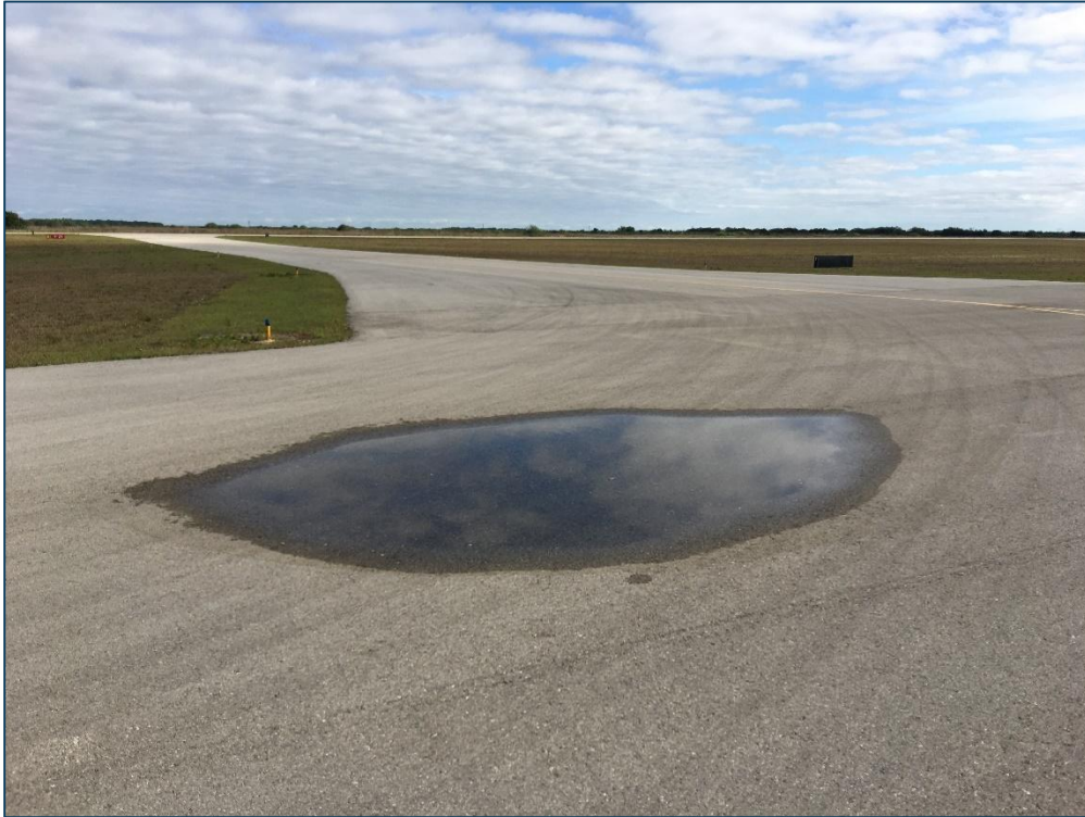
Taxiway B, Section 110, Sample Unit 119 – Depression. Sample Unit not inspected.
