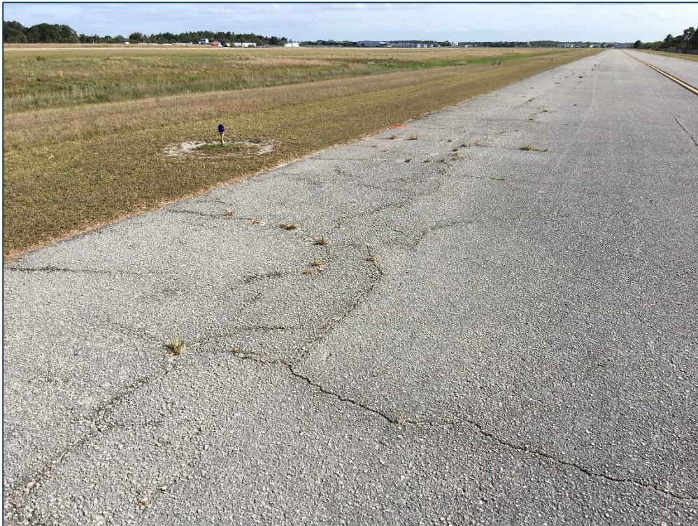
Taxiway A, Section 205, Sample Unit 133 – Low Severity (43) Block Cracking, Medium Severity (43) Block Cracking, Medium Severity (48) Longitudinal and Transverse Cracking, Medium Severity (52) Raveling
