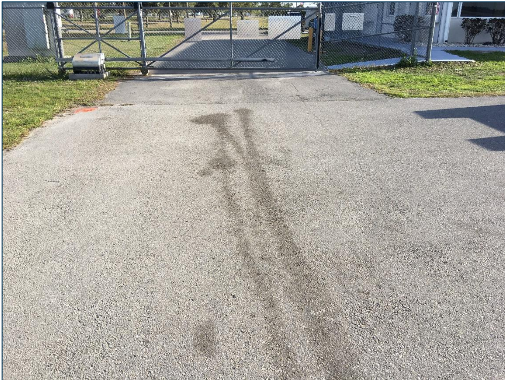
South Apron, Section 4205, Sample Unit 300 – Low Severity (48) Longitudinal and Transverse Cracking, (49) Oil Spillage, Low Severity (52) Raveling, Low Severity (57) Weathering
