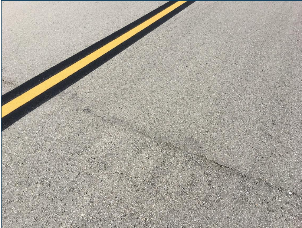
Taxiway A, Section 207, Sample Unit 145 – Low Severity (57) Weathering
