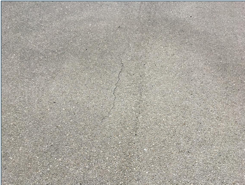
Apron to Hangars, Section 4405, Sample Unit 200 – Low Severity (48) Longitudinal and Transverse Cracking, Low Severity (52) Raveling, Low Severity (57) Weathering
