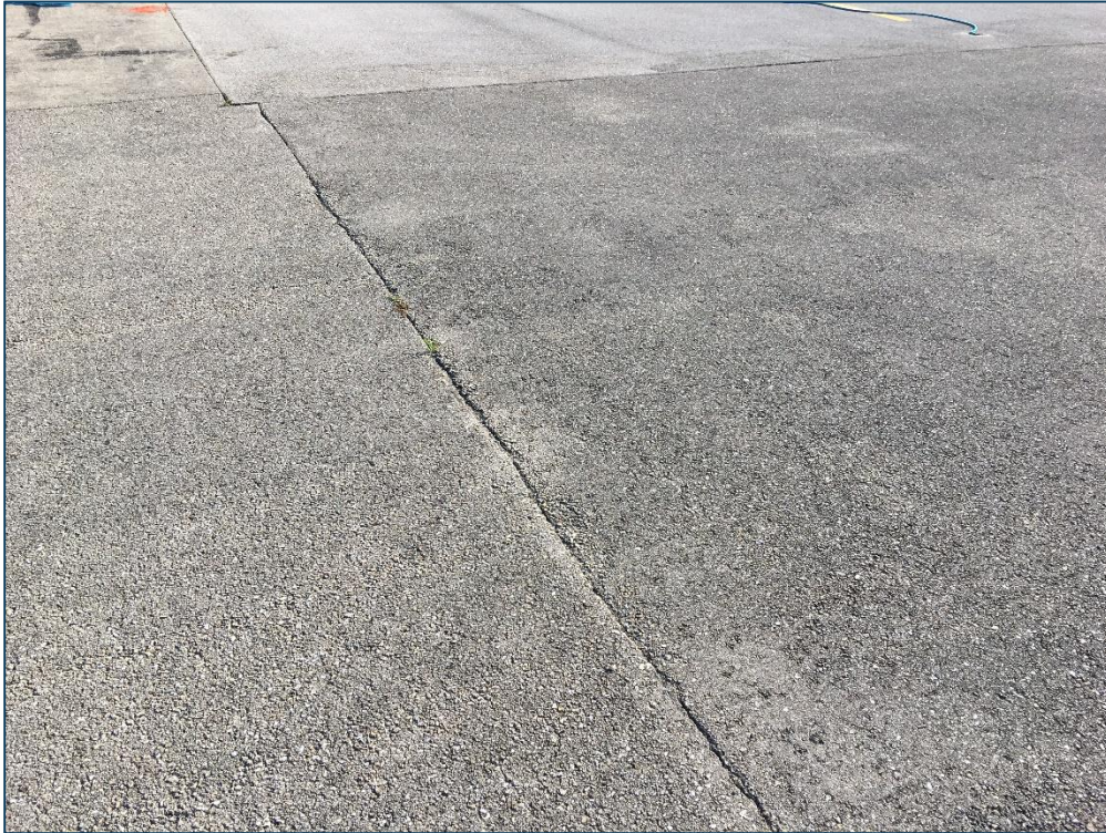
South Apron, Section 4210, Sample Unit 104 – Low Severity (48) Longitudinal and Transverse Cracking, Low Severity (50) Patching, Low Severity (52) Raveling, Low Severity (57) Weathering
