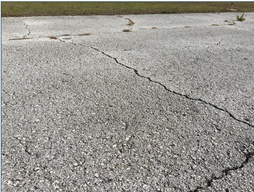
Taxiway B, Section 110, Sample Unit 117 – Low Severity (43) Block Cracking, Medium Severity (43) Block Cracking, Low Severity (48) Longitudinal and Transverse Cracking, Medium Severity (52) Raveling
