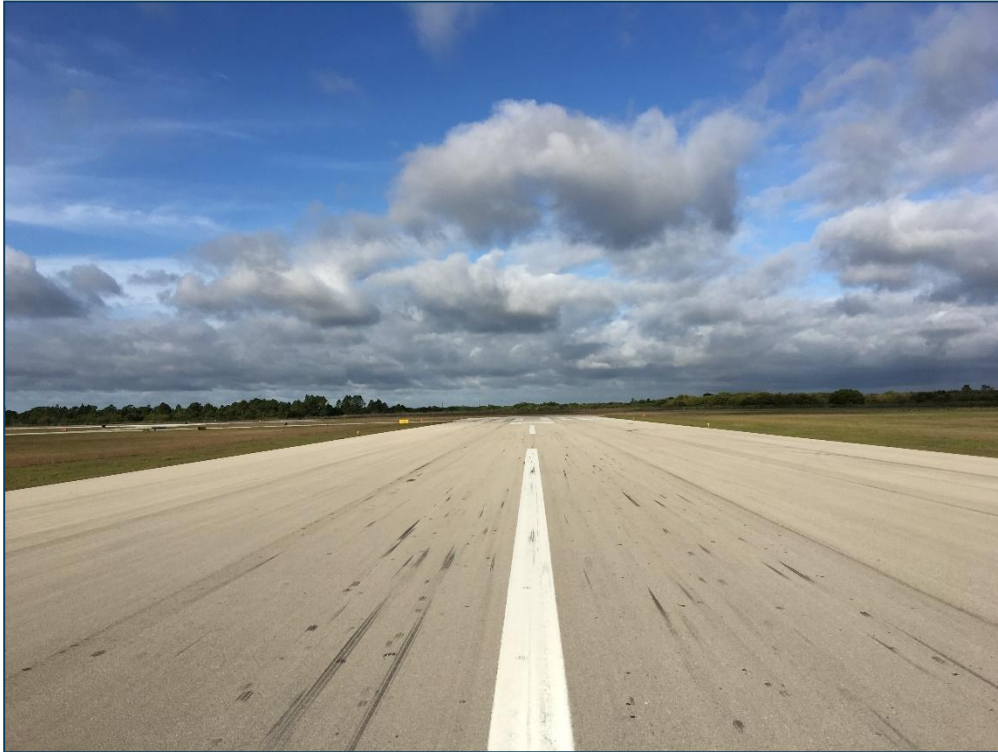
Runway 9-27, Section 6235, Sample Unit 312 – Low Severity (57) Weathering
