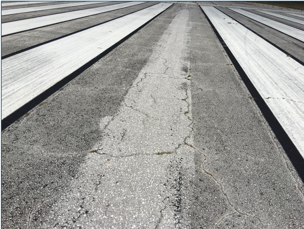
Runway 18-36, Section 6115, Sample Unit 383 – Medium Severity (43) Block Cracking, Low Severity (48) Longitudinal and Transverse Cracking, Medium Severity (52) Raveling
