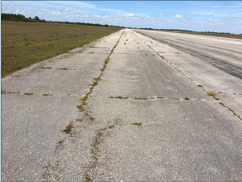
Runway 18-36, Section 6120, Sample Unit 150 – Low Severity (43) Block Cracking, Medium Severity (43) Block Cracking, Medium Severity (52) Raveling
