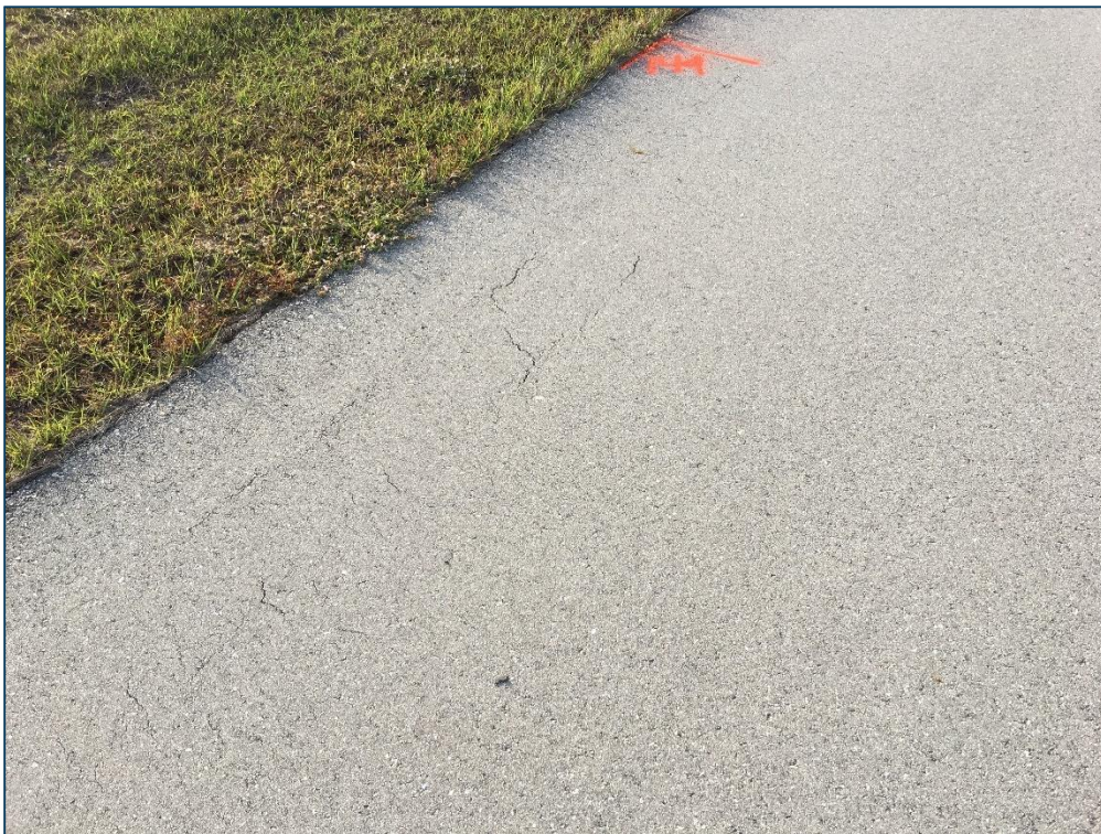
Taxiway B, Section 125, Sample Unit 149 – Low Severity (48) Longitudinal and Transverse Cracking, Low Severity (57) Weathering
