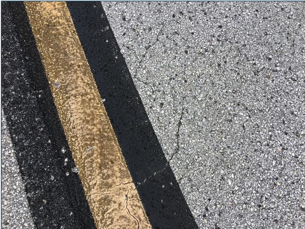
Taxilane to GA Apron, Section 205, Sample Unit 407 – Low Severity (48) Longitudinal and Transverse Cracking, Low Severity (52) Raveling
