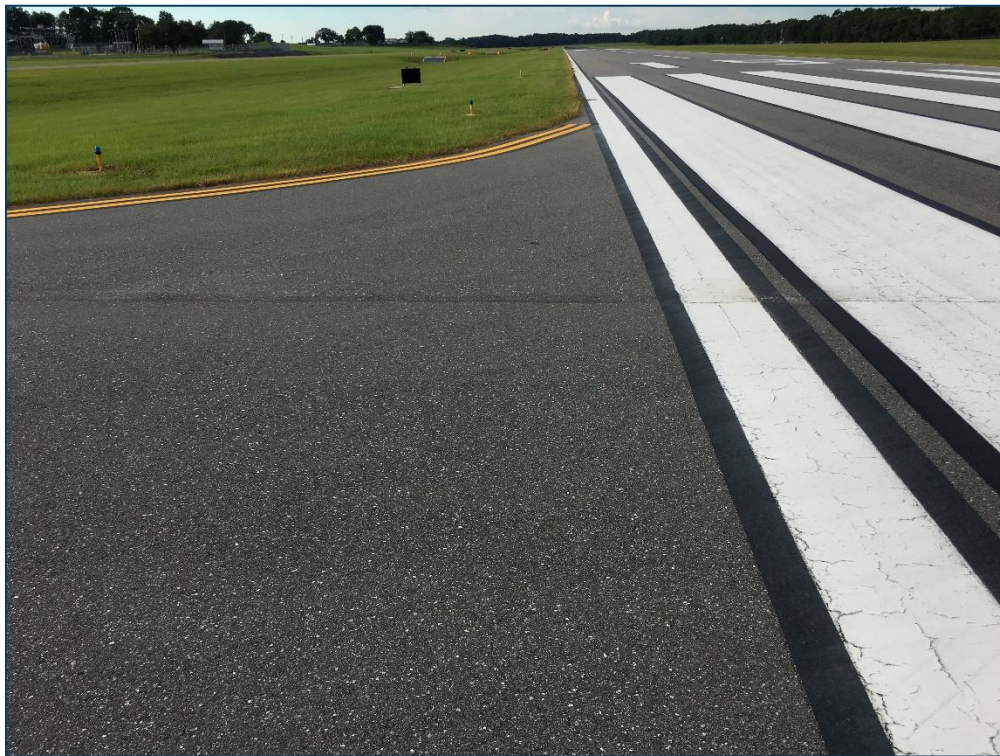
Taxiway A, Section 130, Sample Unit 500 – Low Severity (48) Longitudinal and Transverse Cracking, Low Severity (57) Weathering
