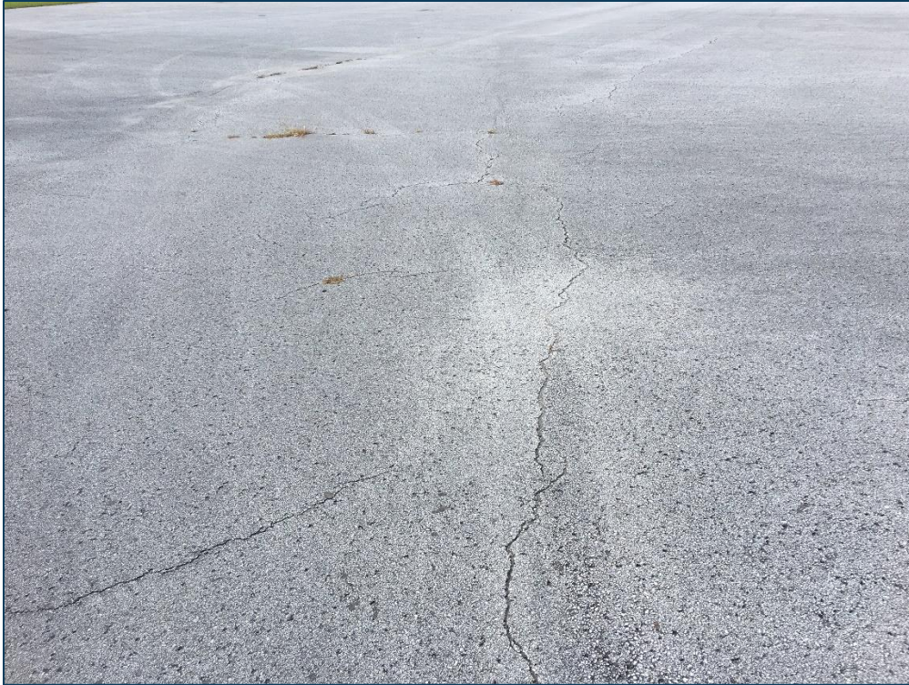
Apron GA, Section 4005, Sample Unit 604 – Low and Medium Severity (48) Longitudinal and Transverse Cracking, Low Severity (52) Raveling, Medium Severity (52) Raveling
