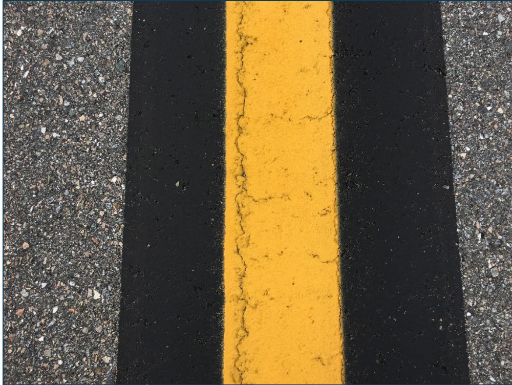
Taxiway A, Section 105, Sample Unit 127 – Low Severity (48) Longitudinal and Transverse Cracking, Low Severity (57) Weathering
