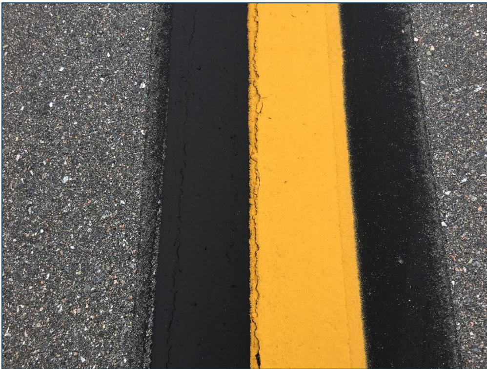
Taxiway A2, Section 120, Sample Unit 300 – Low Severity (48) Longitudinal and Transverse Cracking, Low Severity (57) Weathering
