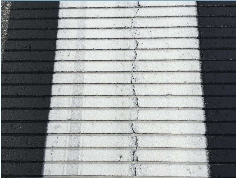
Runway 1-19, Section 6105, Sample Unit 139 – Low Severity (48) Longitudinal and Transverse Cracking, Low Severity (57) Weathering
