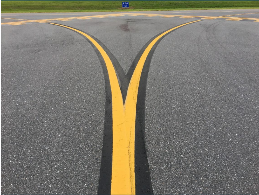
Taxiway A3, Section 125, Sample Unit 401 – Low Severity (57) Weathering
