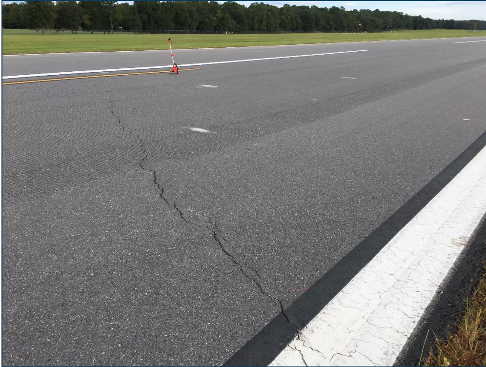
Runway 1-19, Section 6105, Sample Unit 131 – Low Severity (48) Longitudinal and Transverse Cracking, Low Severity (57) Weathering
