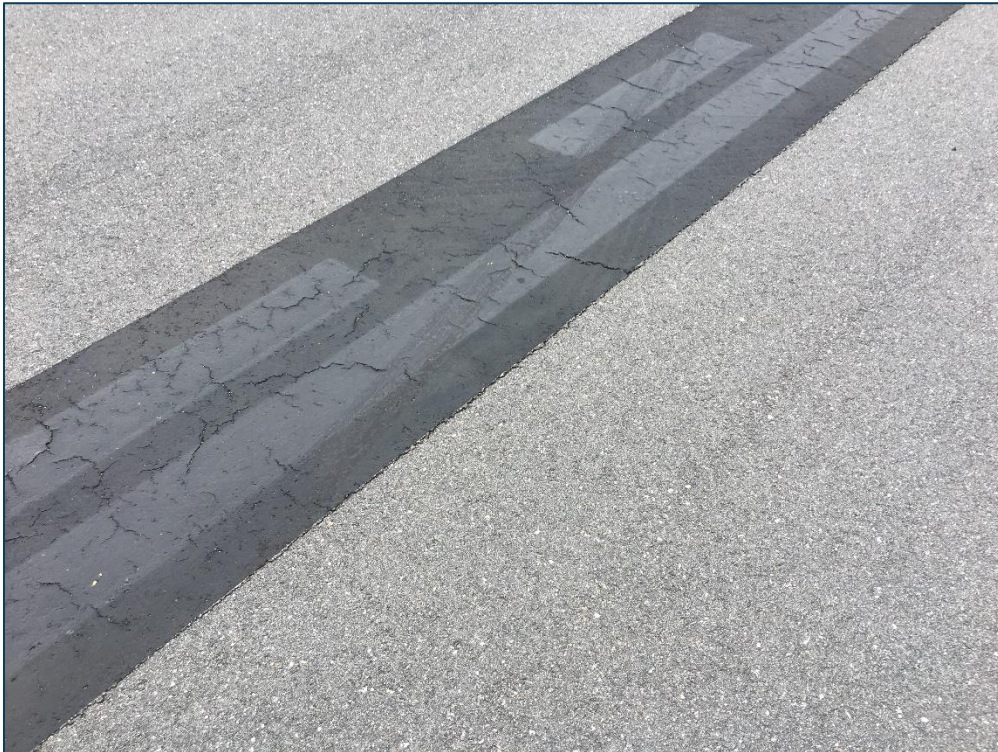
Apron FBO, Section 4210, Sample Unit 403 – Low Severity (48) Longitudinal and Transverse Cracking, Low Severity (57) Weathering
