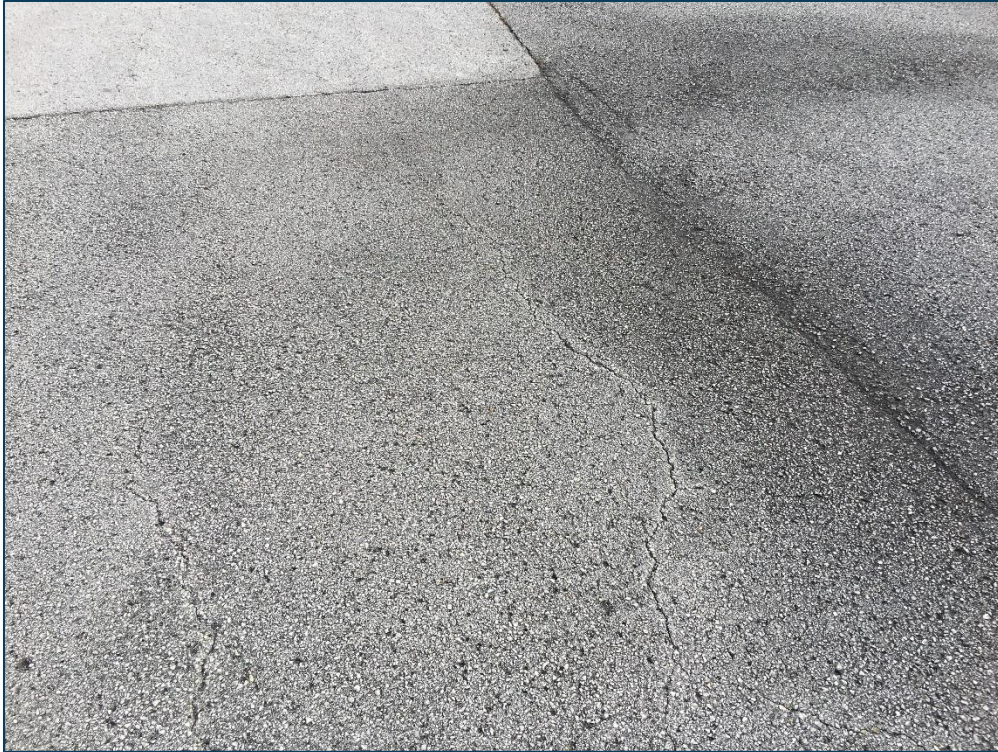
Taxilane to GA Apron, Section 205, Sample Unit 401 – Low Severity (48) Longitudinal and Transverse Cracking, Low Severity (52) Raveling
