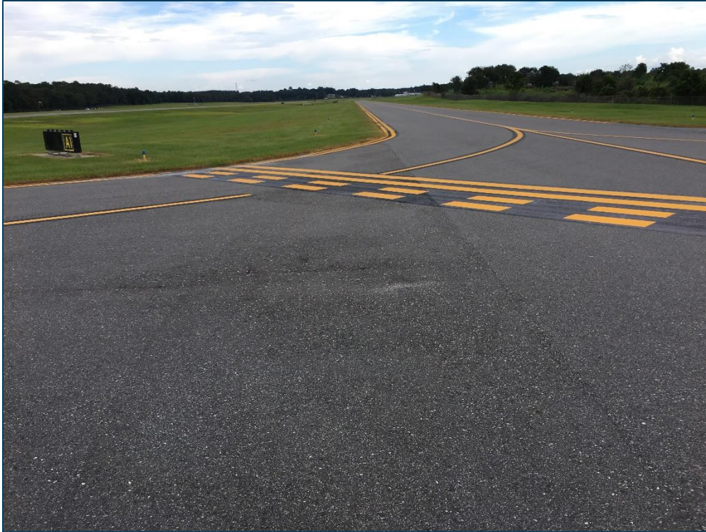
Taxiway A1, Section 115, Sample Unit 201 – Low Severity (45) Depression, Low Severity (57) Weathering
