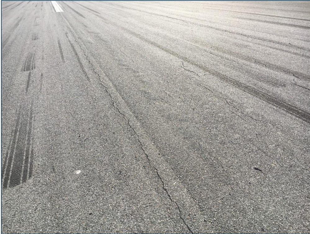
Runway 10-28, Section 6105, Sample Unit 321 – Low and Medium Severity (48) Longitudinal and Transverse Cracking, Low Severity (56) Swelling
