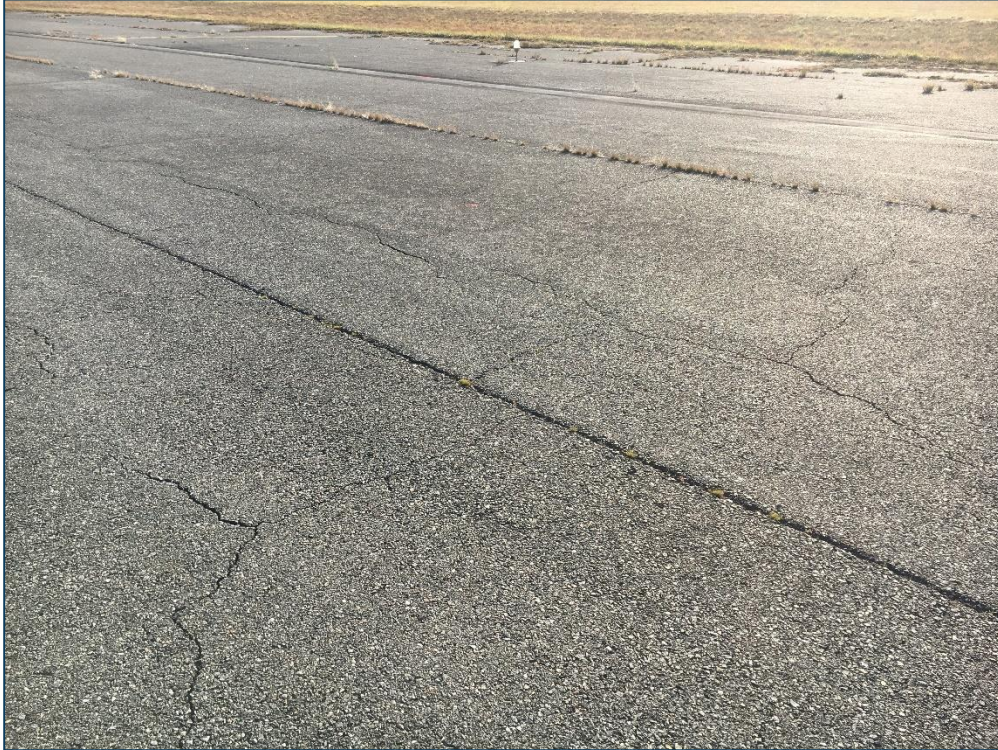
Runway 5-23, Section 6205, Sample Unit 122 – Low Severity (43) Block Cracking, Low and Medium Severity (48) Longitudinal and Transverse Cracking, Low Severity (52) Raveling, Low Severity (53) Rutting
