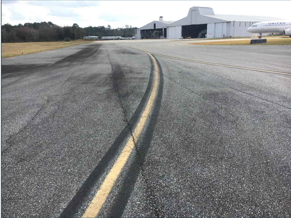
East Apron, Section 4215, Sample Unit 401 – Low and Medium Severity (48) Longitudinal and Transverse Cracking, Low Severity (52) Raveling, Medium Severity (52) Raveling
