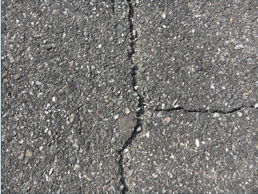
Apron RW 10-28, Section 5125, Sample Unit 202 – Low and Medium Severity (48) Longitudinal and Transverse Cracking, Low Severity (57) Weathering.
