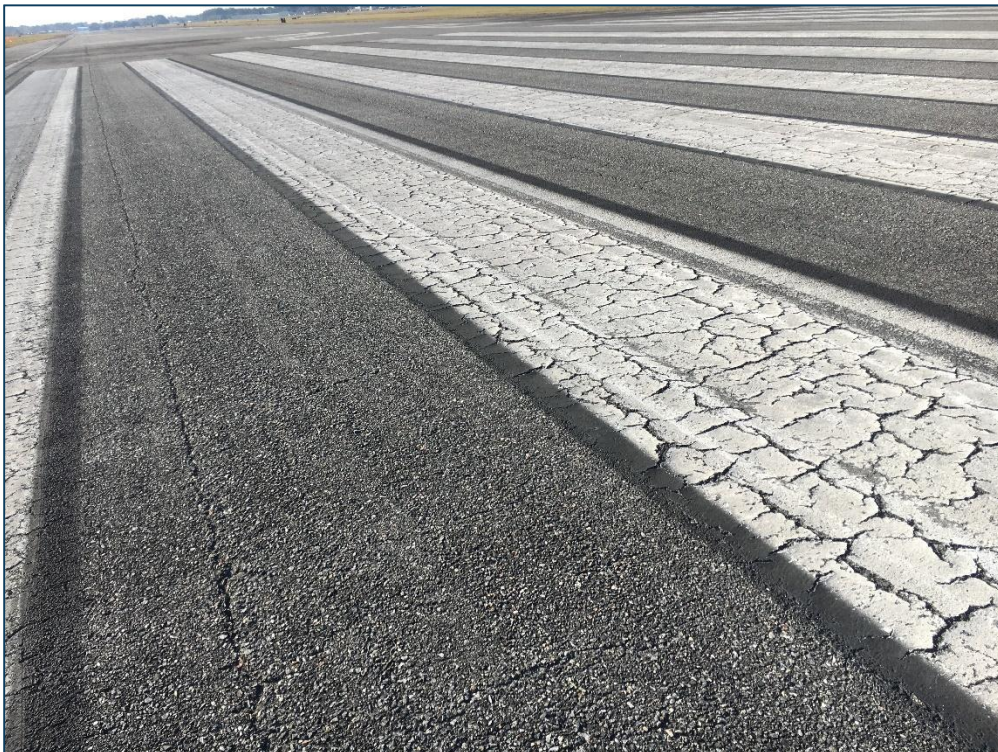
Runway 10-28, Section 6120, Sample Unit 656 – Low and Medium Severity (48) Longitudinal and Transverse Cracking, Low Severity (52) Raveling
