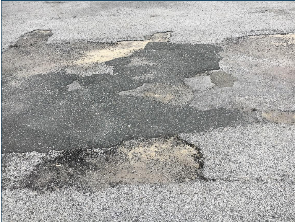
East Apron, Section 4228, Sample Unit 101 – Medium Severity (45) Depression, High Severity (50) Patching, High Severity (52) Raveling
