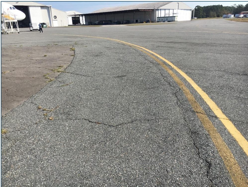
East Apron, Section 4230, Sample Unit 204 – Medium Severity (43) Block Cracking, Low and Medium Severity (48) Longitudinal and Transverse Cracking, Low Severity (52) Raveling
