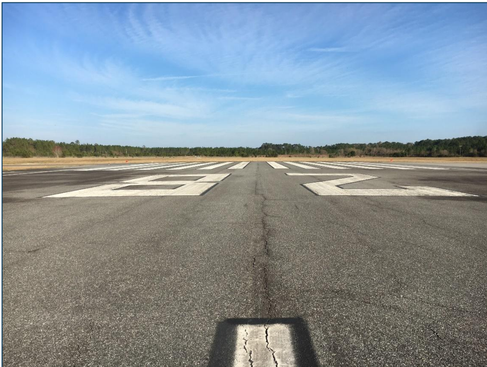
Runway 10-28, Section 6115, Sample Unit 453 – Low and Medium Severity (48) Longitudinal and Transverse Cracking, Low Severity (52) Raveling
