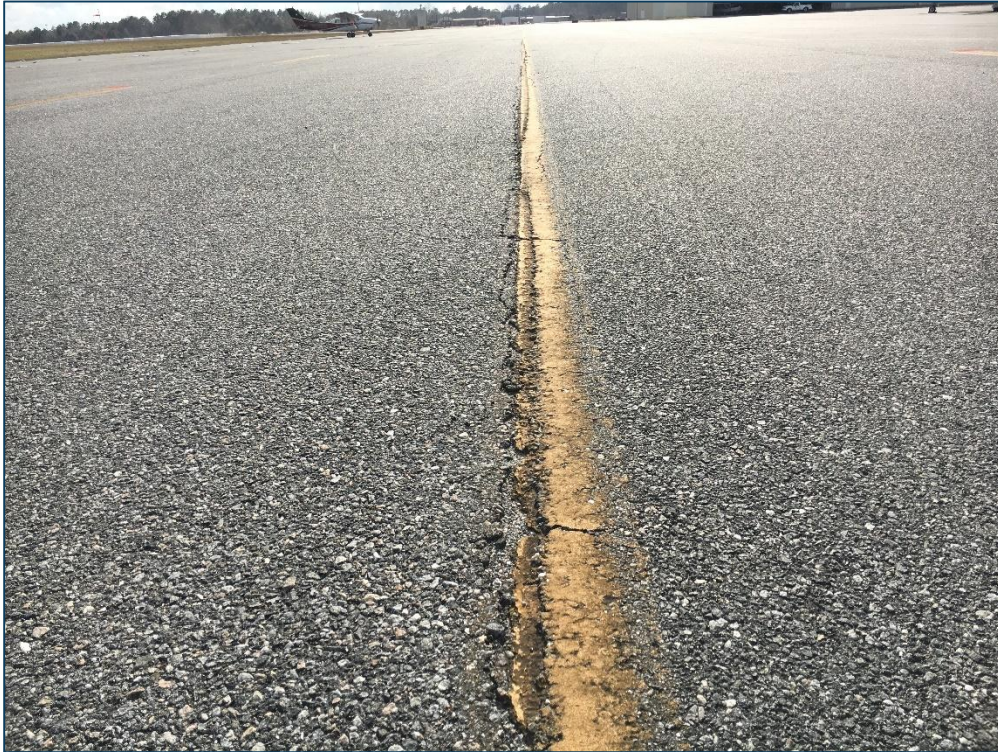
Taxiway C, Section 310, Sample Unit 116 – Low and Medium Severity (48) Longitudinal and Transverse Cracking, Low Severity (52) Raveling, Low Severity (57) Weathering
