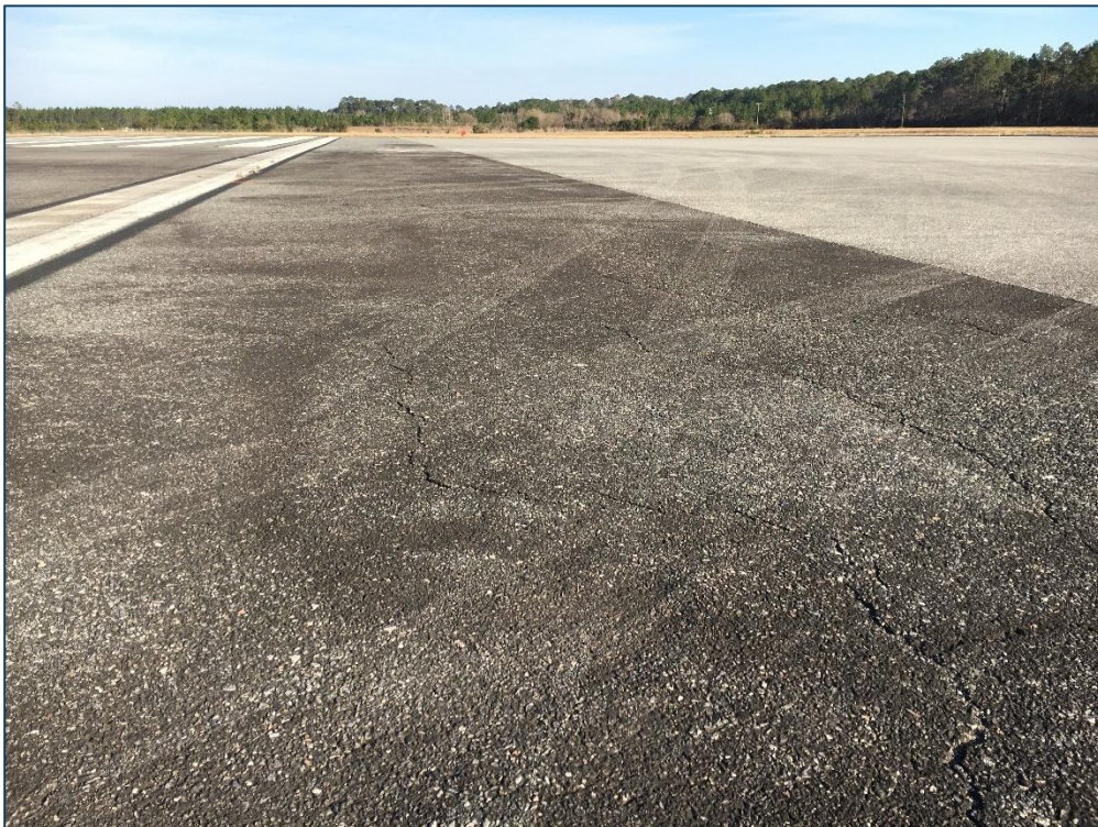
Apron RW 10-28, Section 5115, Sample Unit 105 – Low Severity (48) Longitudinal and Transverse Cracking, Low Severity (56) Swelling, Low Severity (57) Weathering.
