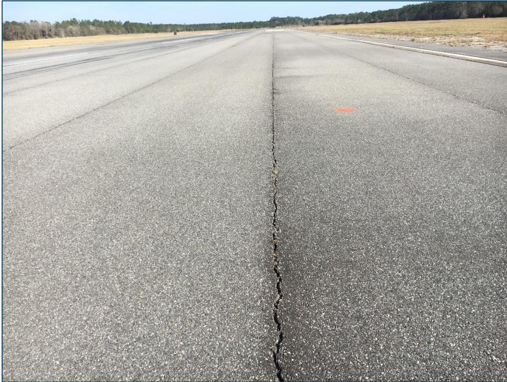
Runway 10-28, Section 6114, Sample Unit 423 – Low and Medium Severity (48) Longitudinal and Transverse Cracking, Low Severity (52) Raveling
