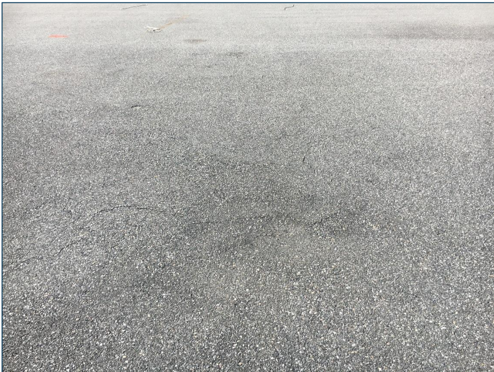
Apron NW, Section 4105, Sample Unit 813 – Low and Medium Severity (48) Longitudinal and Transverse Cracking, Low Severity (52) Raveling, Low Severity (56) Swelling, Low Severity (57) Weathering.
