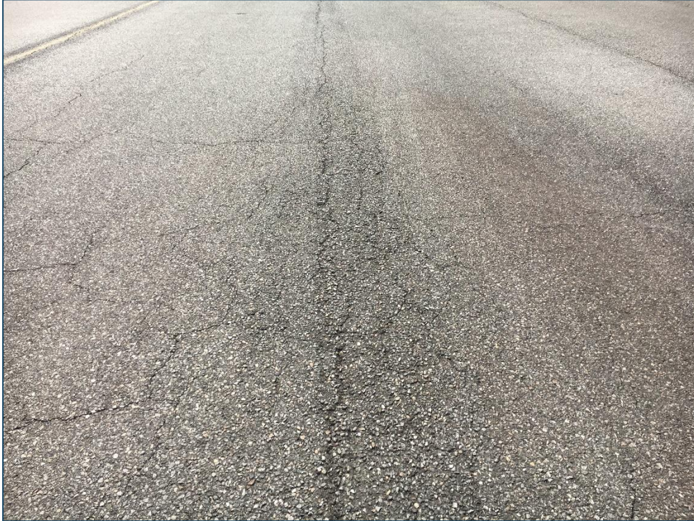
Taxiway D, Section 405, Sample Unit 100 – Low Severity (41) Alligator Cracking, Low Severity (43) Block Cracking, Low and Medium Severity (48) Longitudinal and Transverse Cracking, Low Severity (52) Raveling, Low Severity (53) Rutting
