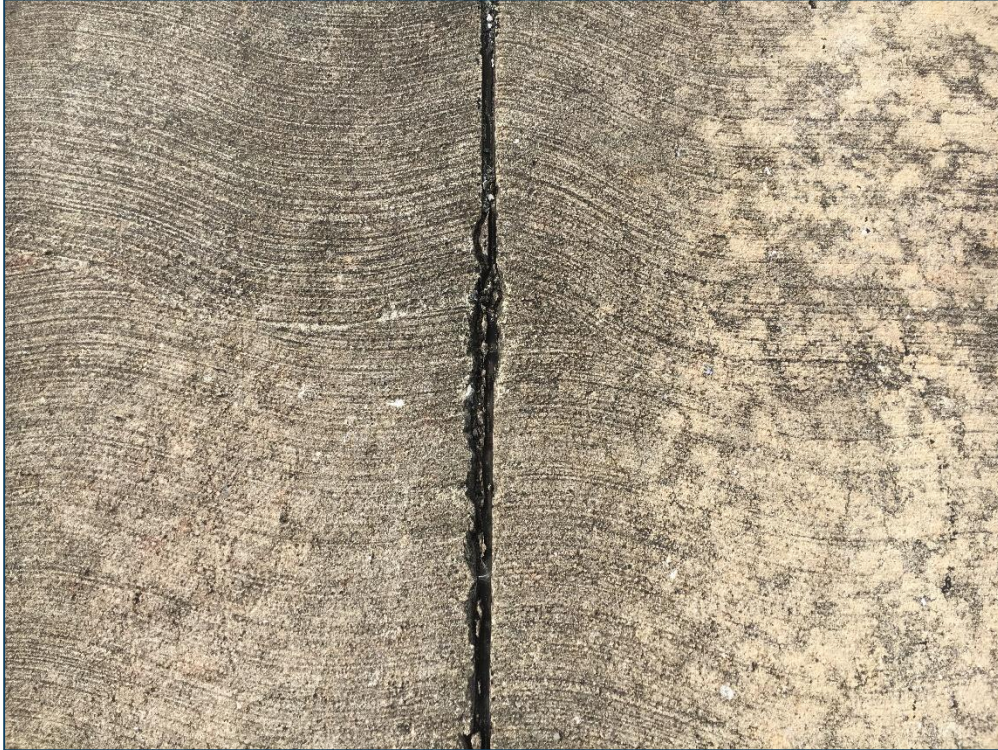
Apron SW, Section 5135, Sample Unit 101 – Medium Severity (65) Joint Seal Damage, (73) Shrinkage Cracks.
