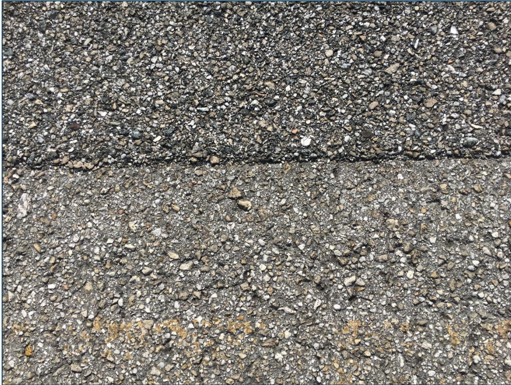
Taxilane T-Hang NW, Section 4125, Sample Unit 102 – Low Severity (48) Longitudinal and Transverse Cracking, Low Severity (52) Raveling, Medium Severity (52) Raveling
