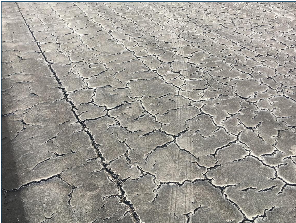
Runway 10-28, Section 6105, Sample Unit 321 – Low and Medium Severity (48) Longitudinal and Transverse Cracking, High Severity (52) Raveling
