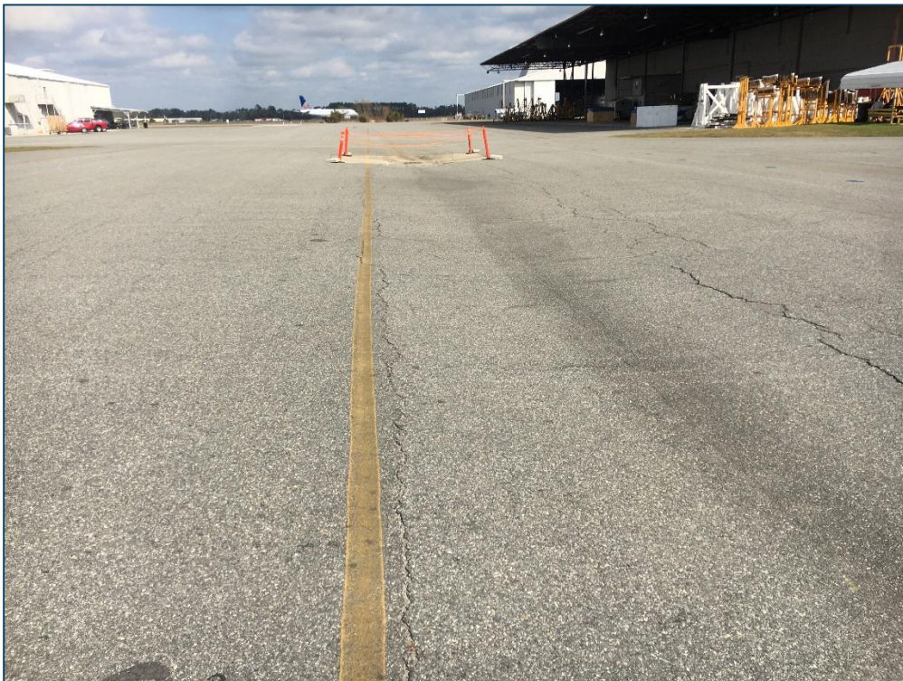
East Apron, Section 4205, Sample Unit 111 – High Severity (45) Depression, Low and Medium Severity (48) Longitudinal and Transverse Cracking, Low Severity (52) Raveling
