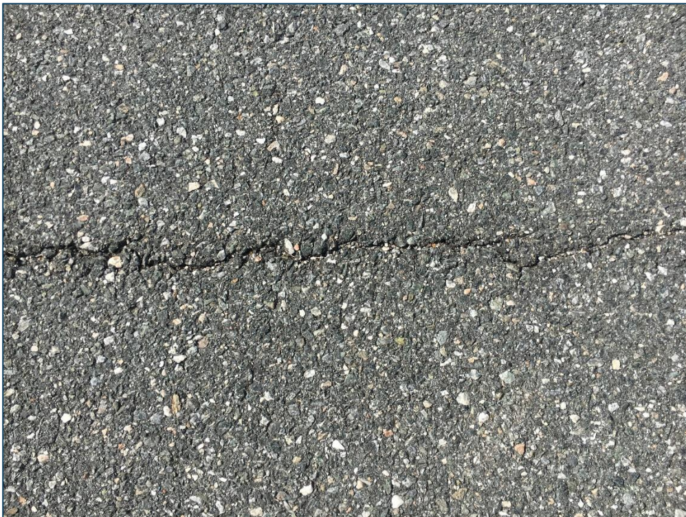
Taxiway A1, Section 140, Sample Unit 708 – Low Severity (48) Longitudinal and Transverse Cracking, Low Severity (52) Raveling, Low Severity (57) Weathering
