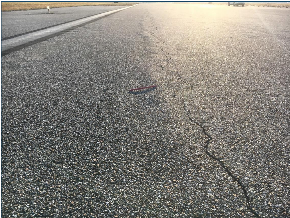
Runway 5-23, Section 6207, Sample Unit 155 – Low and Medium Severity (48) Longitudinal and Transverse Cracking, Low Severity (56) Swelling, Low Severity (57) Weathering
