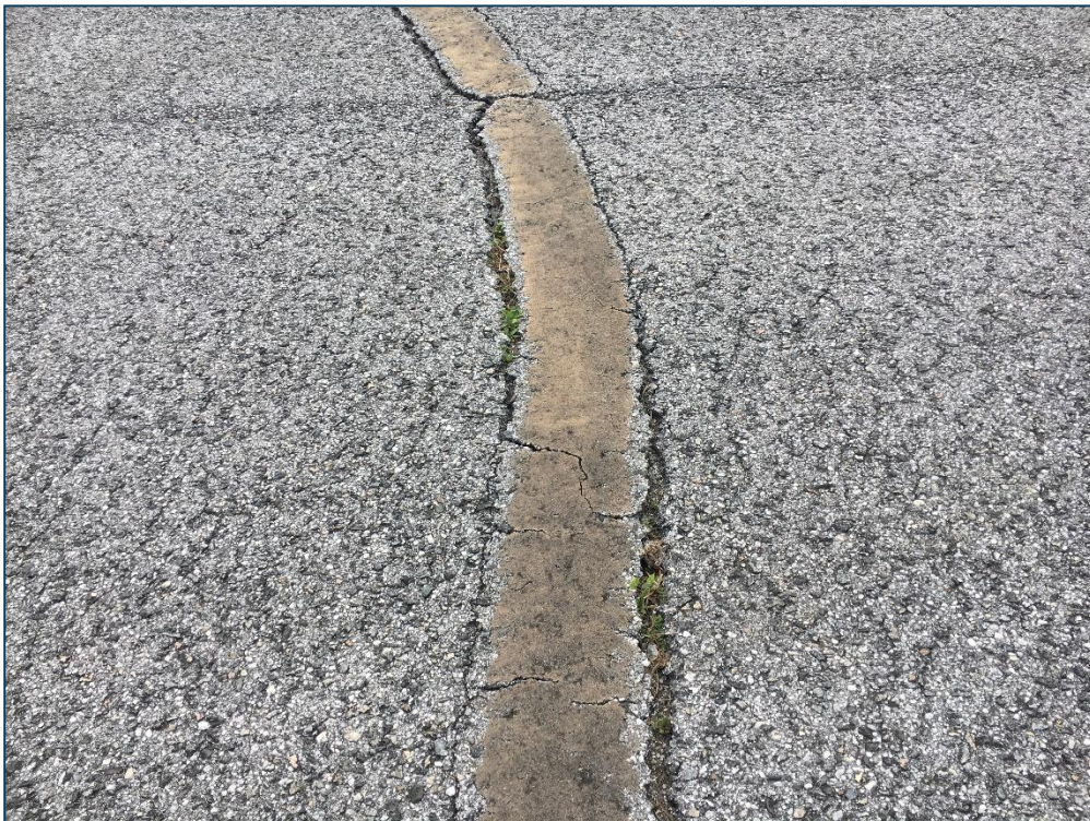
Taxilane to T-Hang NW, Section 4115, Sample Unit 101 – Low and Medium Severity (48) Longitudinal and Transverse Cracking, Low Severity (52) Raveling, Medium Severity (52) Raveling.
