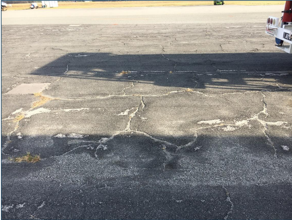
Apron NW, Section 4110, Sample Unit 100 – Medium Severity (43) Block Cracking and Low and Medium Severity (48) Longitudinal and Transverse Cracking, Low Severity (45) Depression, Low Severity (52) Raveling
