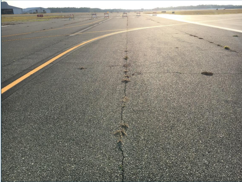
Runway 5-23, Section 6209, Sample Unit 160 – Low and Medium Severity (48) Longitudinal and Transverse Cracking, Low Severity (56) Swelling, Low Severity (57) Weathering
