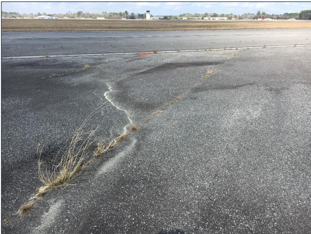
Taxiway D, Section 410, Sample Unit 201 – Low and Medium Severity (48) Longitudinal and Transverse Cracking, Low Severity (52) Raveling
