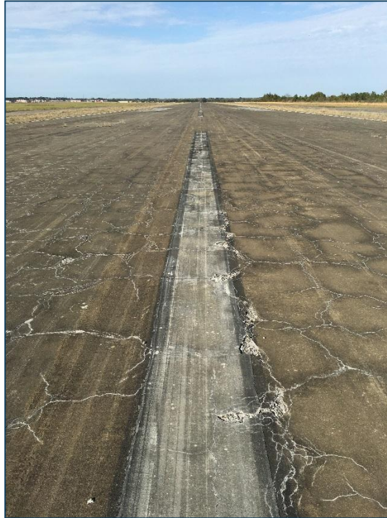
Runway 8-26, Section 6105, Sample Unit 315 – Low Severity (43) Block Cracking, Medium Severity (43) Block Cracking, Low Severity (52) Raveling, High Severity (52) Raveling
