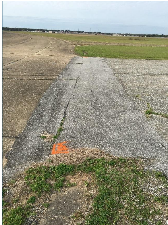
Taxiway F, Section 305, Sample Unit 104 – Medium Severity (43) Block Cracking, Medium Severity (50) Patching, Medium Severity (52) Raveling
