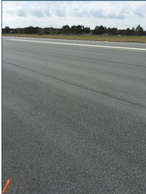
Runway 18-36, Section 6205, Sample Unit 135 – No Distress
