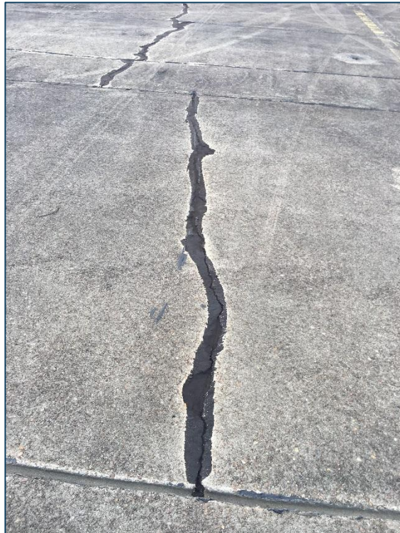
Apron, Section 4105, Sample Unit 326 – Low Severity (63) Longitudinal, Transverse, and Diagonal Cracking, Medium Severity (65) Joint Seal Damage
