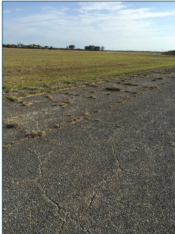
Taxiway G, Section 105, Sample Unit 107 – Medium Severity (43) Block Cracking, Medium Severity (52) Raveling, High Severity (52) Raveling
