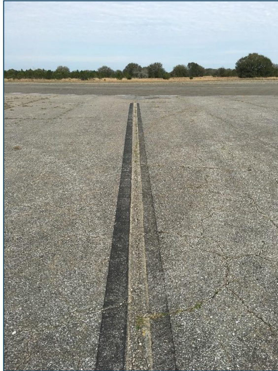
Taxiway F, Section 305, Sample Unit 100 – Medium Severity (43) Block Cracking, Medium Severity (52) Raveling, High Severity (52) Raveling
