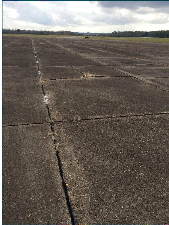
Apron, Section 4105, Sample Unit 246 – Low Severity (63) Longitudinal, Transverse, and Diagonal Cracking, Medium Severity (65) Joint Seal Damage
