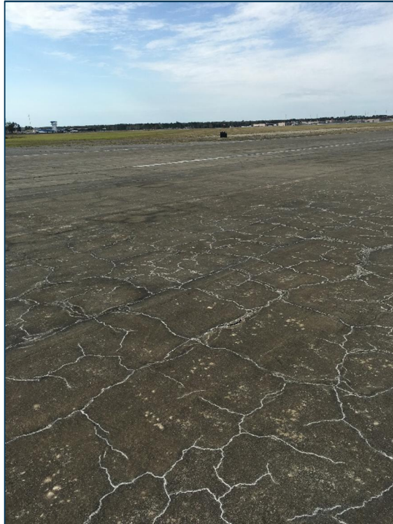
Runway 8-26, Section 6105, Sample Unit 359 – Low Severity (43) Block Cracking, Medium Severity (43) Block Cracking, Low Severity (52) Raveling, High Severity (52) Raveling
