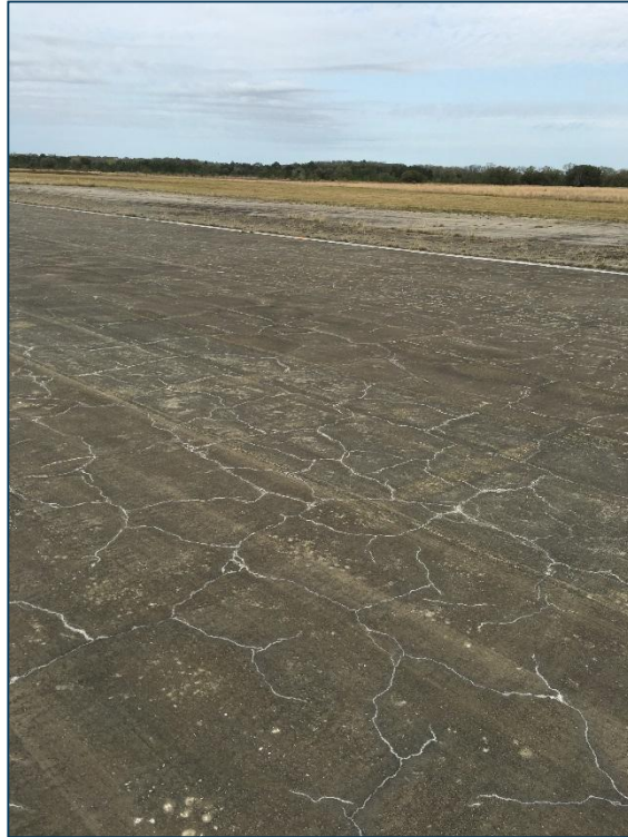
Runway 8-26, Section 6105, Sample Unit 388 – Low Severity (43) Block Cracking, Medium Severity (43) Block Cracking, Low Severity (52) Raveling
