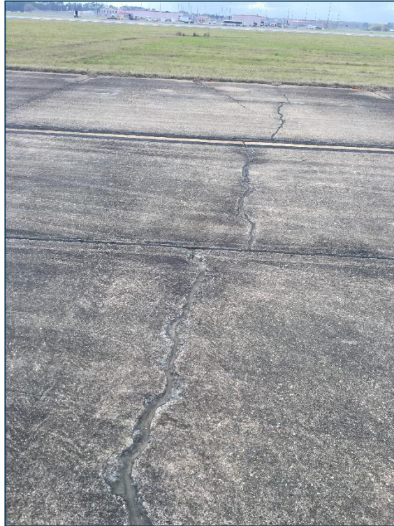
Taxiway Parallel, Section 150, Sample Unit 154 – Low Severity (63) Longitudinal, Transverse, and Diagonal Cracking, Medium Severity (65) Joint Seal Damage
