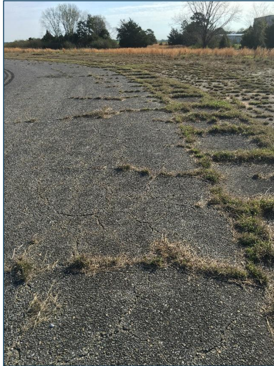
Taxiway G, Section 105, Sample Unit 105 – Medium Severity (43) Block Cracking, Medium Severity (52) Raveling, High Severity (52) Raveling
