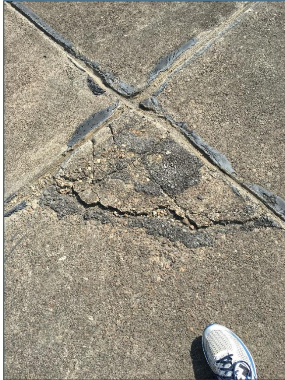
Apron, Section 4105, Sample Unit 711 – Medium Severity (65) Joint Seal Damage, Medium Severity (75) Corner Spalling
