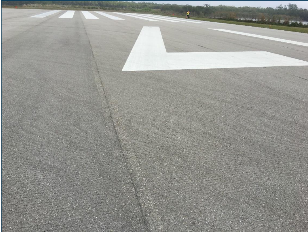
Runway 17-35, Section 6105, Sample Unit 194 – Low Severity (57) Weathering
