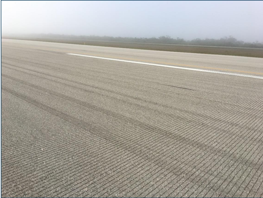
Runway 17-35, Section 6105, Sample Unit 146 – Low Severity (57) Weathering
