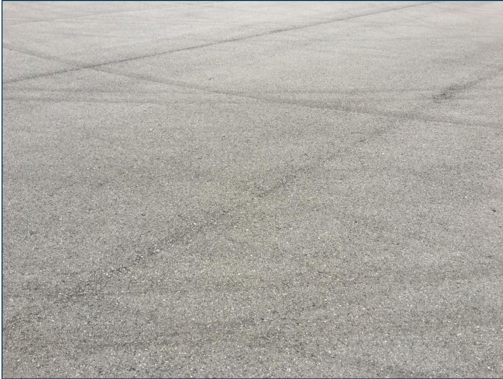
Apron N, Section 4205, Sample Unit 100 – Low Severity (57) Weathering
