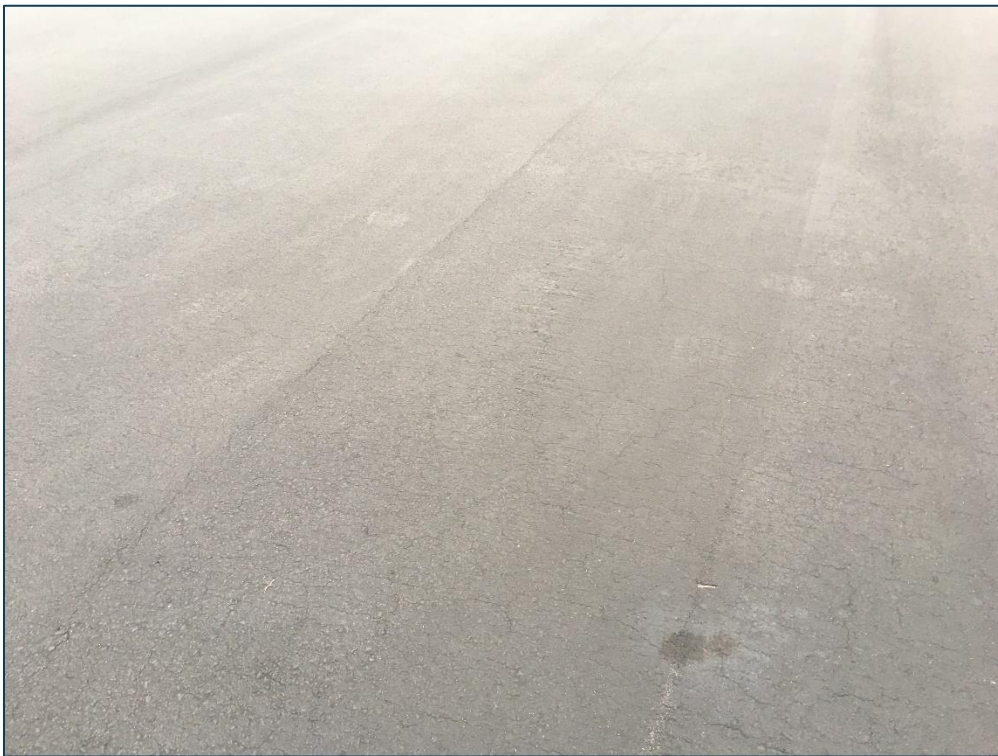
Apron NW, Section 4120, Sample Unit 104 – Low Severity (48) Longitudinal and Transverse Cracking, Low Severity (57) Weathering
