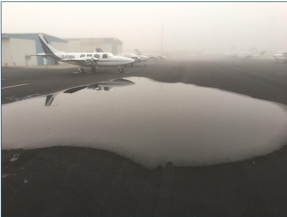
Apron NW, Section 4120, Sample Unit 155 (Not Inspected) – Medium Severity (45) Depression
