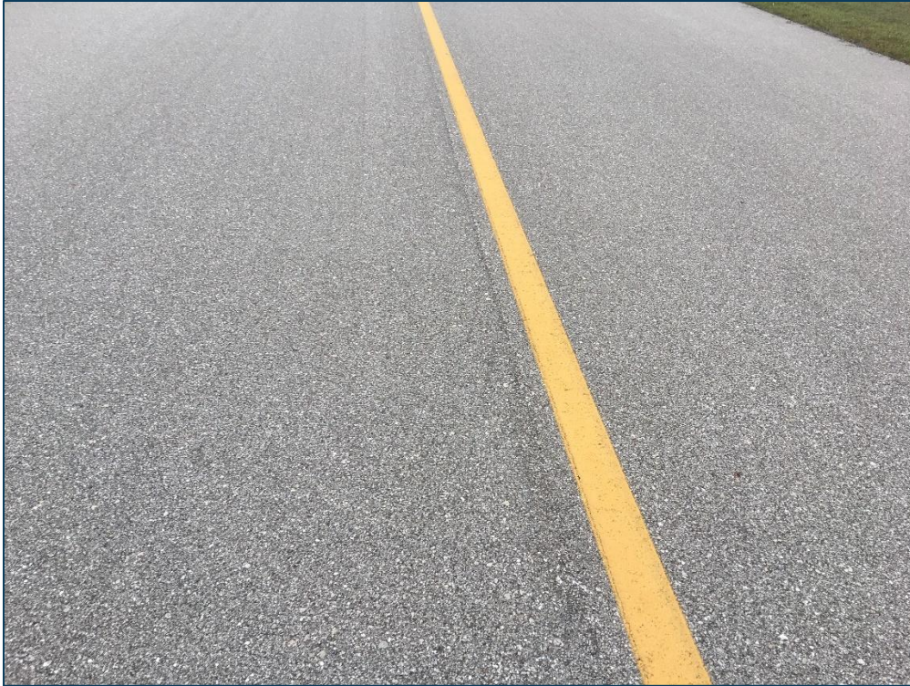
Taxiway A, Section 110, Sample Unit 107 – Low Severity (57) Weathering
