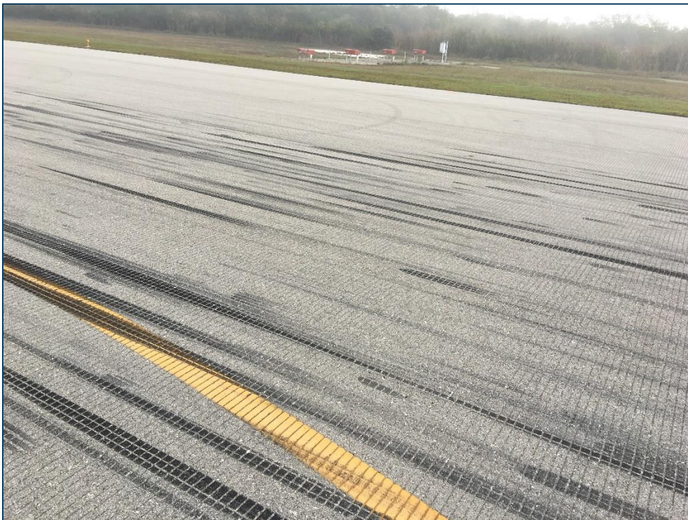
Runway 17-35, Section 6105, Sample Unit 186 – Low Severity (57) Weathering
