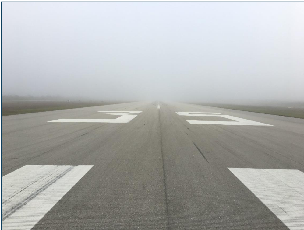
Runway 17-35, Section 6105, Sample Unit 103 – Low Severity (57) Weathering
