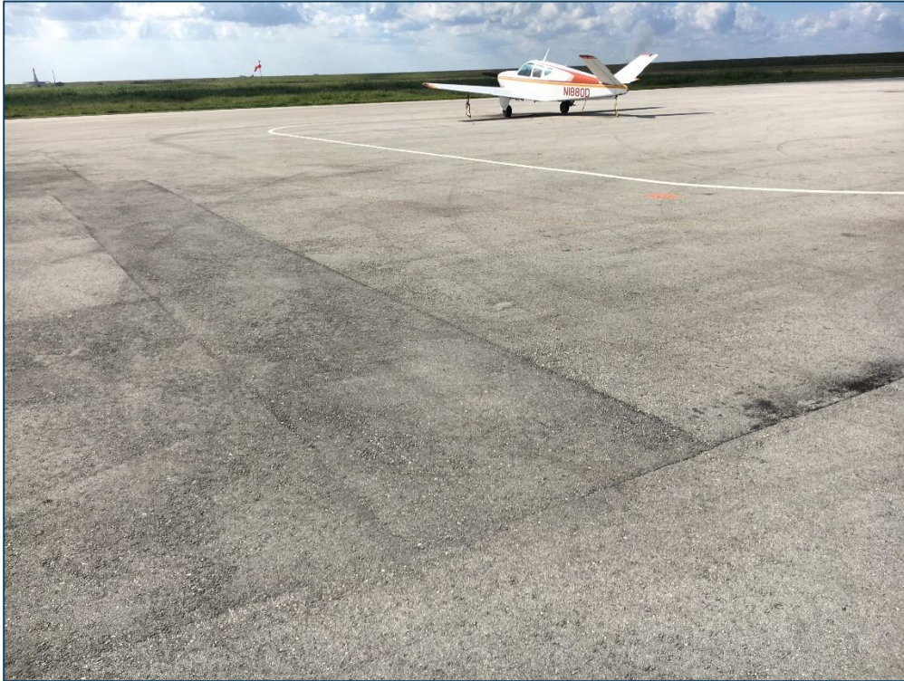
Apron, Section 4105, Sample Unit 400 – Low Severity (48) Longitudinal and Transverse Cracking, Low Severity (50) Patching, Low Severity (57) Weathering
