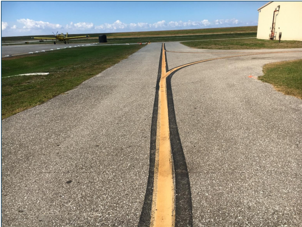
T-Hanger Taxiway, Section 4205, Sample Unit 100 – Low Severity (48) Longitudinal and Transverse Cracking, Low Severity (52) Raveling, Low Severity (57) Weathering
