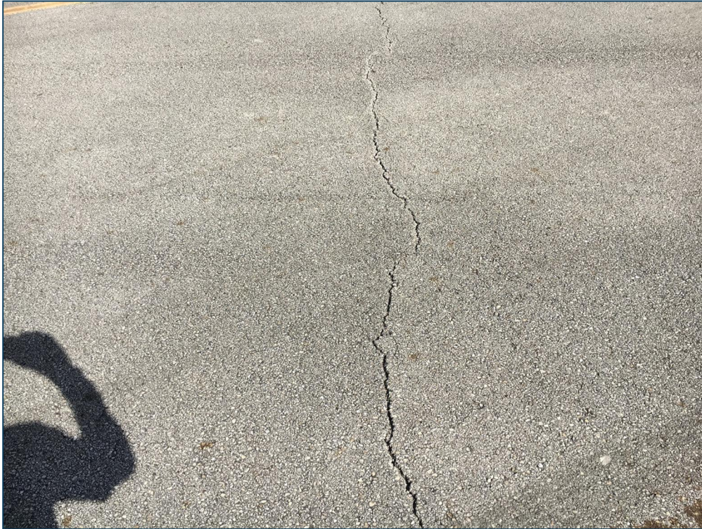
Taxiway D, Section 110, Sample Unit 100 – Low and Medium Severity (48) Longitudinal and Transverse Cracking, Low Severity (52) Raveling, Low Severity (57) Weathering
