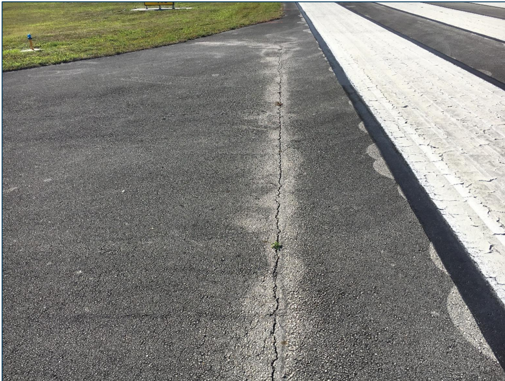
Taxiway A5, Section 115, Sample Unit 100 – Low and Medium Severity (48) Longitudinal and Transverse Cracking, Low Severity (52) Raveling, Low Severity (57) Weathering
