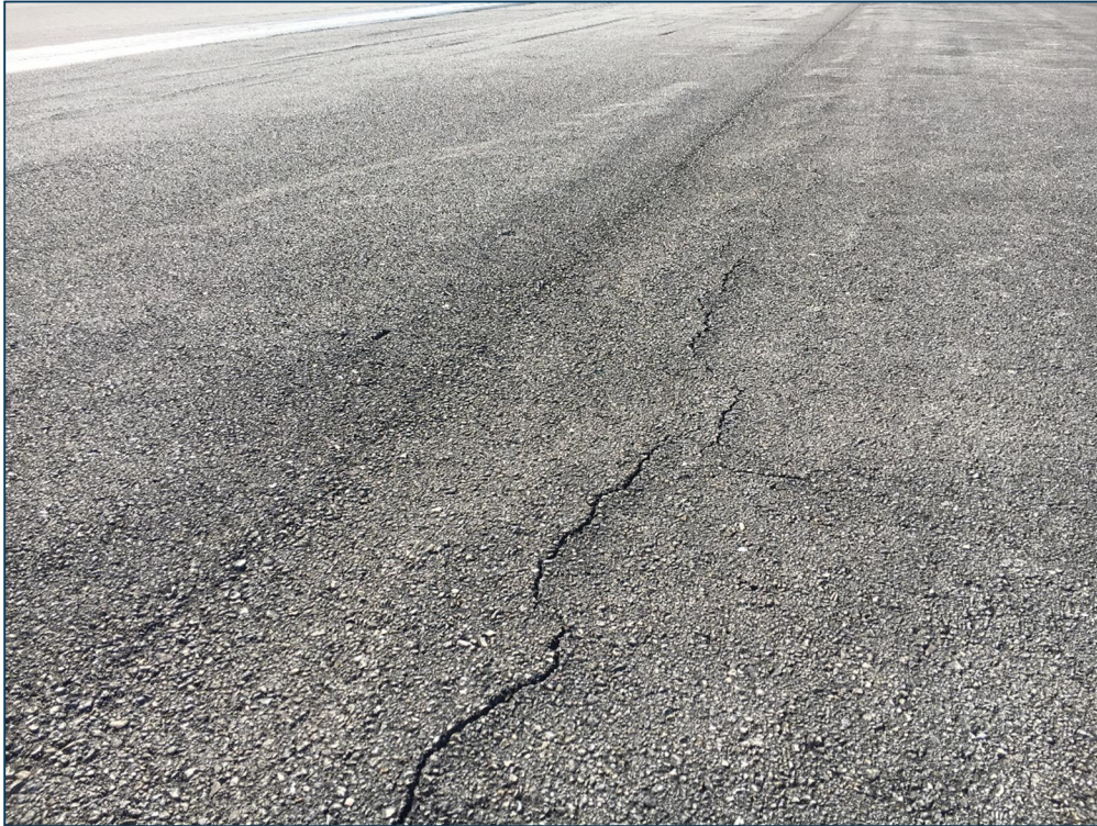
Runway 17-35, Section 6105, Sample Unit 109 – Low and Medium Severity (48) Longitudinal and Transverse Cracking, Low Severity (52) Raveling, Low Severity (56) Swelling, Low Severity (57) Weathering
