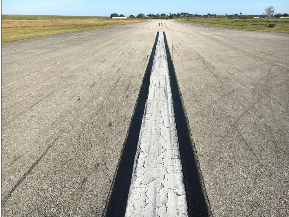
Runway 17-35, Section 6110, Sample Unit 164 – Low and Medium Severity (48) Longitudinal and Transverse Cracking, Low Severity (52) Raveling, Low Severity (57) Weathering
