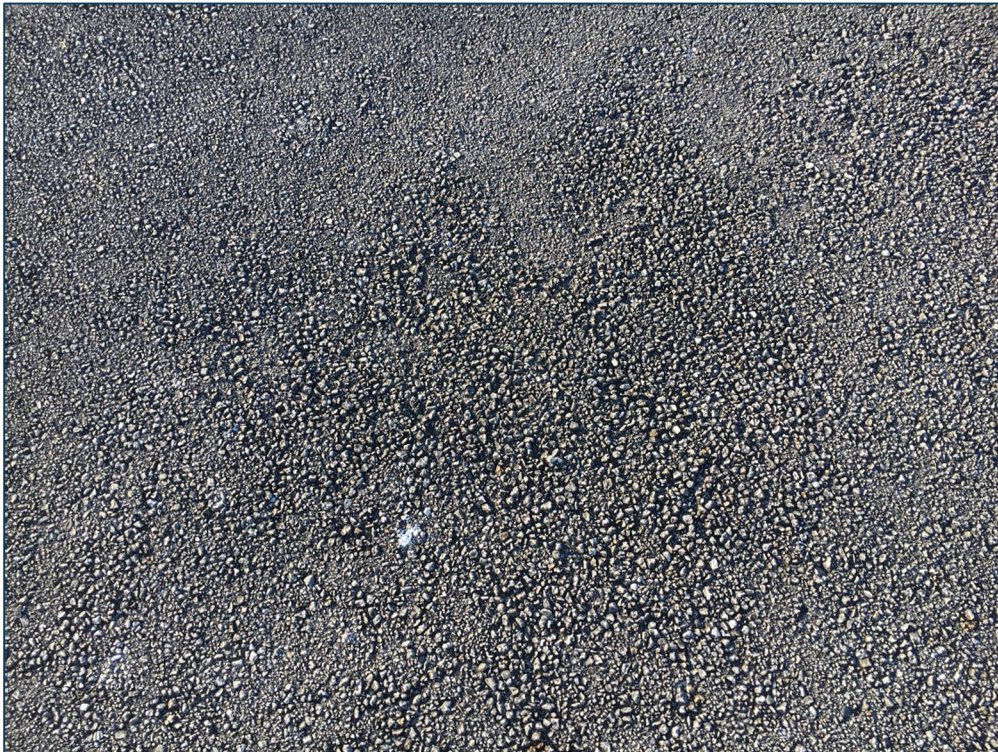
Taxiway A2, Section 125, Sample Unit 100 – Low Severity (52) Raveling, Low Severity (57) Weathering
