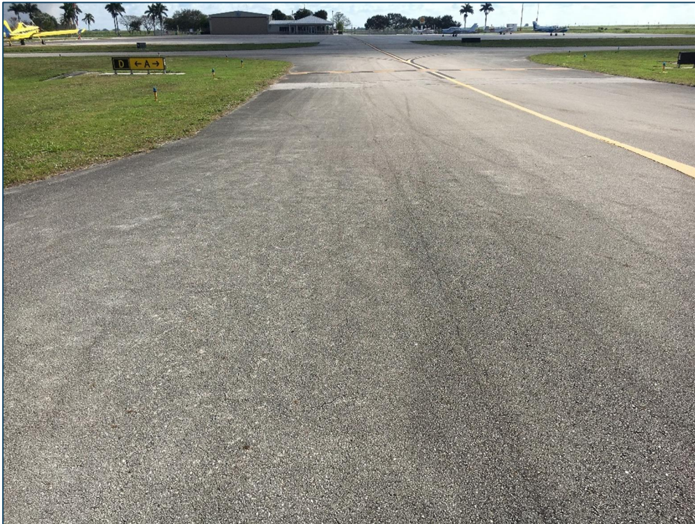
Taxiway D, Section 110, Sample Unit 100 – Low Severity (48) Longitudinal and Transverse Cracking, Low Severity (52) Raveling, Low Severity (56) Swelling, Low Severity (57) Weathering
