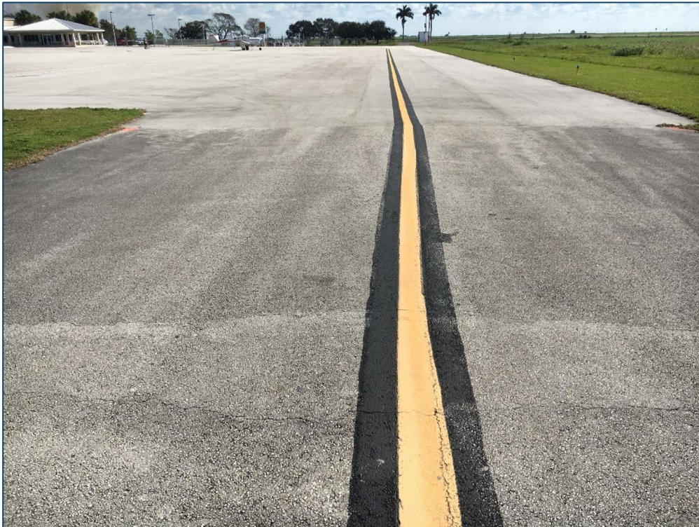
Taxiway A3, Section 130, Sample Unit 104 – Low Severity (48) Longitudinal and Transverse Cracking, Low Severity (57) Weathering
