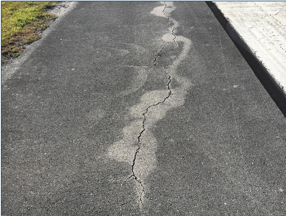
Runway 17-35, Section 6105, Sample Unit 105 – Low and Medium Severity (48) Longitudinal and Transverse Cracking, Low Severity (52) Raveling, Low Severity (56) Swelling, Low Severity (57) Weathering
