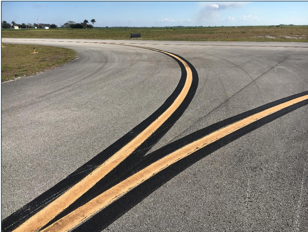
Taxiway A4, Section 120, Sample Unit 101 – Low Severity (48) Longitudinal and Transverse Cracking, Low Severity (52) Raveling, Low Severity (57) Weathering
