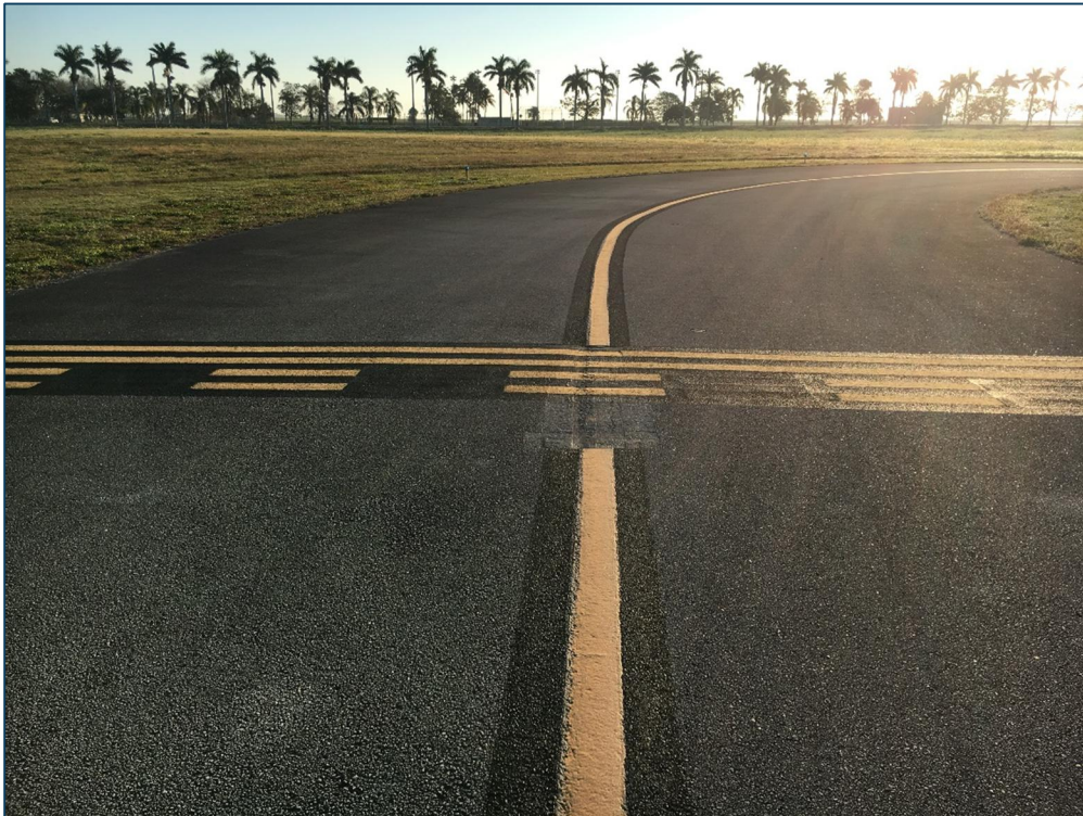
Taxiway A, Section 105, Sample Unit 100 – Low Severity (48) Longitudinal and Transverse Cracking, Low Severity (52) Raveling, Low Severity (57) Weathering
