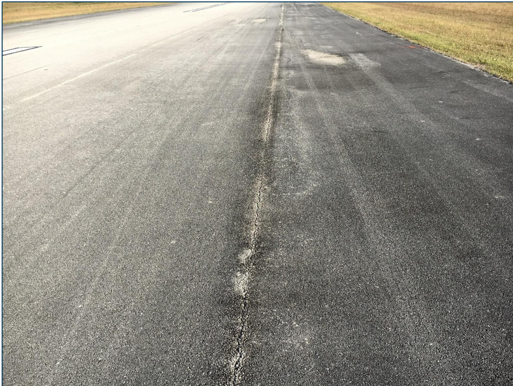
Runway 17-35, Section 6110, Sample Unit 145 – Low and Medium Severity (48) Longitudinal and Transverse Cracking, Low Severity (52) Raveling, Low Severity (56) Swelling, Low Severity (57) Weathering
