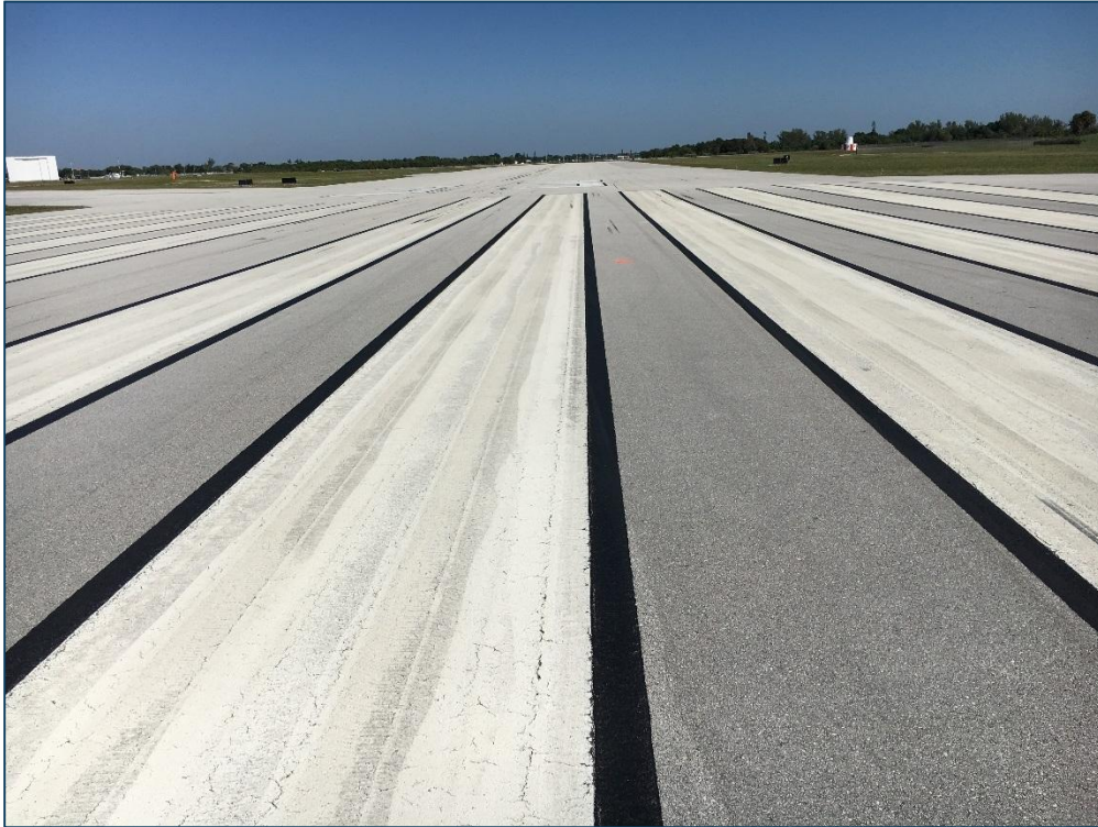
Runway 15-33, Section 6305, Sample Unit 303 - Low Severity (57) Weathering
