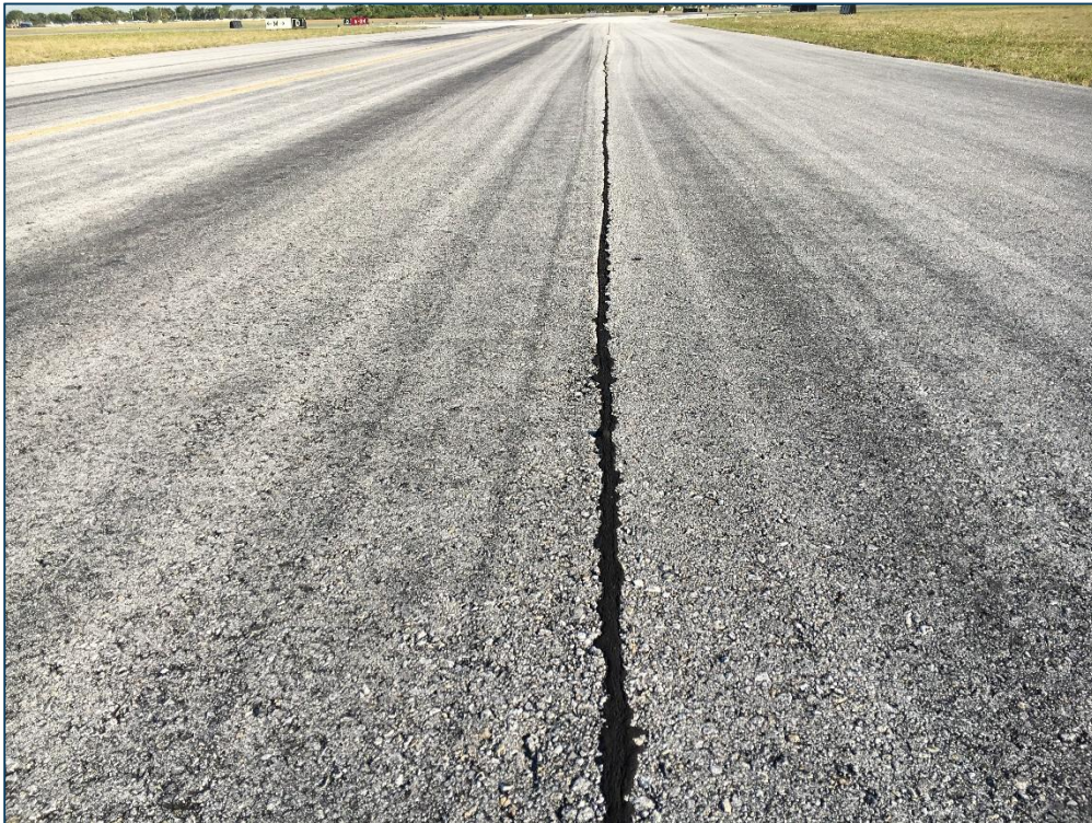
Taxiway D, Section 405, Sample Unit 420 - Low Severity (48) Longitudinal and Transverse Cracking, Low Severity (52) Raveling, Low Severity (57) Weathering
