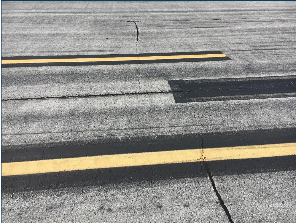
Runway 6-24, Section 6205, Sample Unit 306 - Low Severity (48) Longitudinal and Transverse Cracking, Low Severity (52) Raveling, Low Severity (57) Weathering
