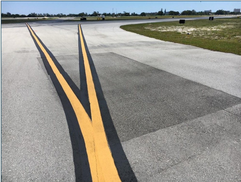
Taxiway M, Section 1306, Sample Unit 211 - Low Severity (48) Longitudinal and Transverse Cracking, Low Severity (50) Patching, Low Severity (52) Raveling, Low Severity (57) Weathering
