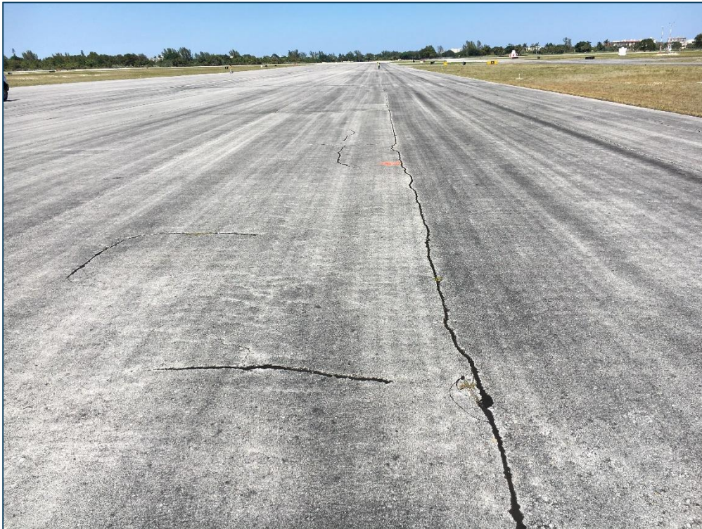
Runway 6-24, Section 6205, Sample Unit 323 - Low Severity (48) Longitudinal and Transverse Cracking, Low Severity (52) Raveling, Low Severity (57) Weathering
