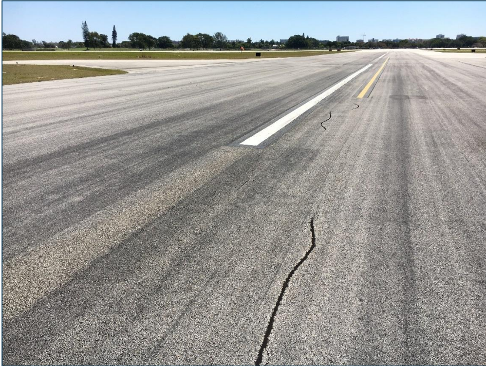
Runway 10-28, Section 6105, Sample Unit 141 - Low Severity (48) Longitudinal and Transverse Cracking, Low Severity (52) Raveling, Low Severity (56) Swelling
