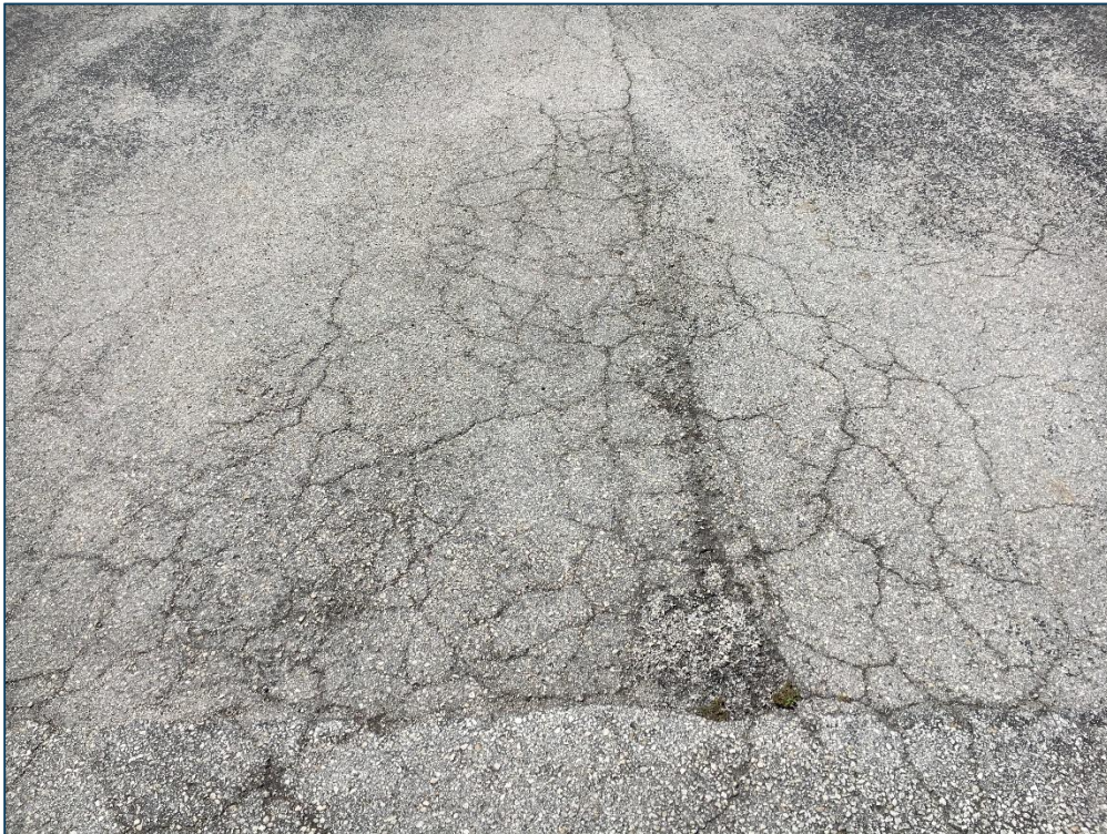
Taxilane To Hangars, Section 4315, Sample Unit 700 - Low Severity (41) Alligator Cracking, Low Severity (45) Depression, Low Severity (52) Raveling
