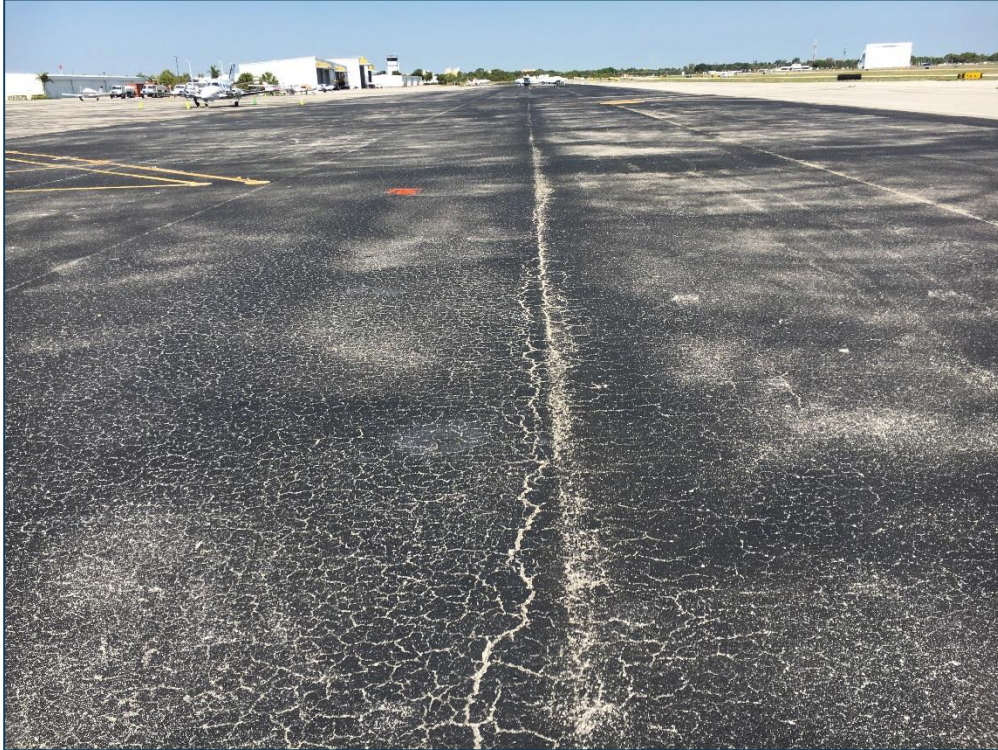
South Apron, Section 4105, Sample Unit 329 - Low Severity (43) Block Cracking, Low Severity (48) Longitudinal and Transverse Cracking, Low Severity (52) Raveling
