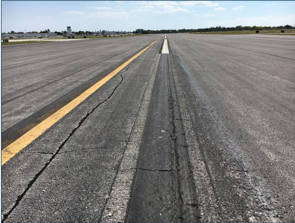
Runway 6-24, Section 6205, Sample Unit 346 - Low Severity (48) Longitudinal and Transverse Cracking, Low Severity (50) Patching, Low Severity (52) Raveling, Low Severity (57) Weathering
