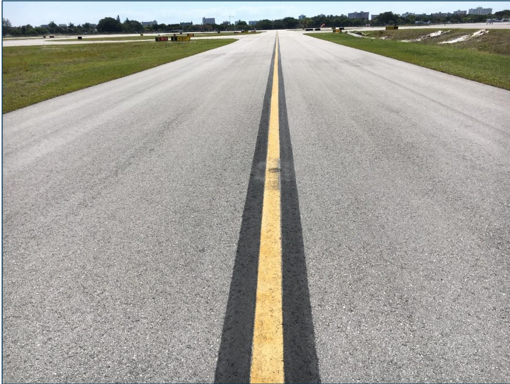
Taxiway K, Section 1110, Sample Unit 121 - Low Severity (57) Weathering
