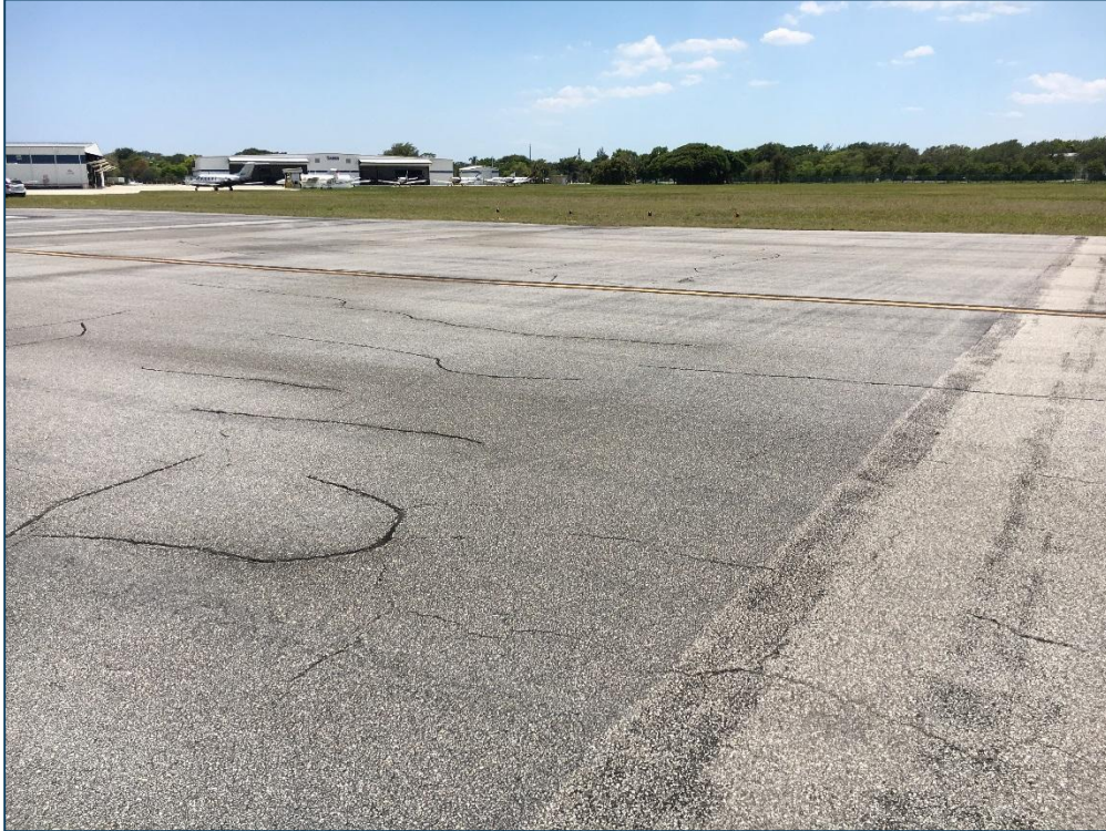
Taxiway A, Section 115, Sample Unit 106 - Low Severity (43) Block Cracking, Low Severity (48) Longitudinal and Transverse Cracking, Low Severity (52) Raveling, Low Severity (57) Weathering
