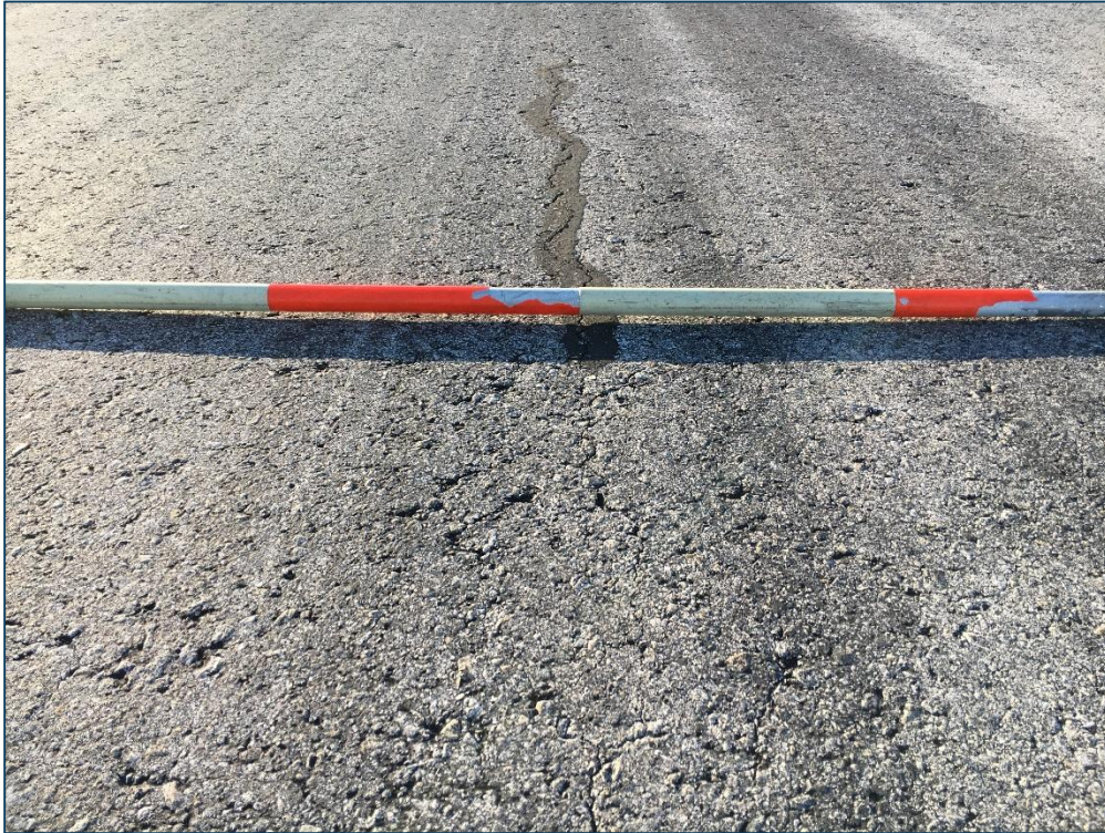
Taxiway D, Section 405, Sample Unit 413 - Low Severity (48) Longitudinal and Transverse Cracking, Low Severity (52) Raveling, Low Severity (53) Rutting, Low Severity (57) Weathering
