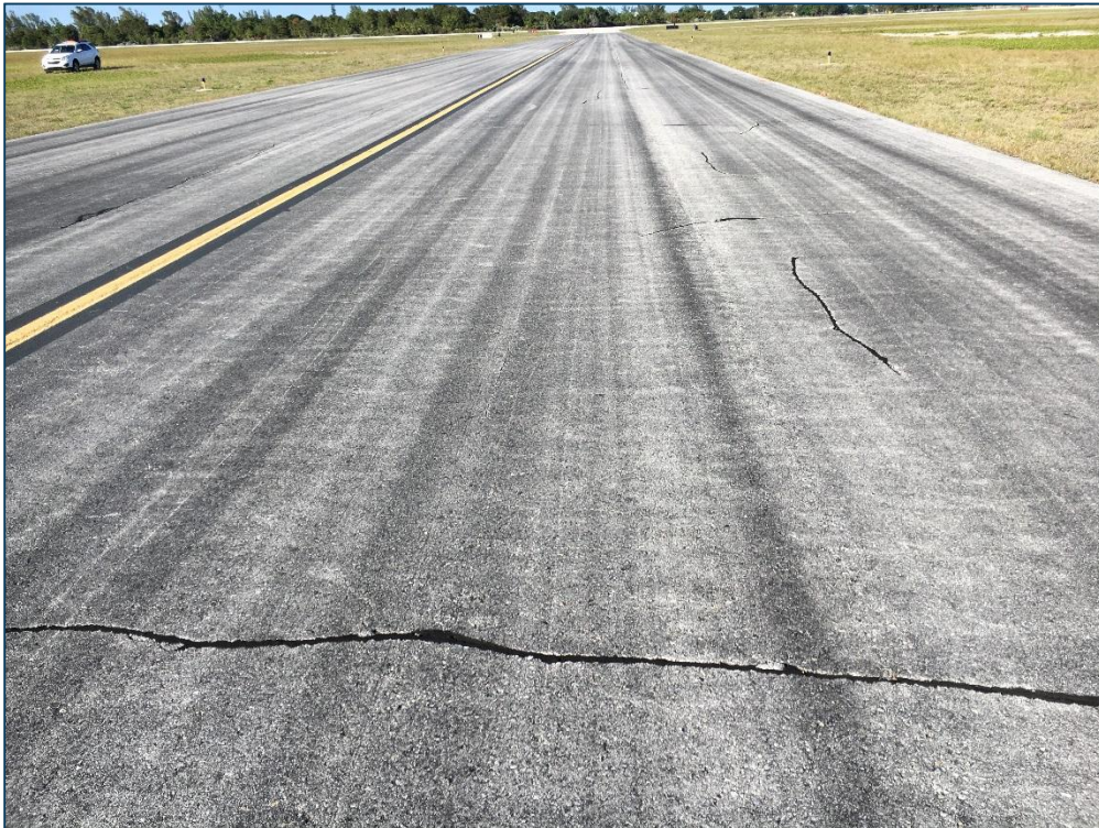
Taxiway F, Section 610, Sample Unit 625 - Low Severity (48) Longitudinal and Transverse Cracking, Low Severity (52) Raveling, Low Severity (57) Weathering
