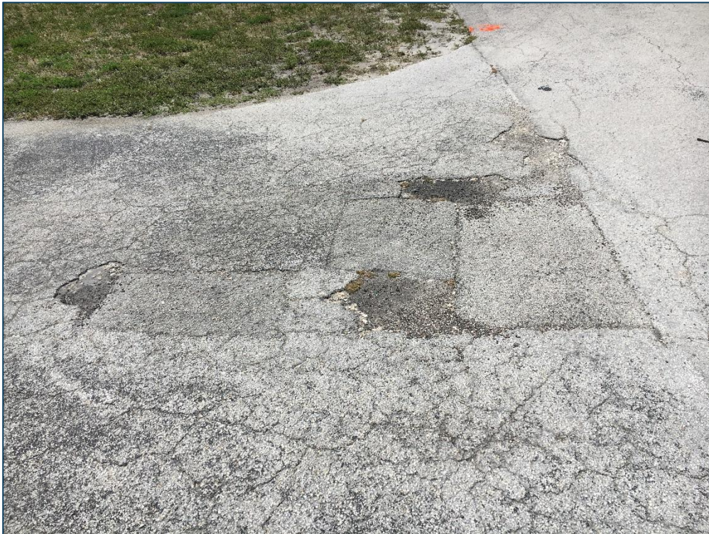
Taxilane To Hangars, Section 4305, Sample Unit 601 - Low Severity (43) Block Cracking, Low Severity (50) Patching, High Severity (50) Patching, Medium Severity (52) Raveling, High Severity (52) Raveling
