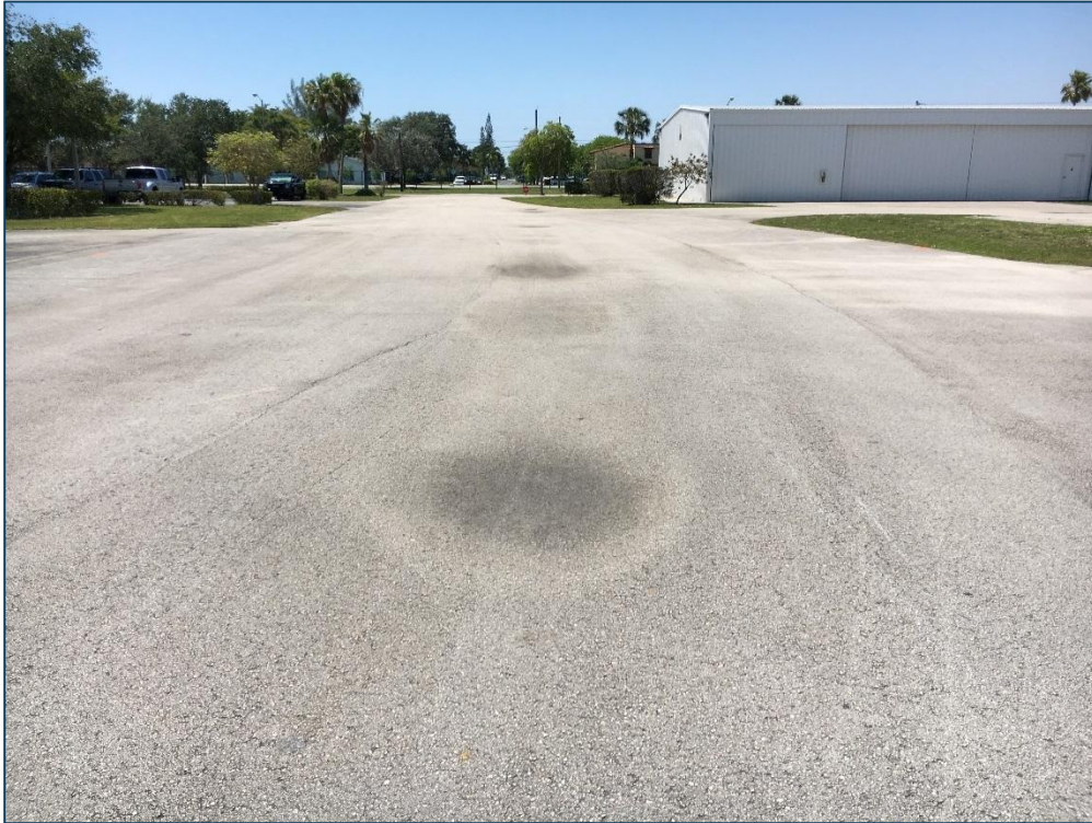
Taxilane To Hangars, Section 4315, Sample Unit 602 - Medium Severity (45) Depression, Low Severity (48) Longitudinal and Transverse Cracking, Low Severity (52) Raveling, Low Severity (57) Weathering
