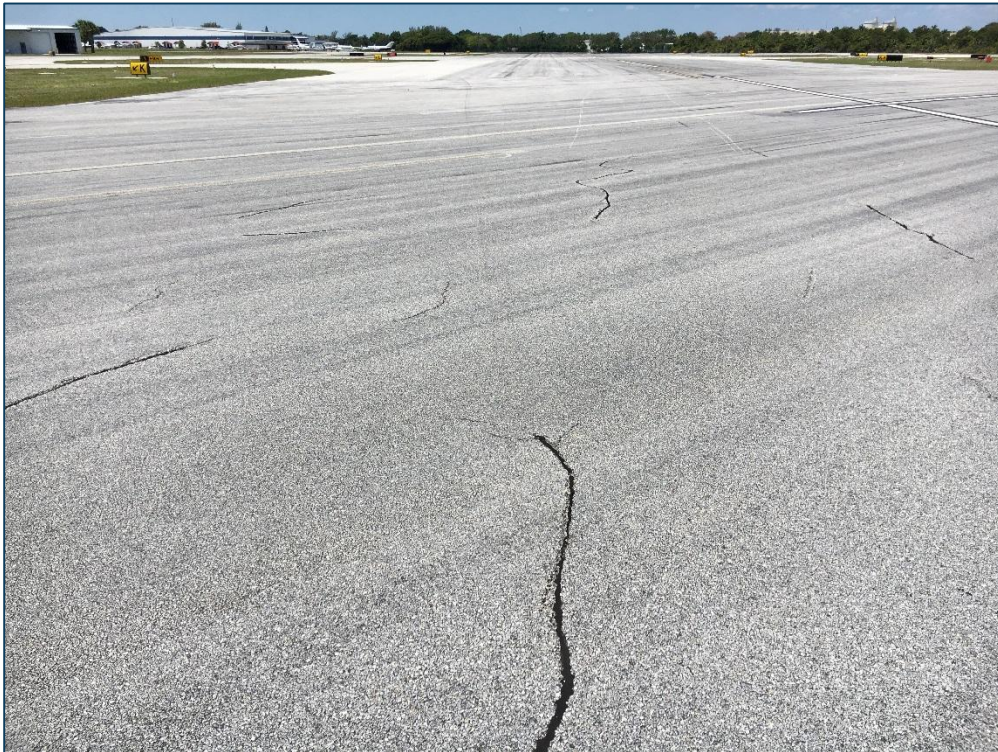
Runway 10-28, Section 6105, Sample Unit 117 - Low Severity (48) Longitudinal and Transverse Cracking, Low Severity (52) Raveling
