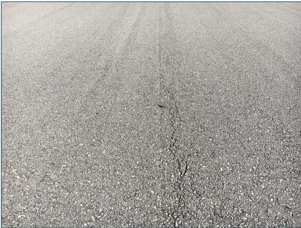
Runway 15-33, Section 6310, Sample Unit 112 - Low Severity (48) Longitudinal and Transverse Cracking, Low Severity (57) Weathering
