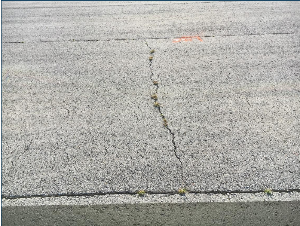
North Apron - Old RW, Section 4205, Sample Unit 321 - Low and Medium Severity (48) Longitudinal and Transverse Cracking, Low Severity (52) Raveling, Low Severity (57) Weathering
