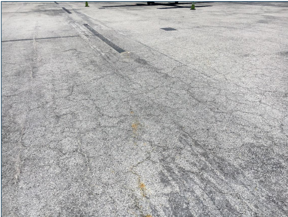
South Apron, Section 4125, Sample Unit 201 - Low Severity (43) Block Cracking, Low Severity (52) Raveling, Medium Severity (52) Raveling
