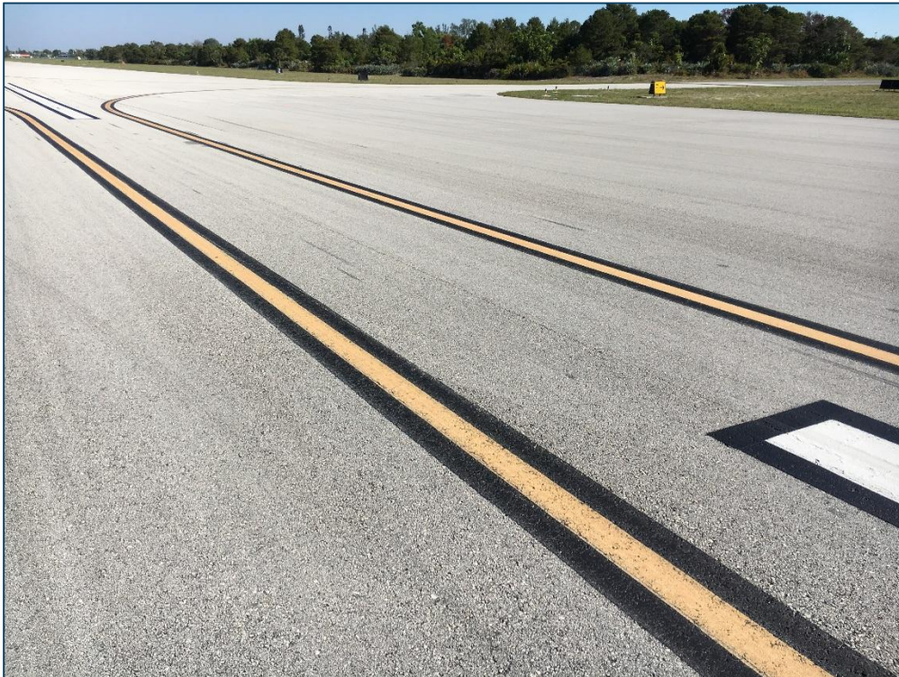
Runway 15-33, Section 6305, Sample Unit 325 - Low Severity (57) Weathering
