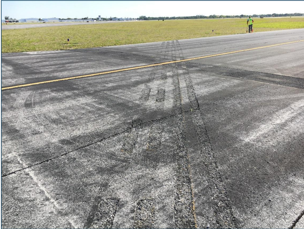
Taxiway F, Section 610, Sample Unit 601 - Medium Severity (48) Longitudinal and Transverse Cracking, Low Severity (50) Patching, Low Severity (52) Raveling, Low Severity (57) Weathering
