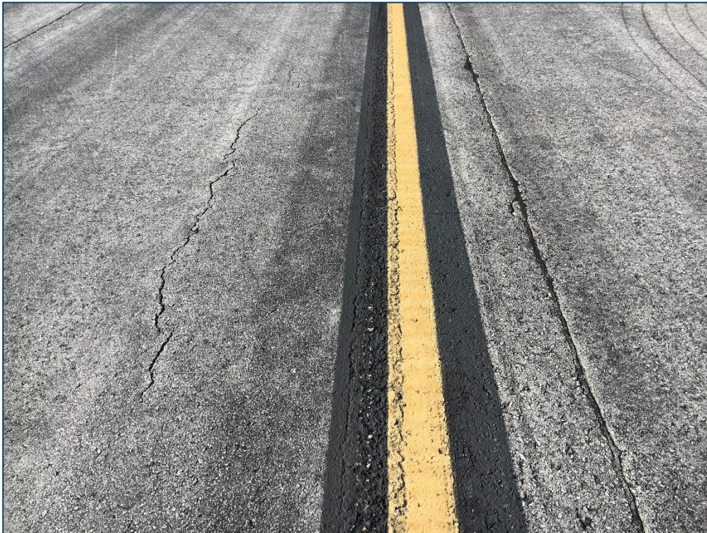
Taxiway B, Section 210, Sample Unit 706 - Low Severity (48) Longitudinal and Transverse Cracking, Low Severity (52) Raveling, Low Severity (57) Weathering
