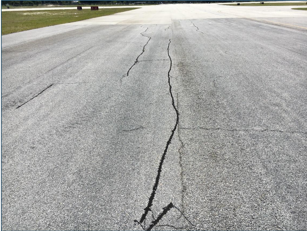
Runway 10-28, Section 6105, Sample Unit 152 - Low Severity (48) Longitudinal and Transverse Cracking, Low Severity (52) Raveling, Medium Severity (52) Raveling, Low Severity (56) Swelling
