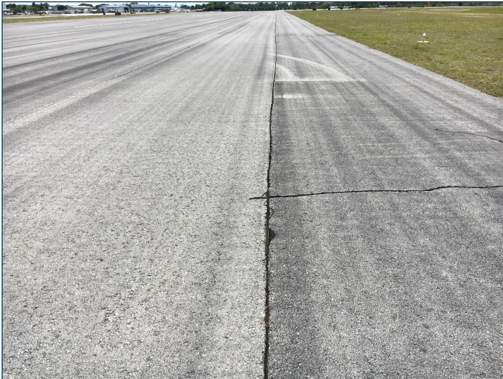
Runway 6-24, Section 6210, Sample Unit 132 - Low Severity (48) Longitudinal and Transverse Cracking, Low Severity (52) Raveling, Low Severity (57) Weathering
